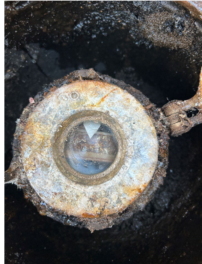
2: Bung-hole in tank with meter
