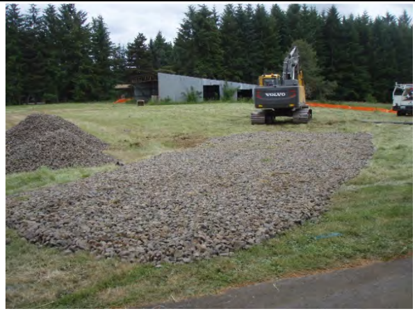
Installing construction entrance
