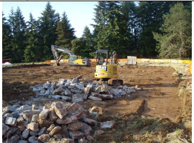
Excavation of concrete pad in Decision Unit 4
