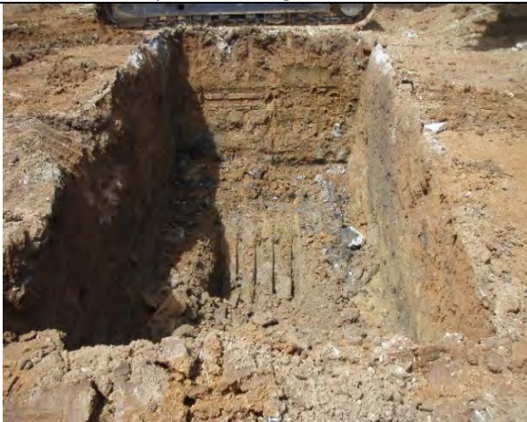
Excavation of vault
