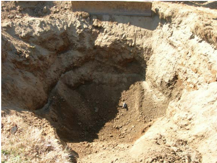
View into excavation, cat blade for scale.
