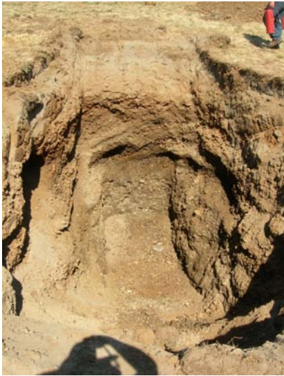
View into excavation at 13 feet depth.
