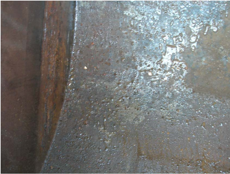
The interior of the tank was cleaned before it was removed.
