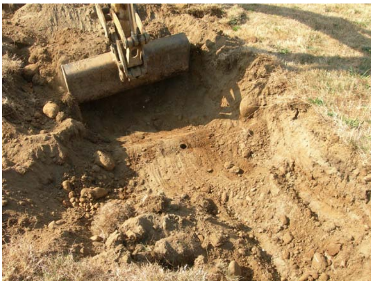
Exposing the tank.
