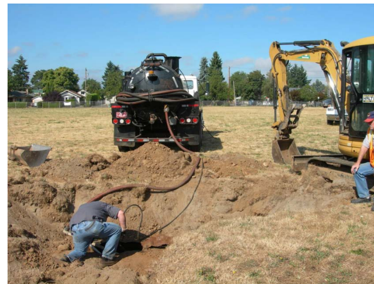
The tank was pumped and cleaned by ORRCO.
