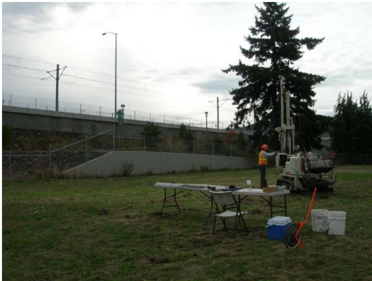
Push probe rig set up on delineation boring location.
