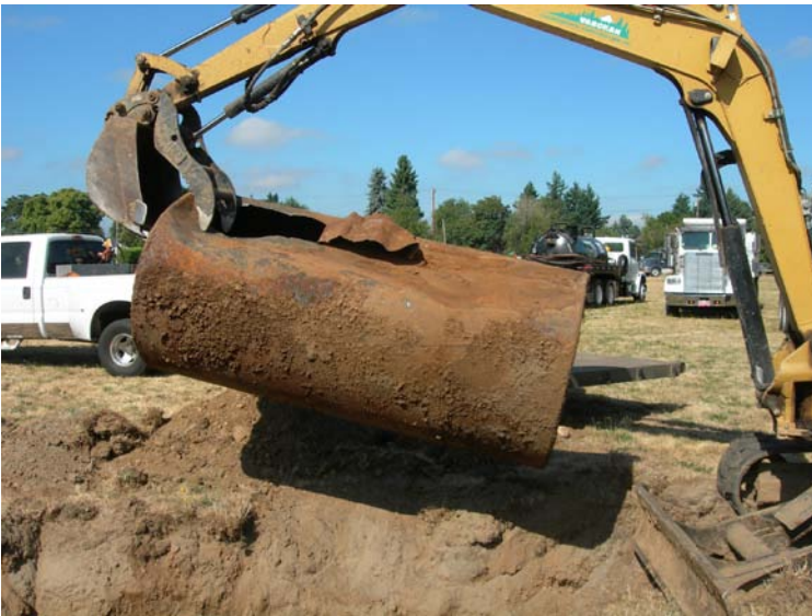
Removing the tank from the excavation.
