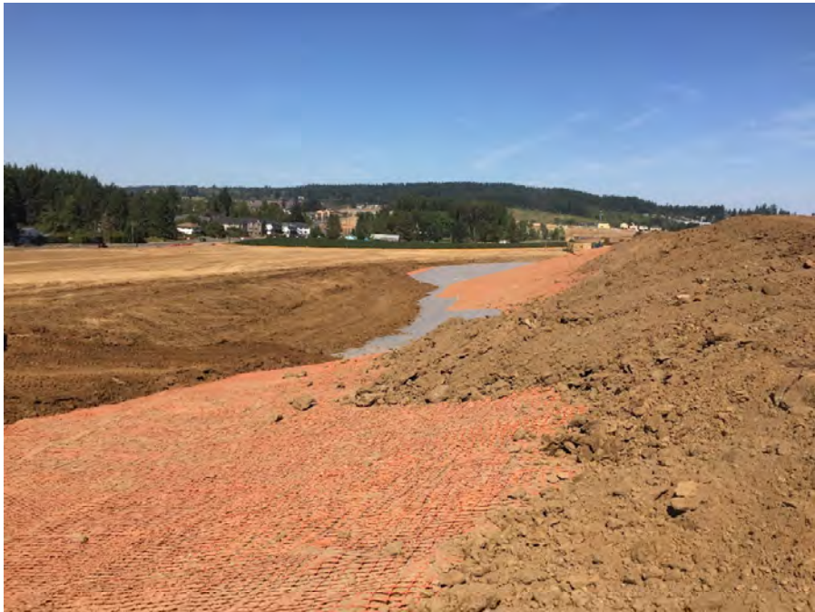
PLACING FILL ABOVE THE DEMARCATION LAYER OF THE PARK DISPOSAL CELL. PHOTOGRAPH TAKEN FACING NORTH.
