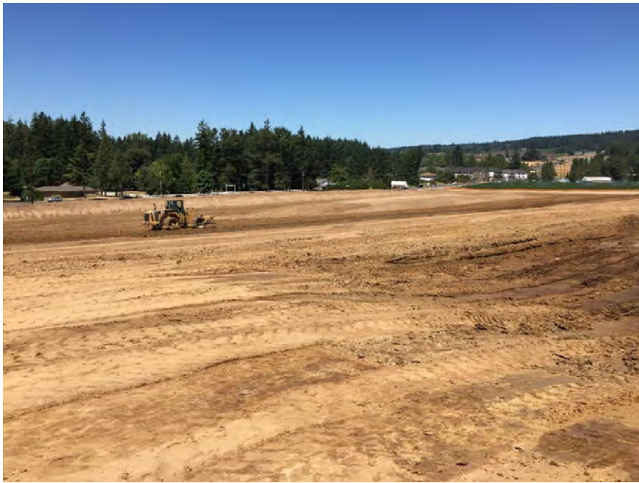
INITIAL GRADING OF THE WESTERN PORTION OF THE PROJECT SITE USING SCRAPPERS AND BULLDOZERS. PHOTOGRAPH TAKEN FACING WEST.
