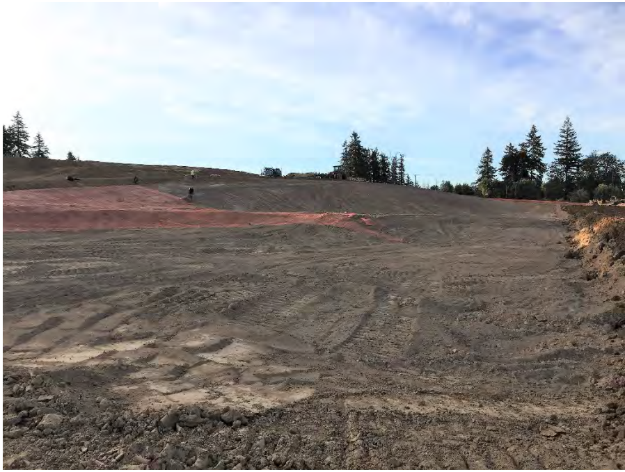
DEMARCATIION LAYER BEING INSTALLED ON THE SLOPES OF THE PARK DISPOSAL CELL. PHOTOGRAPH TAKEN FACING SOUTH.
