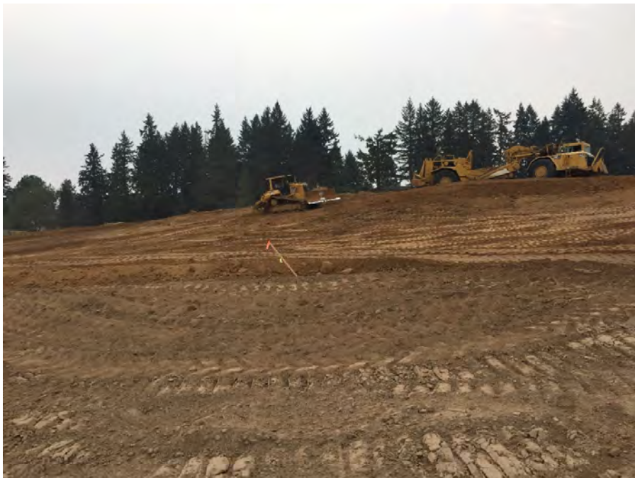
EXCAVATION OF THE PARK DISPOSAL CELL USING SCRAPPERS. PHOTOGRAPH TAKEN FACING SOUTHWEST.
