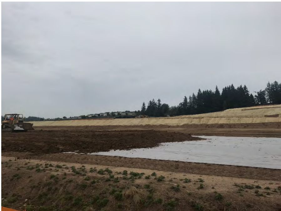
DEMARCATIION LAYER AT THE CONDOMINIUM DISPOSAL CELL. PHOTOGRAPH TAKEN EAST.
