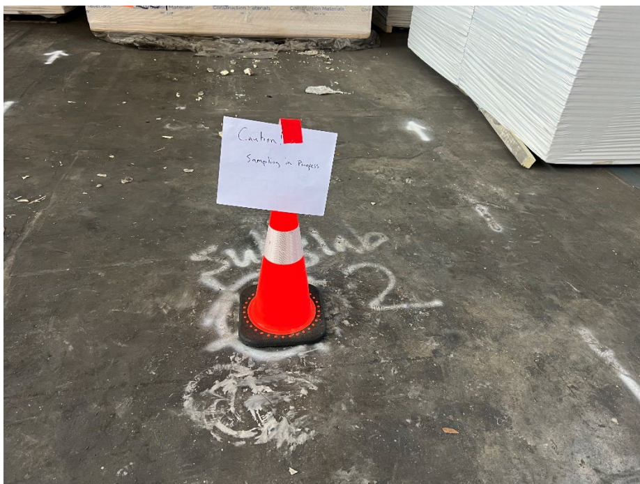
Photo 6. The passive samplers were collected after 14 days and the holes in the concrete slab were patched and sealed with hydraulic cement.
