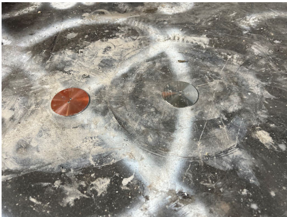
Photo 5. Waterloo membrane samplers installed for the collection of sub-slab samples SSV-2 and SSV-DUP.
