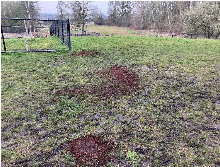
PHOTO I.D. 13: AREA OF SOIL CAP REPAIRS WITHIN THE LARGE DOG PARK IN DISPOSAL CELL #2 WHERE SMALL HOLES HAD BEEN OBSERVED. PHOTOGRAPH TAKEN FACING WEST.
