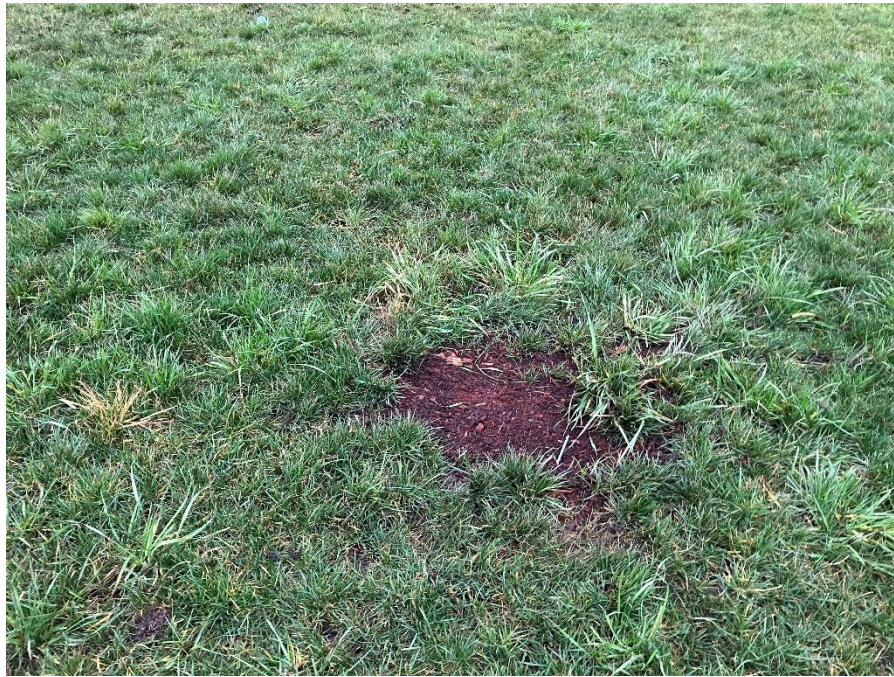
PHOTO I.D. 9: AREA OF SOIL CAP REPAIR WHERE A HOLE WAS OBSERVED WITHIN THE LARGE DOG PARK IN DISPOSAL CELL #2. PHOTOGRAPH TAKEN FACING WEST.
