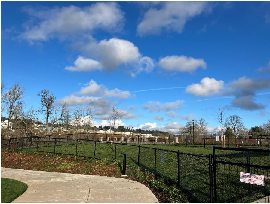
PHOTO I.D. 1: WEST PORTION OF DISPOSAL CELL #2. PHOTOGRAPH TAKEN FACING NORTHEAST.
