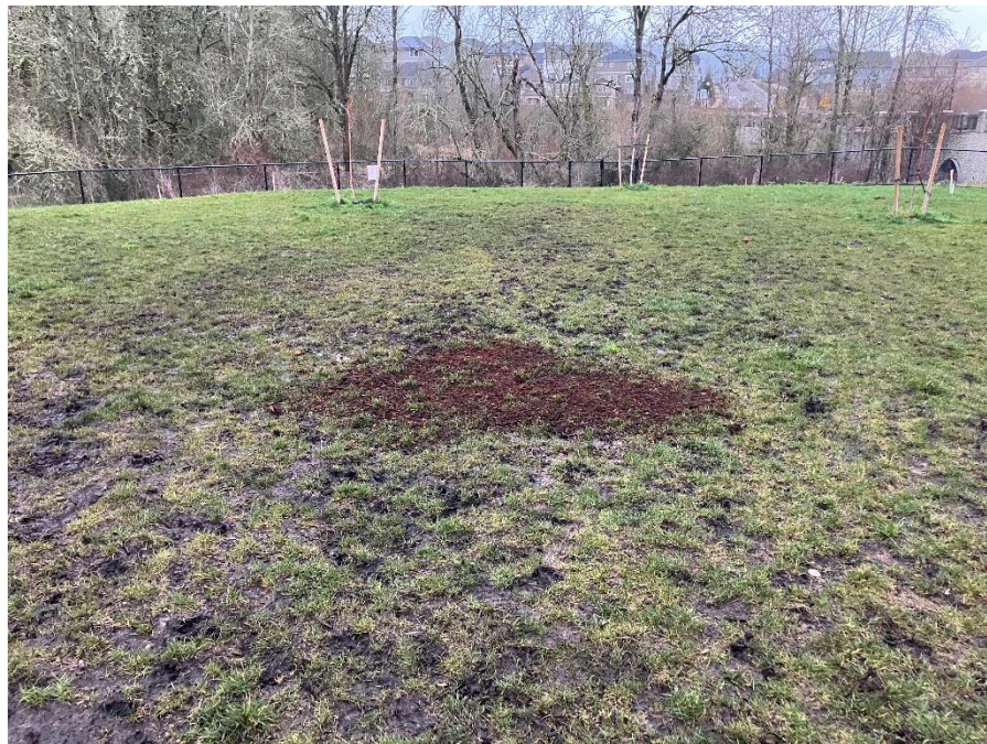
PHOTO I.D. 14: AREA OF SOIL CAP REPAIR WITHIN THE LARGE DOG PARK IN DISPOSAL CELL #2 WHERE A SMALL HOLE HAD BEEN OBSERVED. PHOTOGRAPH TAKEN FACING NORTH.
