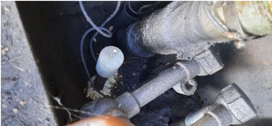
9: UDC with anode spike
