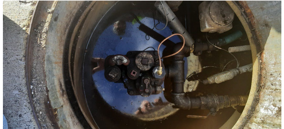
24: On road diesel sump with water present
