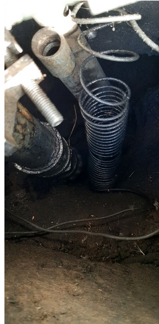
10: Direct bury UDC with spike anode
