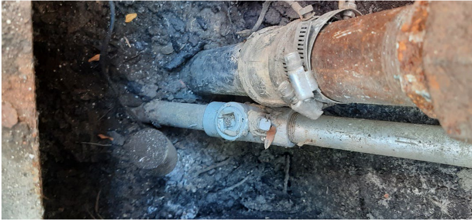
7: Direct bury UDC with anode spike
