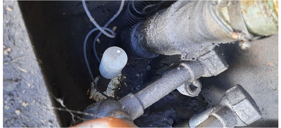
8: Direct bury UDC with anode spike
