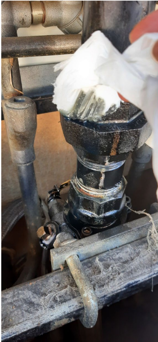
13: Pipe leak in UDC #1
