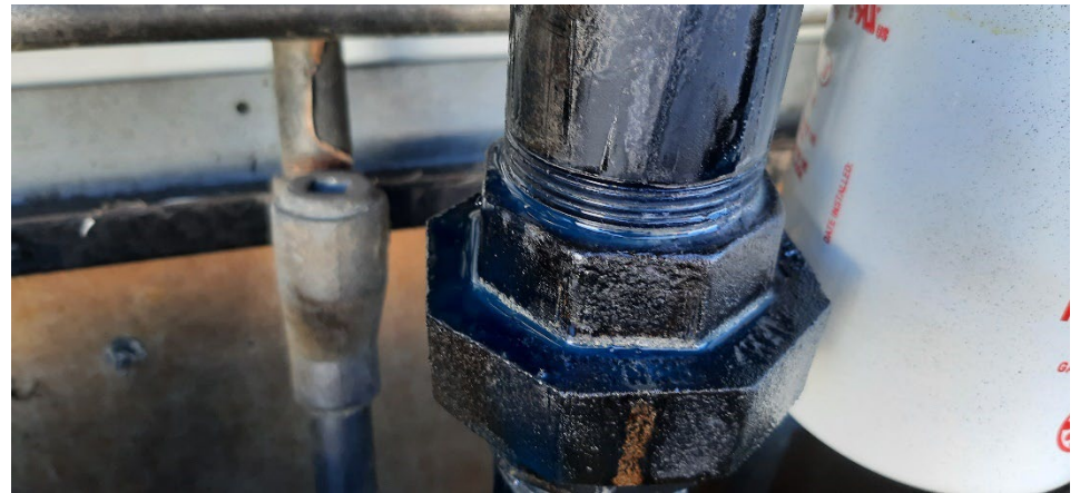
12: UDC #1 leaking supreme pipe
