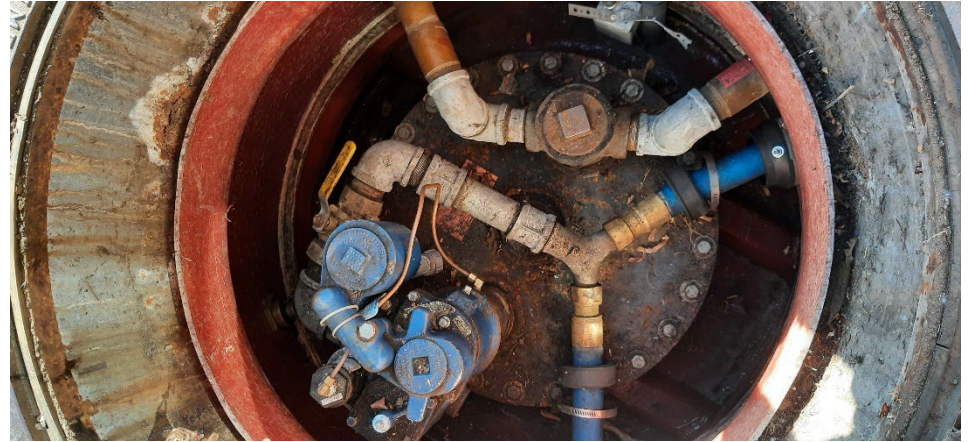
18: Unleaded sump with manifold of 20,000 gallon tanks
