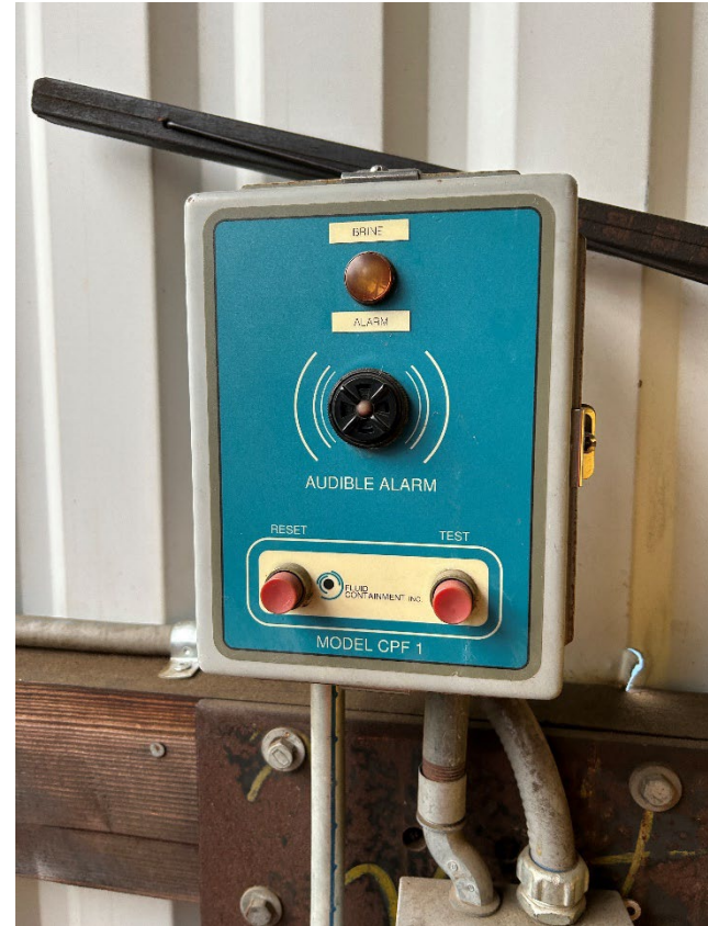
6: Alarm connect to the brine sensor
