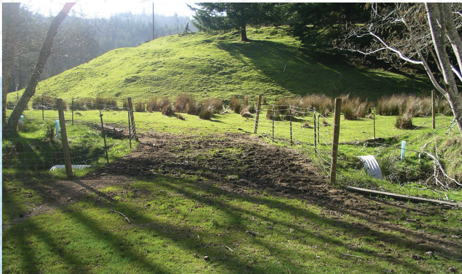
Livestock crossing with a fish passage culvert over Gallagher creek.
