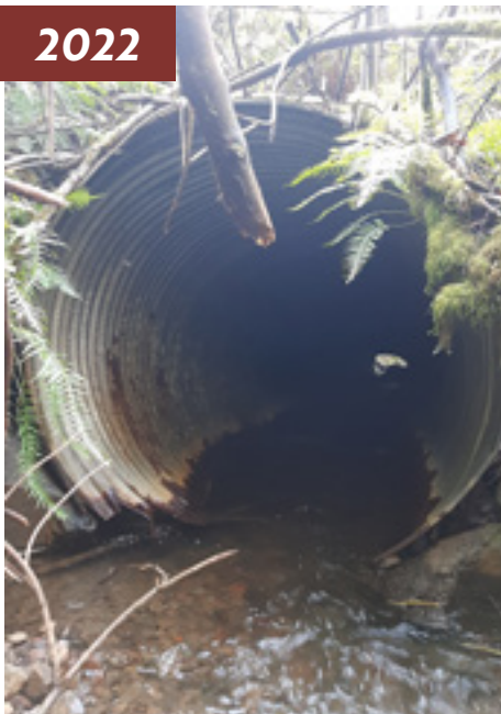
Failing culvert slated to be replaced in 2025
