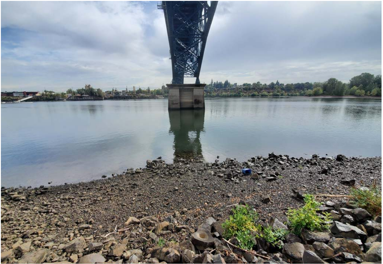
STA: 7+00 - Top of rock armor looking east
