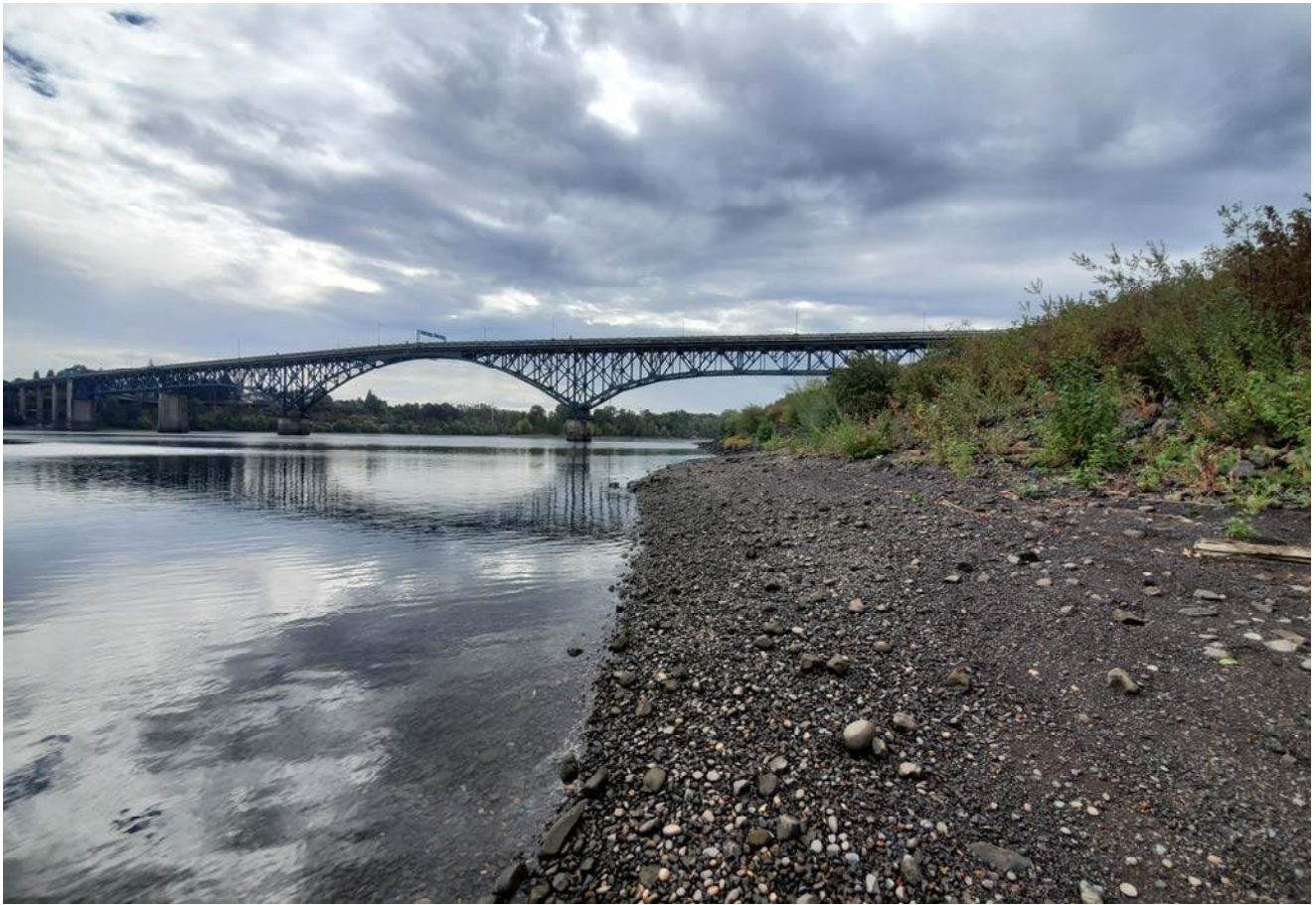
STA: 13+00 - Edge of water looking upstream
