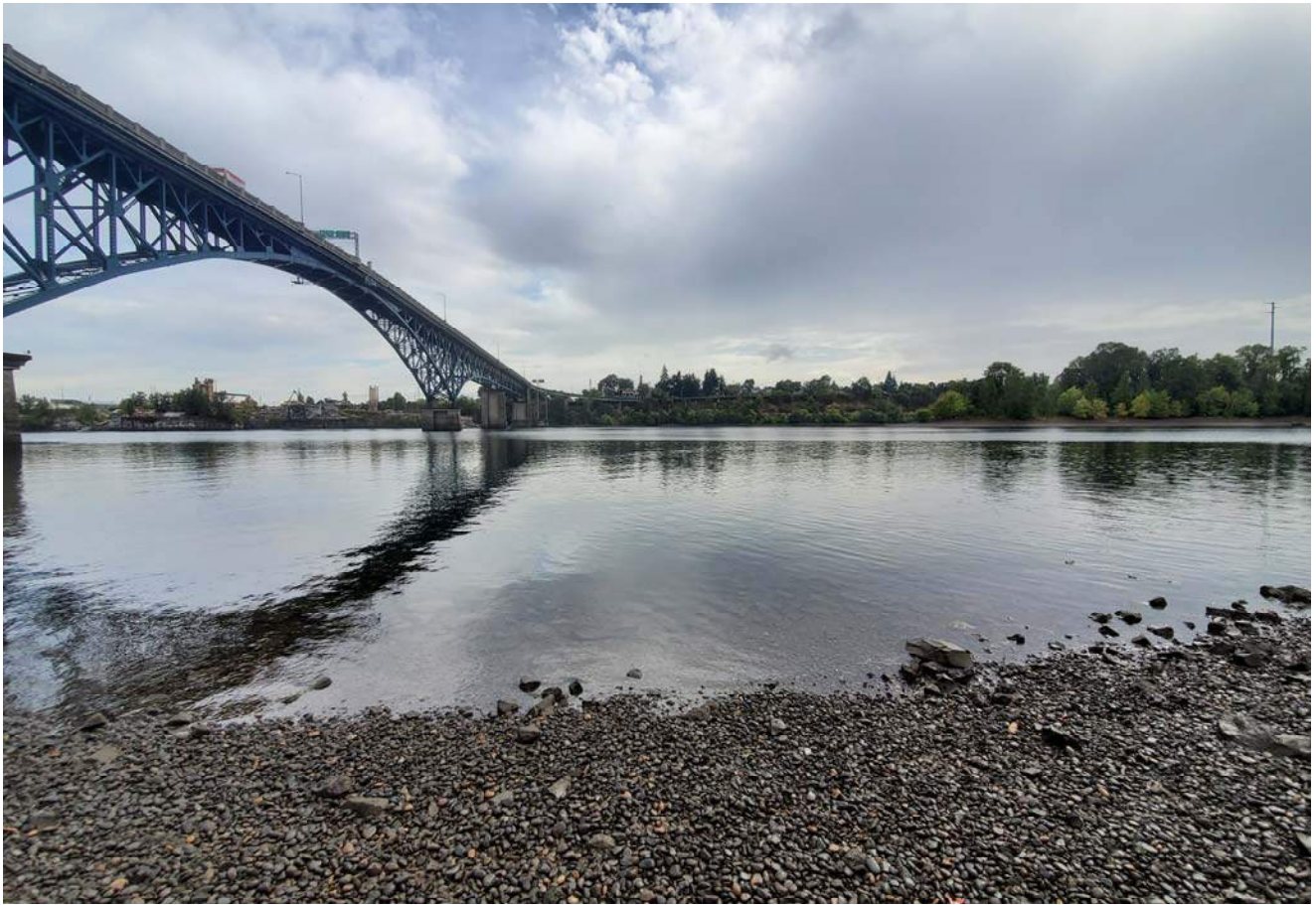
STA: 5+00 - Toe of slope looking east
