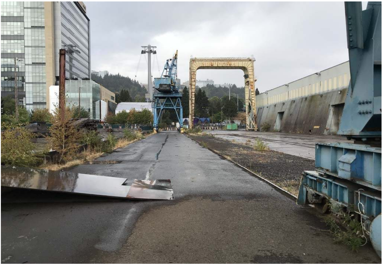
Upland, crane rails looking west
