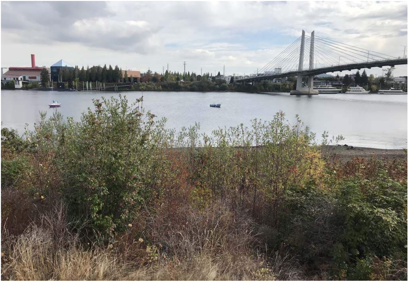
STA: 23+50 - Top of bank looking east
