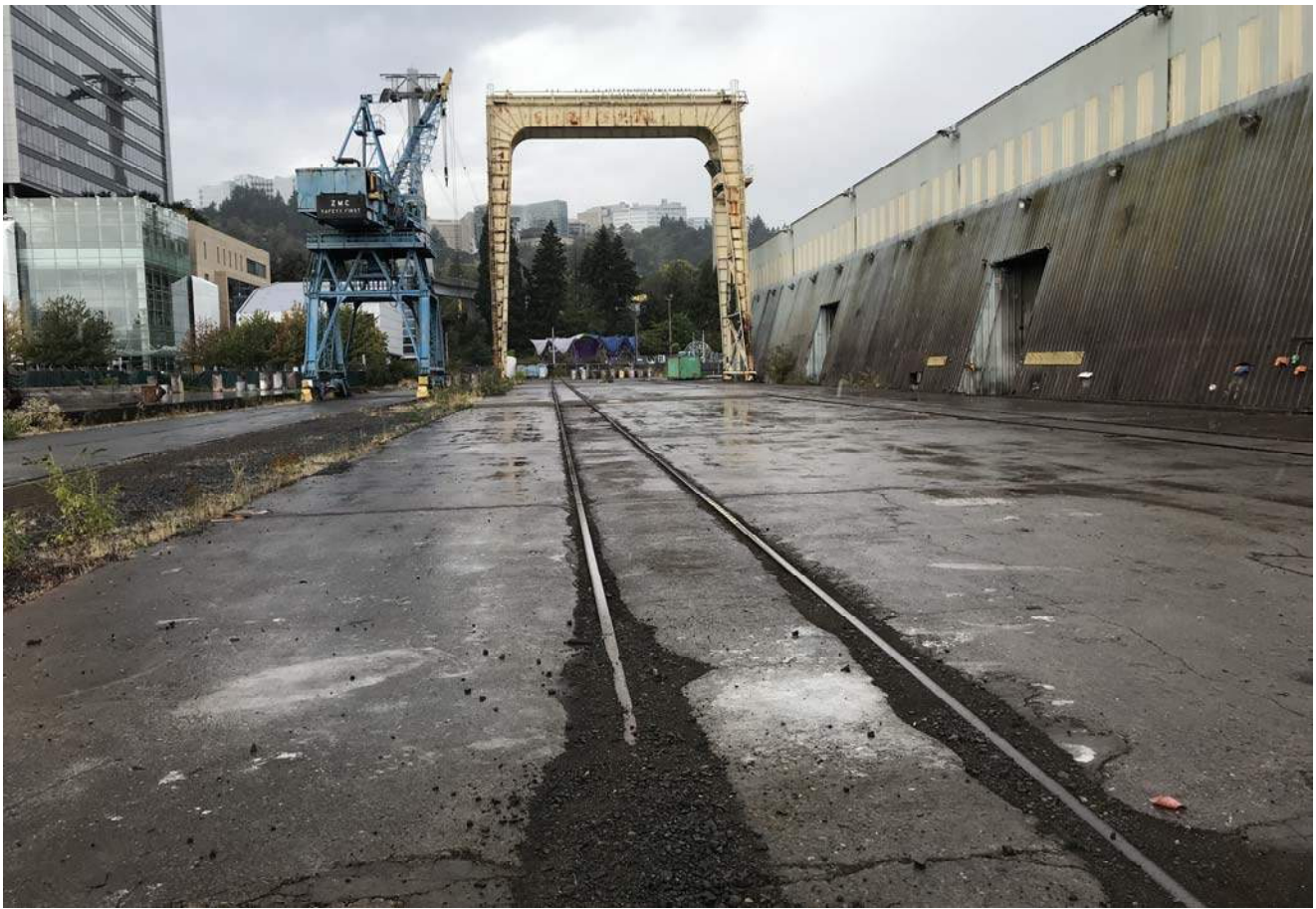
Upland, barge construction area looking west
