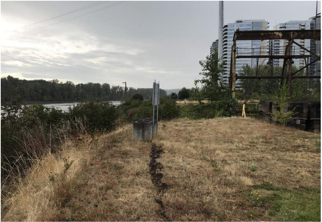
STA: 3+00 - Top of bank looking upstream
