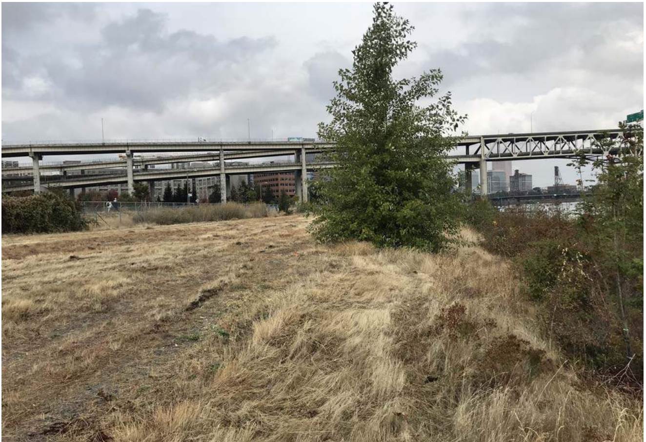
STA: 19+50 - Top of bank looking downstream
