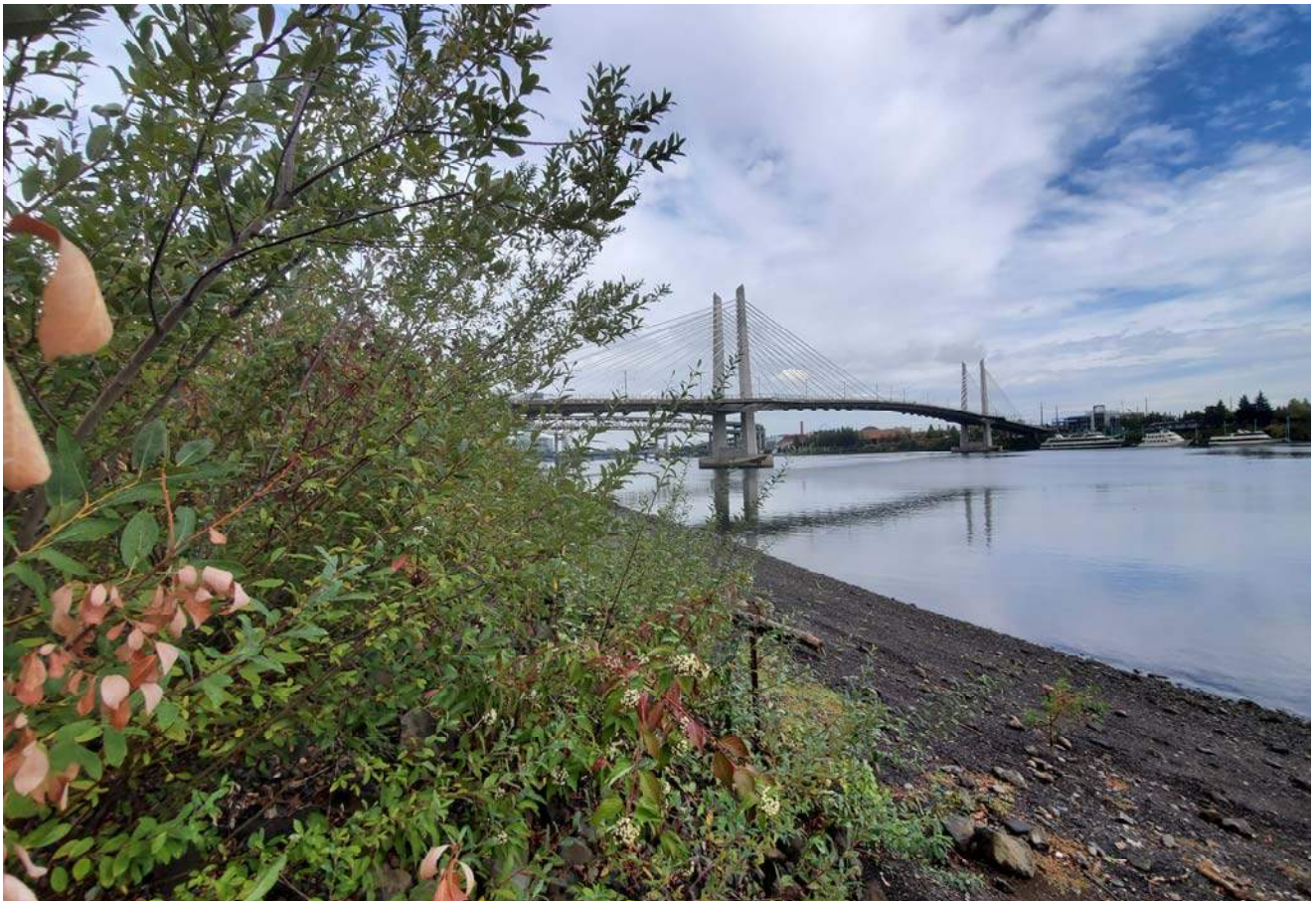
STA: 13+00 - Toe of slope looking downstream
