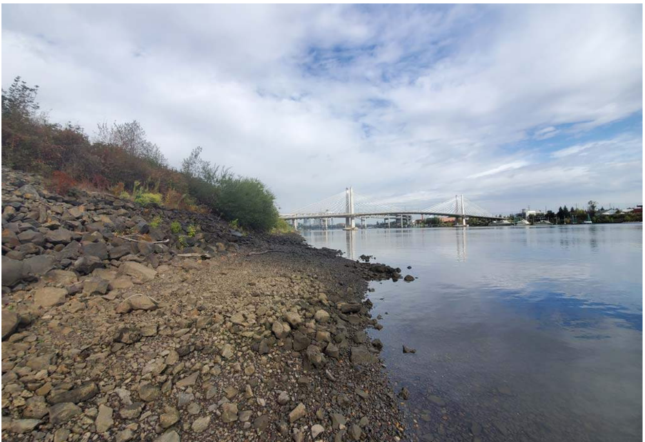
STA: 7+00 - Toe of slope looking downstream
