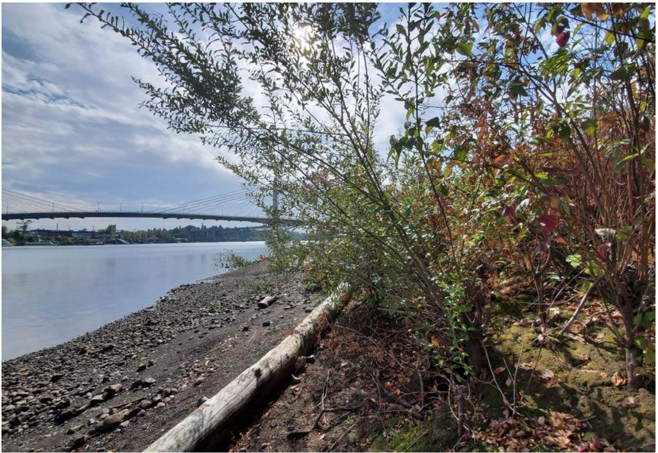
STA: 25+50 - Toe of slope looking upstream
