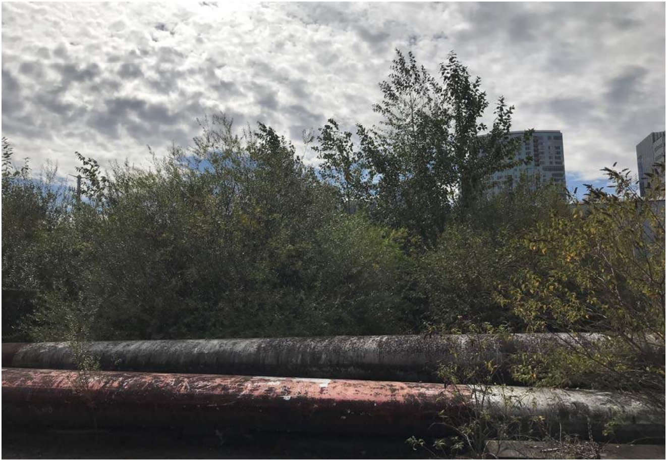
Infiltration facility, north edge looking south
