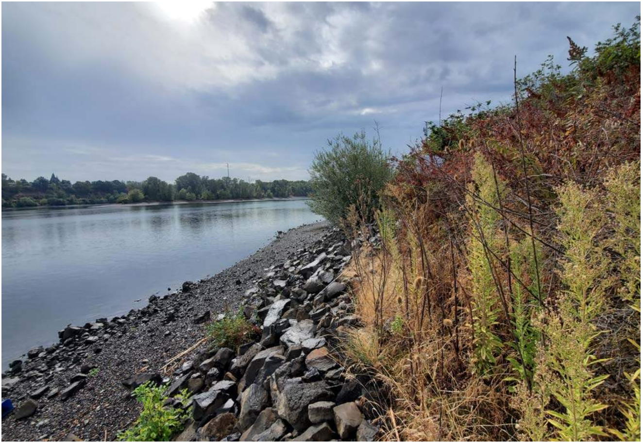
STA: 7+00 - Top of rock armor looking upstream
