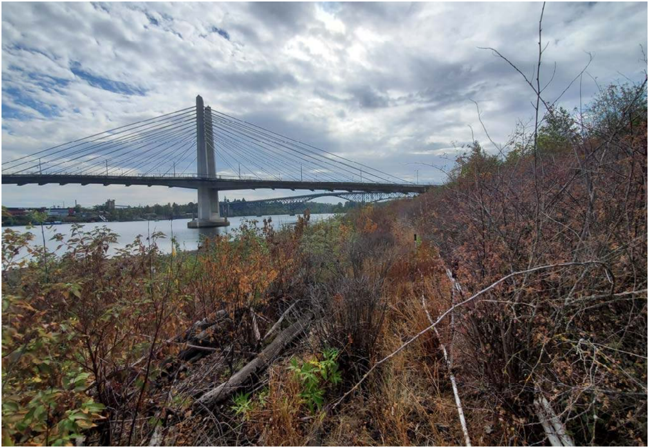
STA: 21+50 - Toe of slope looking upstream
