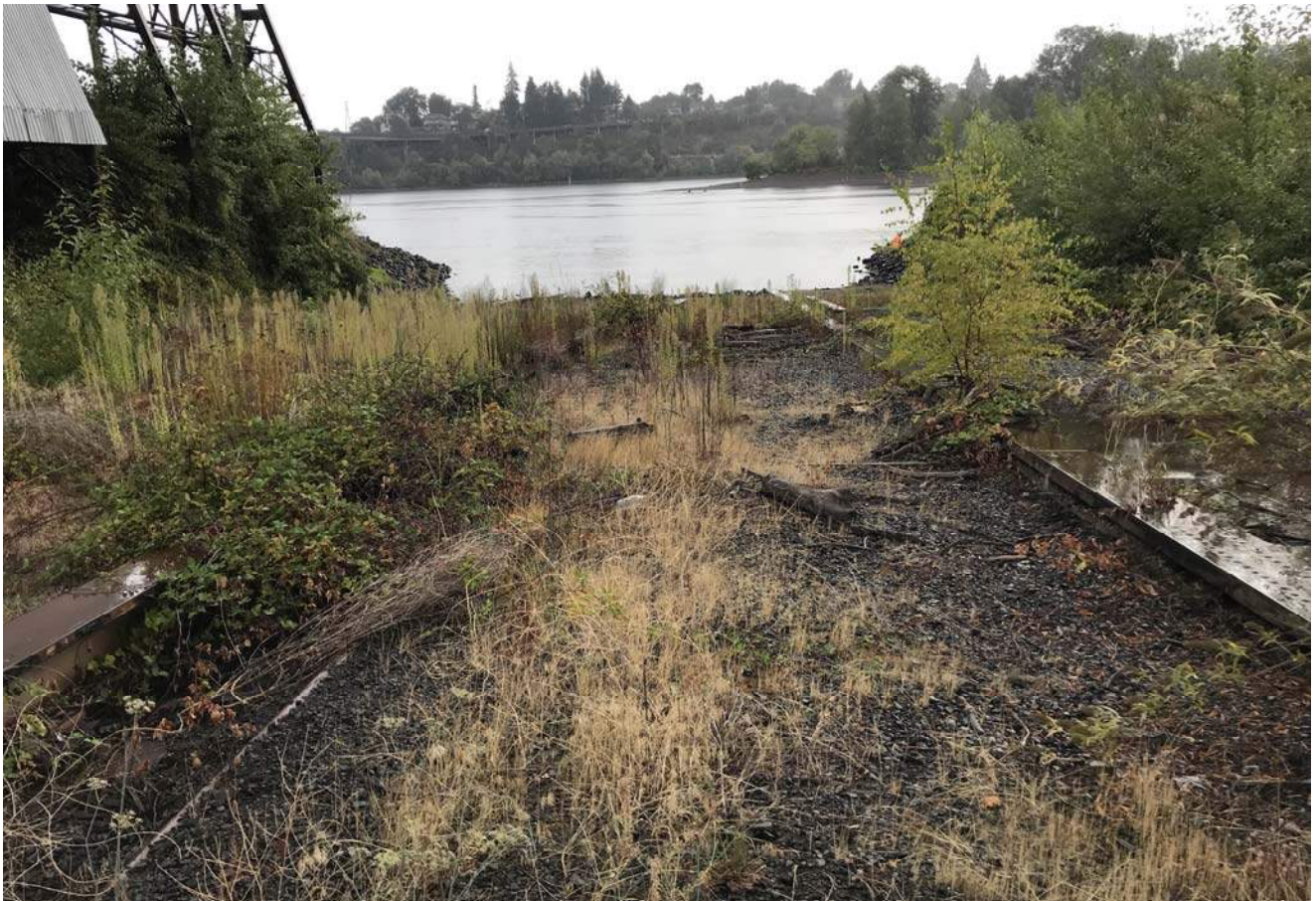
Slipway ramp, looking east
