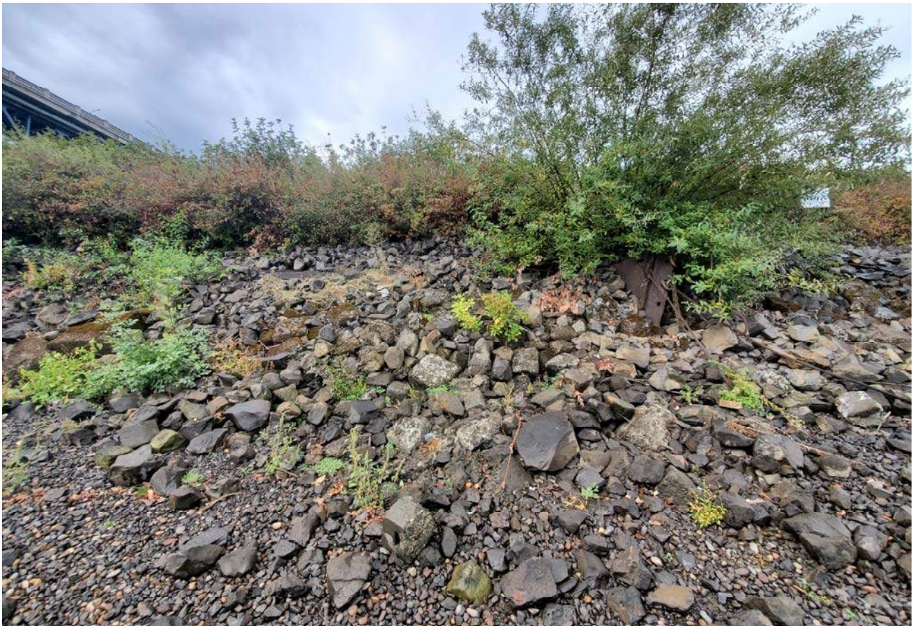
STA: 9+00 - Toe of slope looking west
