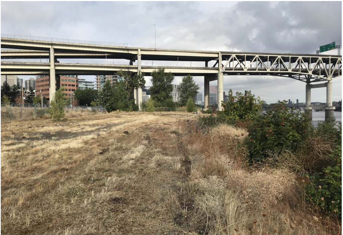
STA: 23+50 - Top of bank looking downstream
