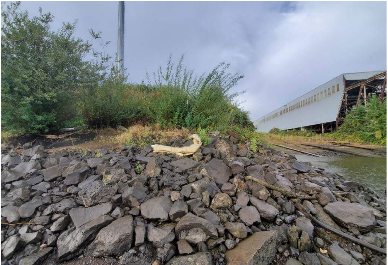
STA: 0+25 - Toe of slope looking west
