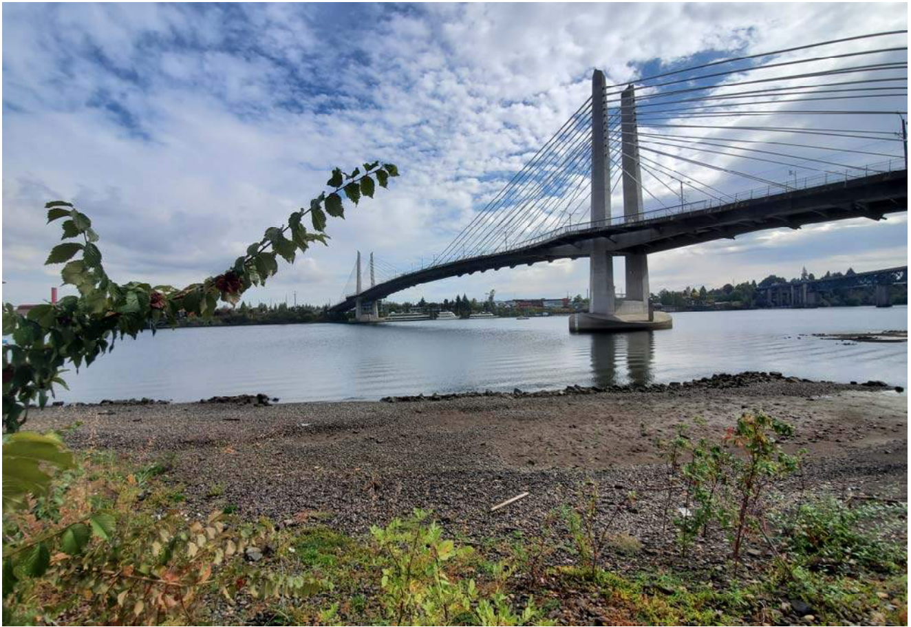
STA: 19+50 - Toe of slope looking east
