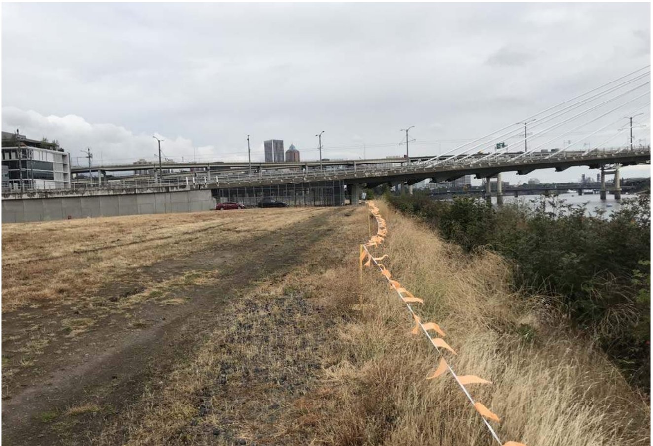
STA: 13+00 - Top of bank looking downstream
