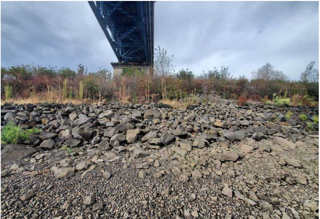
STA: 7+00 - Toe of slope looking west
