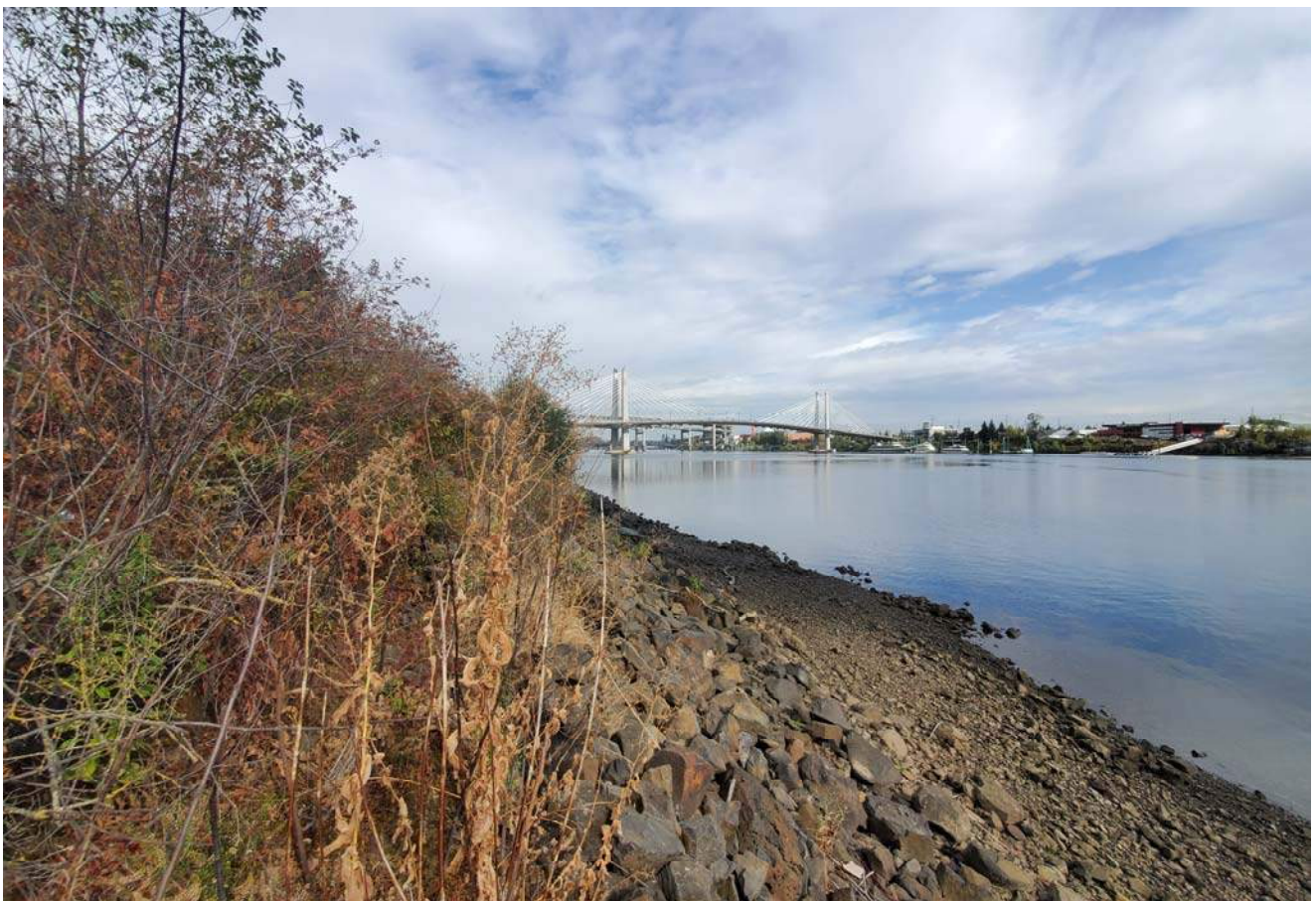
STA: 7+00 - Top of rock armor looking downstream
