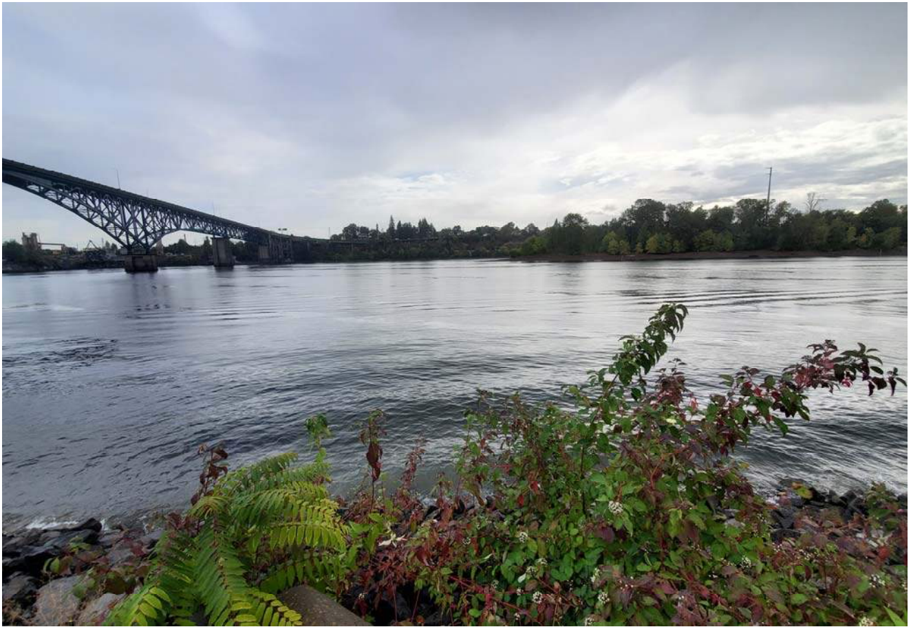
STA: 3+00 - Top of rock armor looking east
