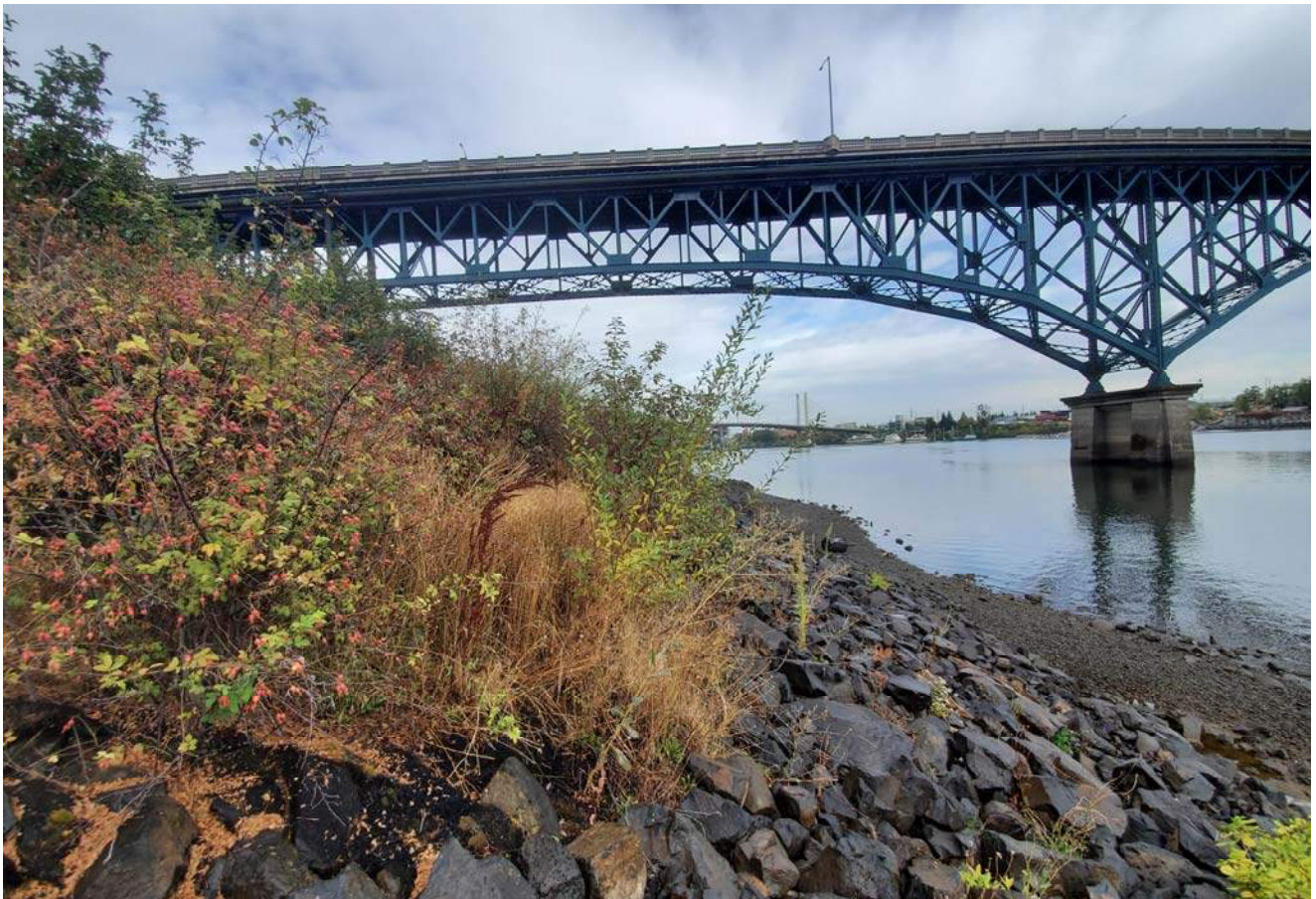
STA: 5+00 - Top of rock armor looking downstream
