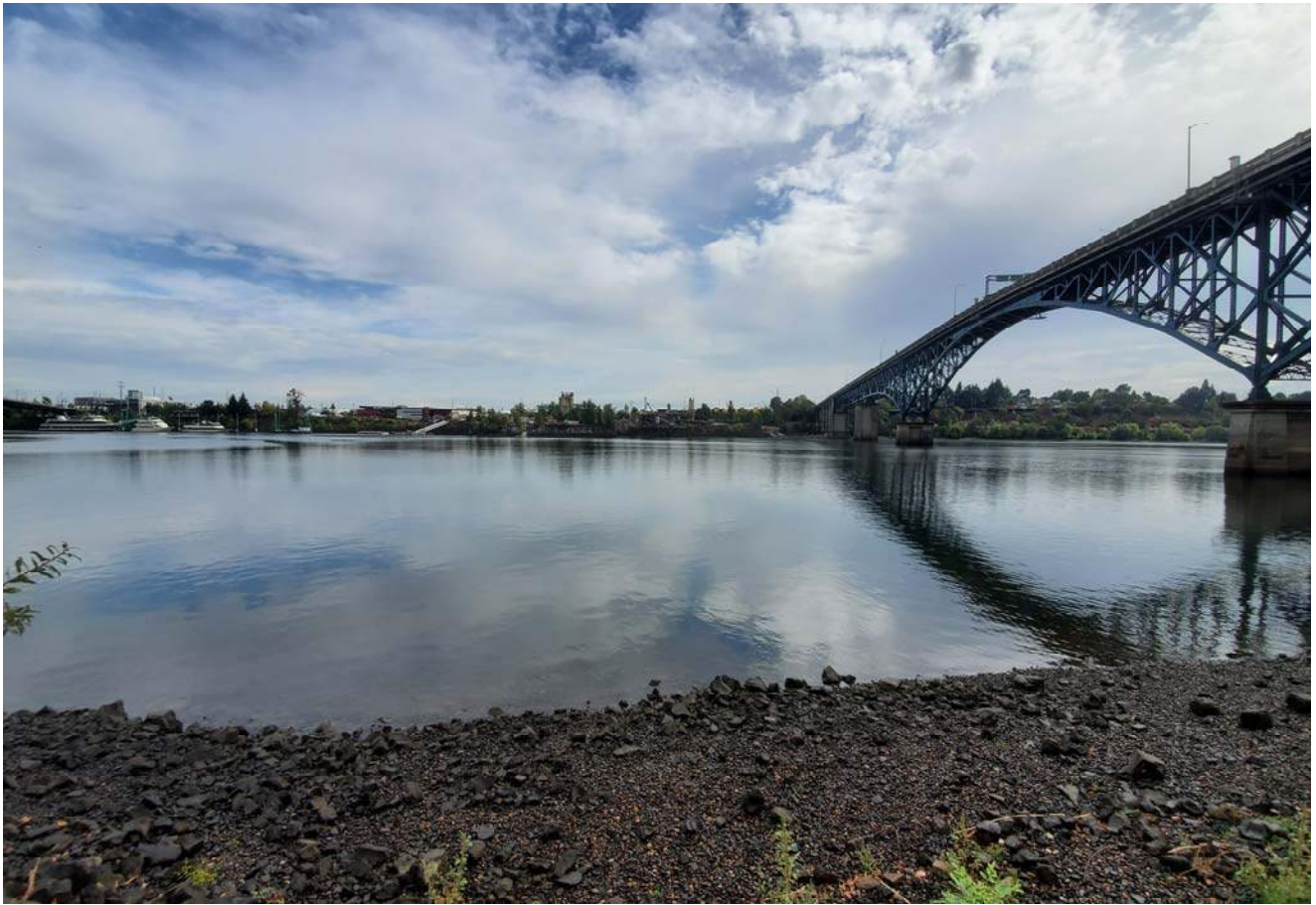
STA: 9+00 - Top of rock armor looking east
