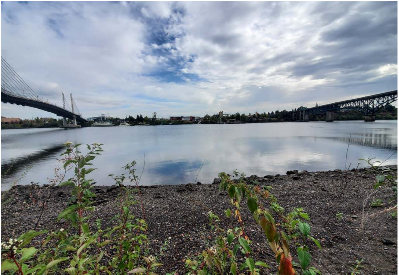
STA: 15+00 - Toe of slope looking east
