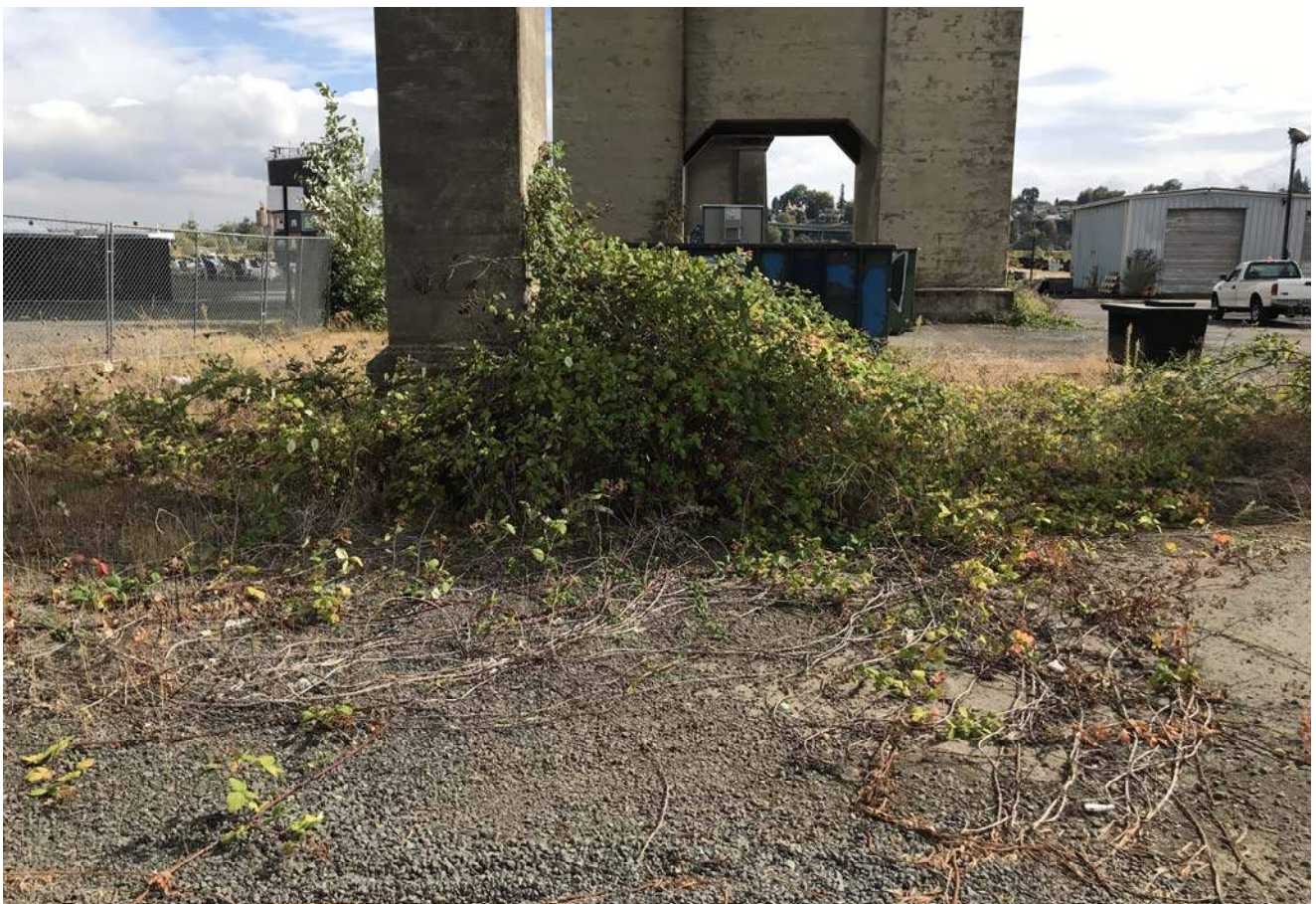
Upland cap beneath Ross Island Bridge, looking east
