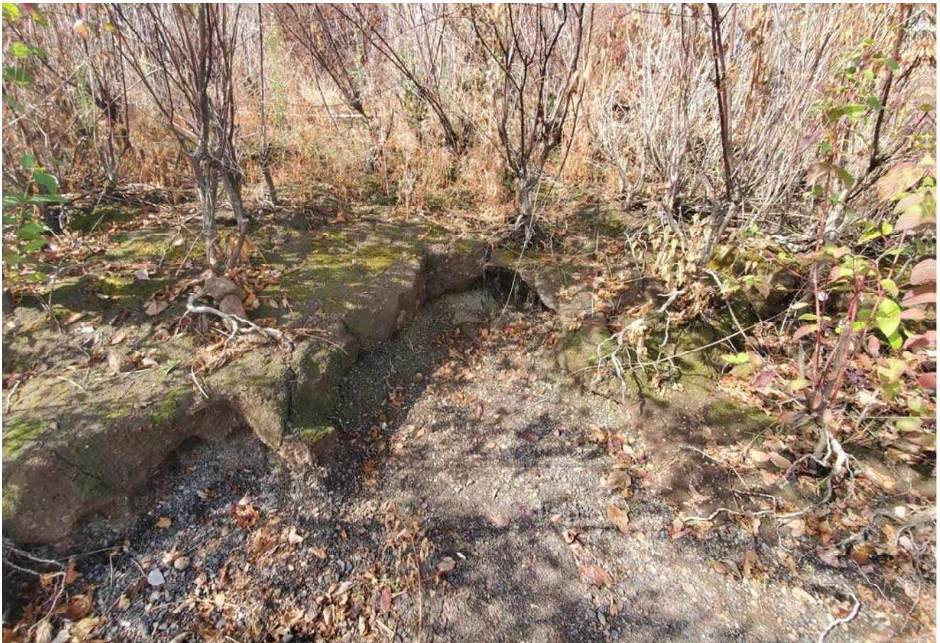
STA: 25+50 - Toe of slope looking west
