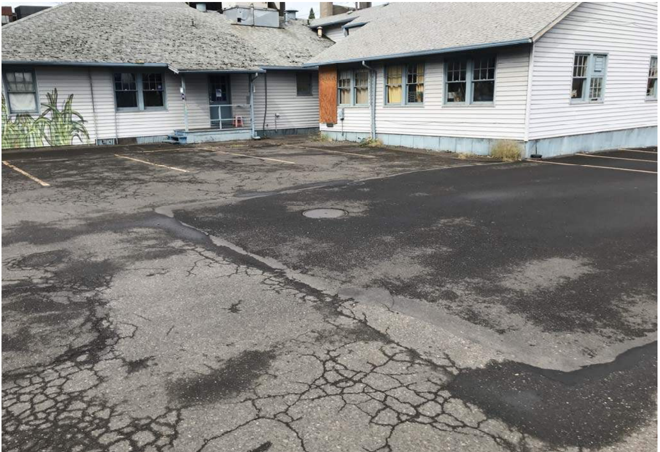
Operational area and office building, looking northwest
