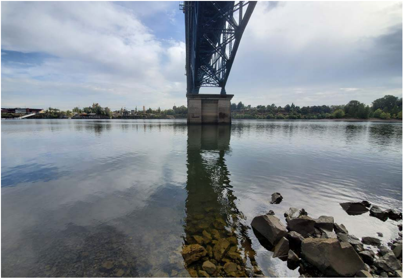
STA: 7+00 - Toe of slope looking east
