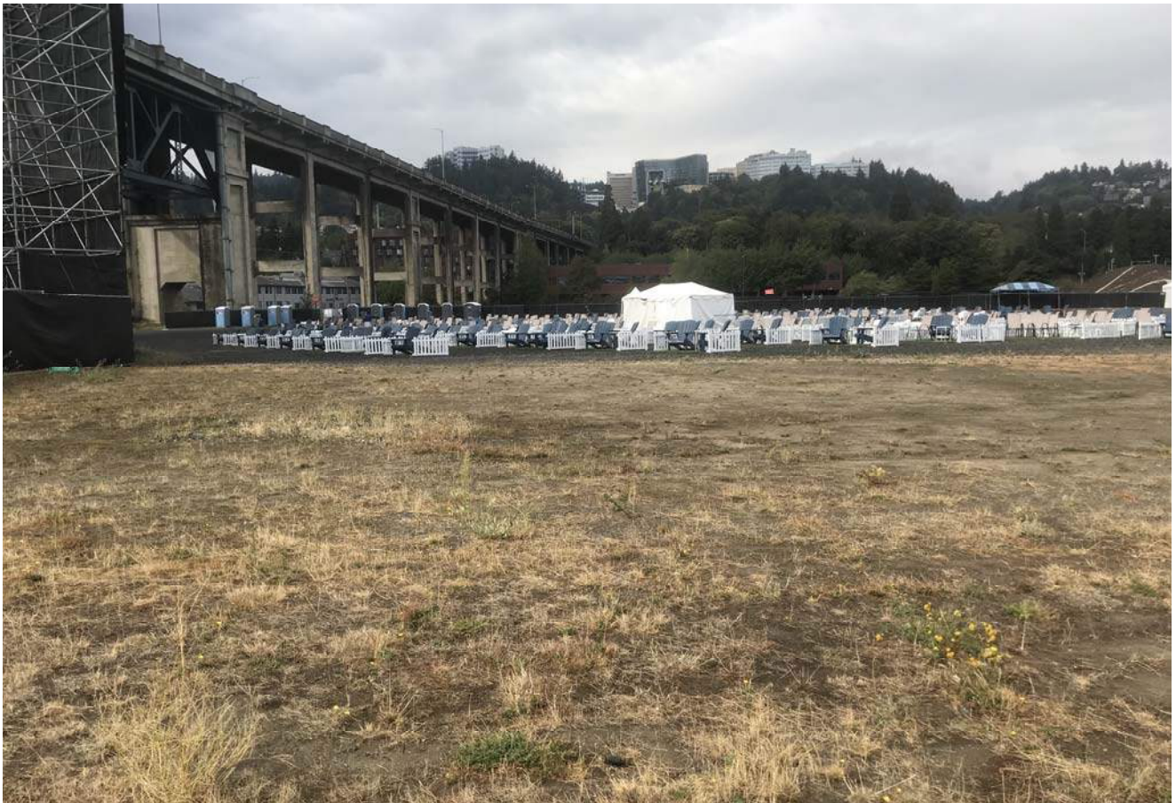
STA: 9+00 - Top of bank looking west
