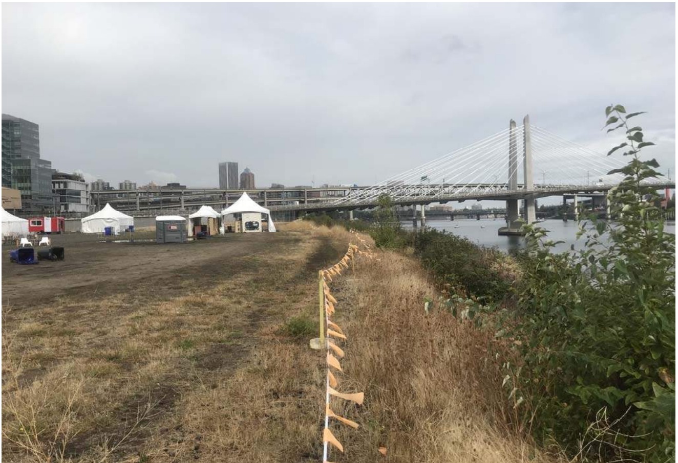
STA: 9+00 - Top of bank looking downstream
