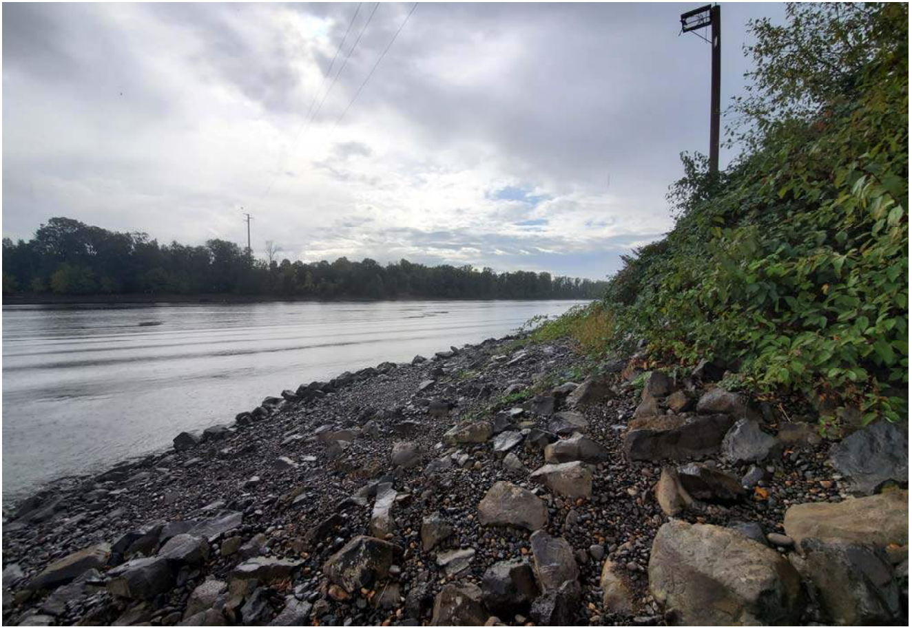
STA: 0+25 - Toe of slope looking upstream
