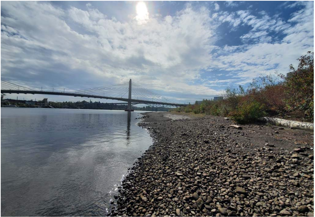
STA: 25+50 - Edge of water looking upstream
