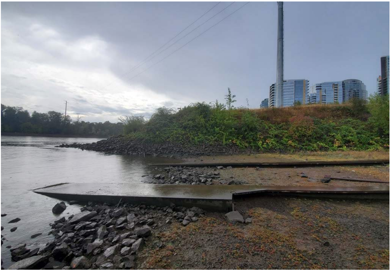
Lower slipway ramp, looking upstream
