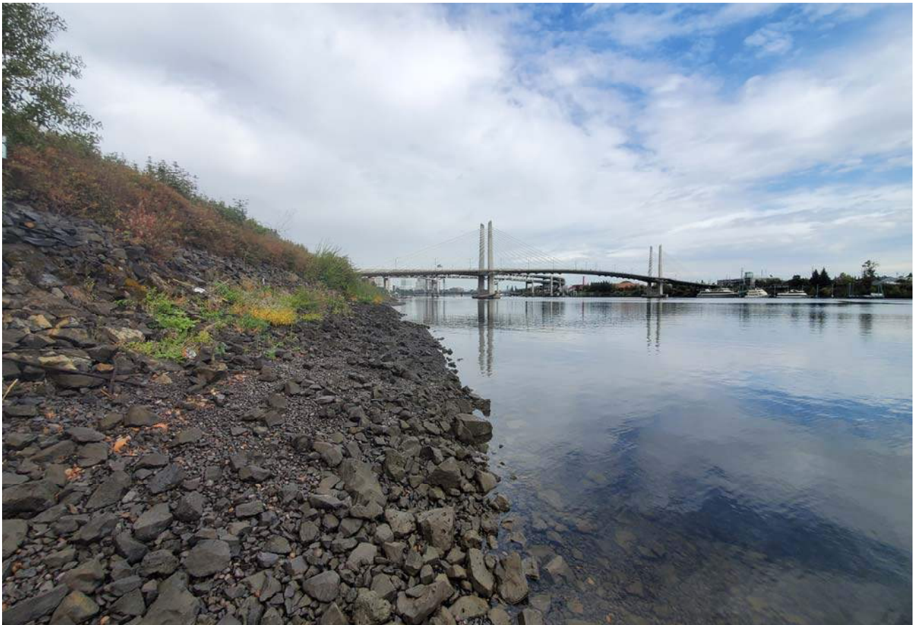
STA: 9+00 - Toe of slope looking downstream
