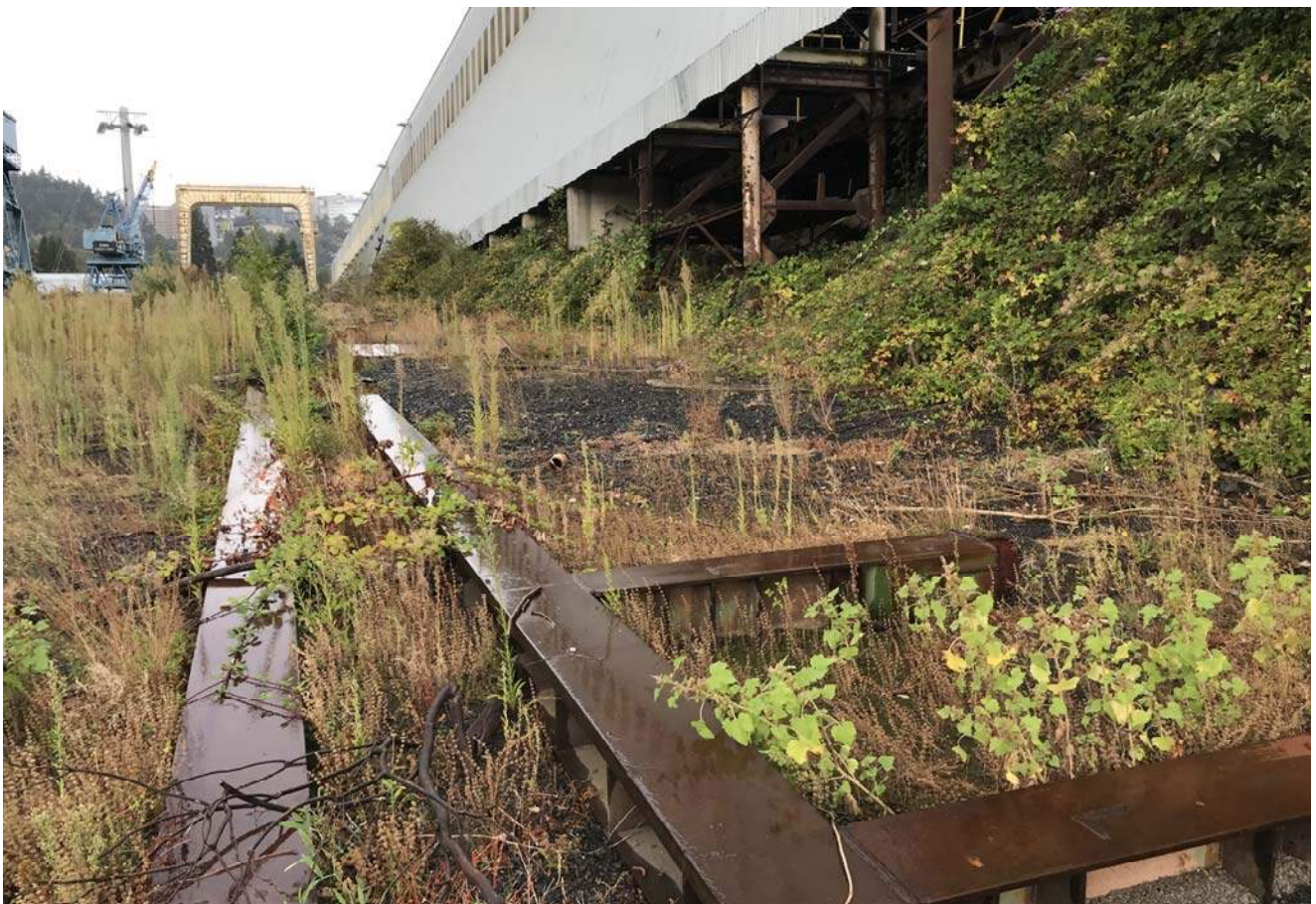
Slipway ramp, looking west
