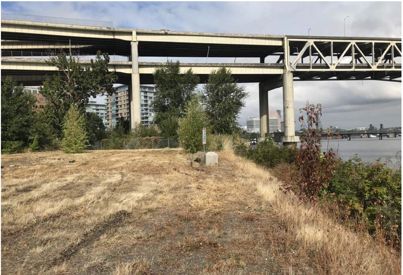
STA: 25+50 - Top of bank looking downstream
