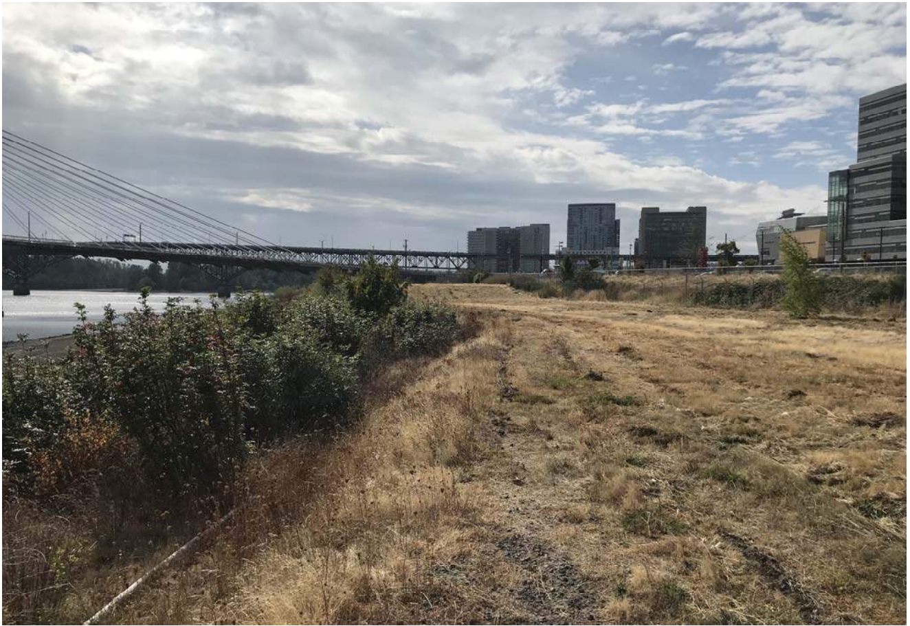
STA: 25+50 - Top of bank looking upstream
