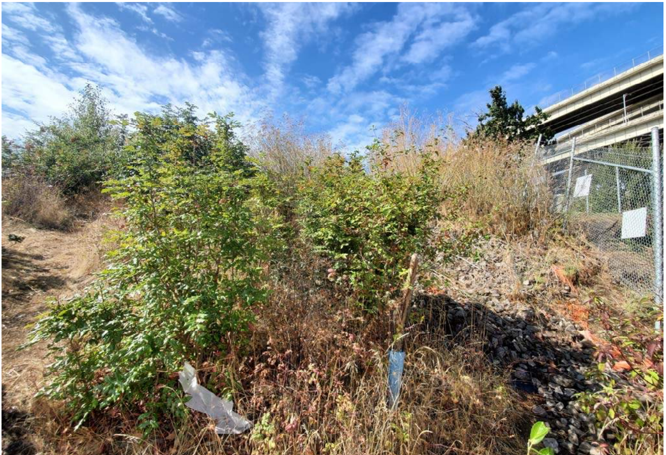
STA: 26+50 - Toe of slope looking west
