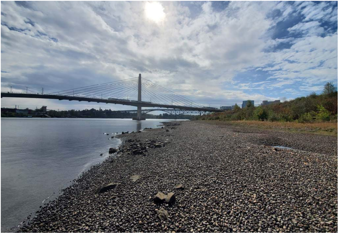
STA: 23+50 - Edge of water looking upstream
