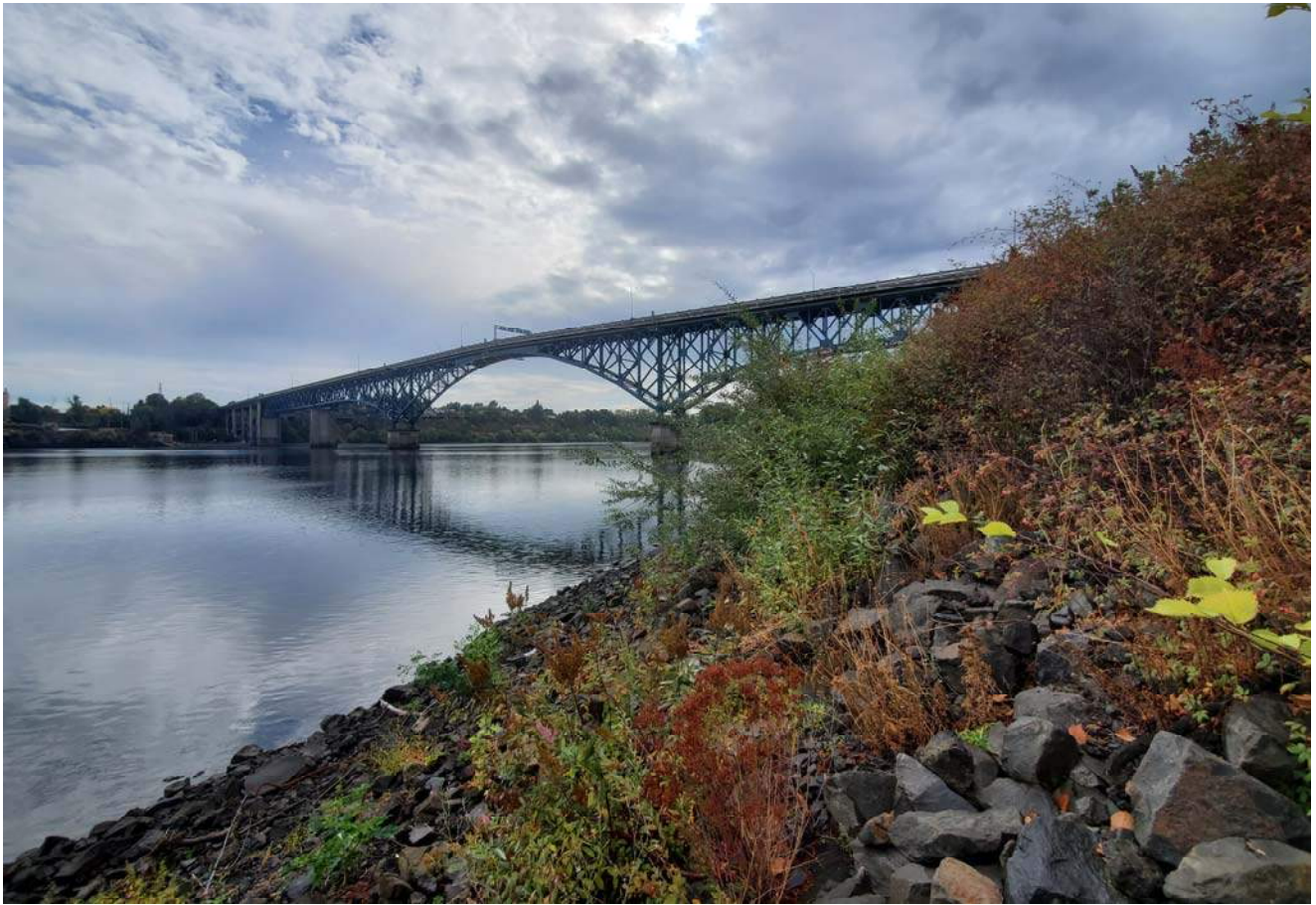
STA: 11+00 - Top of rock armor looking upstream
