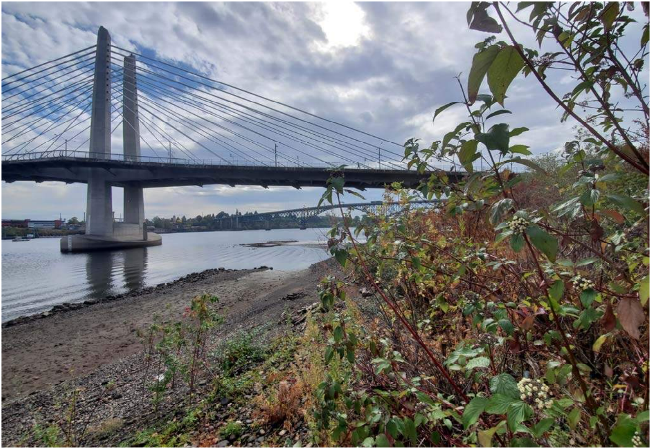
STA: 19+50 - Toe of slope looking upstream
