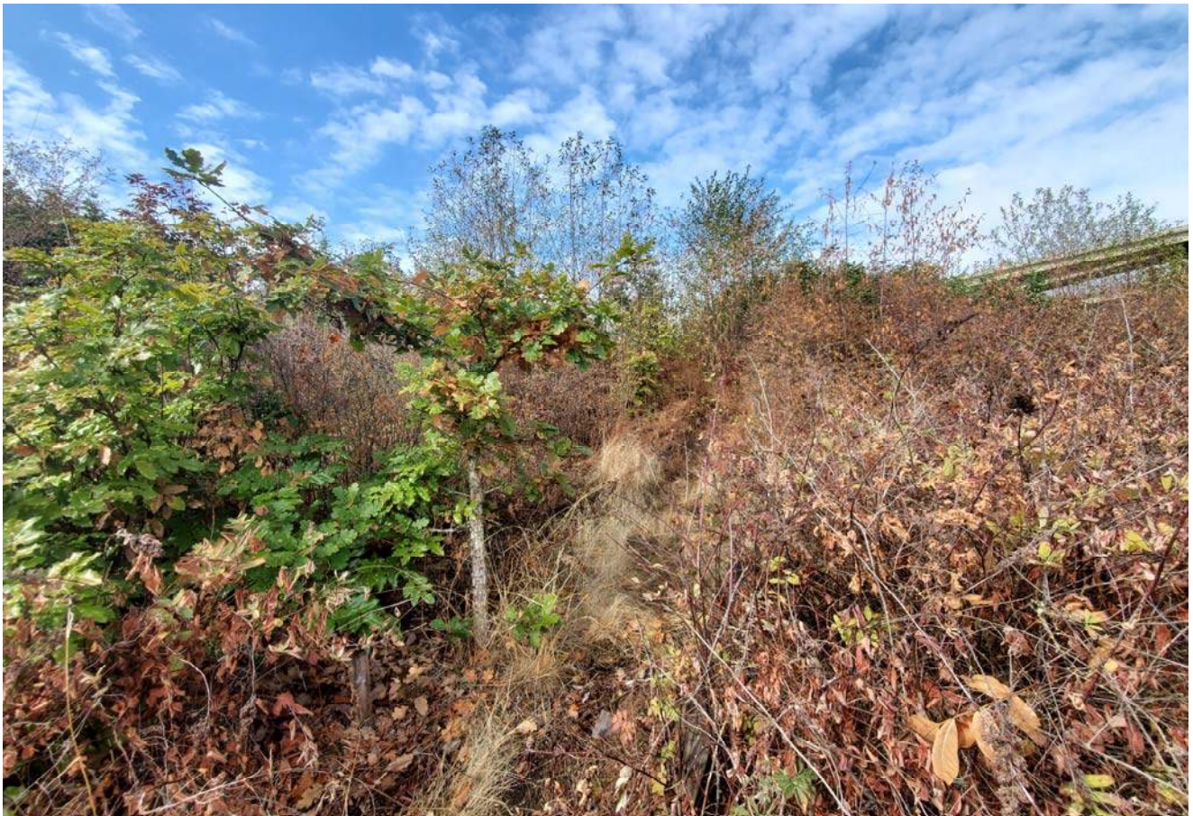
STA: 23+50 - Toe of slope looking west
