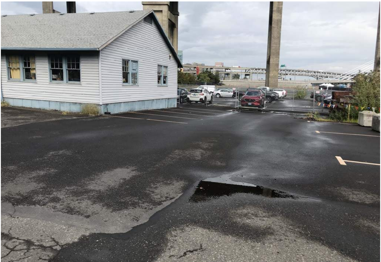
Operational area and office building, looking north
