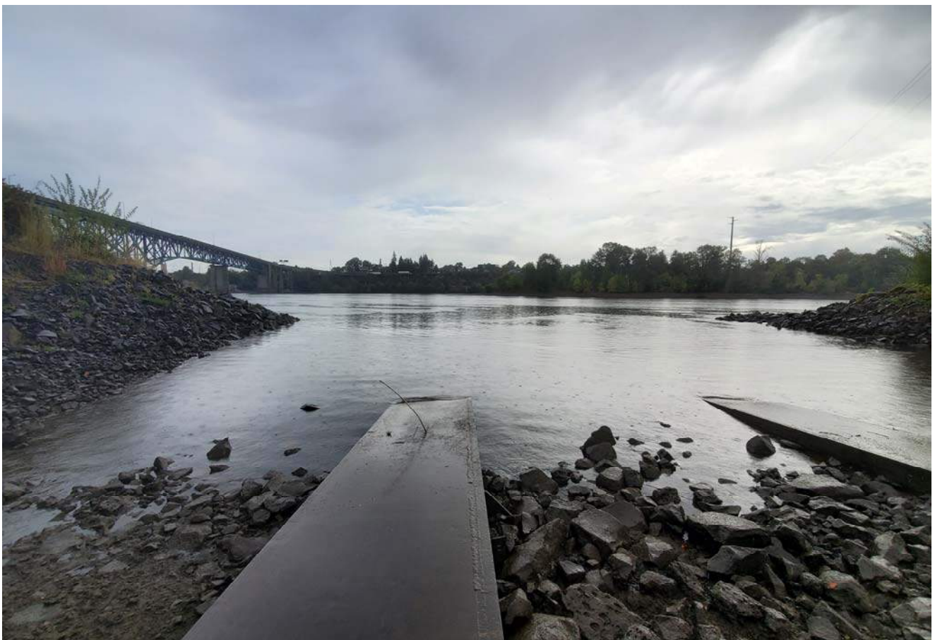
Lower slipway ramp, looking east
