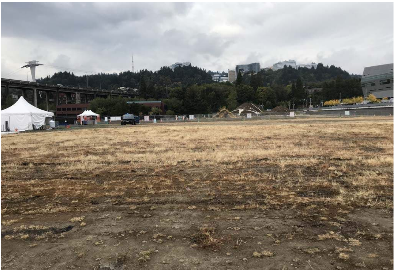
STA: 13+00 - Top of bank looking west
