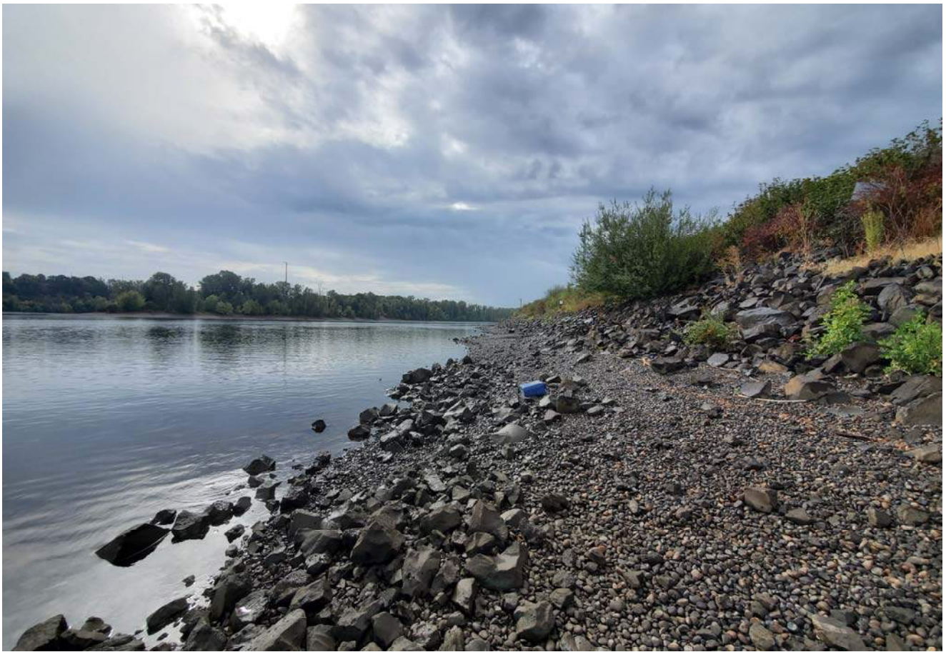
STA: 7+00 - Toe of slope looking upstream
