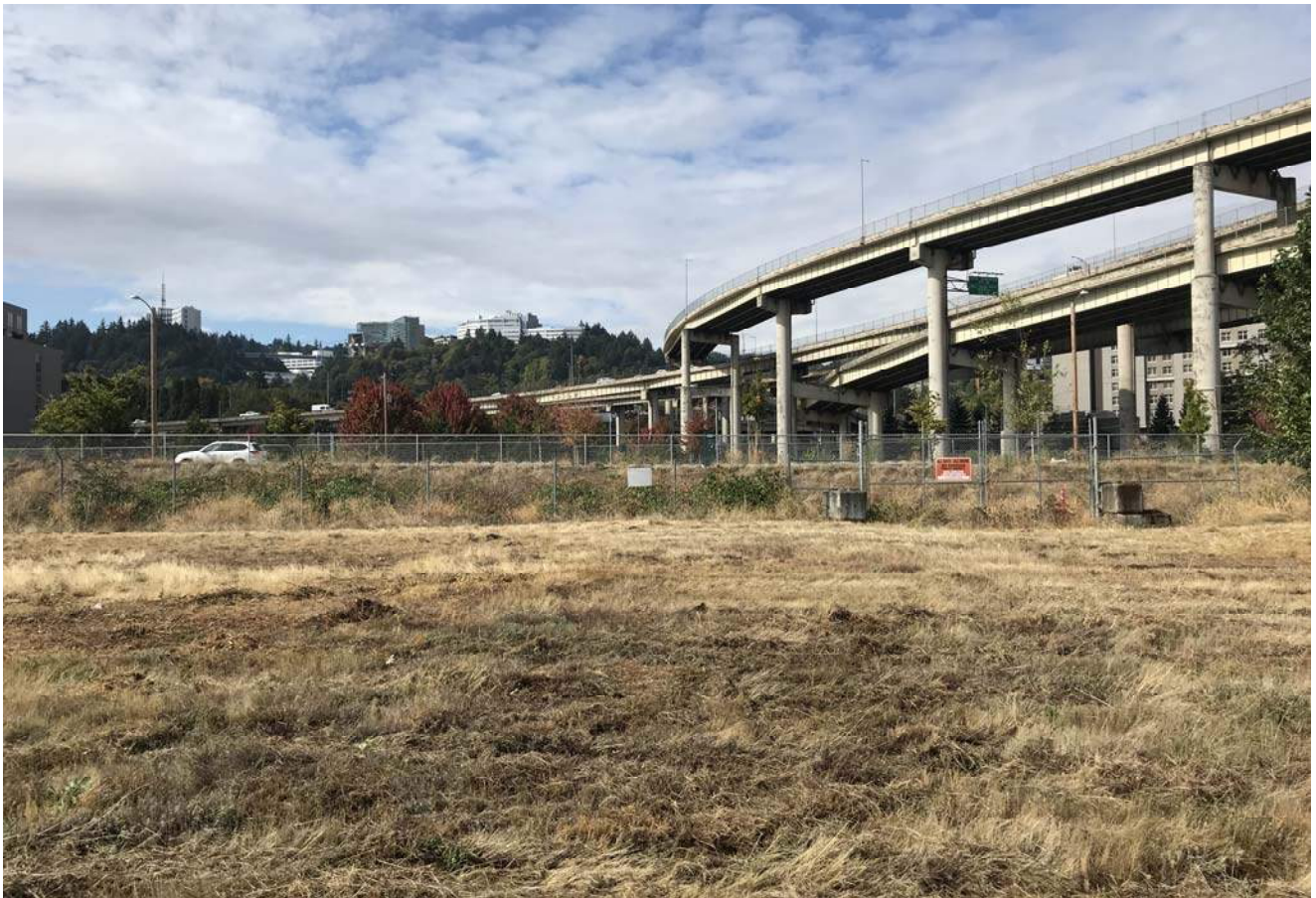
STA: 25+50 - Top of bank looking west
