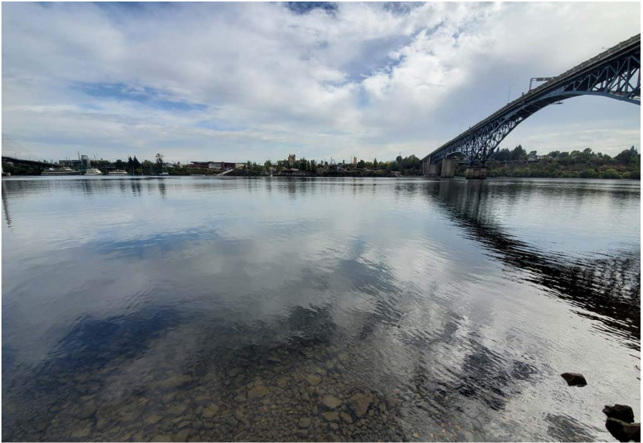
STA: 9+00 - Toe of slope looking east
