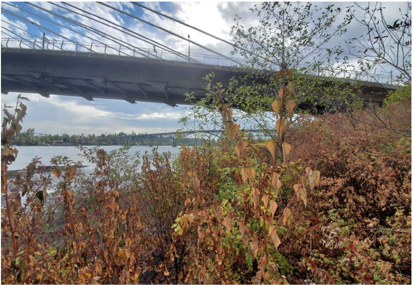
STA: 17+00 - Toe of slope looking upstream
