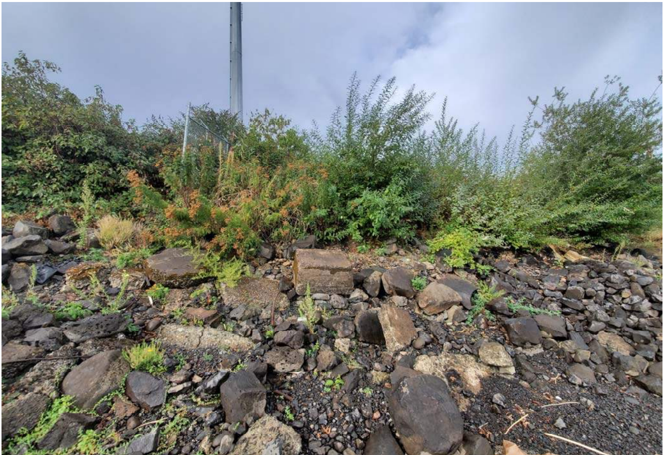
STA: 0+00 - Toe of slope looking west
