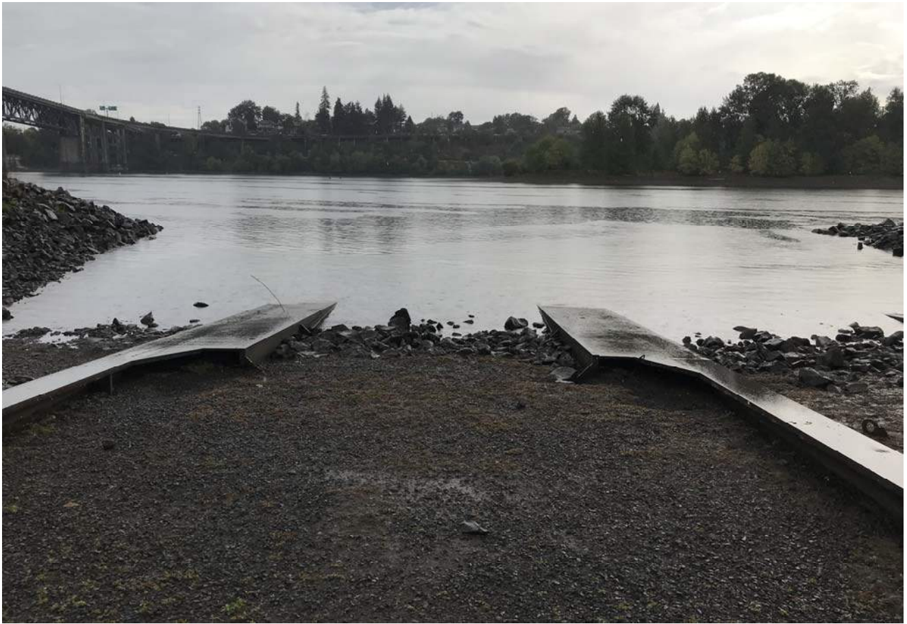
Middle slipway ramp, looking east
