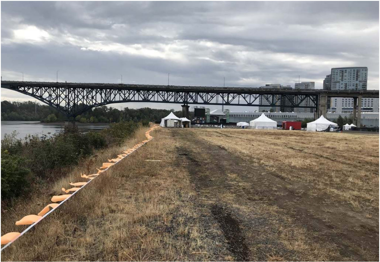
STA: 15+00 - Top of bank looking upstream
