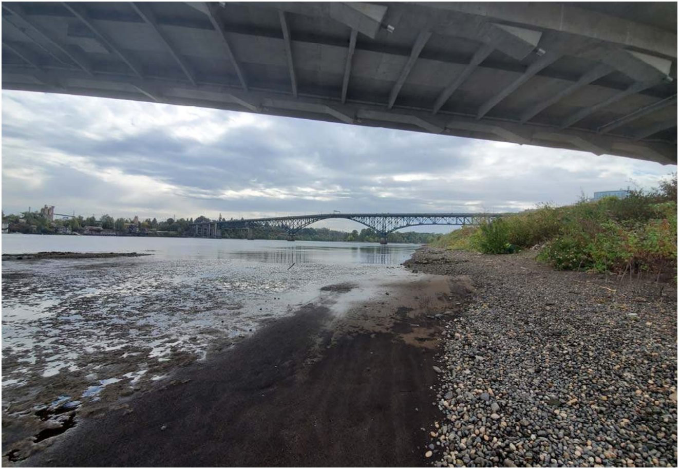
STA: 17+00 - Edge of water looking upstream
