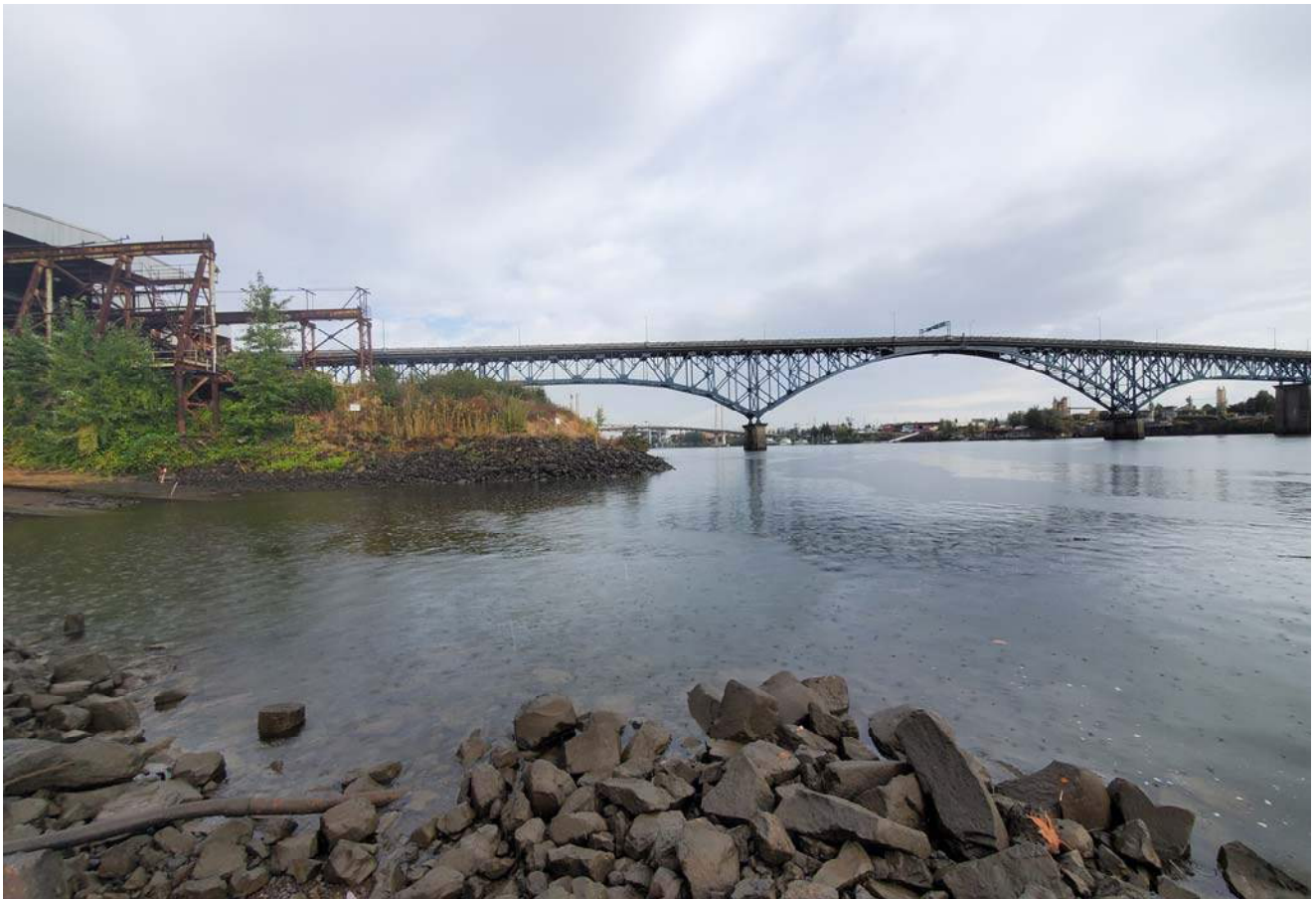
STA: 0+25 - Toe of slope looking downstream
