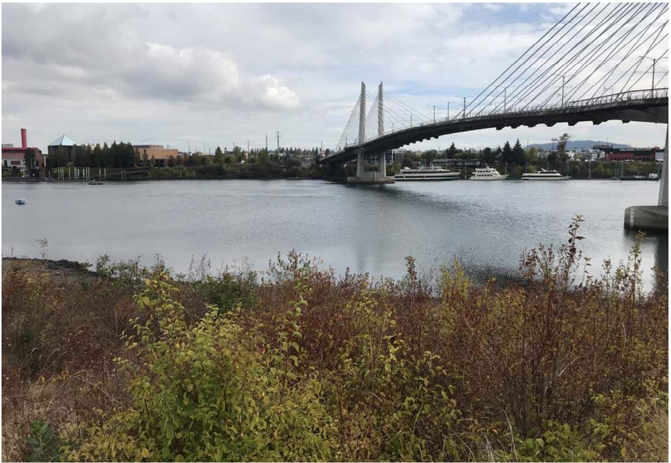
STA: 19+50 - Top of bank looking east
