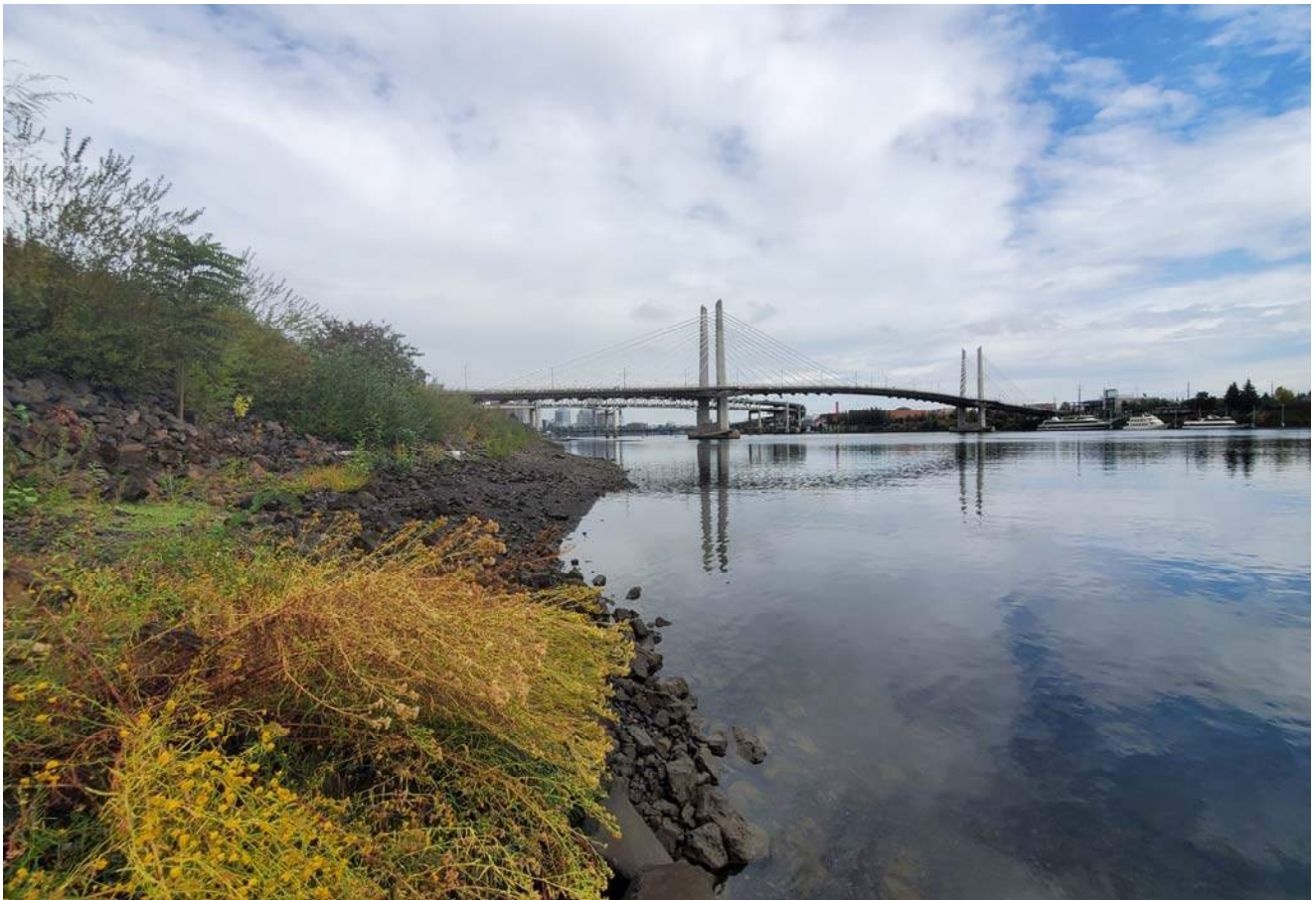
STA: 11+00 - Toe of slope looking downstream
