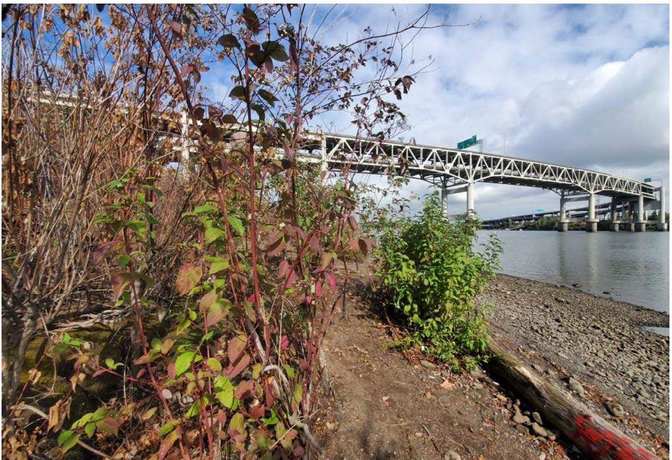
STA: 25+50 - Toe of slope looking downstream
