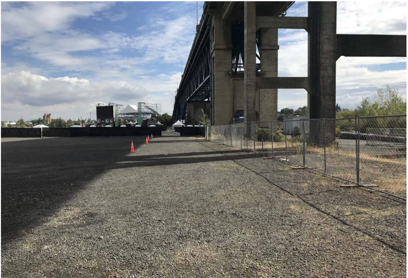
Upland cap, Ross Island Bridge northwest corner looking east
