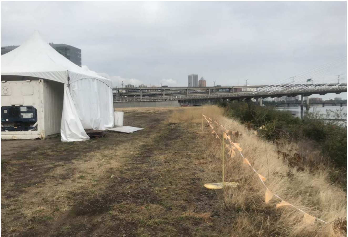
STA: 11+00 - Top of bank looking downstream
