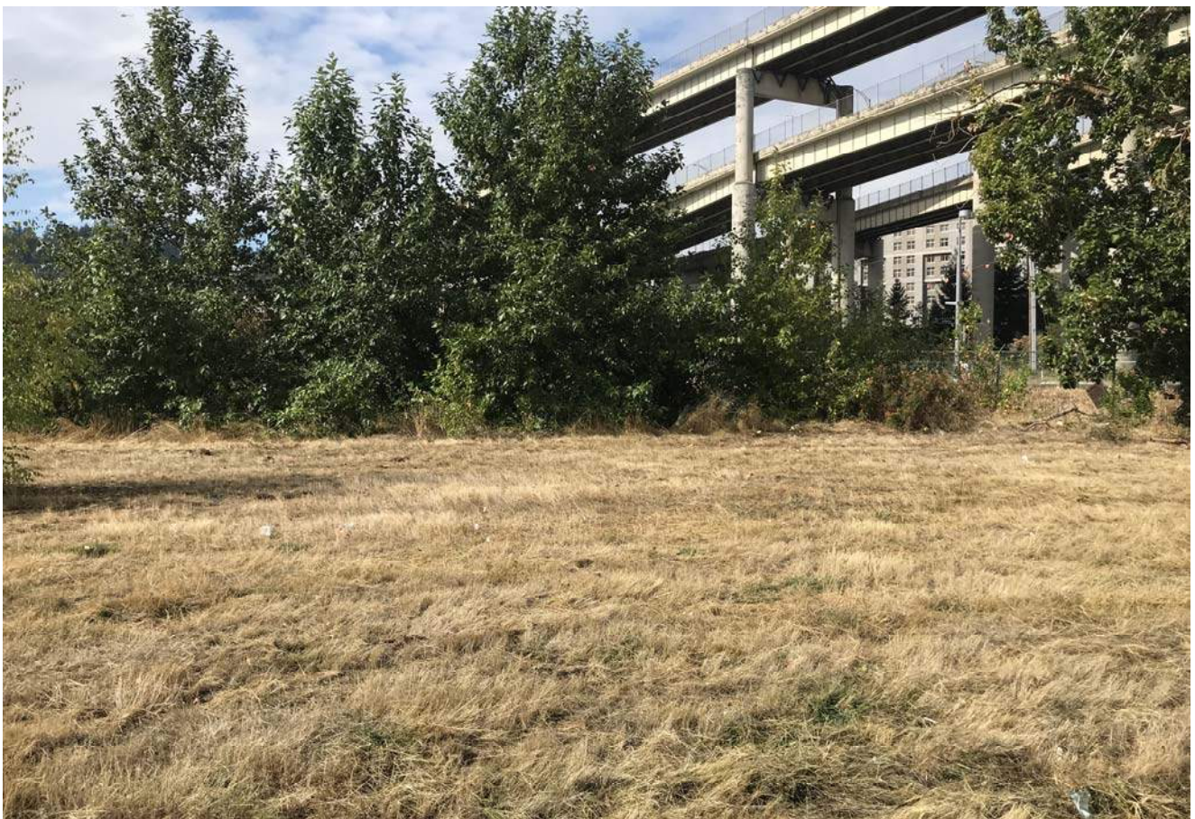
STA: 26+50 - Top of bank looking west
