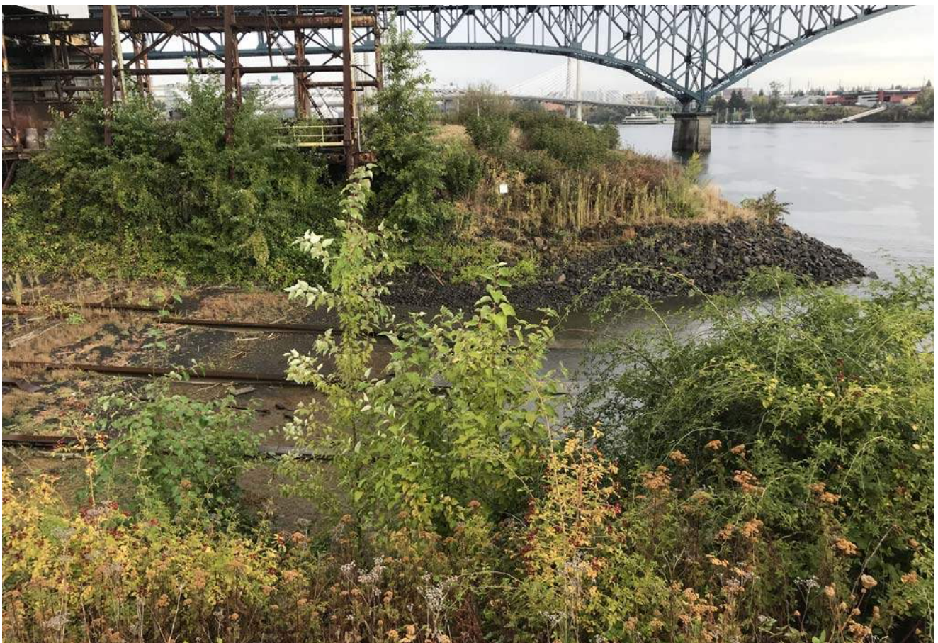
STA:0+25 - Top of bank looking downstream
