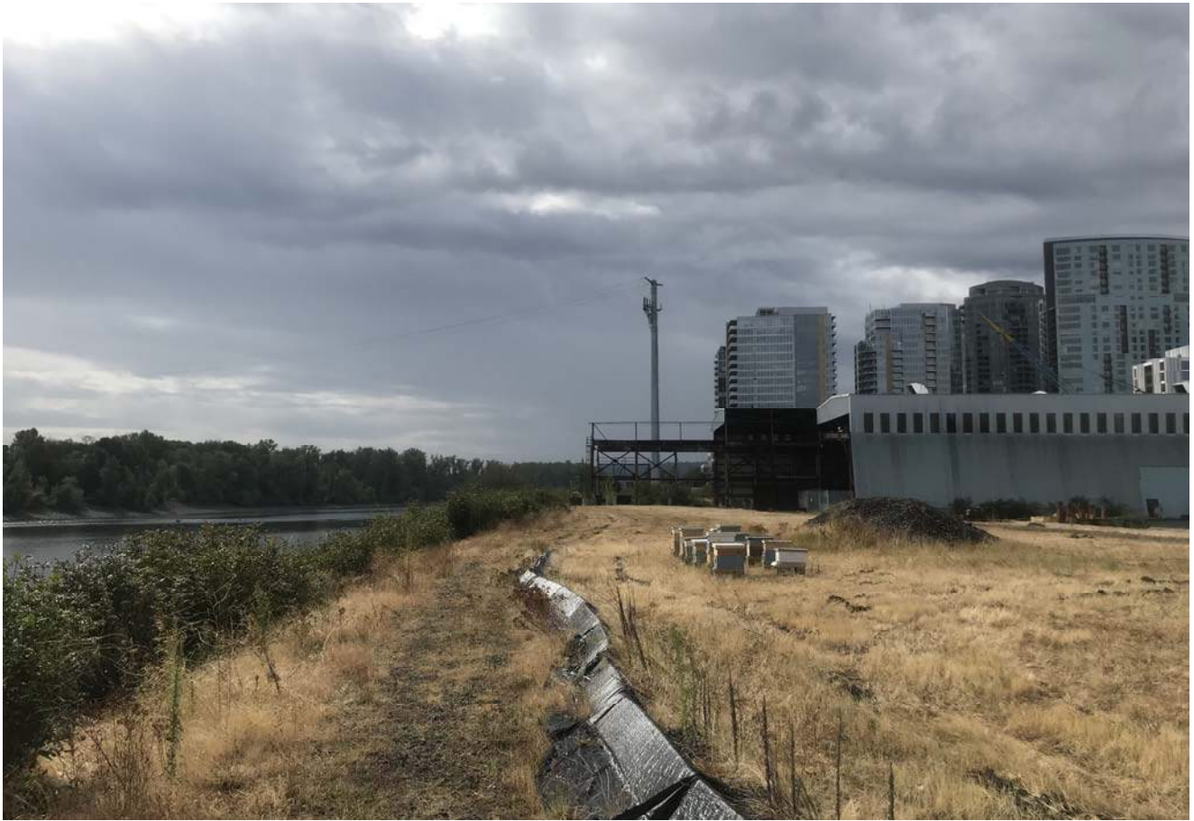
STA: 7+00 - Top of bank looking upstream
