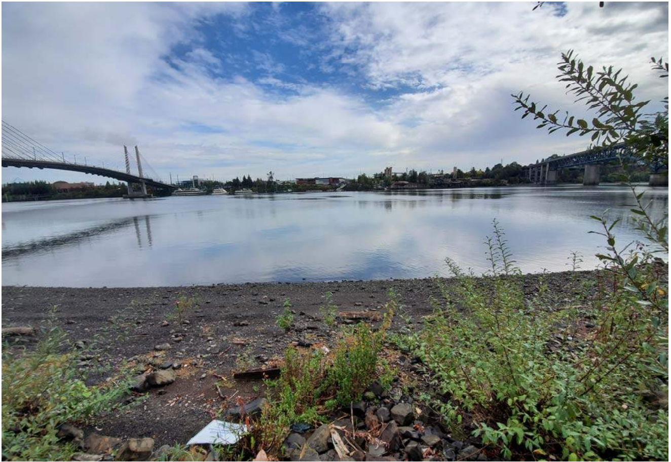
STA: 13+00 - Toe of slope looking east
