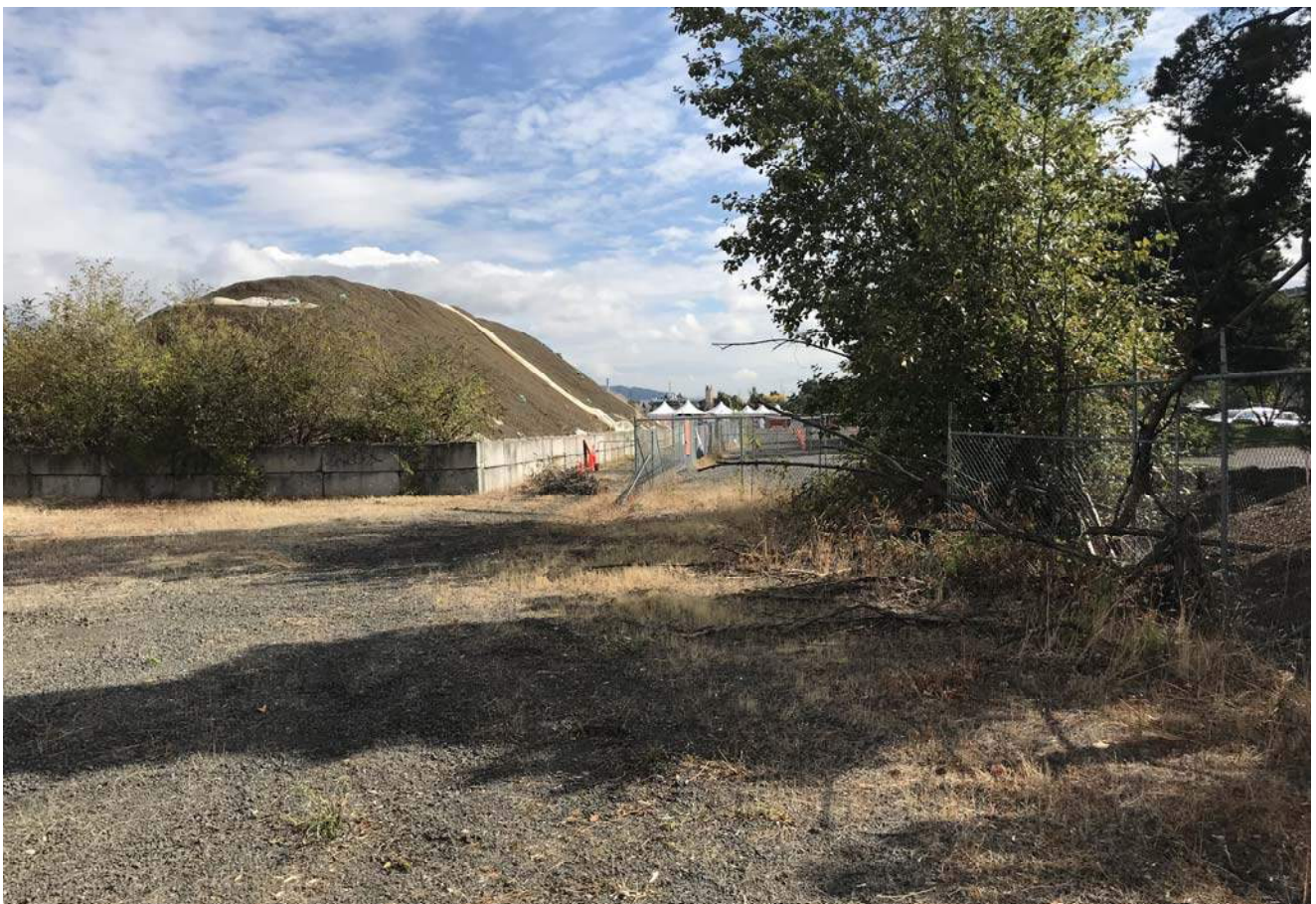
Upland cap, west edge looking east
