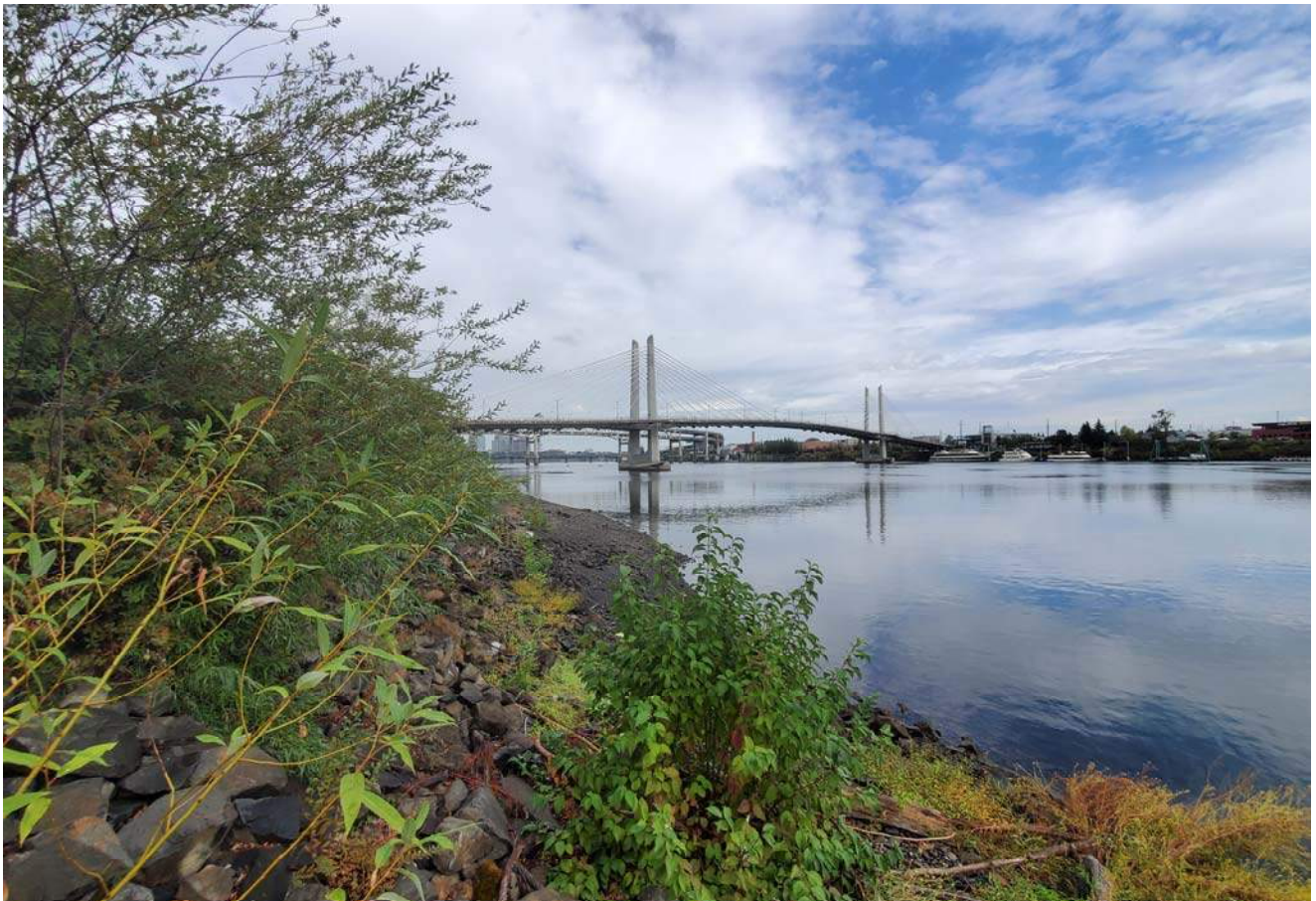
STA: 11+00 - Top of rock armor looking downstream
