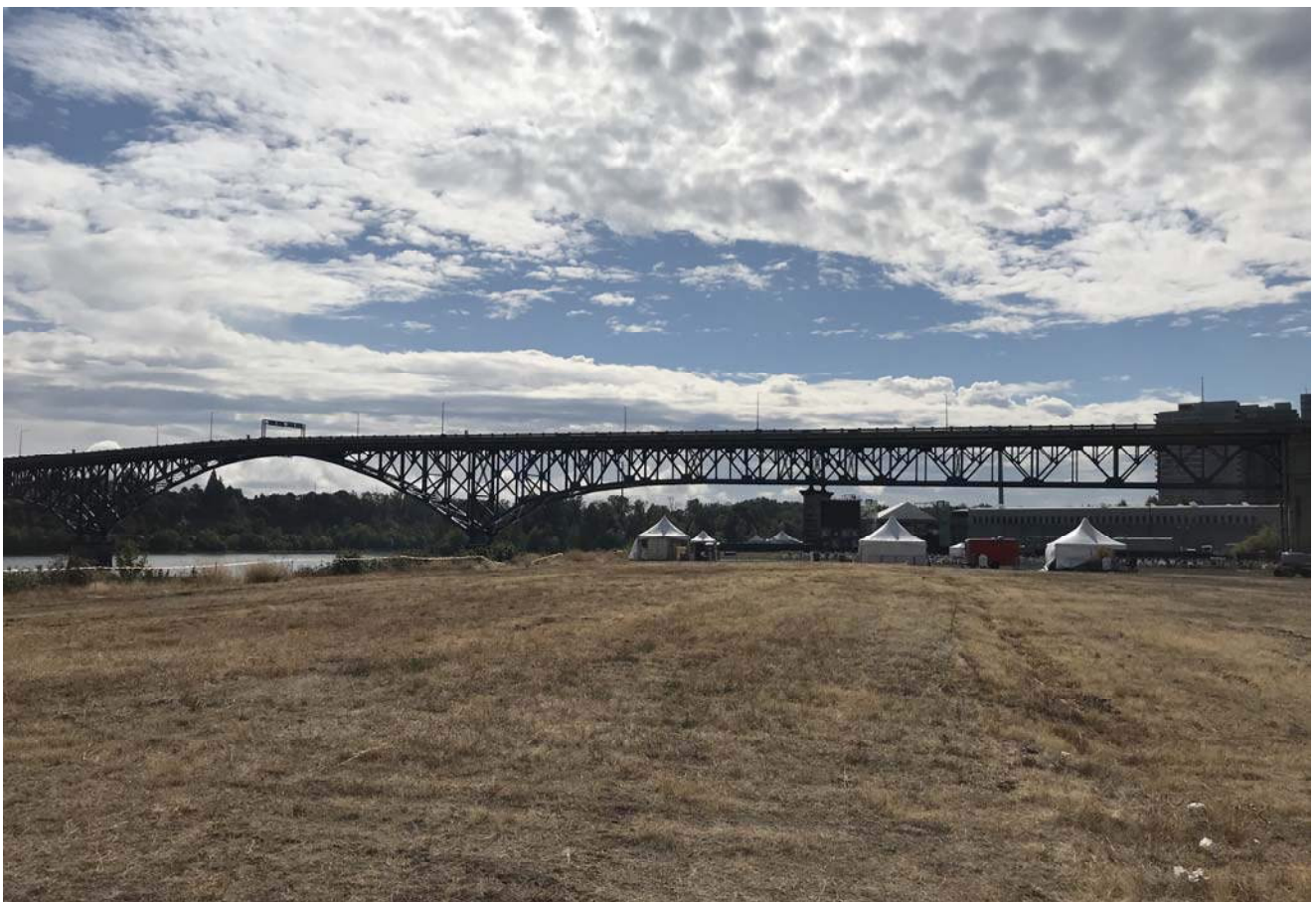
Upland cap, northeast corner looking south
