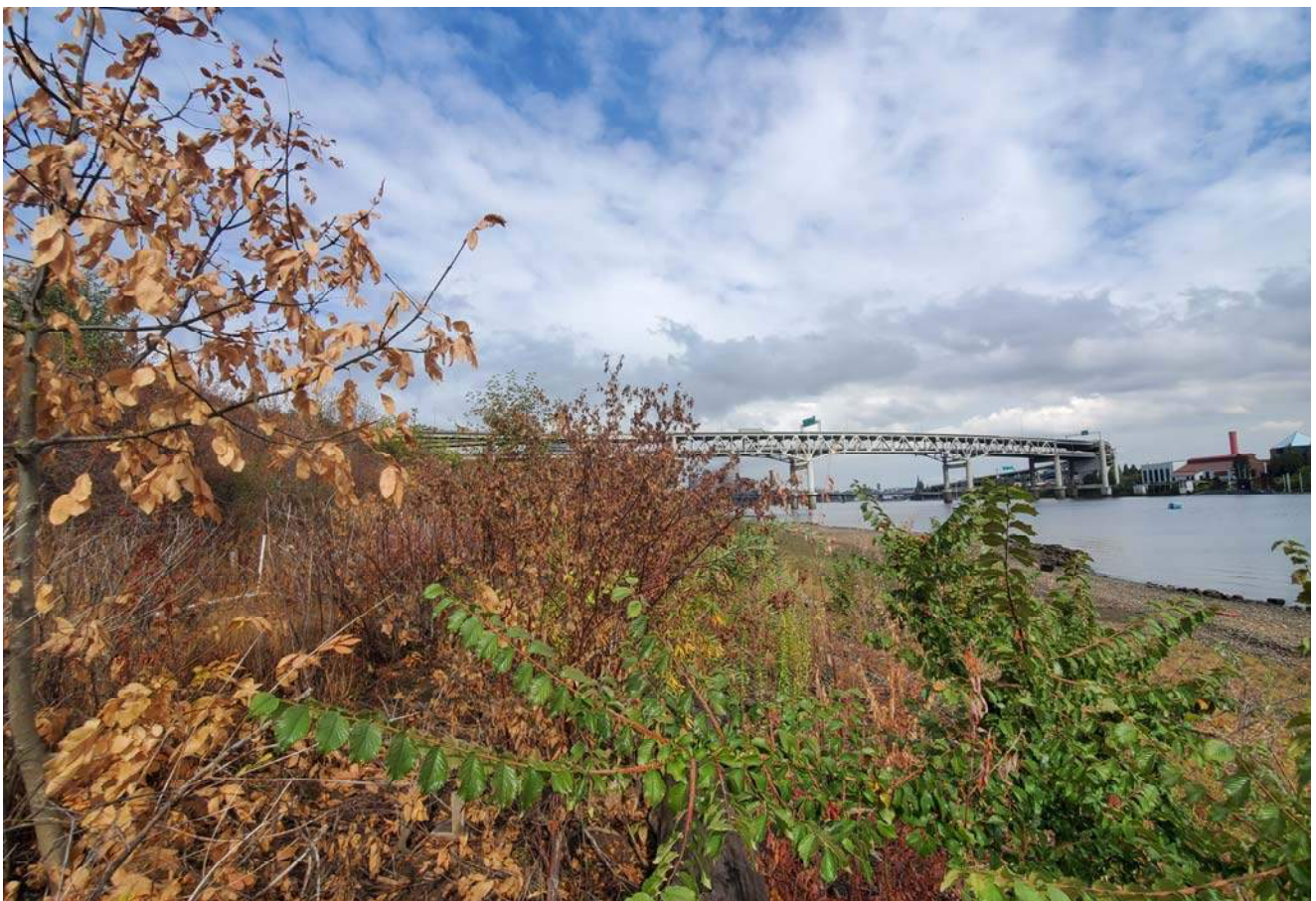
STA: 19+50 - Toe of slope looking downstream
