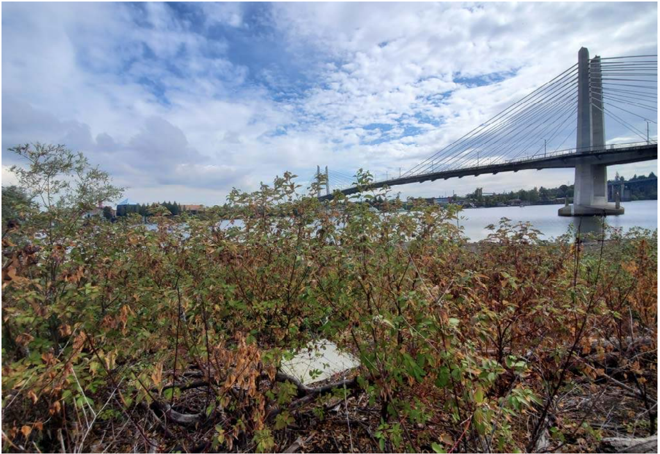
STA: 21+50 - Toe of slope looking east
