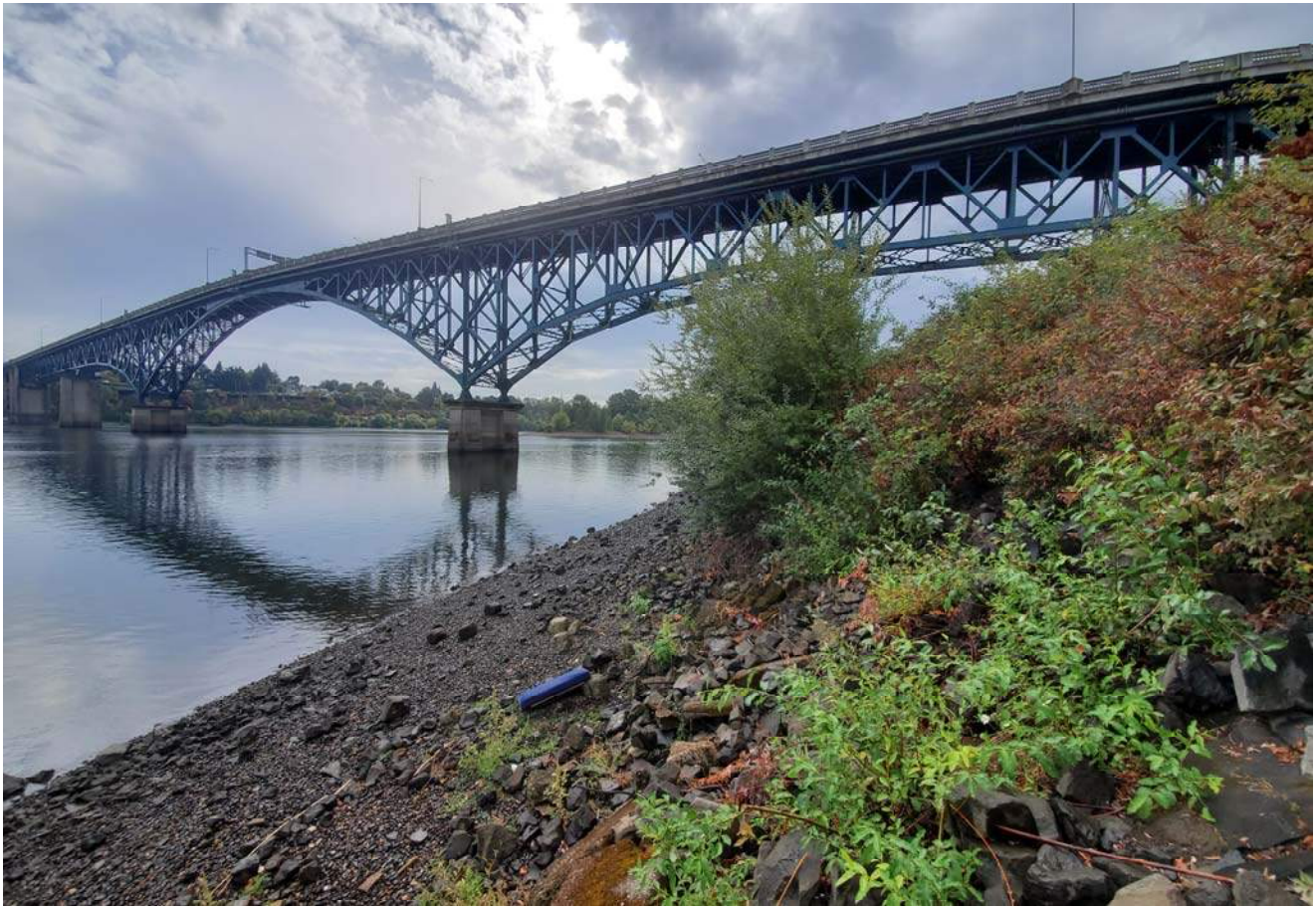
STA: 9+00 - Top of rock armor looking upstream
