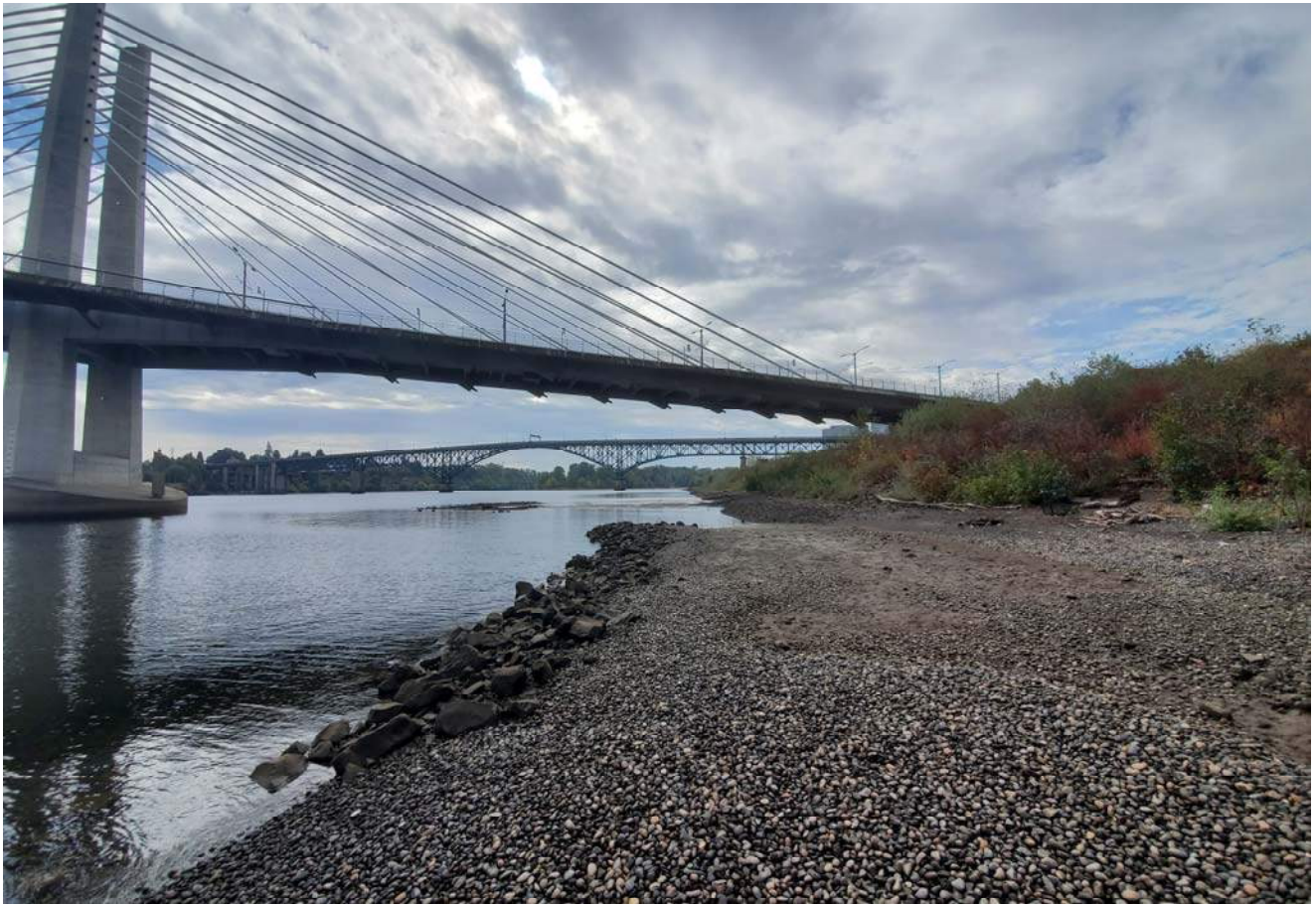
STA: 19+50 - Edge of water looking upstream
