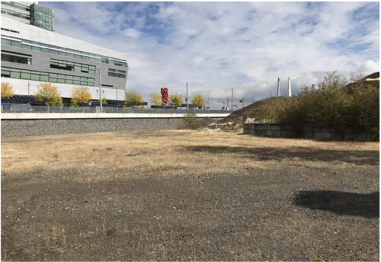
Upland cap, west edge looking northeast
