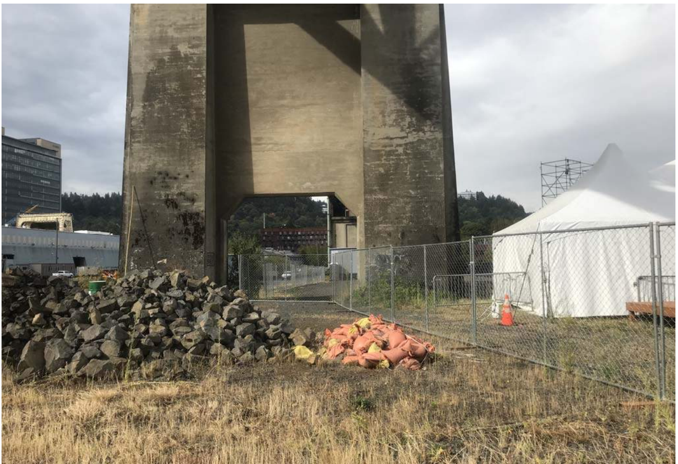
STA: 7+00 - Top of bank looking west
