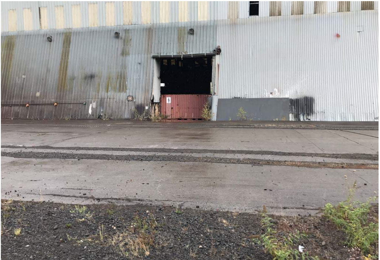
Upland cap, middle barge building looking north
