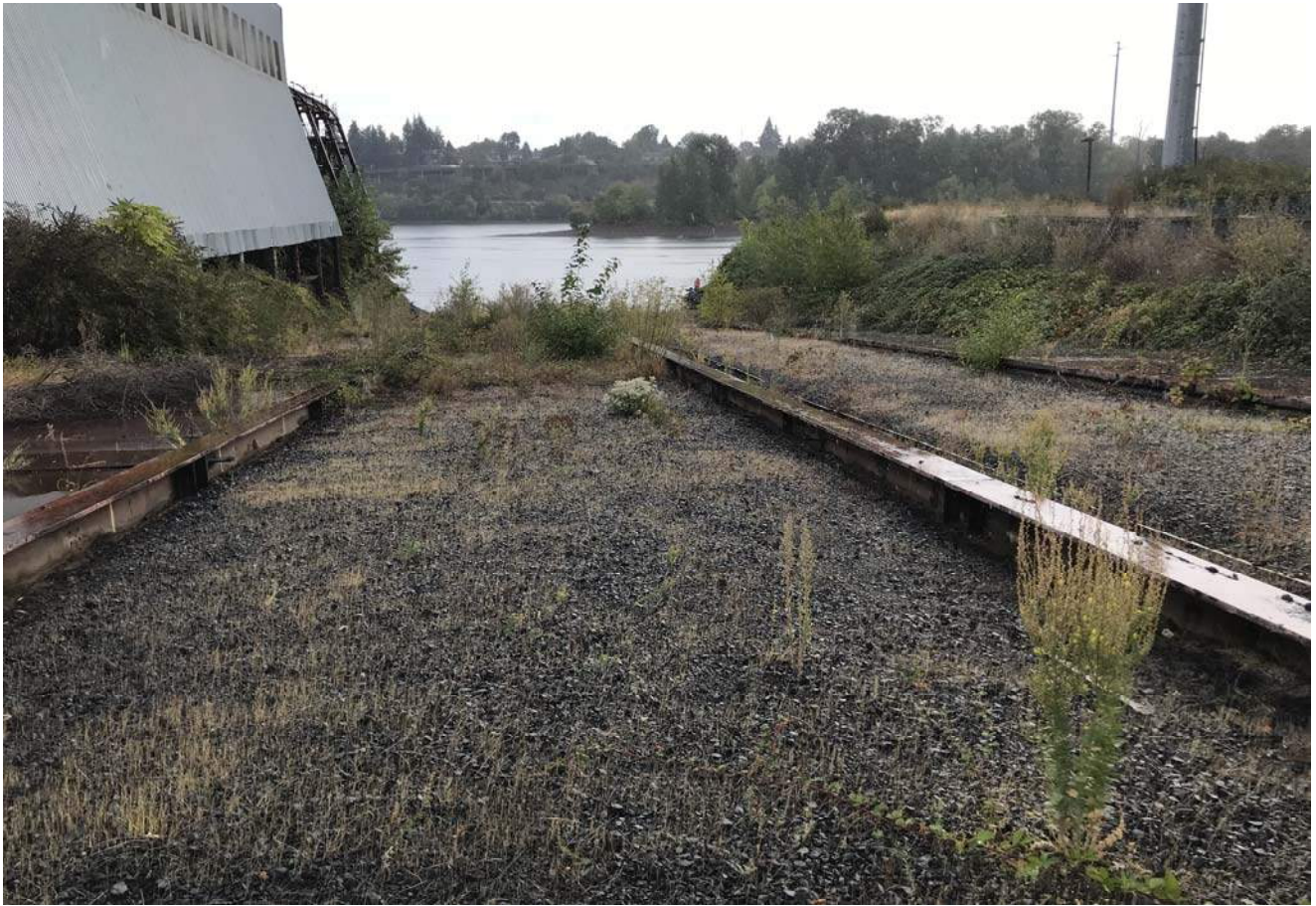
Slipway ramp, looking east
