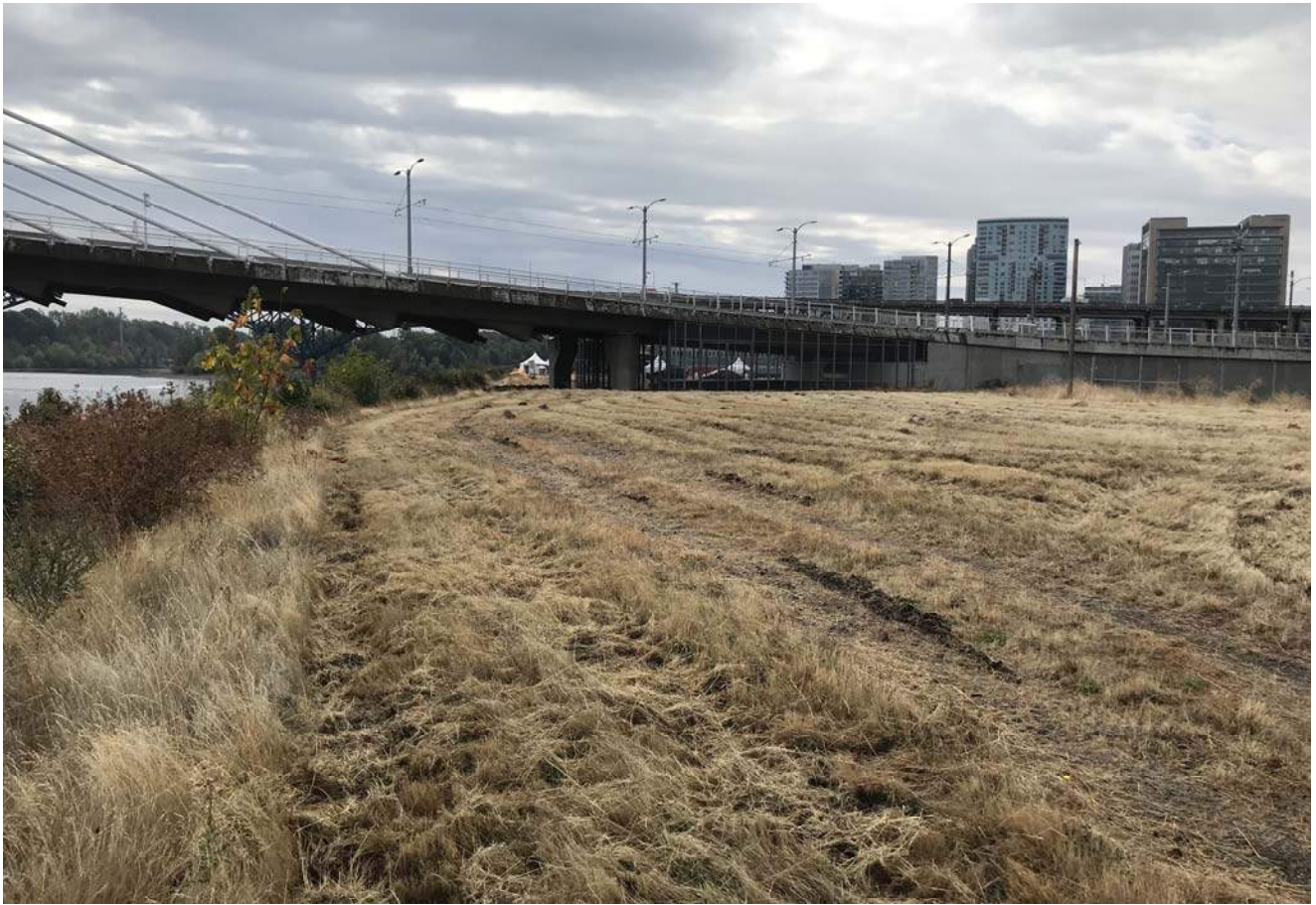
STA: 19+50 - Top of bank looking upstream
