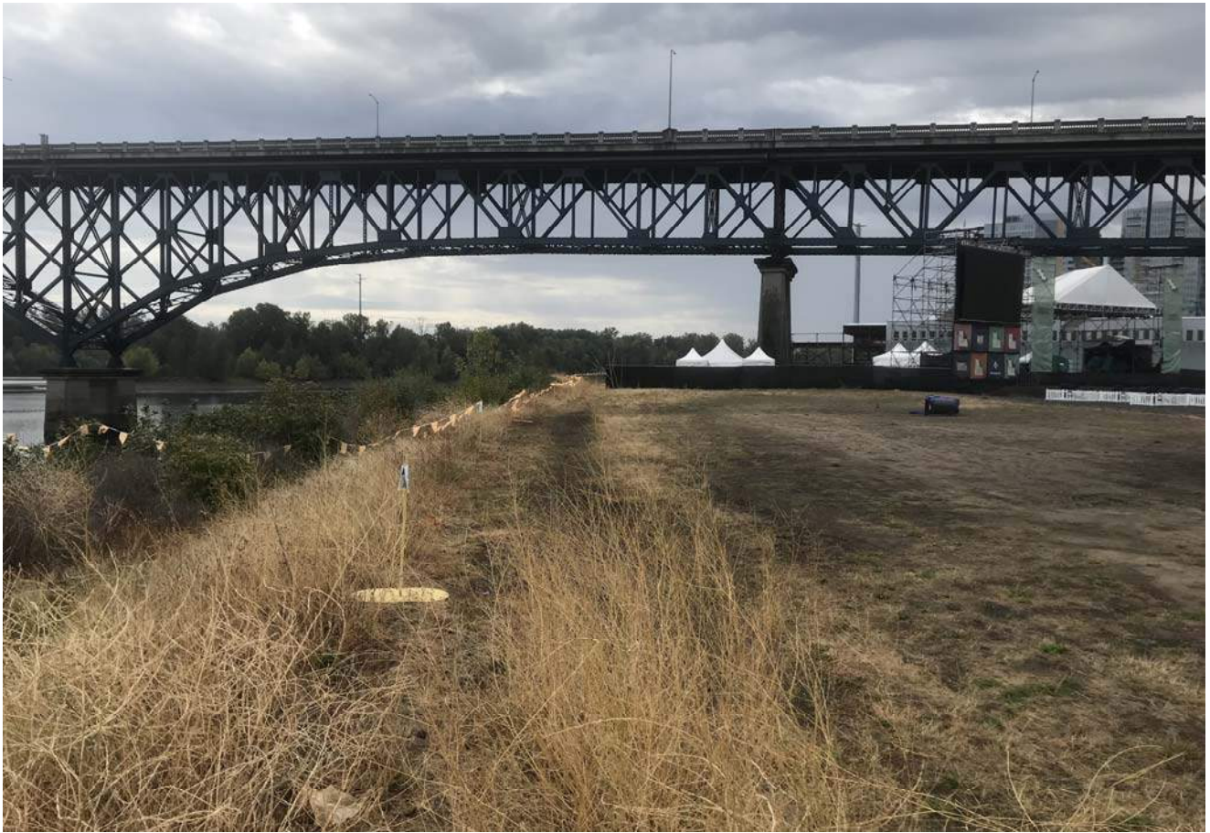
STA: 11+00 - Top of bank looking upstream
