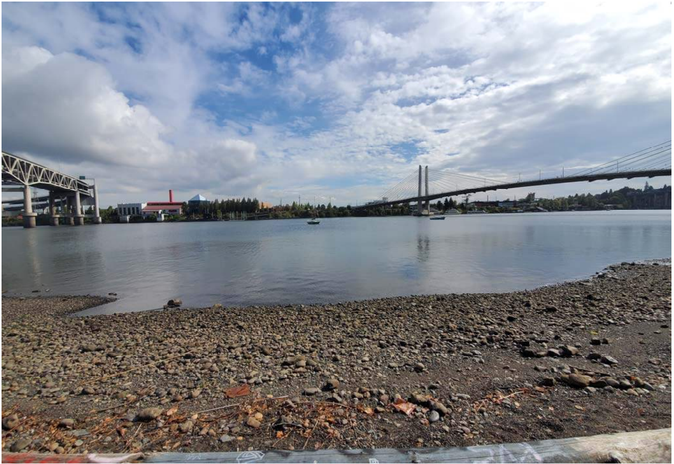
STA: 25+50 - Toe of slope looking east
