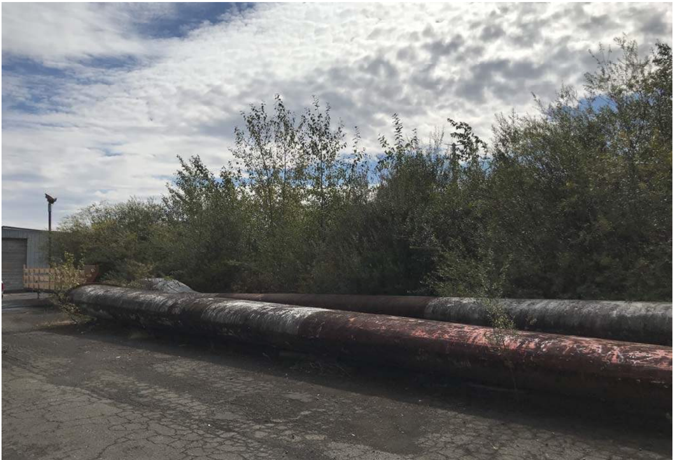
Infiltration facility, north edge looking southeast
