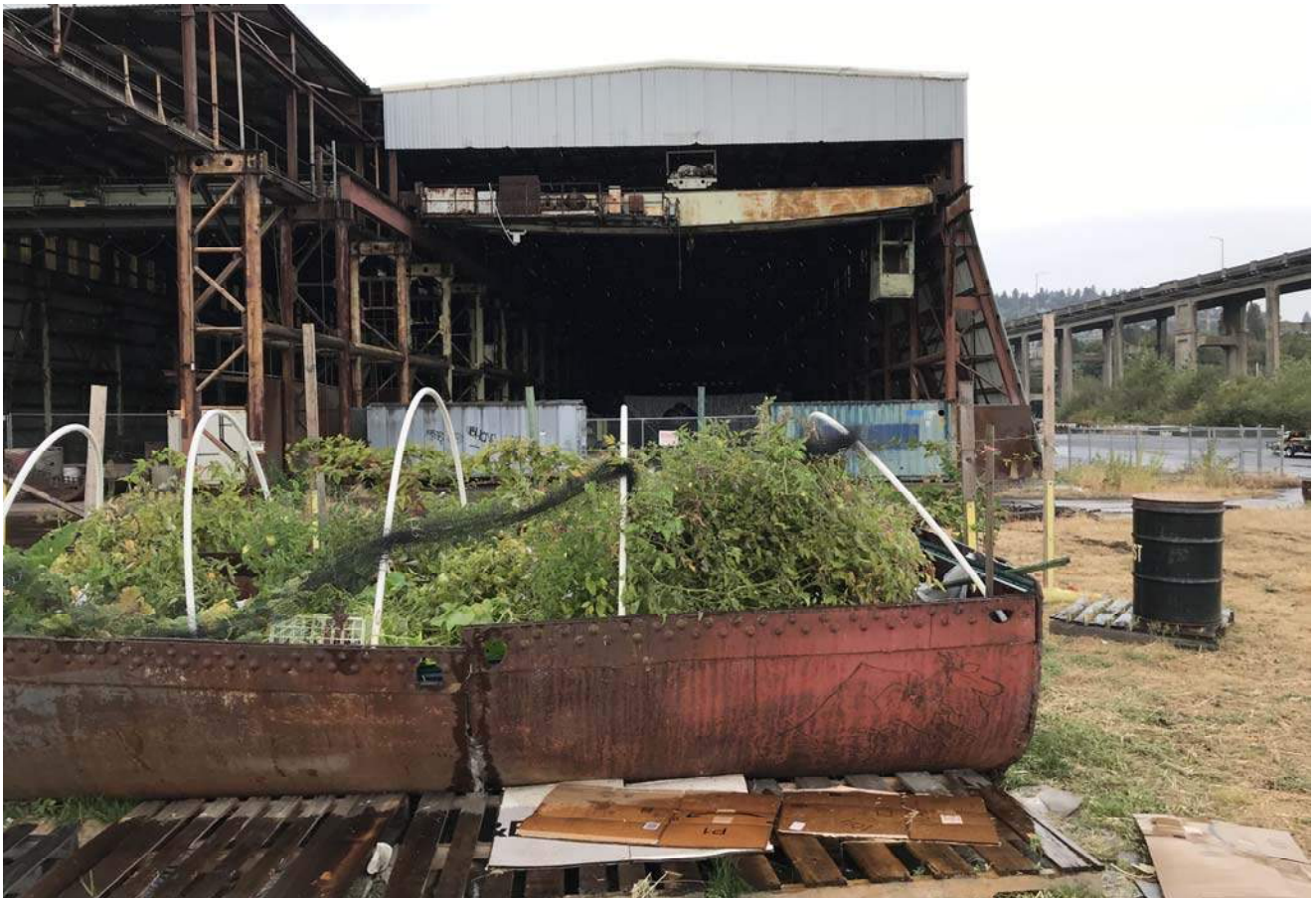
STA: 3+00 - Top of bank looking west
