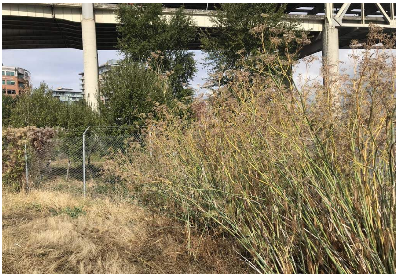
STA: 26+50 - Top of bank looking downstream
