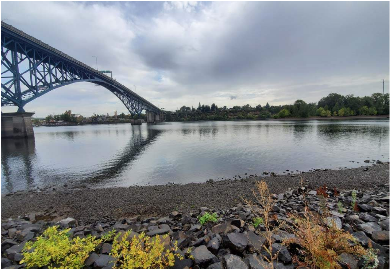
STA: 5+00 - Top of rock armor looking east
