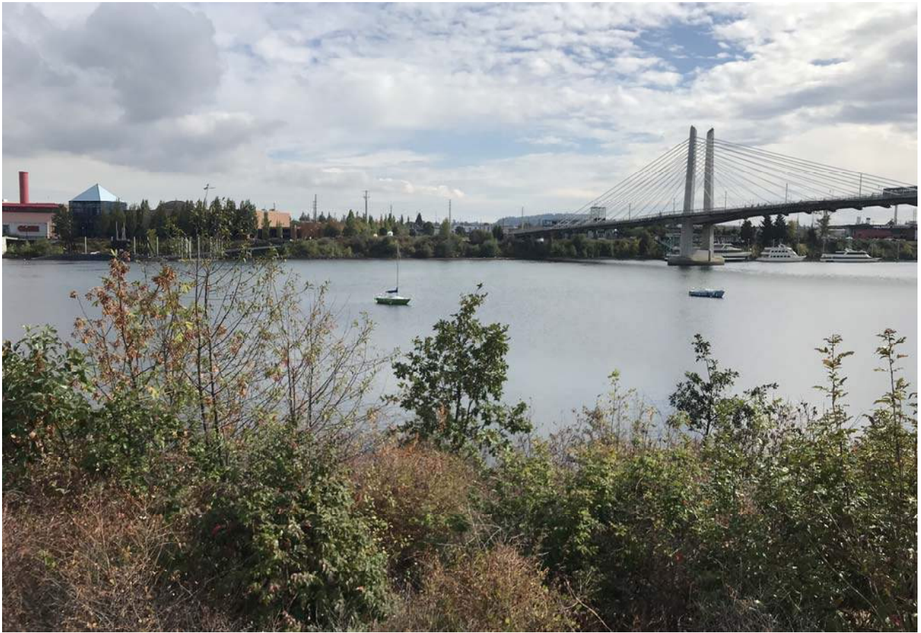
STA: 25+50 - Top of bank looking east
