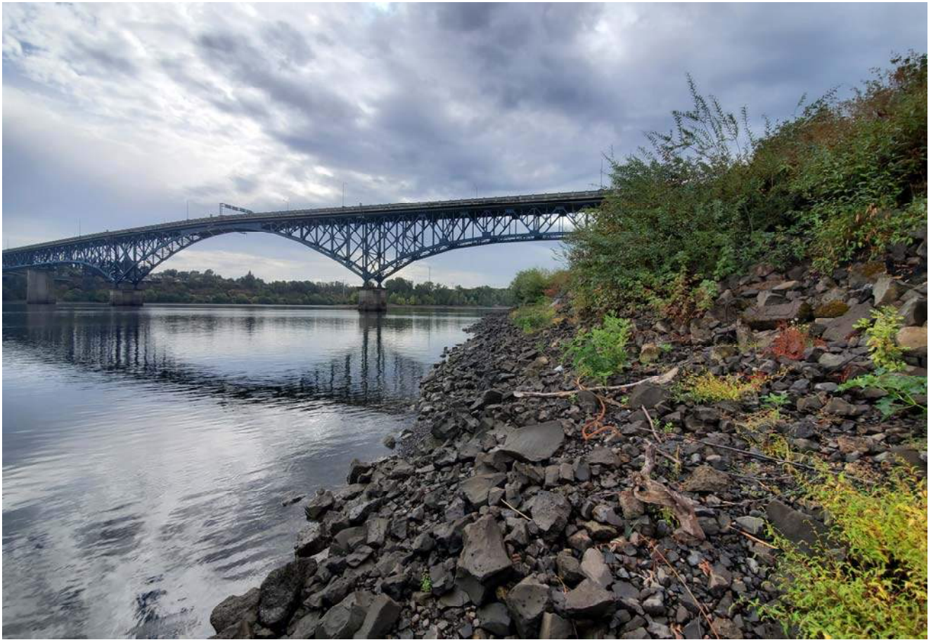
STA: 11+00 - Toe of slope looking upstream
