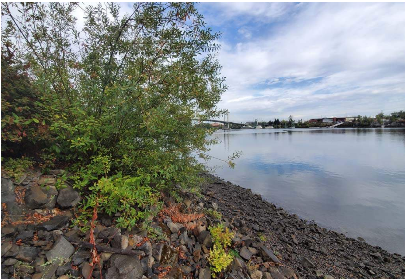
STA: 9+00 - Top of rock armor looking downstream
