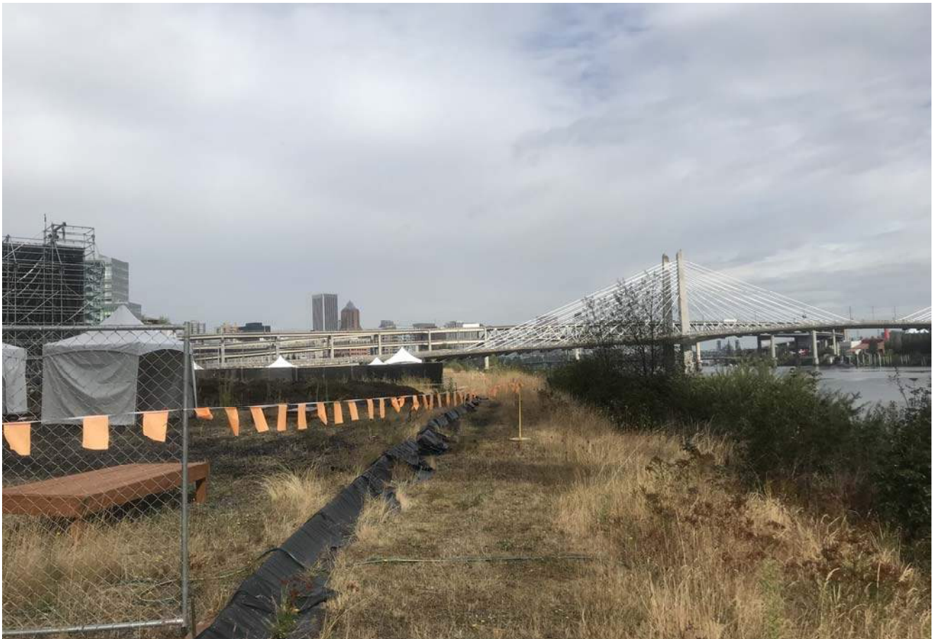
STA: 7+00 - Top of bank looking downstream
