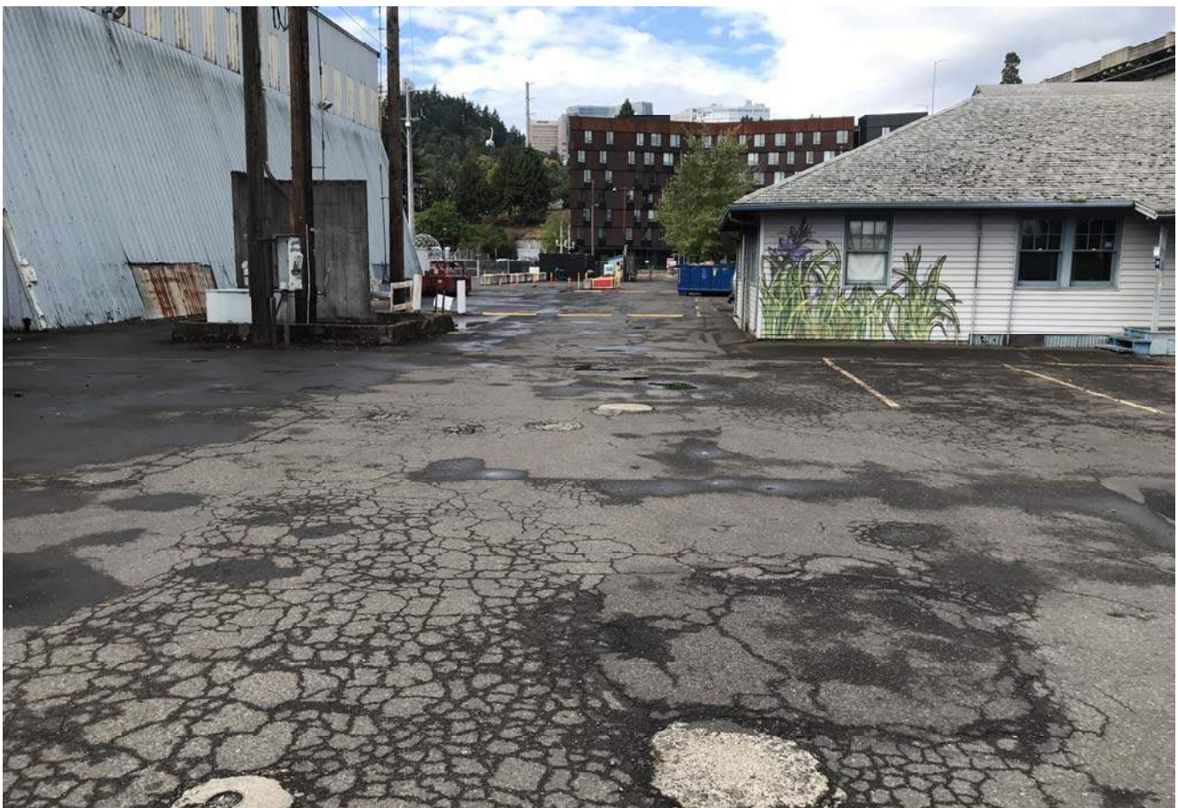
Operational area between barge building and office building, looking west
