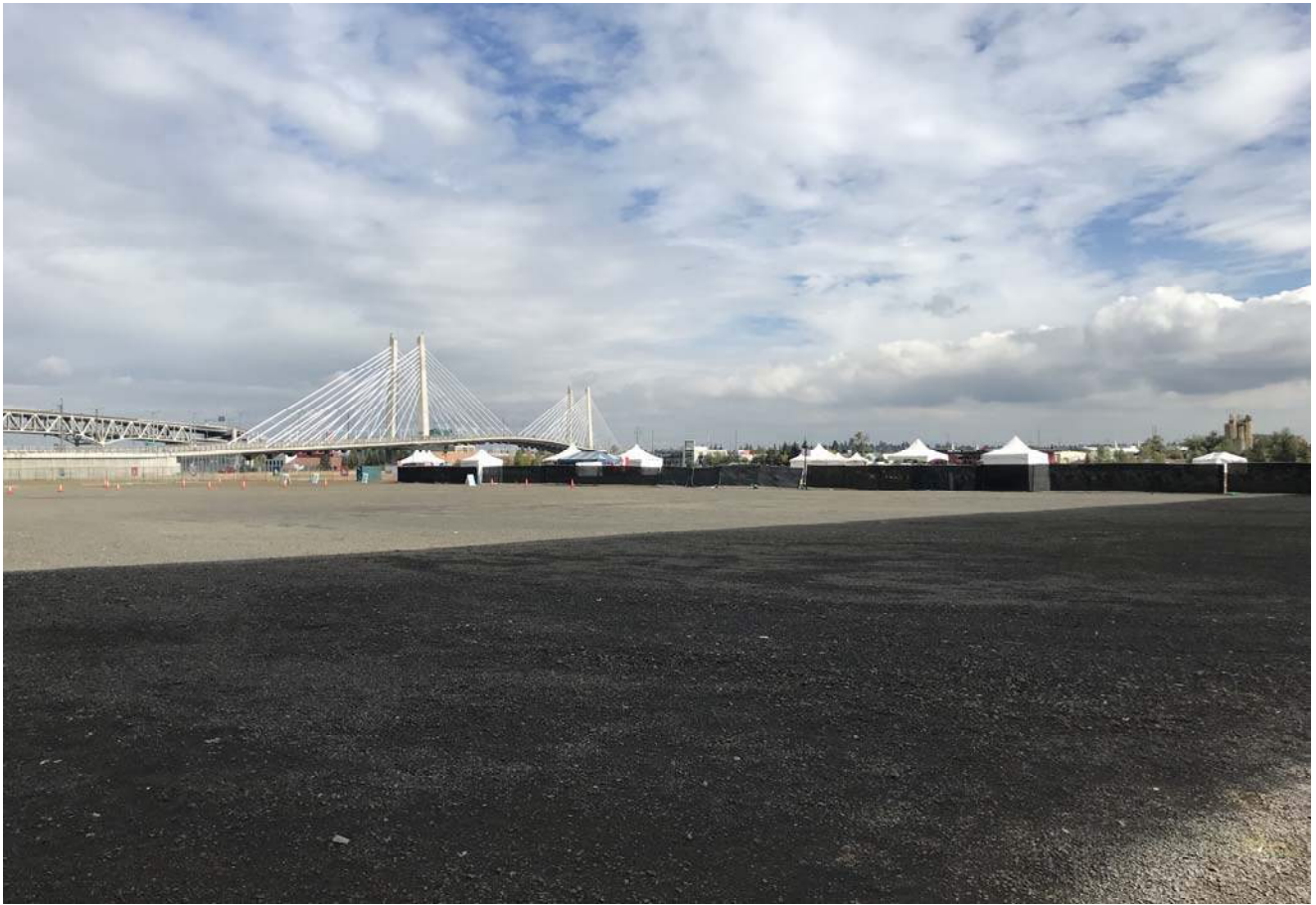
Upland cap, Ross Island Bridge northwest corner looking northeast
