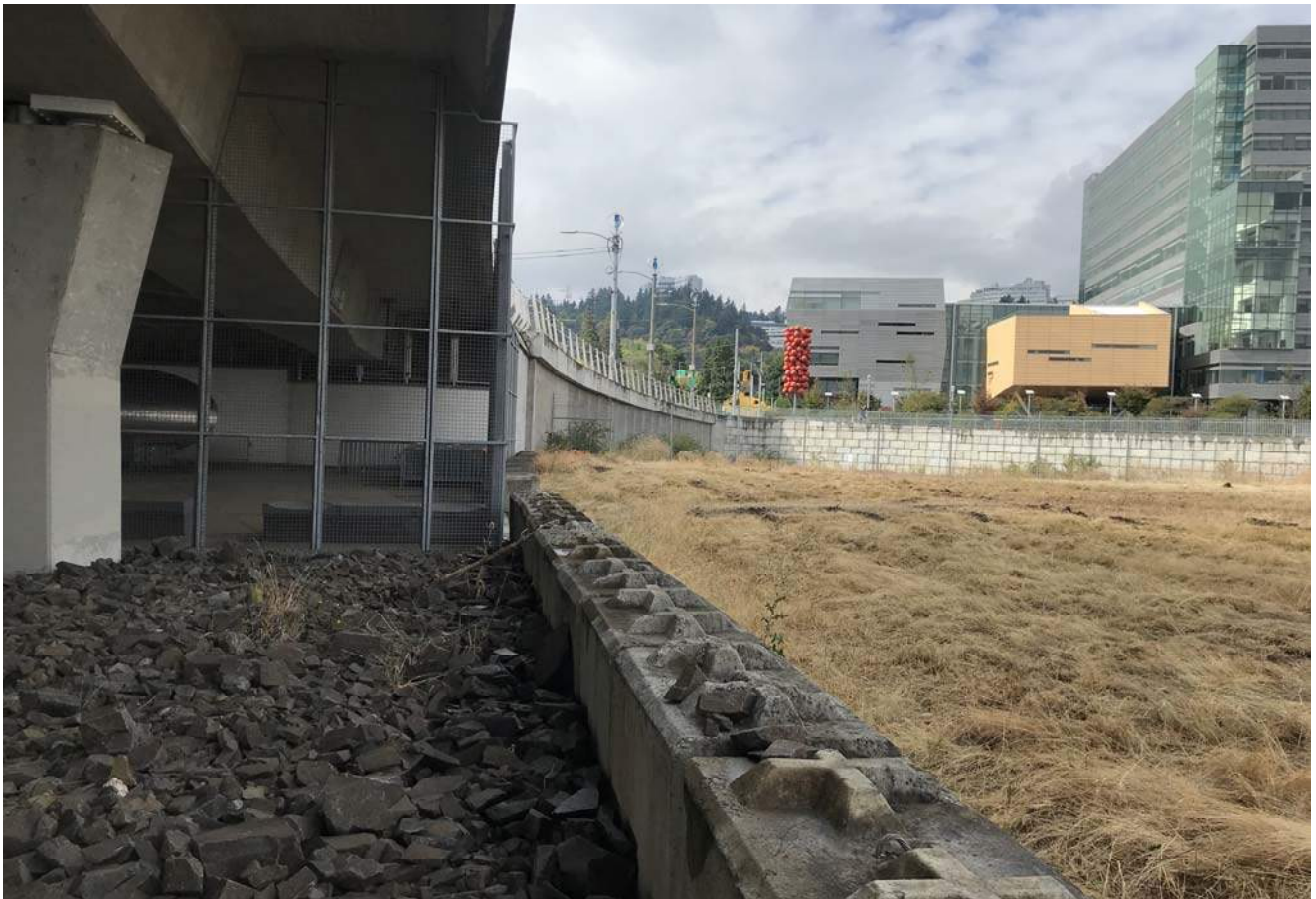
STA: 17+00 - Top of bank looking west
