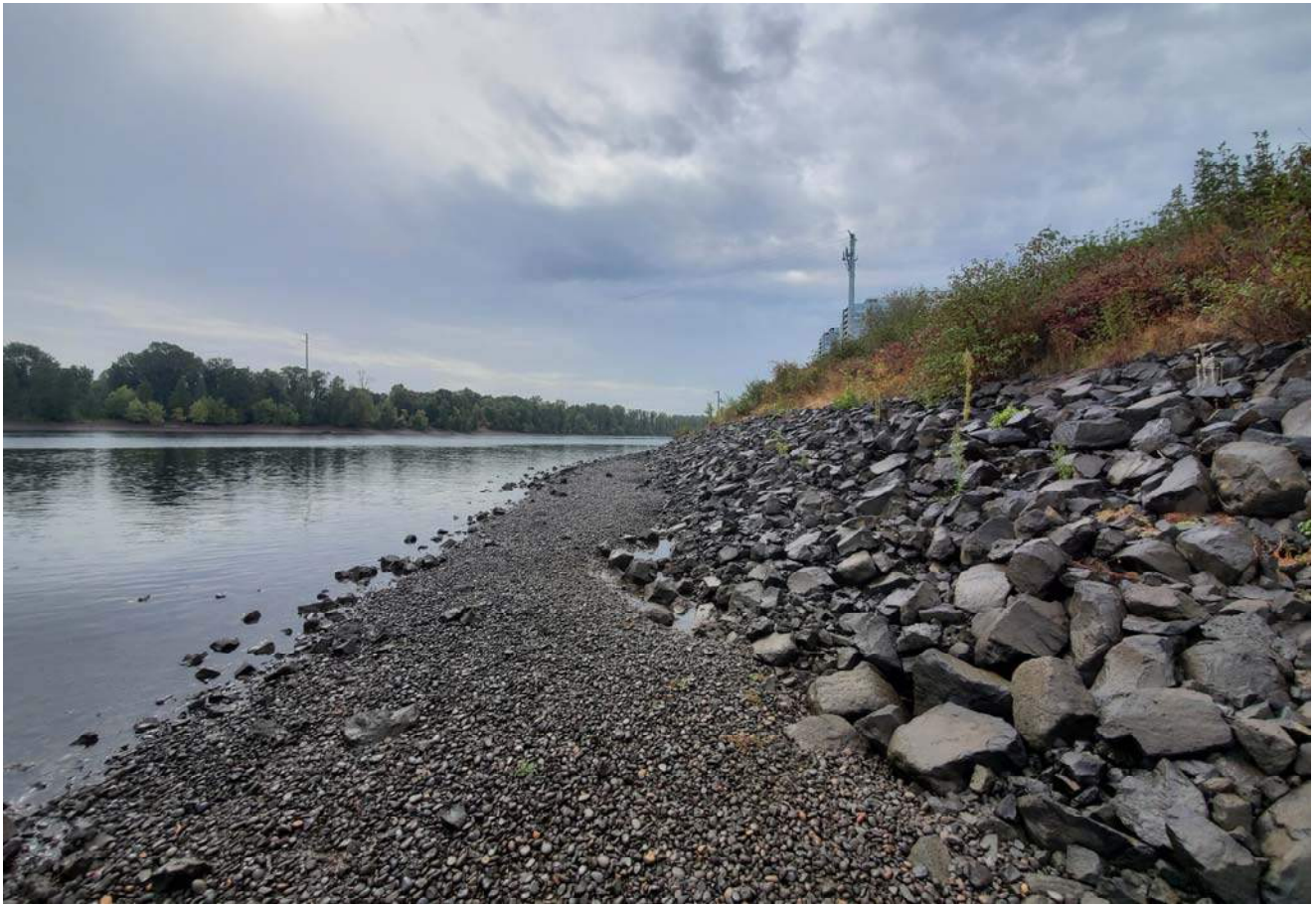
STA: 5+00 - Toe of slope looking upstream
