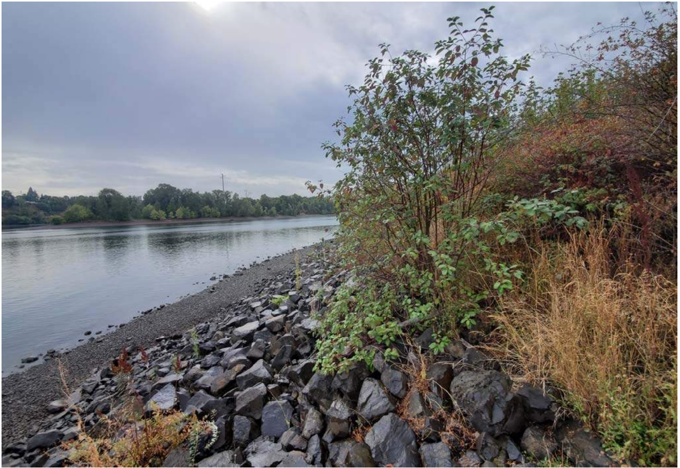
STA: 5+00 - Top of rock armor looking upstream
