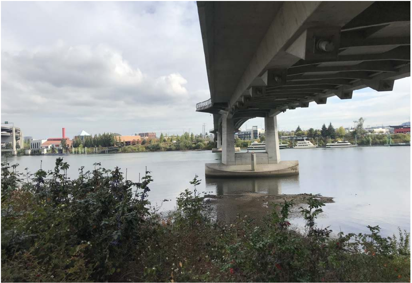
STA: 17+00 - Top of bank looking east
