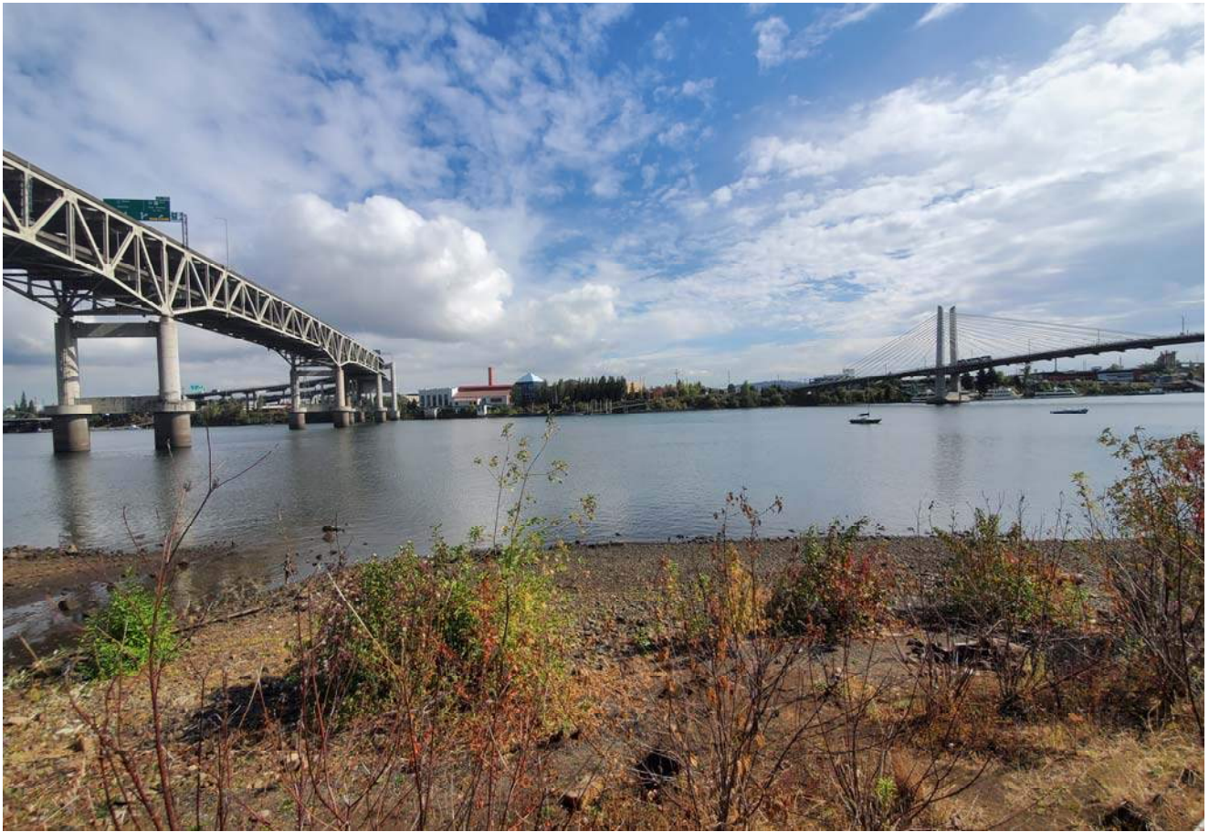
STA: 26+50 - Toe of slope looking east
