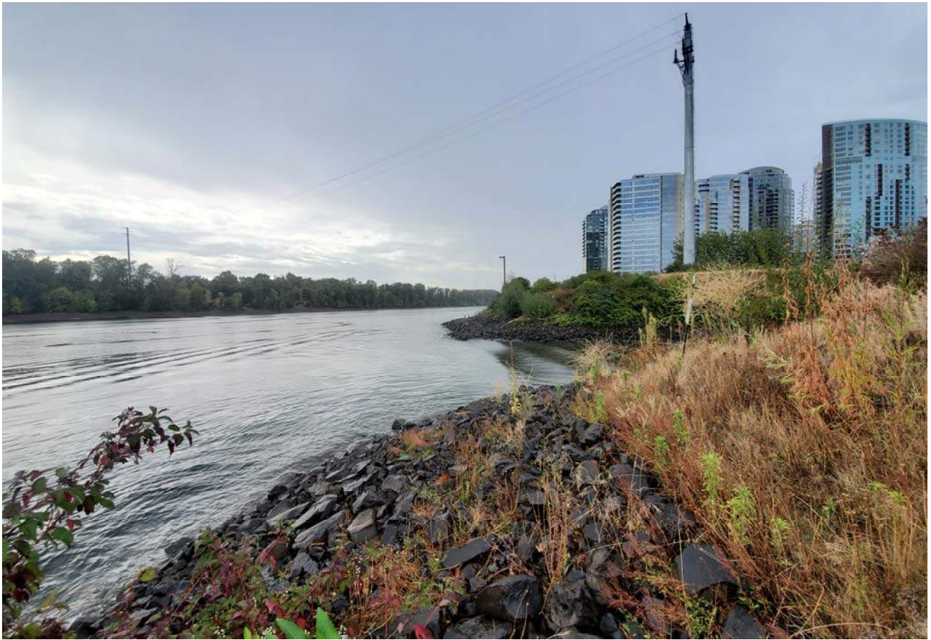
STA: 3+00 - Top of rock armor looking upstream
