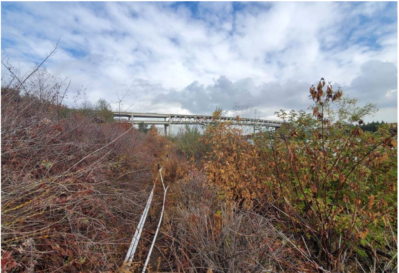
STA: 21+50 - Toe of slope looking downstream
