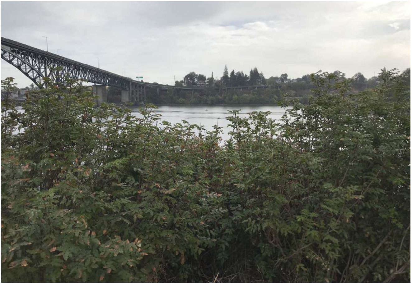
STA: 3+00 - Top of bank looking east
