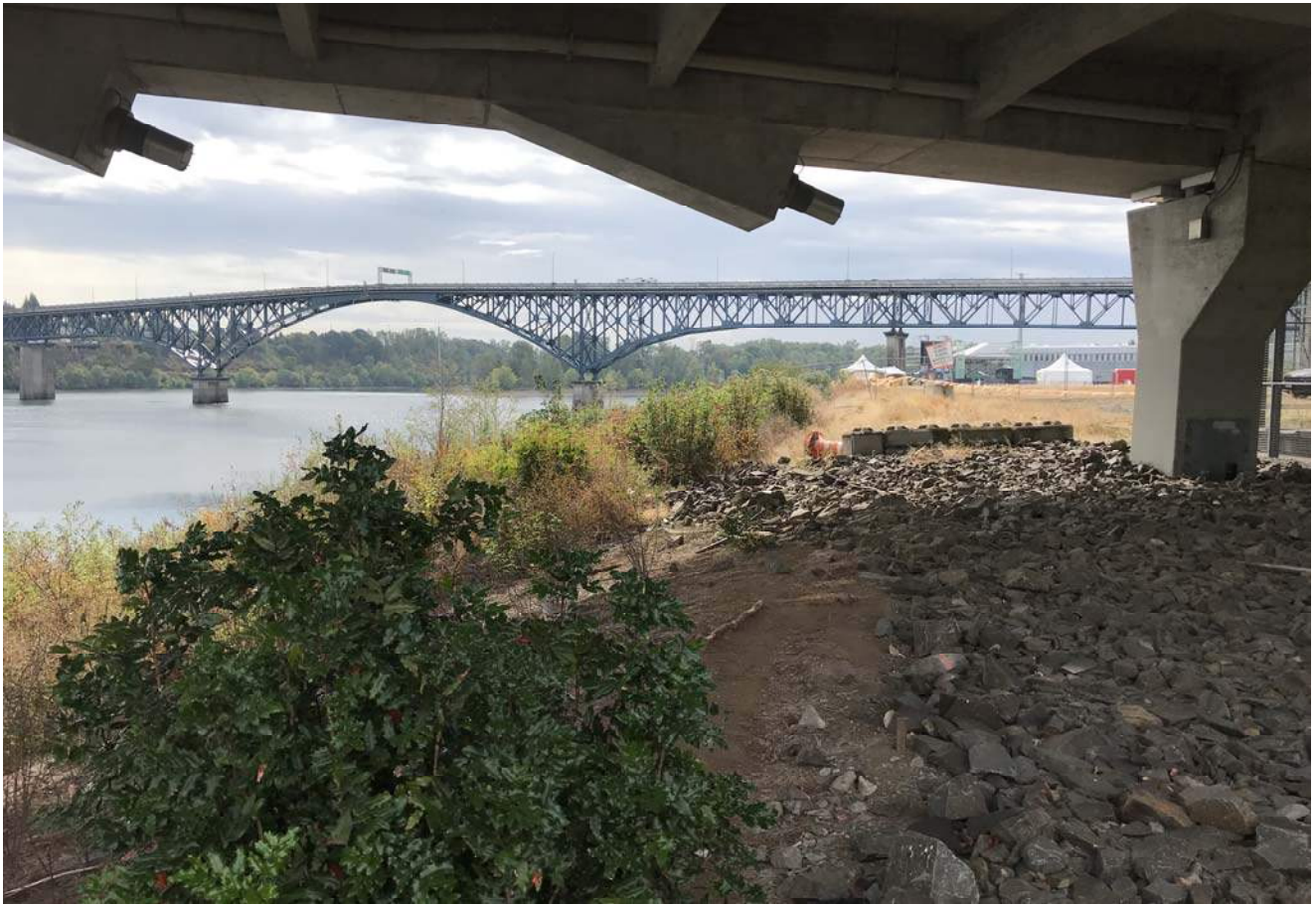
STA: 17+00 - Top of bank looking upstream
