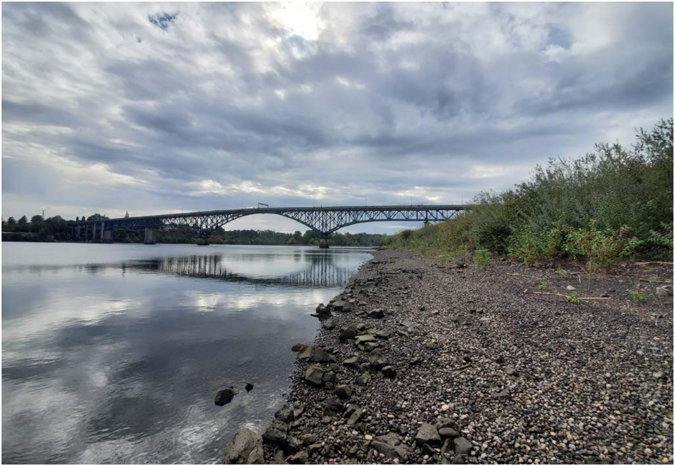
STA: 15+00 - Edge of water looking upstream
