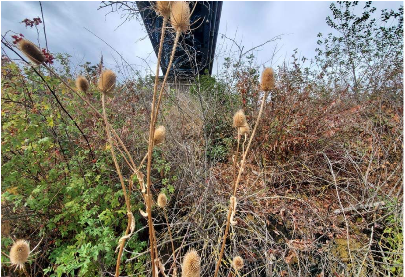
STA: 7+00 - Top of rock armor looking west
