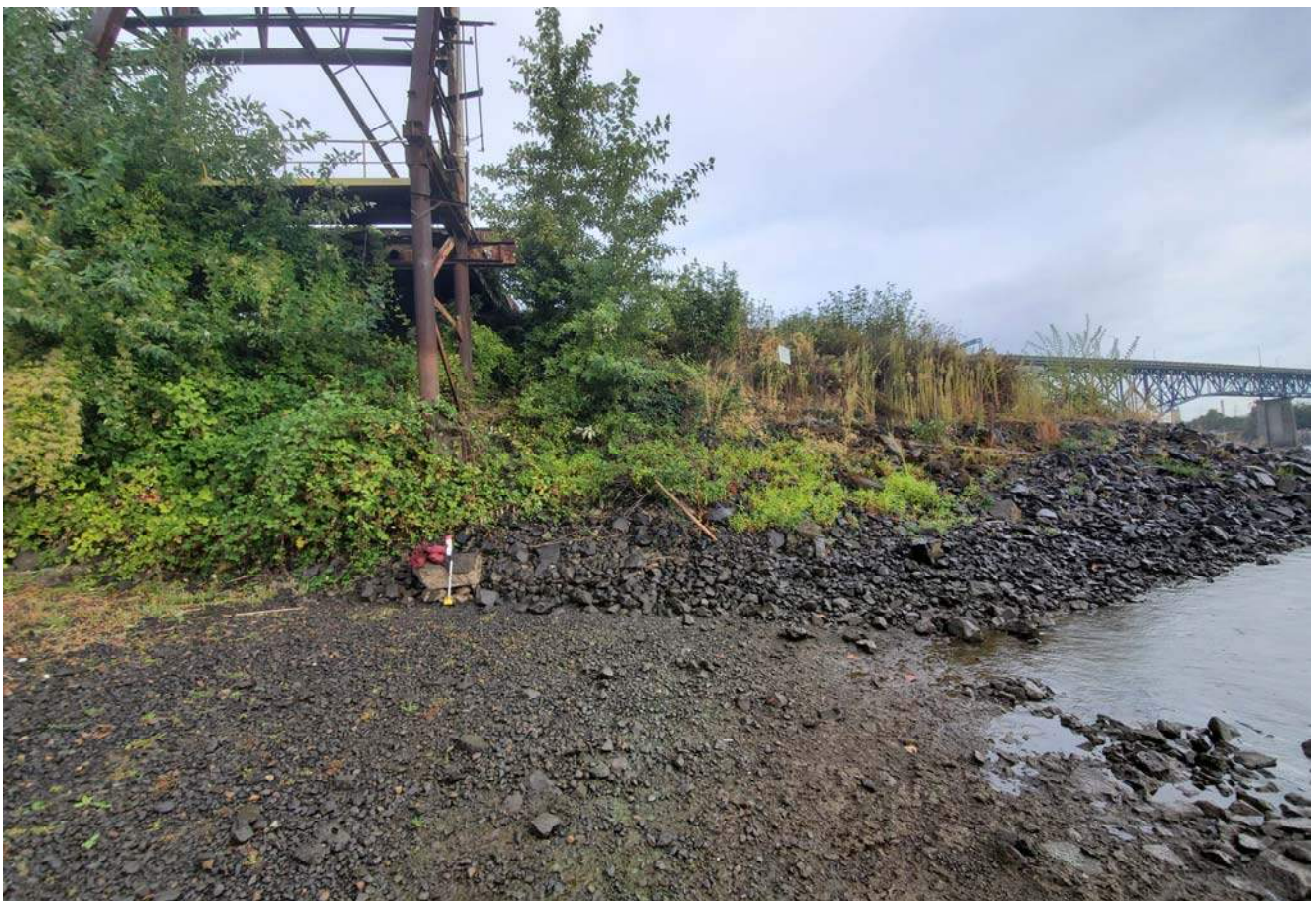
Lower slipway ramp, looking downstream
