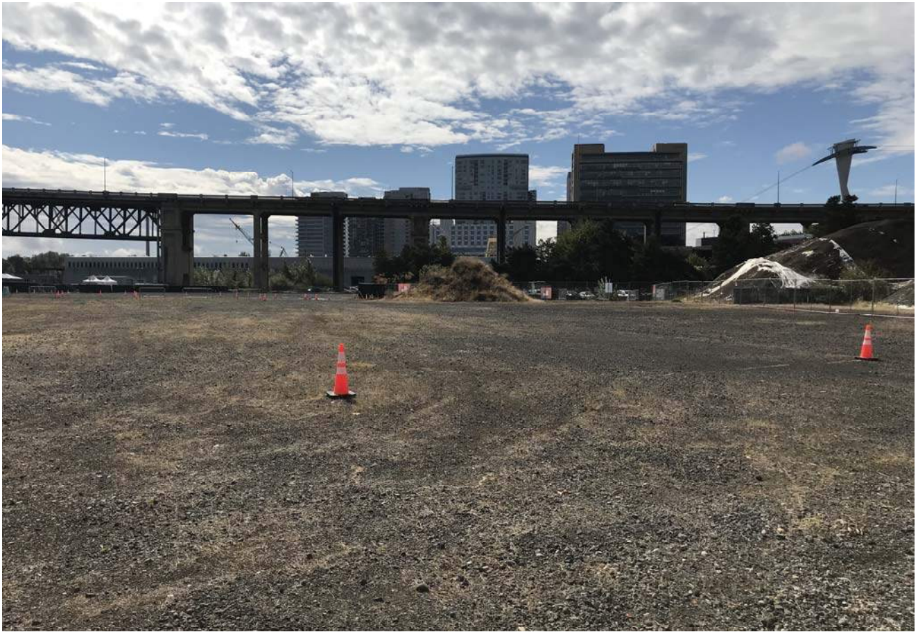
Upland cap, north edge looking south
