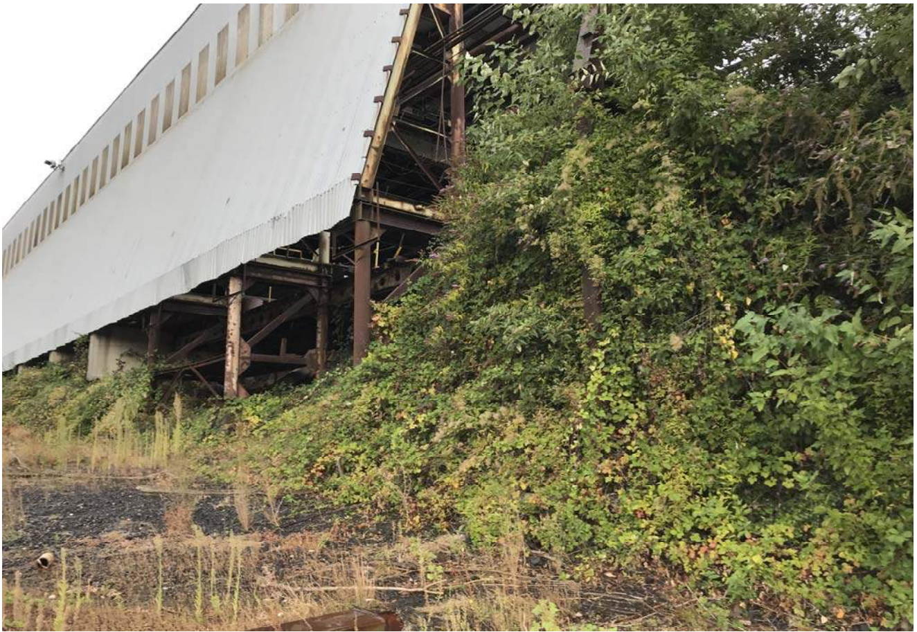
Slipway ramp, looking northwest
