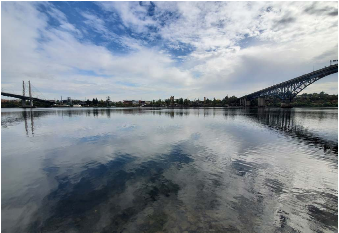
STA: 11+00 - Toe of slope looking east
