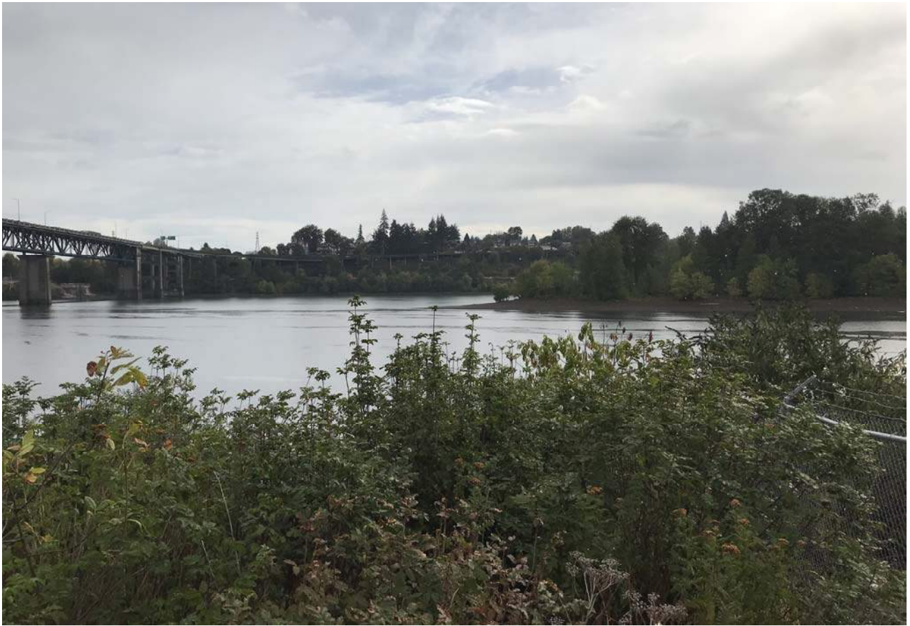
STA: 0+00 - Top of bank looking east
