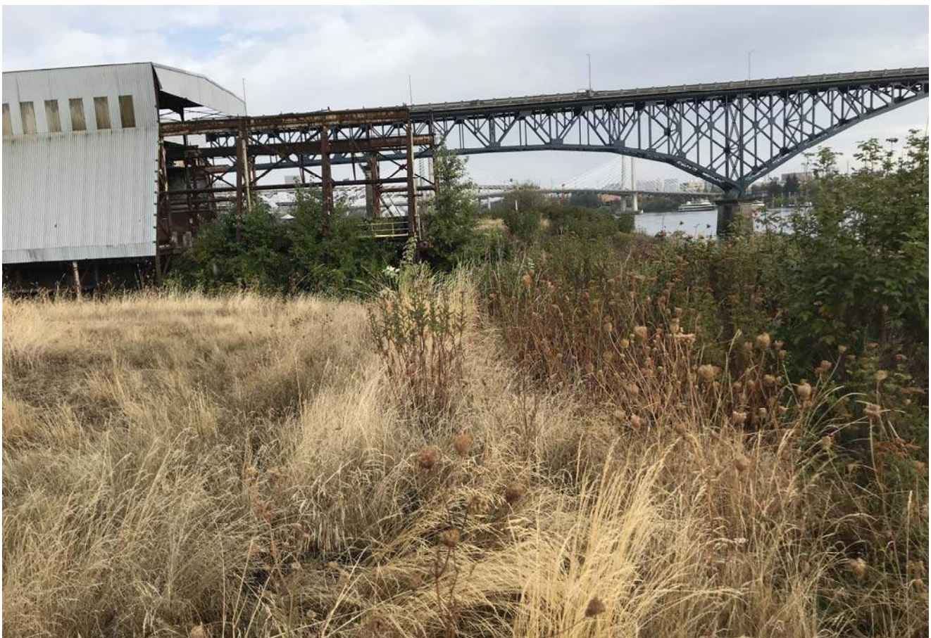
STA: 0+00 - Top of bank looking downstream
