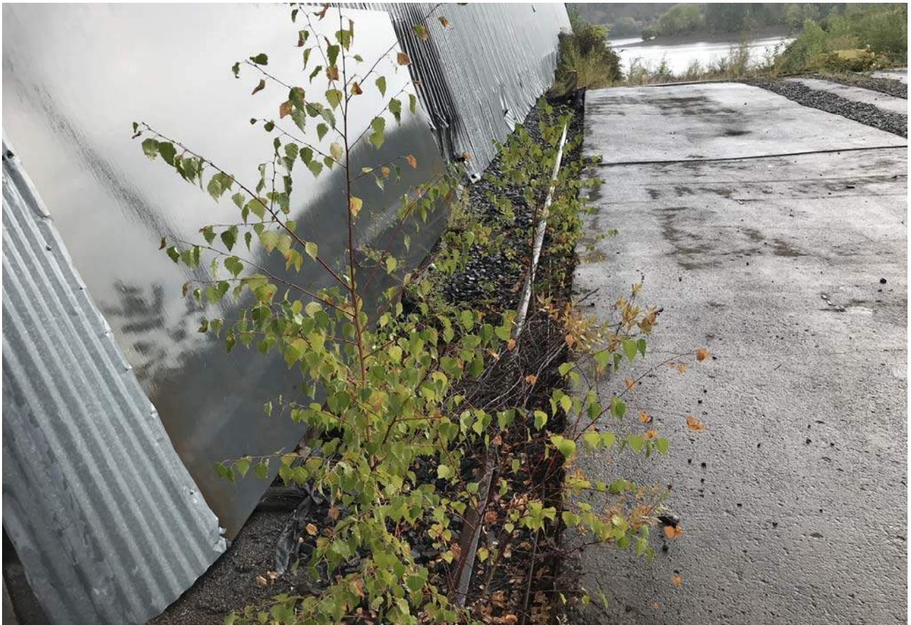
Upland, south face of barge building looking east
