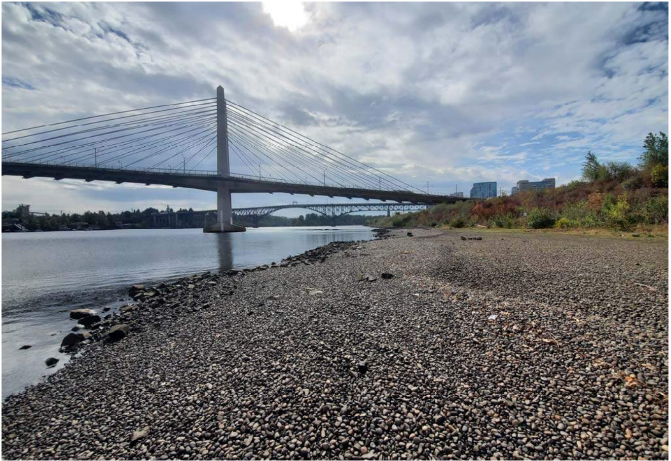
STA: 21+50 - Edge of water looking upstream
