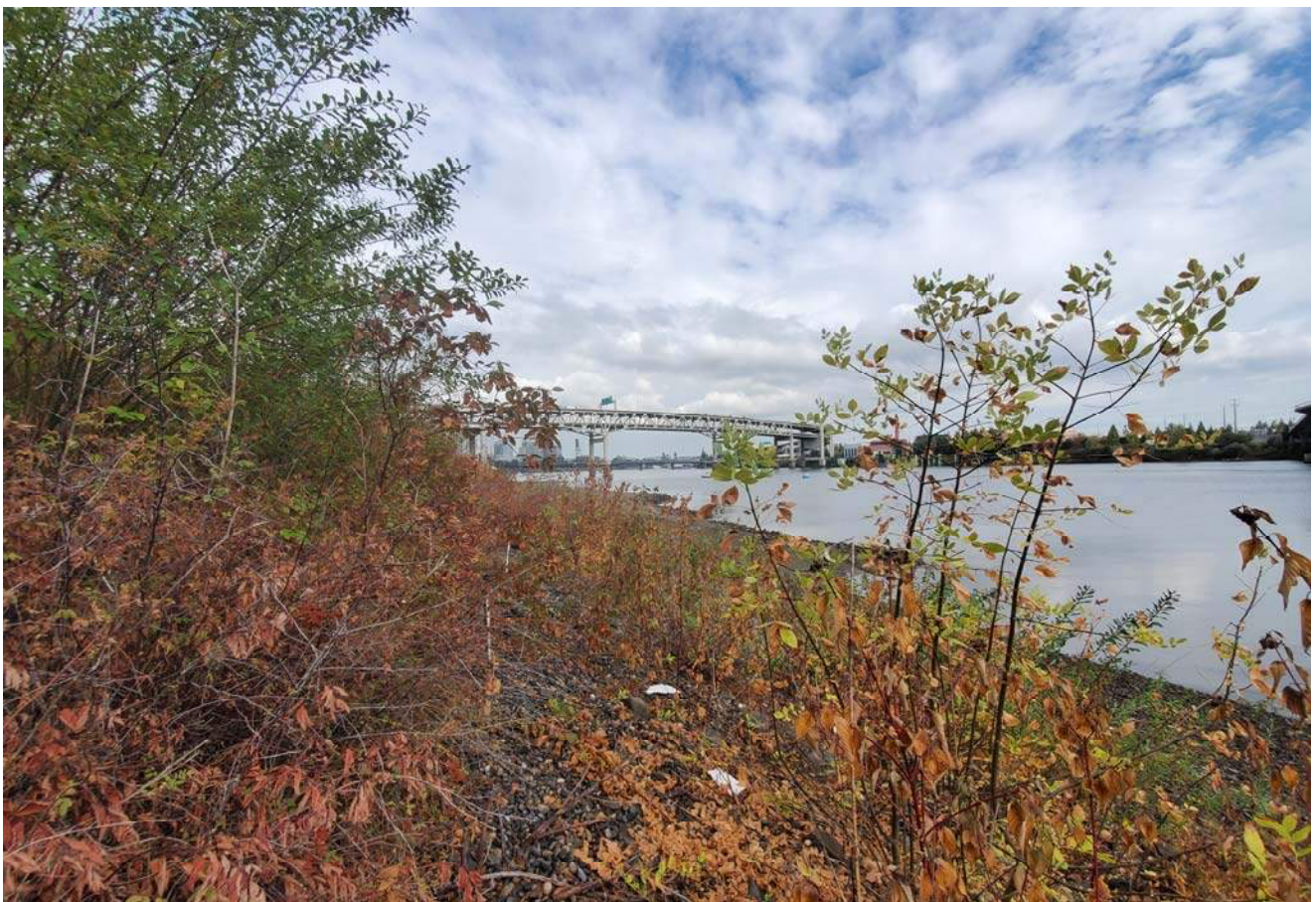
STA: 17+00 - Toe of slope looking downstream
