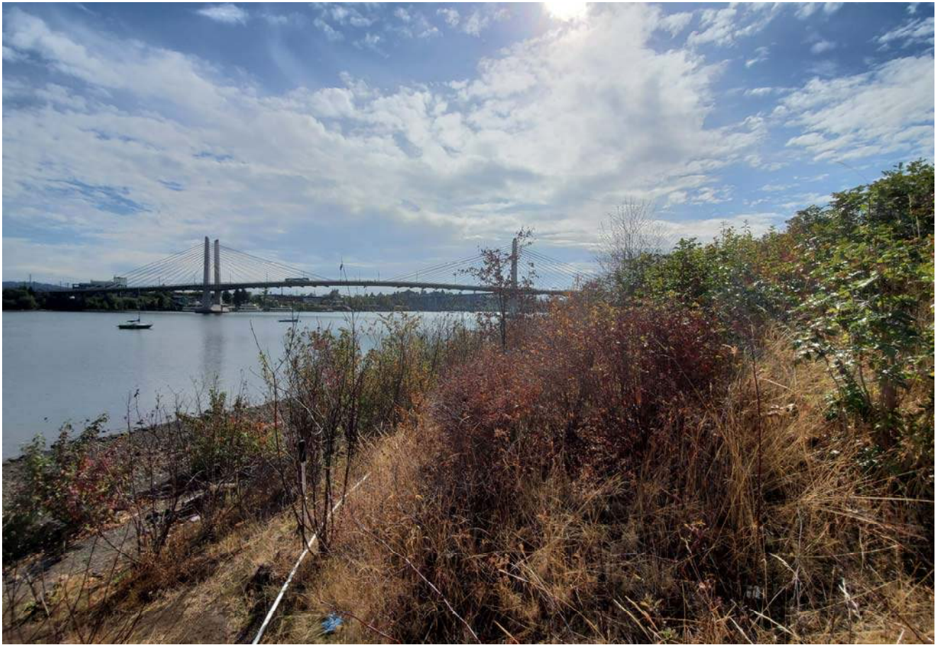
STA: 26+50 - Toe of slope looking upstream
