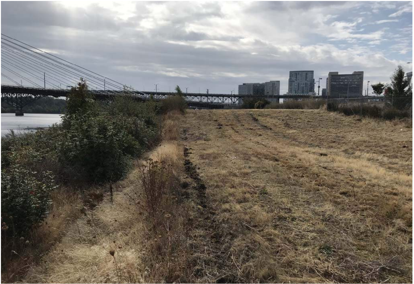
STA: 23+50 - Top of bank looking upstream
