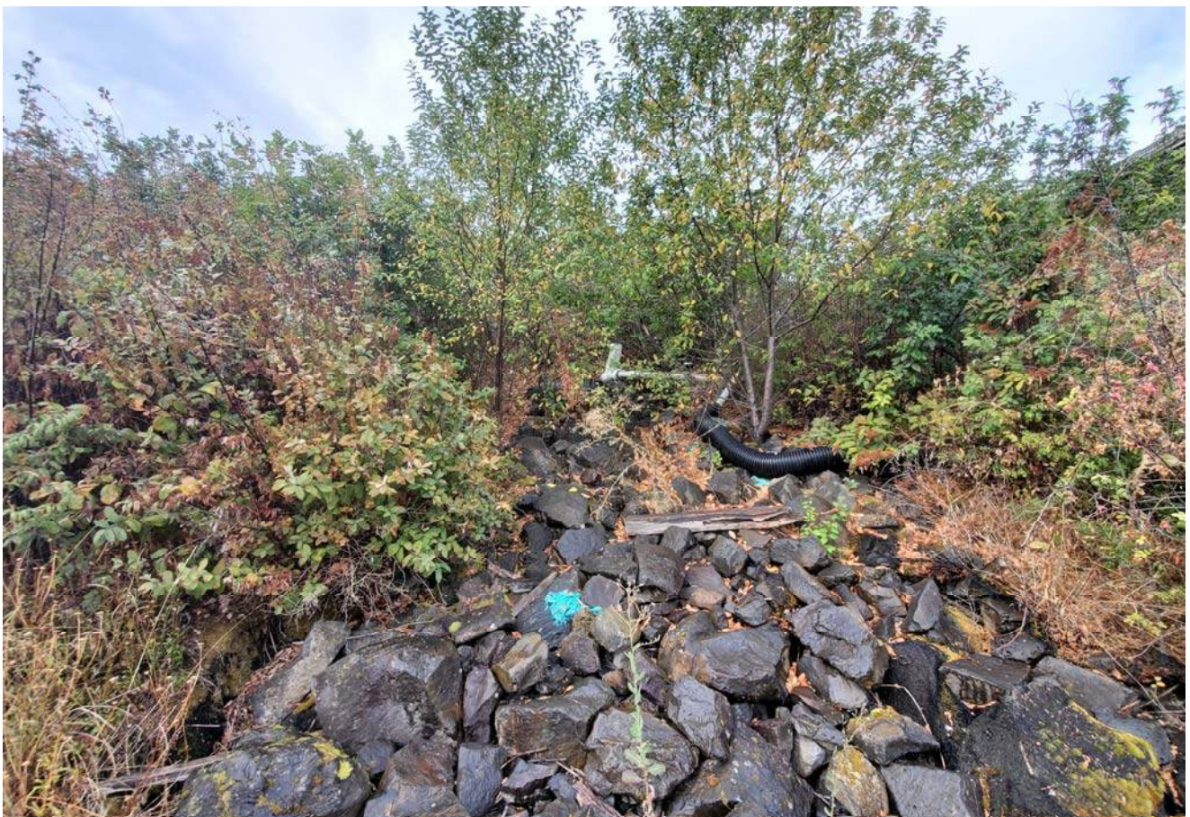
STA: 5+00 - Top of rock armor looking west
