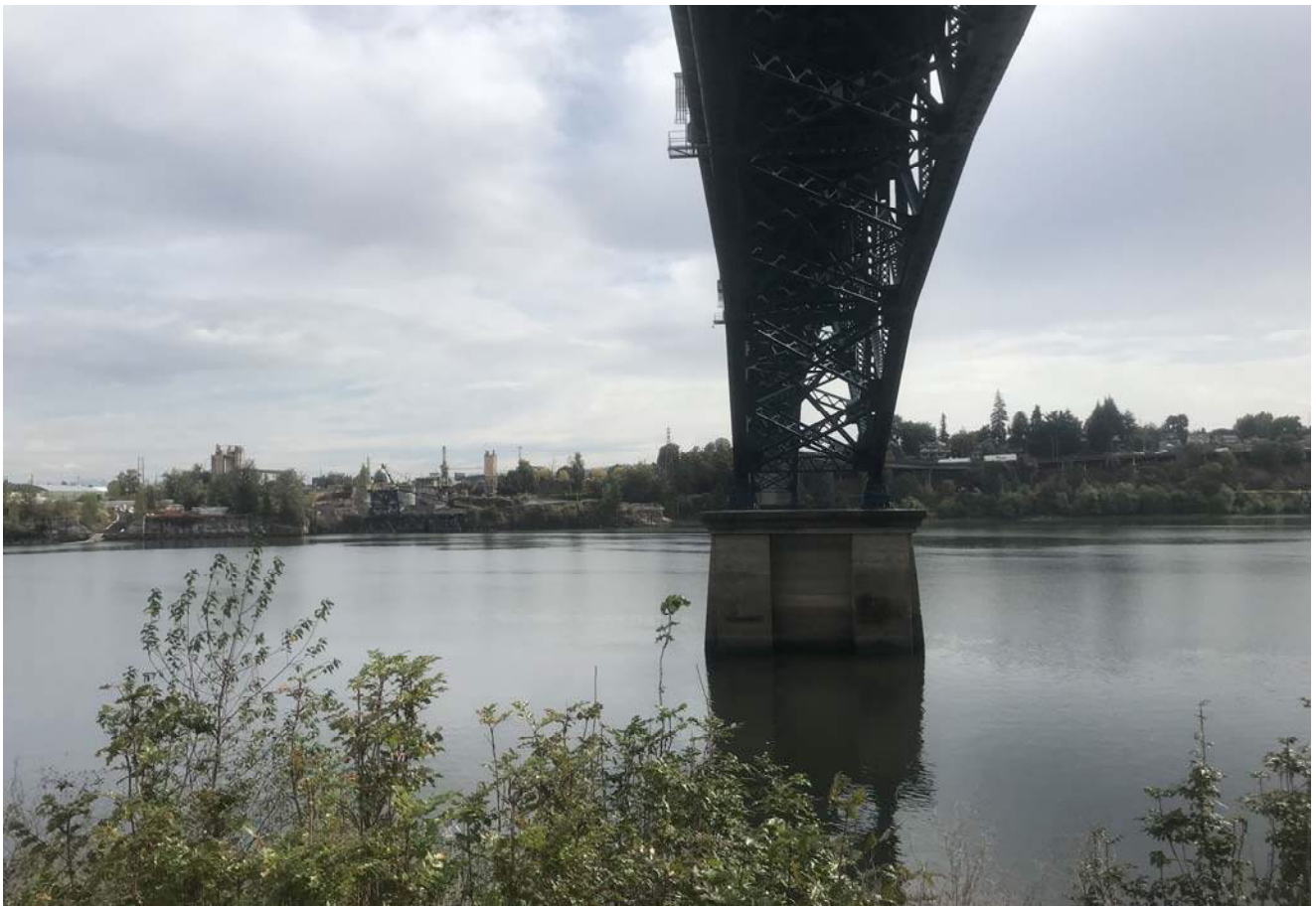
STA: 7+00 - Top of bank looking east
