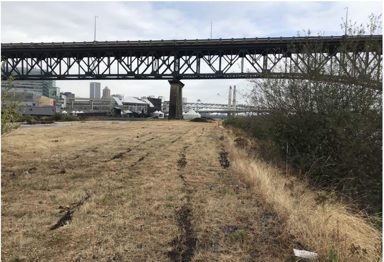
STA: 3+00 - Top of bank looking downstream
