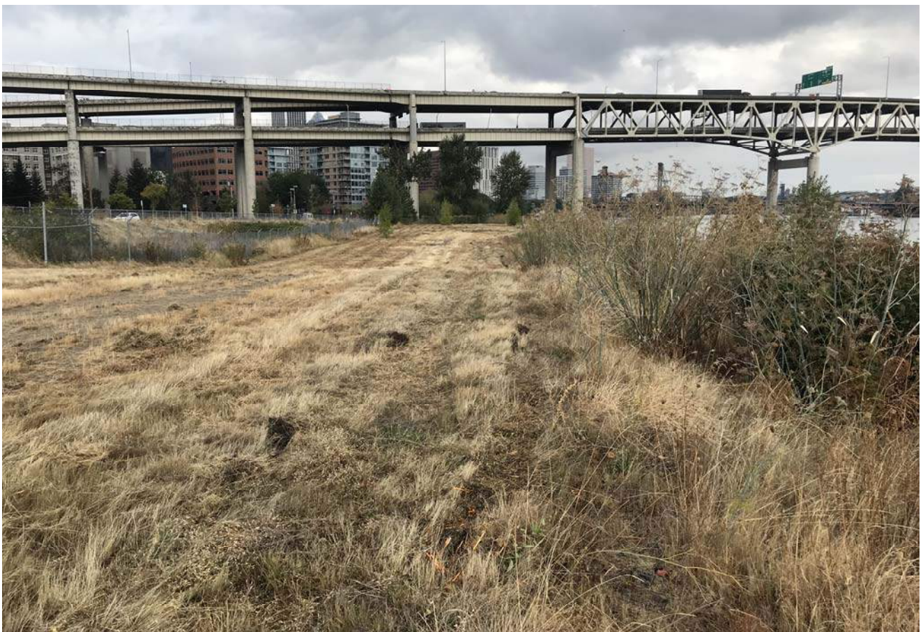
STA: 21+50 - Top of bank looking downstream
