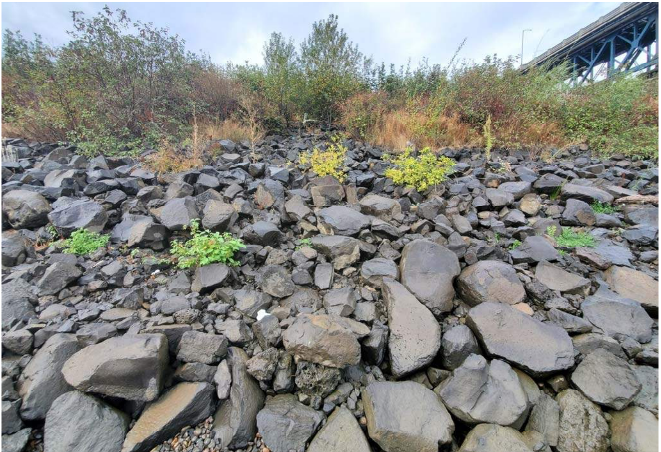
STA: 5+00 - Toe of slope looking west
