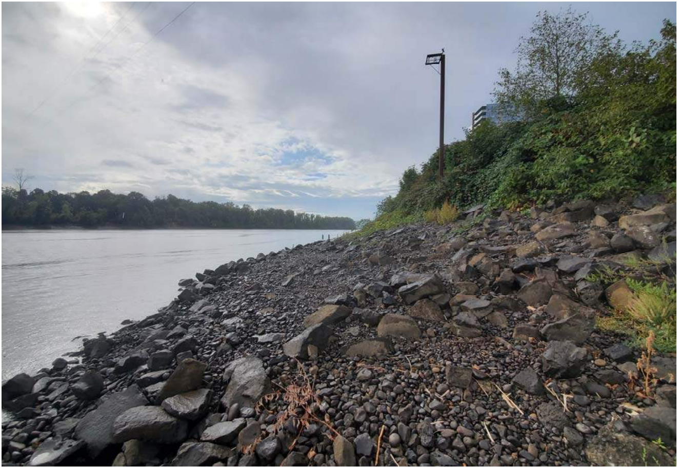
STA: 0+00 - Toe of slope looking upstream
