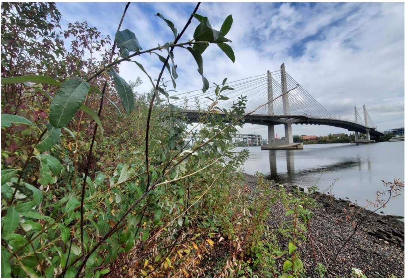
STA: 15+00 - Toe of slope looking downstream
