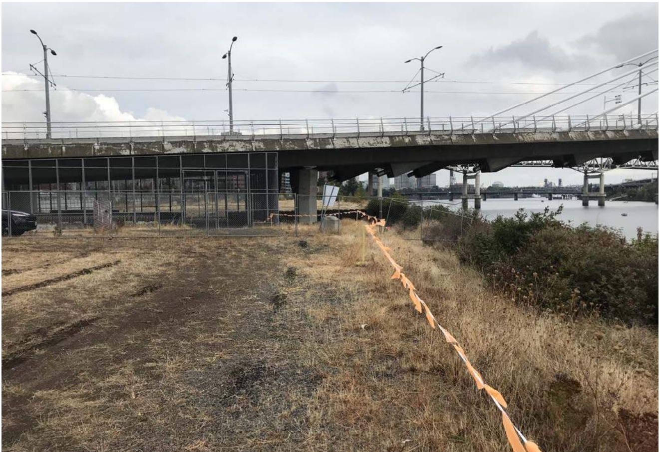
STA: 15+00 - Top of bank looking downstream
