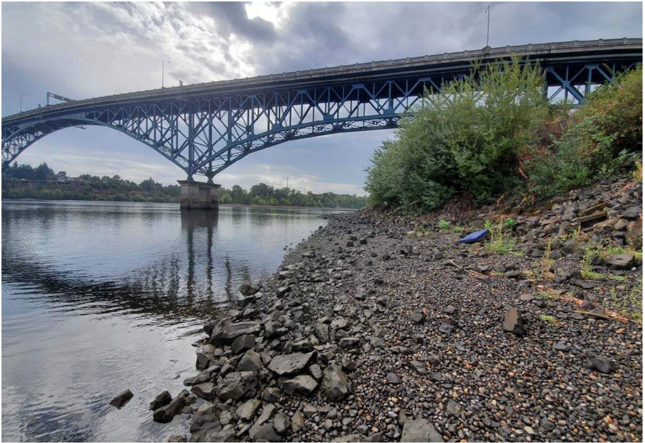
STA: 9+00 - Toe of slope looking upstream
