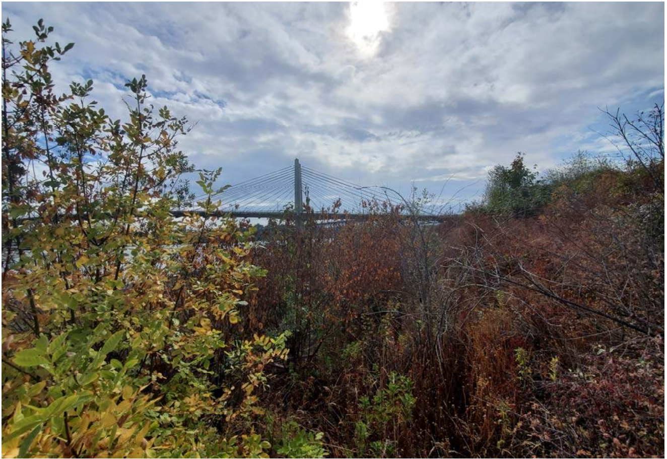
STA: 23+50 - Toe of slope looking upstream
