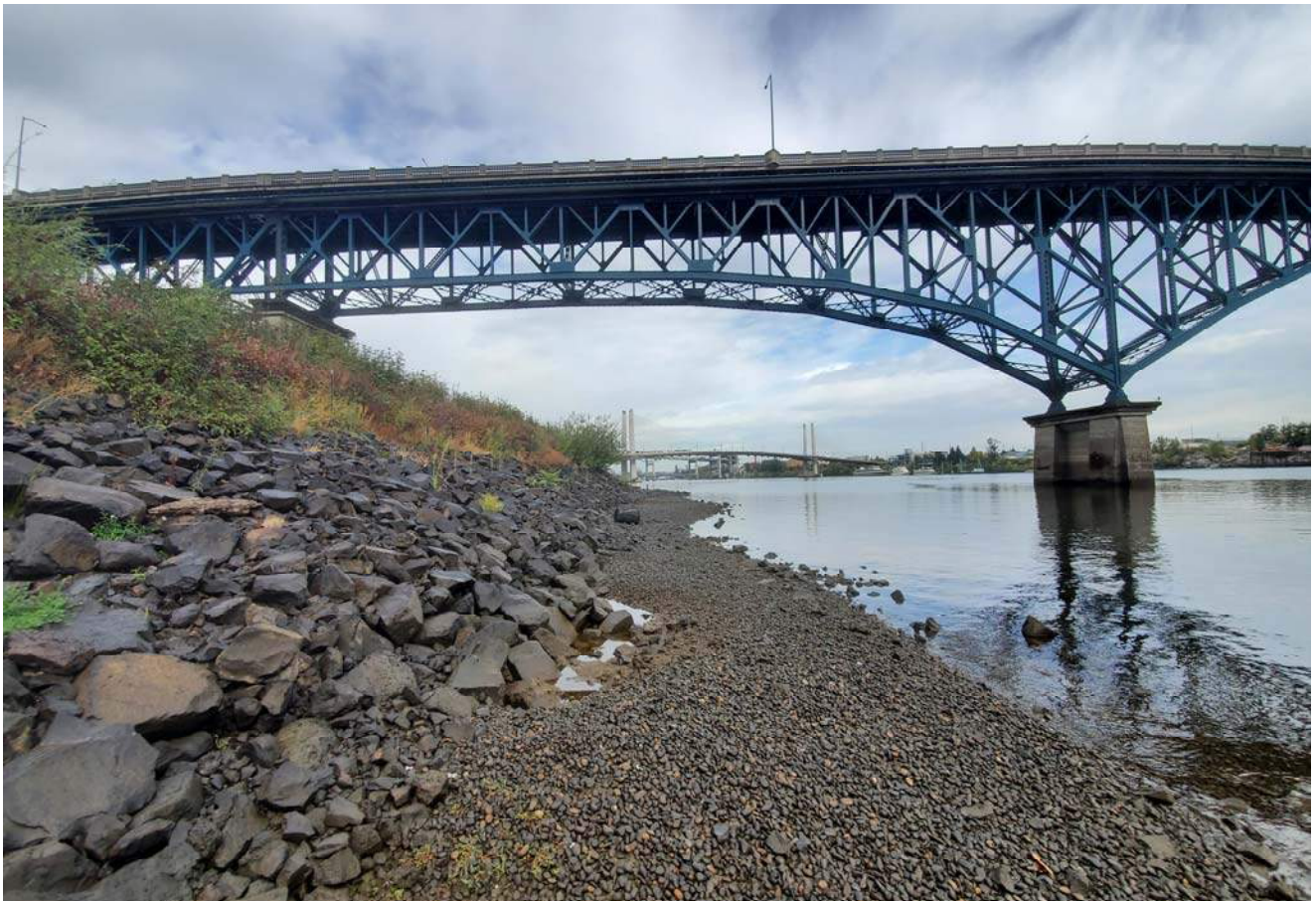
STA: 5+00 - Toe of slope looking downstream
