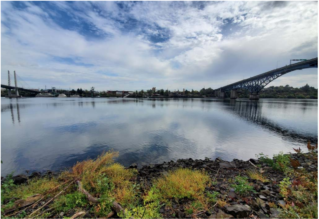
STA: 11+00 - Top of rock armor looking east
