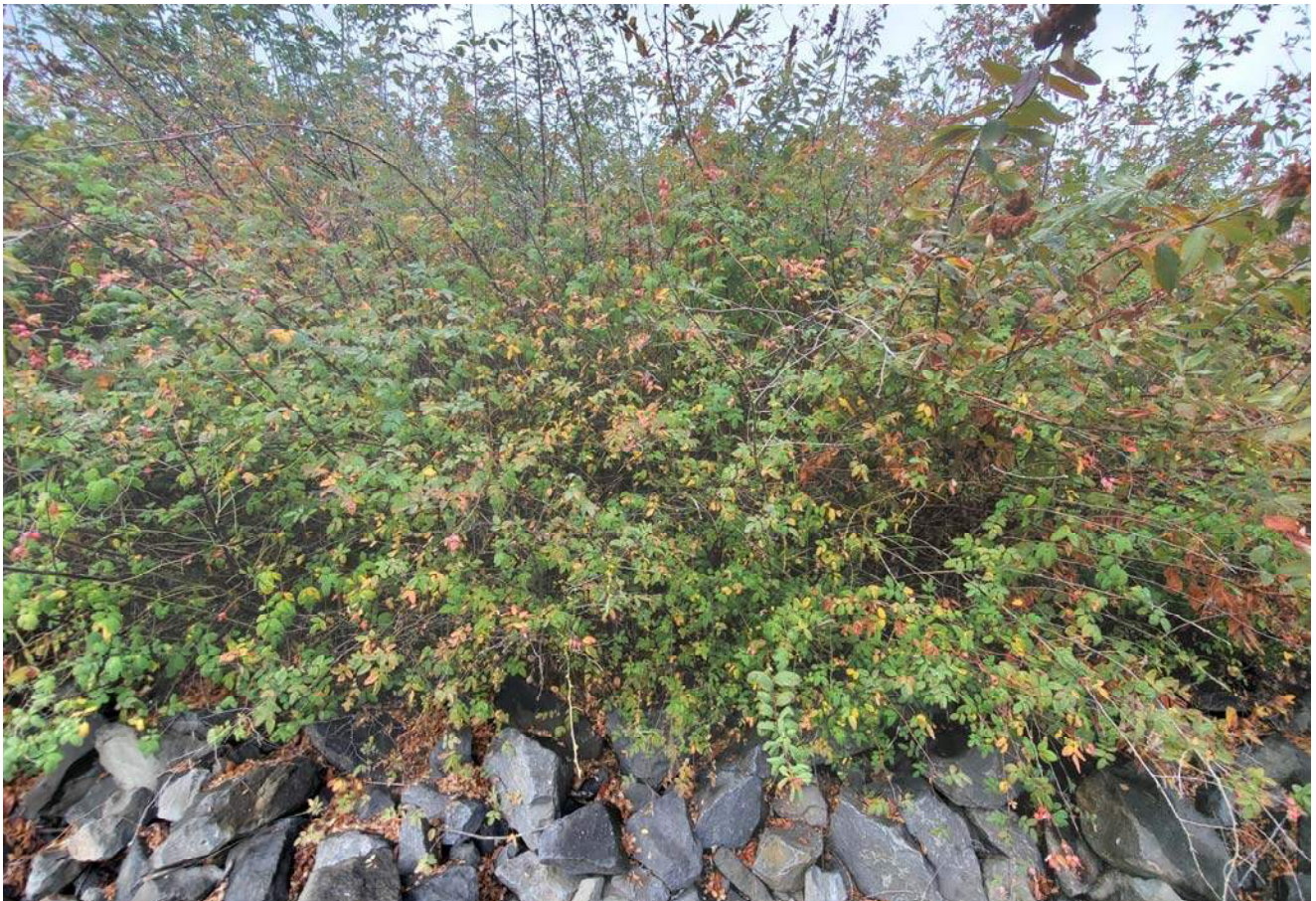
STA: 9+00 - Top of rock armor looking west
