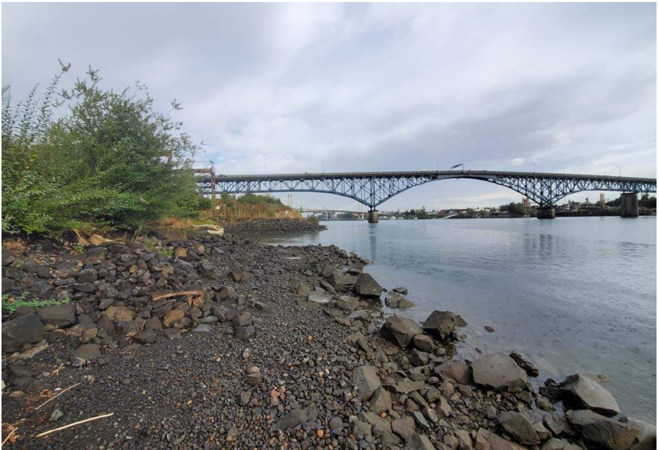
STA: 0+00 - Toe of slope looking downstream
