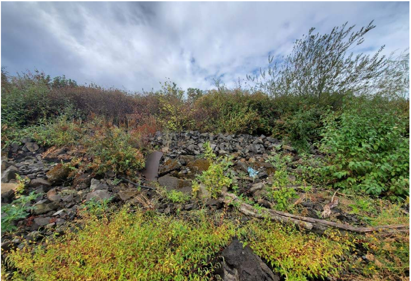
STA: 11+00 - Toe of slope looking west
