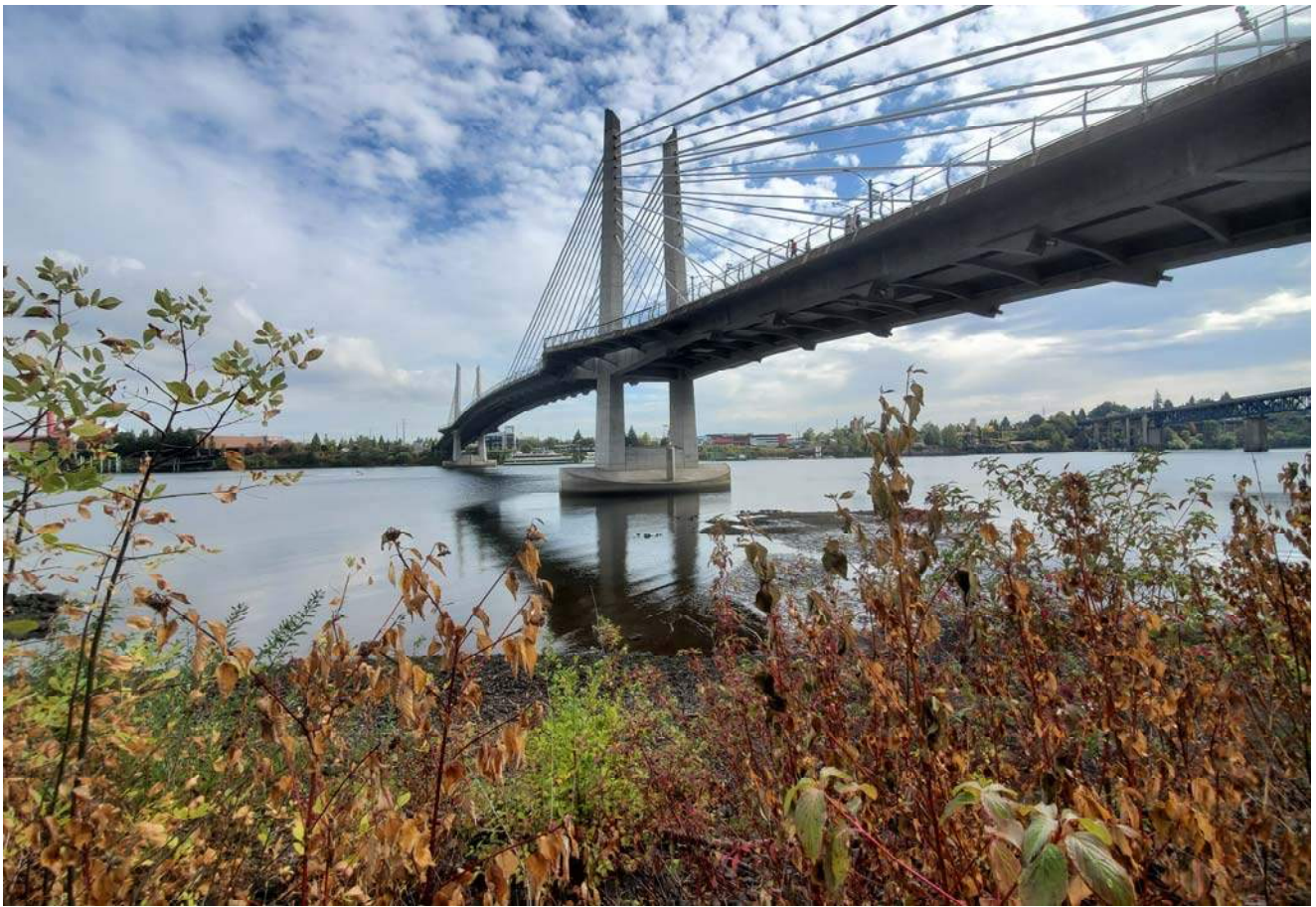
STA: 17+00 - Toe of slope looking east
