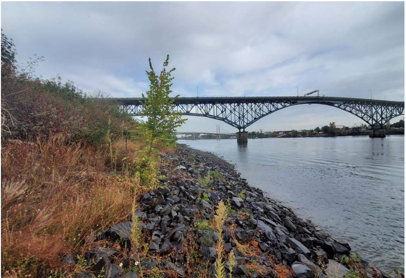
STA: 3+00 - Top of rock armor looking downstream
