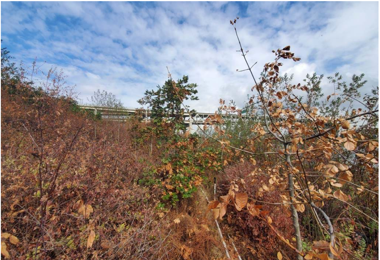
STA: 23+50 - Toe of slope looking downstream
