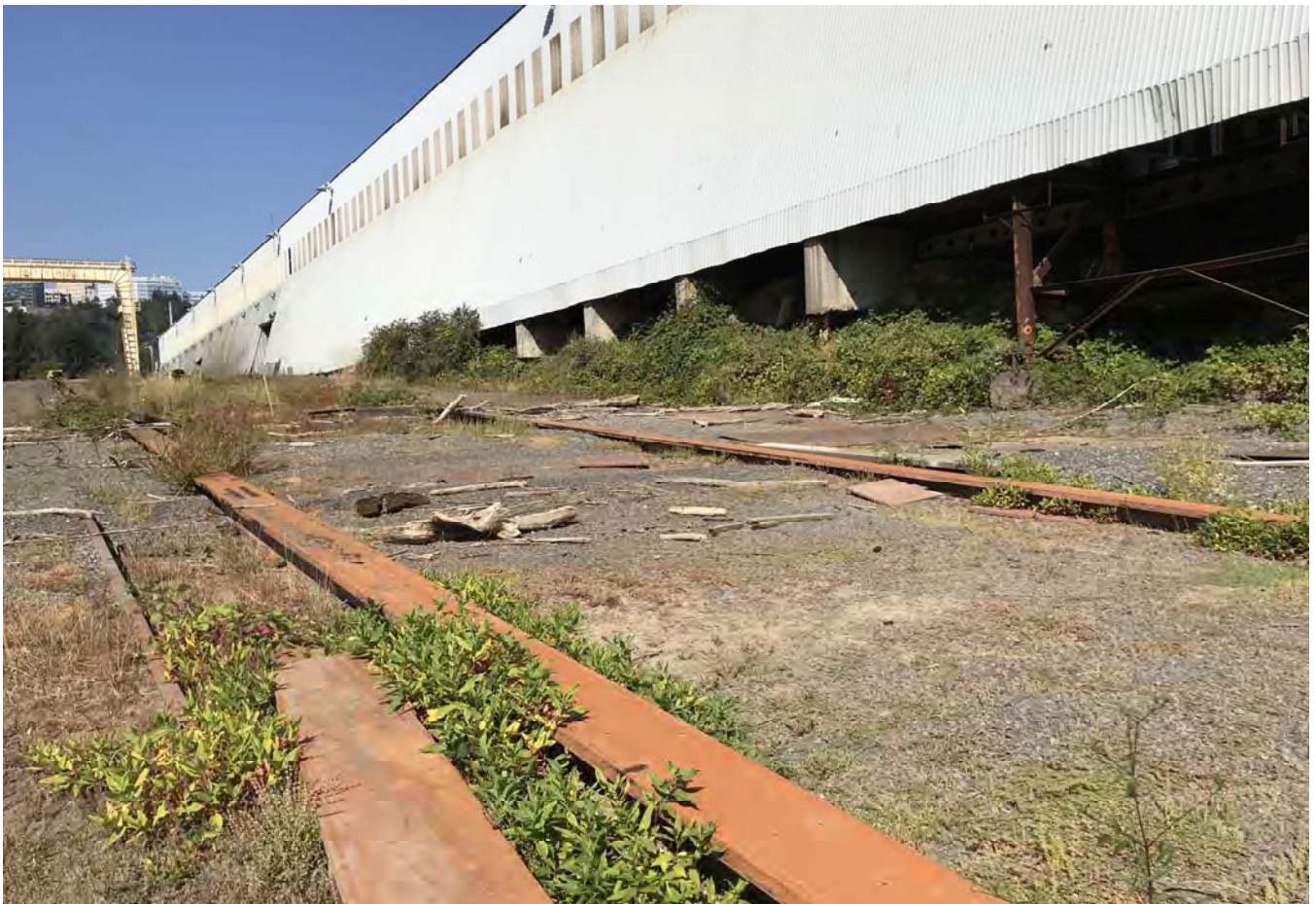
Slipway ramp looking northwest.
