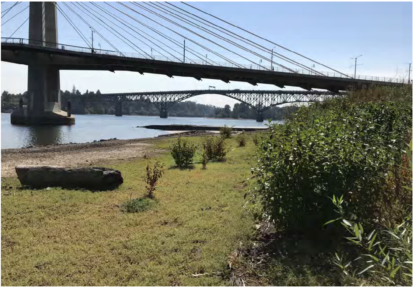
STA: 21+50 - Toe of slope looking upstream.
