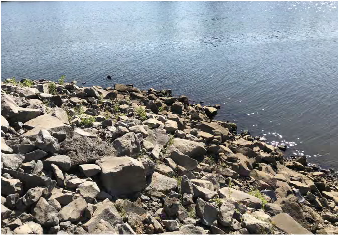
North slope of slipway ramp looking east.
