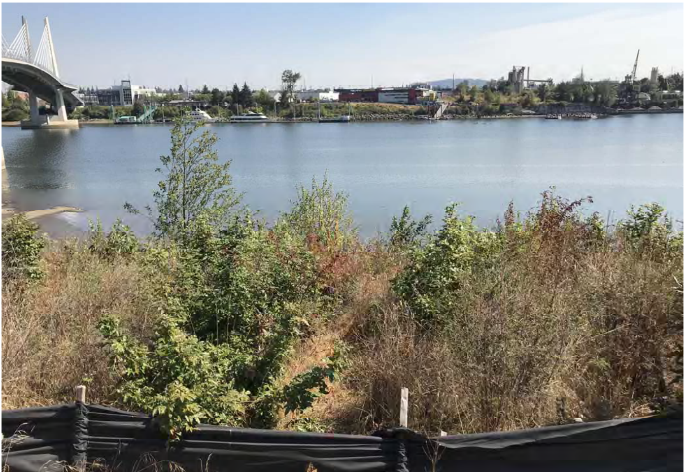
STA: 15+00 - Top of bank looking east.
