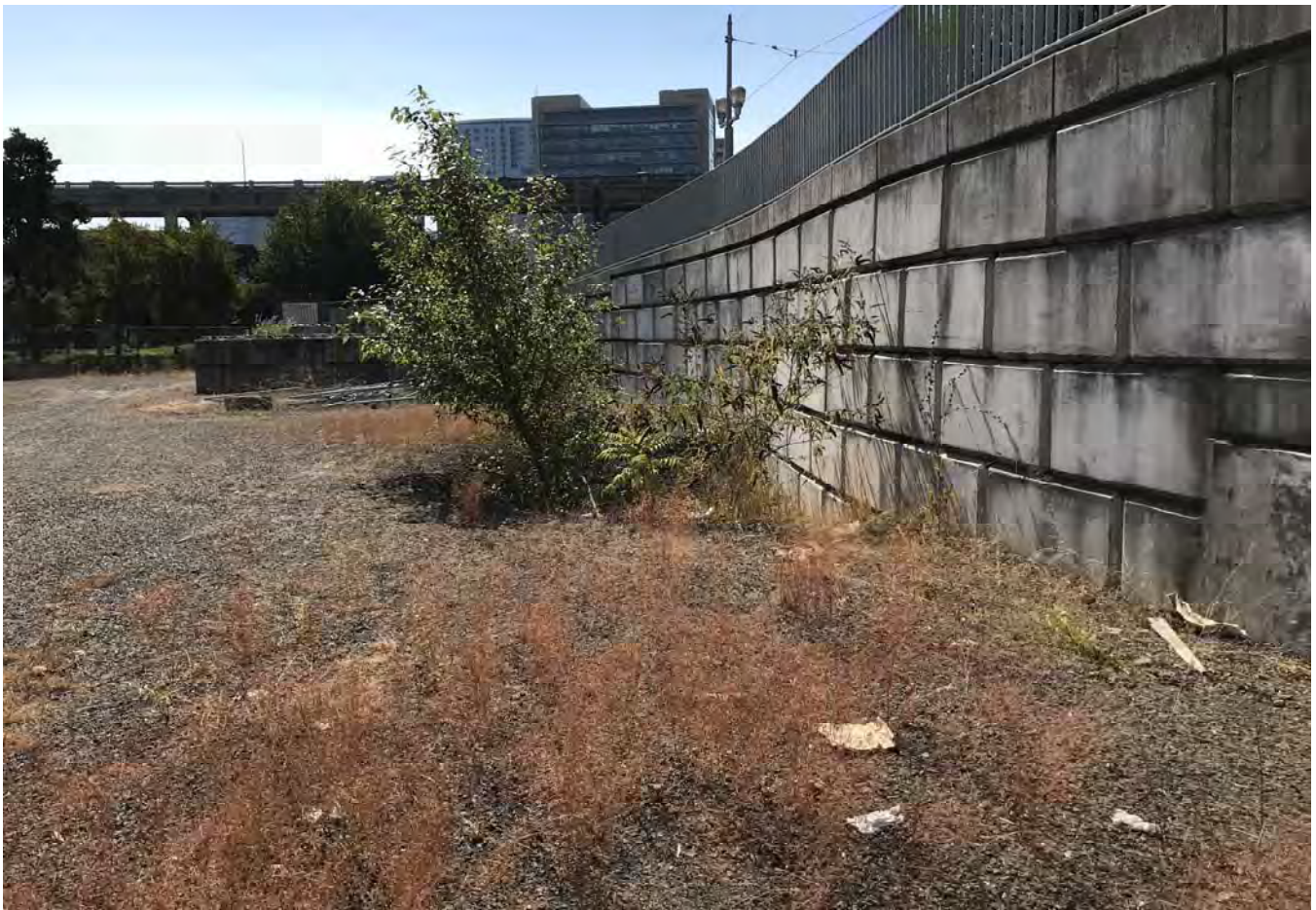
Northwest corner of upland cap looking south.
