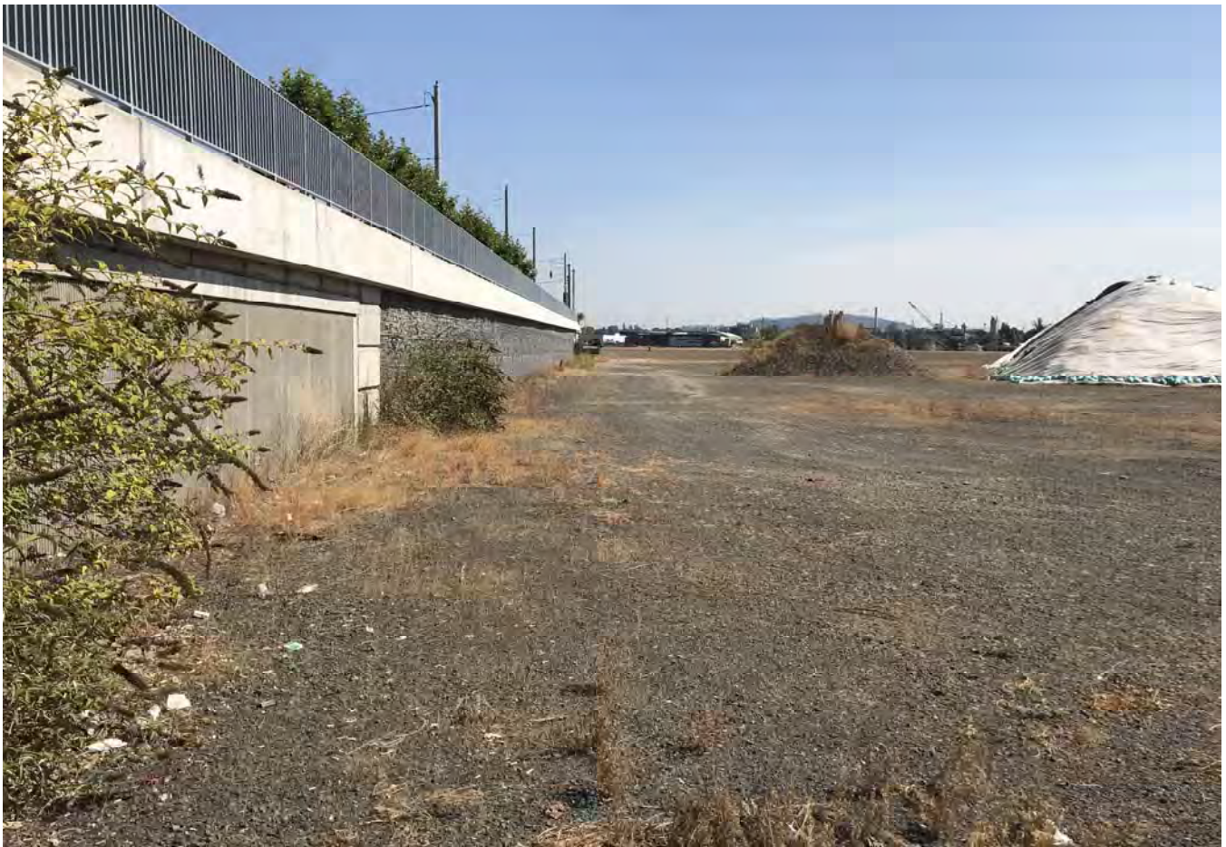
Northwest corner of upland cap looking east.
