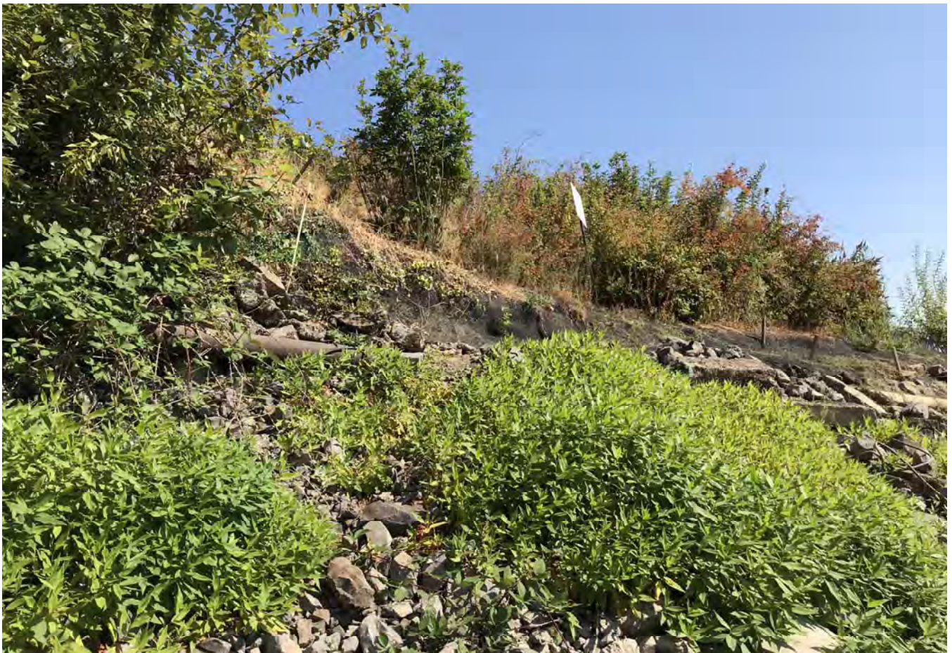
North slope of slipway ramp looking north.
