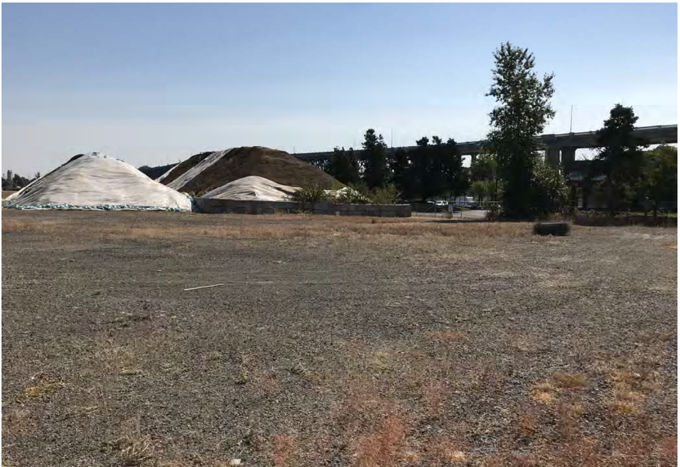
Northwest corner of upland cap looking southeast.
