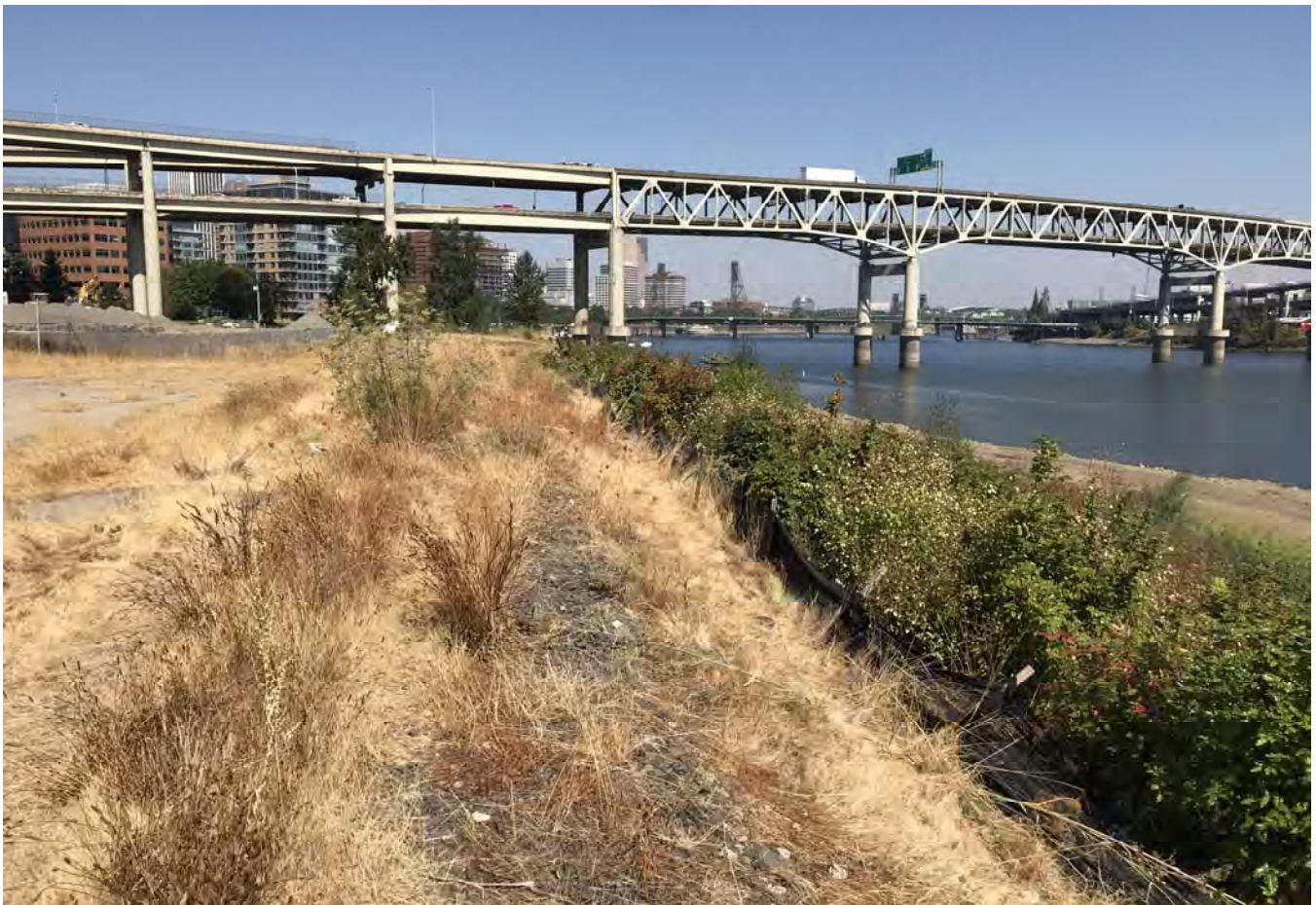
STA: 21+50 - Top of bank looking downstream.
