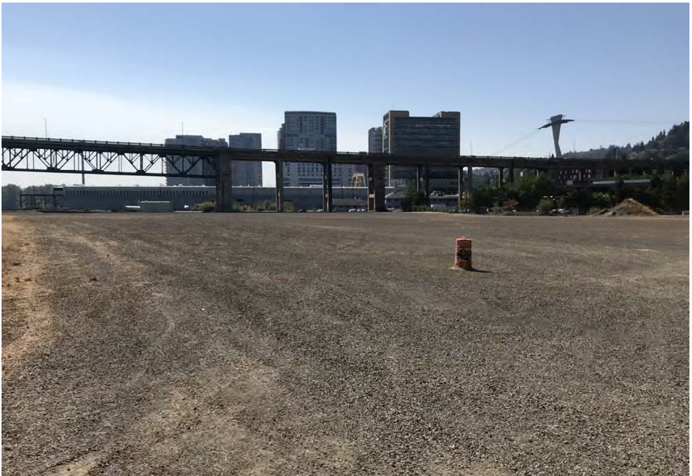
Northeast corner of upland cap looking southwest.
