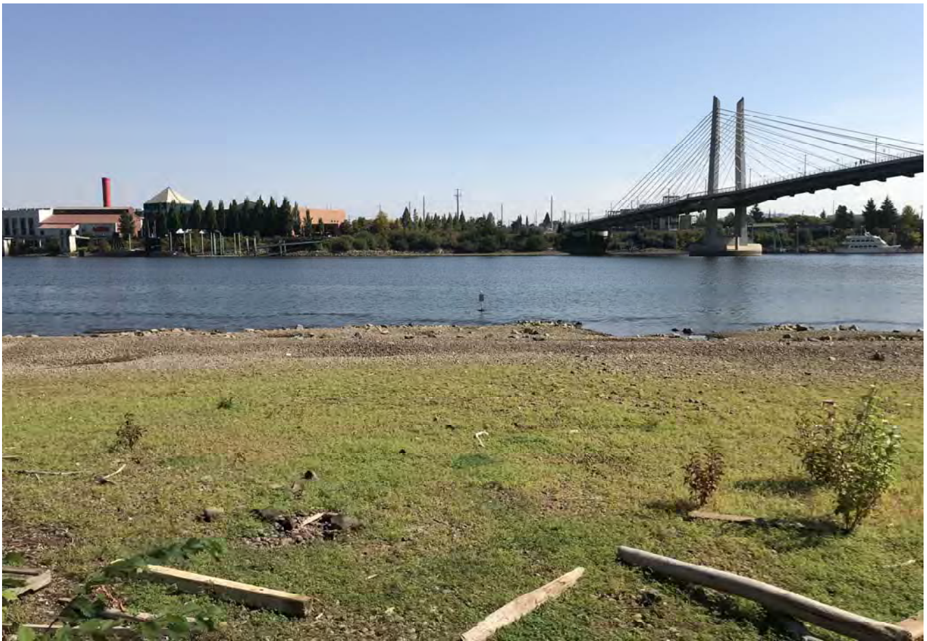
STA: 23+50 - Toe of slope looking east.
