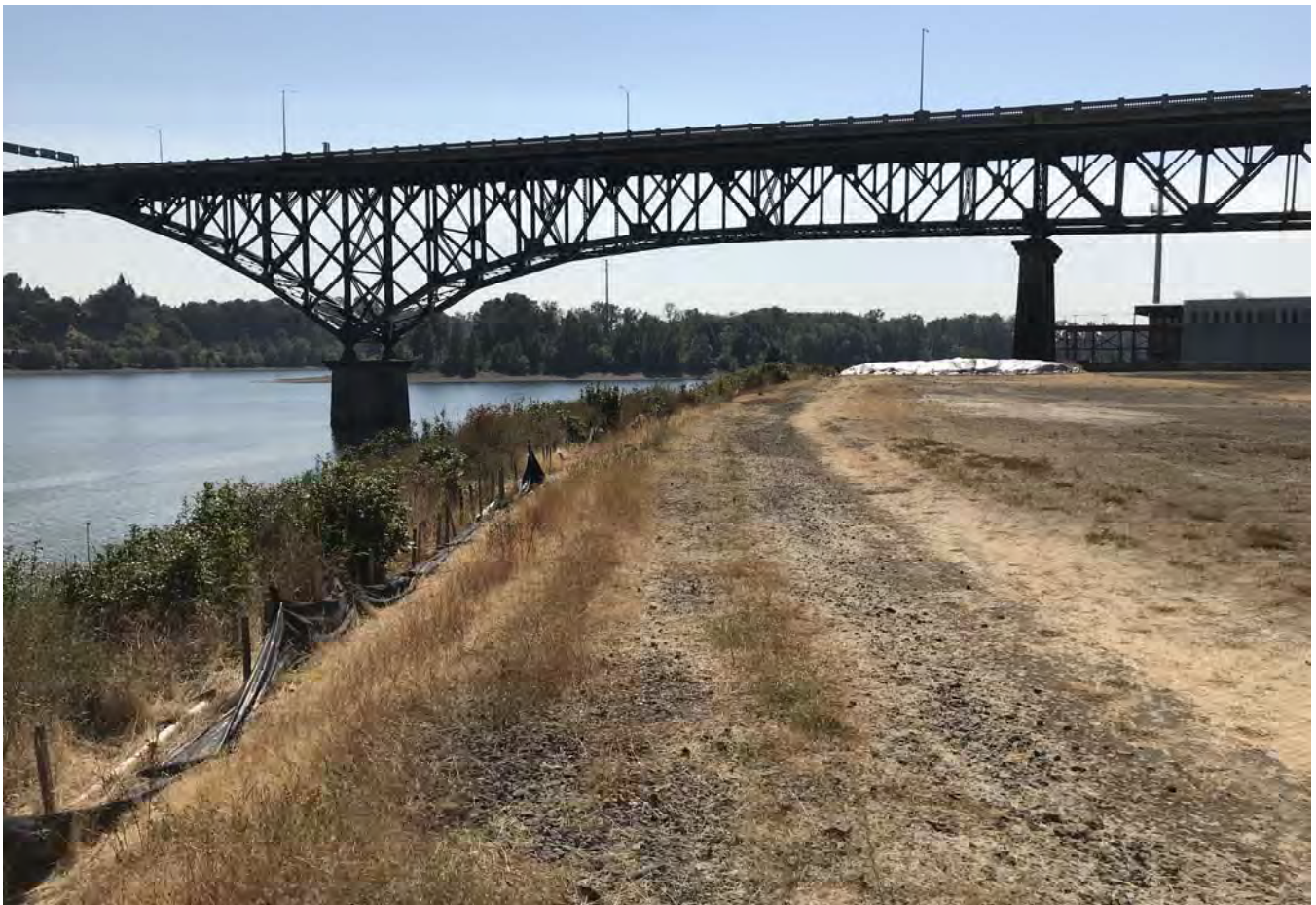
STA: 11+00 - Top of bank looking upstream.
