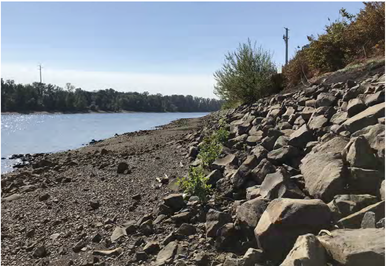
STA: 7+00 - Bottom of rock armor looking upstream.
