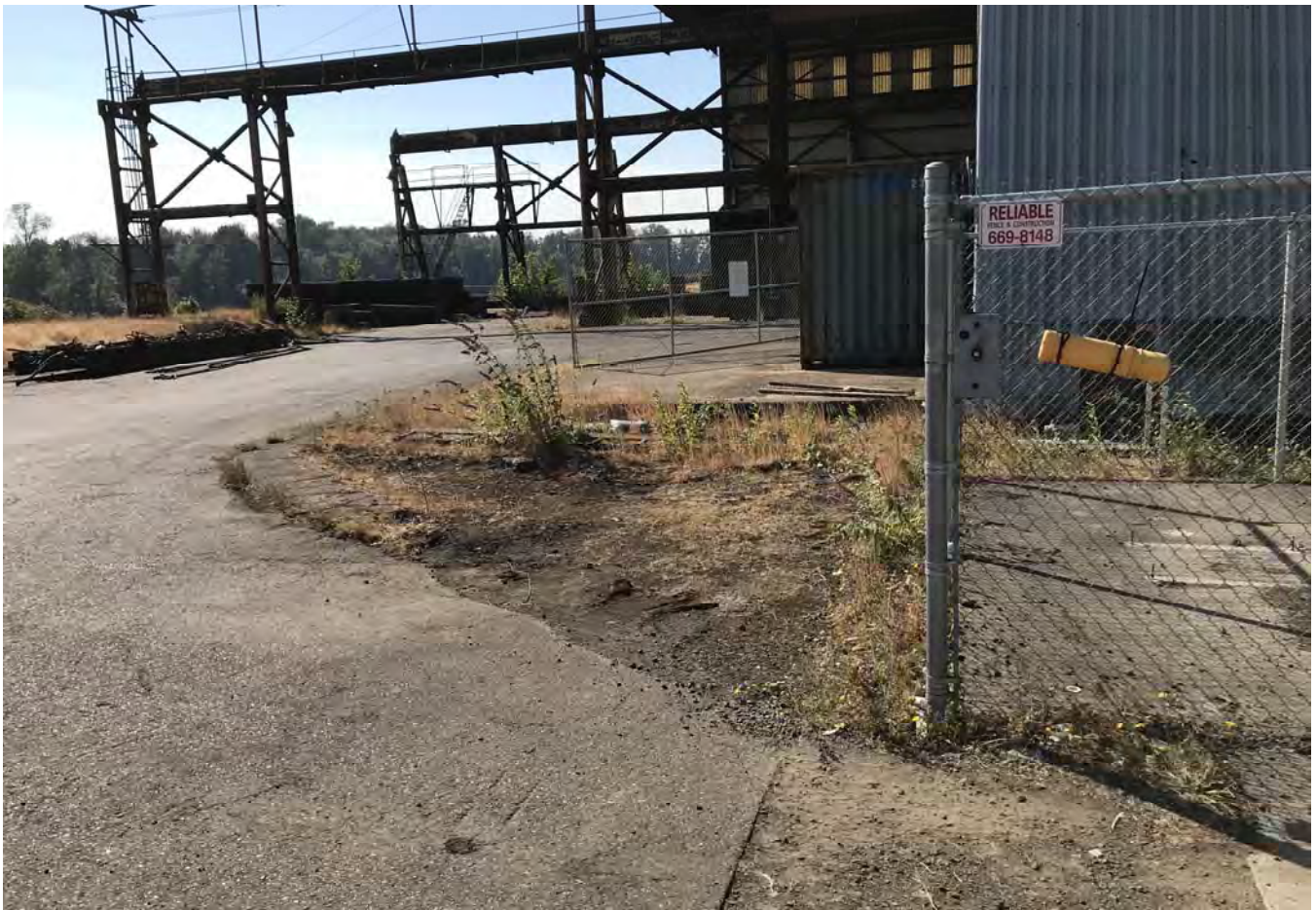
Operational area north of barge building looking southeast.
