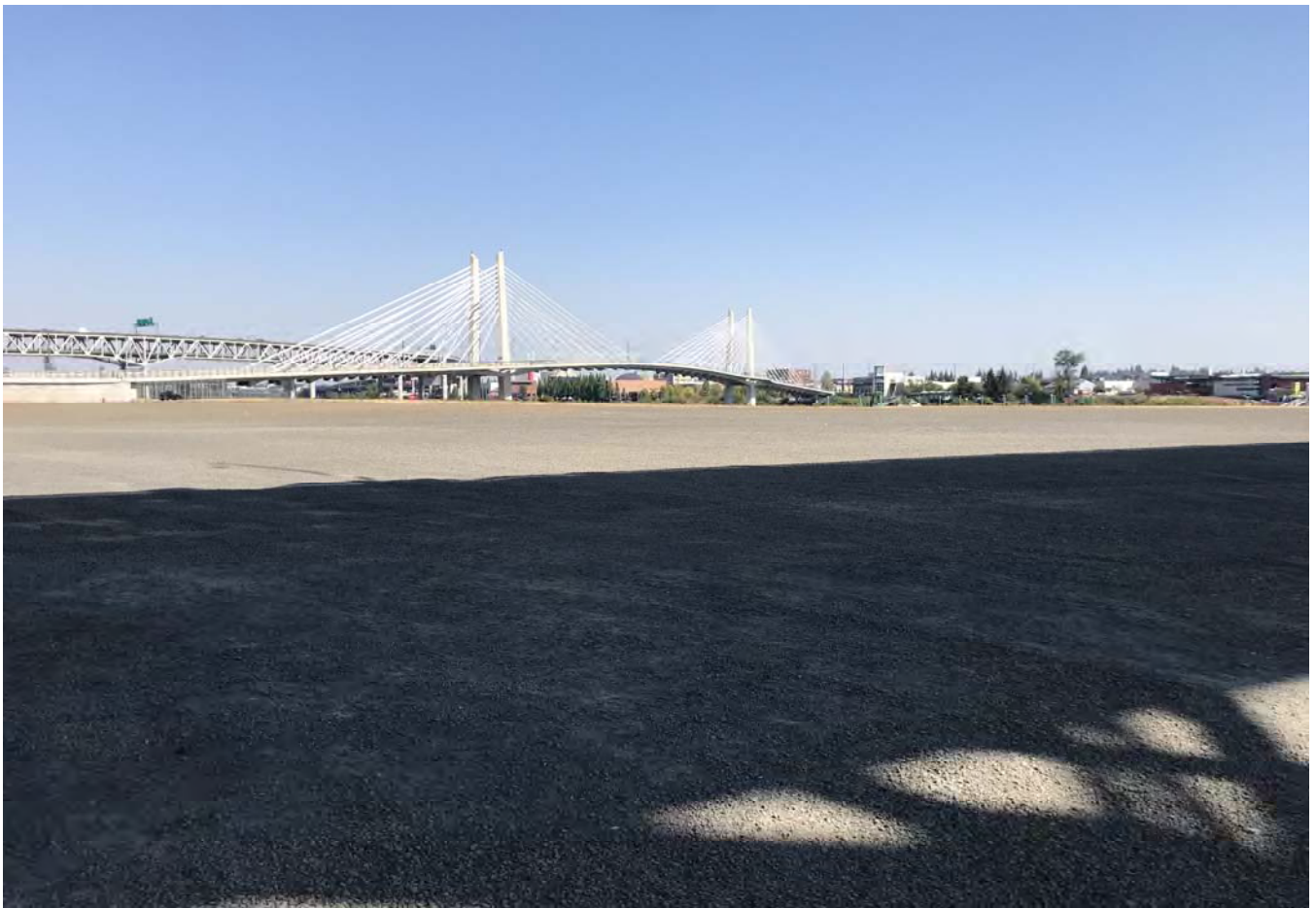
Upland cap beneath Ross Island Bridge looking northeast.
