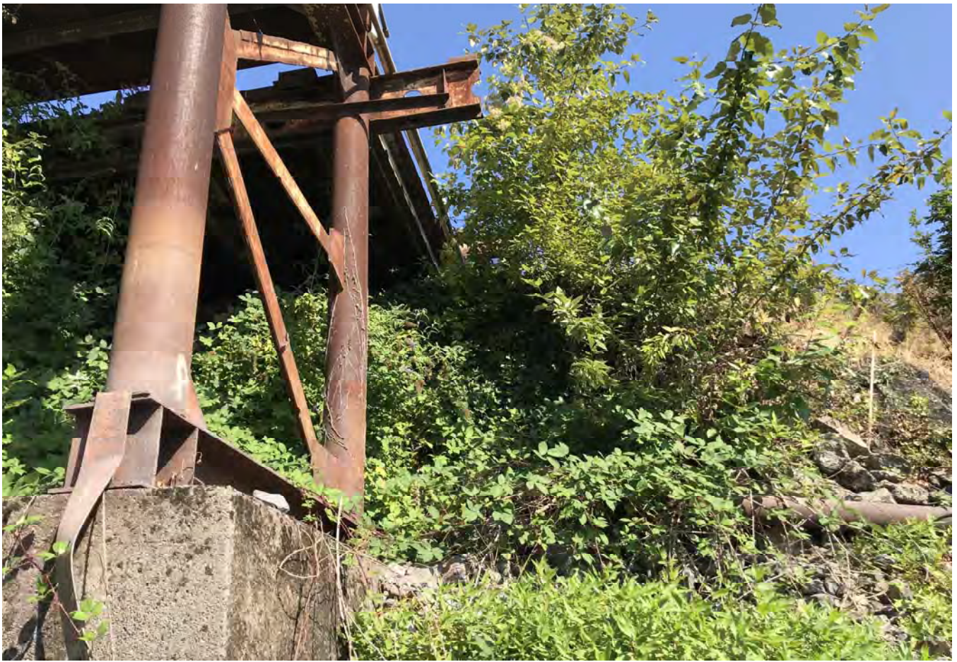
East end of barge building looking northwest.
