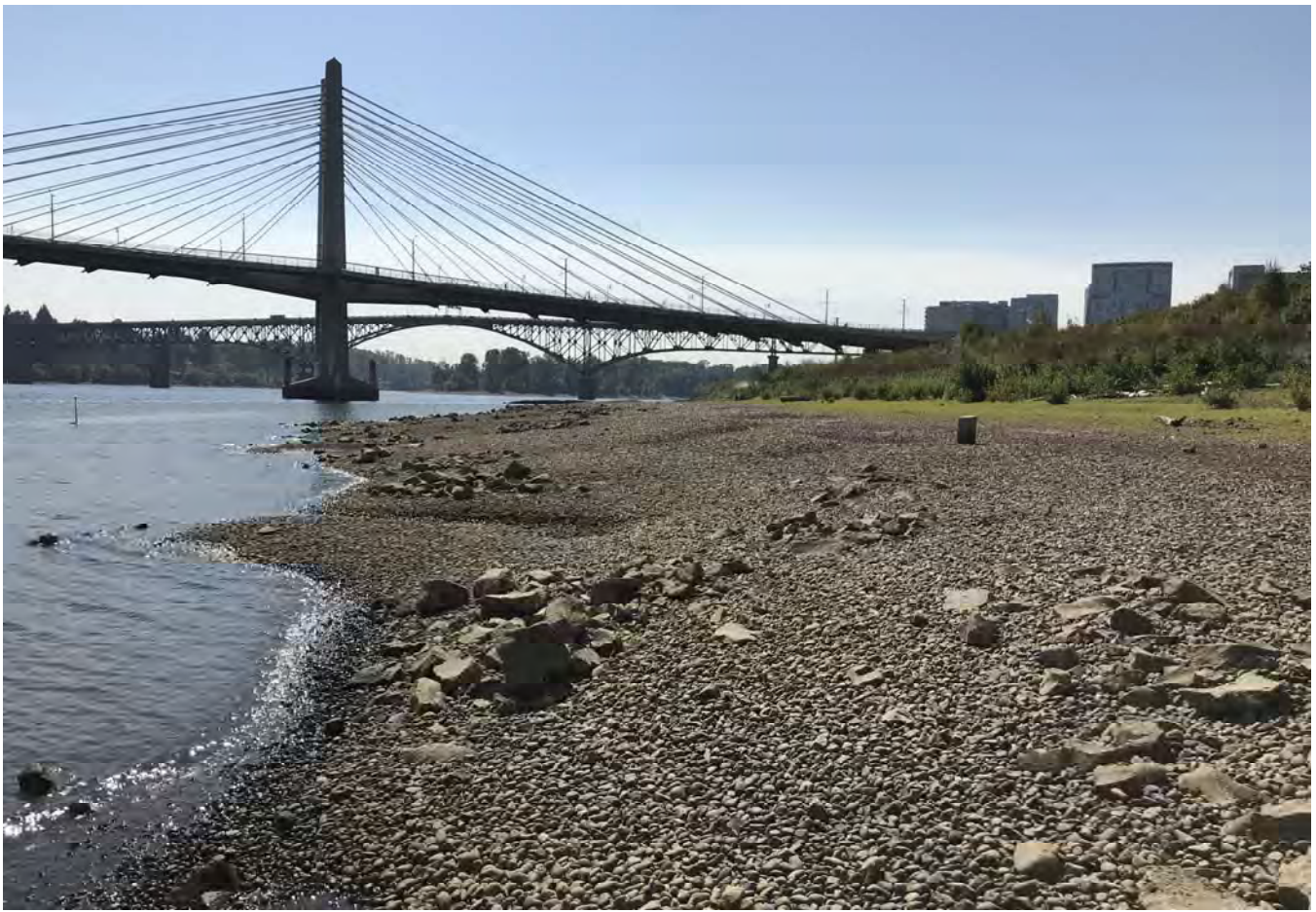
STA: 25+50 - Edge of water looking upstream.
