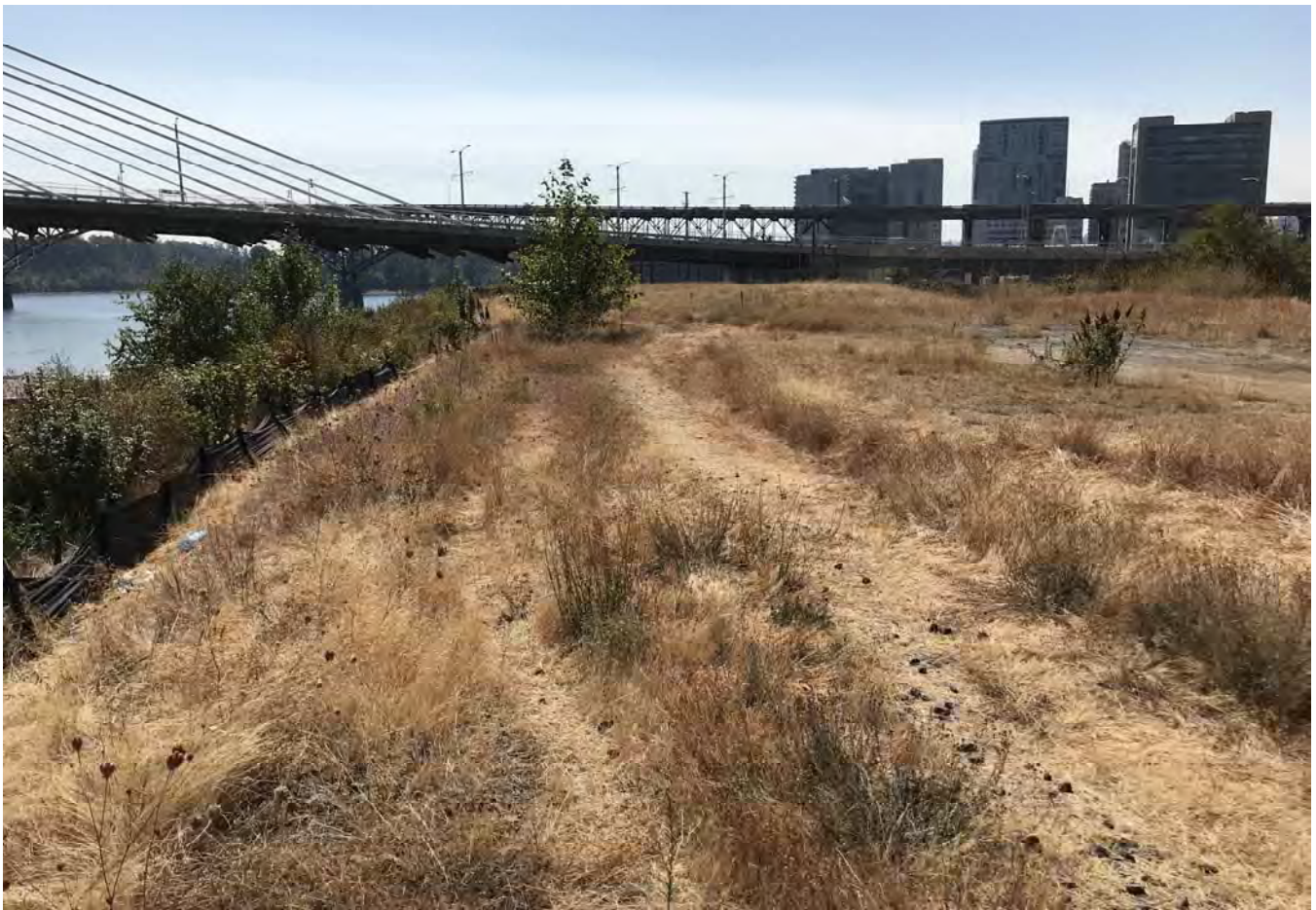
STA: 21+50 - Top of bank looking upstream.
