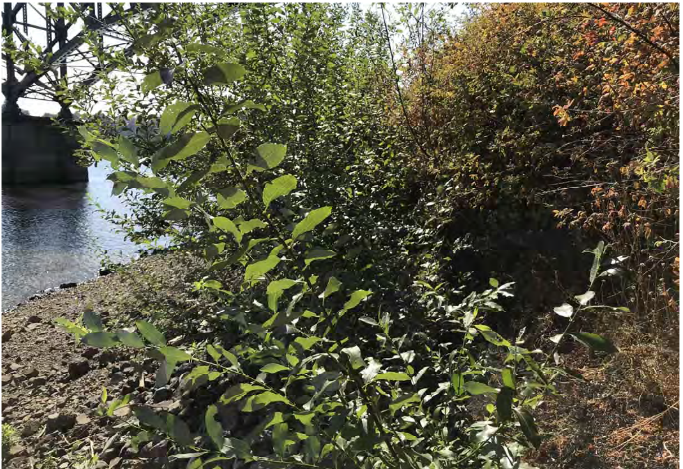
STA: 9+00 - Top of rock armor looking upstream.
