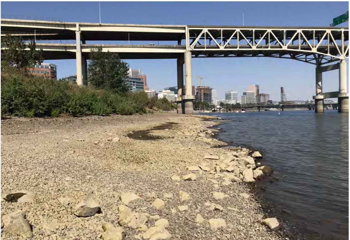
STA: 25+50 - Edge of water looking downstream.
