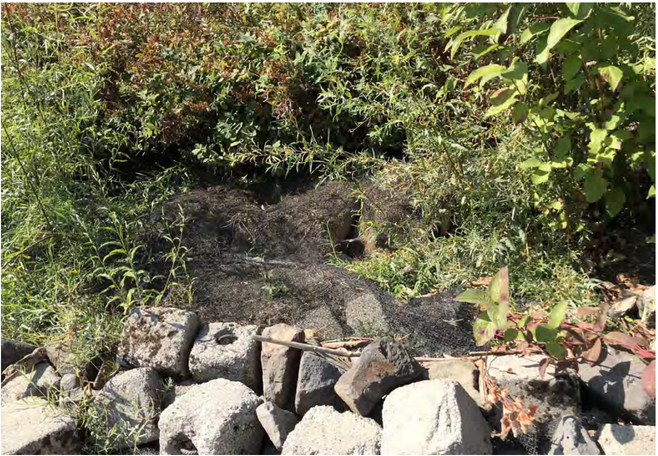
STA: 11+00 - Bottom of rock armor looking west.
