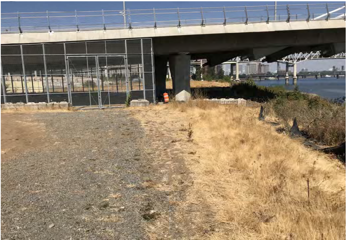
STA: 15+00 - Top of bank looking downstream.
