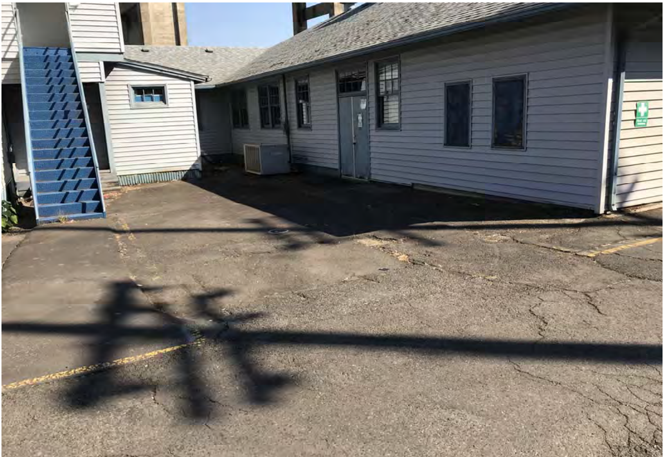
Office building, southeast corner looking north.
