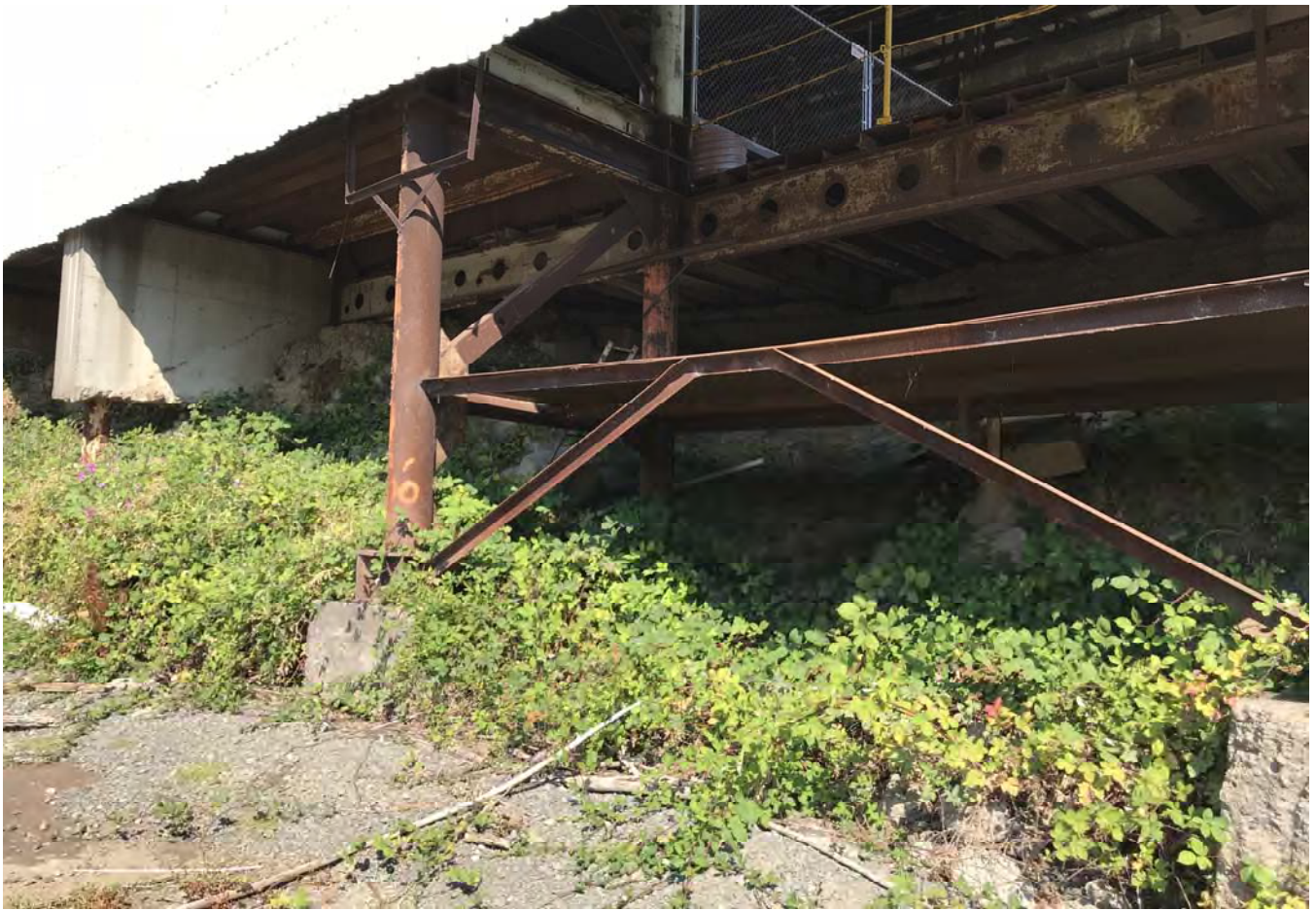
Underside of barge building structure looking northwest from slipway.
