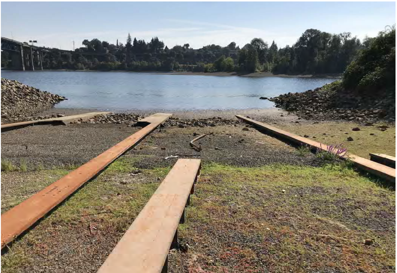
Slipway ramp looking east.
