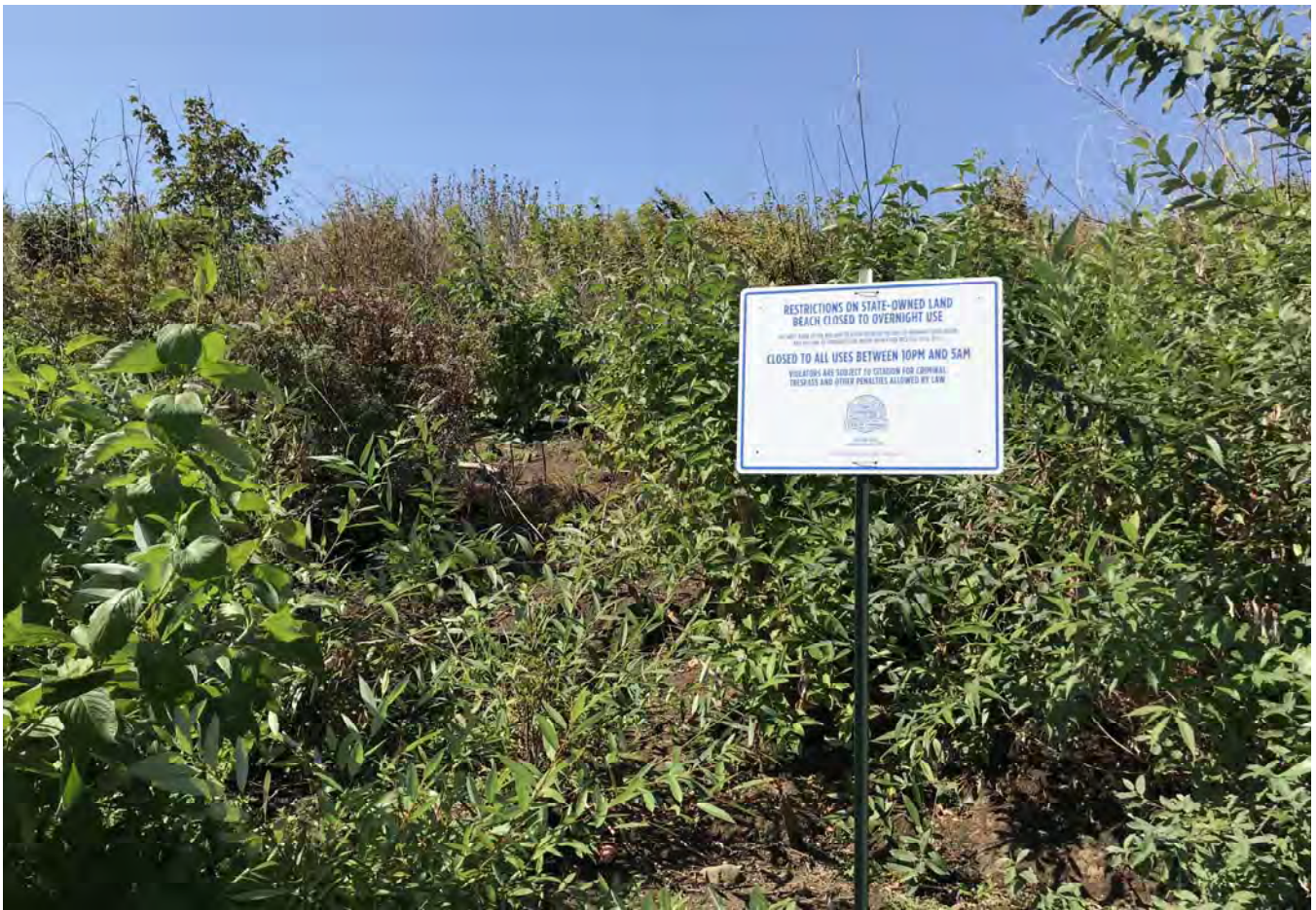
STA: 25+50 - Toe of slope looking west.
