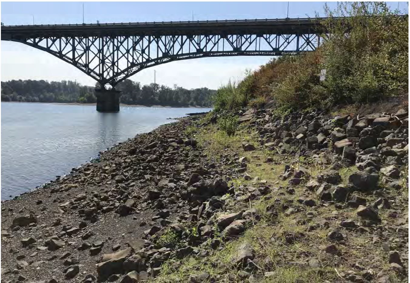
STA: 11+50 - Toe of slope looking upstream.
