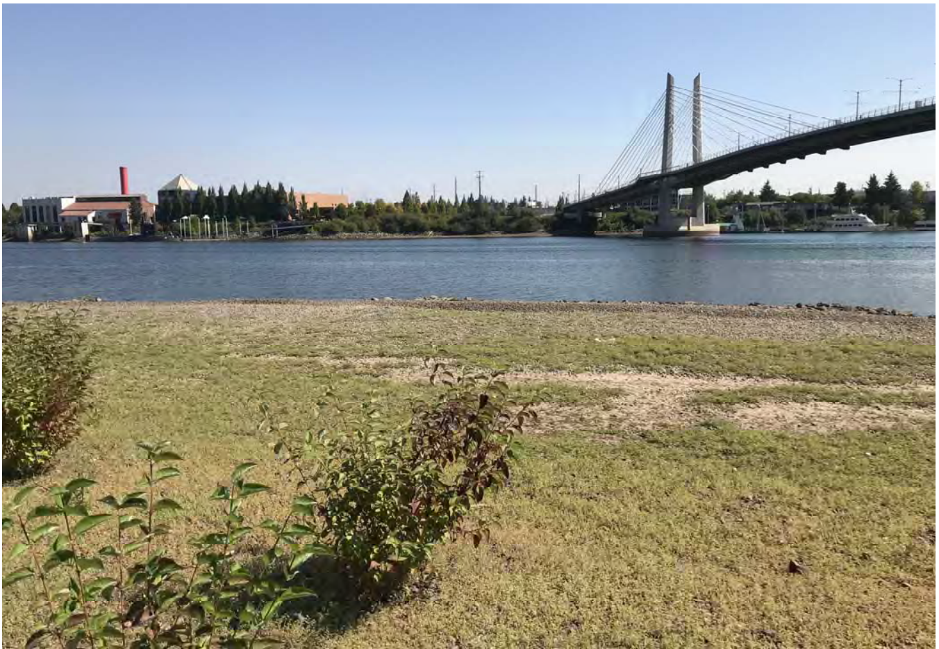
STA: 21+50 - Toe of slope looking east.
