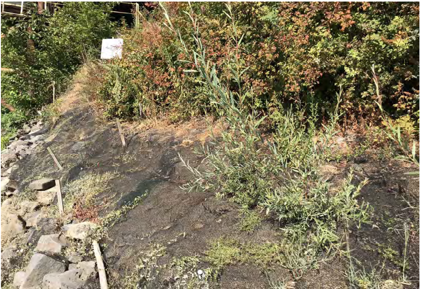
North slope of slipway ramp at top of rock armor looking west.
