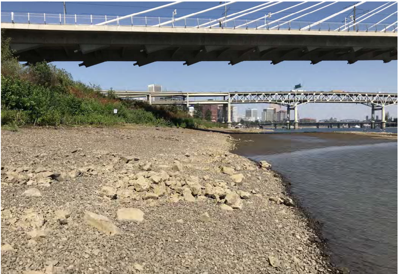
STA: 15+00 - Edge of water looking downstream.
