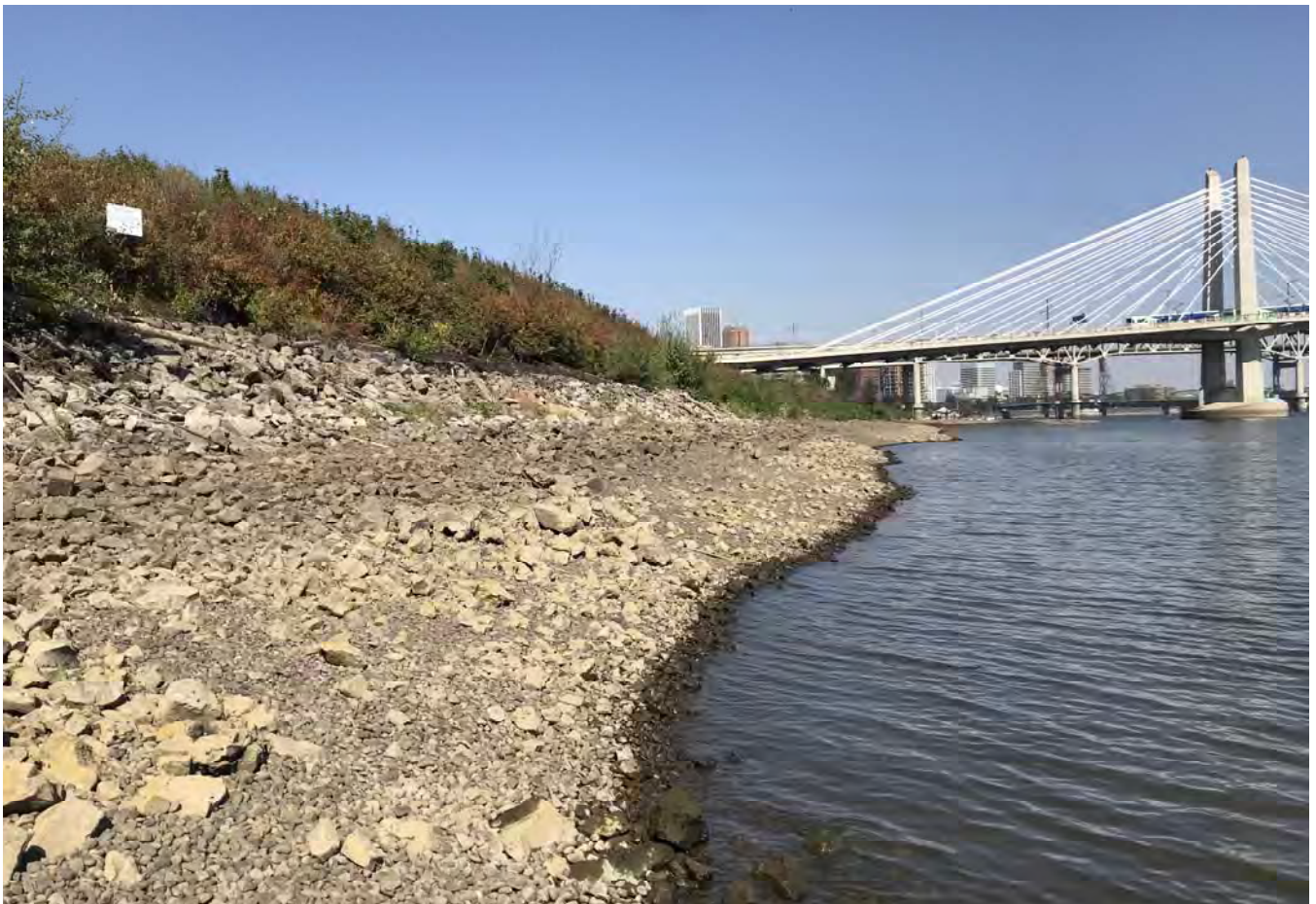
STA: 9+00 - Edge of water looking downstream.
