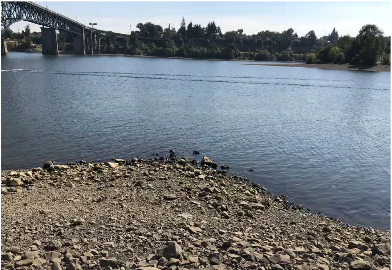
STA: 3+00 - Top of rock armor looking east.
