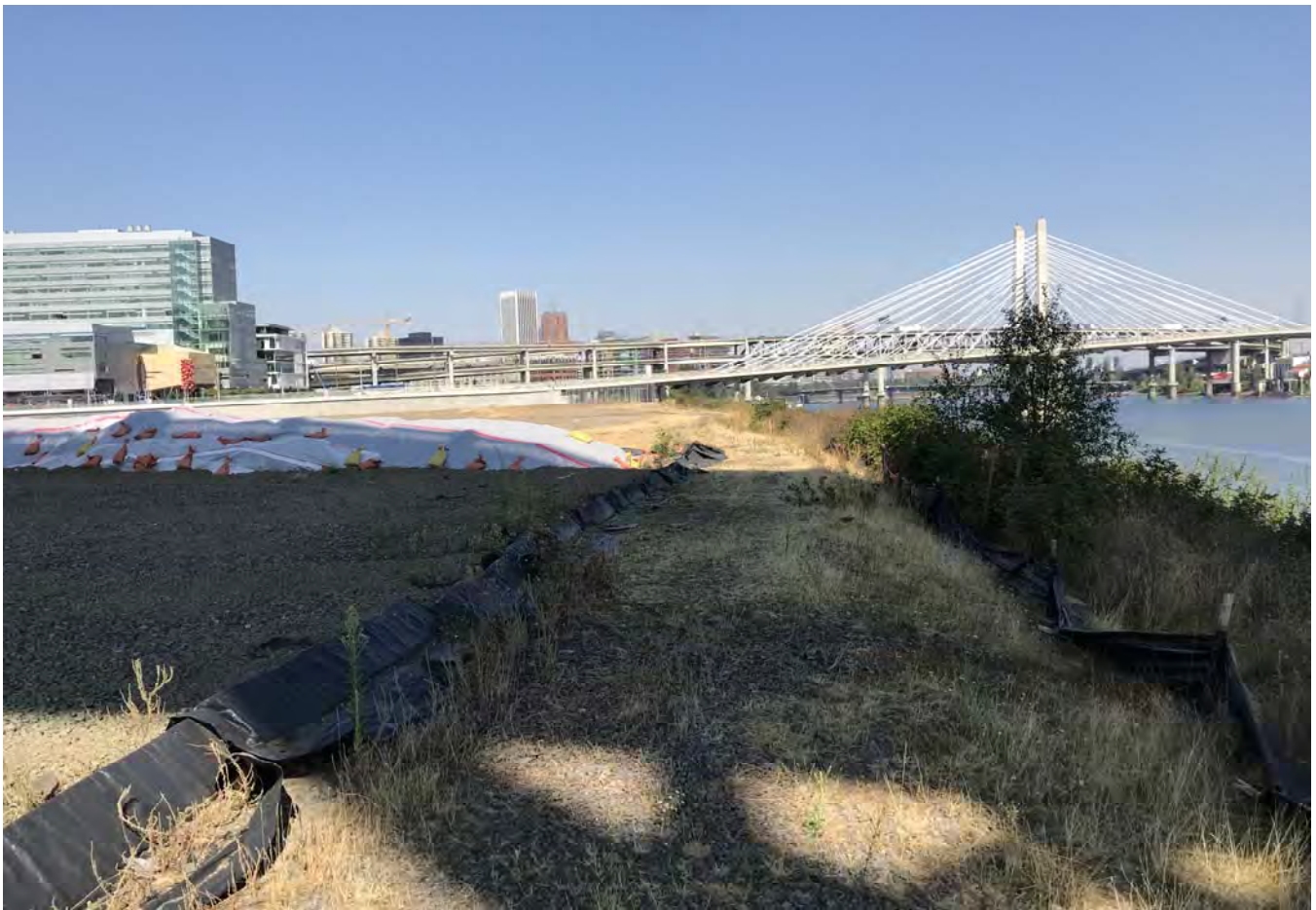
STA: 7+00 - Top of bank looking downstream.
