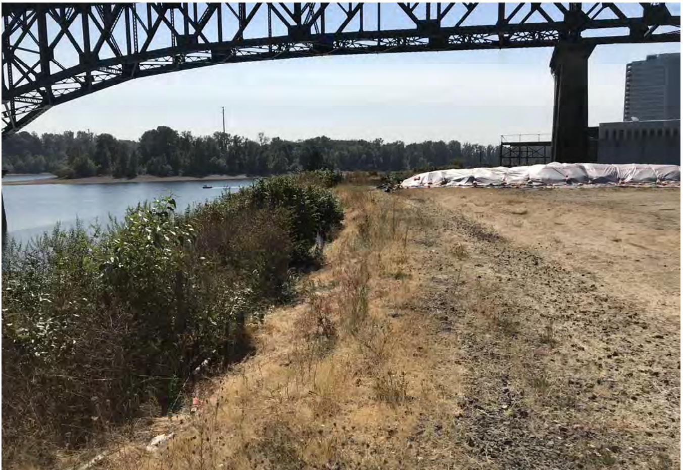
STA: 9+00 - Top of bank looking upstream.
