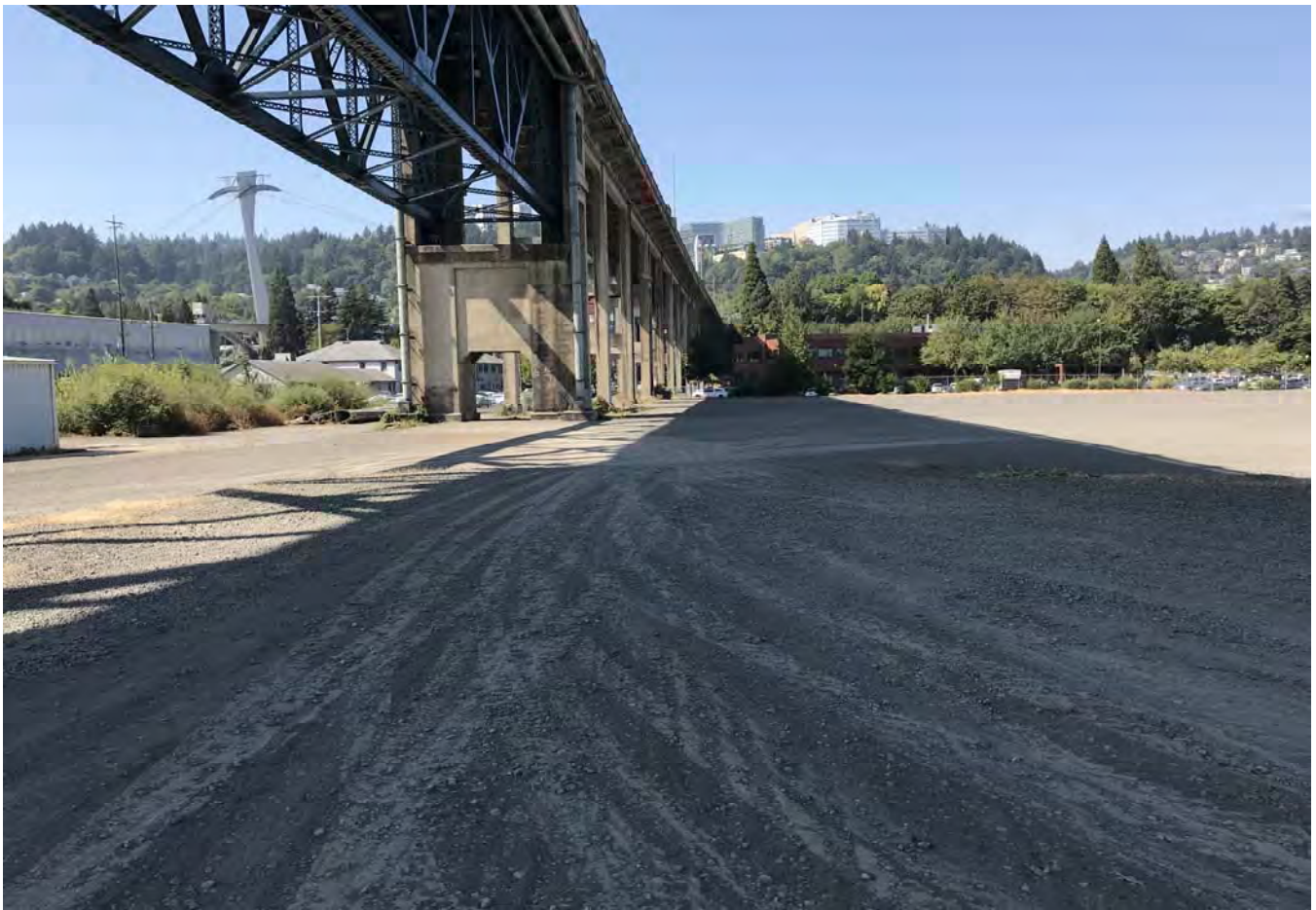
Upland cap, Southeast corner looking west.
