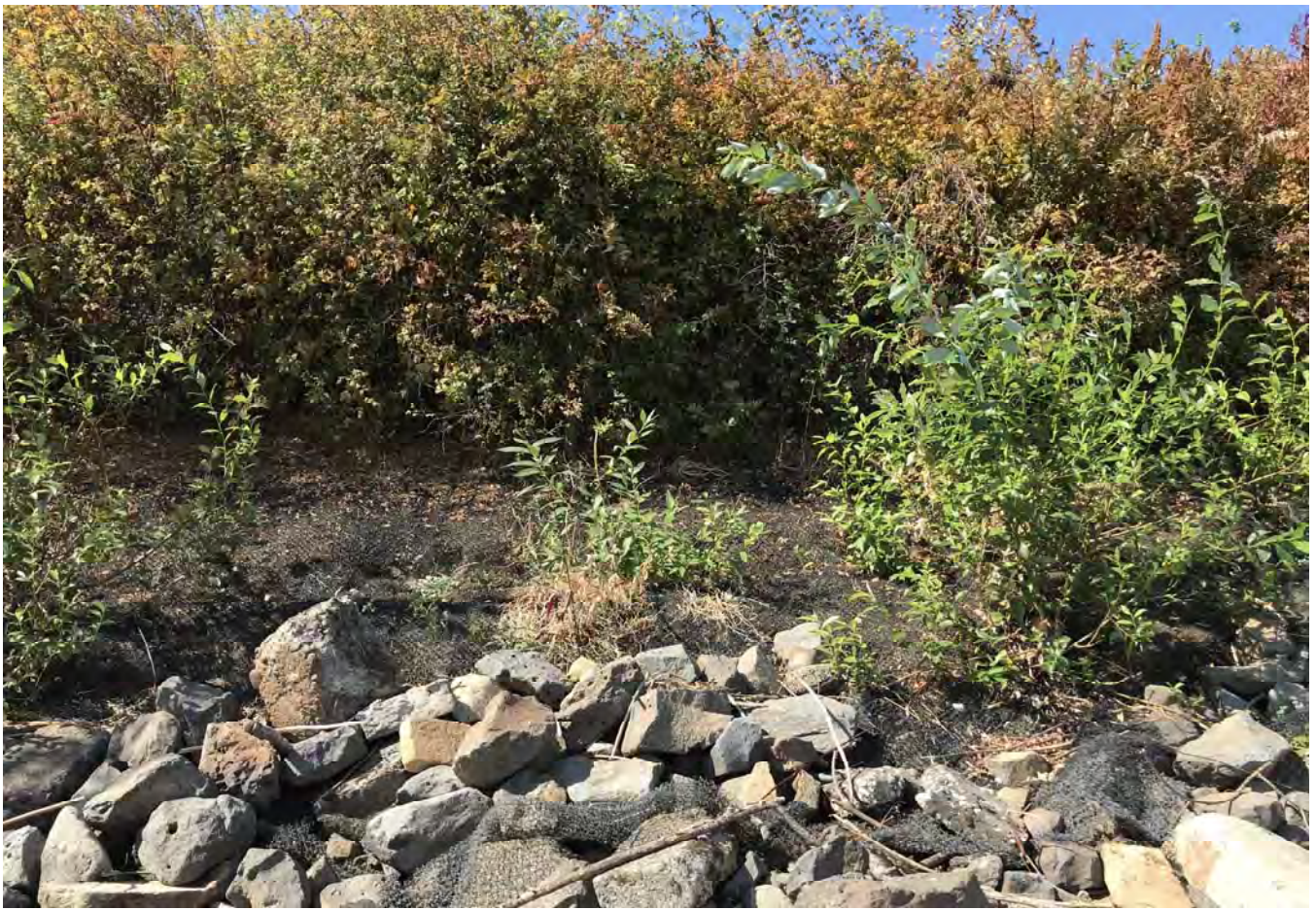
STA: 9+00 - Bottom of rock armor looking west.
