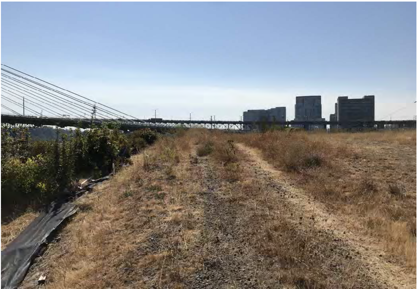
STA: 23+50 - Top of bank looking upstream.
