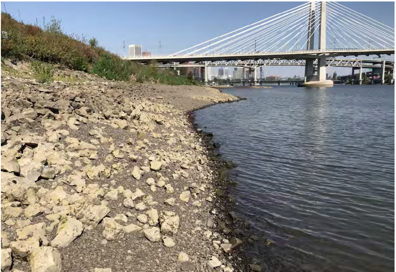
STA: 11+00 - Edge of water looking downstream.
