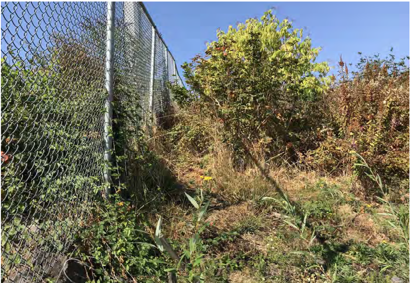
STA: 0+00 - Top of rock armor looking west.
