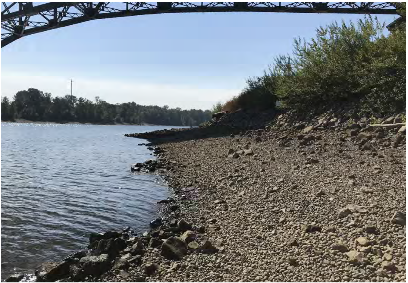
STA: 9+00 - Edge of water looking upstream.
