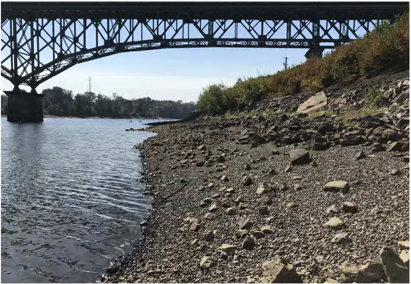
STA: 11+00 - Edge of water looking upstream.
