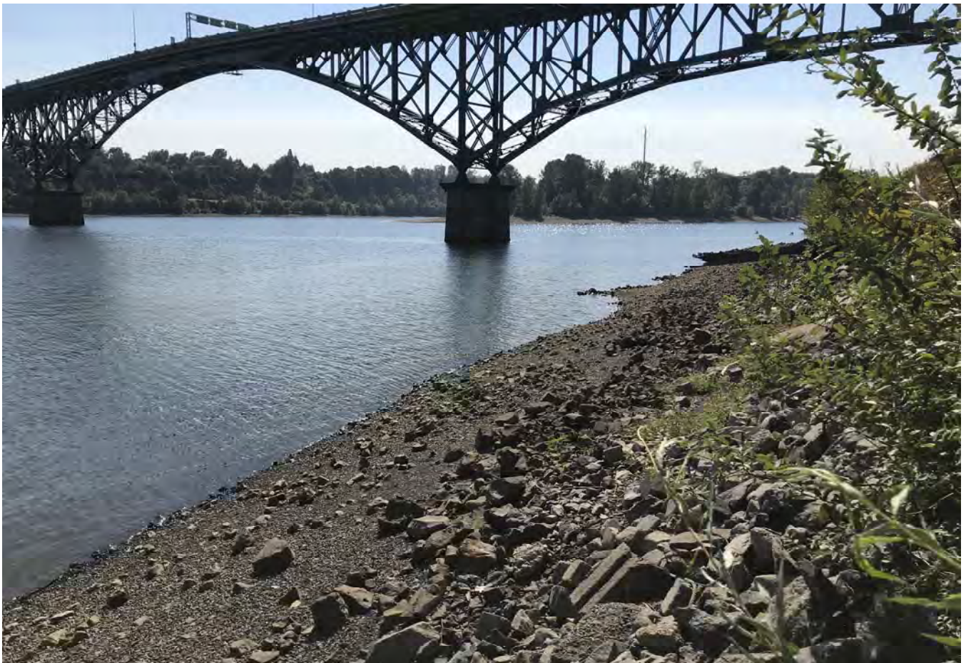
STA: 11+00 - Top of rock armor looking upstream.
