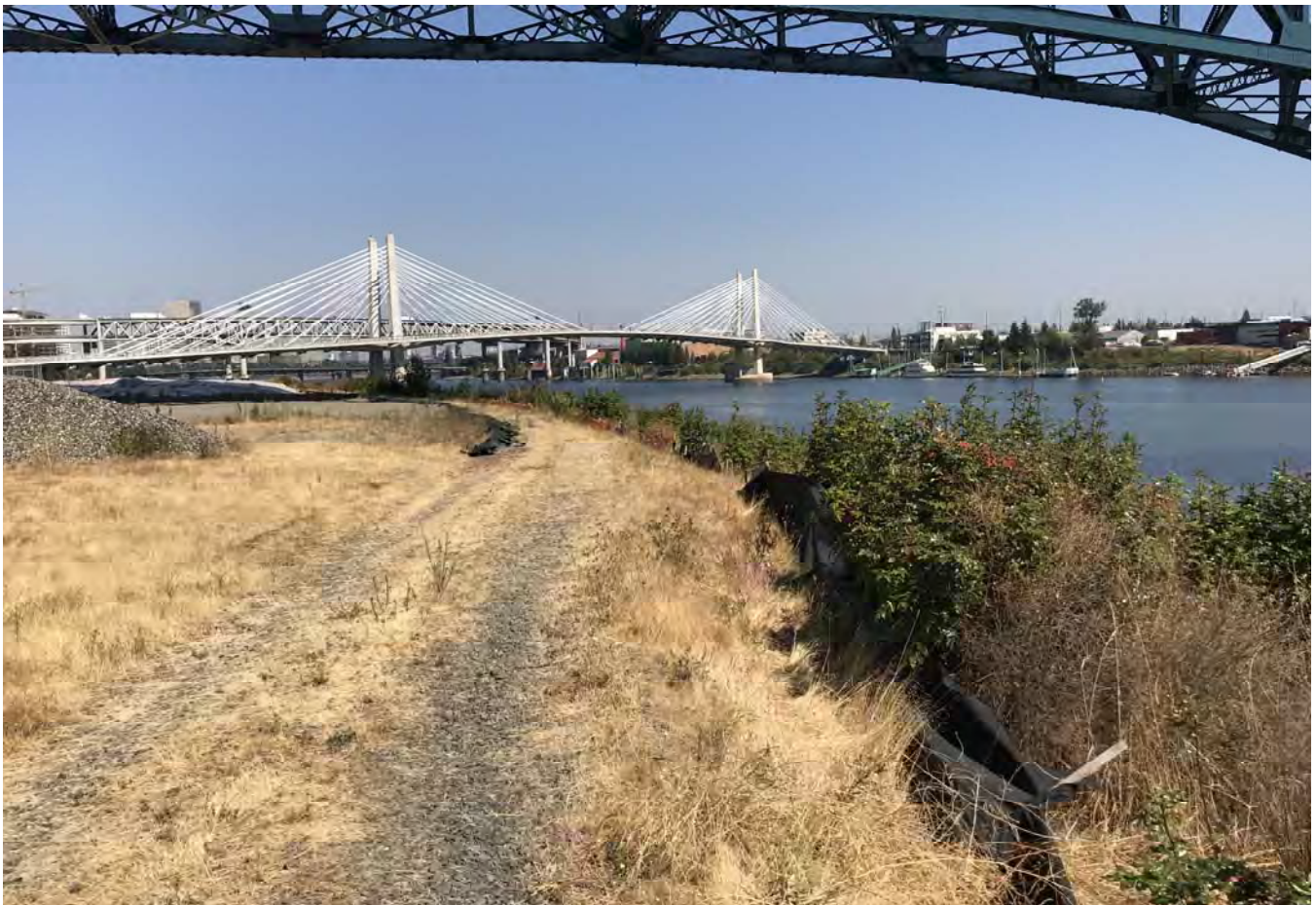
STA: 5+00 - Top of bank looking downstream.
