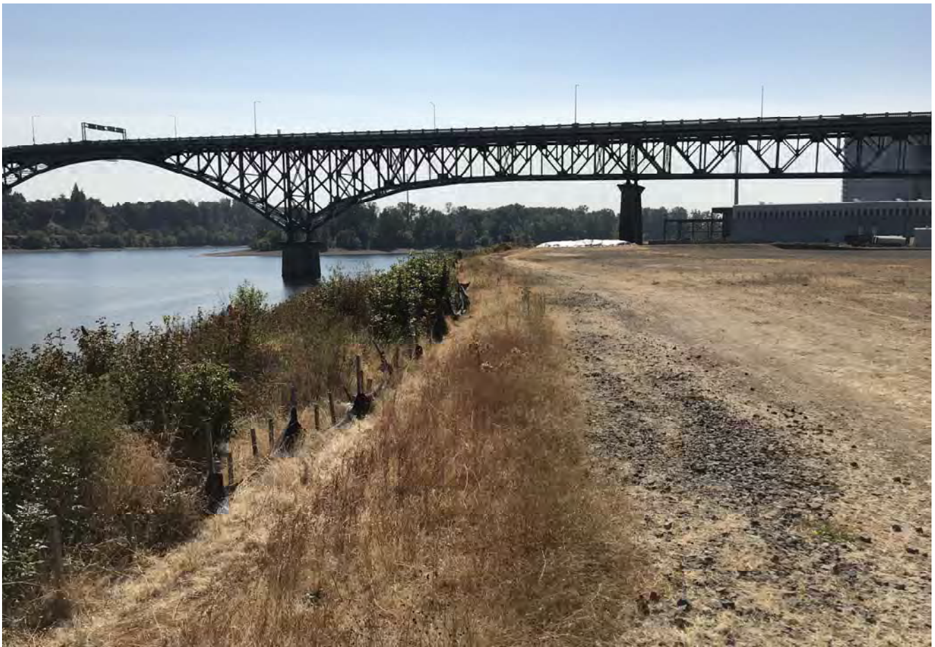
STA: 13+00 - Top of bank looking upstream.
