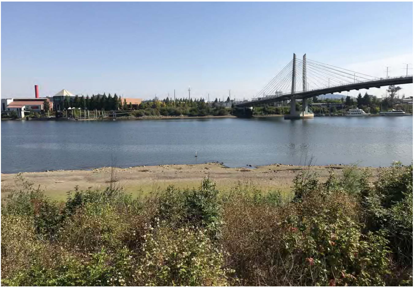
STA: 23+50 - Top of bank looking east.
