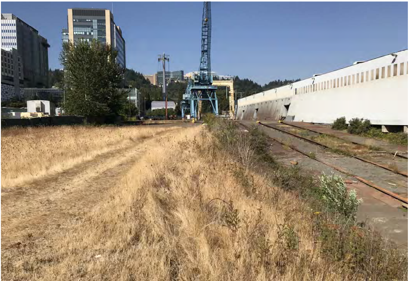
STA: 0+25 - Top of bank looking west.
