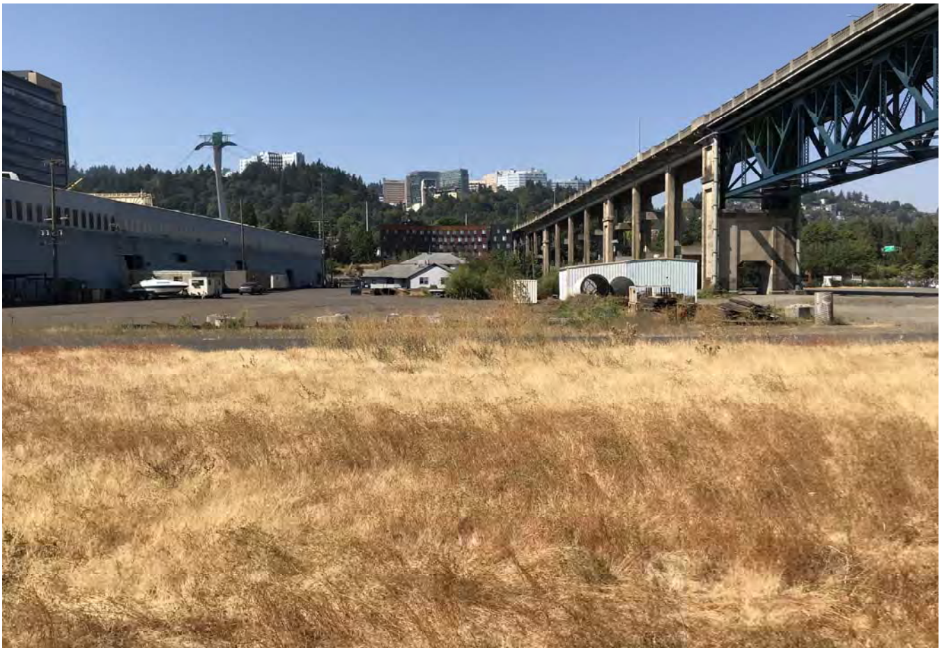
STA: 5+00 - Top of bank looking west.
