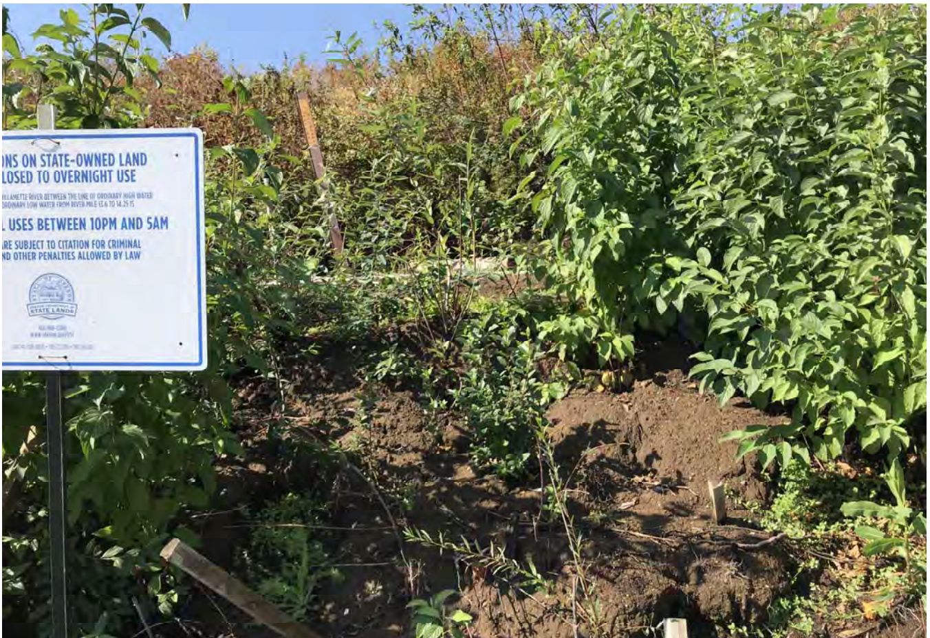
STA: 13+00 - Toe of slope looking west.
