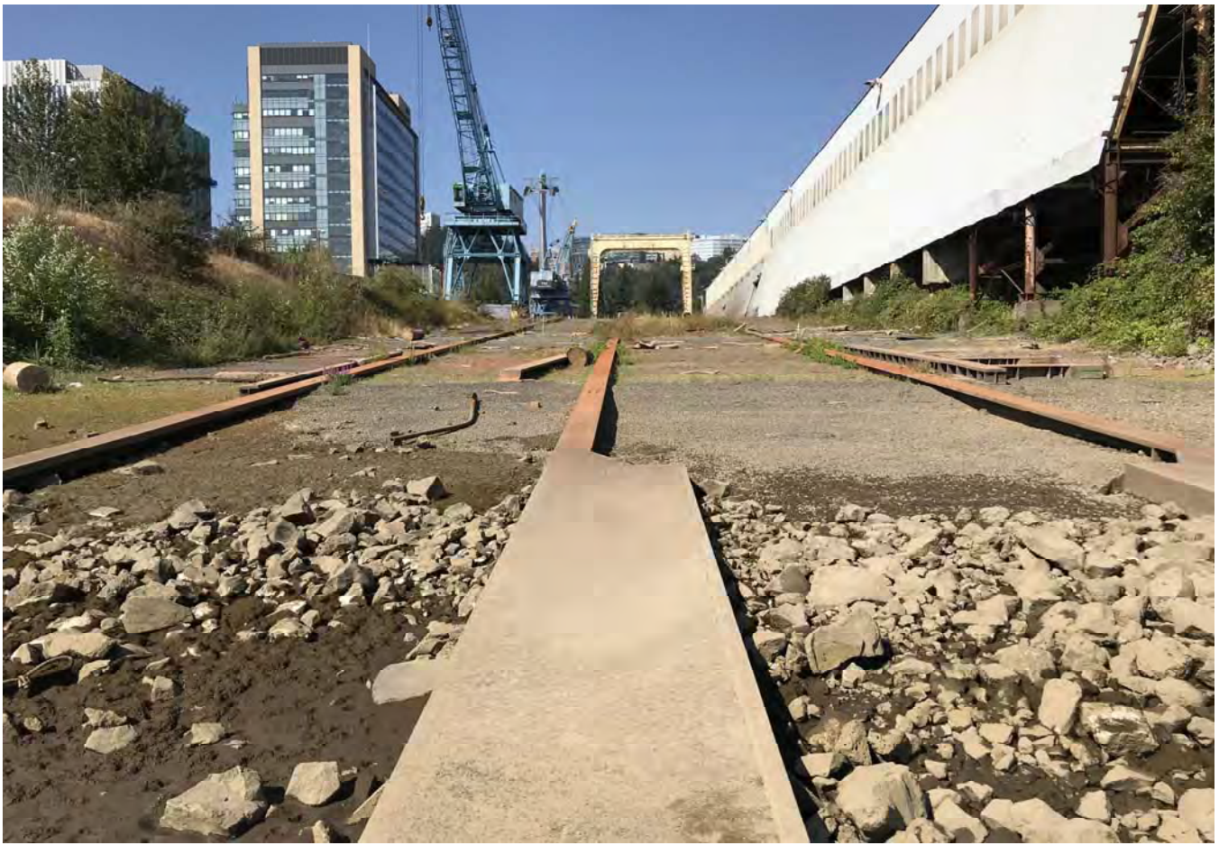
Slipway ramp looking west.
