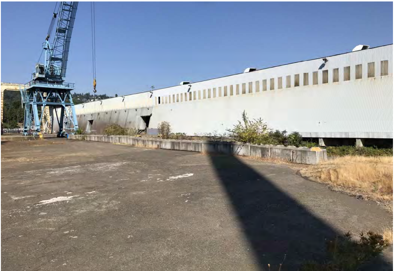
Edge of south slipway greenway looking northwest.
