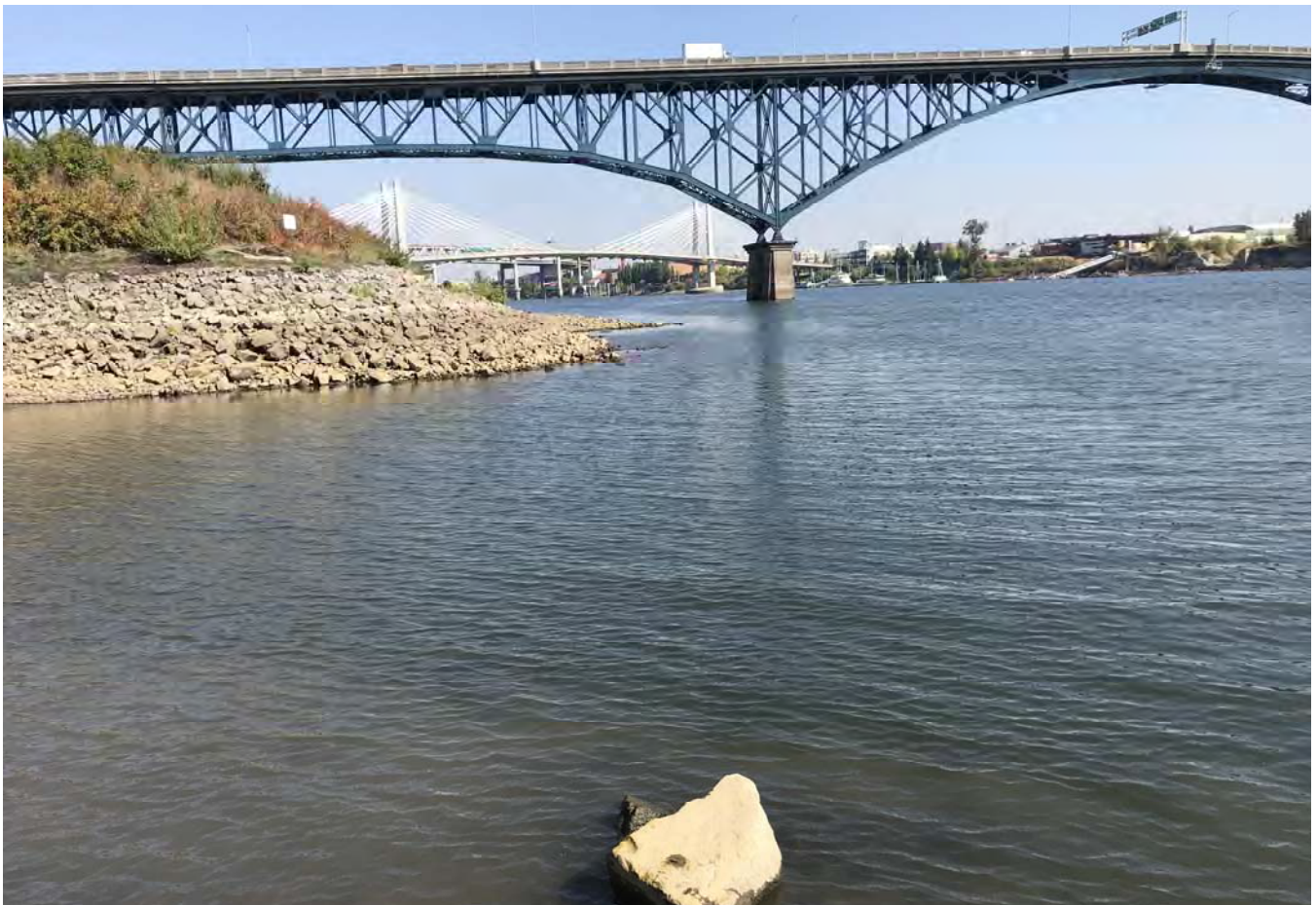
STA: 0+25 - Edge of water looking downstream.
