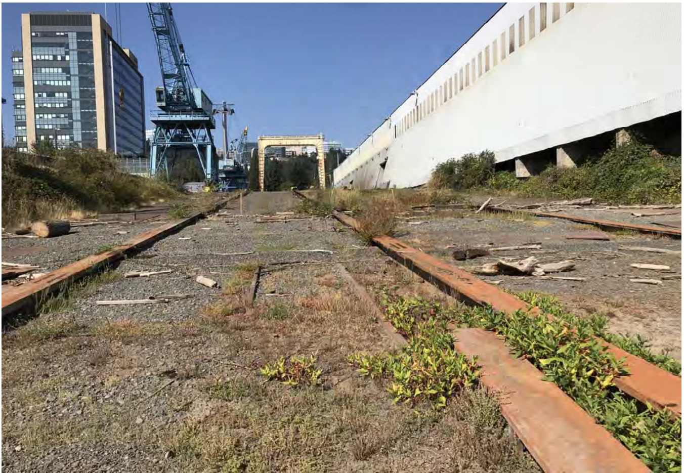
Slipway ramp looking west.
