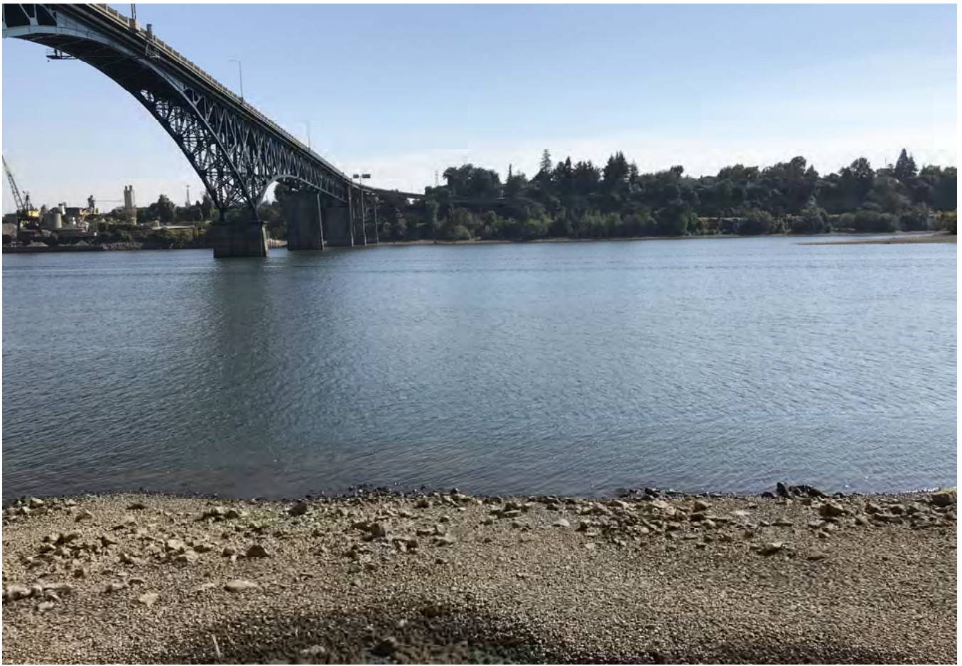
STA: 5+00 - Top of rock armor looking east.
