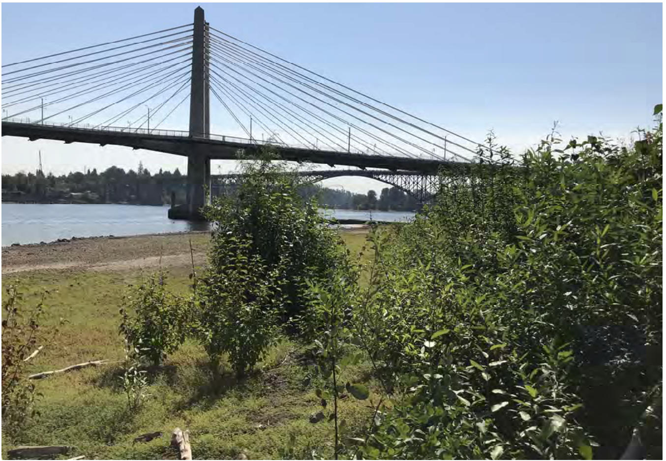
STA: 23+50 - Toe of slope looking upstream.
