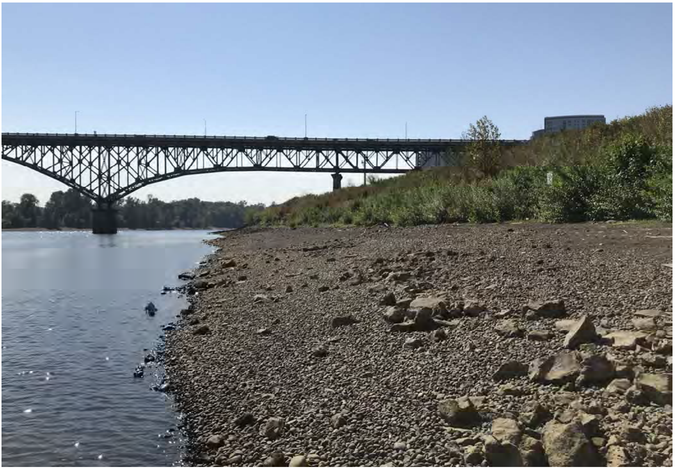
STA: 15+00 - Edge of water looking upstream.
