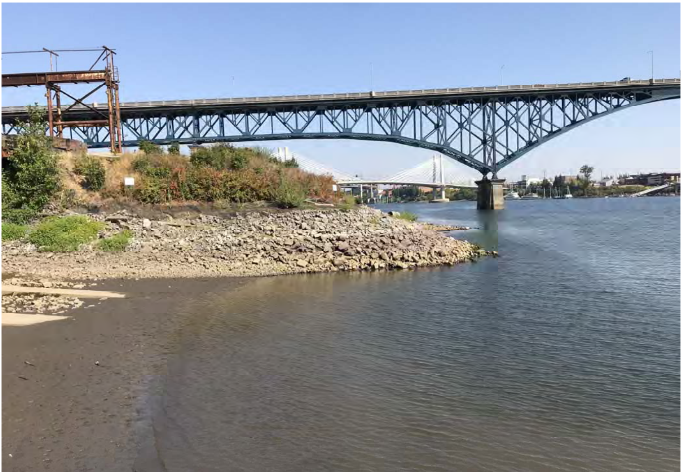
STA: 0+25 - Top of rock armor looking downstream.
