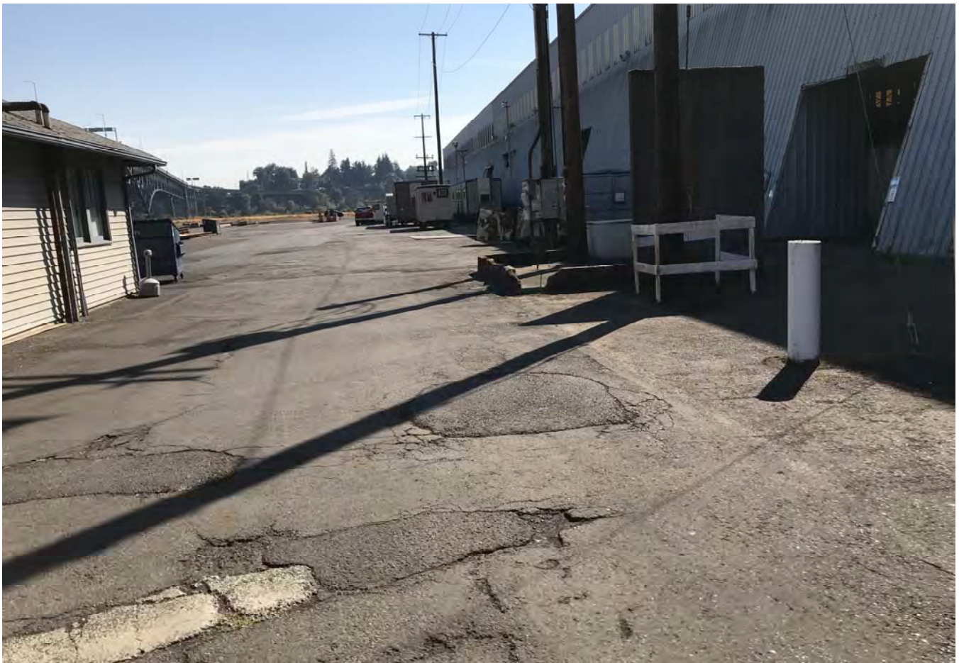
Office building looking east.
