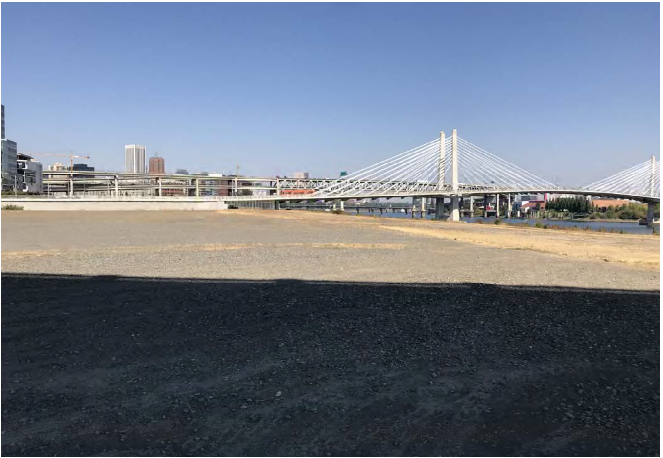
Upland cap, Southeast corner of site looking north.
