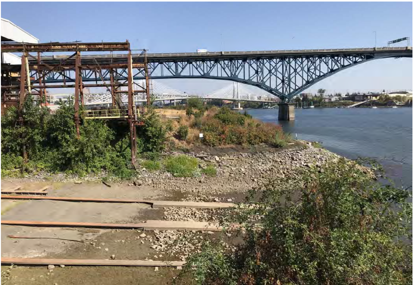
STA: 0+25 - Top of bank looking downstream.
