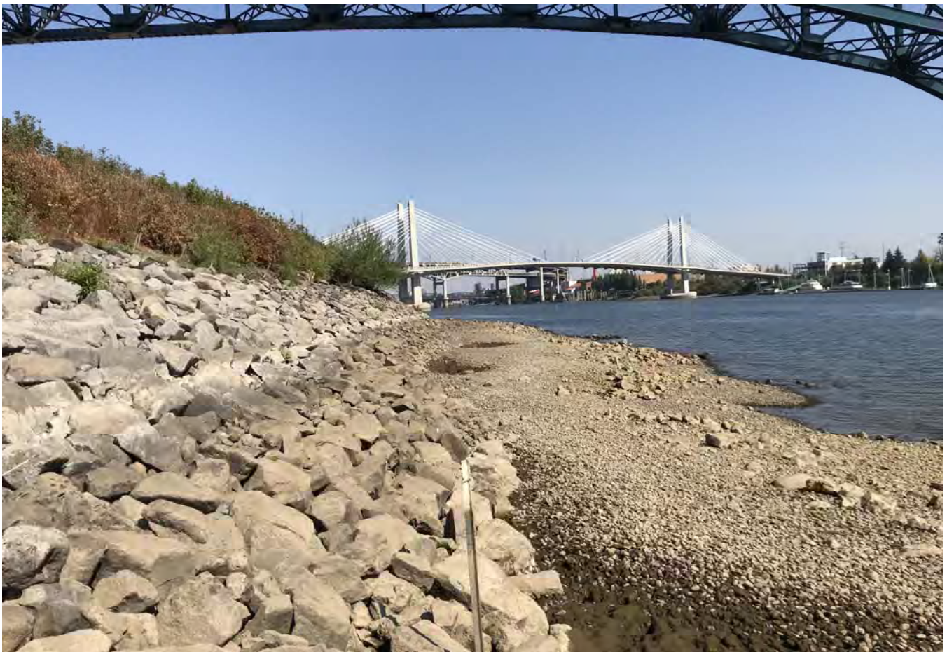
STA: 5+00 - Bottom of rock armor looking downstream.
