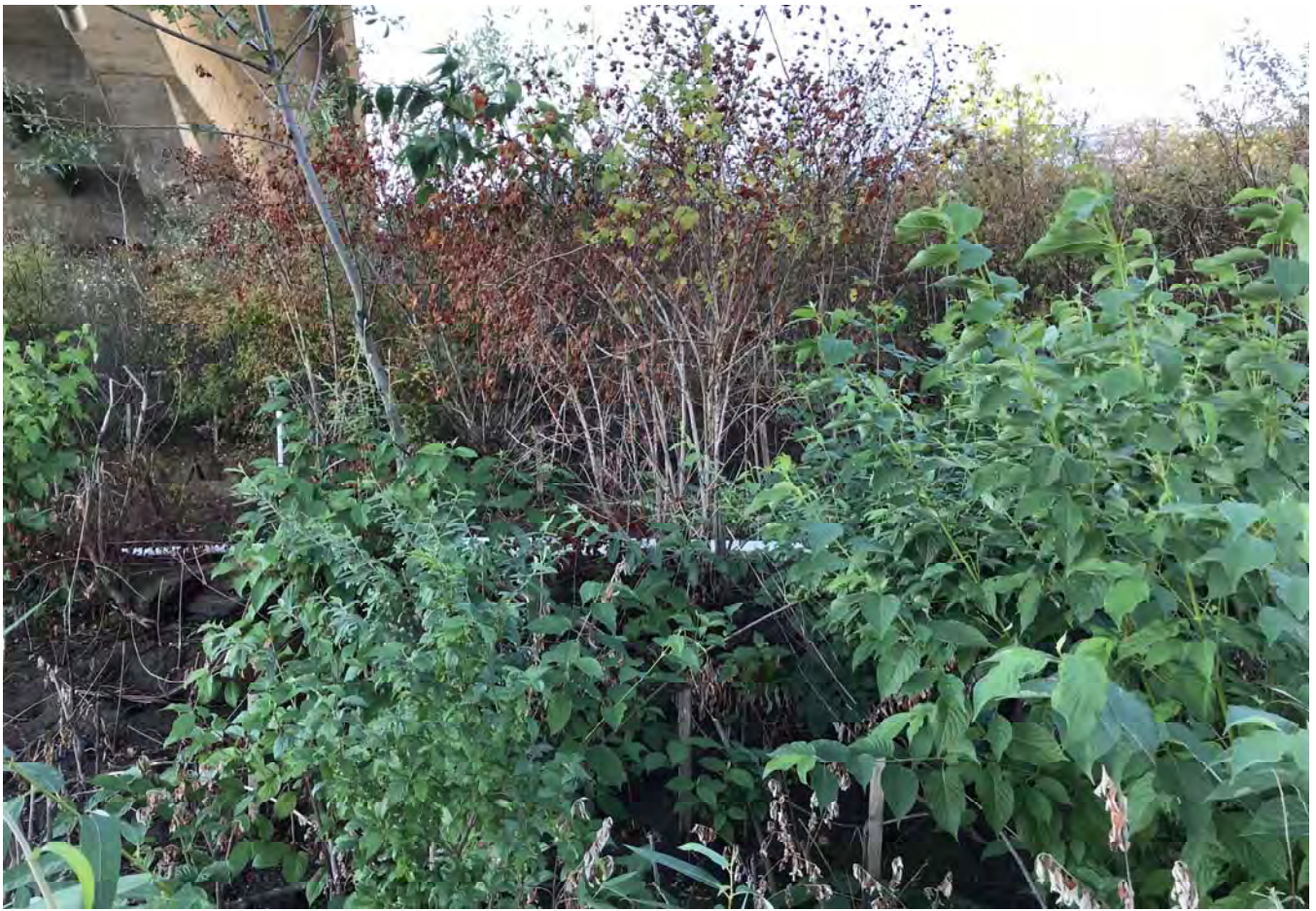
STA: 17+00 - Toe of slope looking west.
