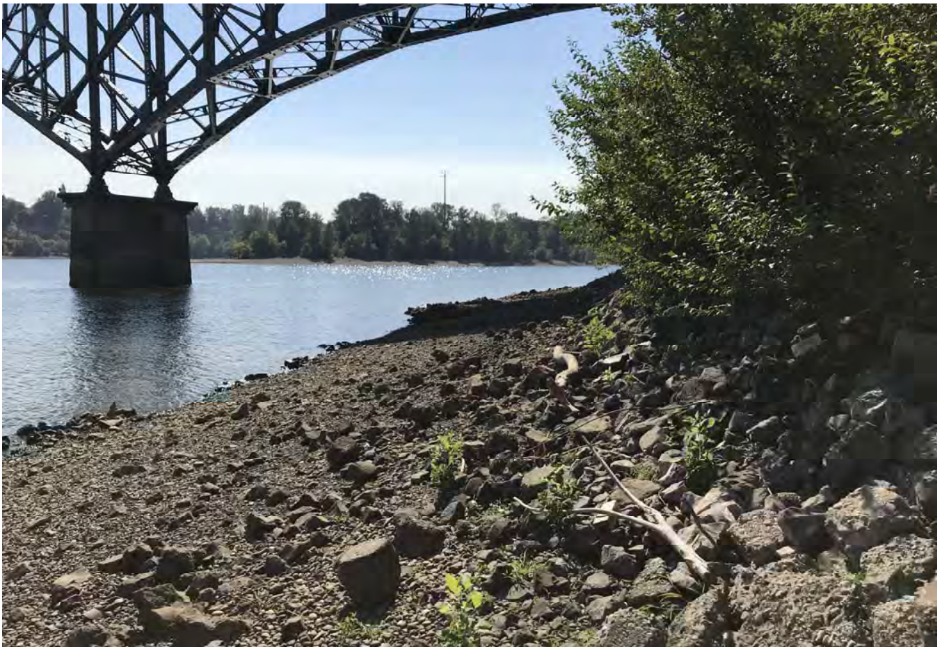
STA: 9+00 - Bottom of rock armor looking upstream.
