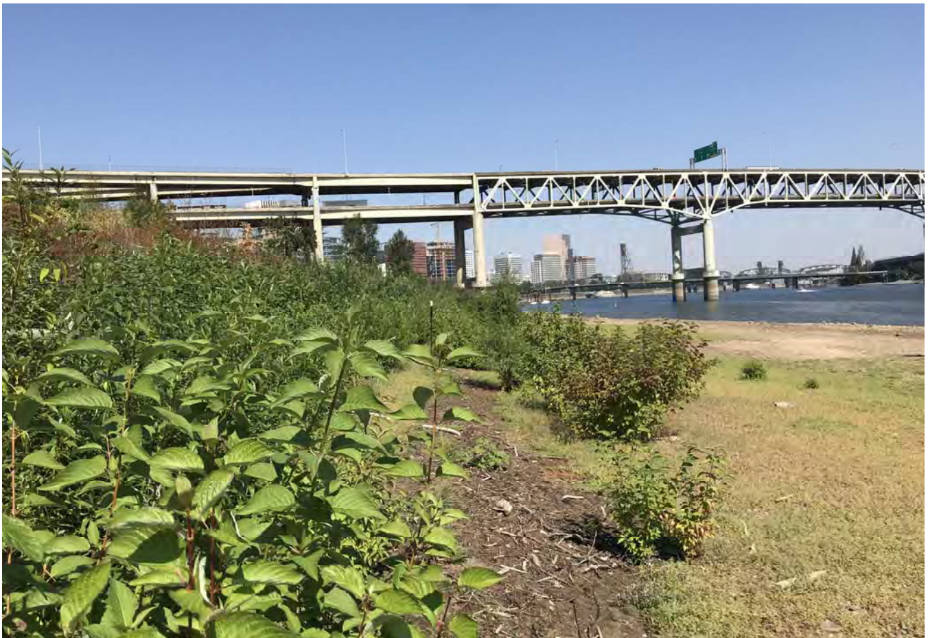
STA: 21+50 - Toe of slope looking downstream.
