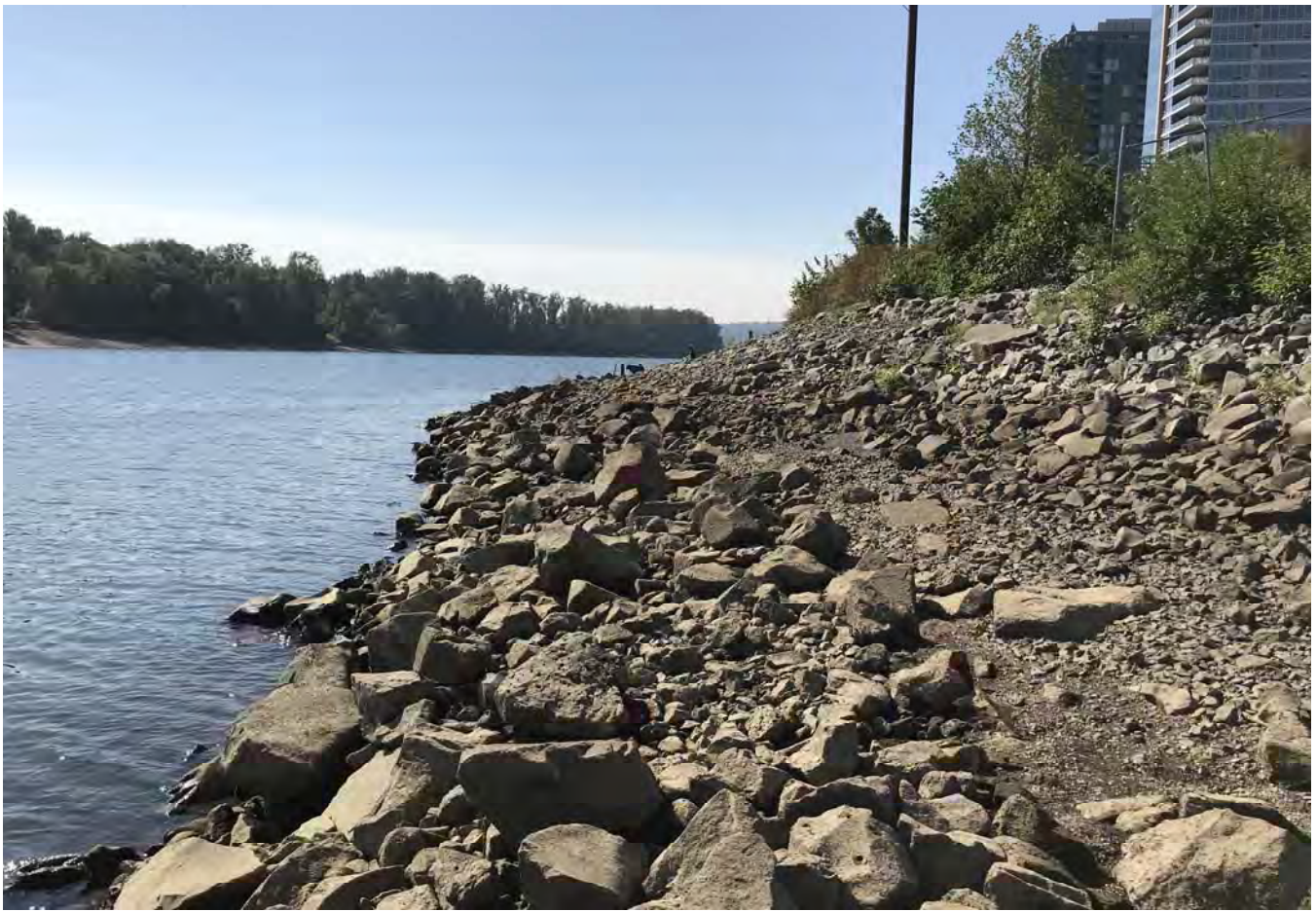
STA: 0+25 - Edge of water looking upstream.
