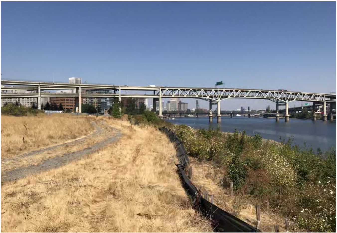
STA: 17+00 - Top of bank looking downstream.
