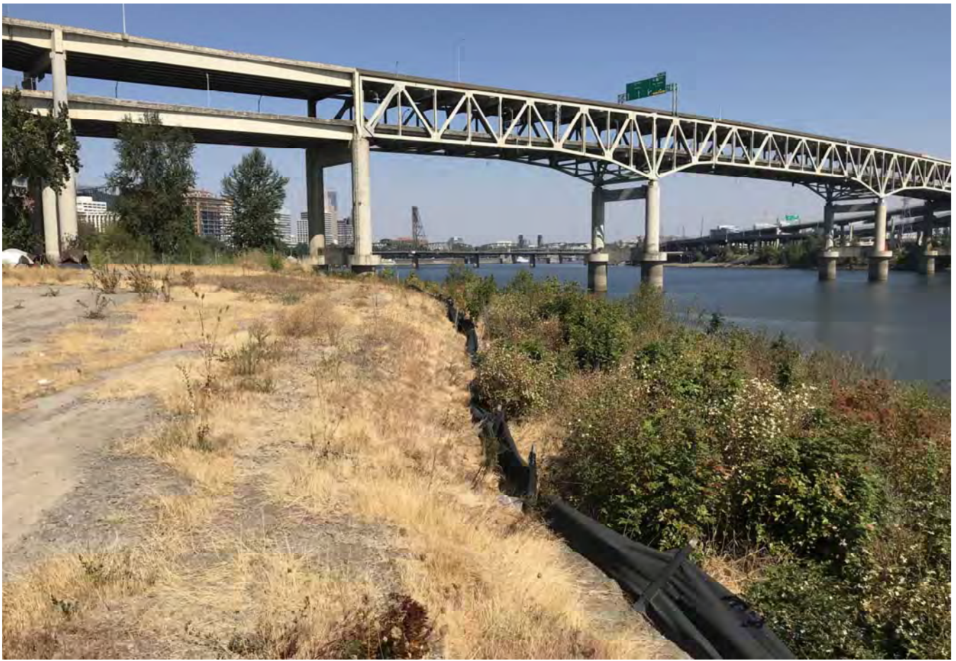
STA: 25+50 - Top of bank looking downstream.
