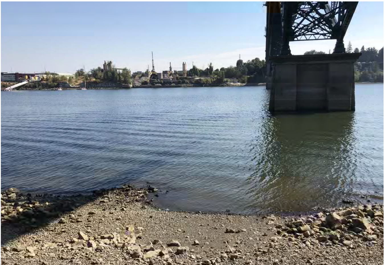
STA: 7+00 - Top of rock armor looking east.
