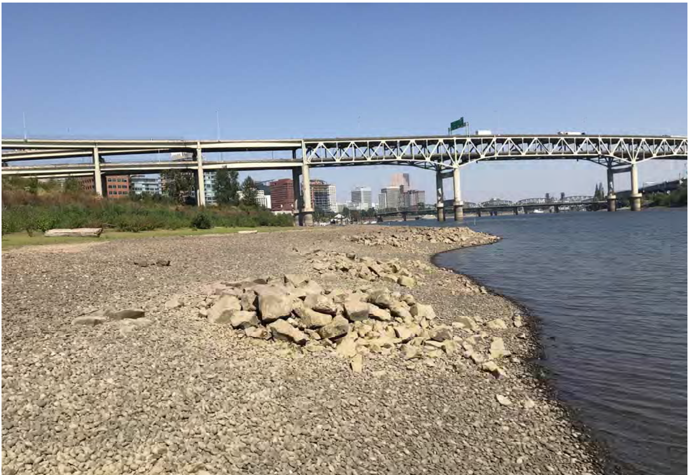
STA: 19+50 - Edge of water looking downstream.
