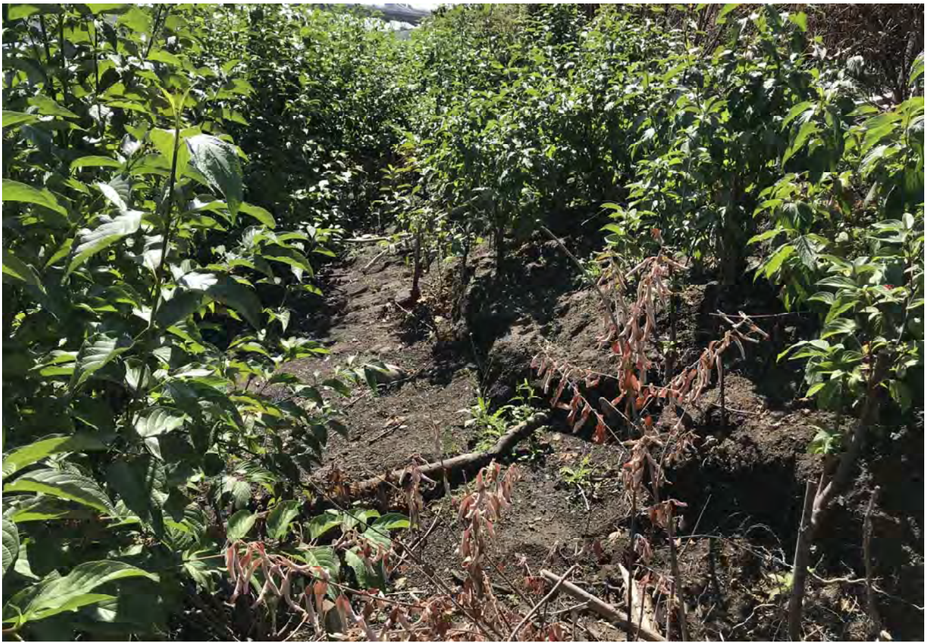
STA: 26+50 - Minor bank erosion on lower bank; with topsoil still in place.
