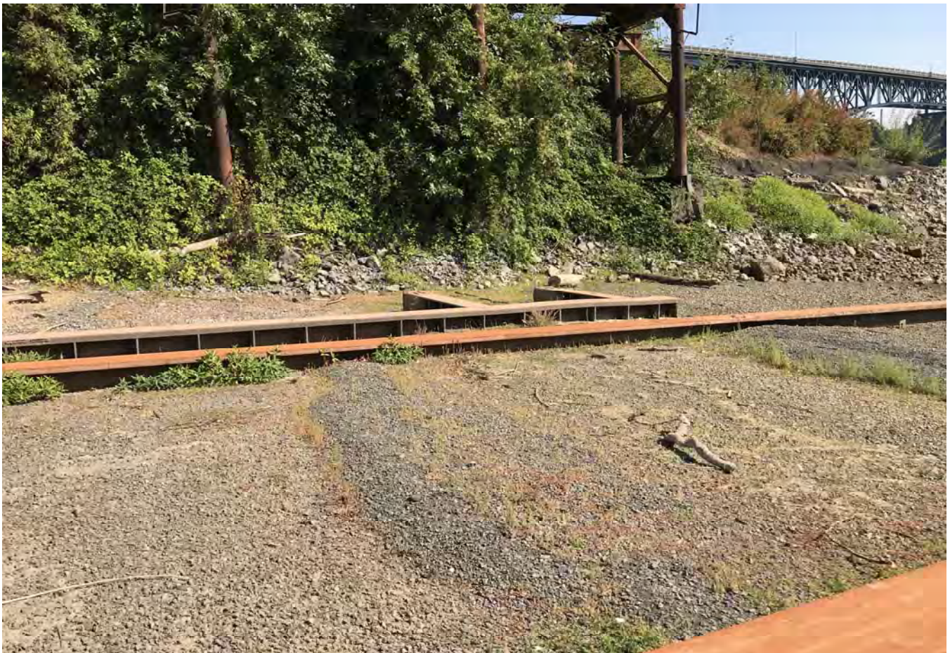
Slipway rails and barge building structure looking northeast.
