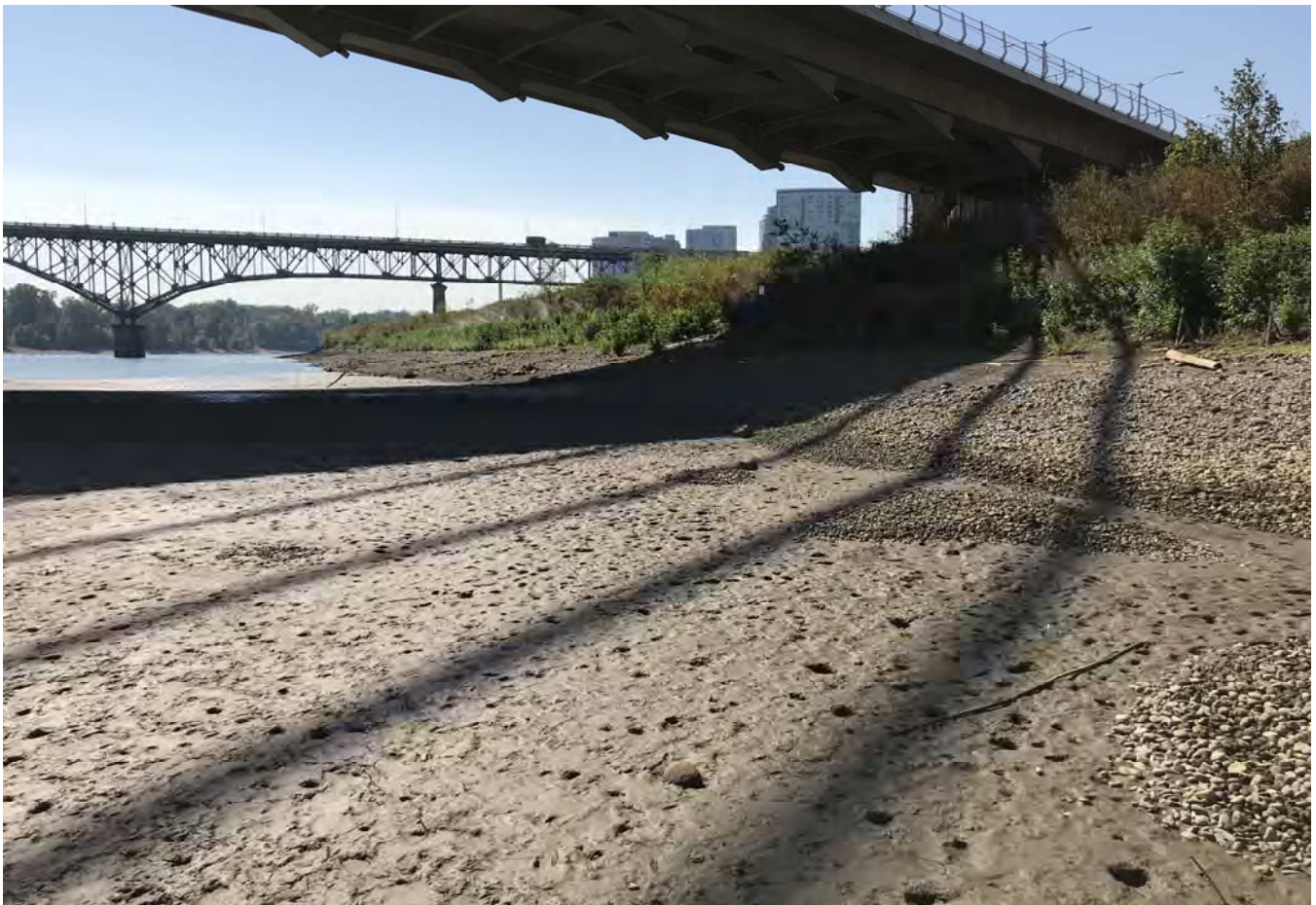
STA: 19+50 - Edge of water looking southwest.
