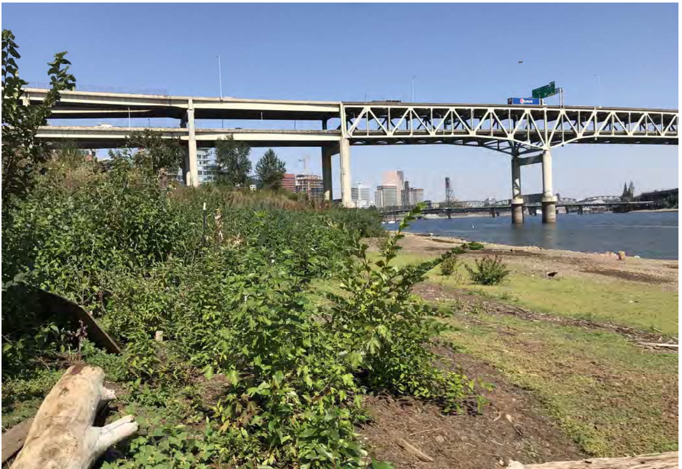
STA: 23+50 - Toe of slope looking downstream.
