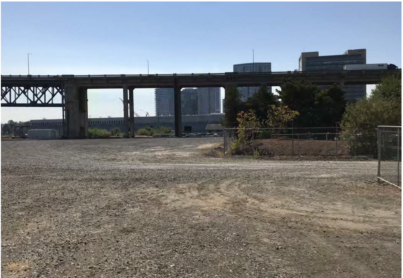
Upland cap center of site looking south.
