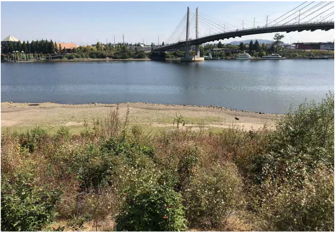
STA: 21+50 - Top of bank looking east.
