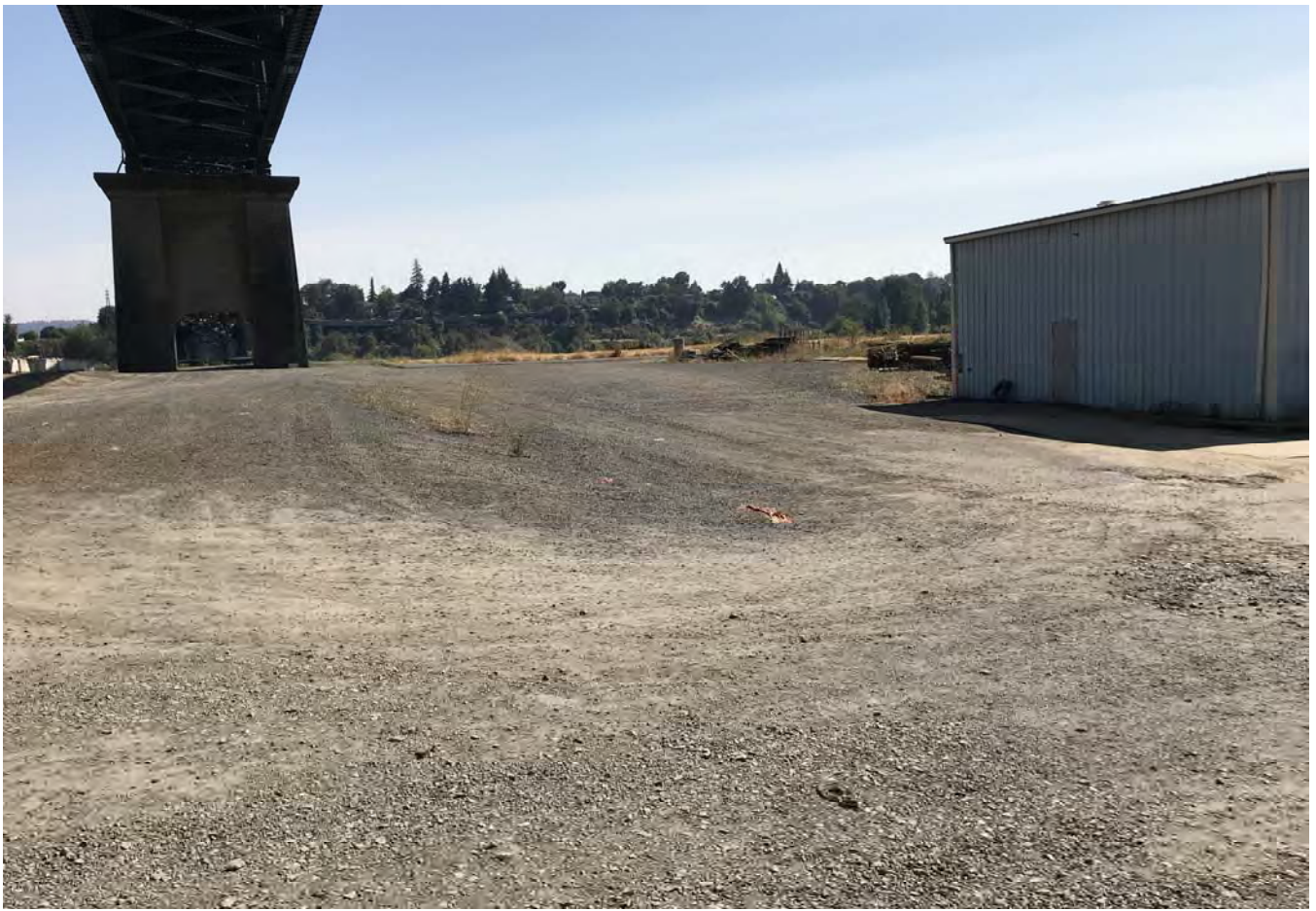
Operational area and boat building looking east.
