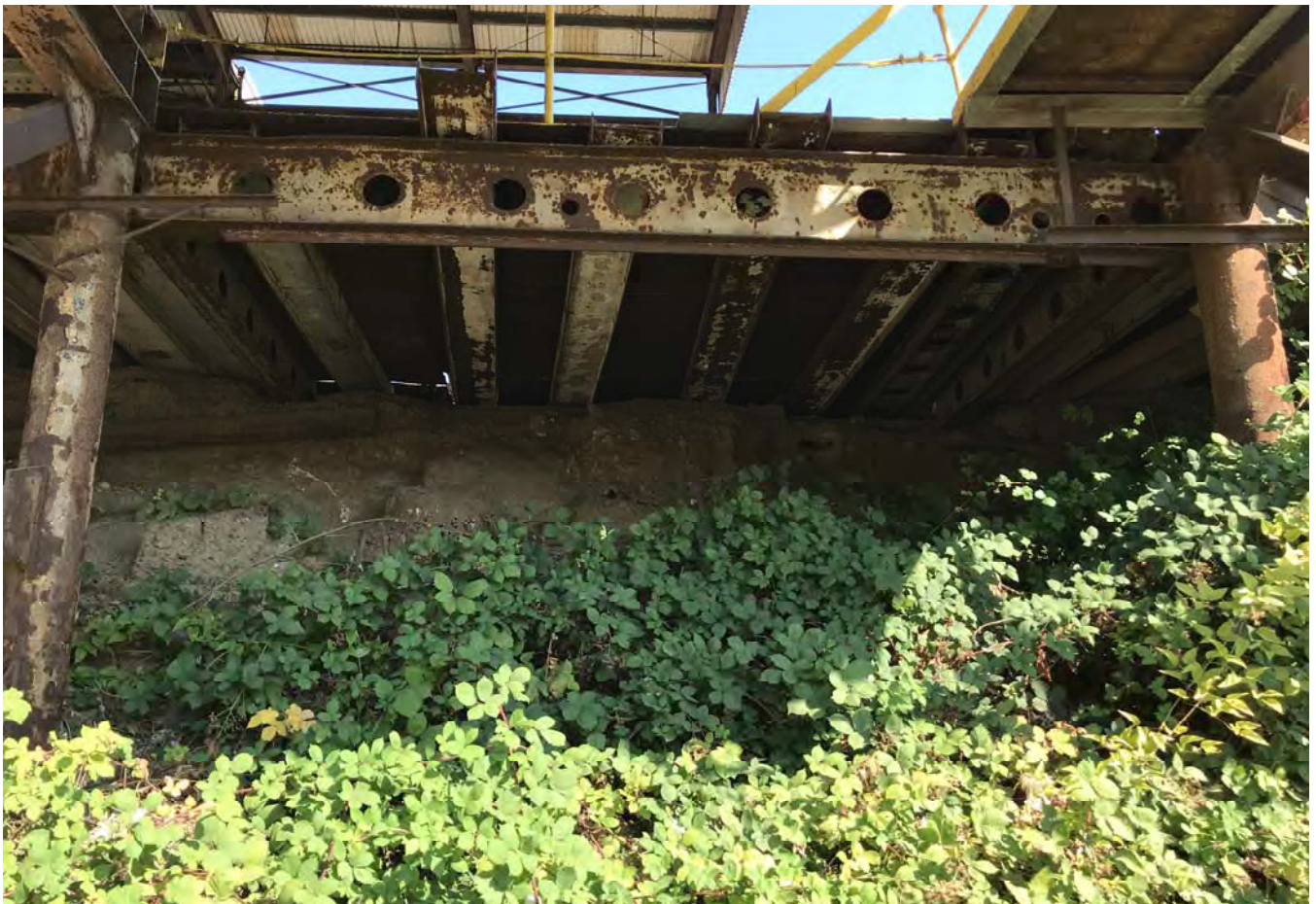
Underside of barge building structure looking north from slipway.
