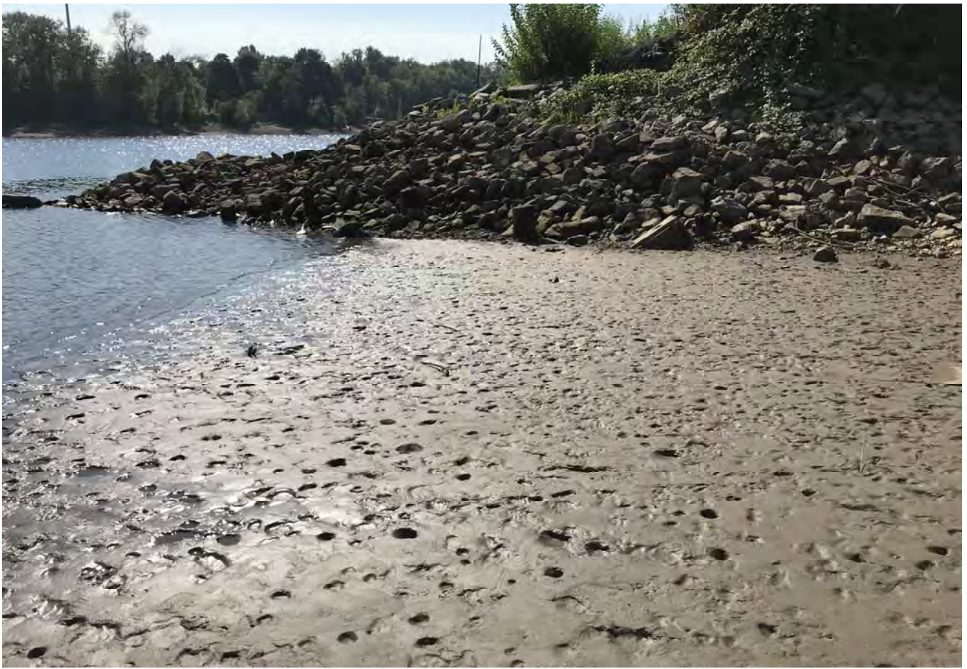
Sediment buildup in the slipway ramp looking southeast.
