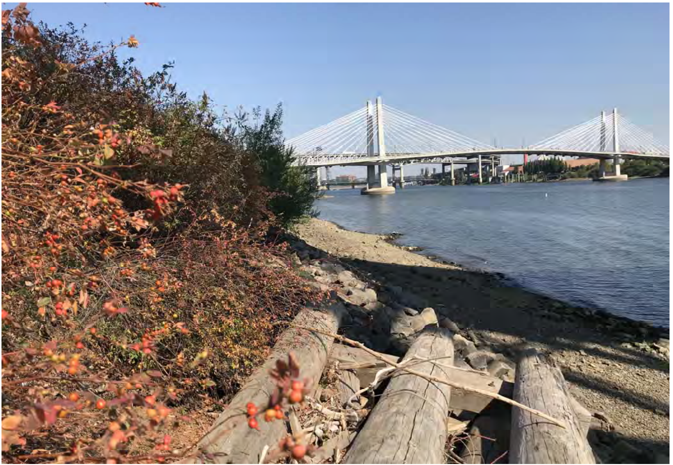
STA: 7+00 - Top of rock armor looking downstream.
