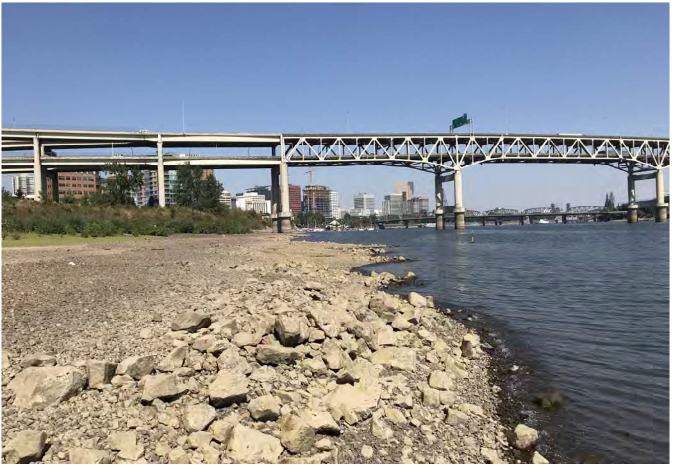
STA: 21+50 - Edge of water looking downstream.
