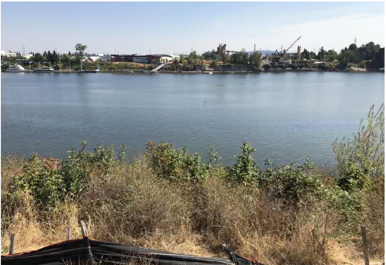
STA: 11+00 - Top of bank looking east.
