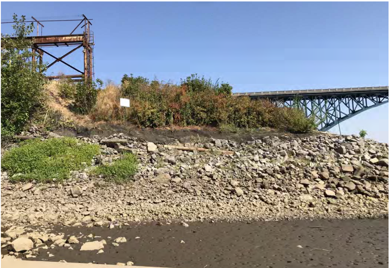
North slope of slipway ramp looking north.
