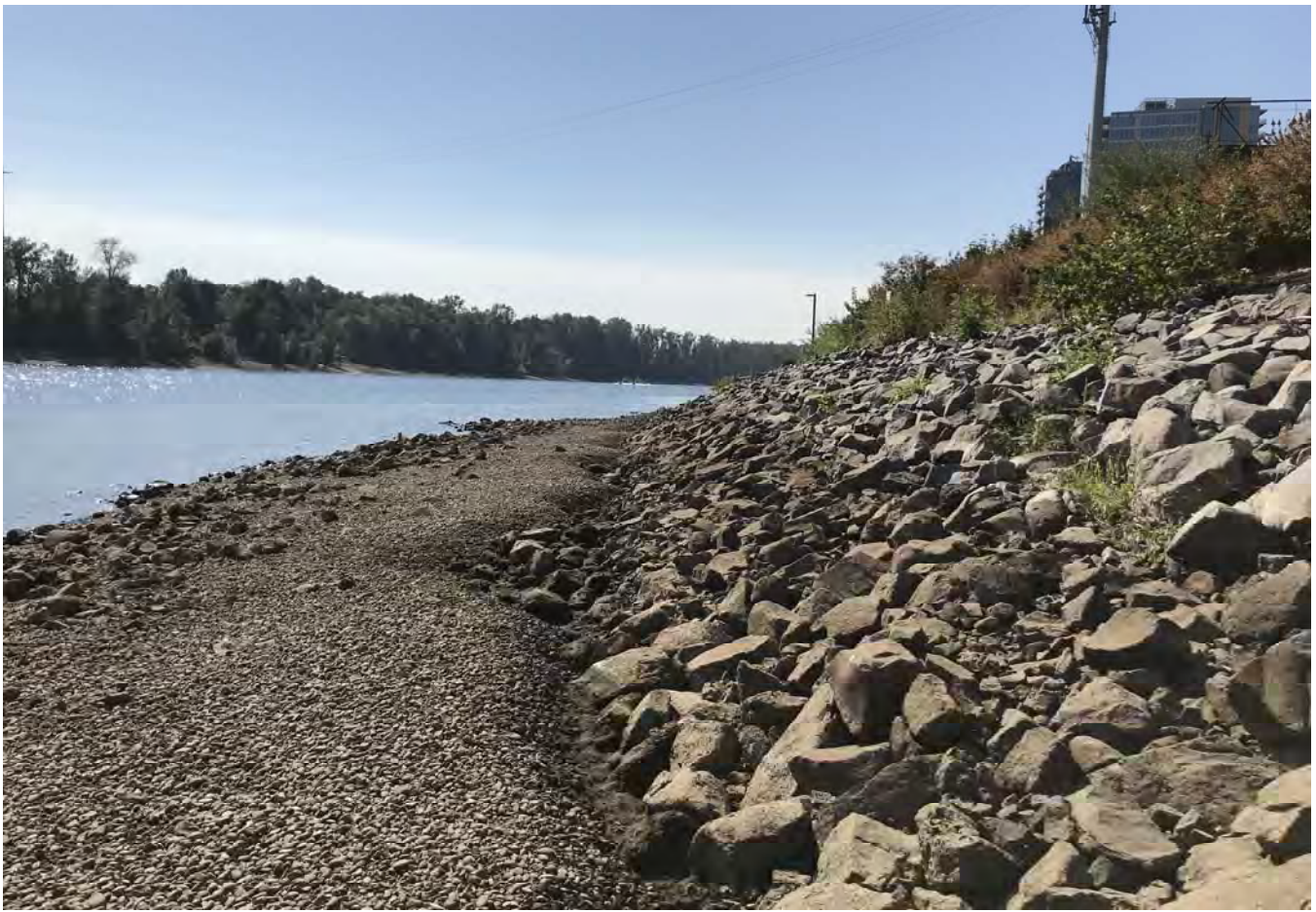
STA: 5+00 - Bottom of rock armor looking upstream.
