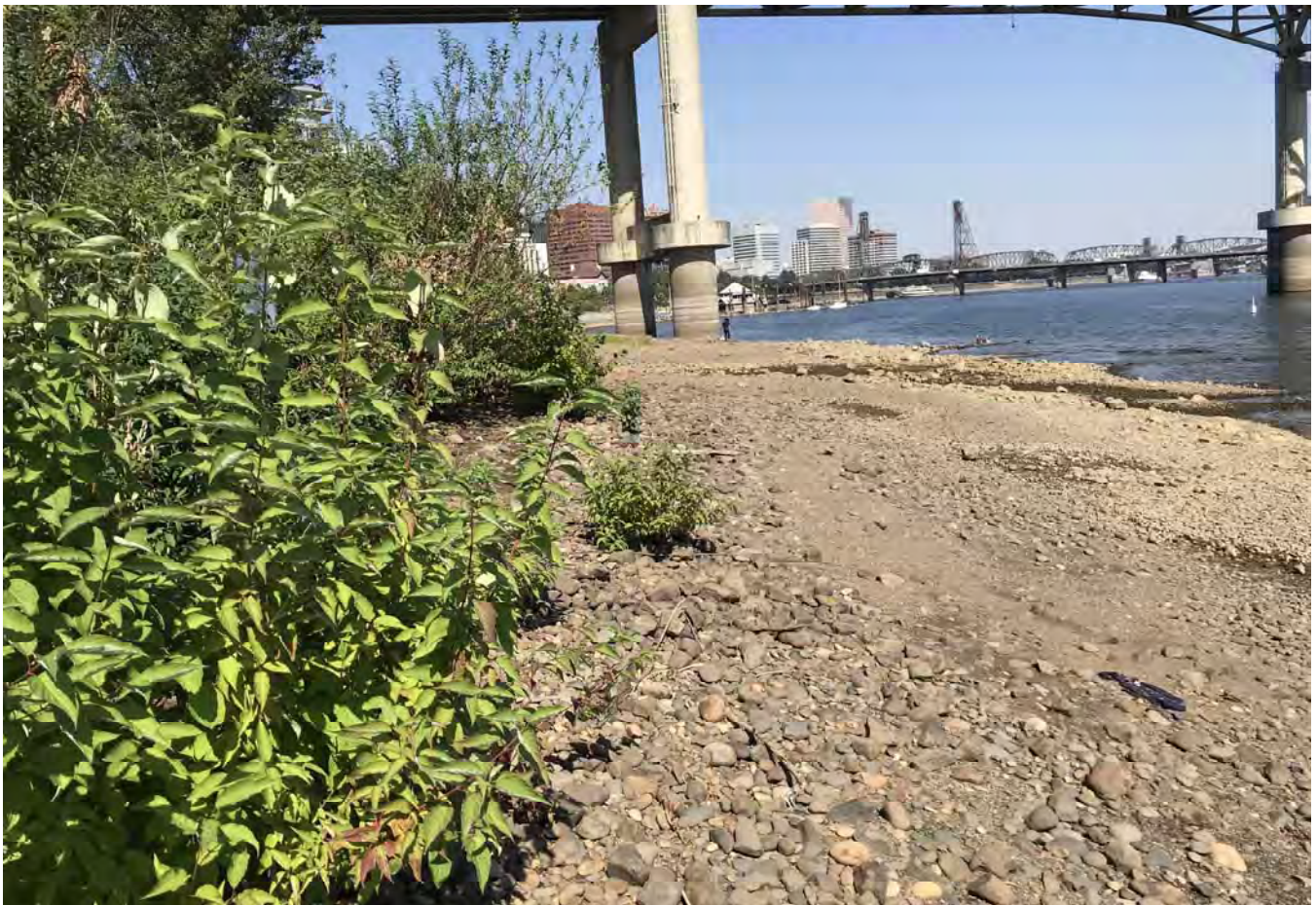
STA: 26+50 - Toe of slope looking downstream.
