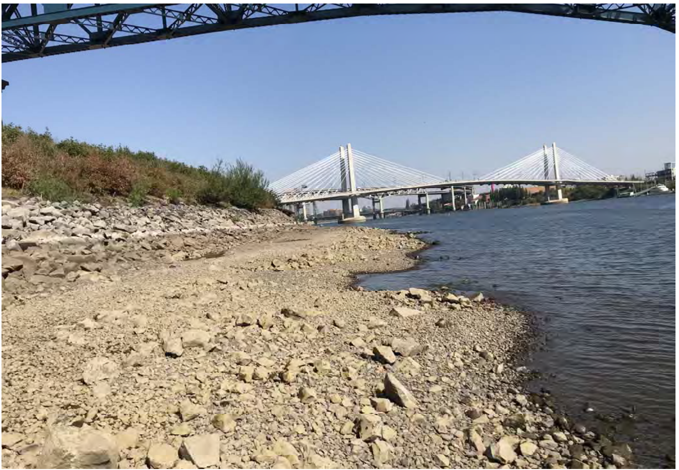
STA: 5+00 - Edge of water looking downstream.
