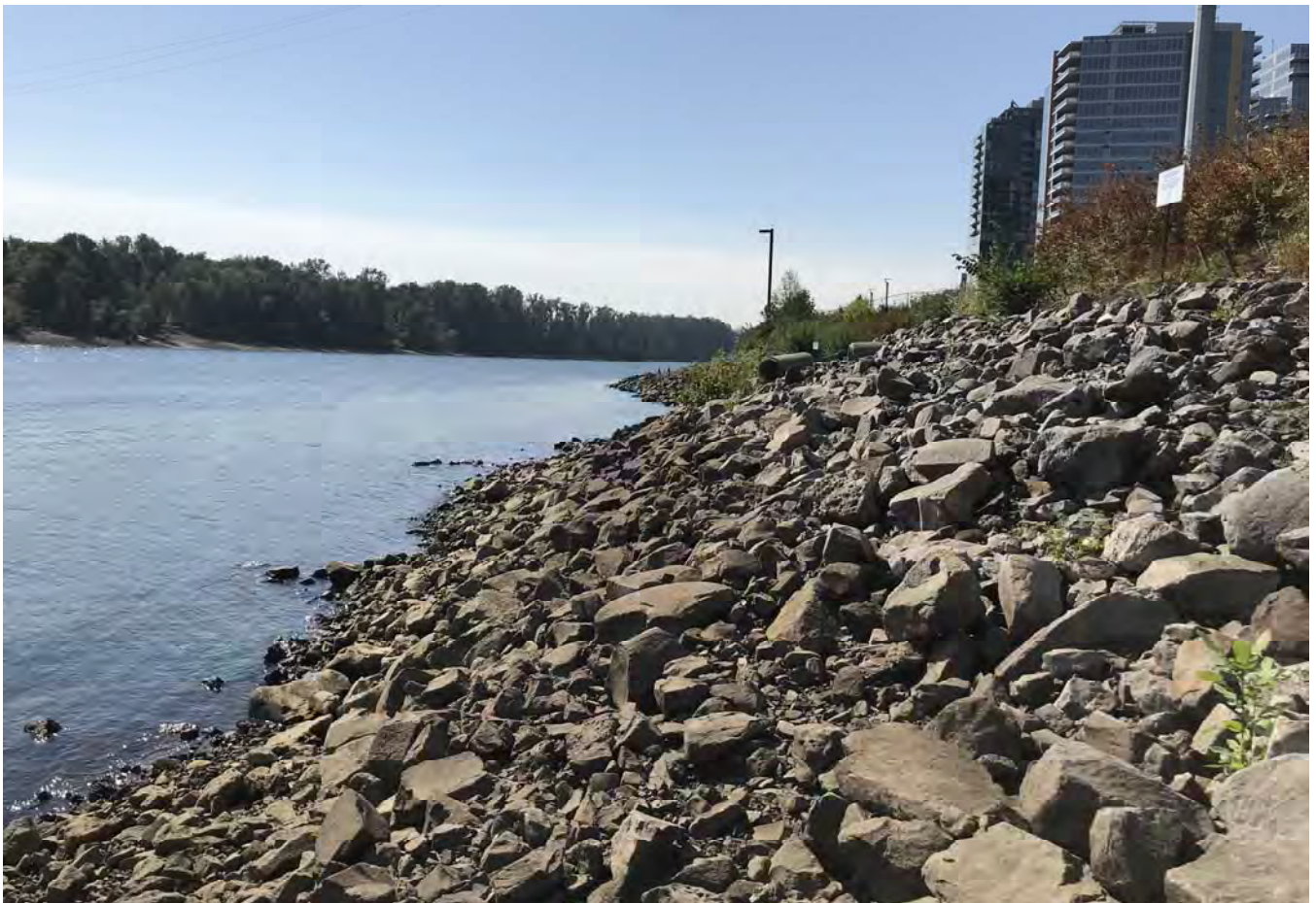
STA: 3+00 - Bottom of rock armor looking upstream.
