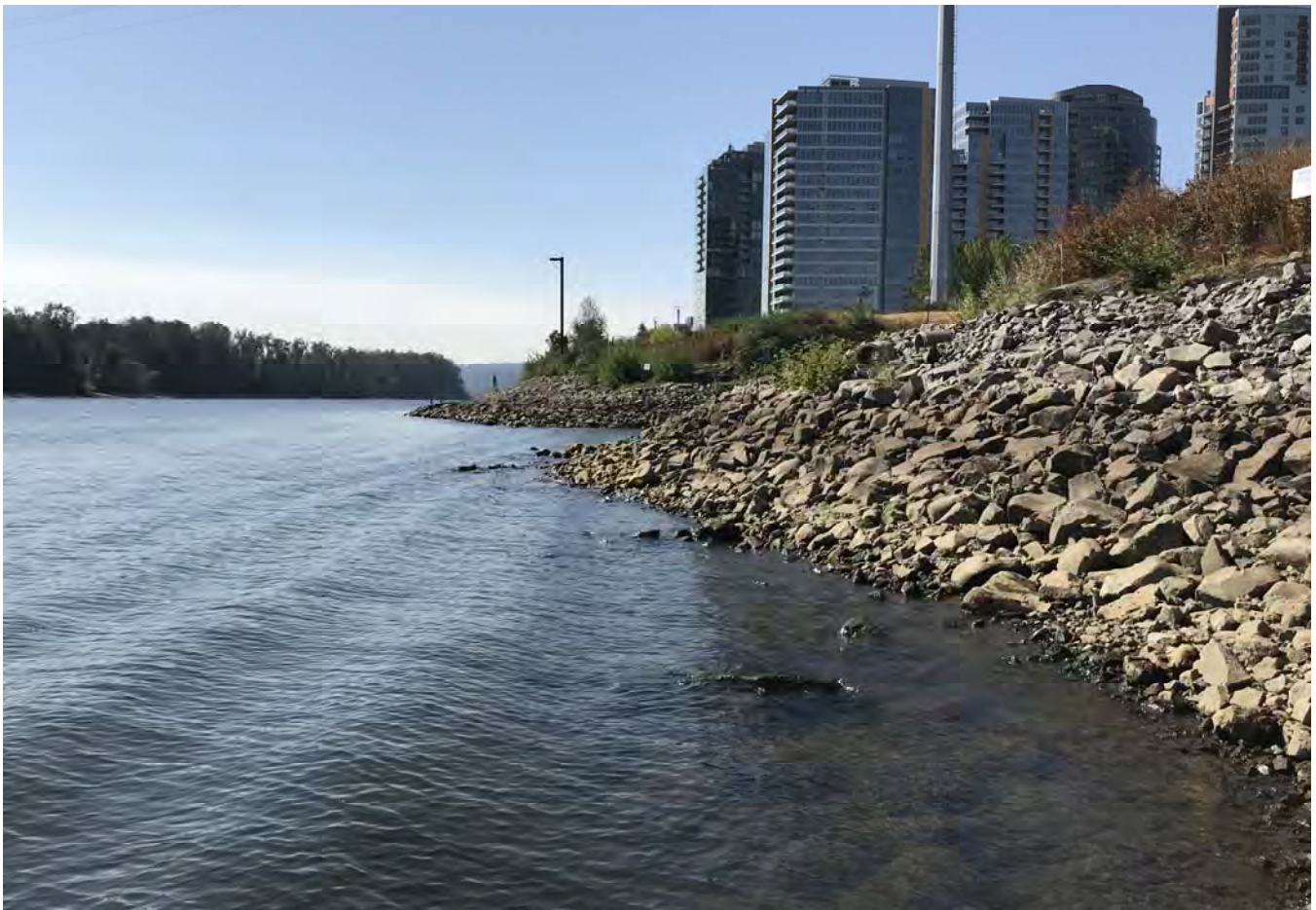
STA: 3+00 - Edge of water looking upstream.
