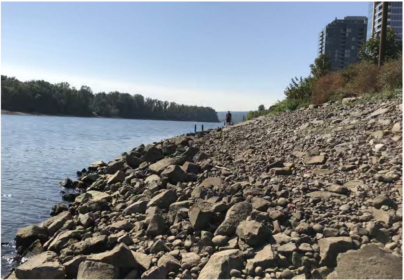
STA: 0+00 - Edge of water looking upstream.
