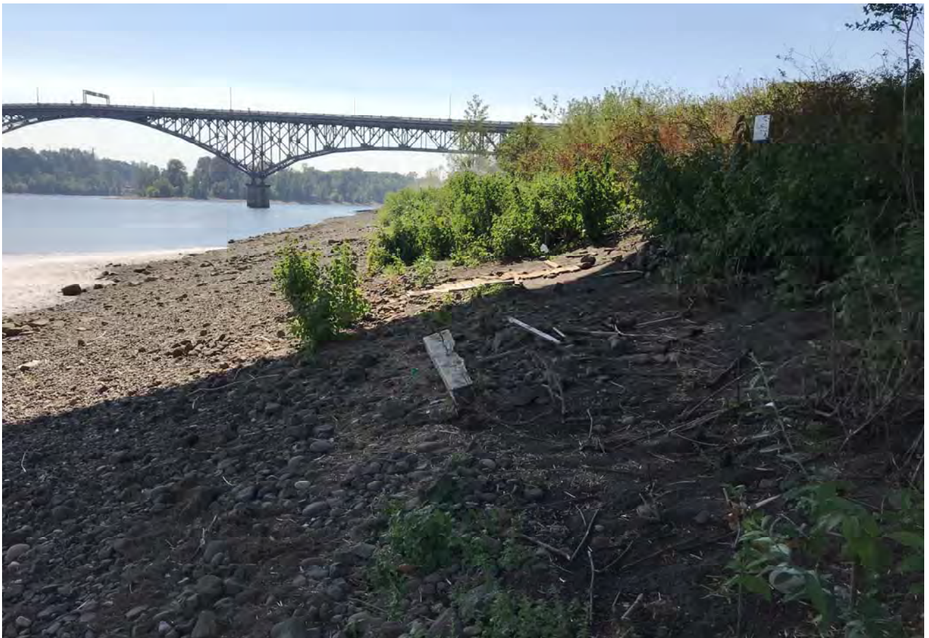
STA: 17+00 - Toe of slope looking upstream.
