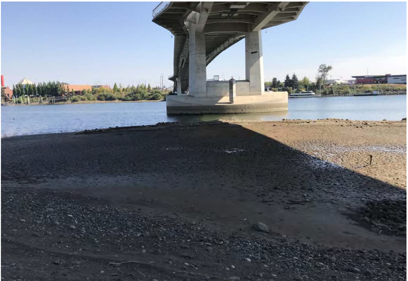
STA: 17+00 - Toe of slope looking east.
