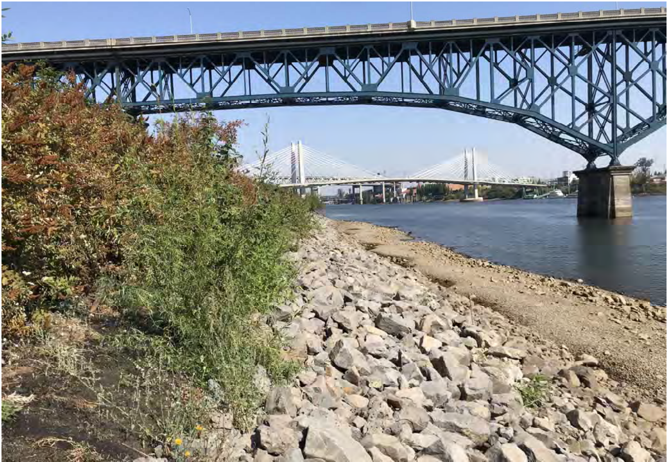
STA: 3+00 - Top of rock armor looking downstream.
