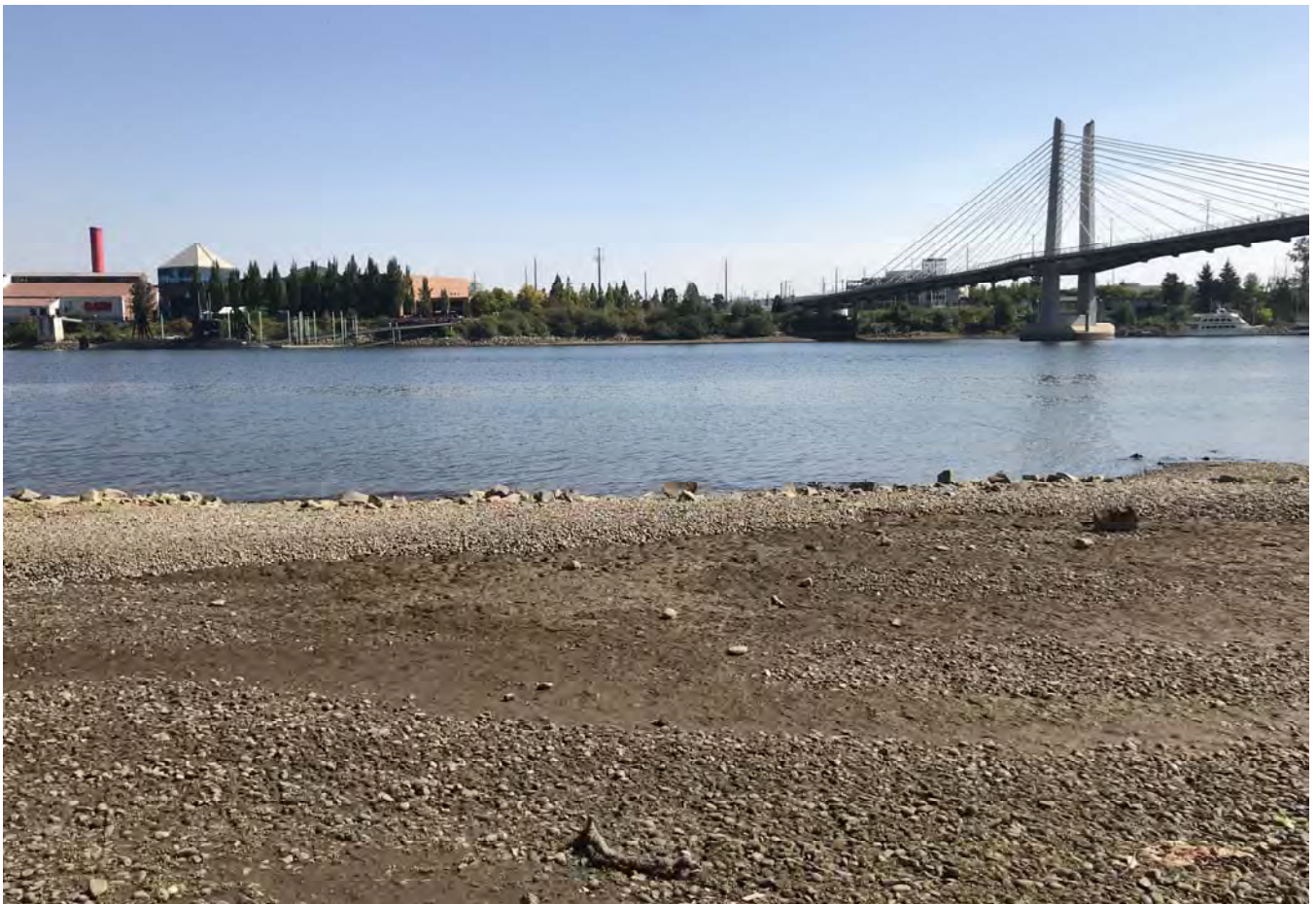
STA: 25+50 - Toe of slope looking east.
