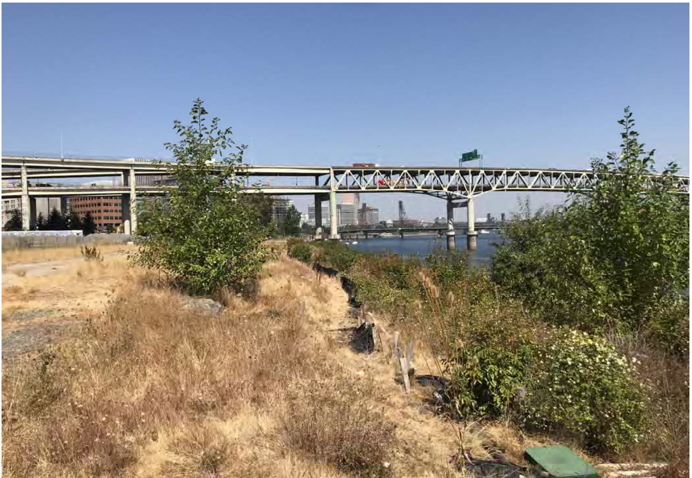
STA: 19+50 - Top of bank looking downstream.
