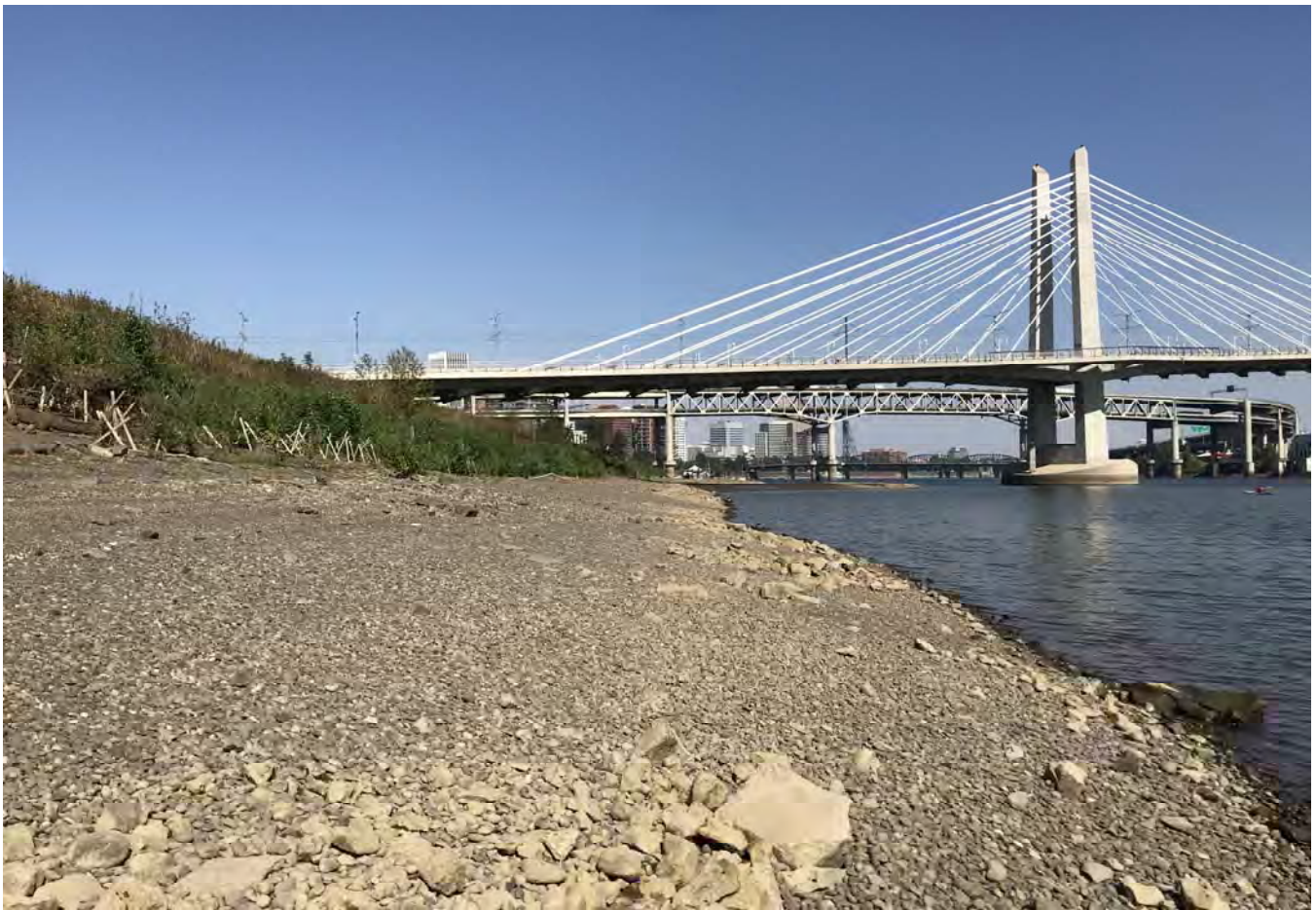
STA: 11+50 - Edge of water looking downstream.
