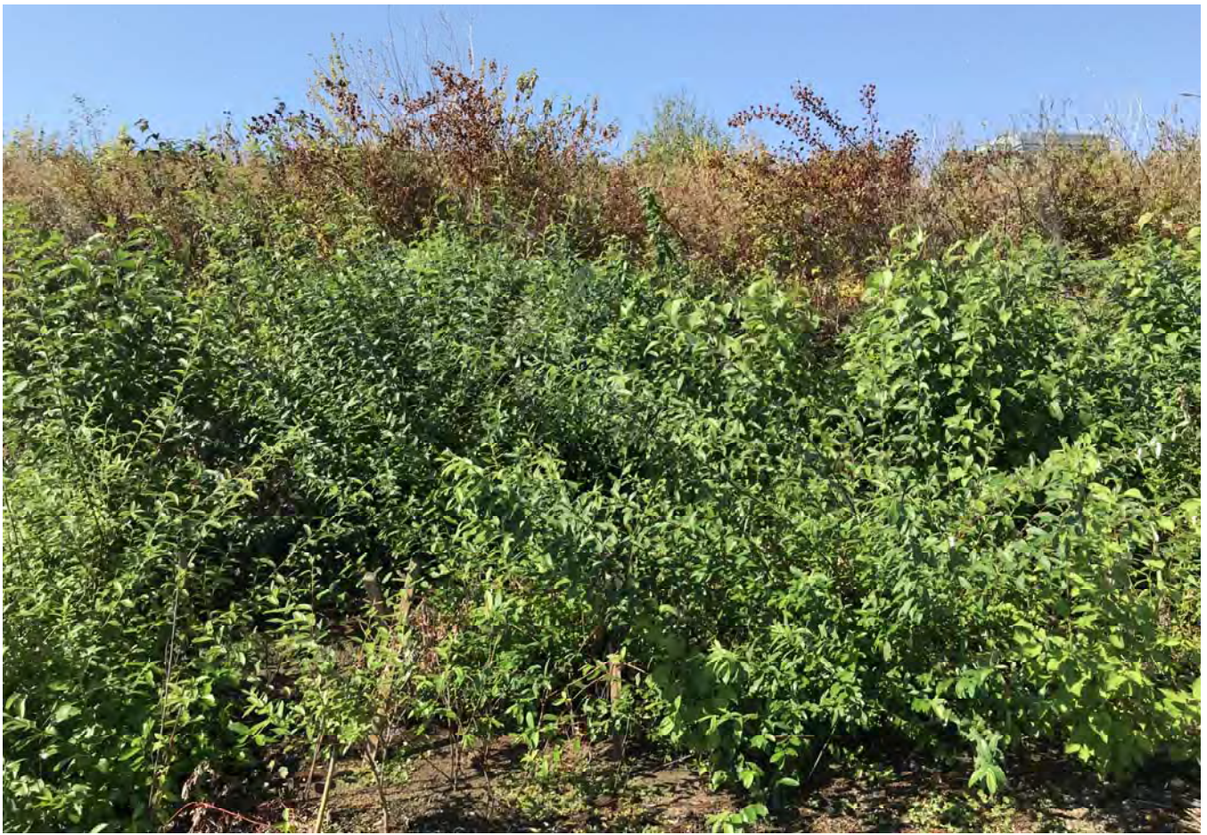
STA: 15+00 - Toe of slope looking west.
