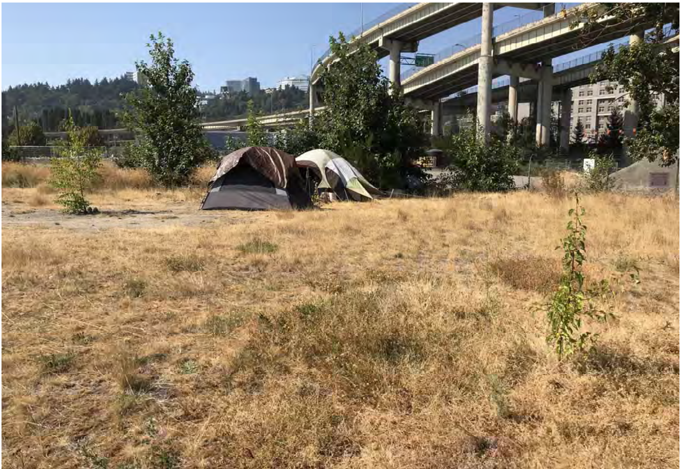
STA: 26+50 - Top of bank looking west.
