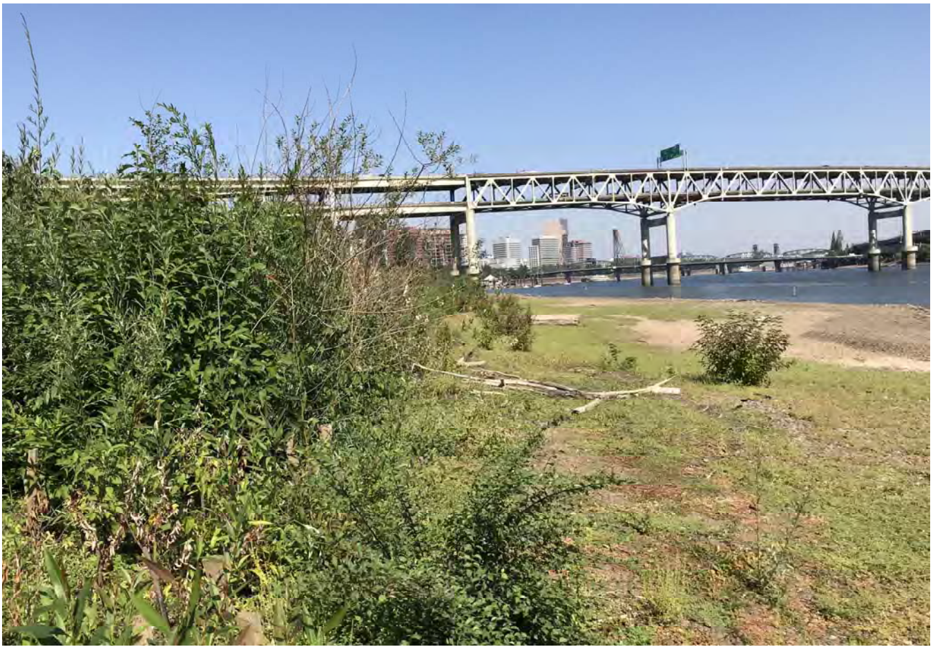
STA: 19+50 - Toe of slope looking downstream.
