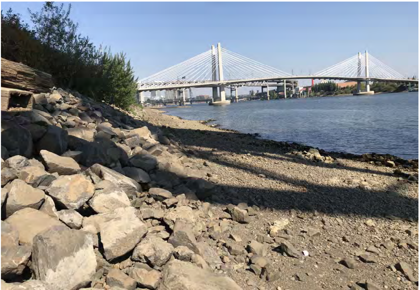
STA: 7+00 - Bottom of rock armor looking downstream.
