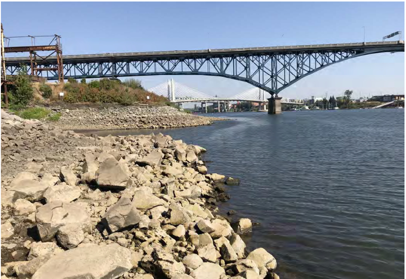
STA: 0+00 - Edge of water looking downstream.
