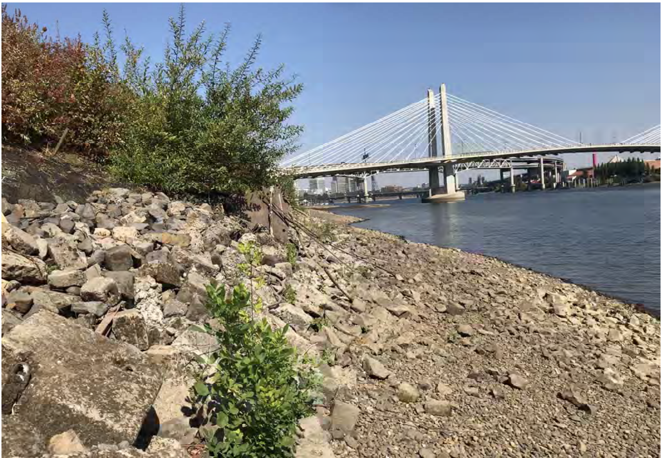
STA: 9+00 - Bottom of rock armor looking downstream.
