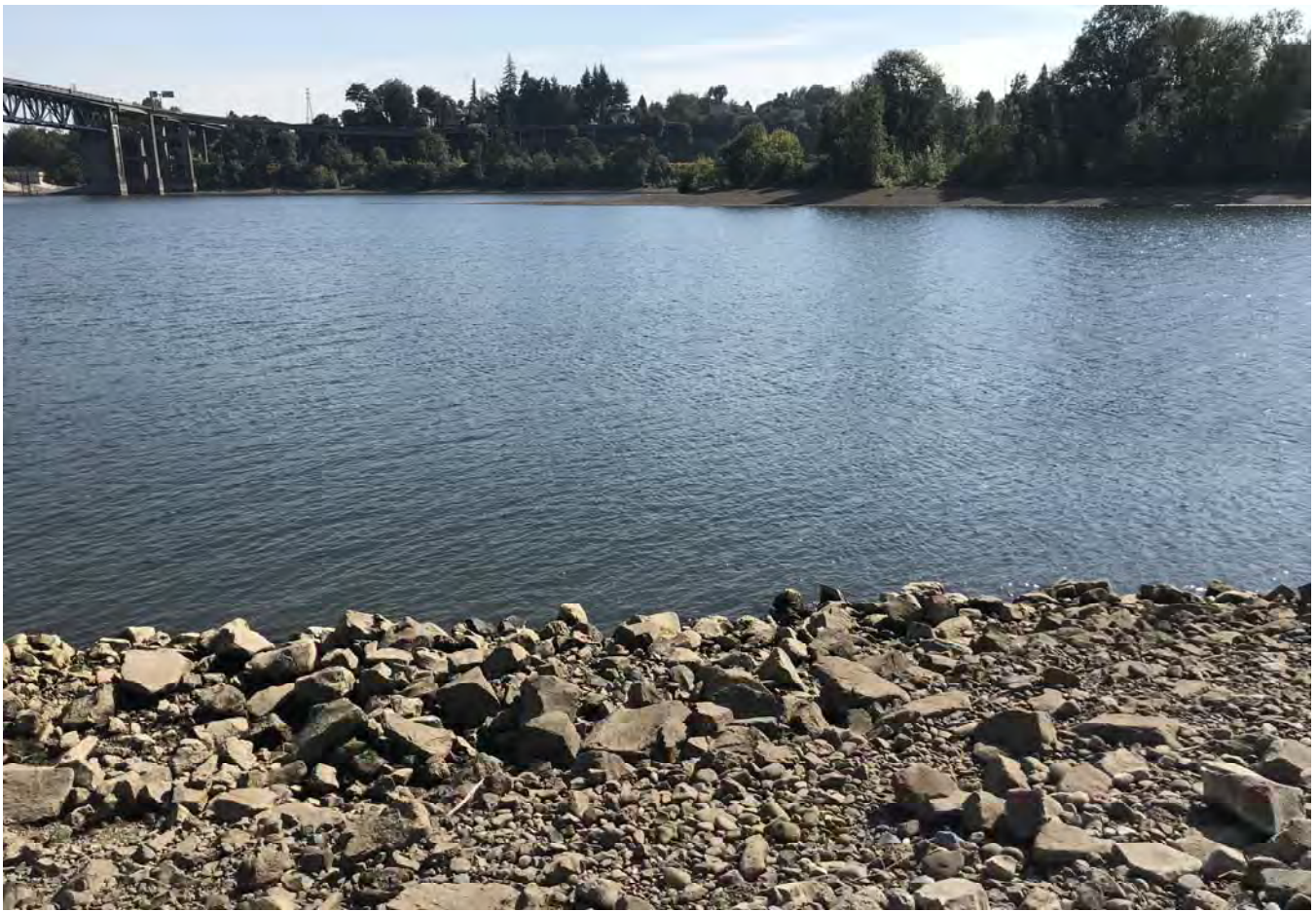
STA: 0+00 - Top of rock armor looking east.
