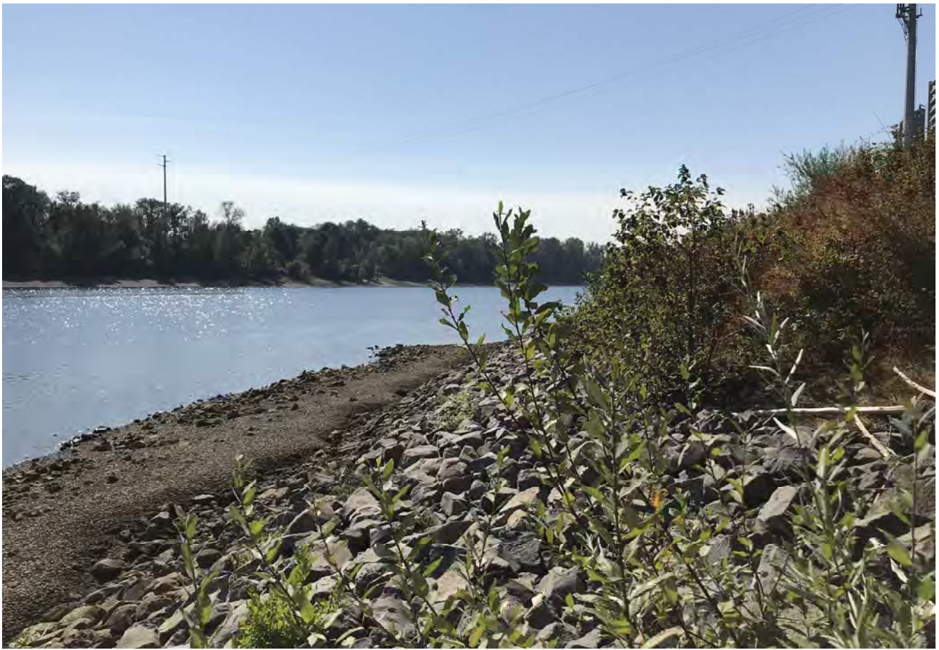
STA: 5+00 - Top of rock armor looking upstream.
