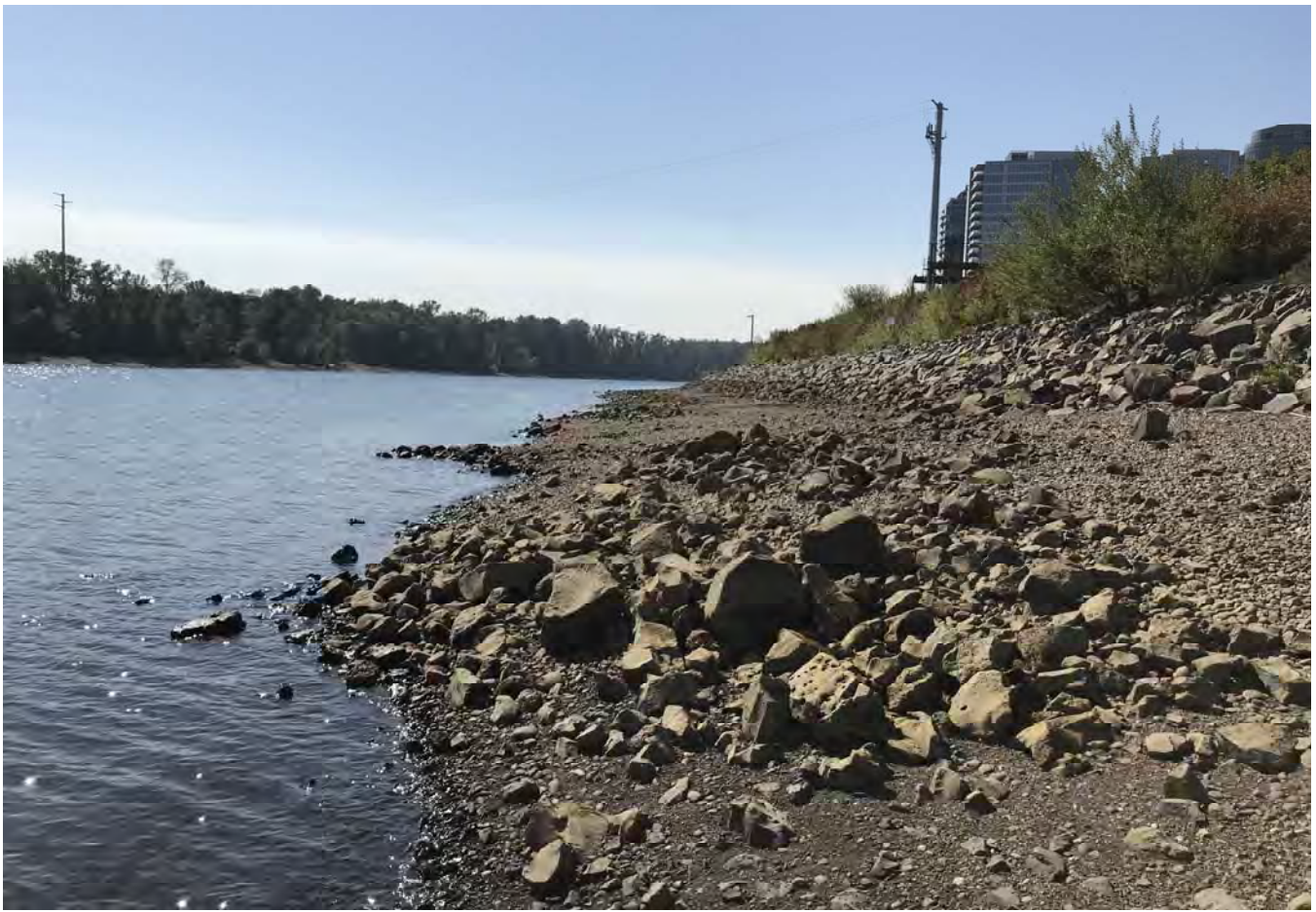
STA: 7+00 - Edge of water looking upstream.
