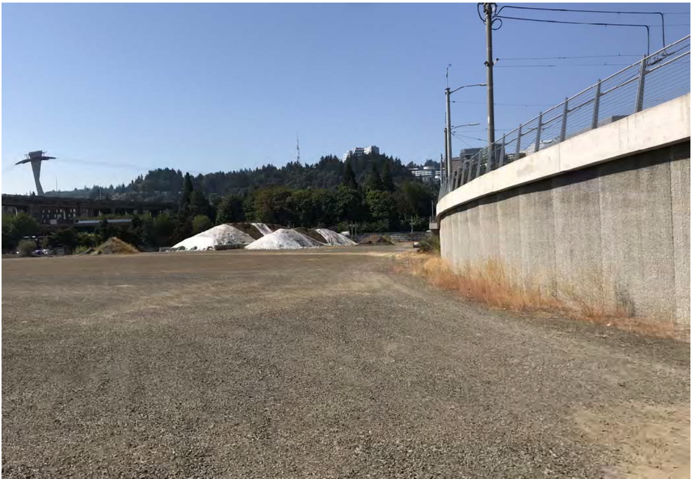
Northeast corner of upland cap, looking west.
