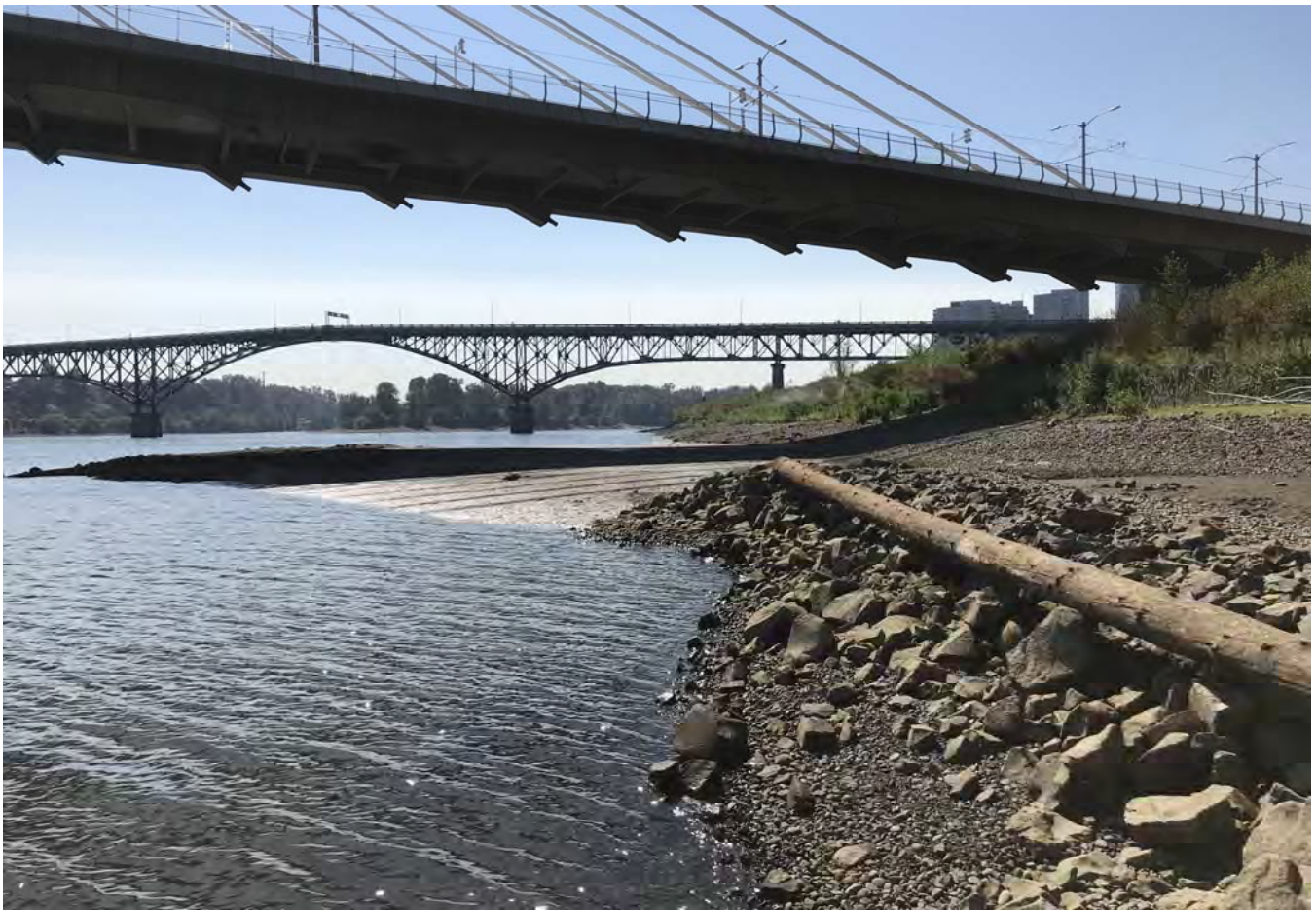
STA: 19+50 - Edge of water looking upstream.
