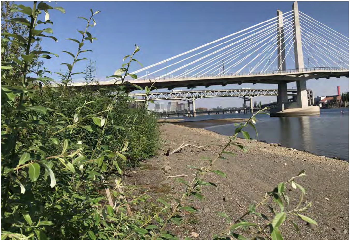
STA: 13+00 - Toe of slope looking downstream.
