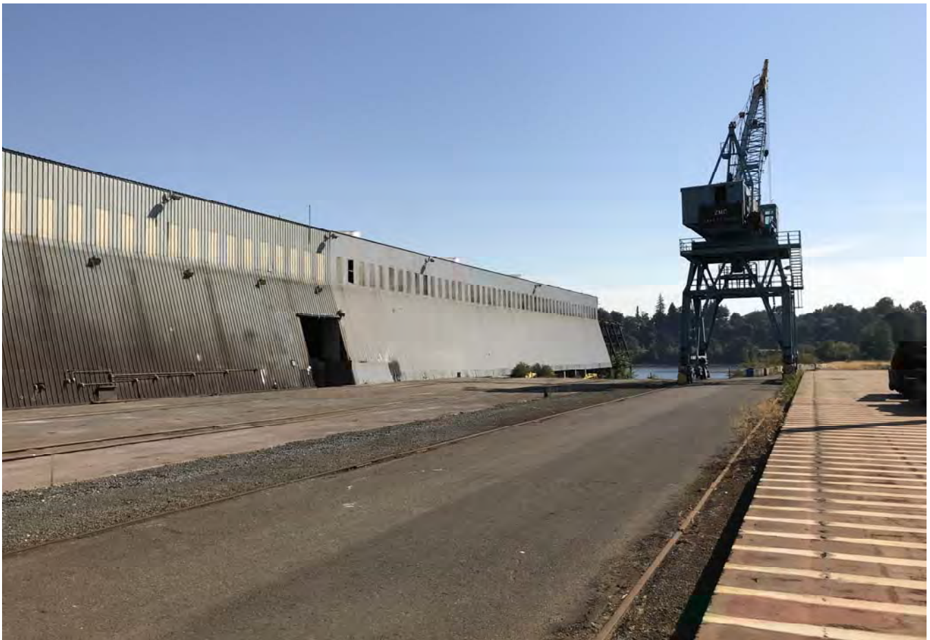
Barge building looking northeast.
