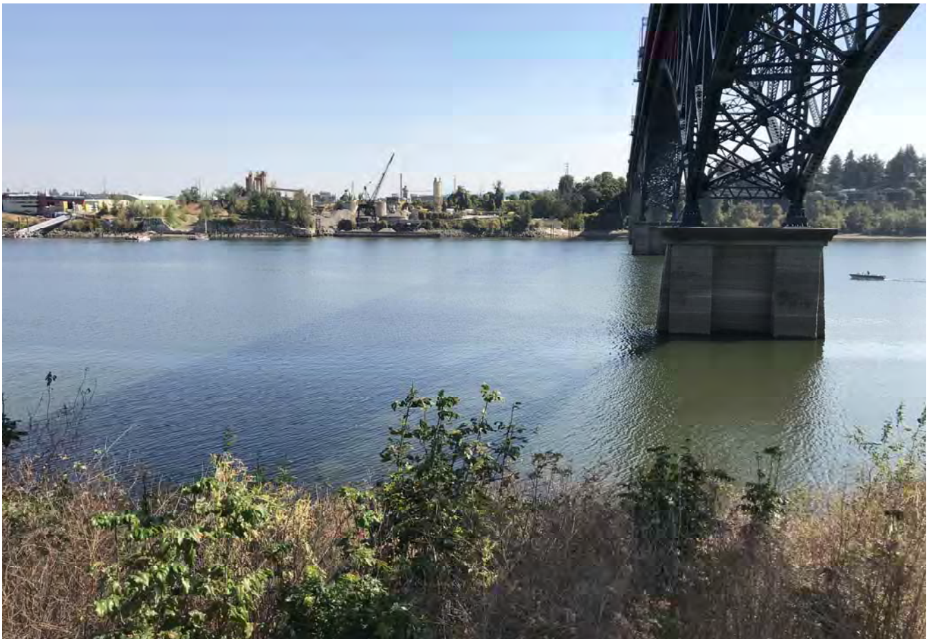
STA: 7+00 - Top of bank looking east.
