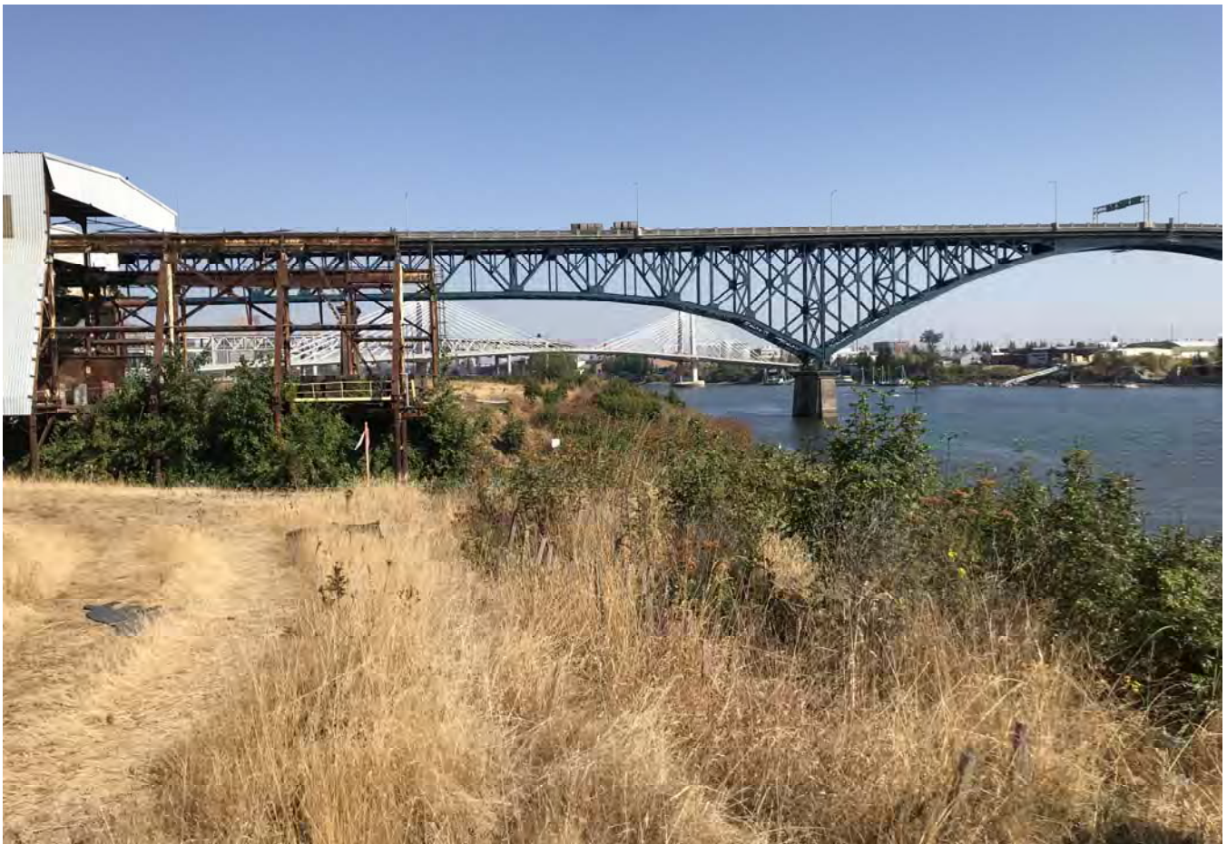
STA: 0+00 - Top of bank looking downstream.
