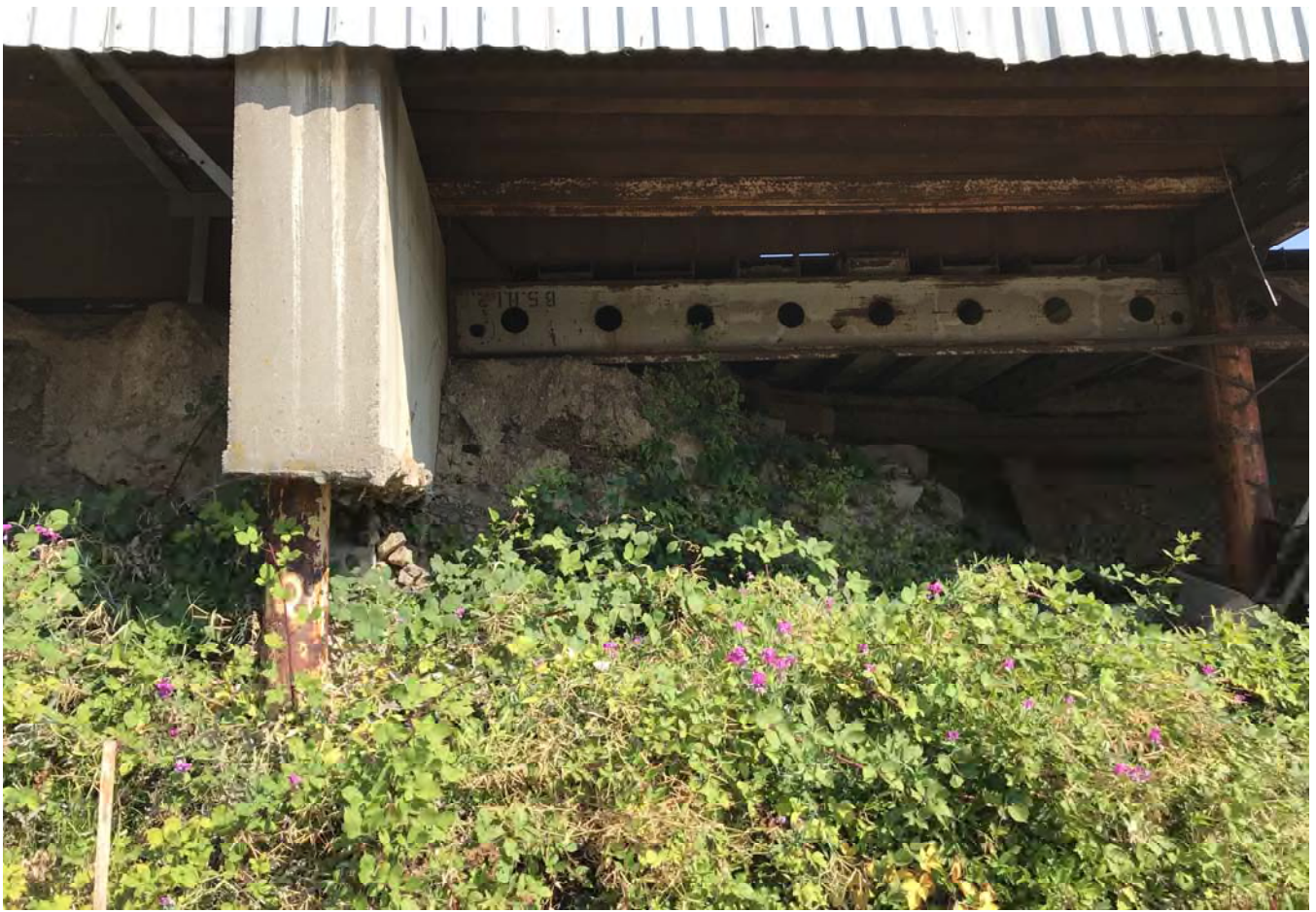
Underside of barge building structure looking north from slipway.
