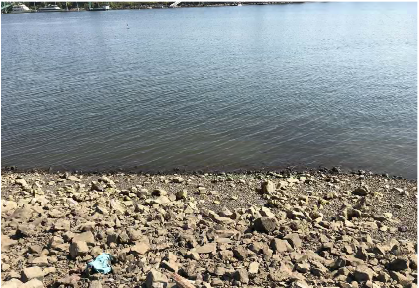
STA: 11+00 - Top of rock armor looking east.
