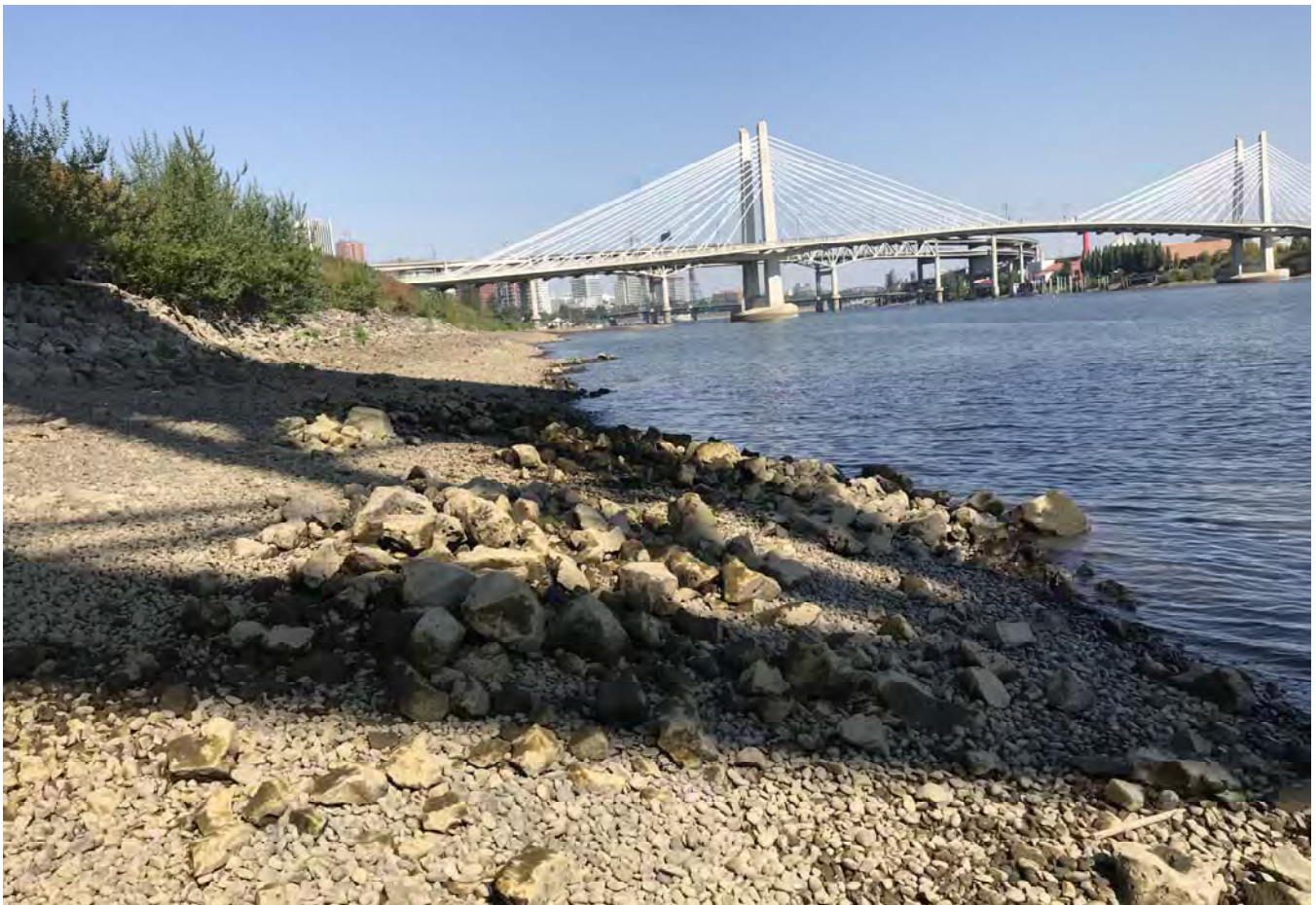
STA: 7+00 - Edge of water looking downstream.
