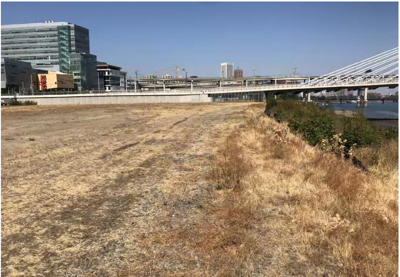
STA: 11+00 - Top of bank looking downstream.
