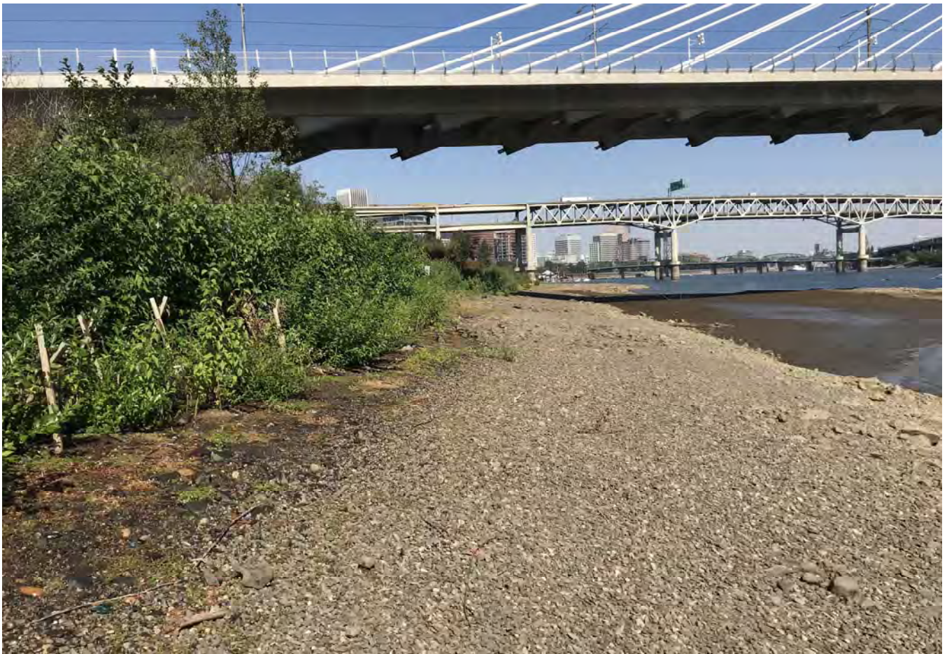
STA: 15+00 - Toe of slope looking downstream.
