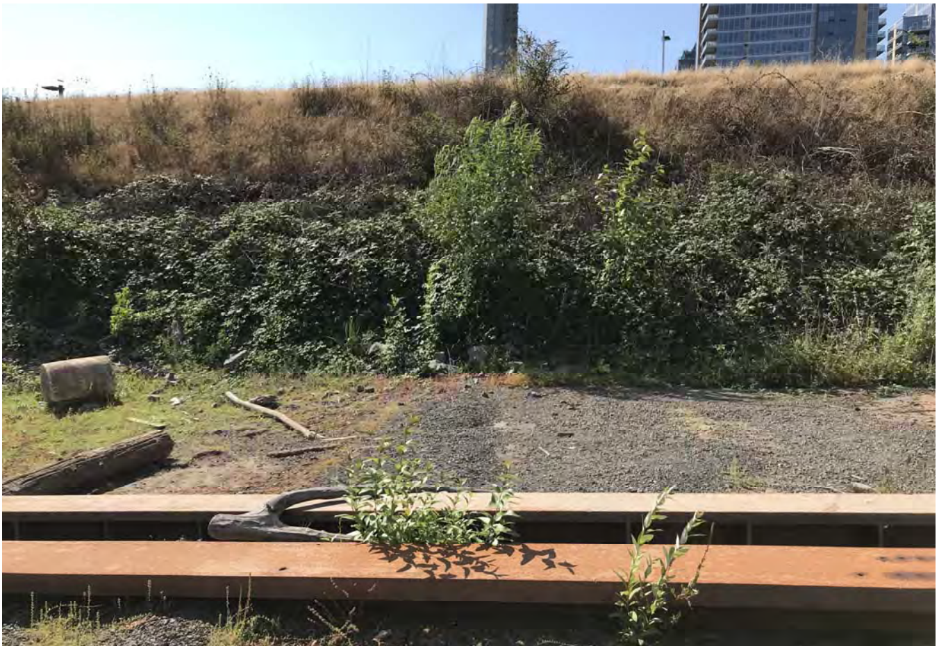
Slipway ramp looking south.
