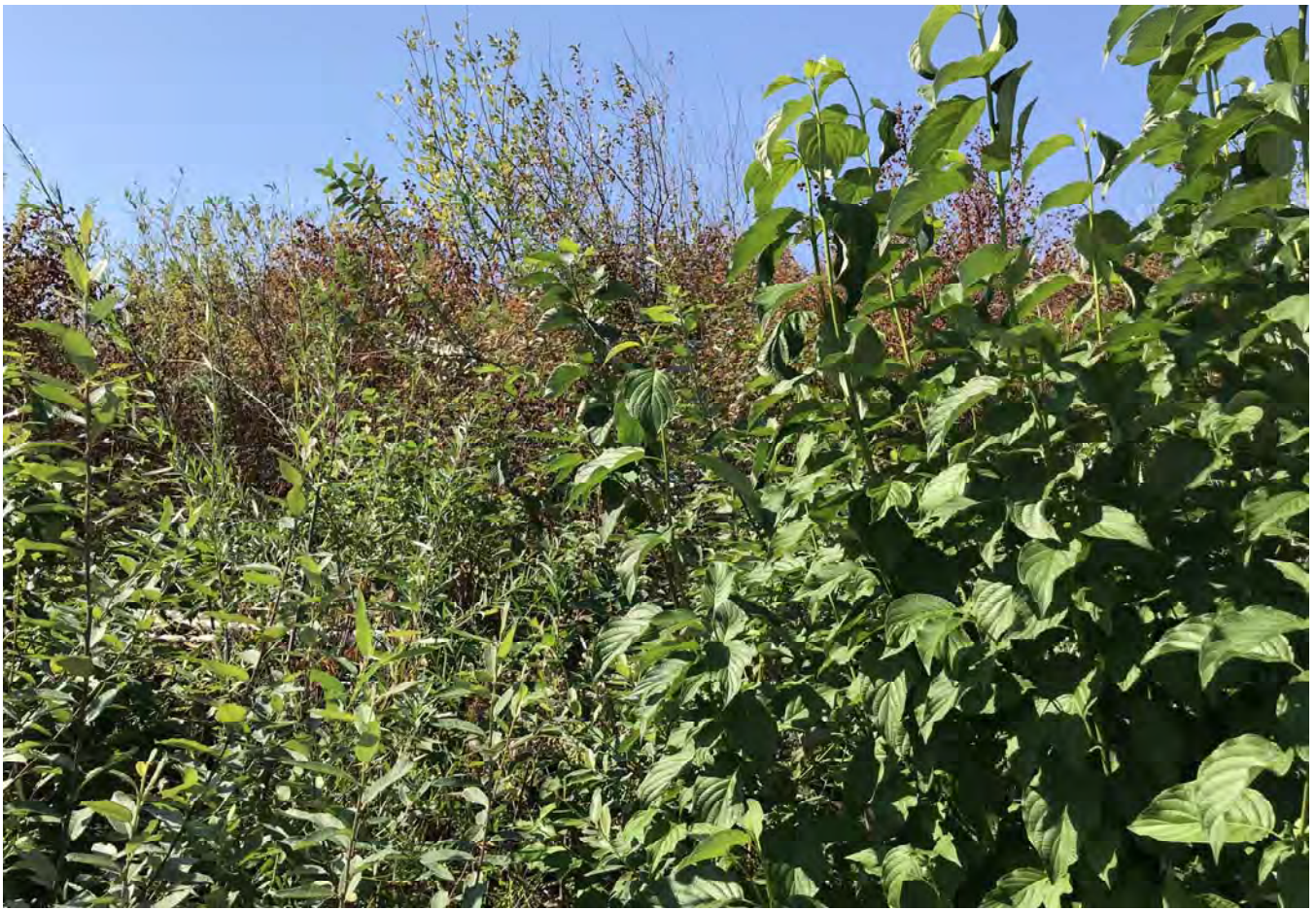
STA: 19+50 - Toe of slope looking west.
