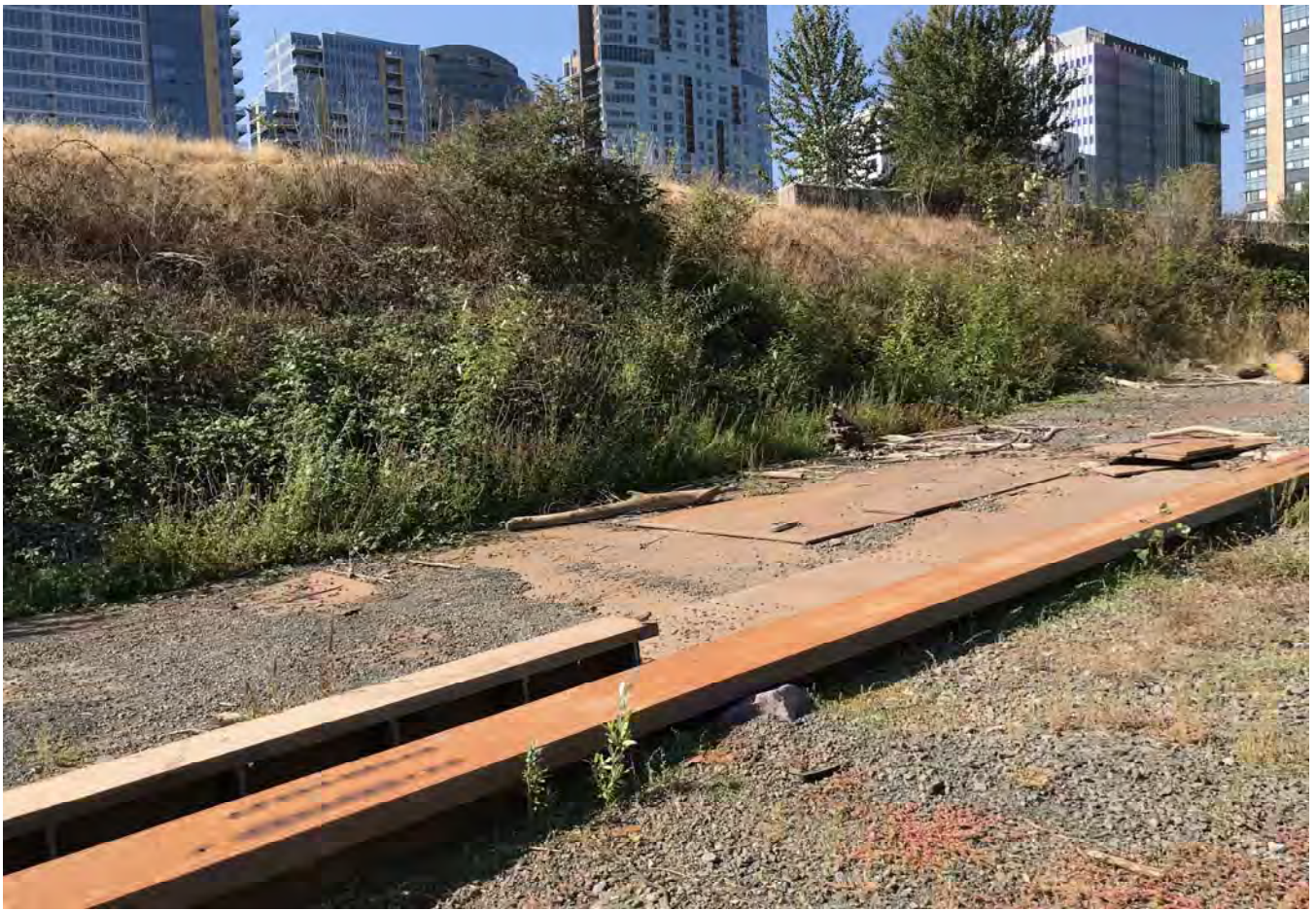
Slipway ramp looking southwest.
