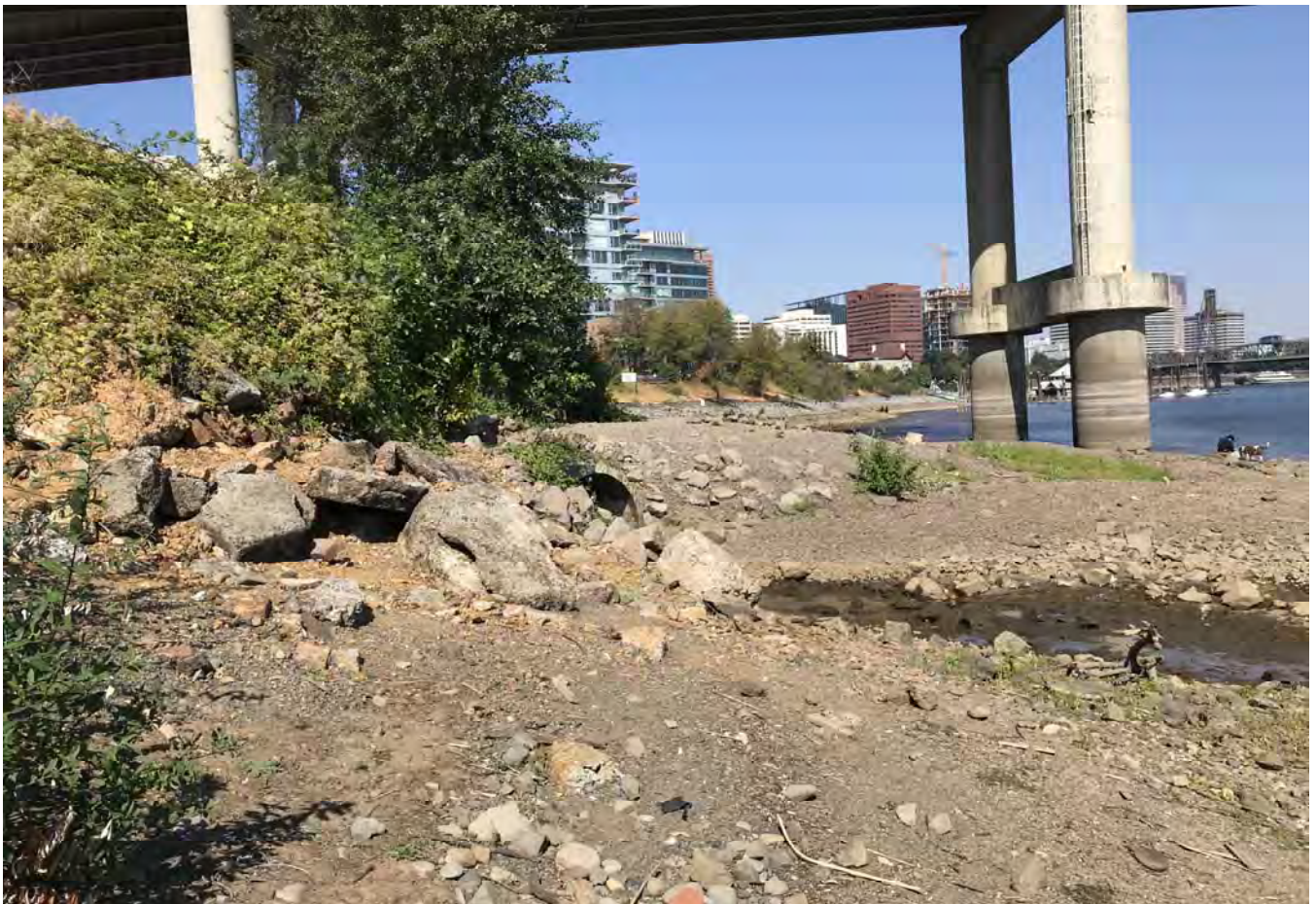
City stormwater outfall 07B.
