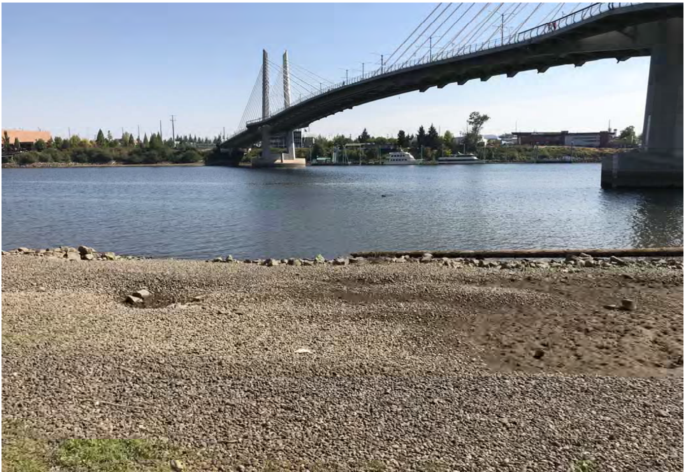
STA: 19+50 - Toe of slope looking east.
