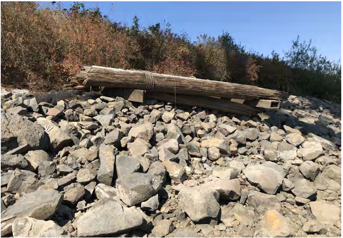
STA: 7+00 - River pilings beached on rock armor.
