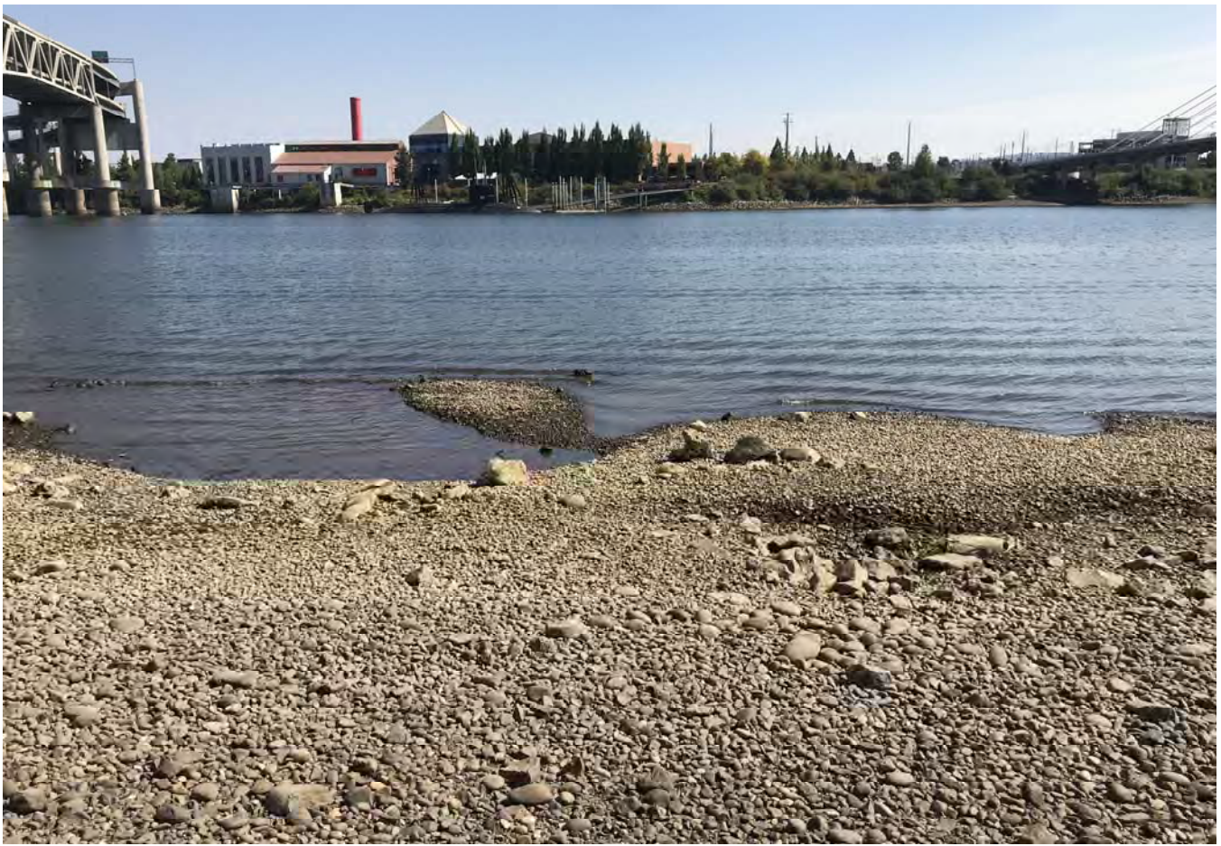
STA: 26+50 - Toe of slope looking east.
