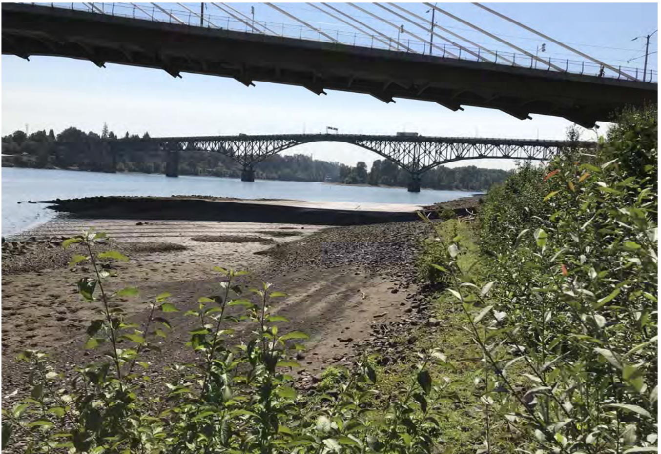
STA: 19+50 - Toe of slope looking upstream.
