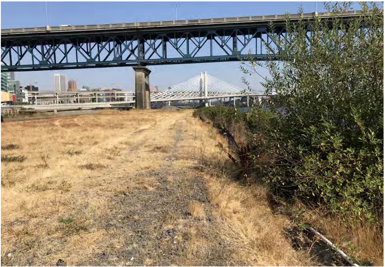
STA: 3+00 - Top of bank looking downstream.
