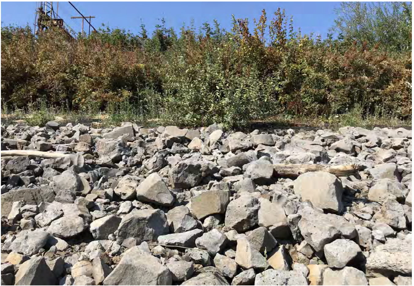
STA: 3+00 - Bottom of rock armor looking west.
