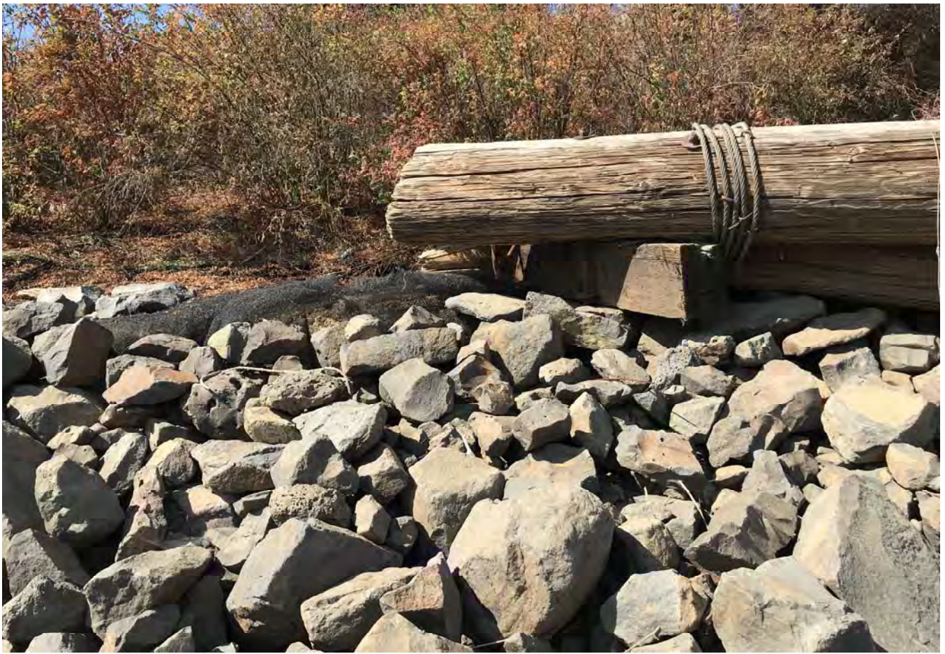
STA: 7+00 - Bottom of rock armor looking west.
