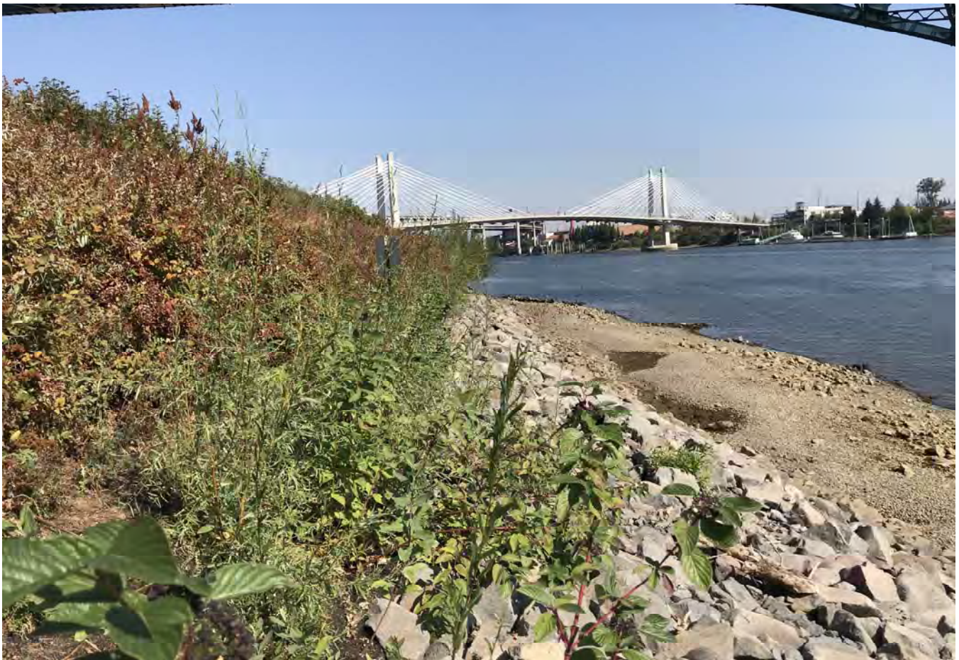
STA: 5+00 - Top of rock armor looking downstream.
