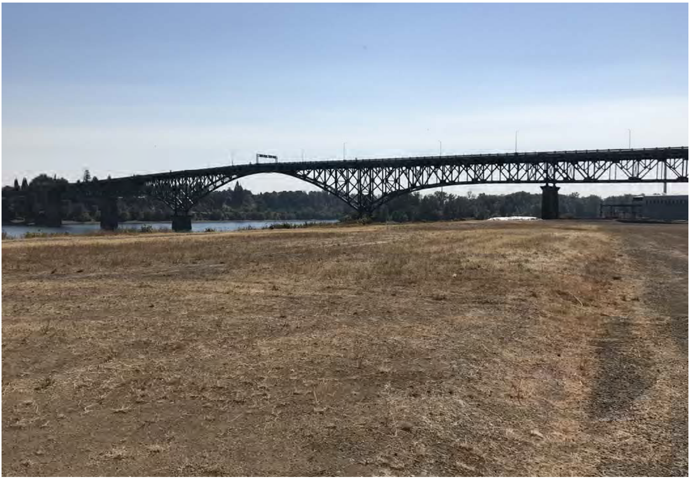
Northeast corner of upland cap looking south.
