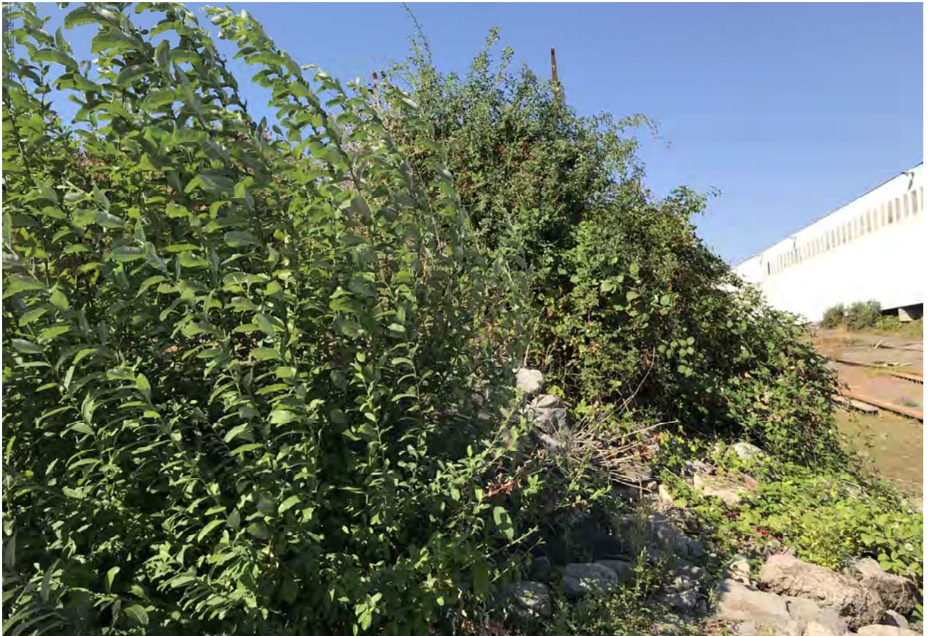
STA: 0+25 - Top of rock armor looking west.
