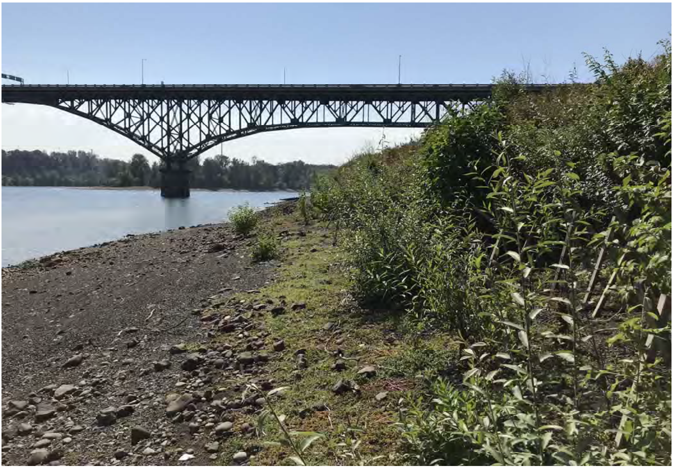
STA: 13+00 - Toe of slope looking upstream.
