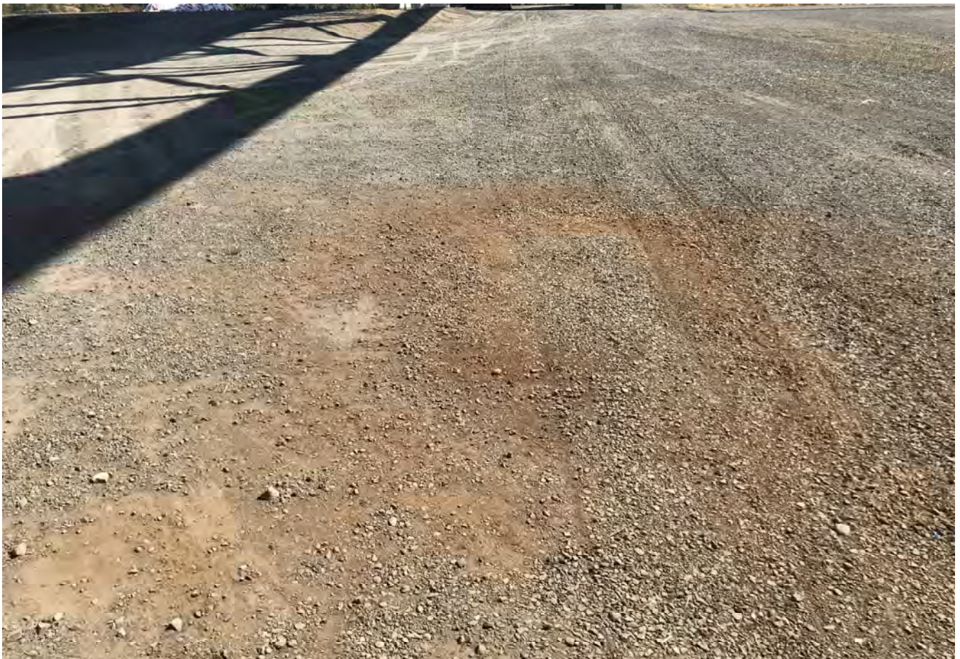
Gravel cap beneath Ross Island Bridge.
