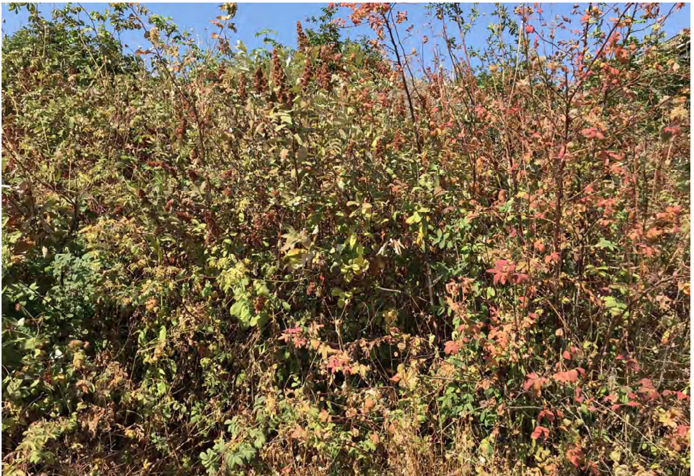
STA: 5+00 - Top of rock armor looking west.
