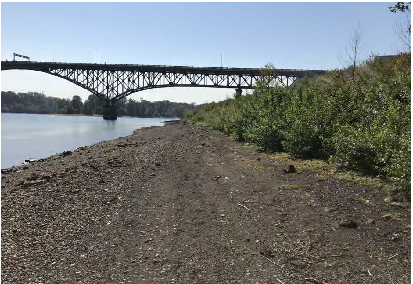
STA: 15+00 - Toe of slope looking upstream.
