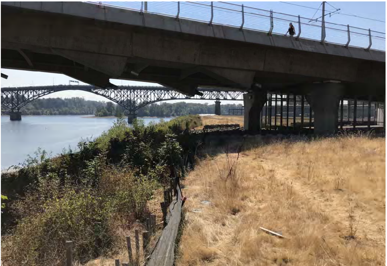
STA: 17+00 - Top of bank looking upstream.
