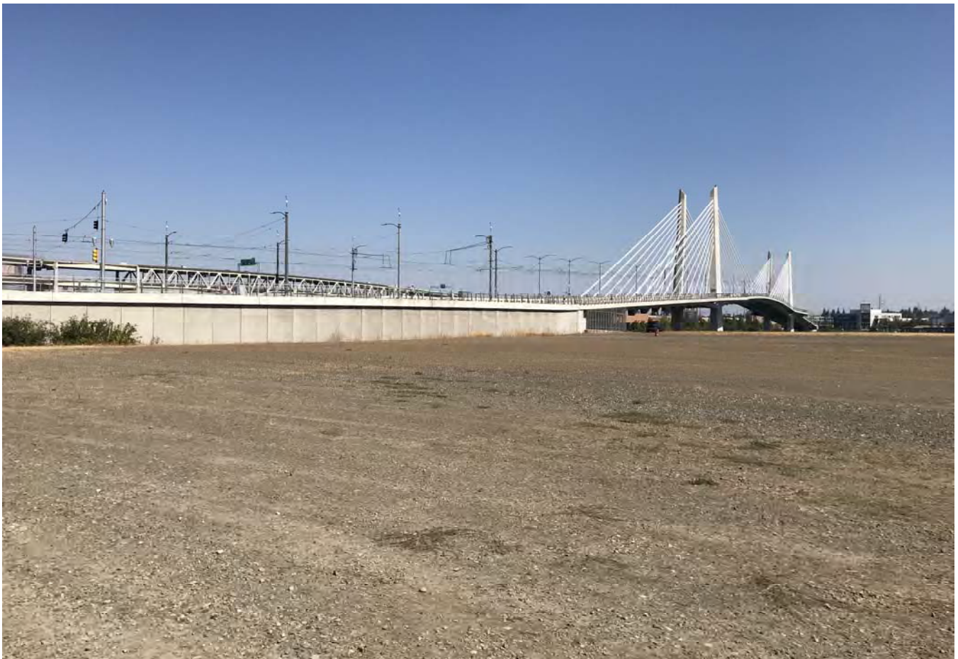
Upland cap center of site looking northeast.
