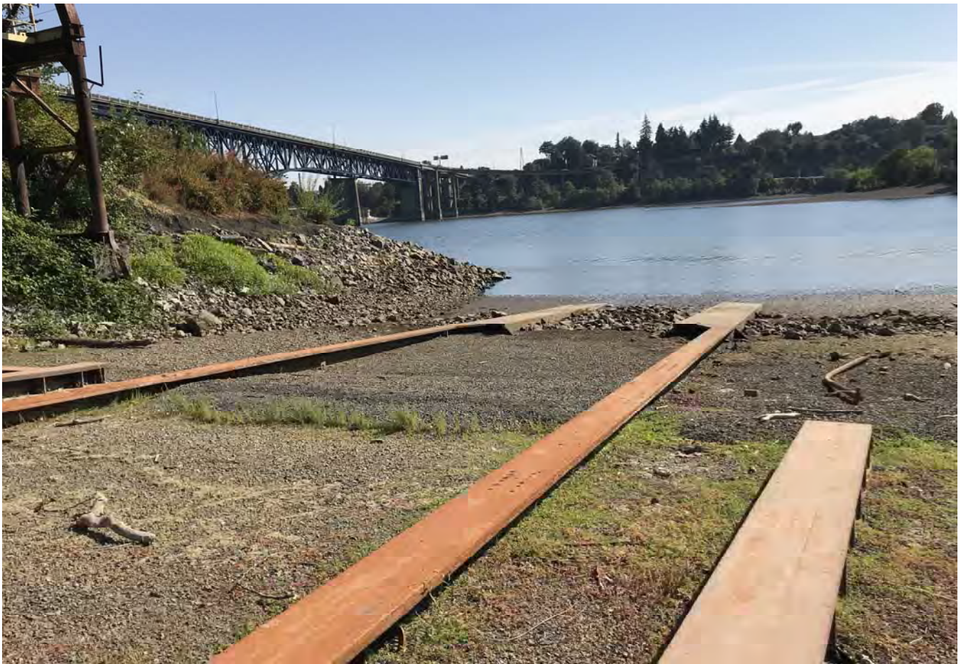
Slipway ramp rails looking east.
