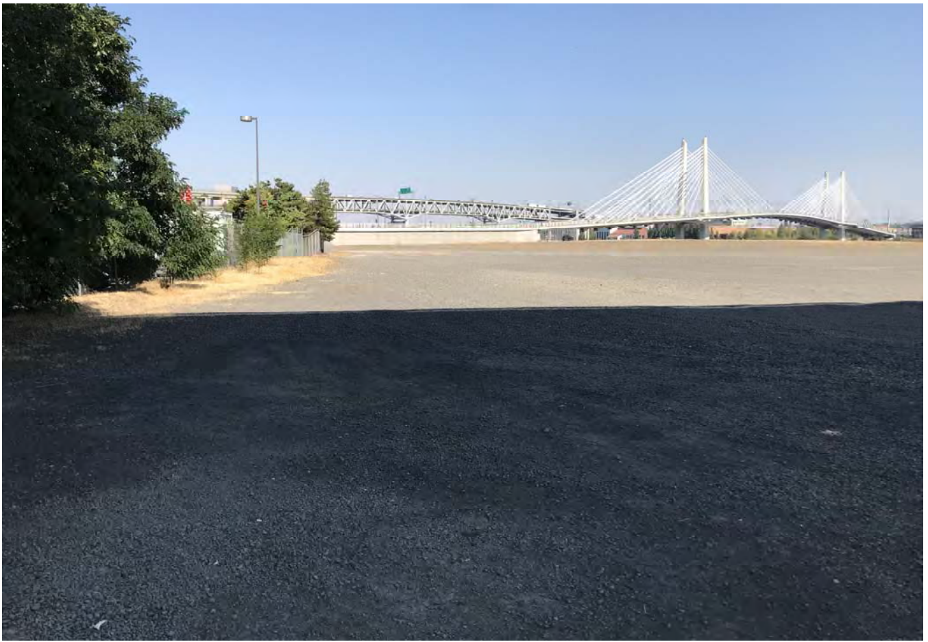
Upland cap southwest corner of site looking north.
