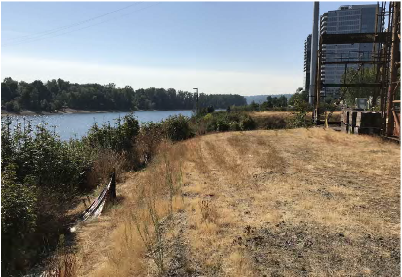
STA: 3+00 - Top of bank looking upstream.
