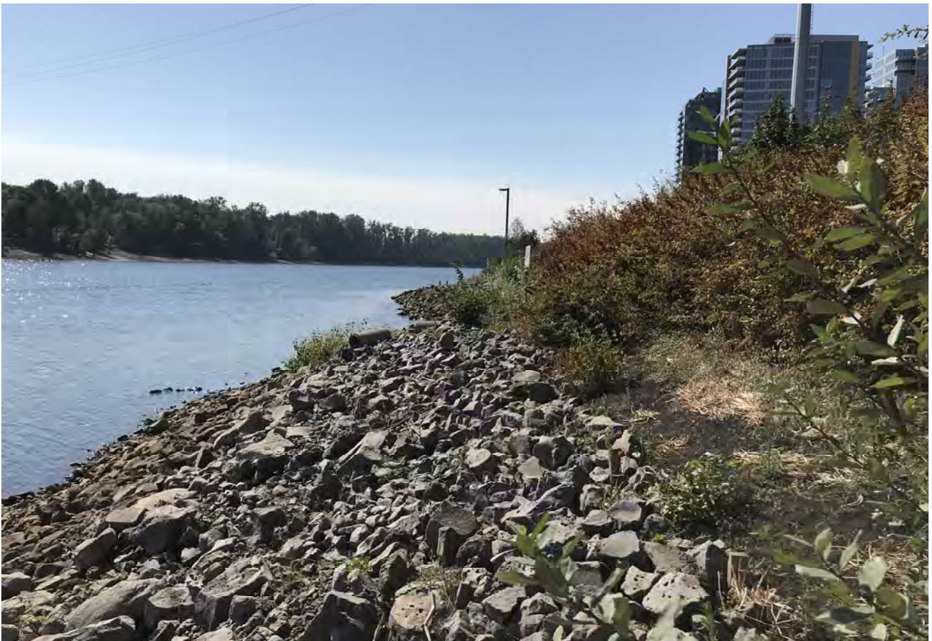
STA: 3+00 - Top of rock armor looking upstream.
