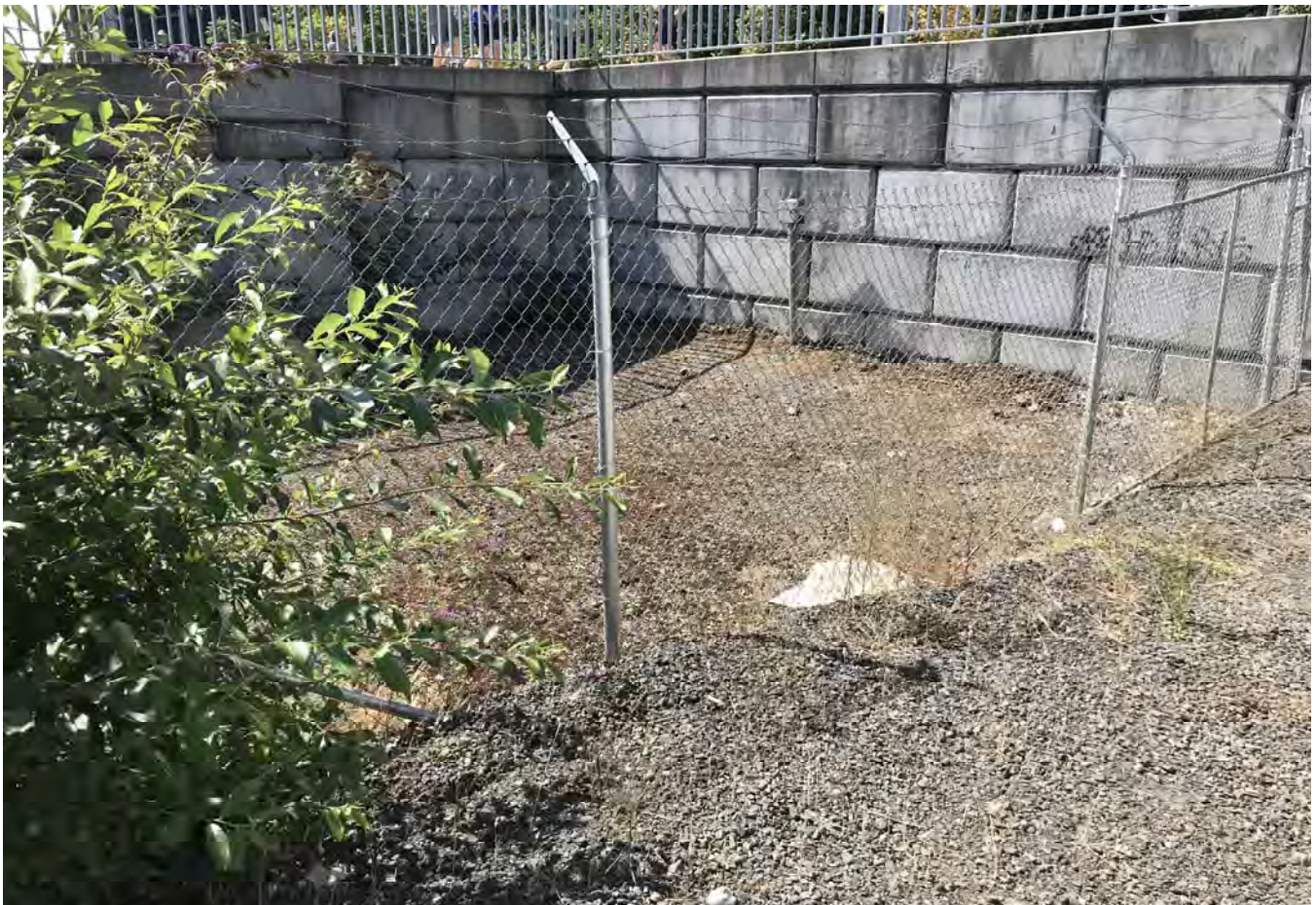
Upland cap near site entrance from Southwest Moody looking southwest.
