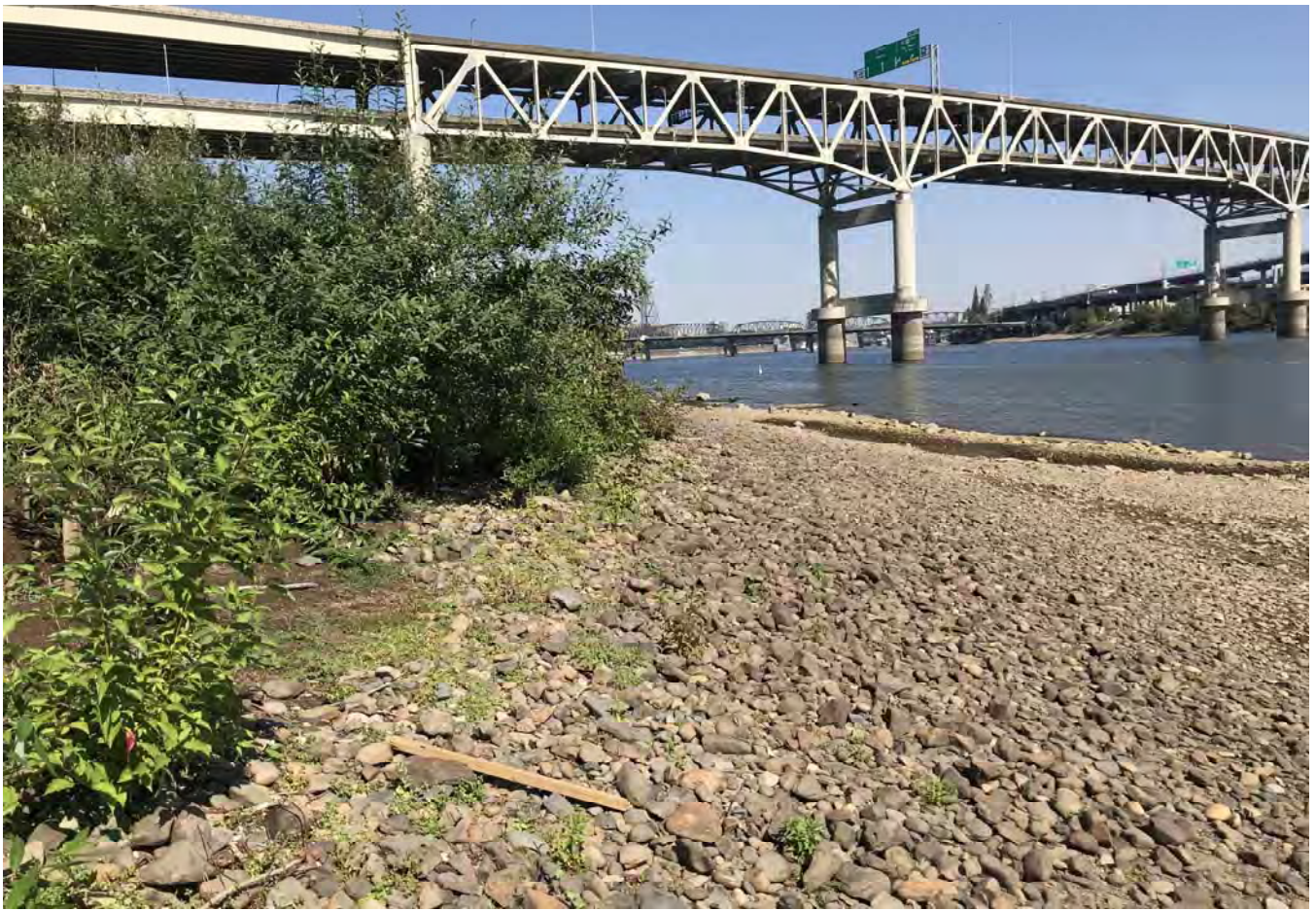
STA: 25+50 - Toe of slope looking downstream.
