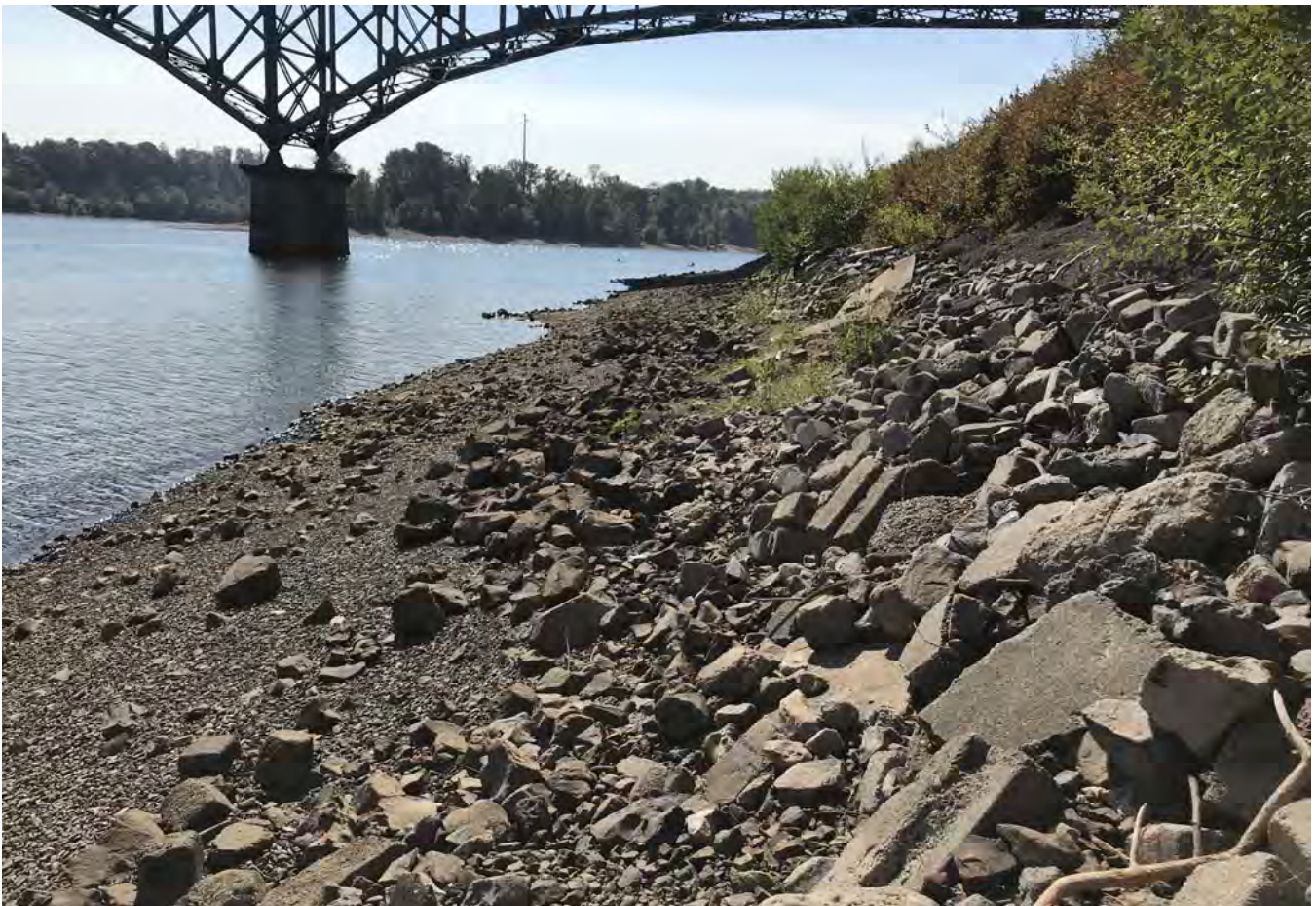
STA: 11+00 - Bottom of rock armor looking upstream.
