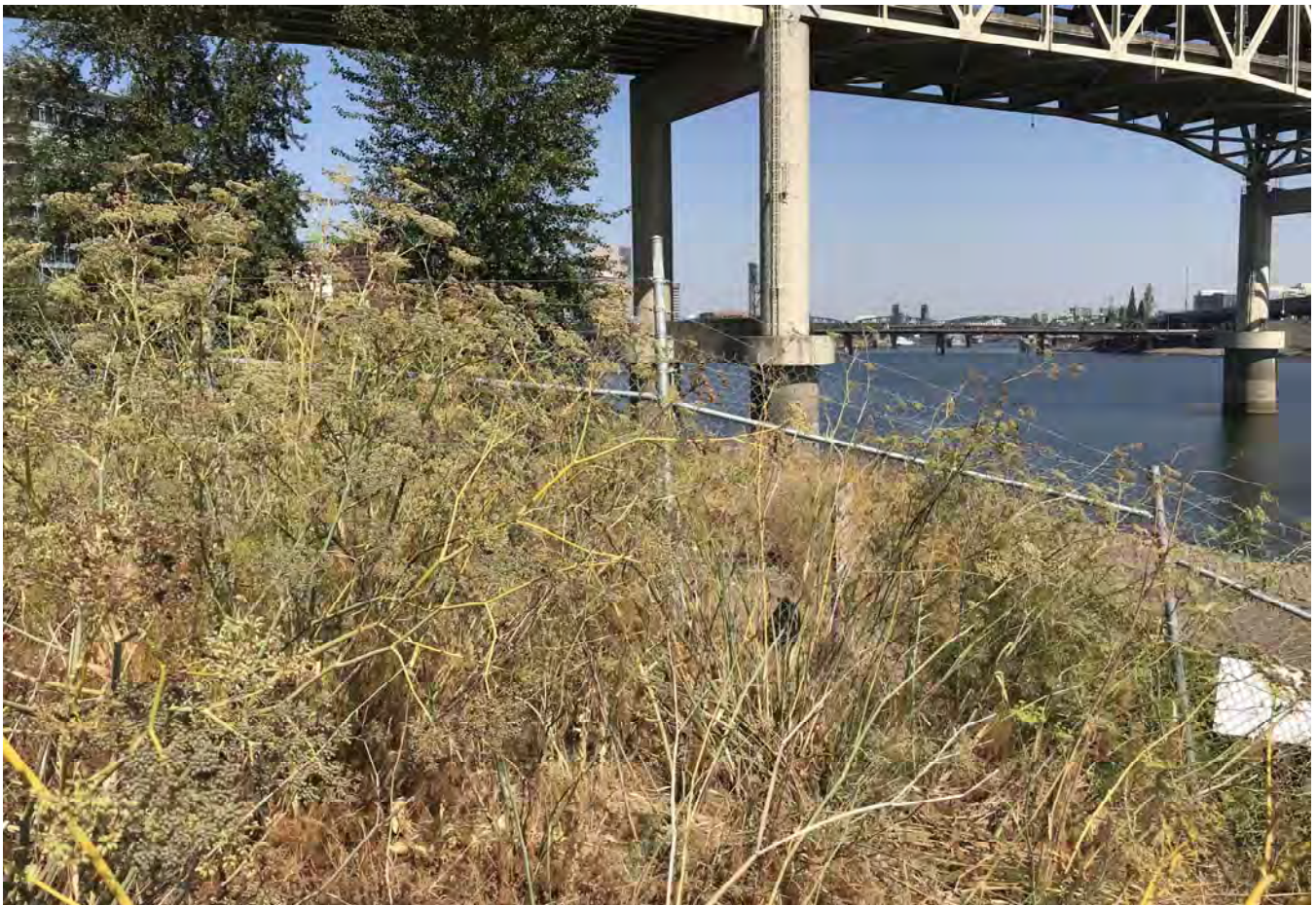
STA: 26+50 - Top of bank looking downstream.
