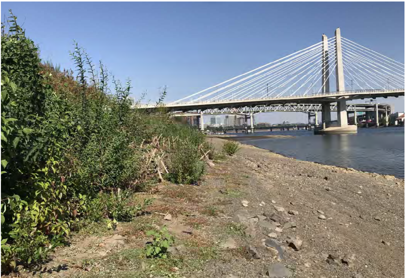
STA: 11+50 - Toe of slope looking downstream.
