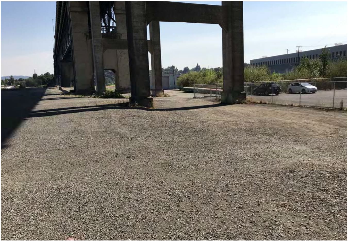
Upland cap under Ross Island Bridge looking east.
