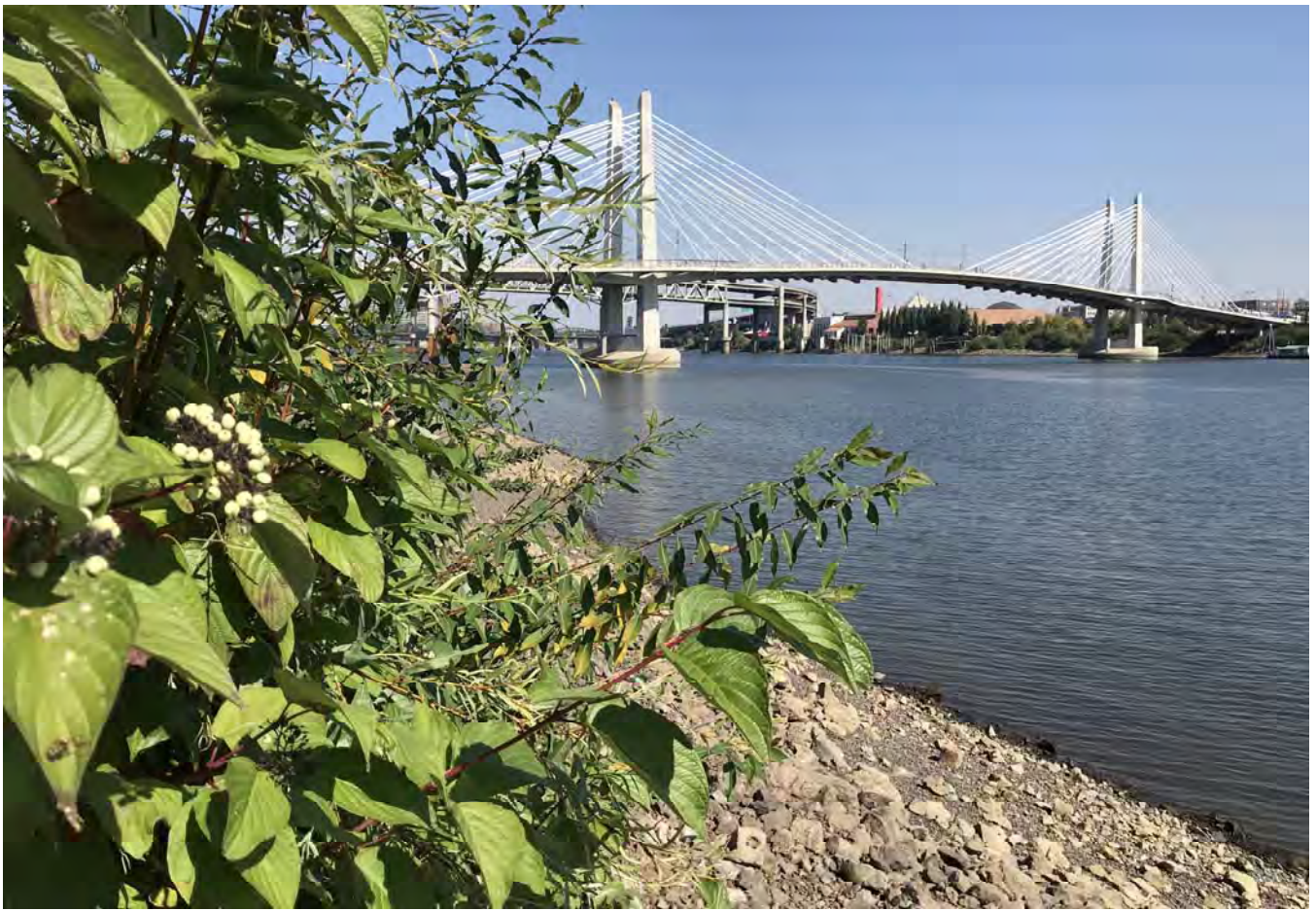
STA: 11+00 - Top of rock armor looking downstream.
