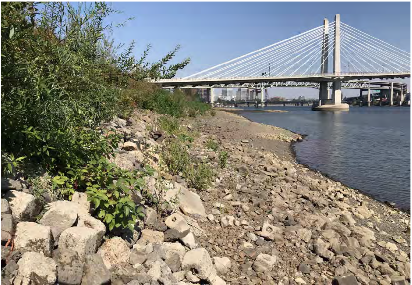
STA: 11+00 - Bottom of rock armor looking downstream.
