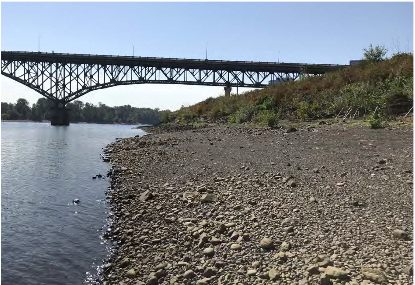
STA: 13+00 - Edge of water looking upstream.
