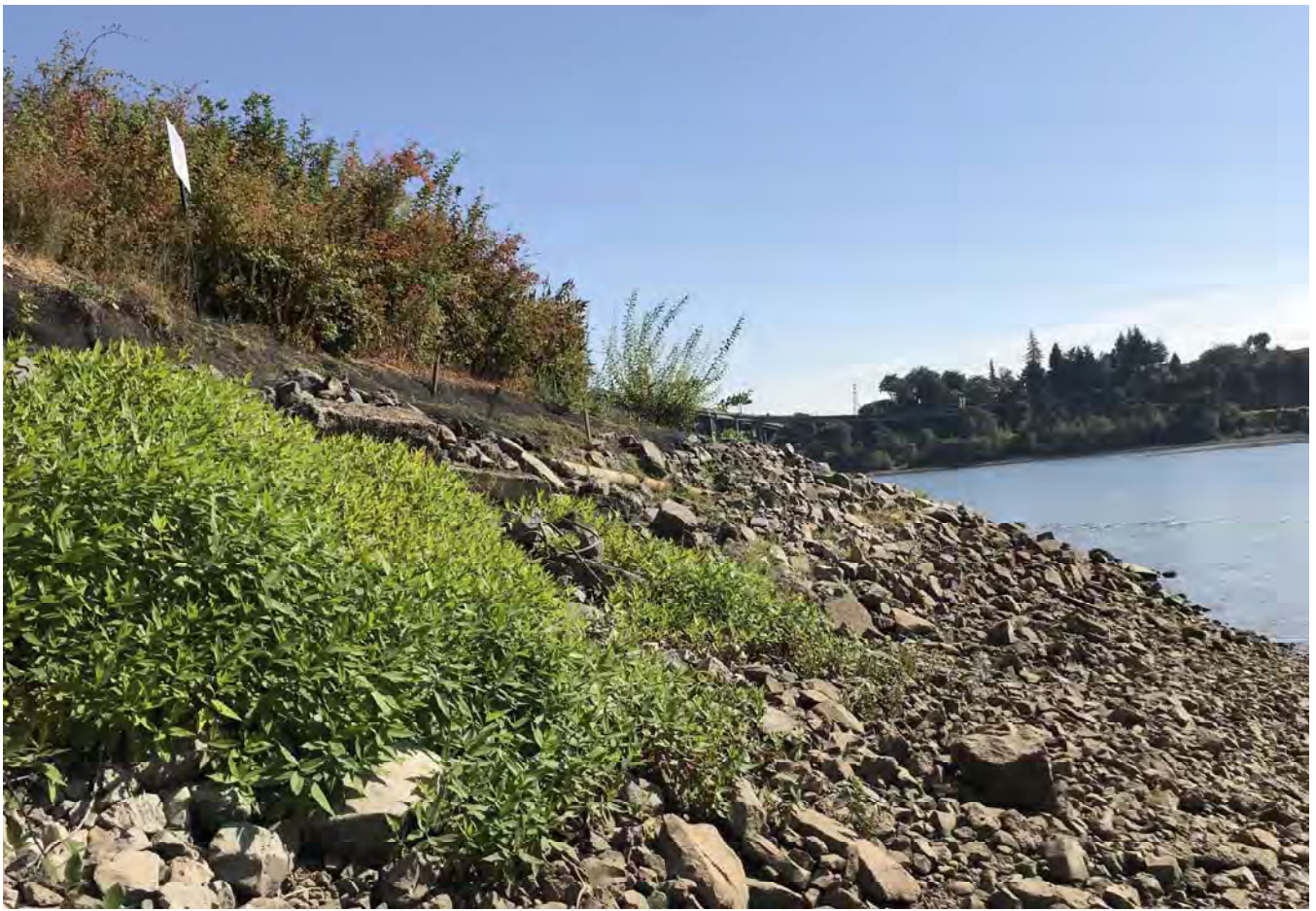
North slope of slipway ramp looking east.
