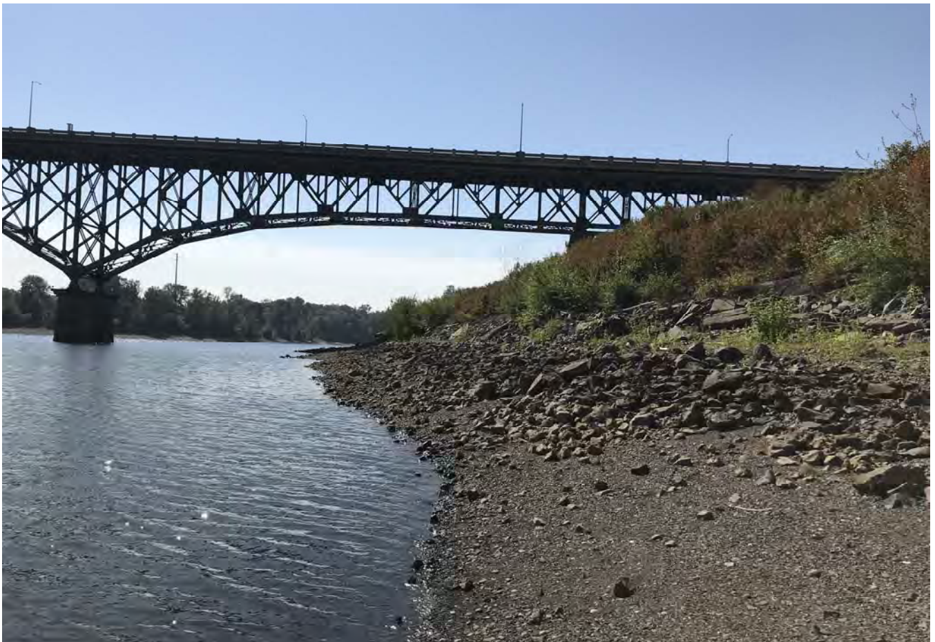
STA: 11+50 - Edge of water looking upstream.
