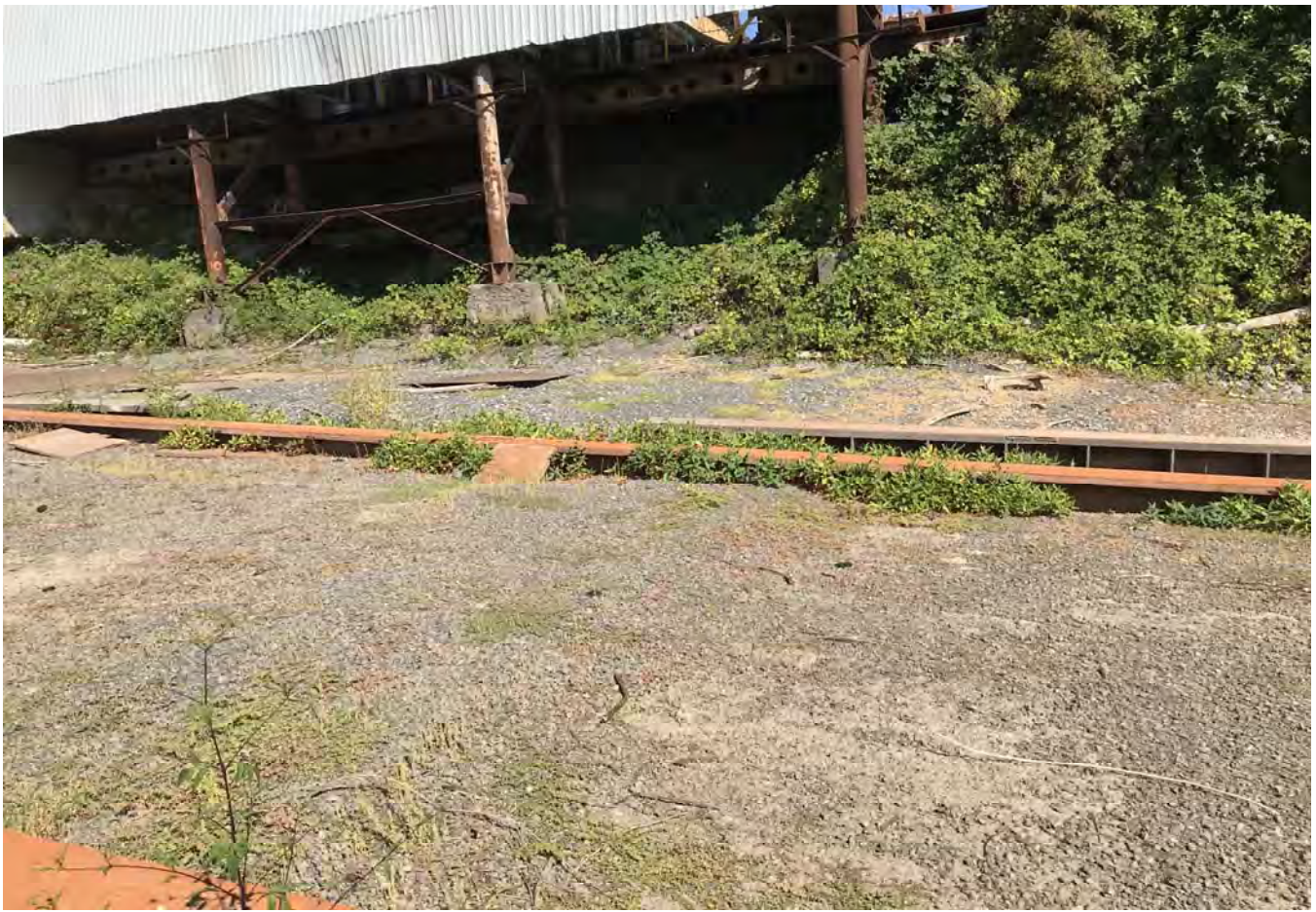
Barge building and slipway ramp looking north.
