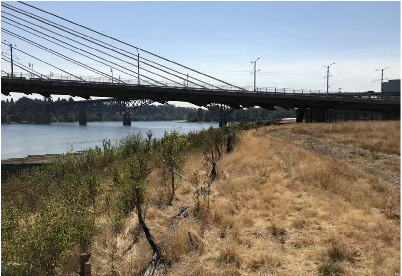
STA: 19+50 - Top of bank looking upstream.
