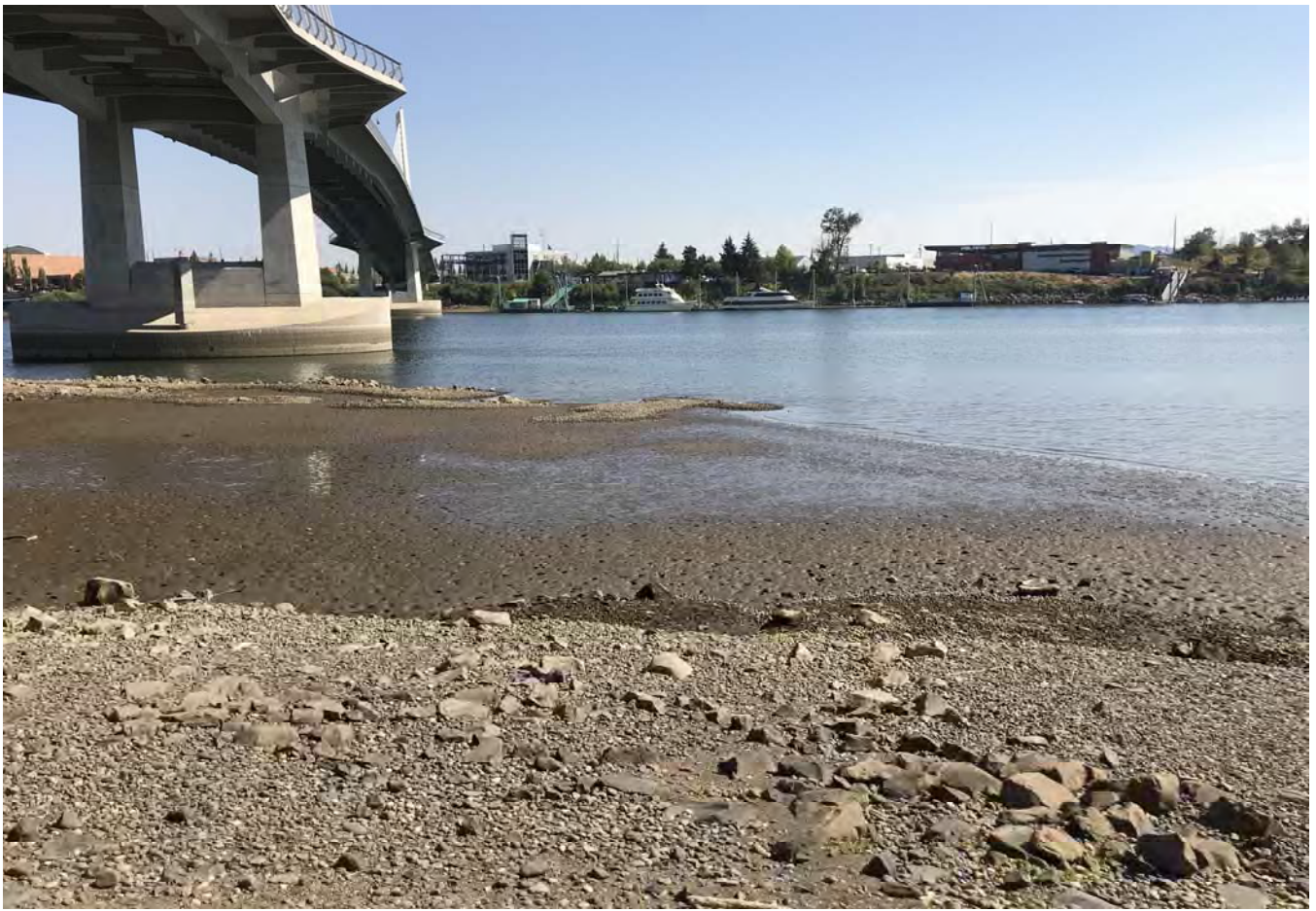
STA: 15+50 - Looking east over shoal area.
