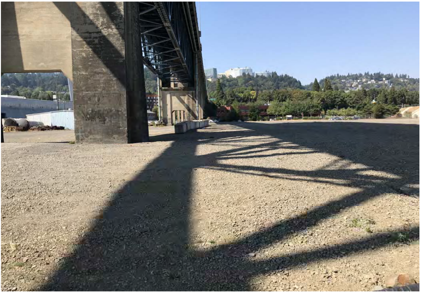
STA: 7+00 - Top of bank looking west.
