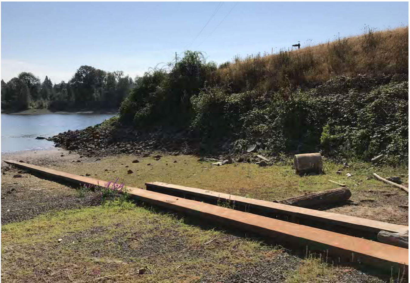
Slipway ramp looking southeast.
