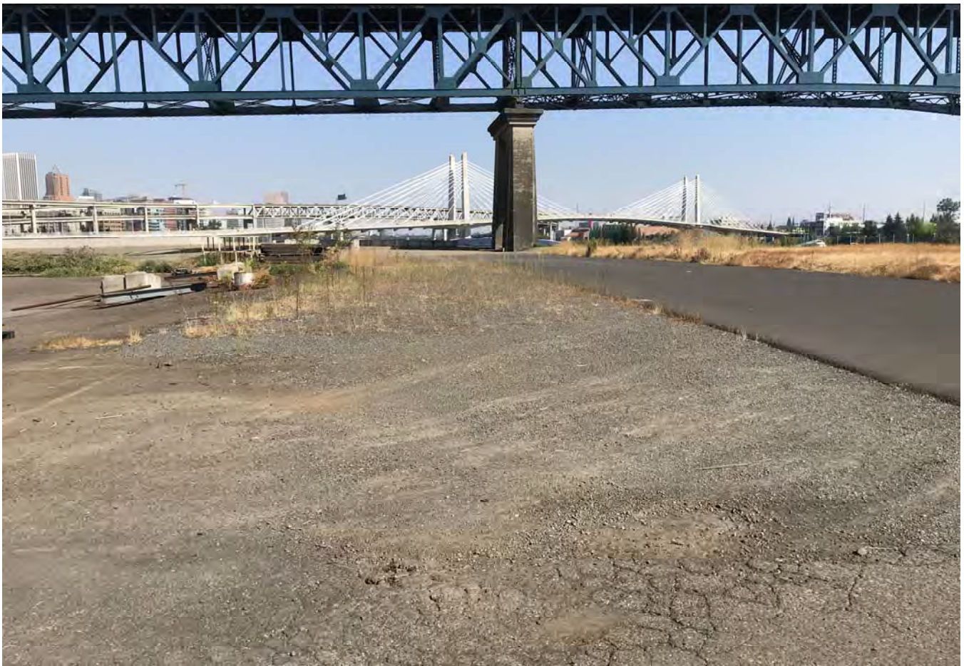
Operational area north of barge building looking north.
