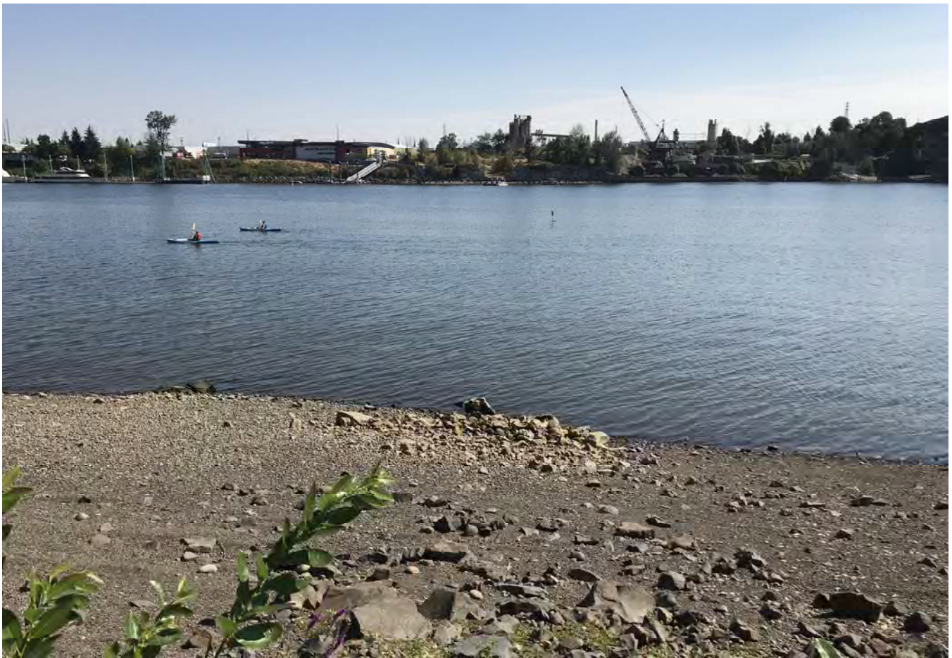
STA: 11+50 - Toe of slope looking east.
