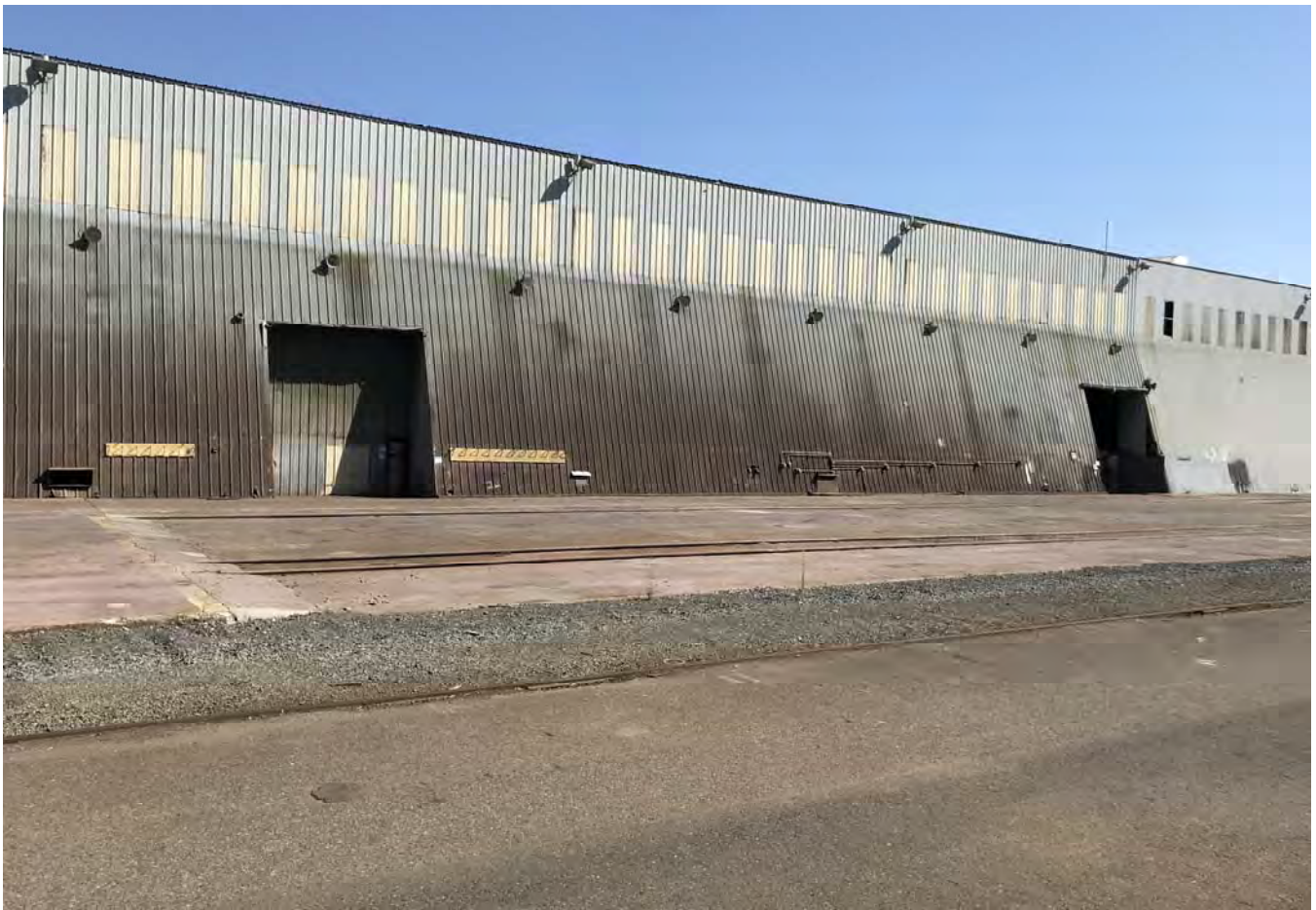
Barge building looking north.
