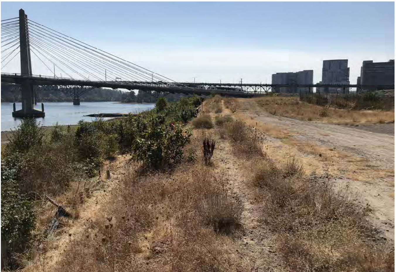
STA: 25+50 - Top of bank looking upstream.
