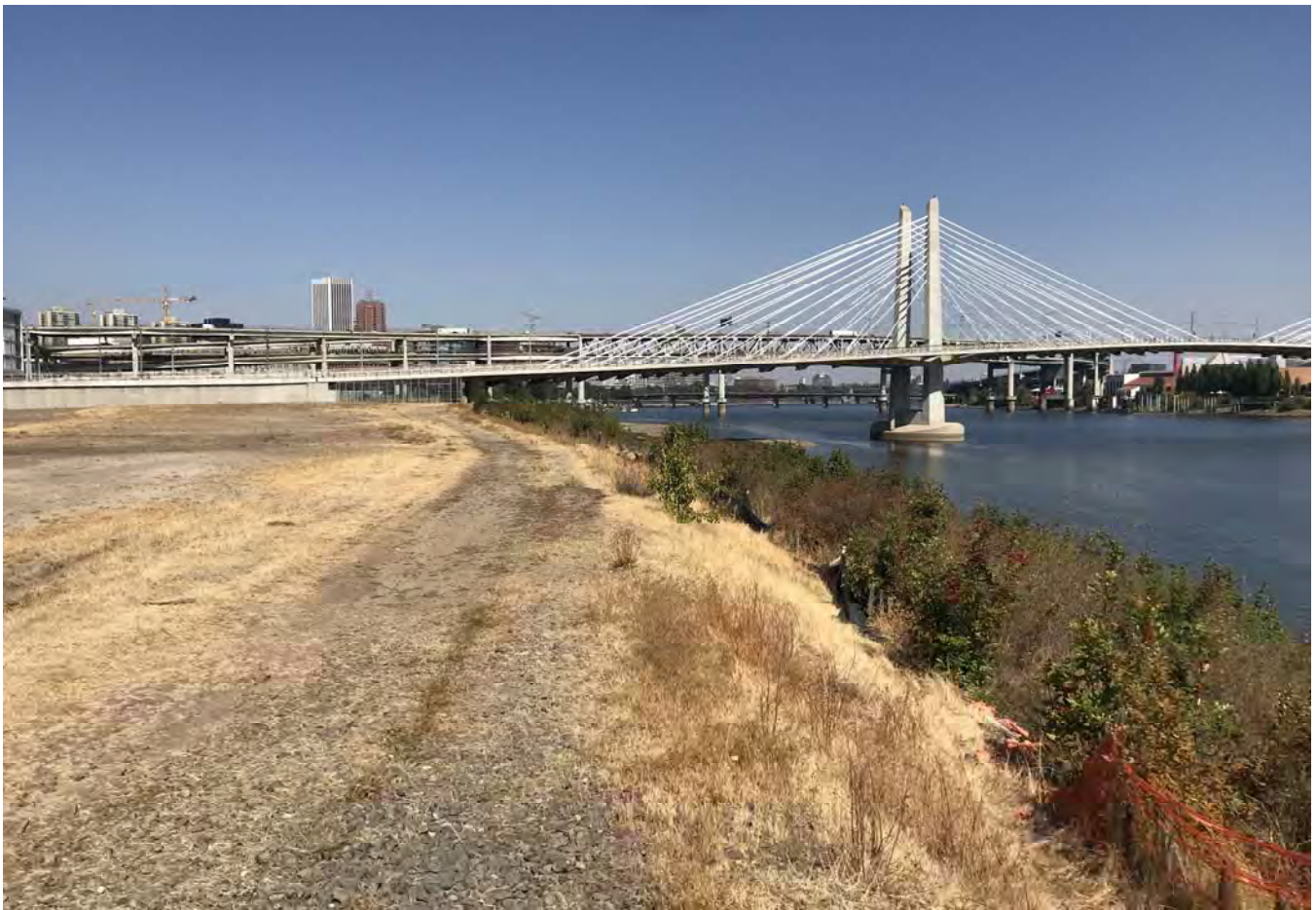
STA: 9+00 - Top of bank looking downstream.
