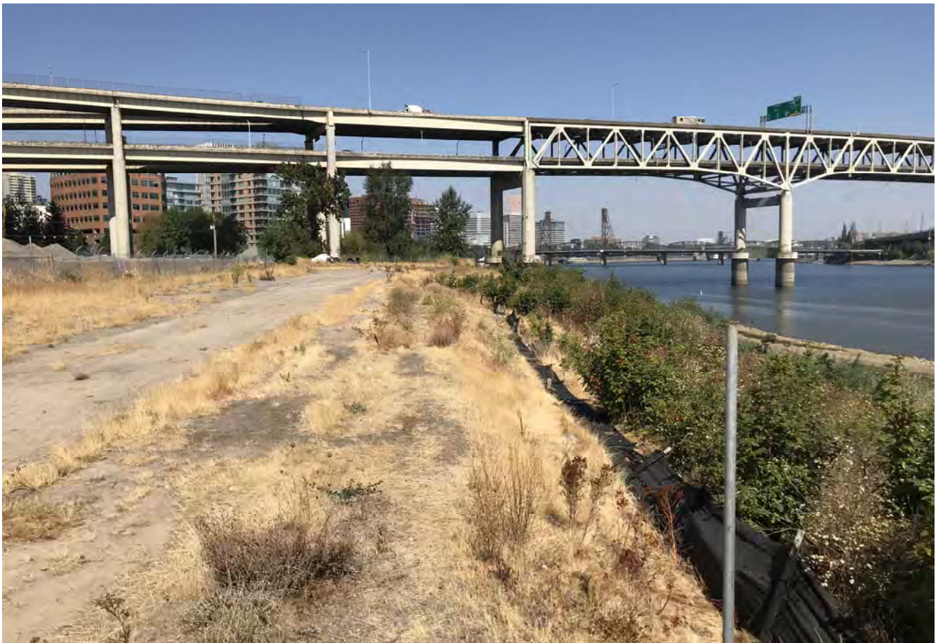
STA: 23+50 - Top of bank looking downstream.
