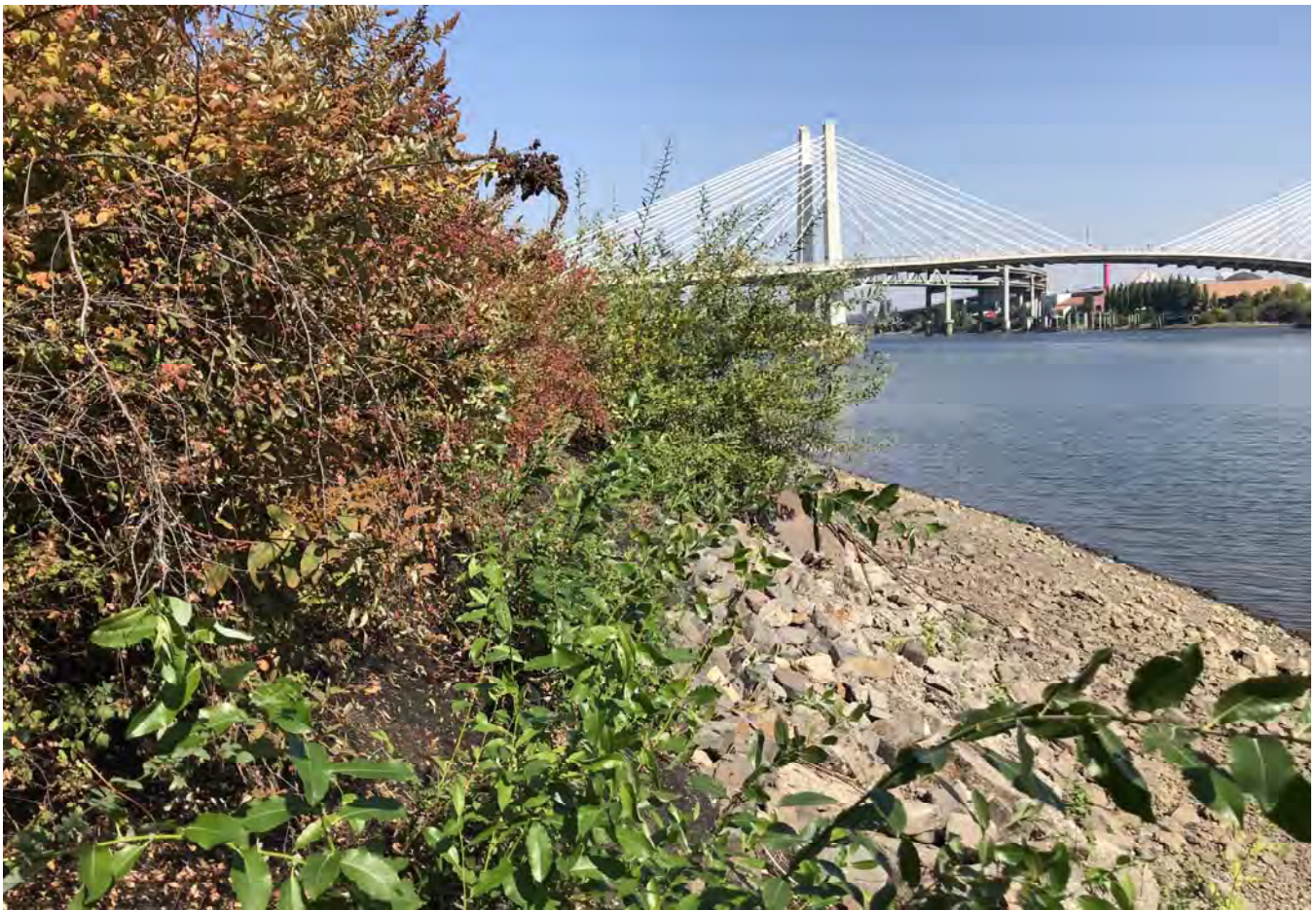
STA: 9+00 - Top of rock armor looking downstream.
