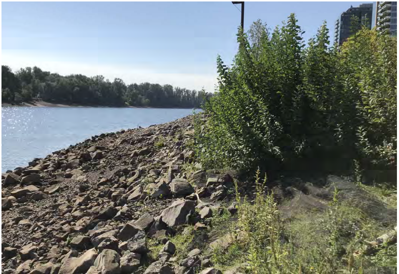
STA: 0+25 - Top of rock armor looking upstream.
