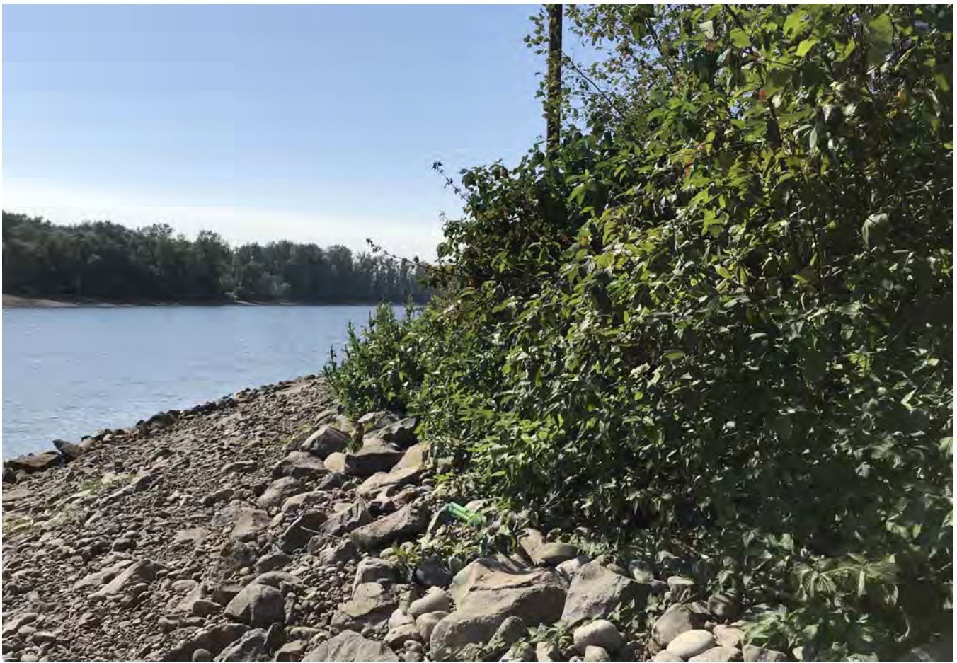
STA: 0+00 - Top of rock armor looking upstream.
