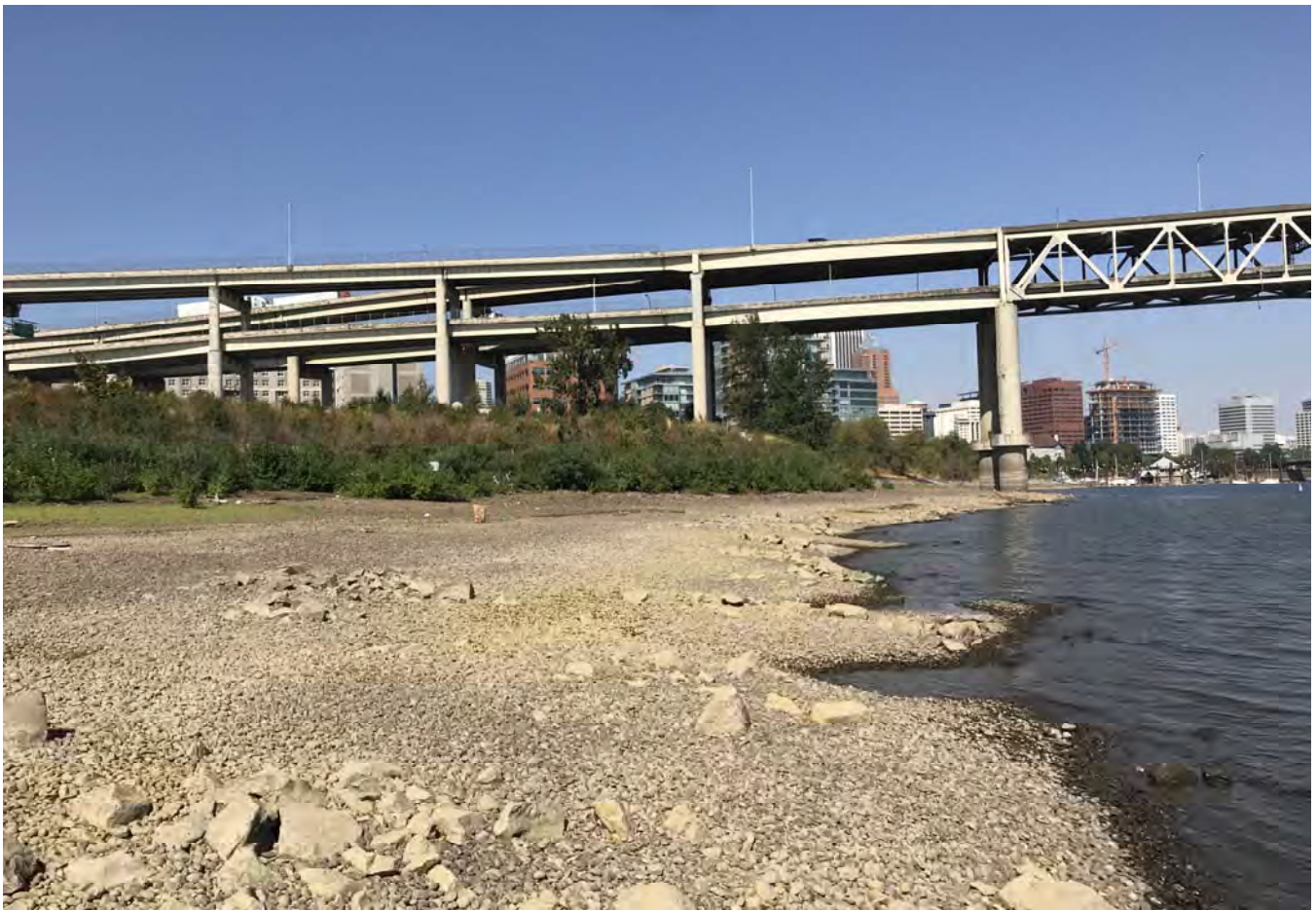
STA: 23+50 - Edge of water looking downstream.
