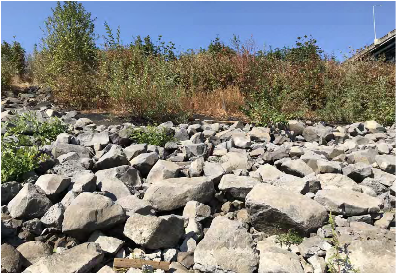
STA: 5+00 - Bottom of rock armor looking west.
