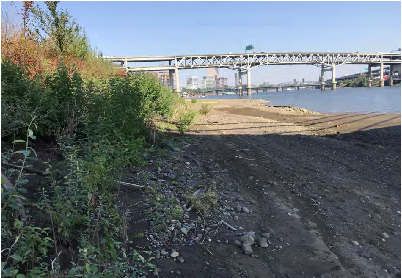
STA: 17+00 - Toe of slope looking downstream.
