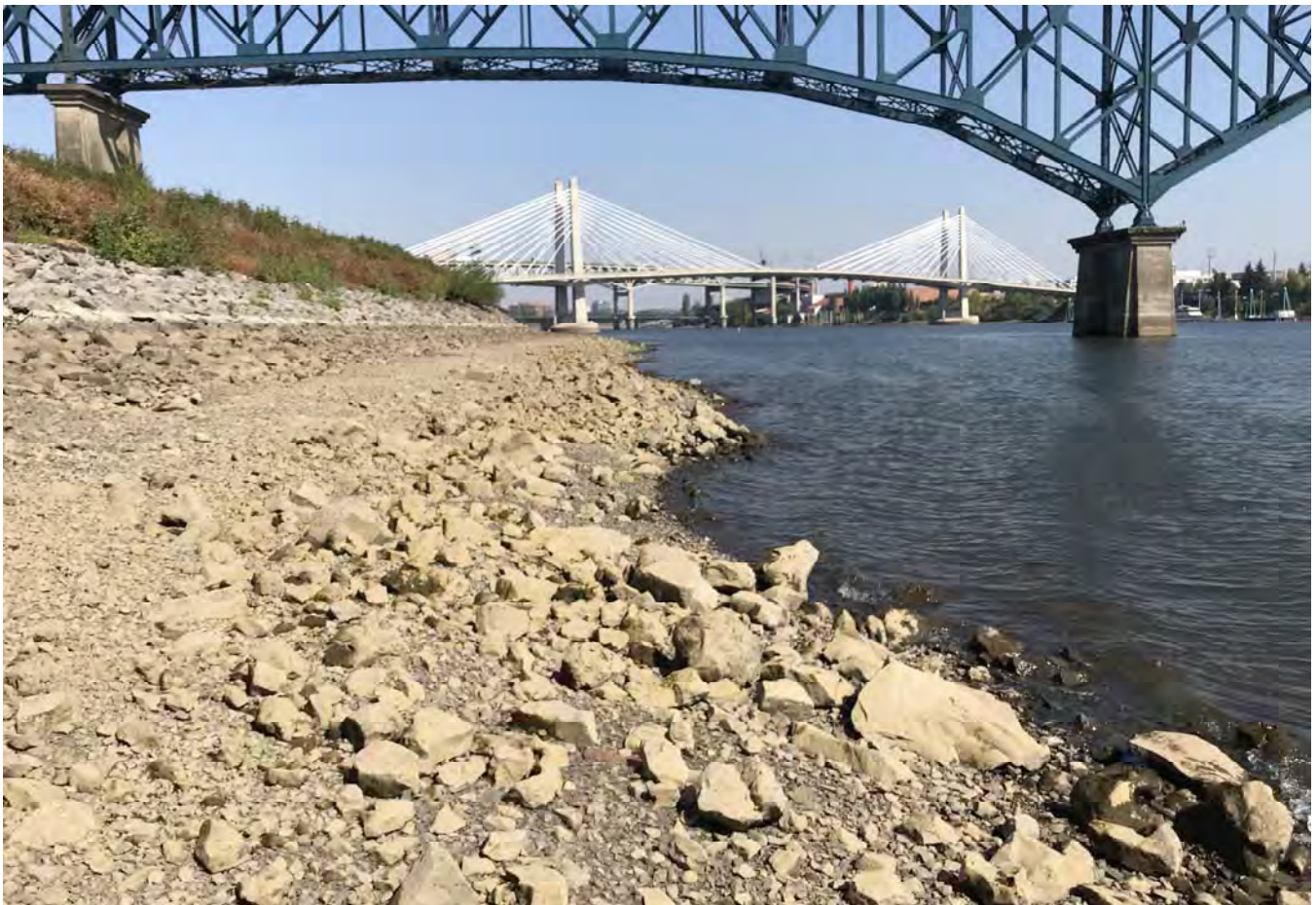
STA: 3+00 - Edge of water looking downstream.
