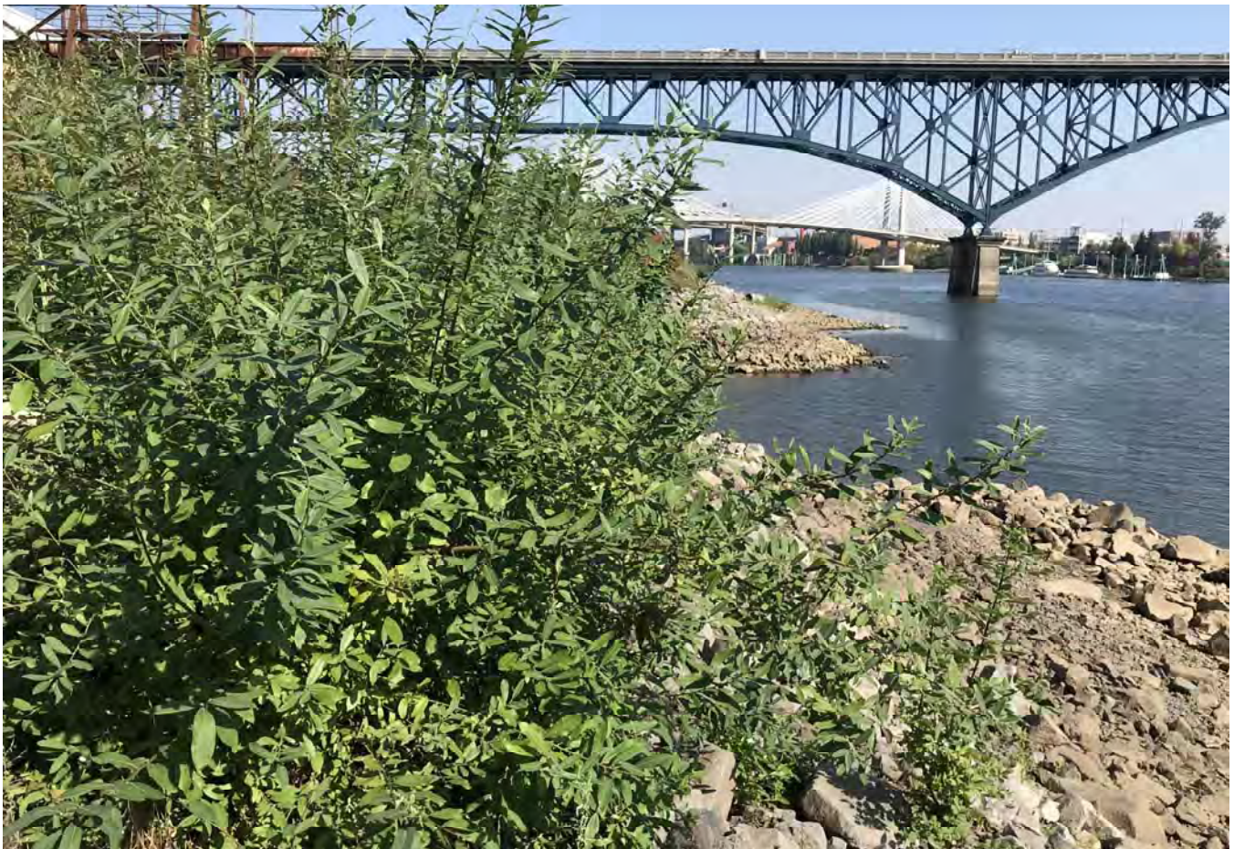
STA: 0+00 - Top of rock armor looking downstream.
