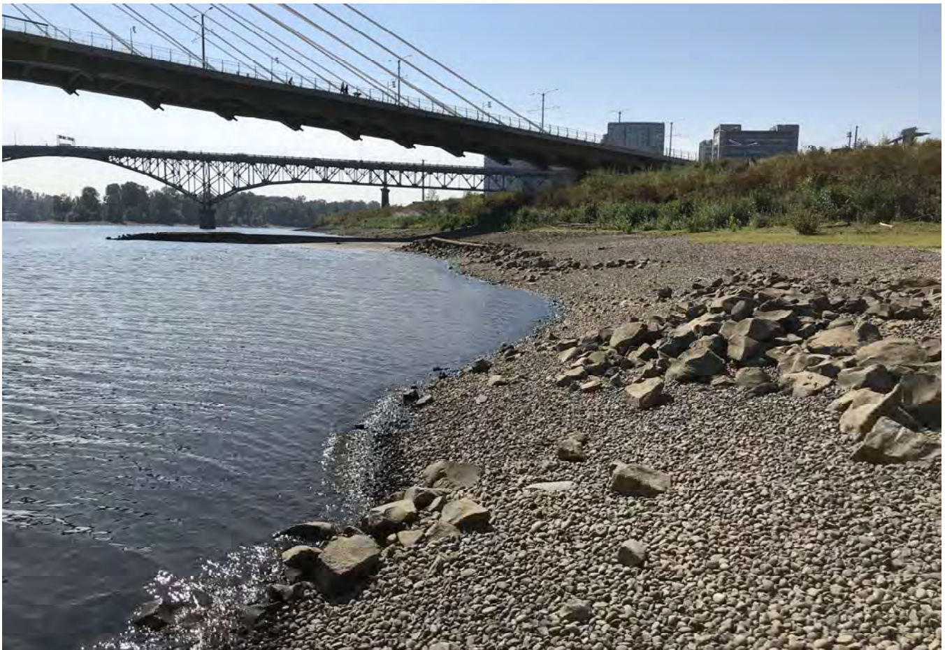
STA: 21+50 - Edge of water looking upstream.
