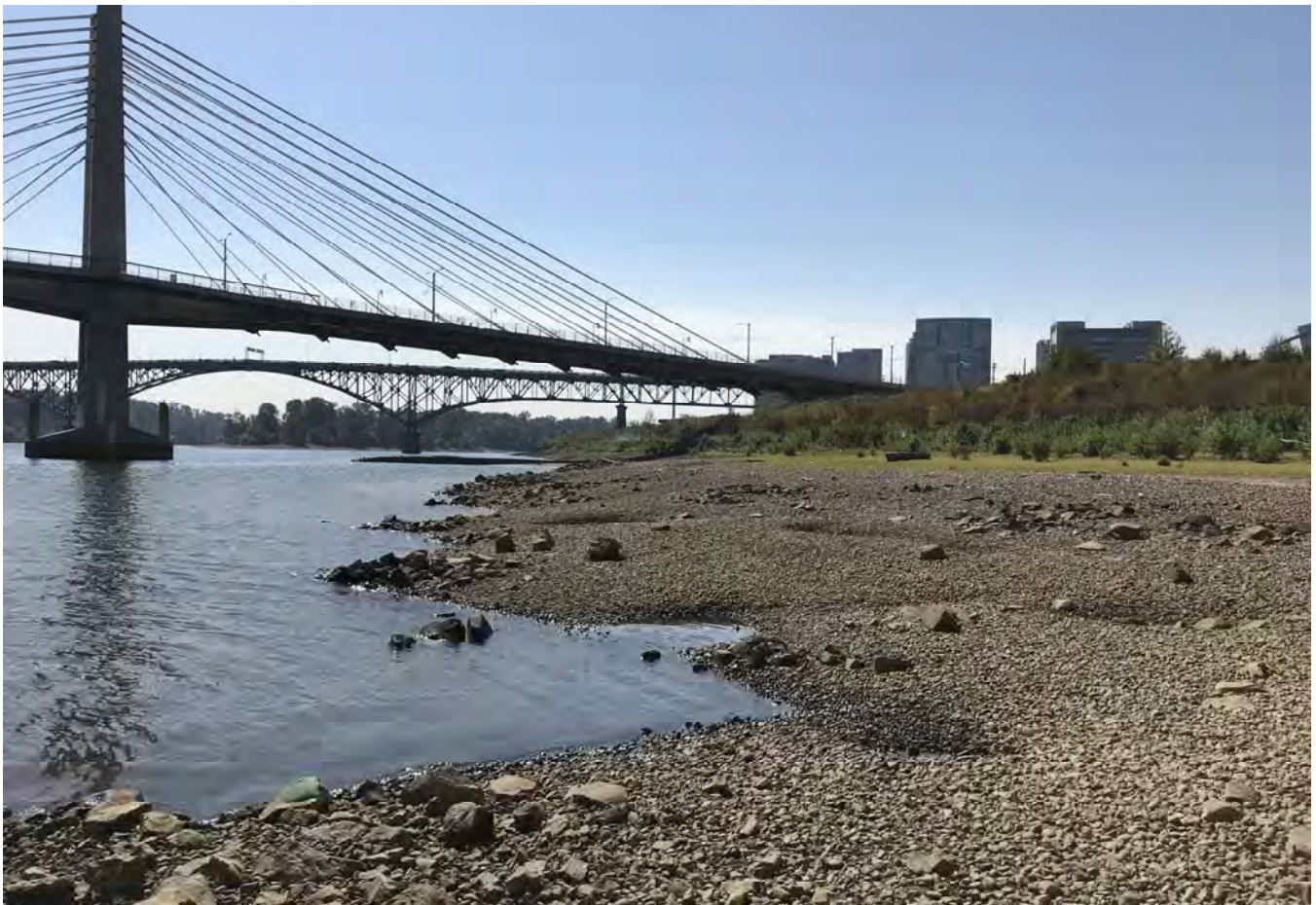
STA: 23+50 - Edge of water looking upstream.
