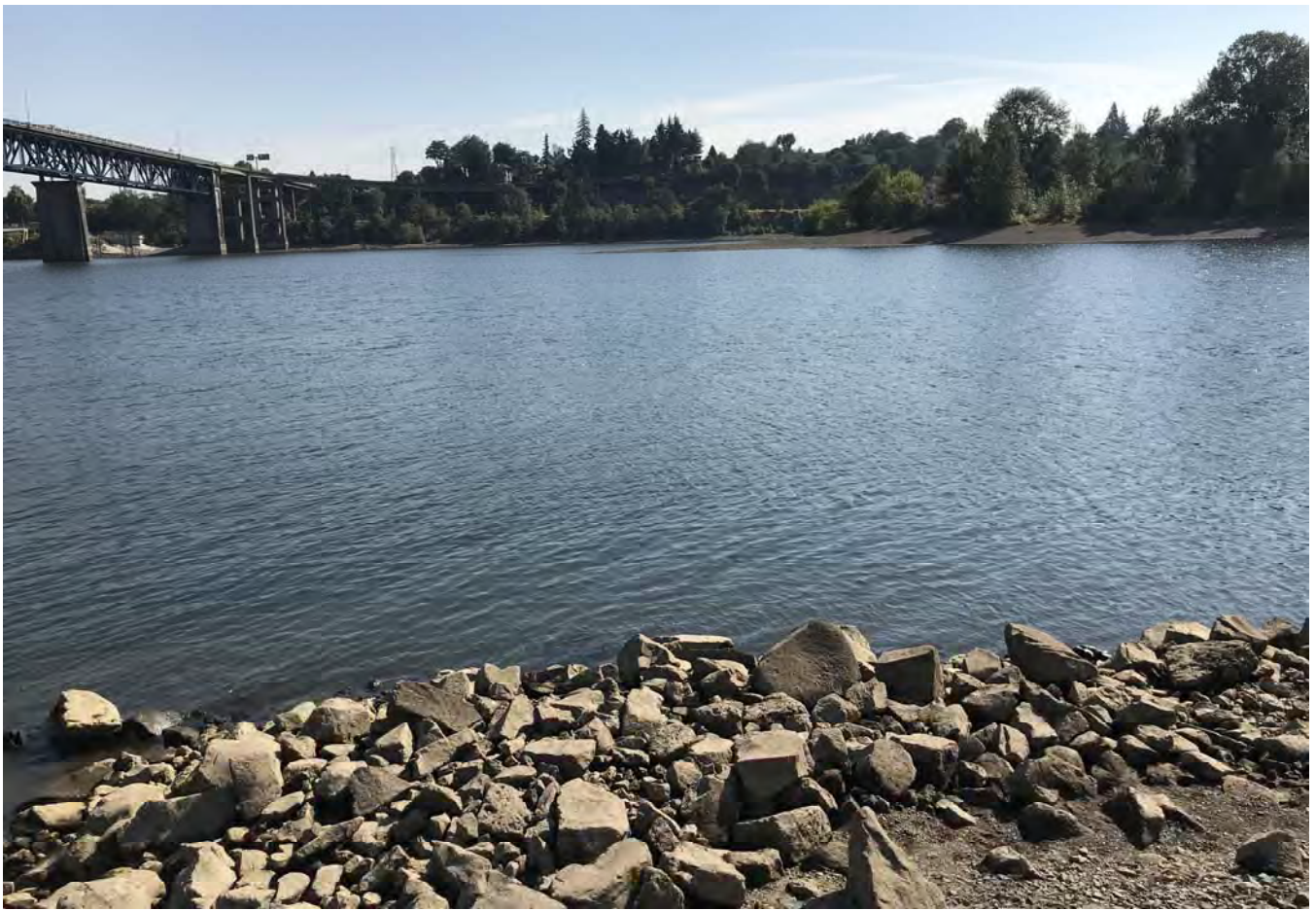
STA: 0+25 - Top of rock armor looking east.
