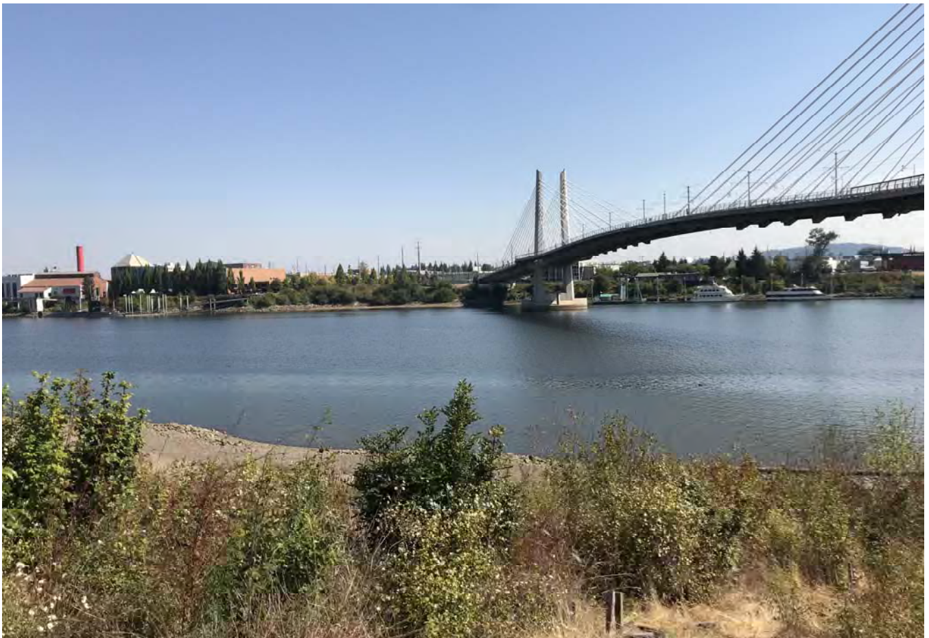
STA: 19+50 - Top of bank looking east.
