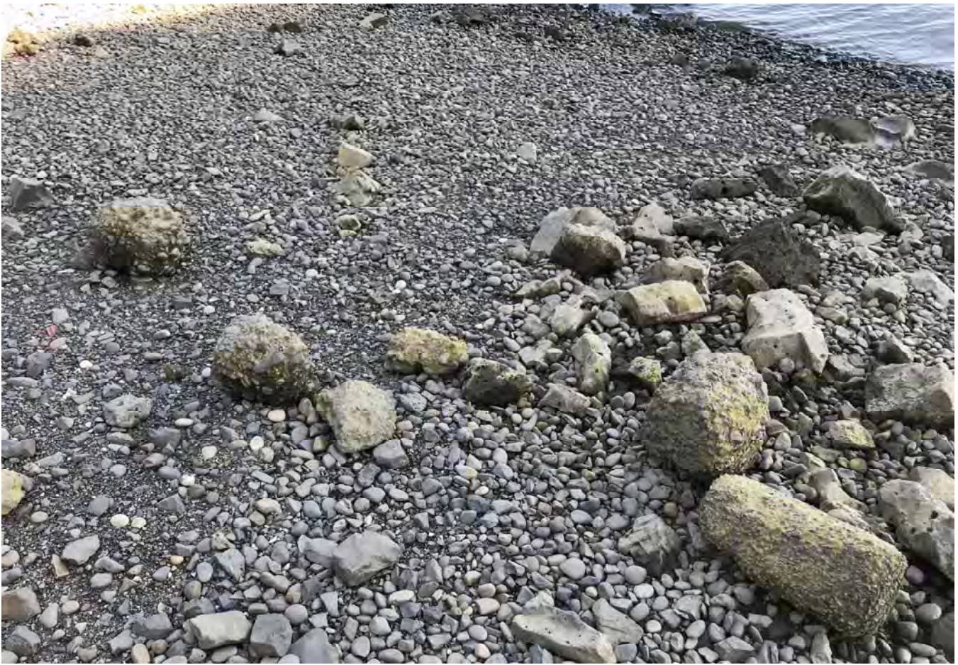
STA: 7+25 - Ballast stones from bank repair area located over sediment cap.
