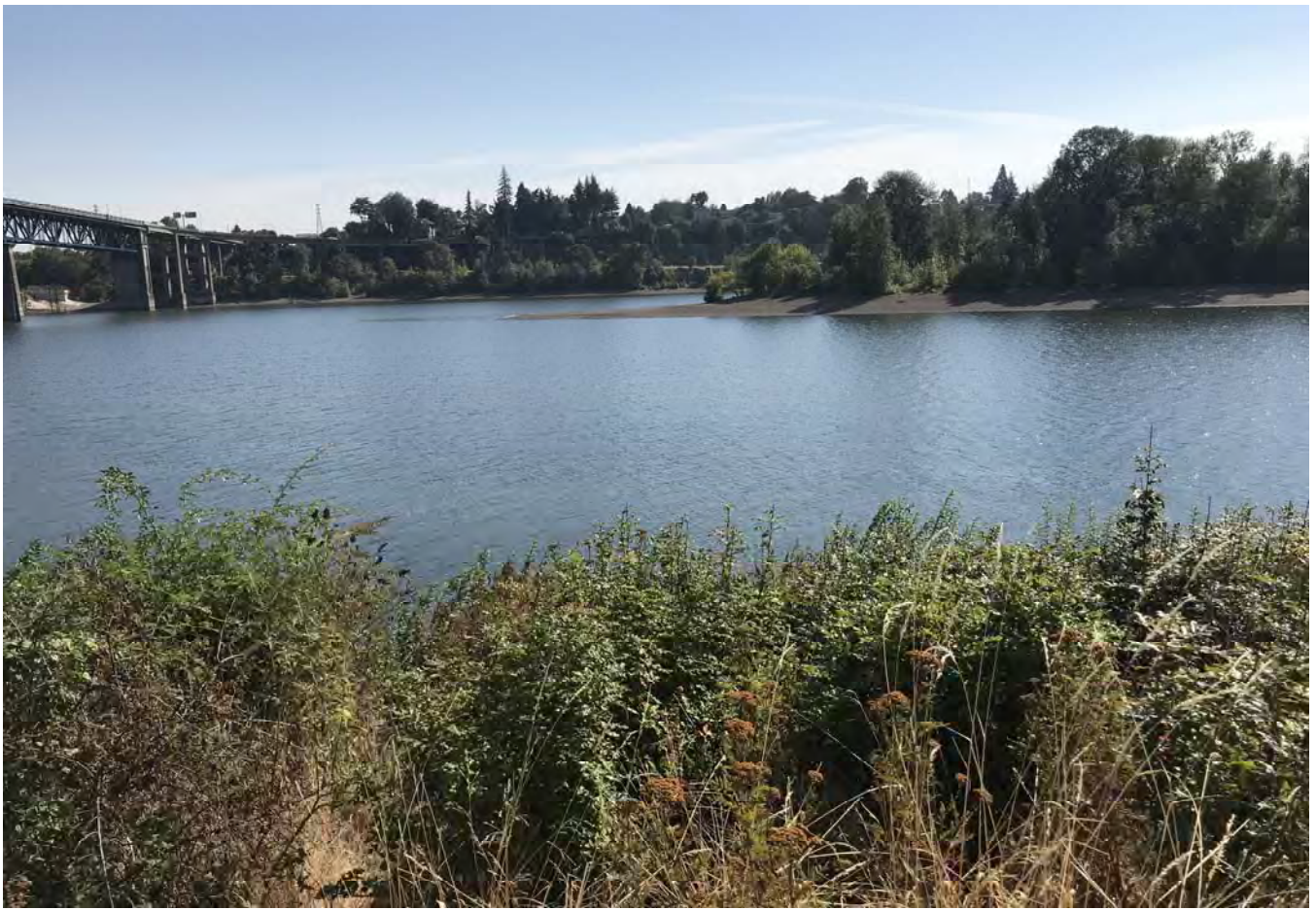
STA: 0+25 - Top of bank looking east.
