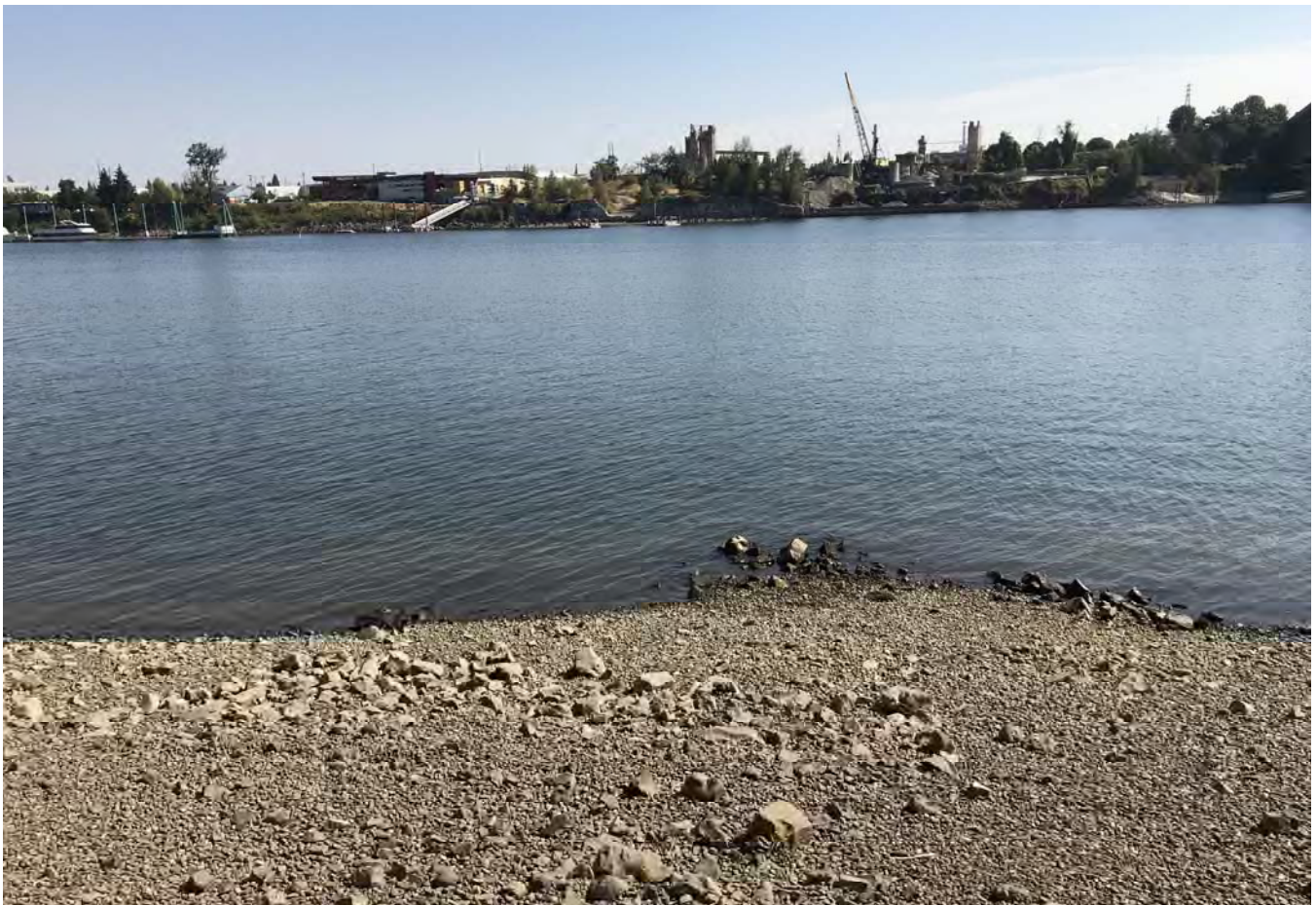
STA: 9+00 - Top of rock armor looking east.
