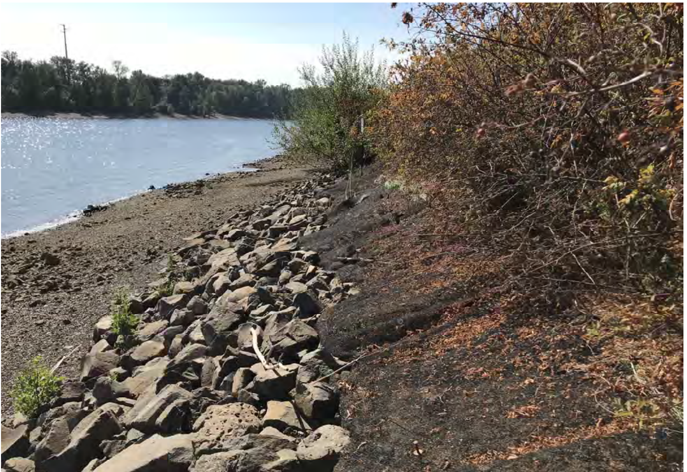
STA: 7+00 - Top of rock armor looking upstream.
