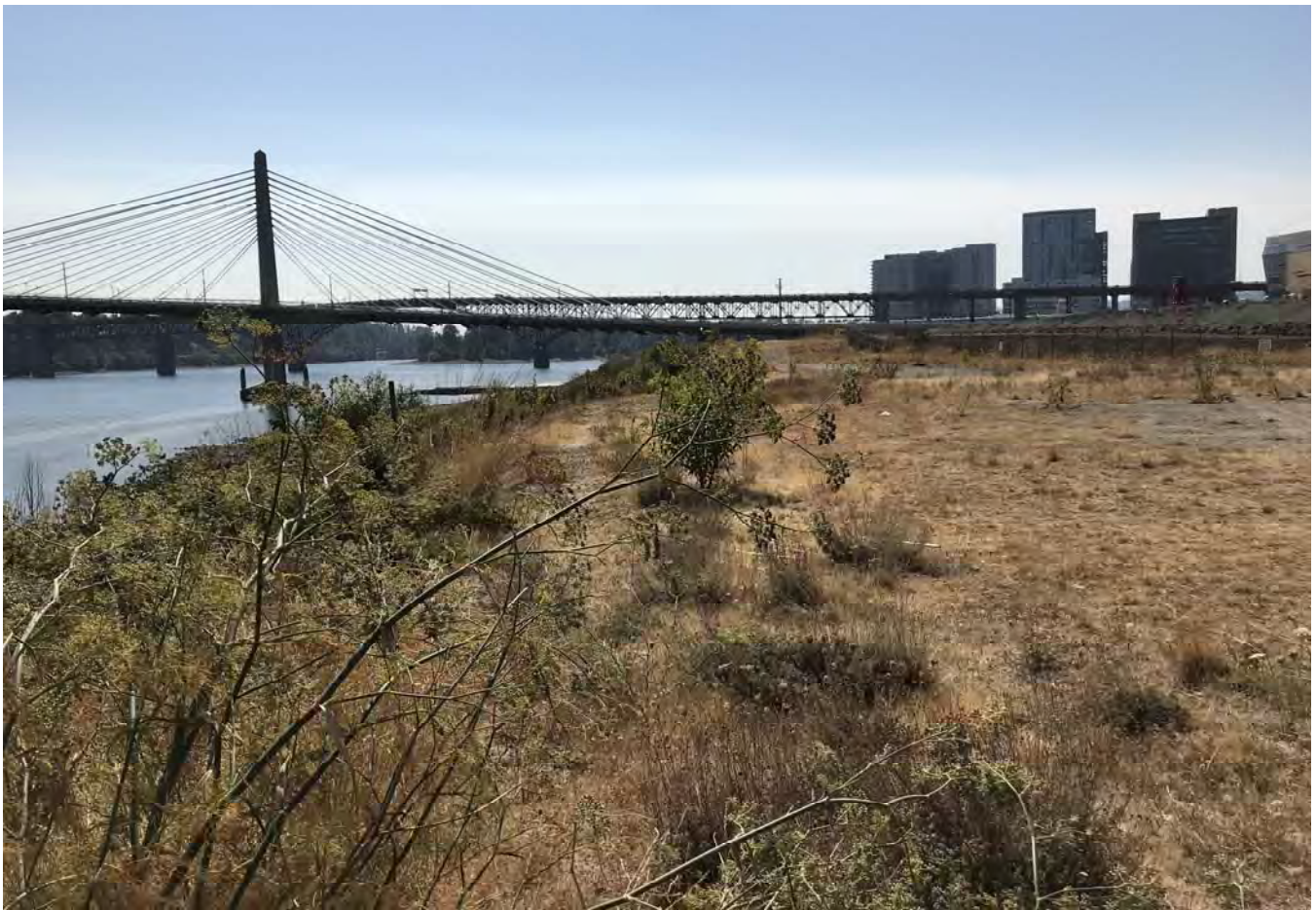
STA: 26+50 - Top of bank looking upstream.
