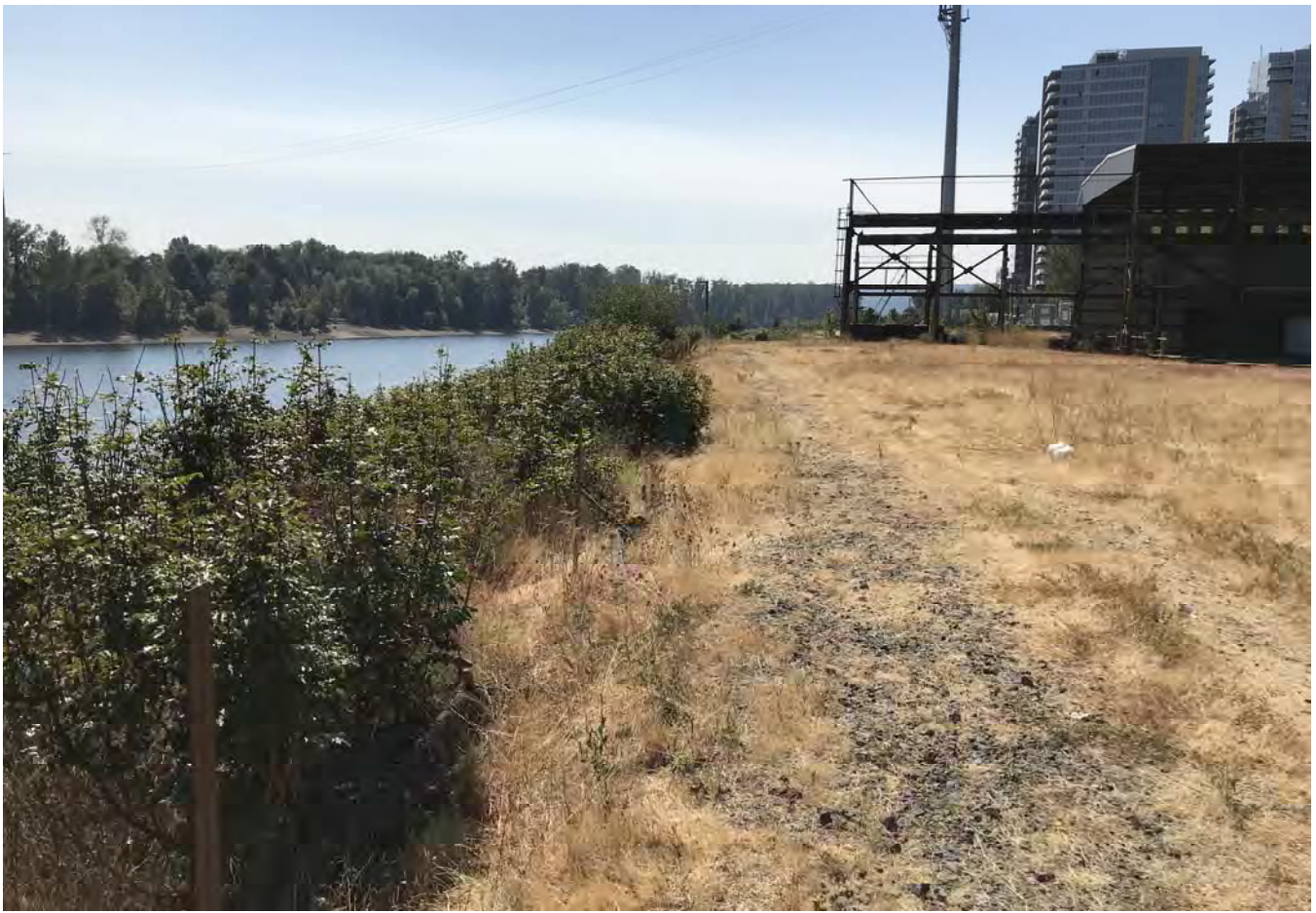
STA: 5+00 - Top of bank looking upstream.
