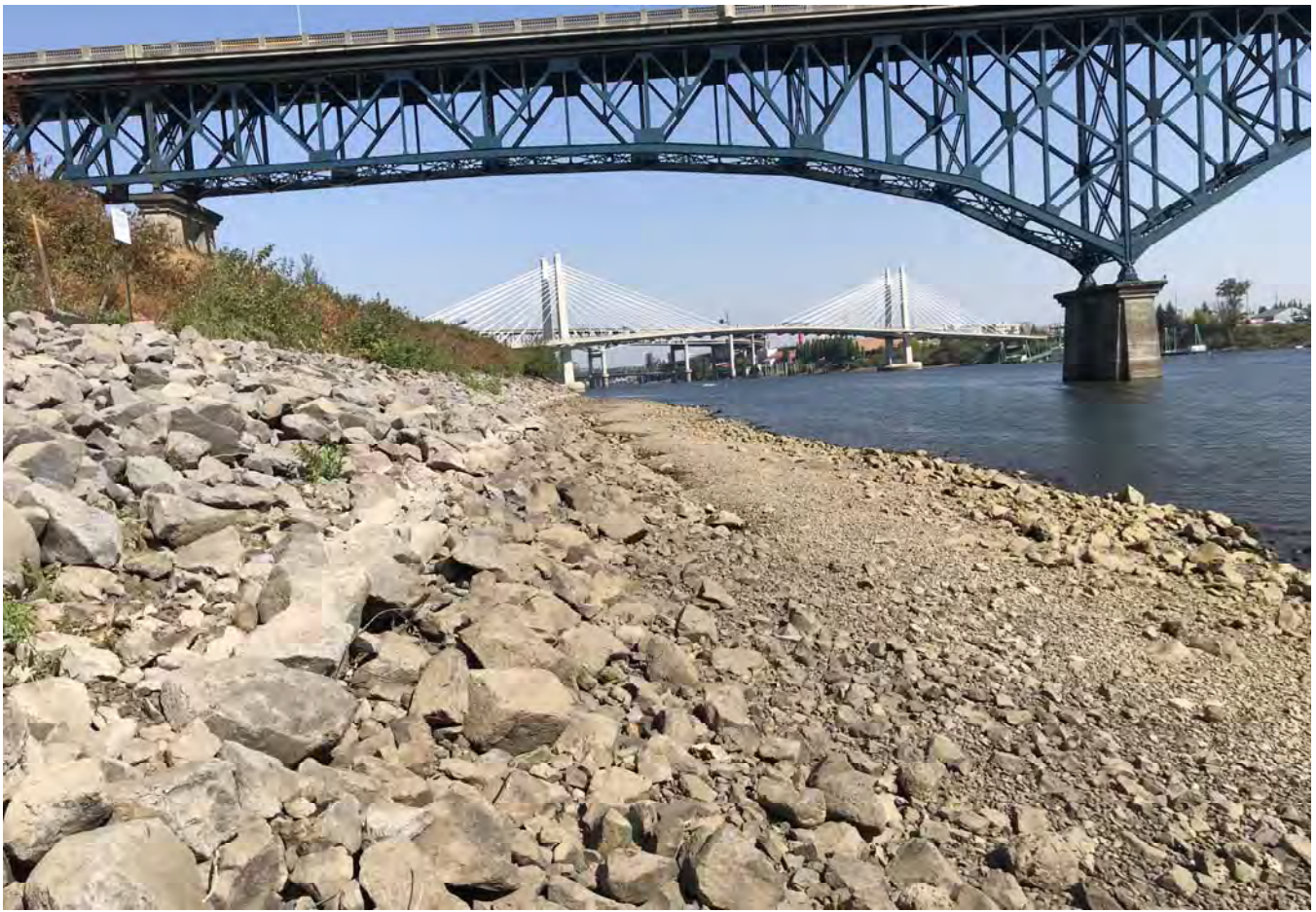
STA: 3+00 - Bottom of rock armor looking downstream.
