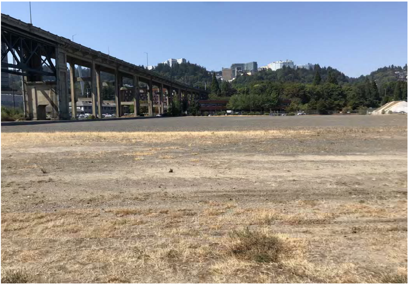
STA: 9+00 - Top of bank looking west.
