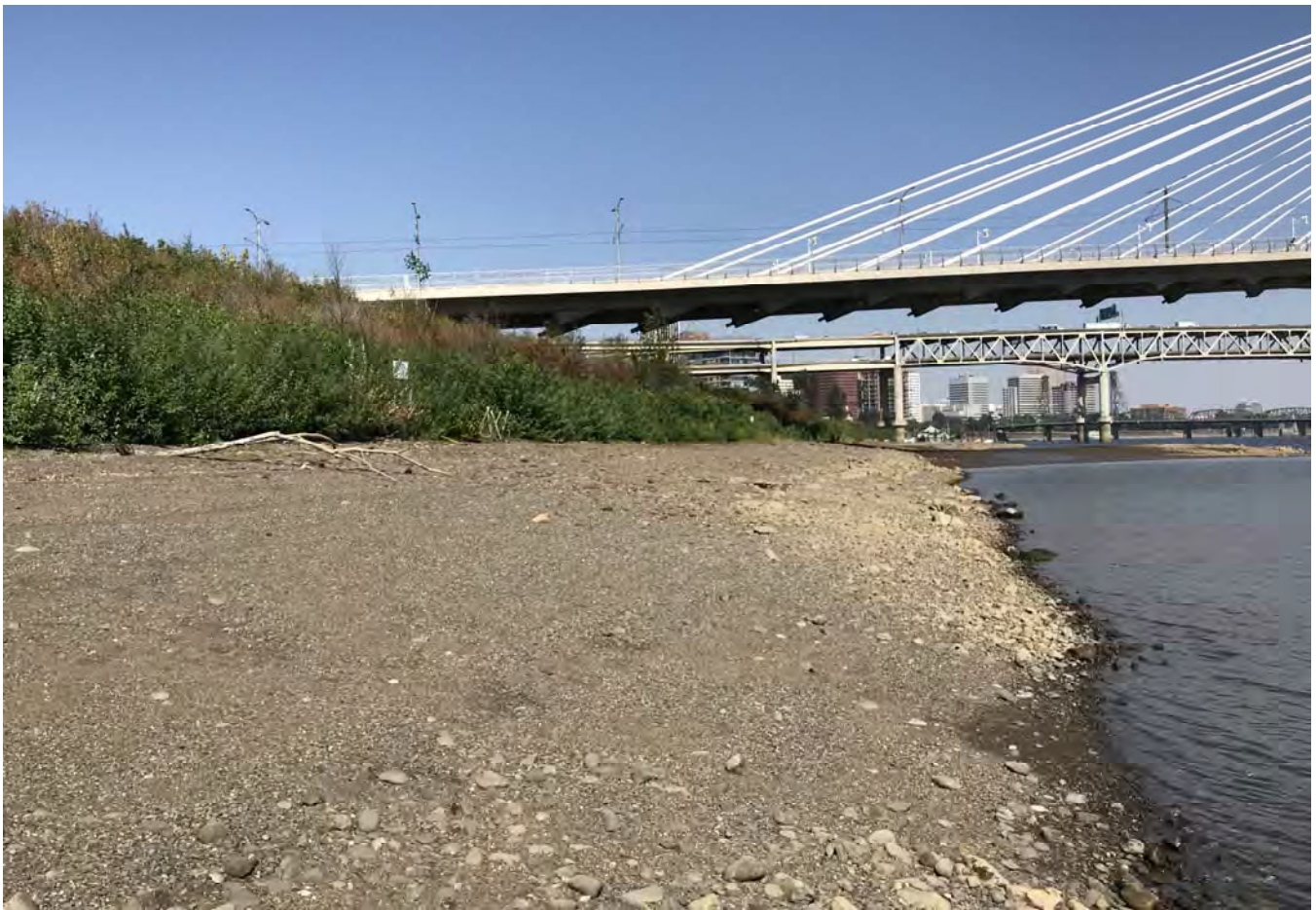
STA: 13+00 - Edge of water looking downstream.
