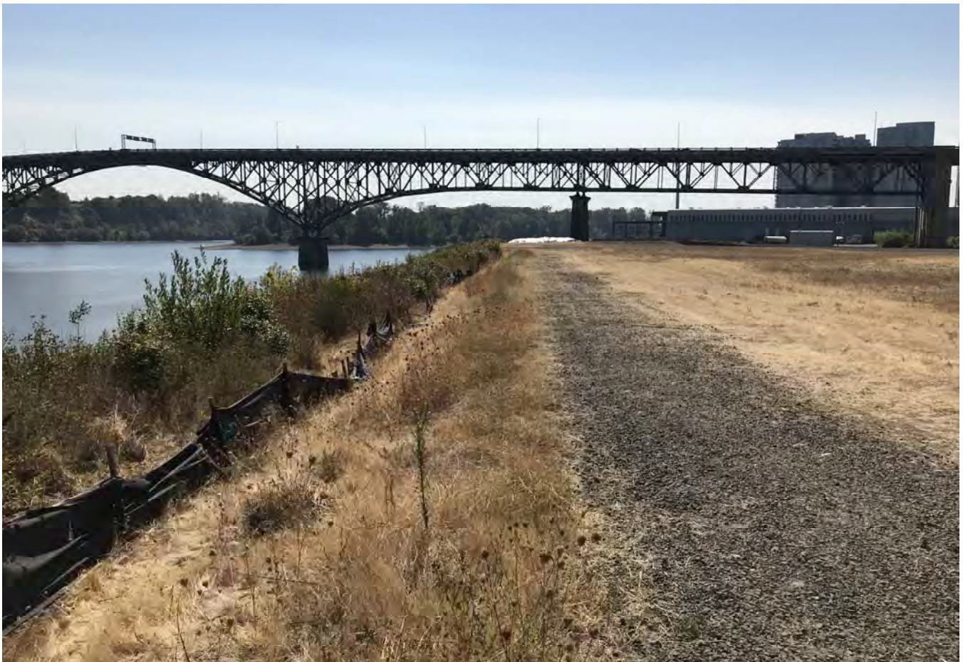
STA: 15+00 - Top of bank looking upstream.
