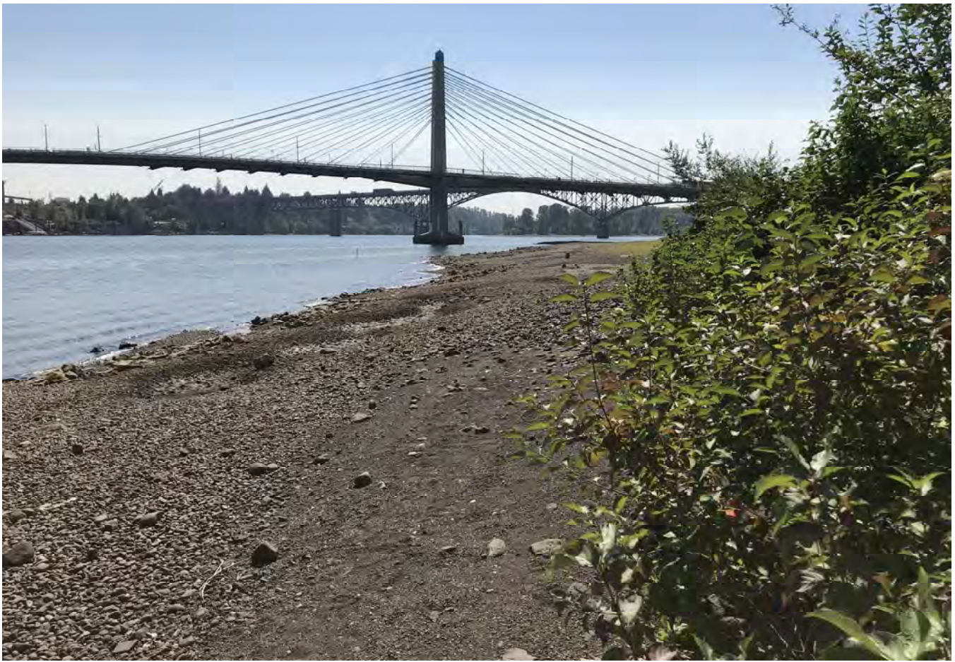
STA: 26+50 - Toe of slope looking upstream.
