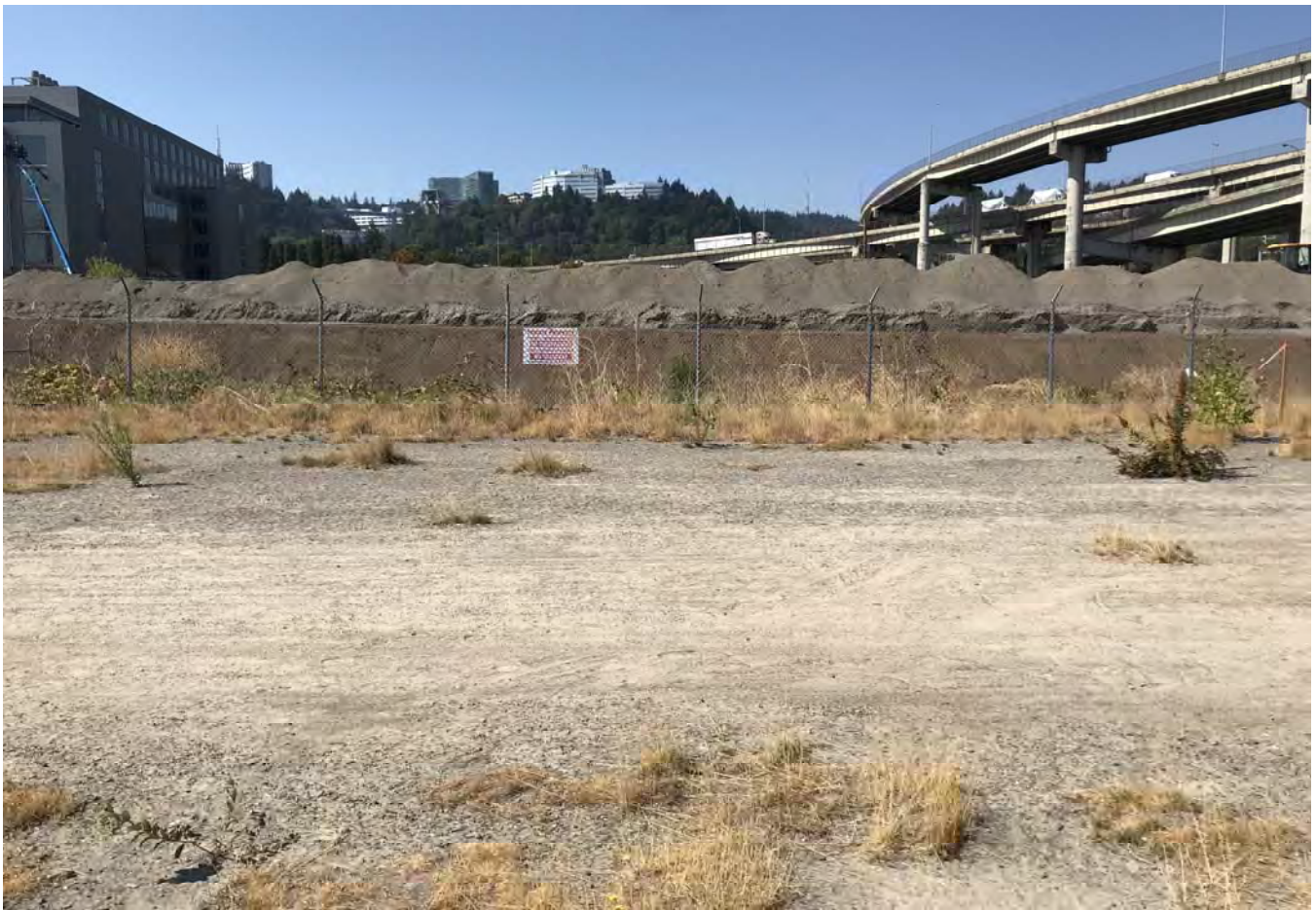
STA: 25+50 - Top of bank looking west.
