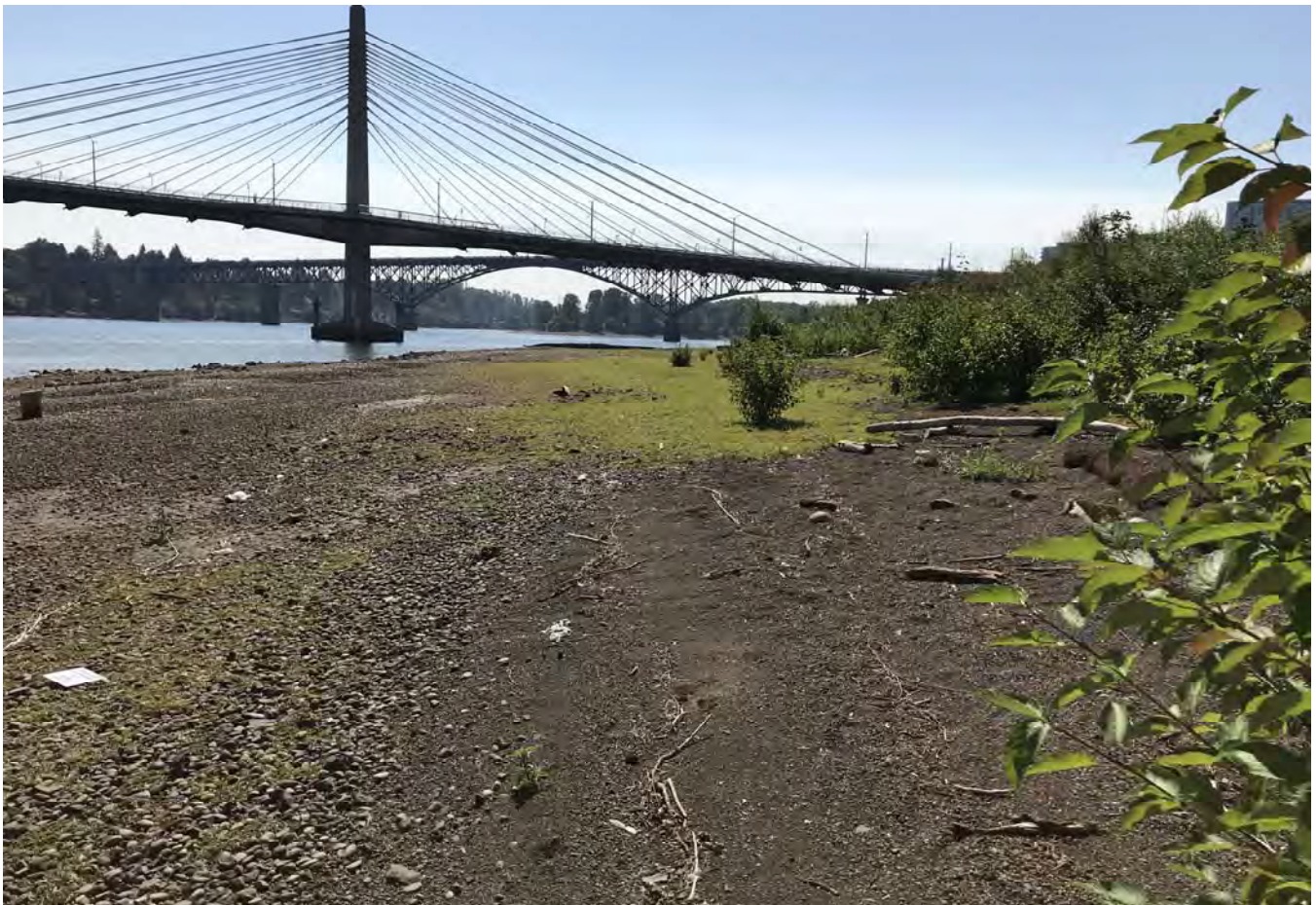
STA: 25+50 - Toe of slope looking upstream.
