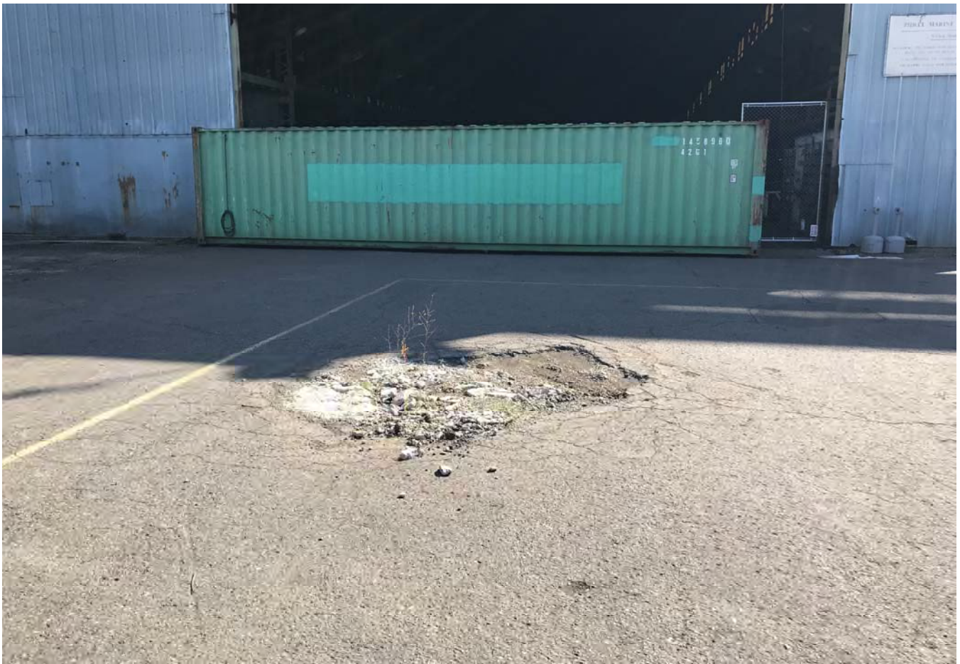
Operational area west of barge building looking east.
