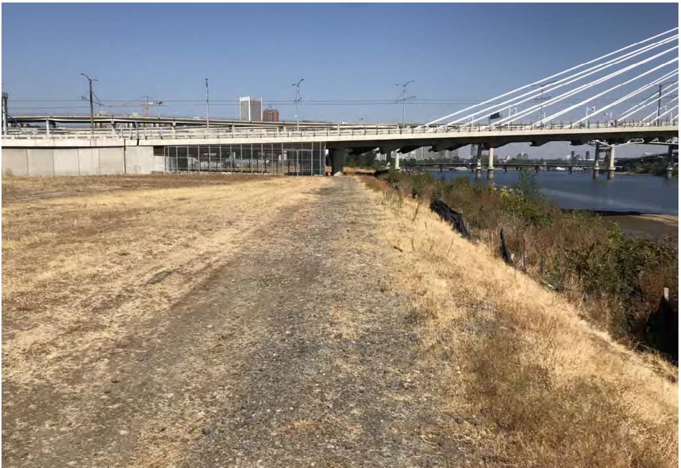
STA: 13+00 - Top of bank looking downstream.
