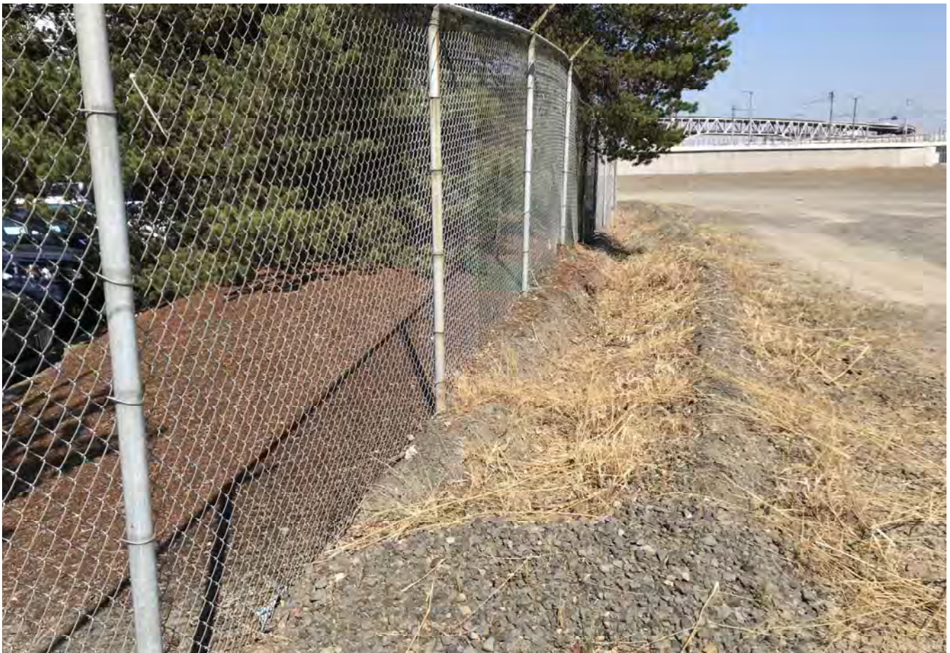
Fence along 3030 Moody property.
