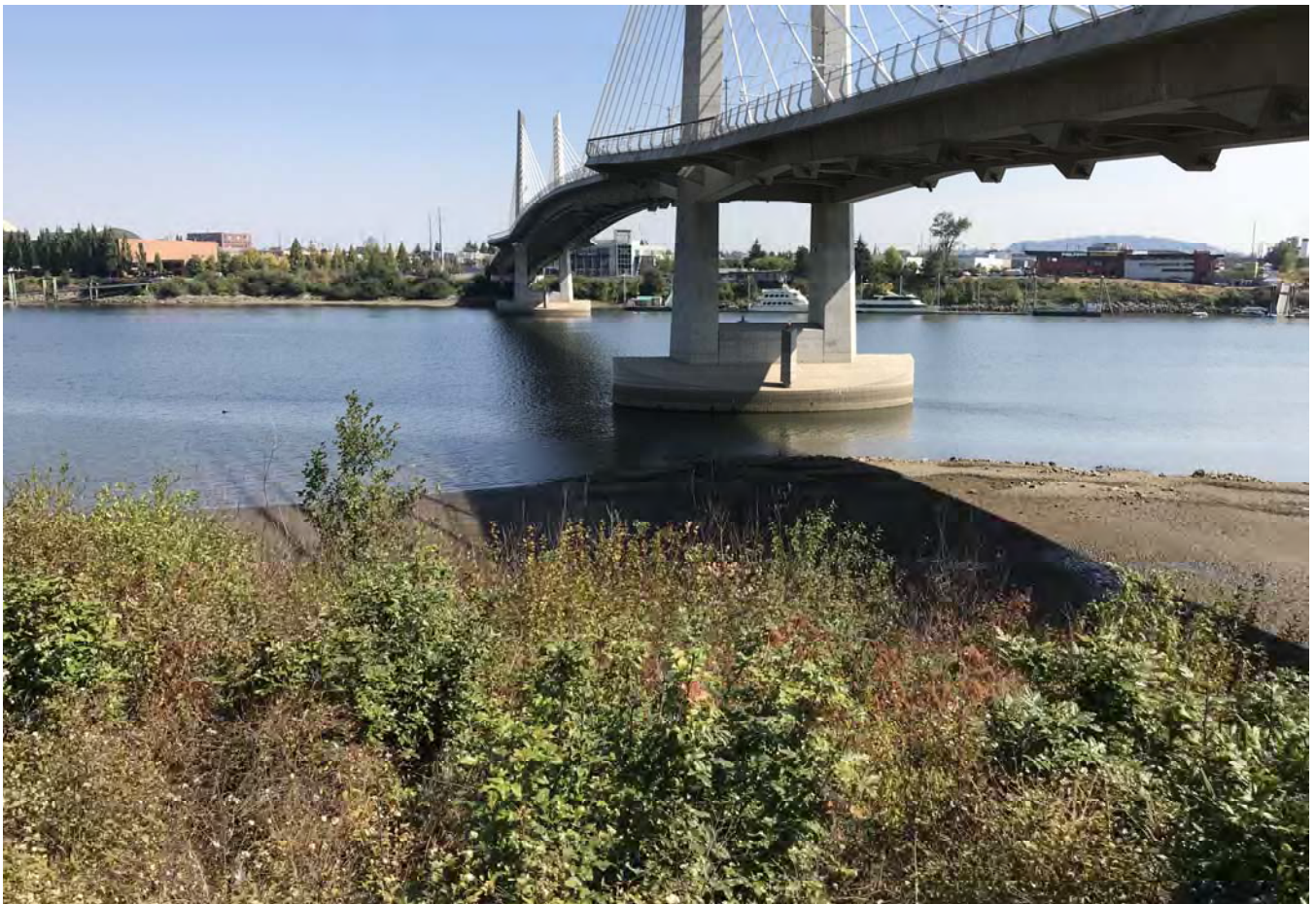
STA: 17+00 - Top of bank looking east.
