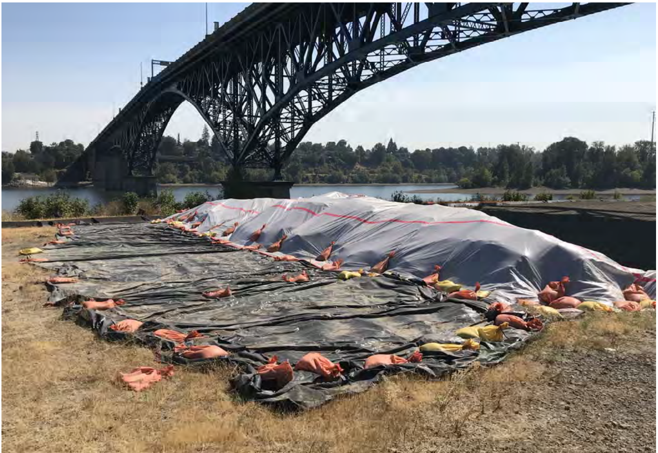
Covered materials from recent Oregon Department of Transportation work on Ross Island Bridge.
