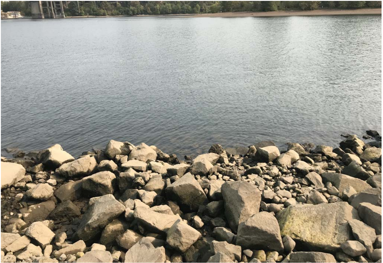
STA: 0+00 - Toe of slope looking east
