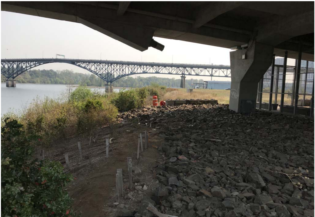
STA: 17+00 - Top of bank looking upstream
