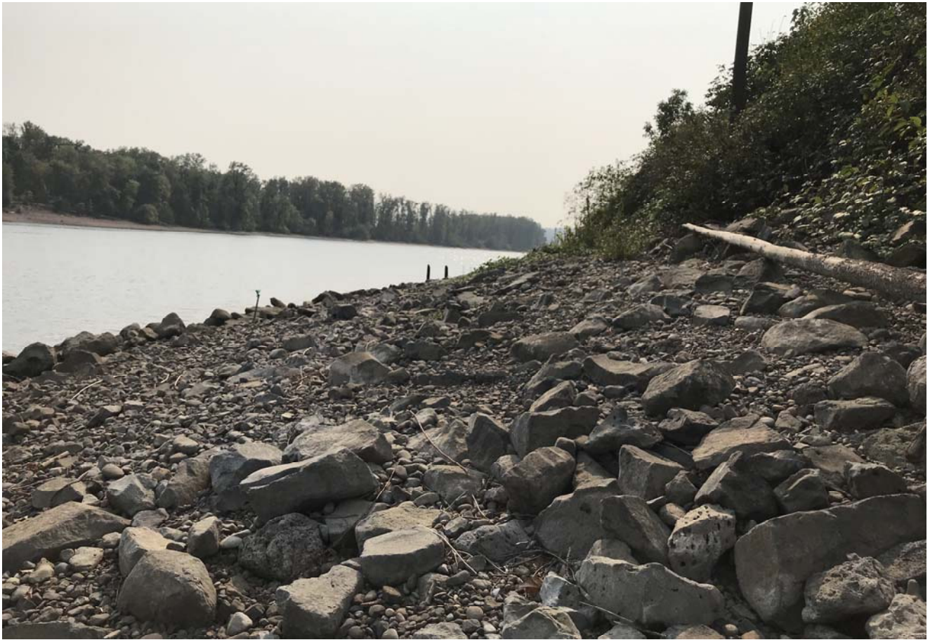
STA: 0+00 - Toe of slope looking upstream
