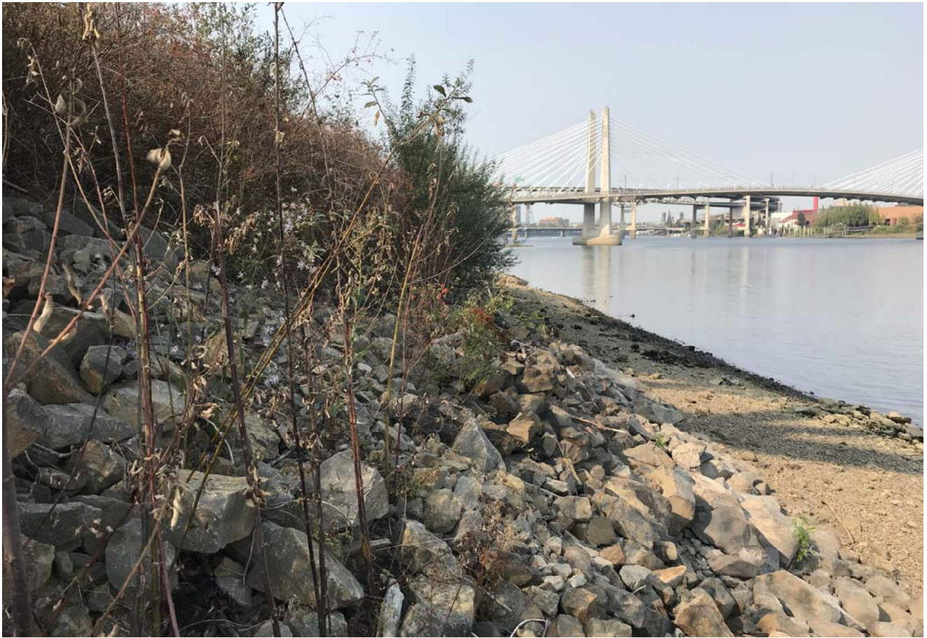
STA: 7+00 - Top of rock armor looking downstream
