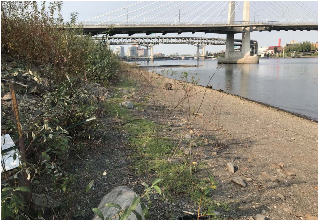
STA: 13+00 - Toe of slope looking downstream
