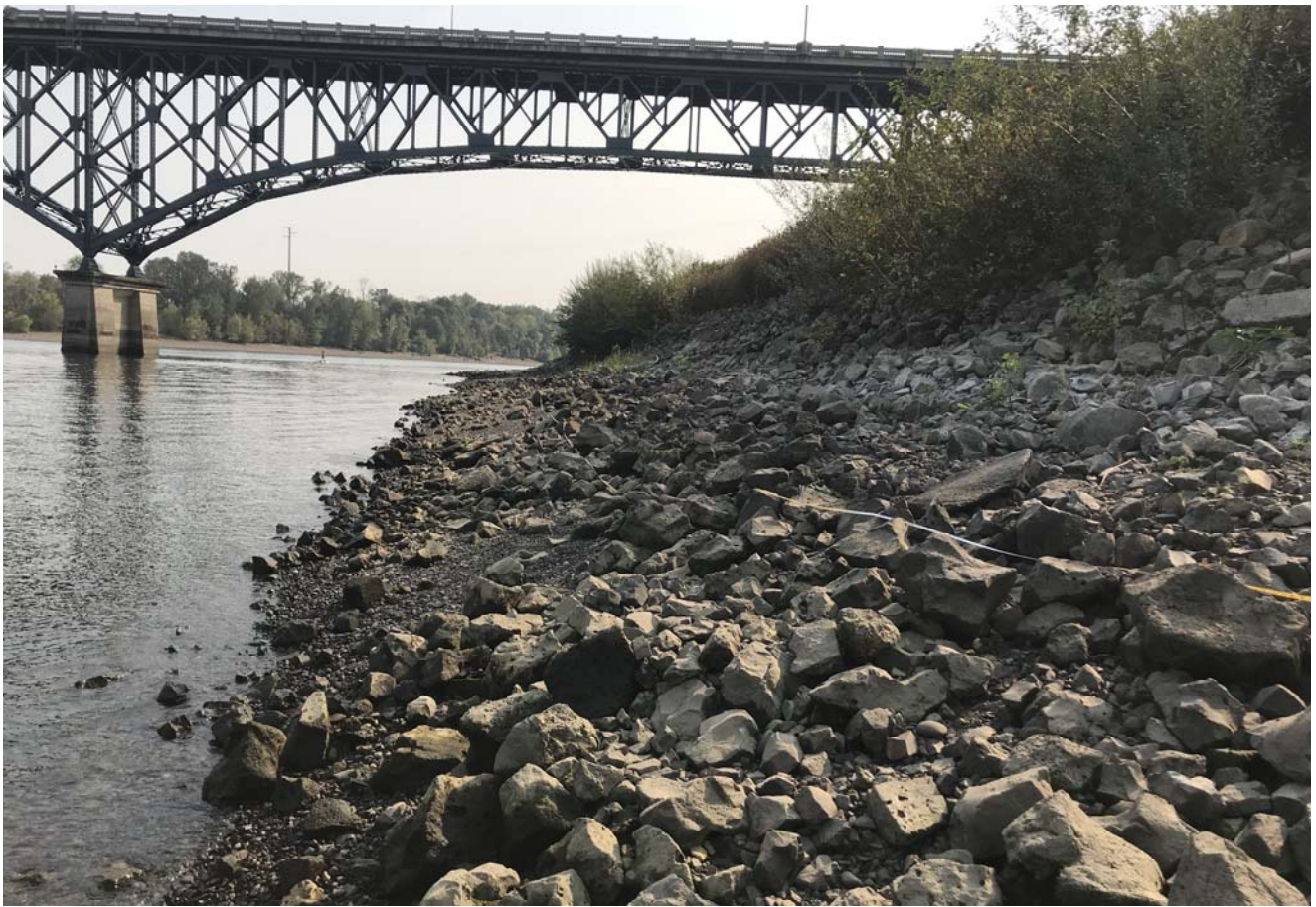
STA: 11+00 - Edge of water looking upstream
