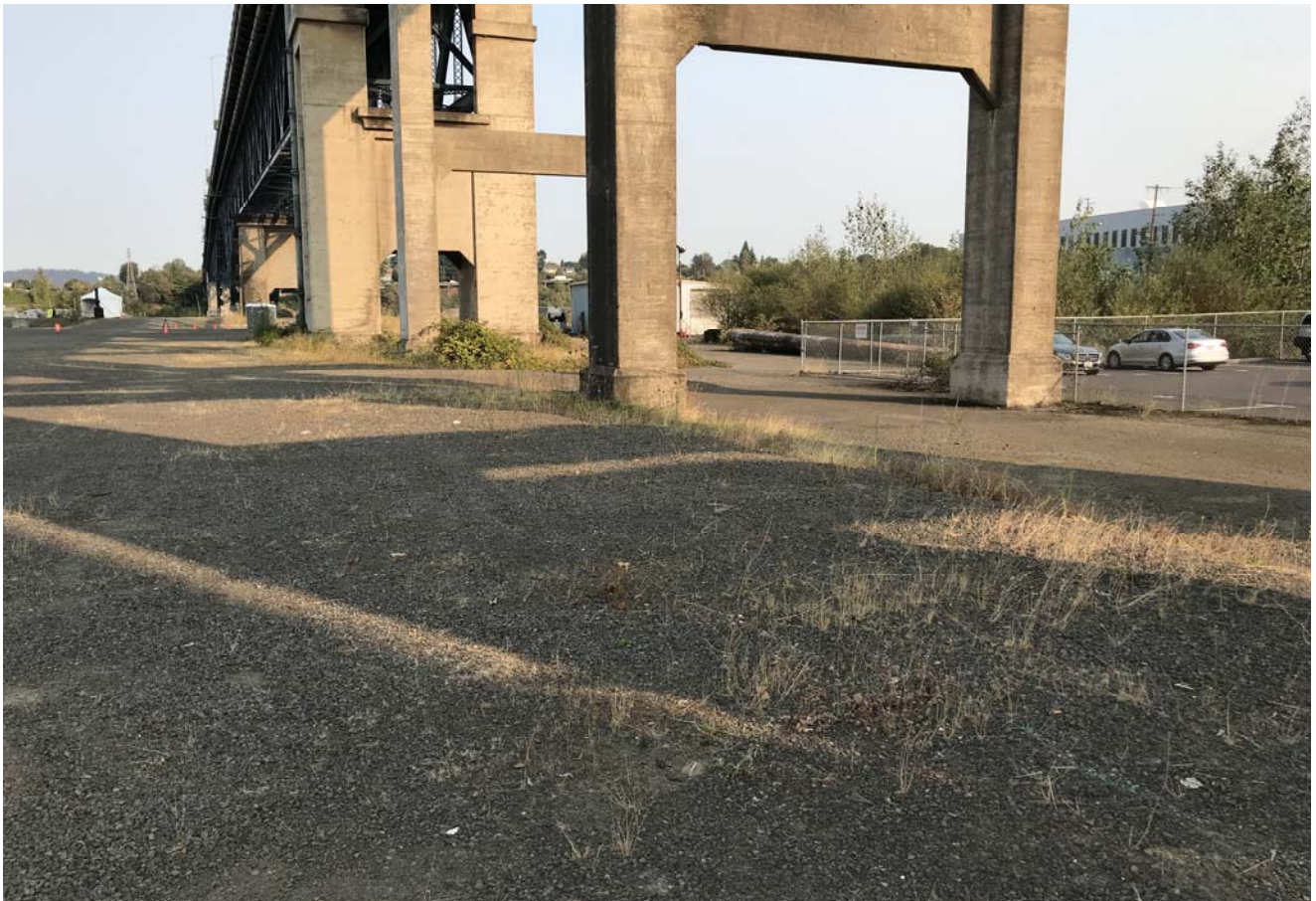
Upland cap - Southwest corner looking east
