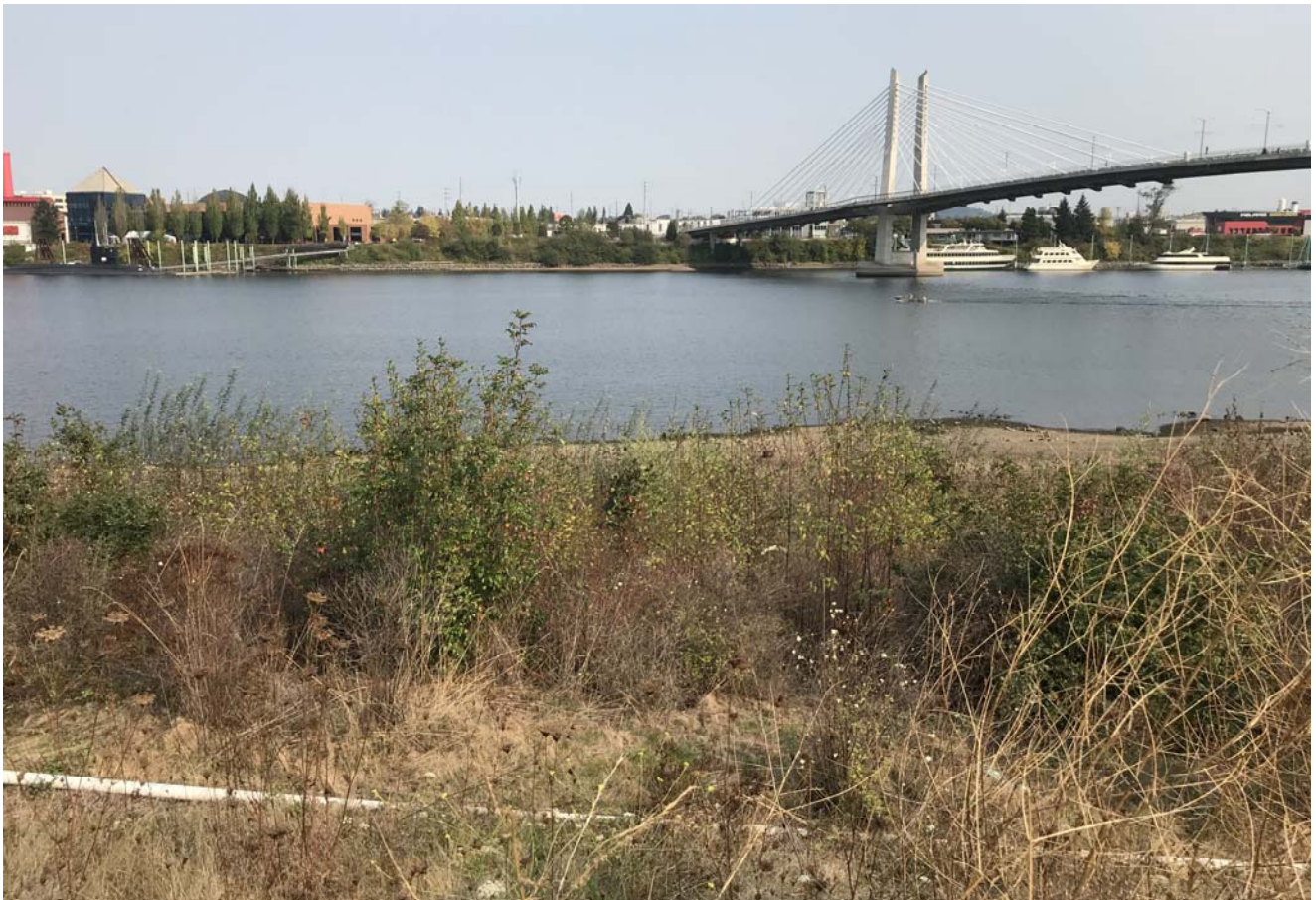
STA: 23+50 - Top of bank looking east
