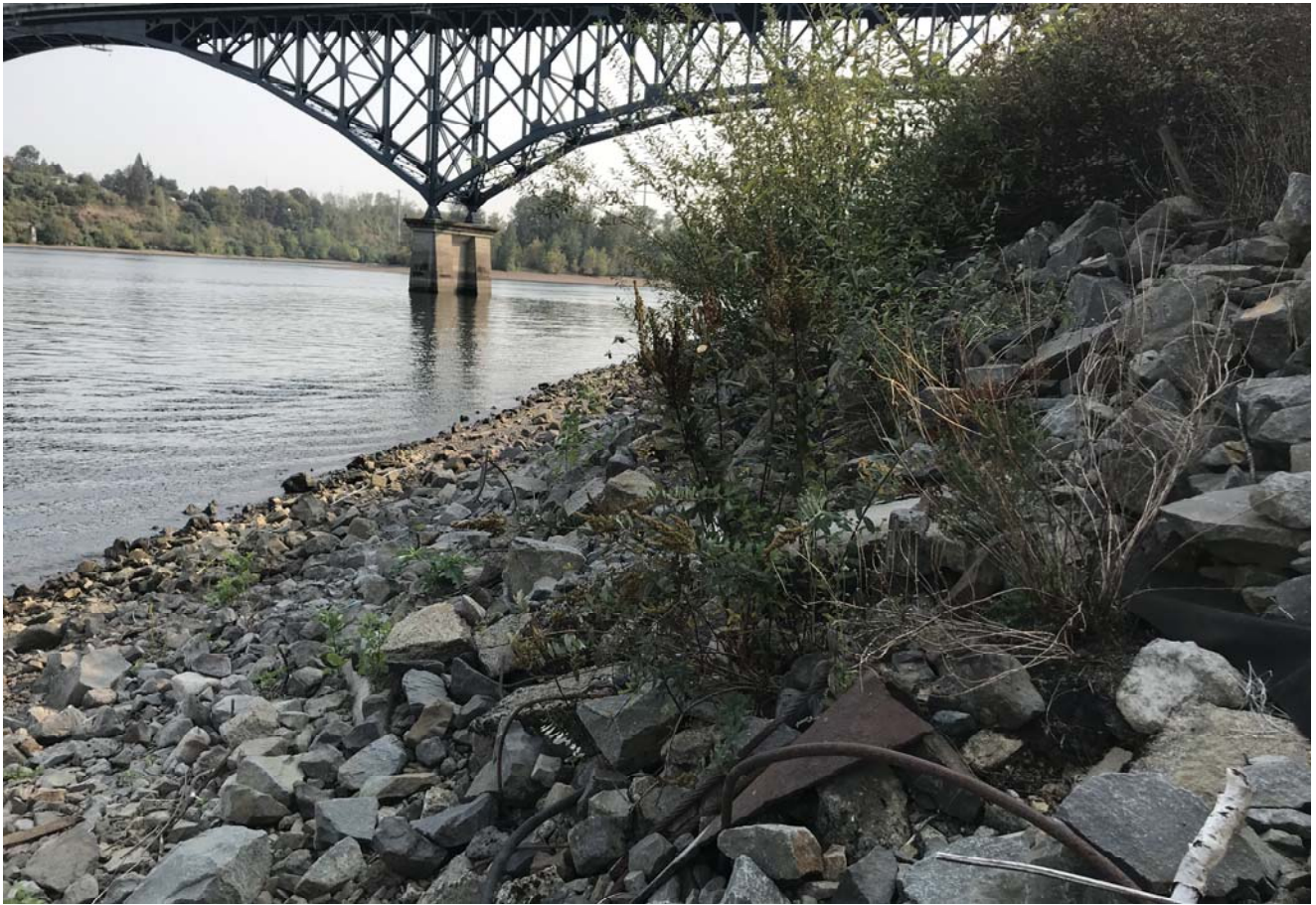
STA: 11+00 - Toe of slope looking upstream
