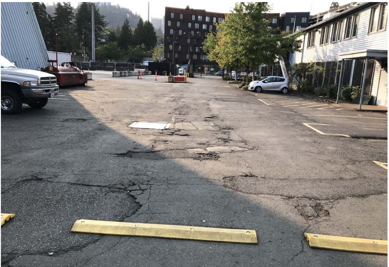
Operation area - Access road between office building and barge building
