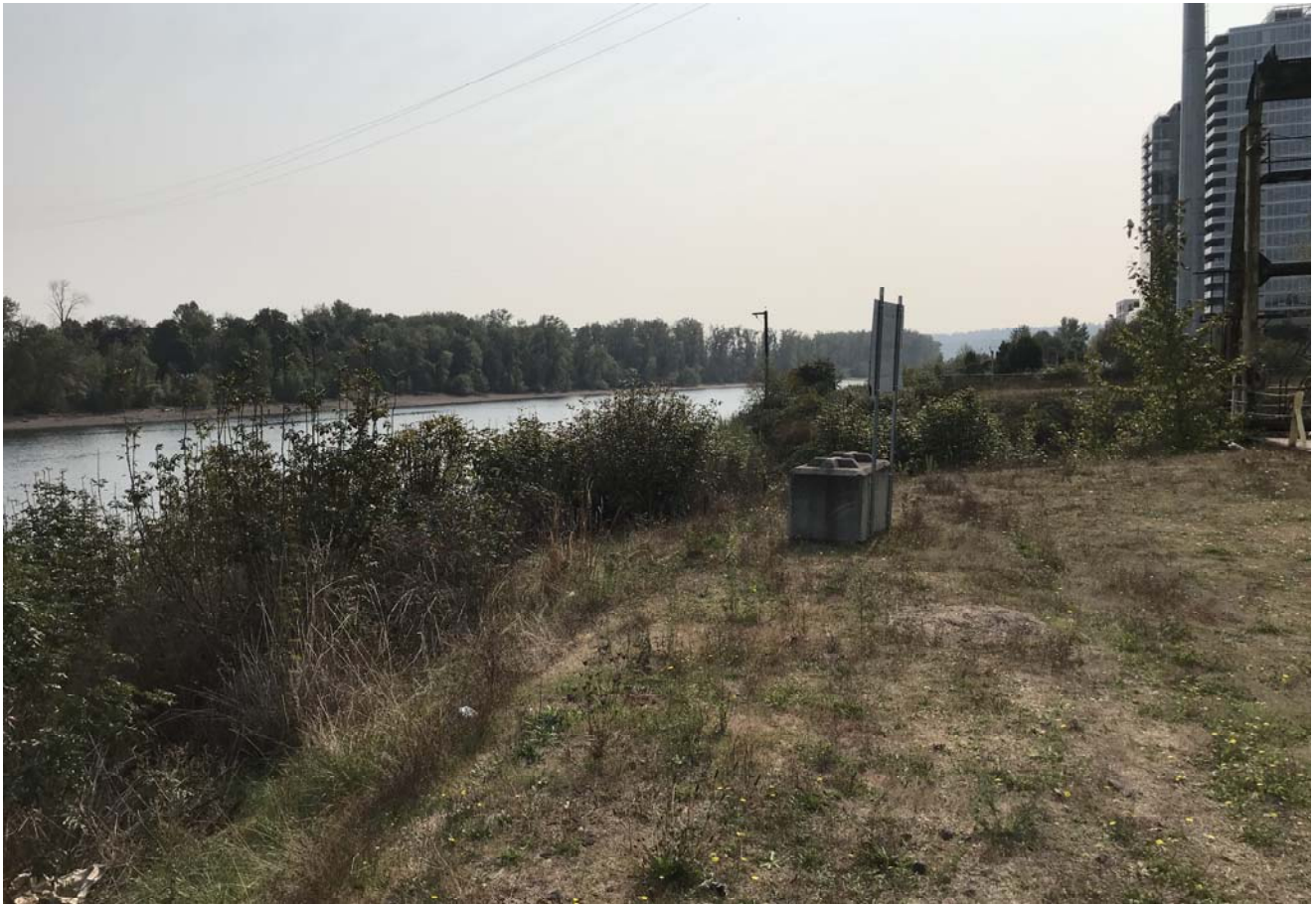
STA: 3+00 - Top of bank looking upstream
