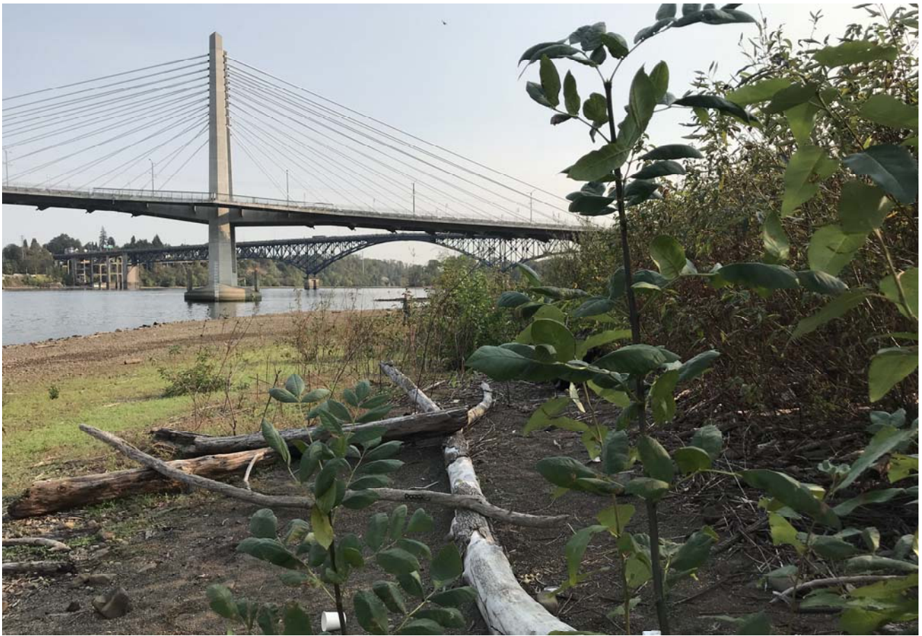
STA: 23+50 - Toe of slope looking upstream
