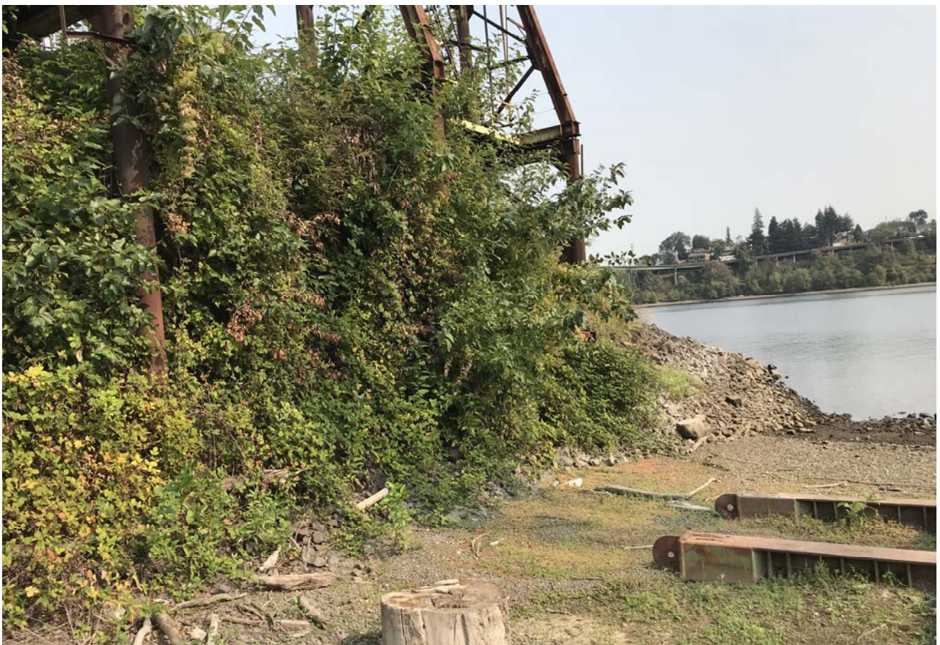
Vegetation growth on north bank of slipway, looking northeast.
