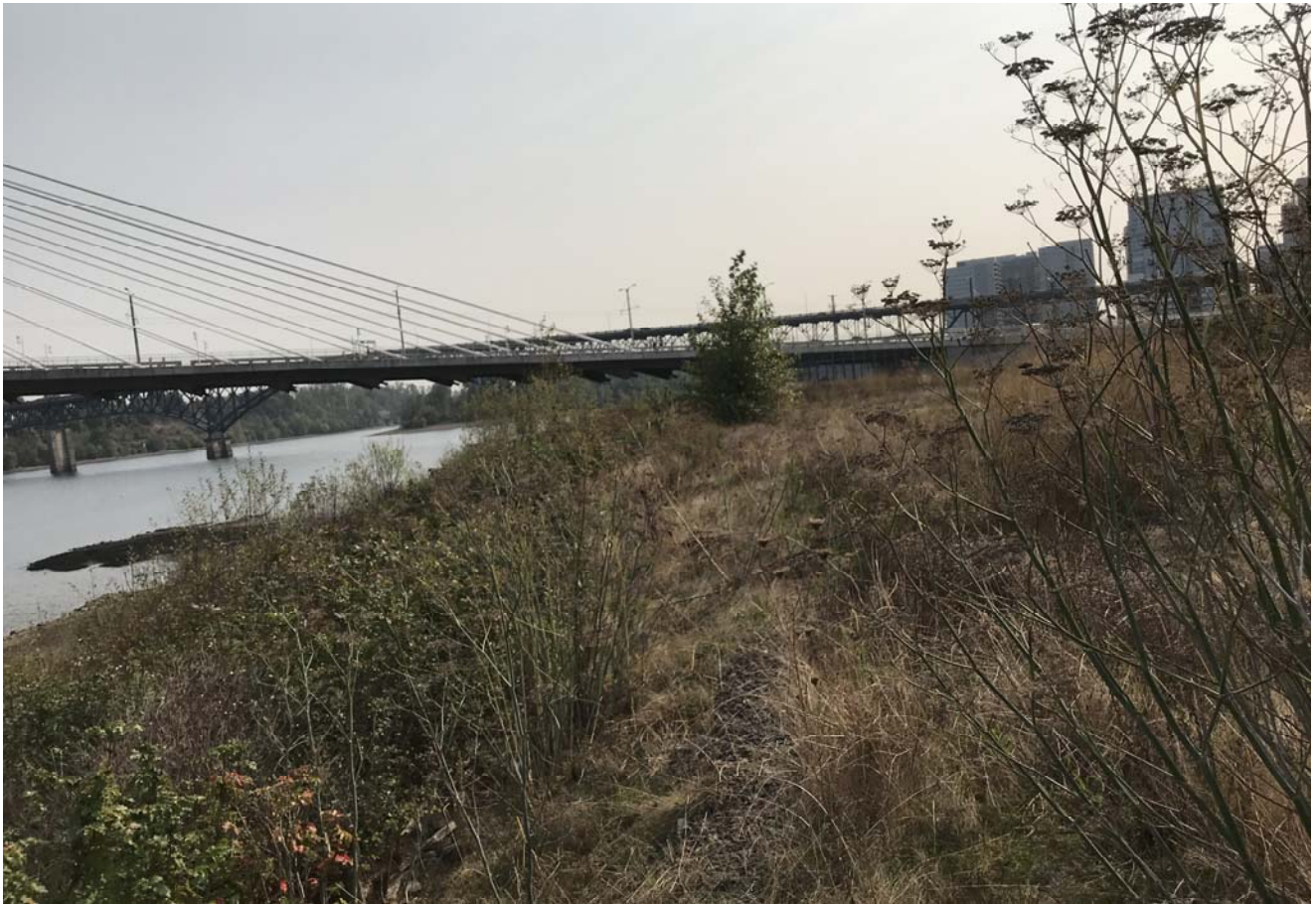
STA: 21+50 - Top of bank looking upstream
