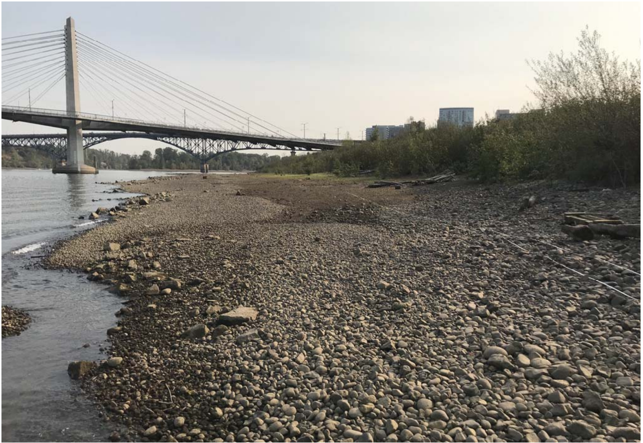
STA: 25+50 - Edge of water looking upstream
