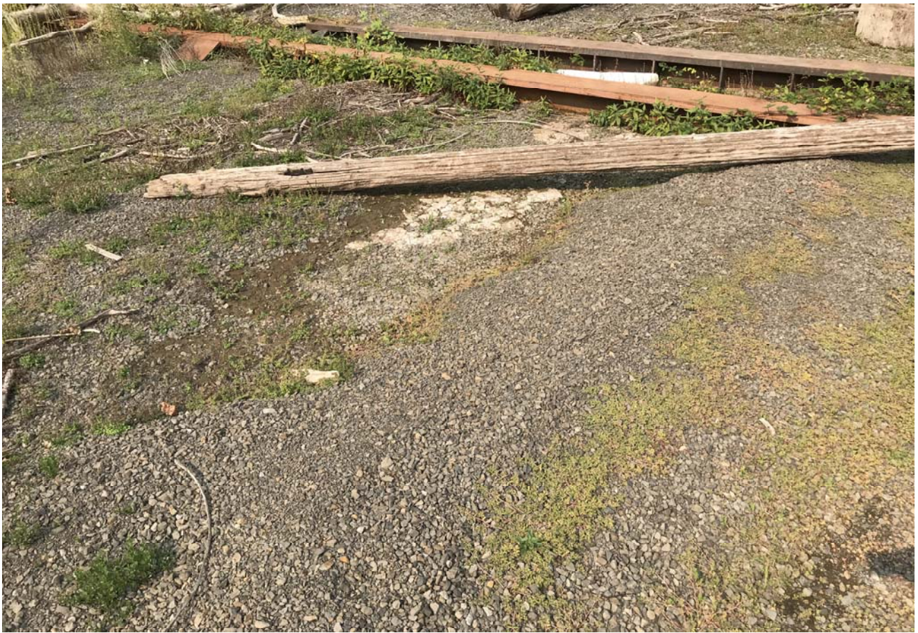
Debris and gravel shoaling in slipway
