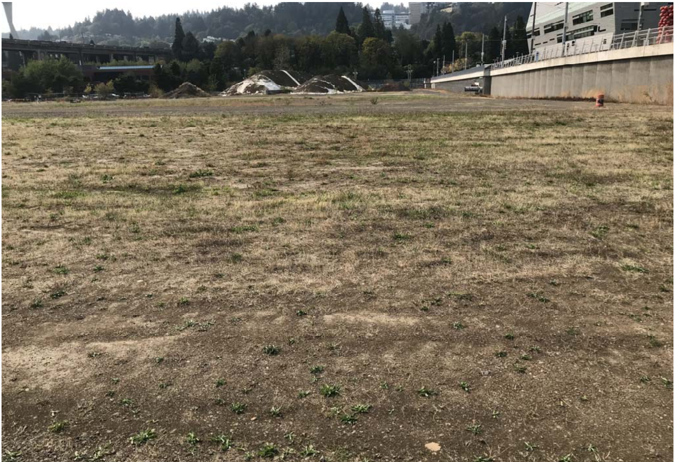
STA: 15+00 - Top of bank looking west
