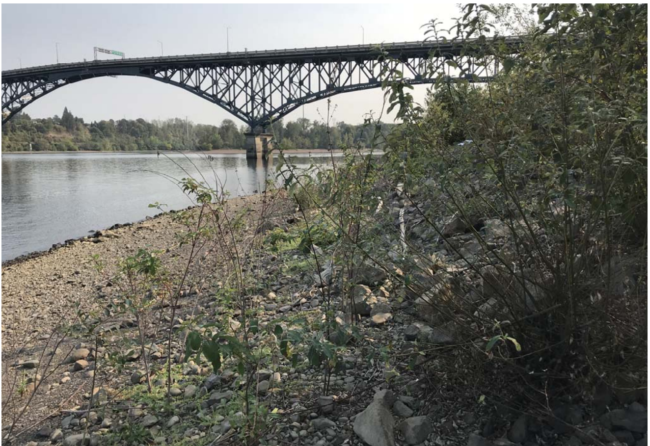
STA: 13+00 - Toe of slope looking upstream
