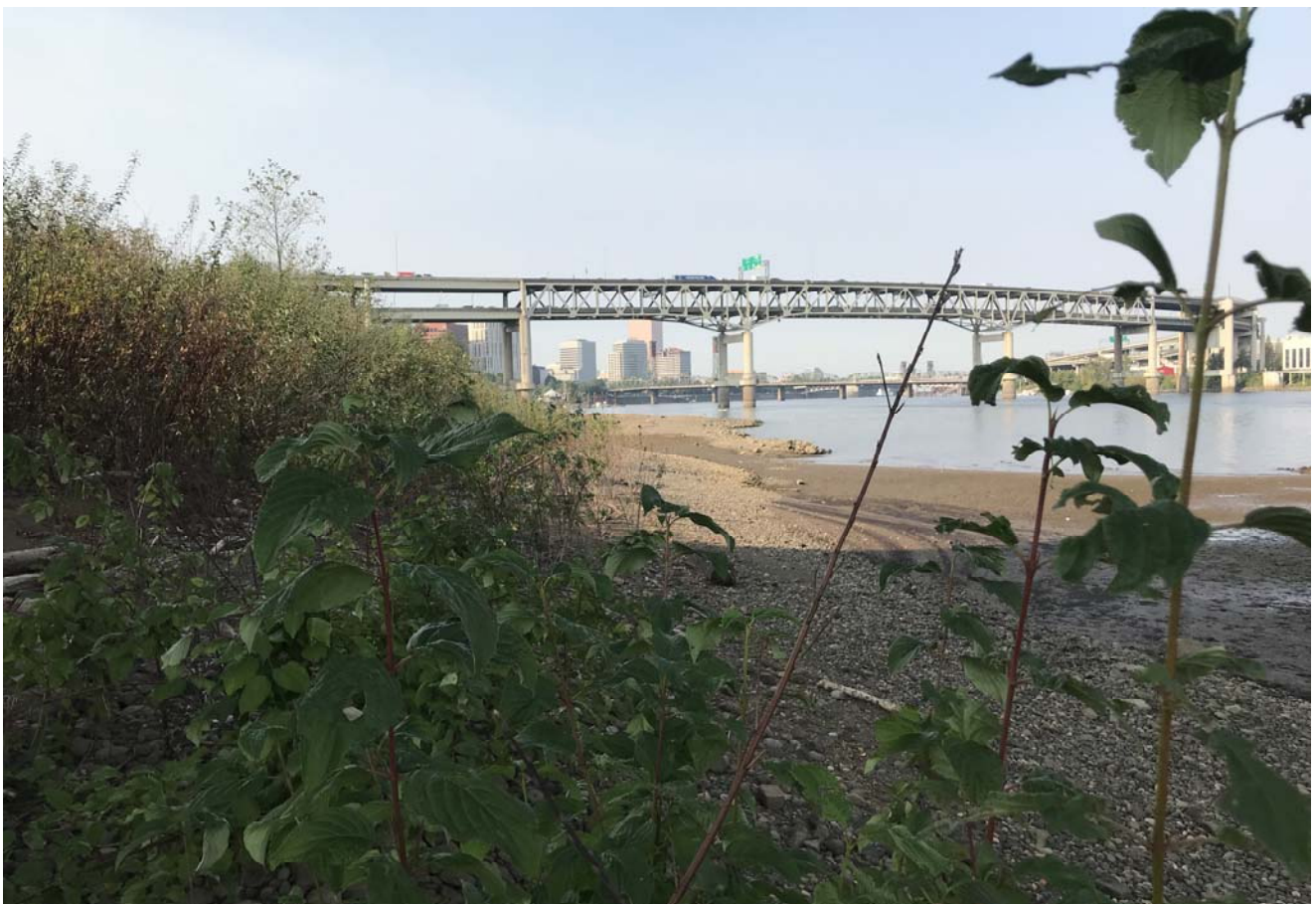
TA: 17+00 - Toe of slope looking downstream
