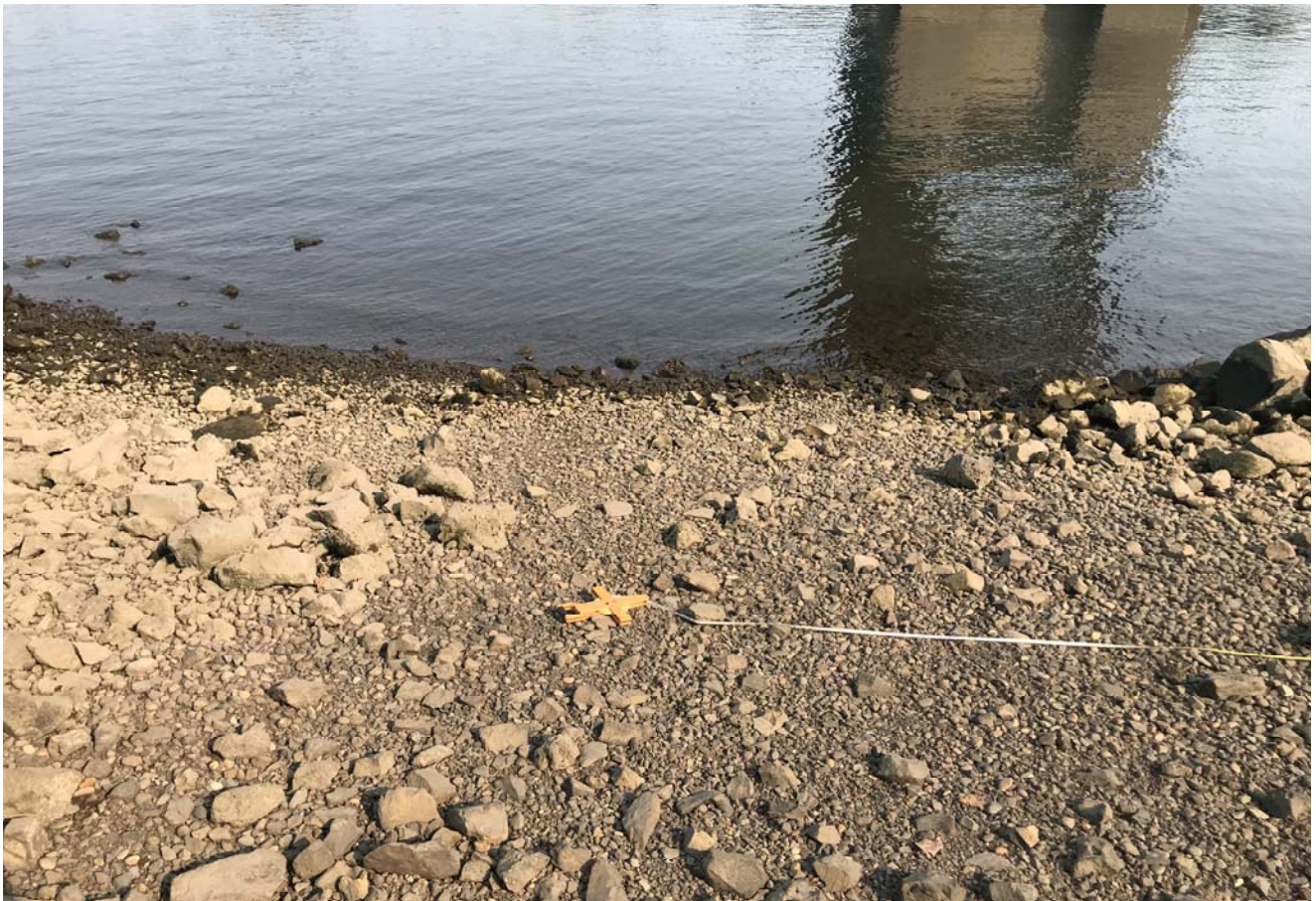
STA: 7+00 - Toe of slope looking east
