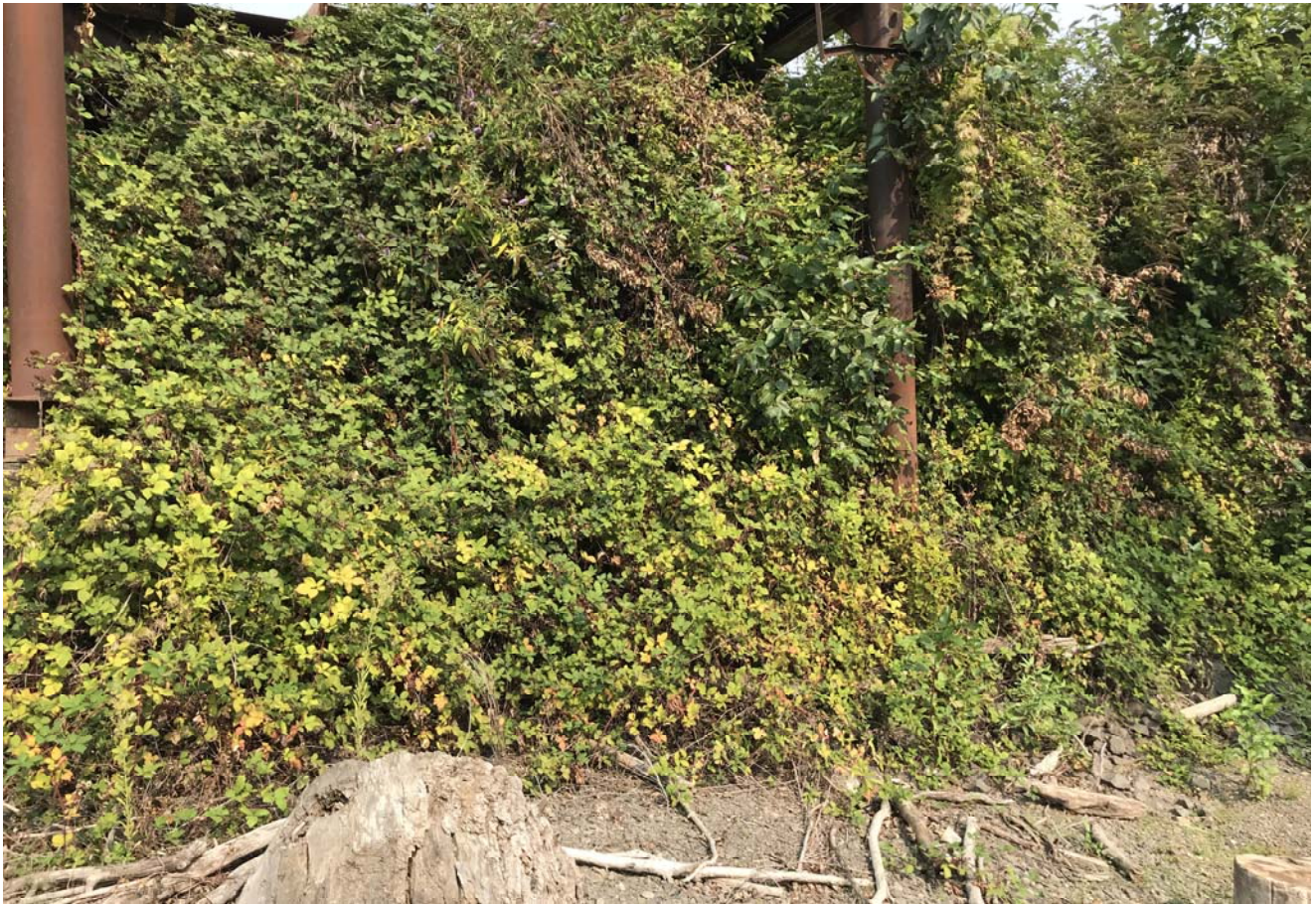
Vegetation growth on north slope of slipway
