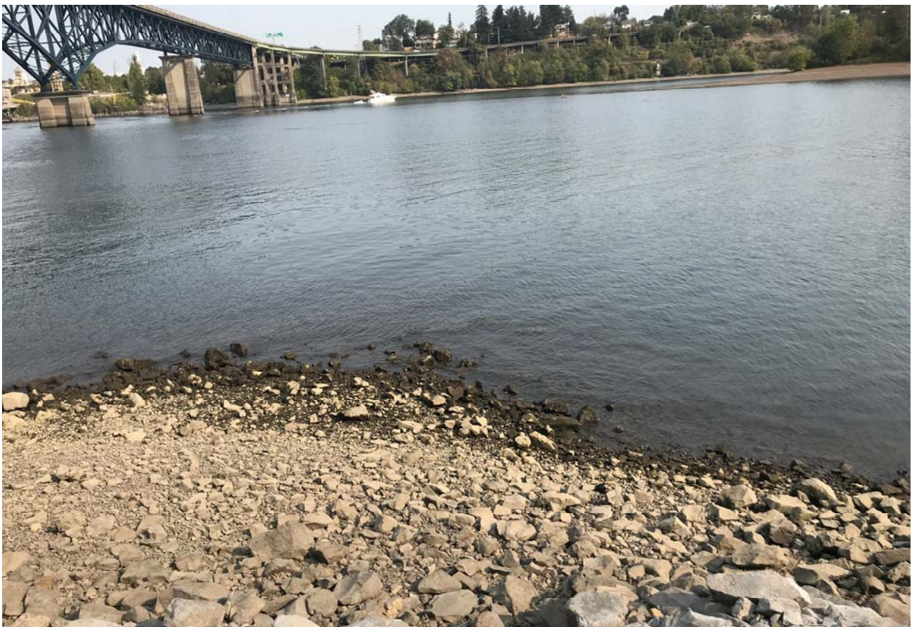
STA: 3+00 - Top of rock armor looking east
