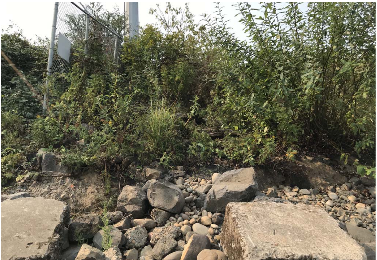
STA: 0+00 - Toe of slope looking west
