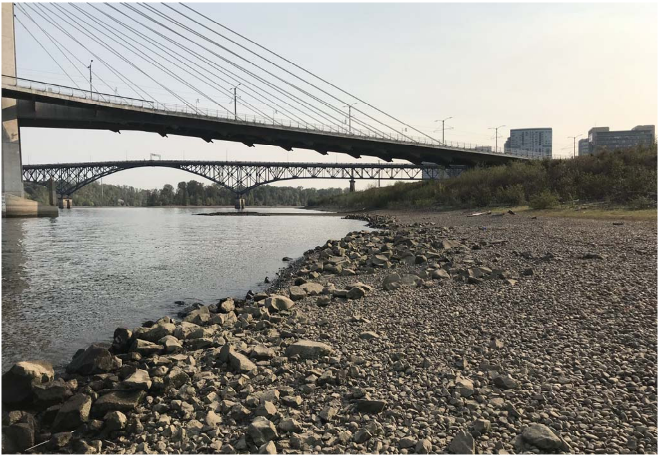
STA: 21+50 - Edge of water looking upstream
