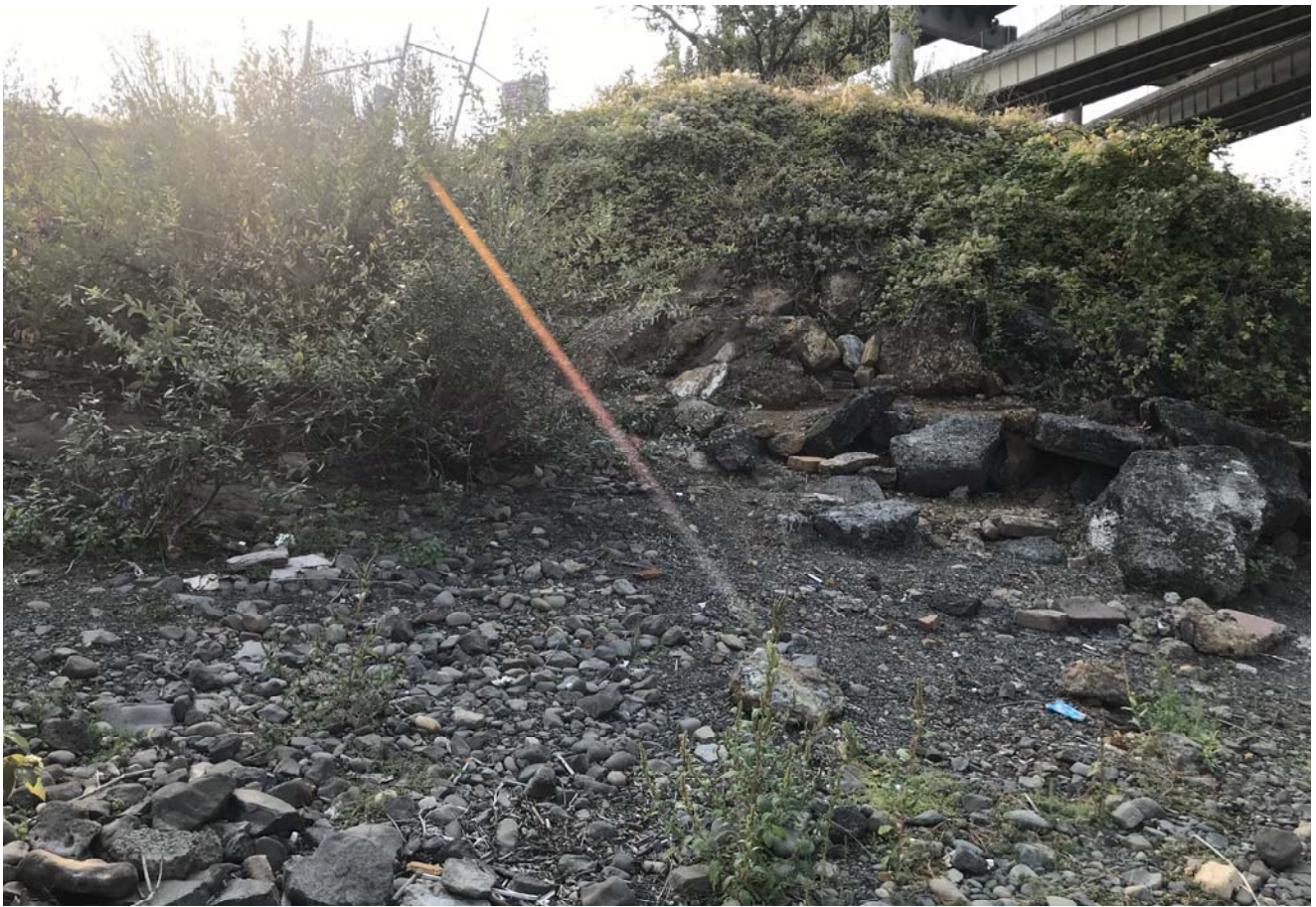
STA: 26+50 - Cap area looking west
