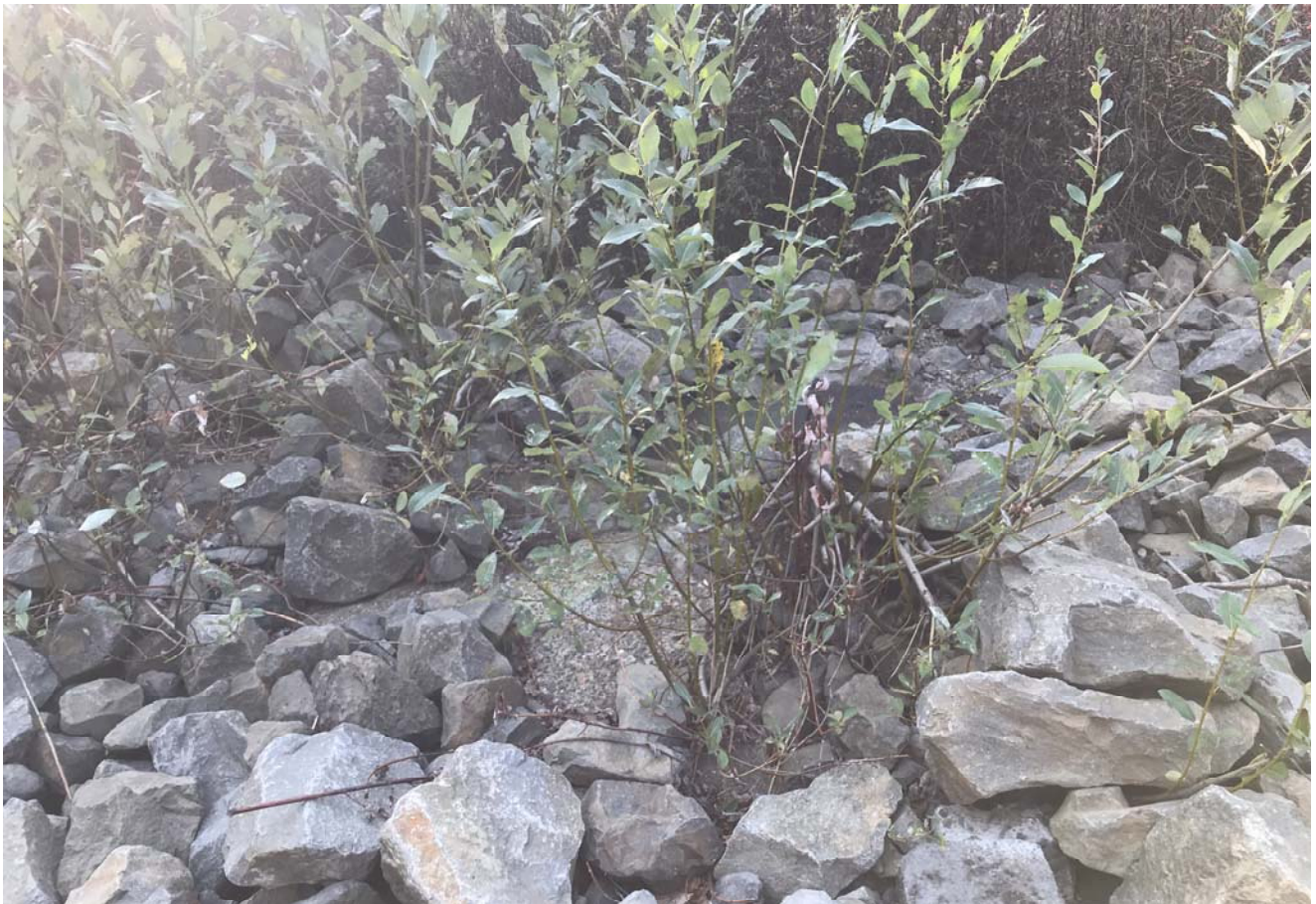
STA: 9+00 - Toe of slope looking west
