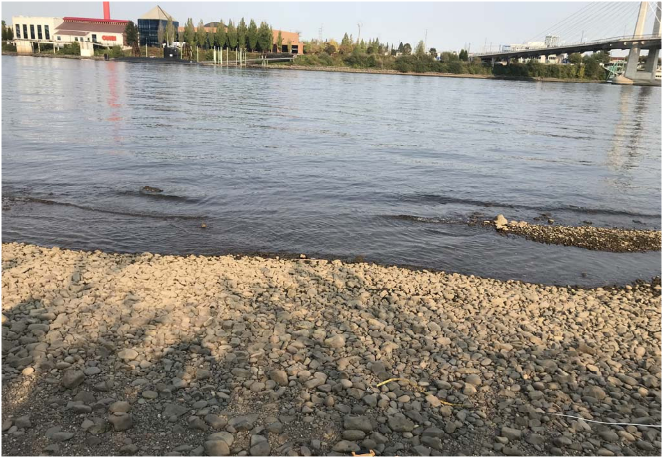
STA: 25+50 - Toe of slope looking east
