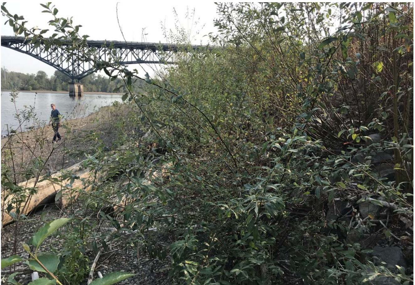
STA: 15+00 - Toe of slope looking upstream
