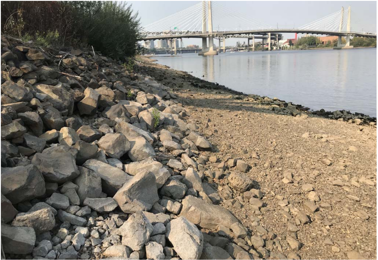
STA: 7+00 - Toe of slope looking downstream
