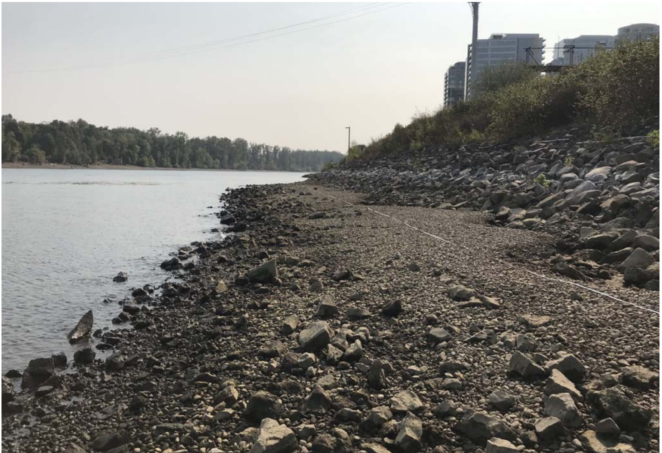
STA: 5+00 - Edge of water looking upstream
