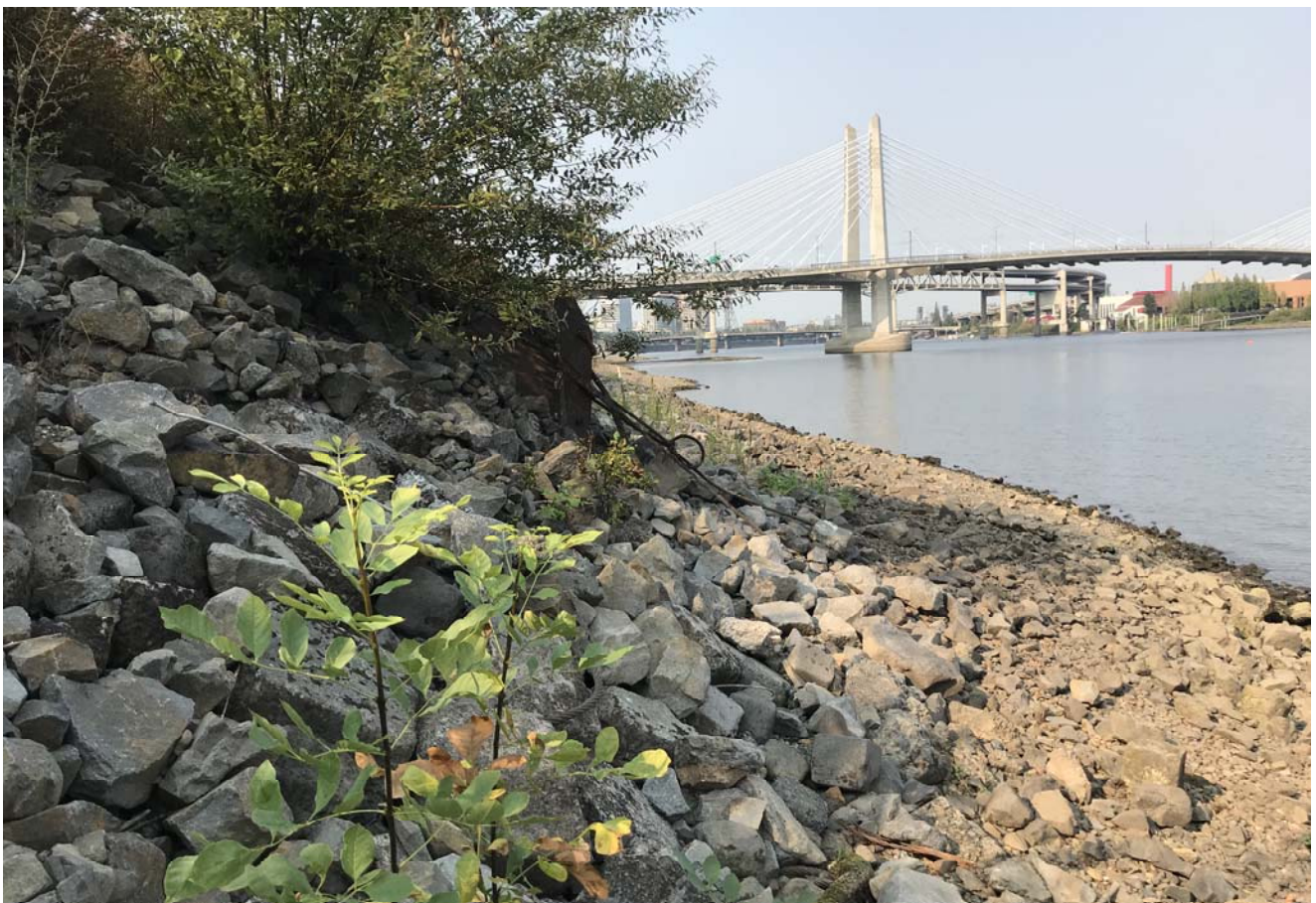
STA: 9+00 - Toe of slope looking downstream
