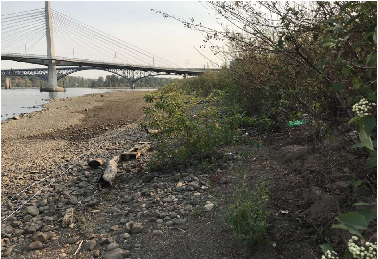
STA: 25+50 - Toe of slope looking upstream
