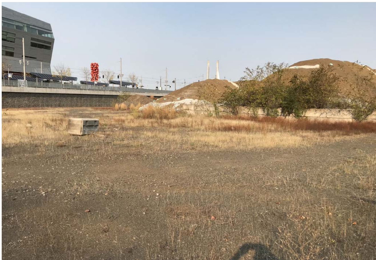
Upland cap - North edge looking northeast
