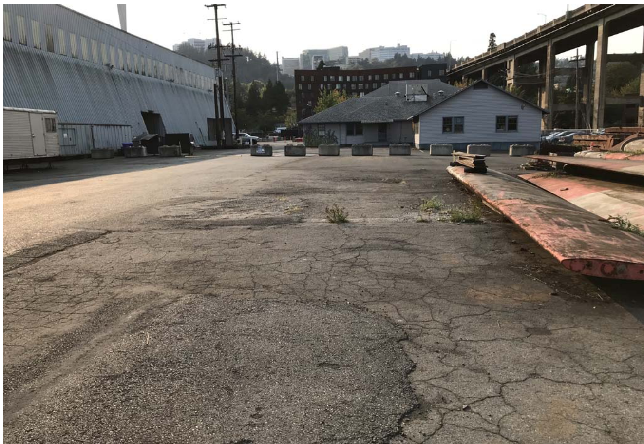
Operational area - Southeast of stormwater pond looking west
