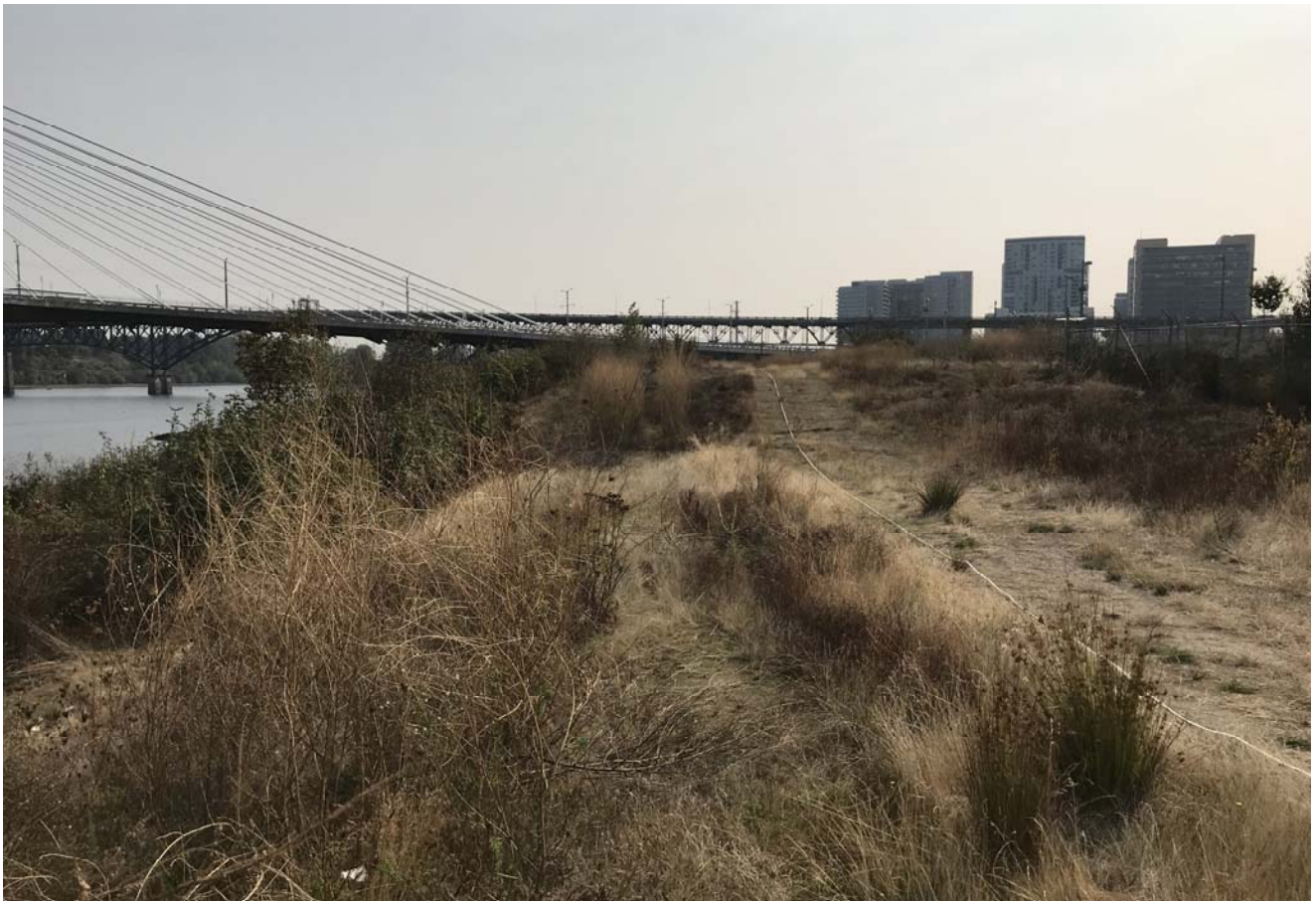
STA: 23+50 - Top of bank looking upstream
