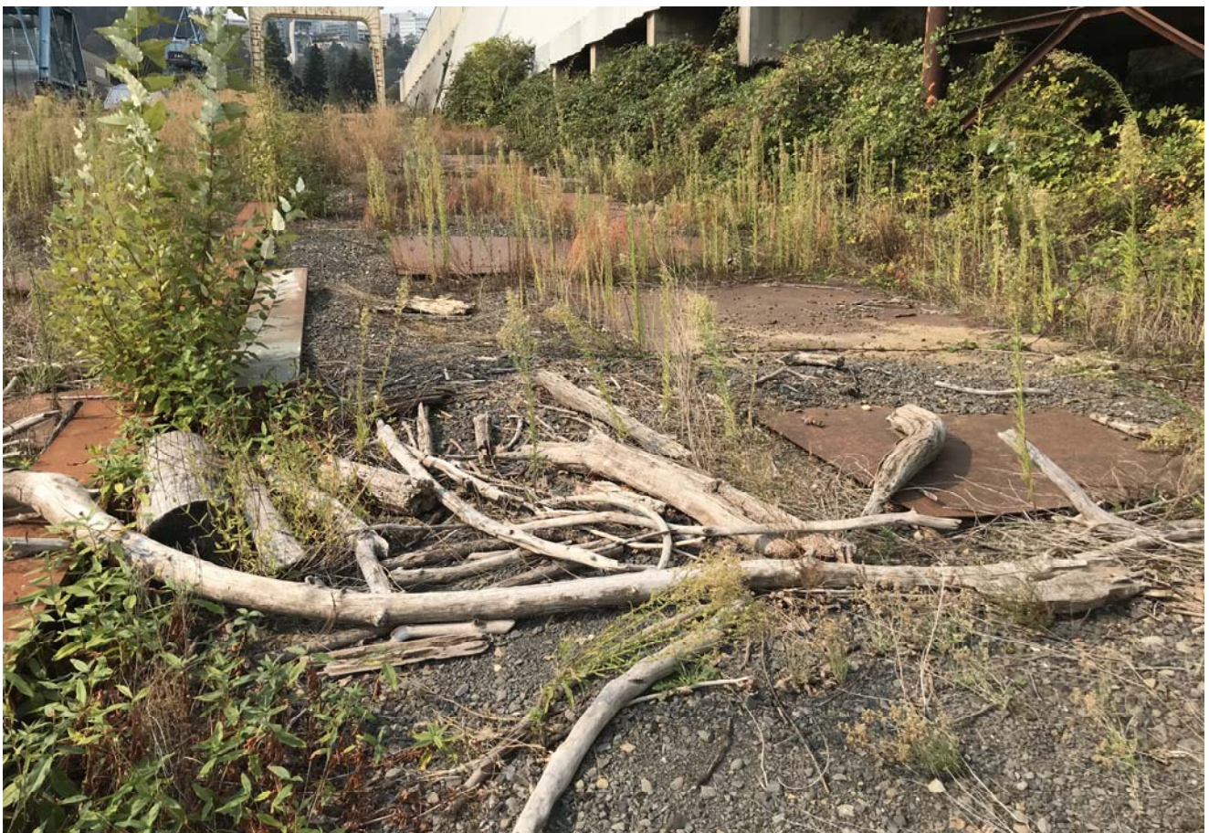
Debris buildup and vegetation growth in the slipway
