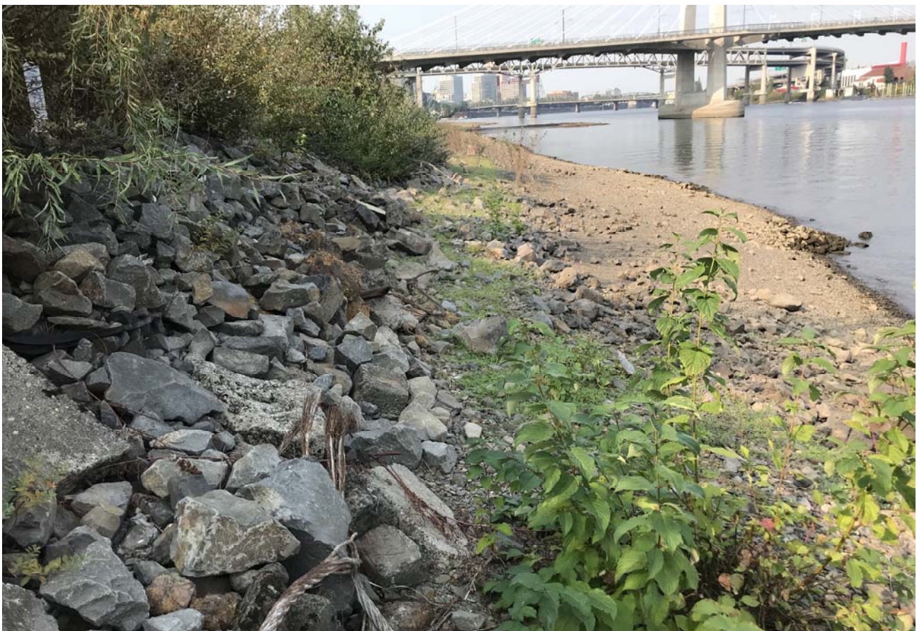
STA: 11+00 - Toe of slope looking downstream
