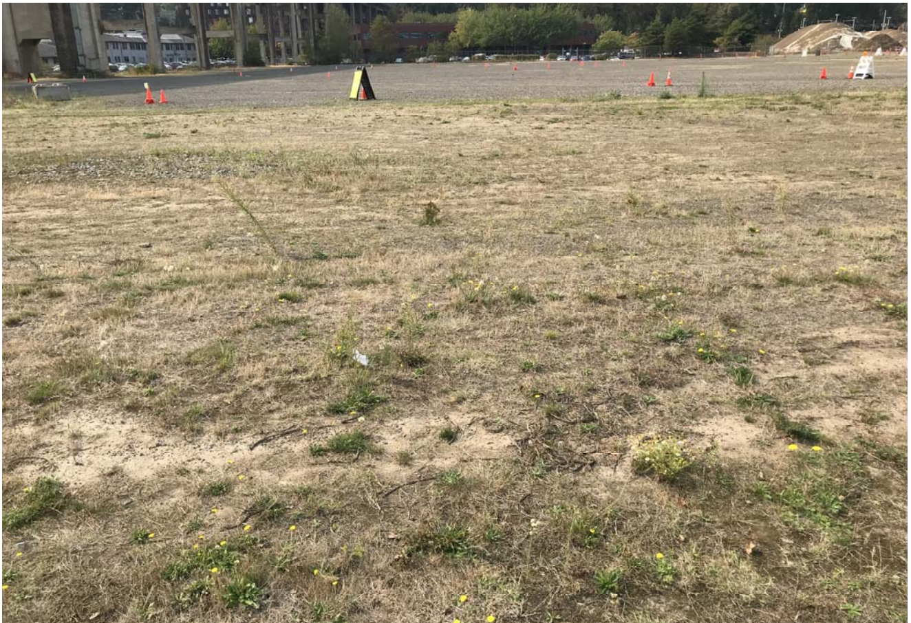
STA: 9+00 - Top of bank looking west
