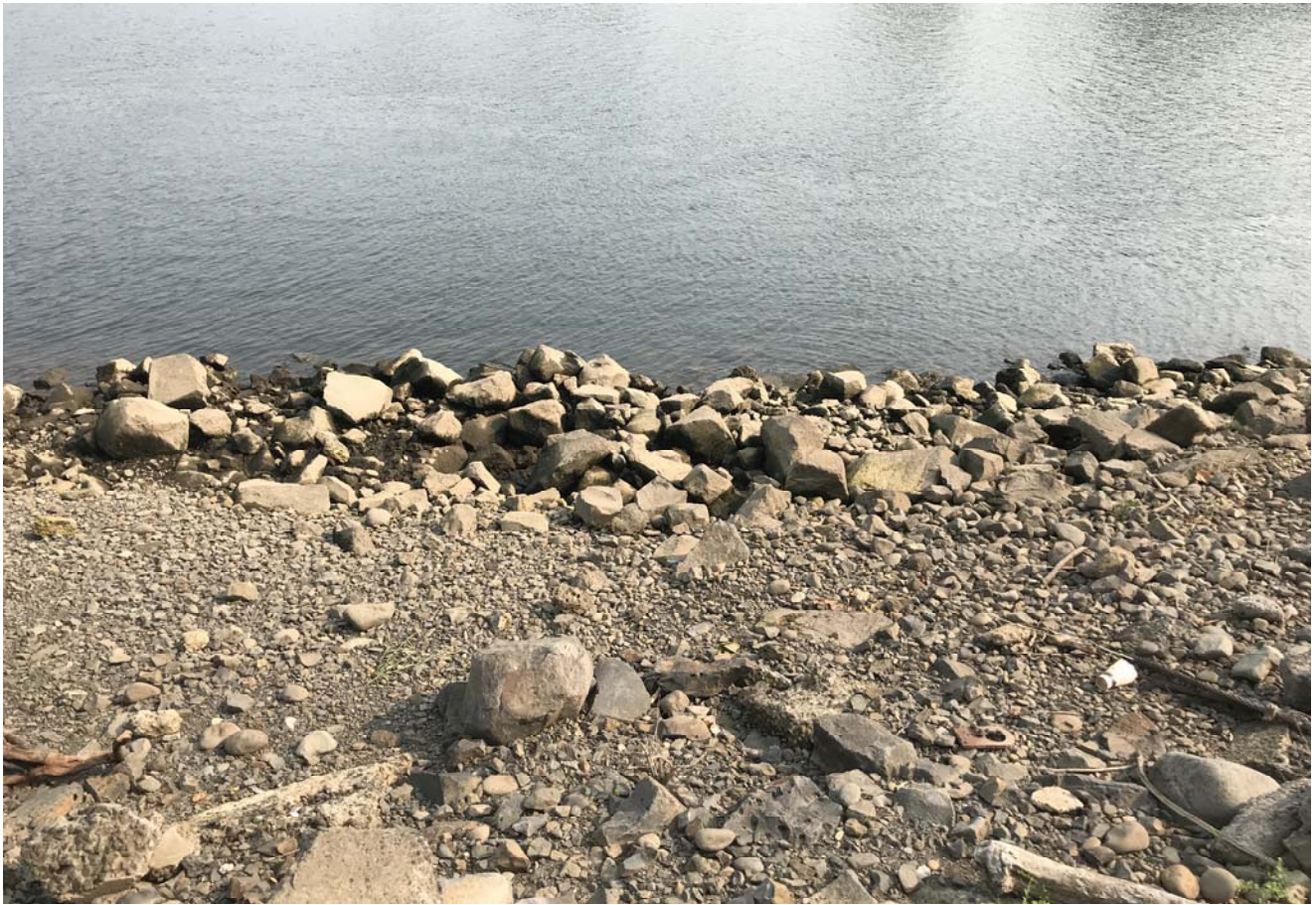
STA: 0+00 - Top of rock armor looking east
