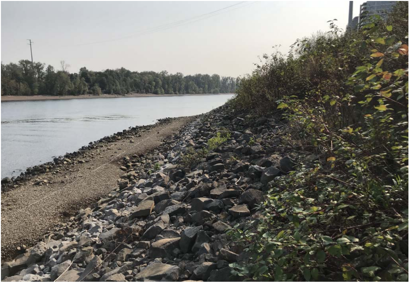
STA: 5+00 - Top of rock armor looking upstream
