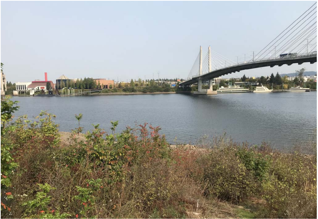
STA: 19+50 - Top of bank looking east
