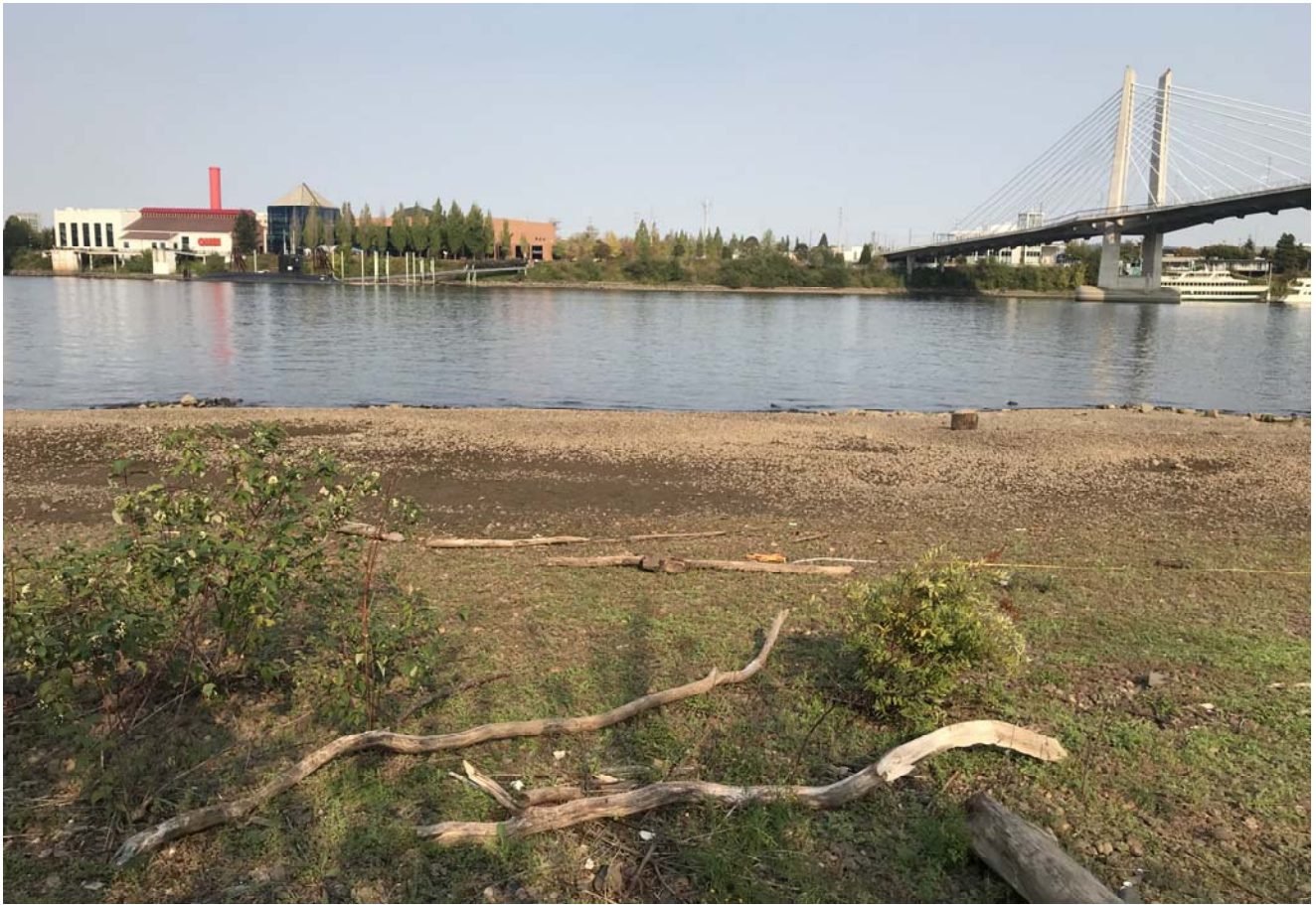
STA: 23+50 - Toe of slope looking east
