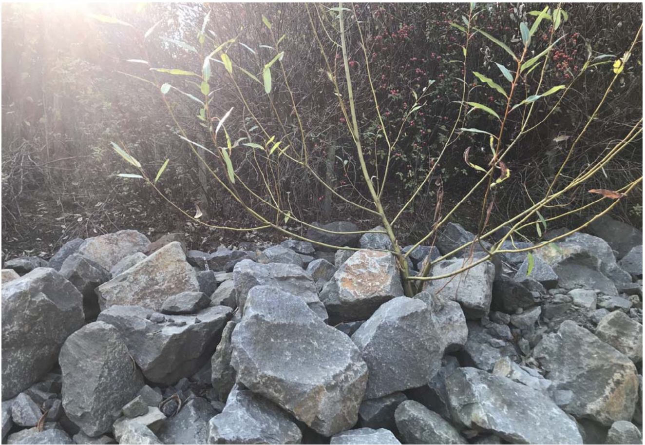
STA: 11+00 - Toe of slope looking west
