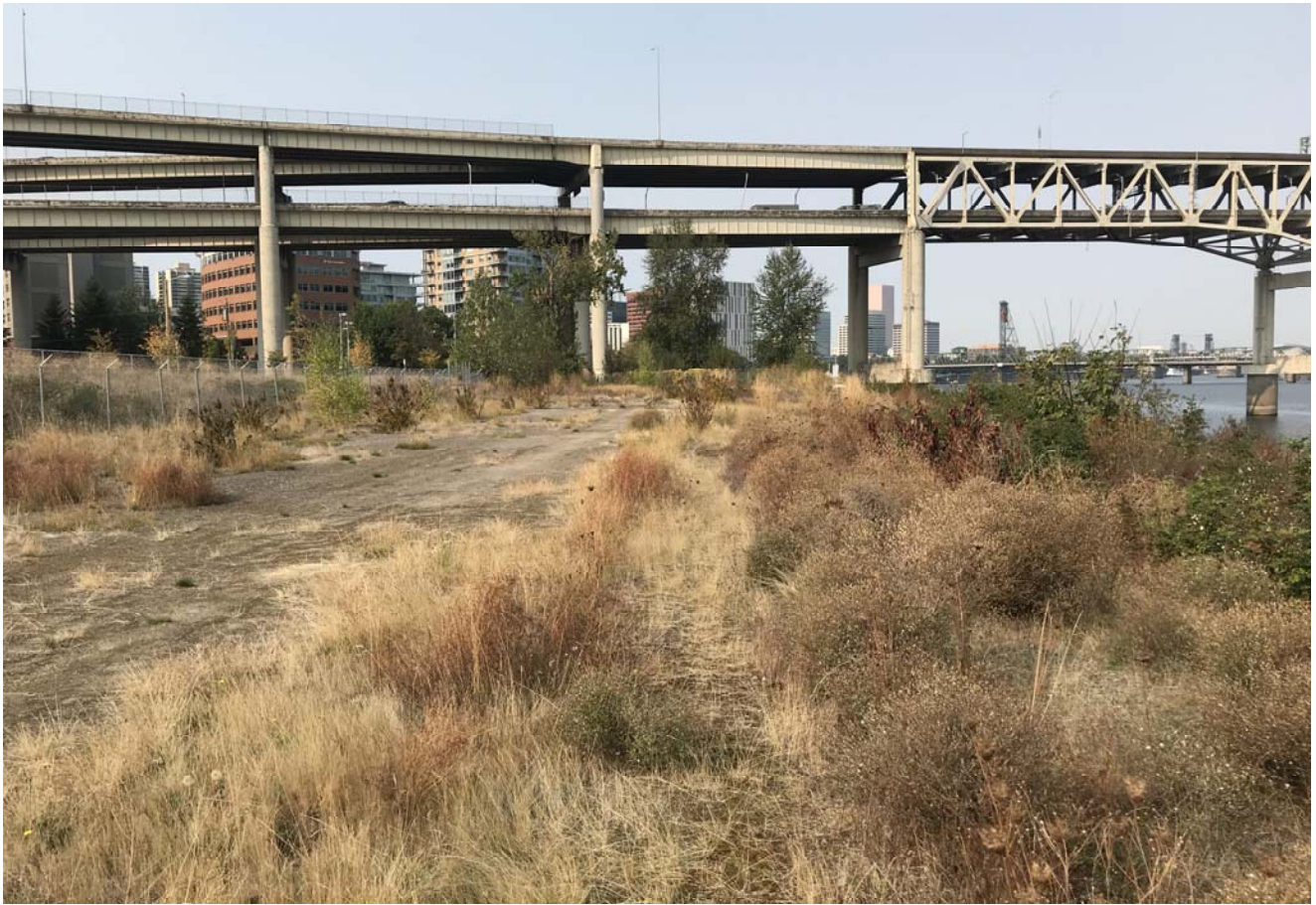
STA: 23+50 - Top of bank looking downstream
