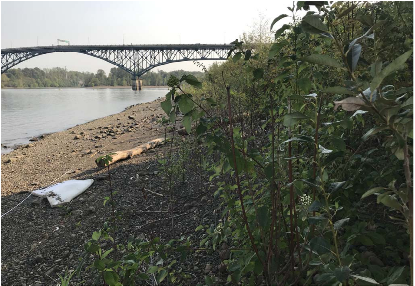
STA: 17+00 - Toe of slope looking upstream
