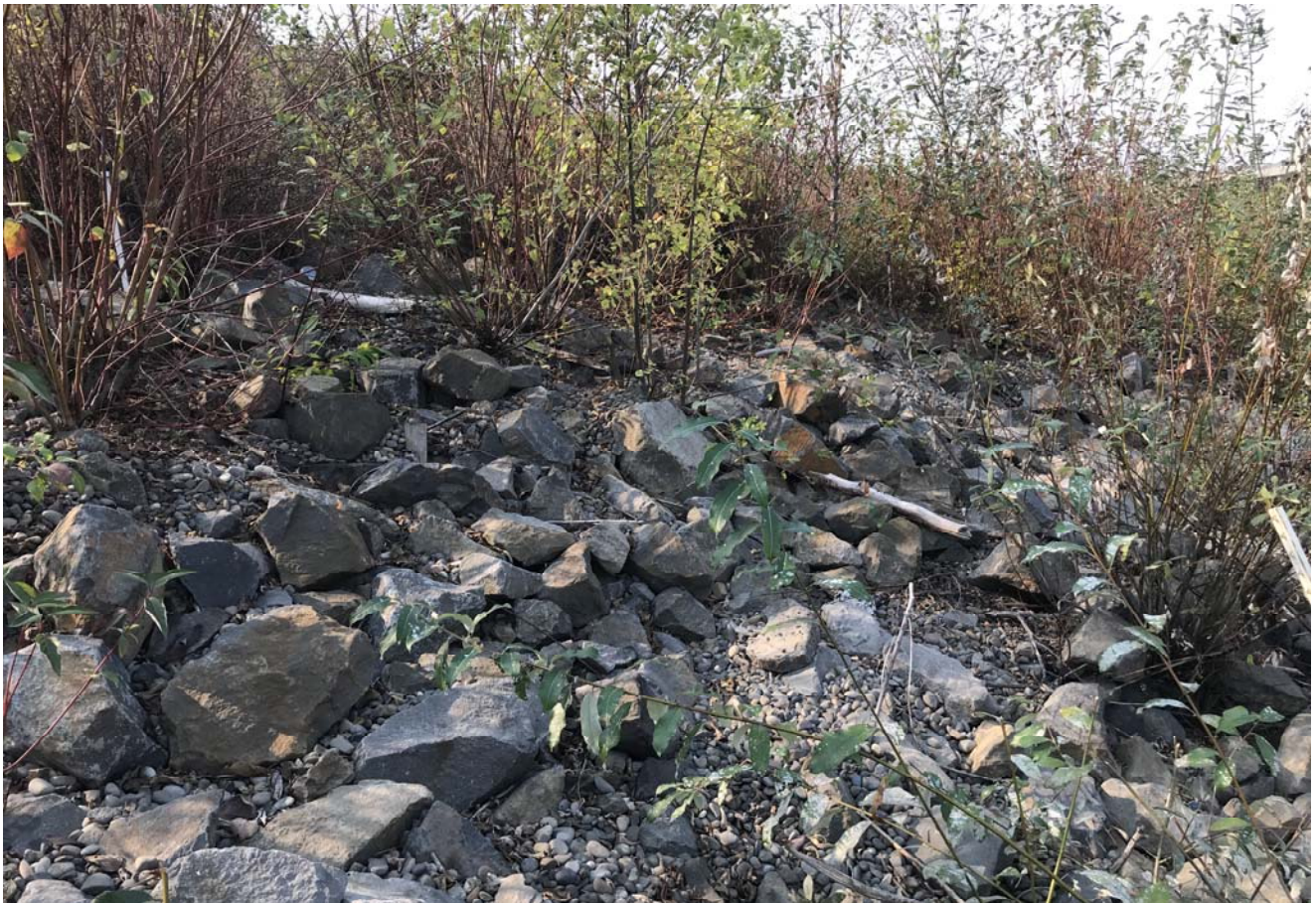
STA: 13+50 - 2018 Bank repair area
