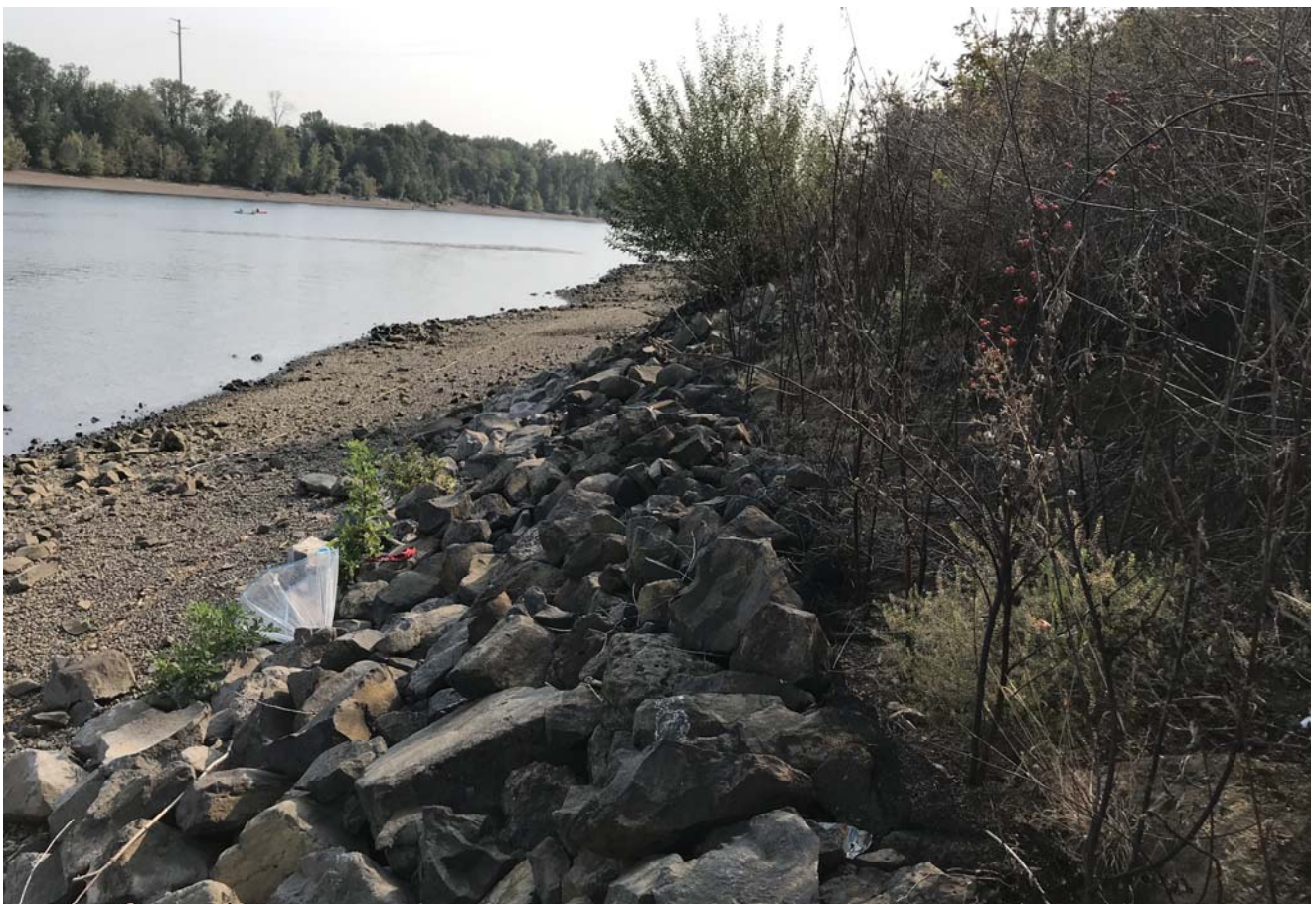
STA: 7+00 - Top of rock armor looking upstream
