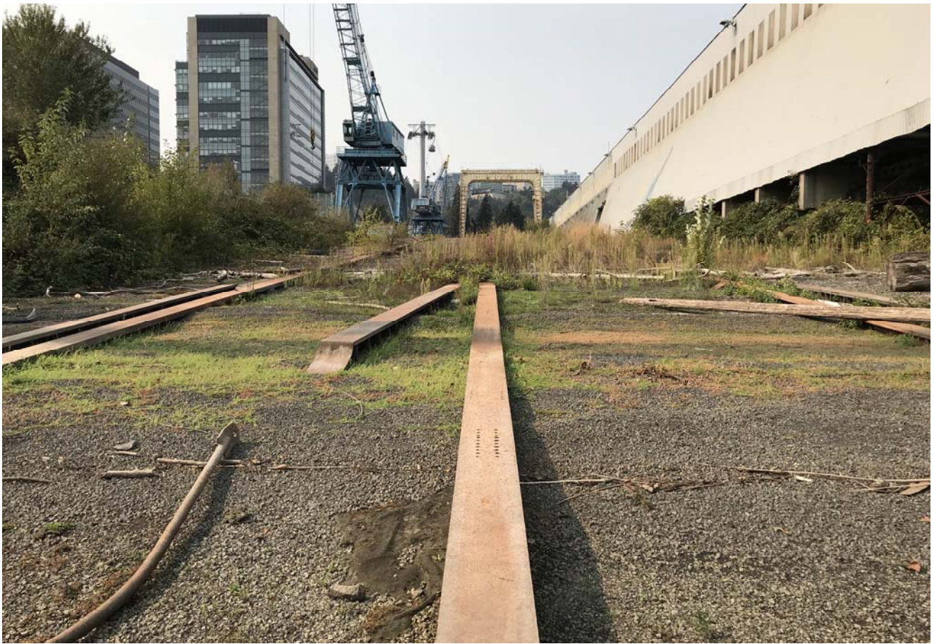
Middle slipway, looking west
