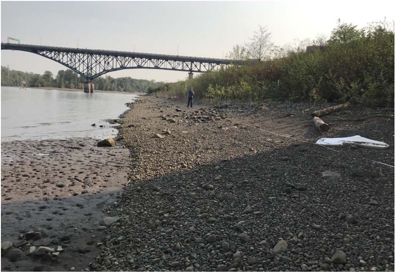
STA: 17+00 - Edge of water looking upstream
