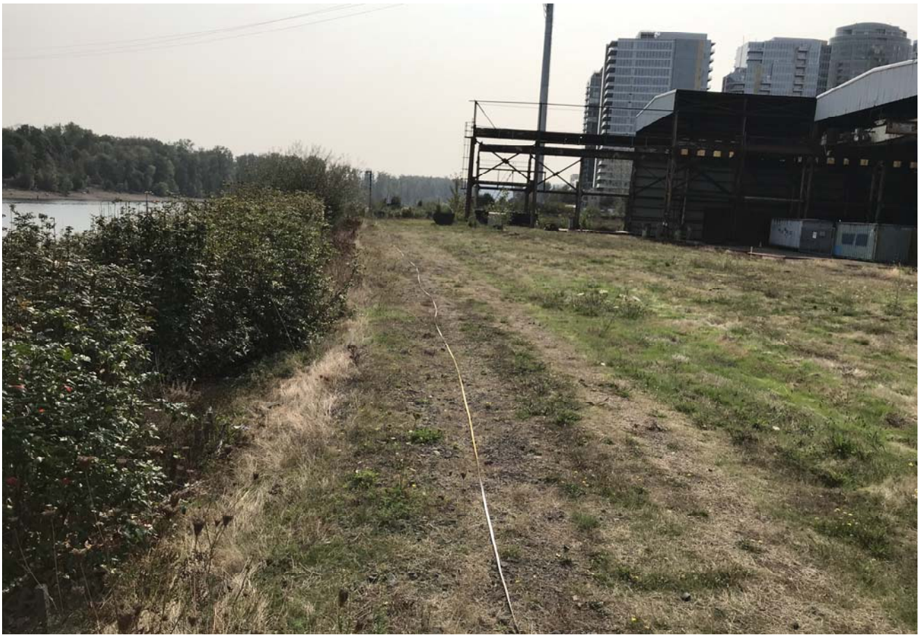
STA: 5+00 - Top of bank looking upstream
