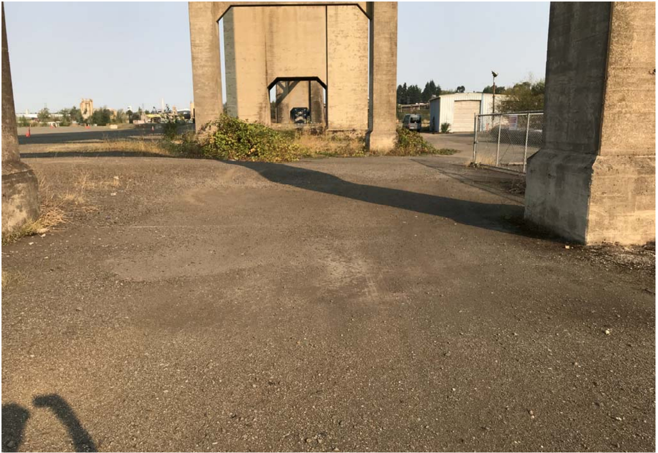
Upland cap beneath Ross Island Bridge in southeast corner
