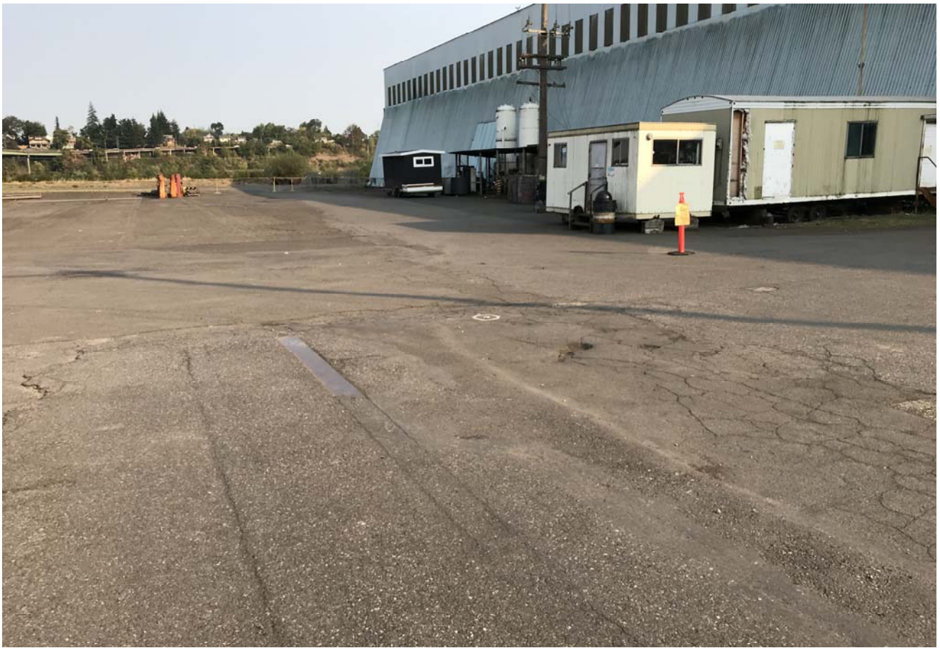
Operational area - Southeast of stormwater pond looking east
