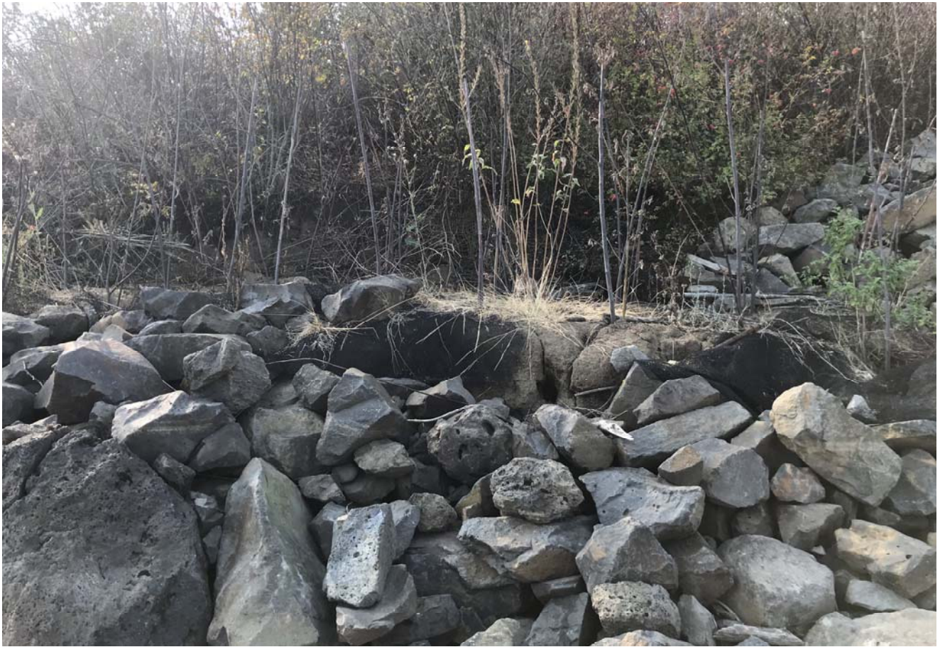
STA: 7+00 - Toe of slope looking west
