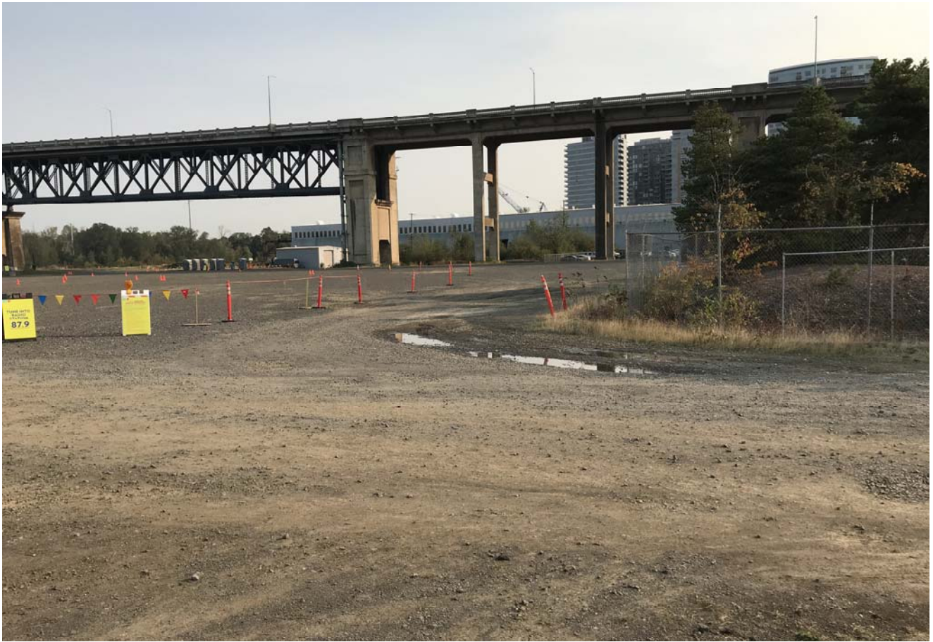
Upland cap - Access road looking southeast
