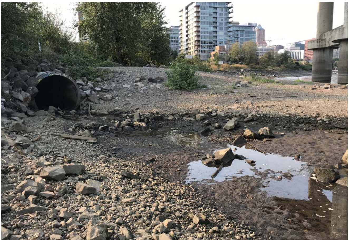
City of Portland stormwater outfall 07b, looking northwest
