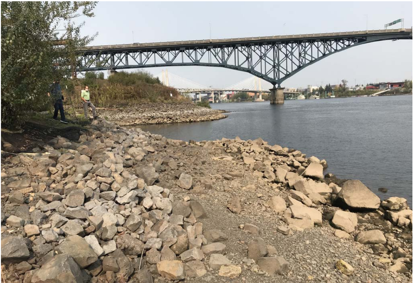
STA: 0+00 - Toe of slope looking downstream
