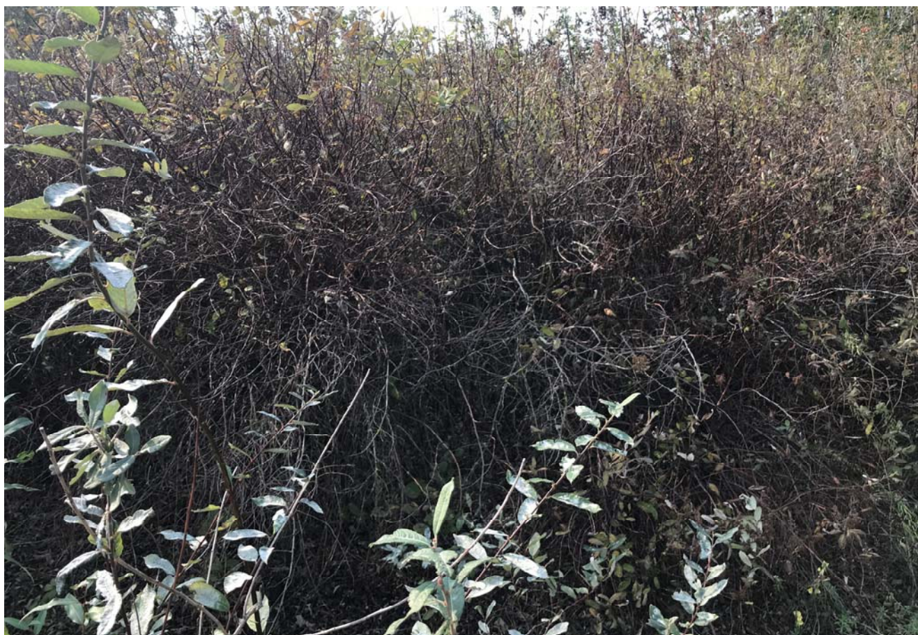
STA: 5+00 - Top of rock armor looking west
