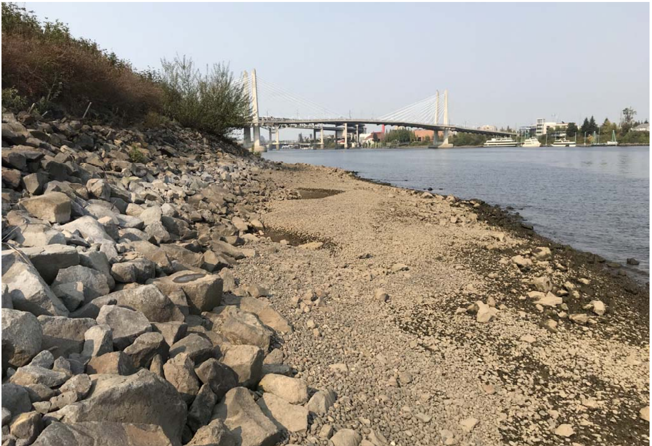
STA: 5+00 - Toe of slope looking downstream
