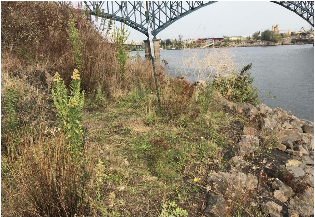
STA: 2+50 - Northeast corner of slipway at top of rock armor, looking northeast
