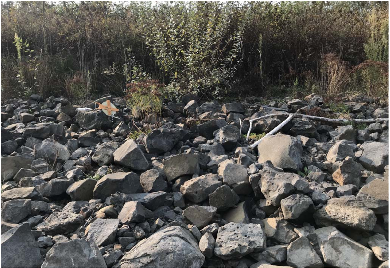
STA: 3+00 - Toe of slope looking west
