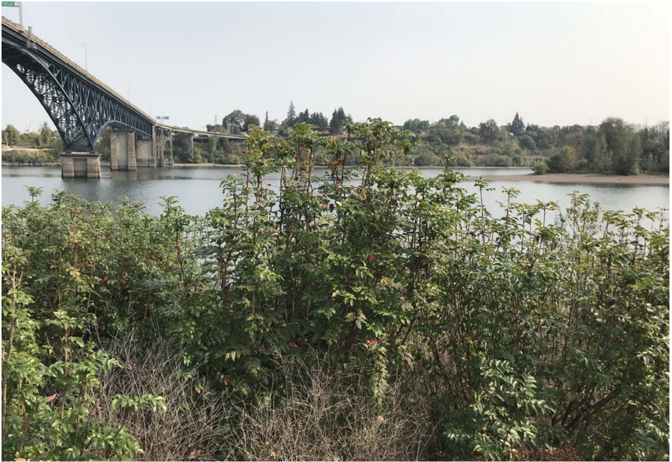
STA: 5+00 - Top of bank looking east
