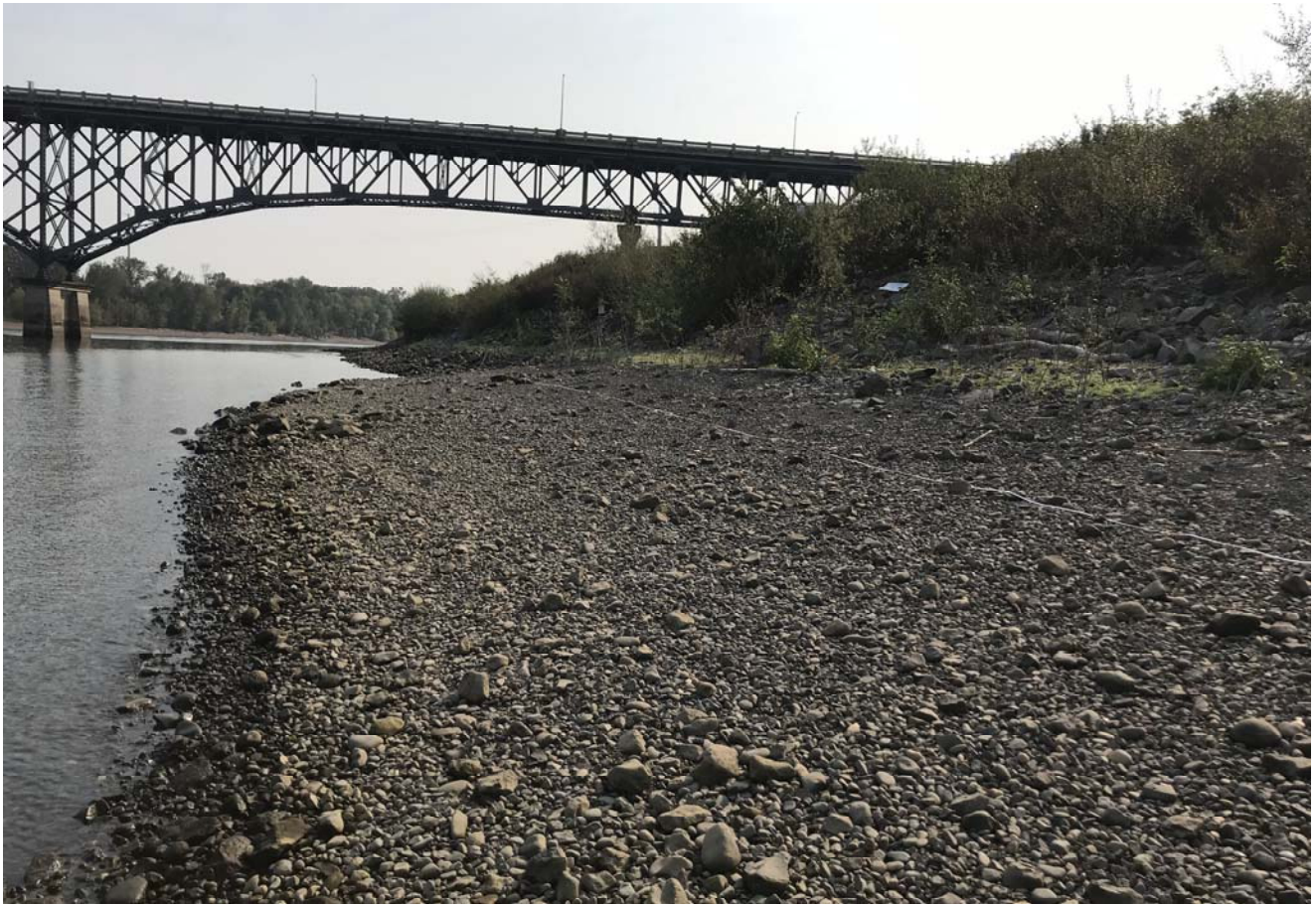
STA: 13+00 - Edge of water looking upstream
