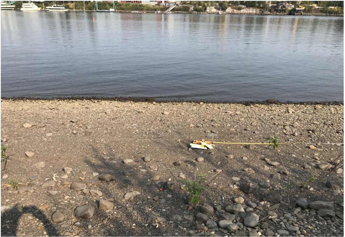
STA: 13+00 - Toe of slope looking east
