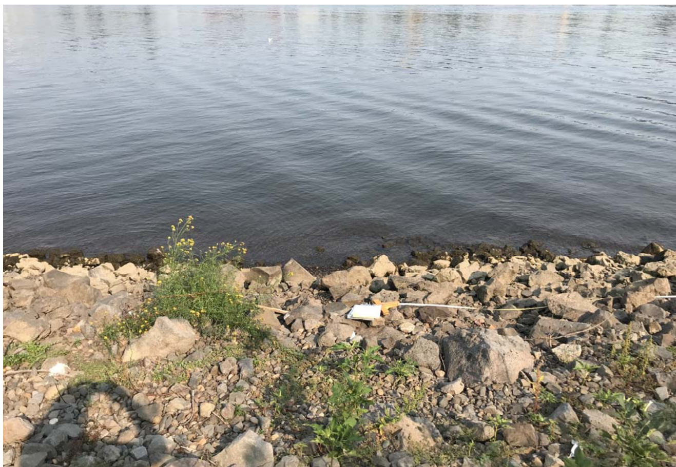
STA: 11+00 - Toe of slope looking east
