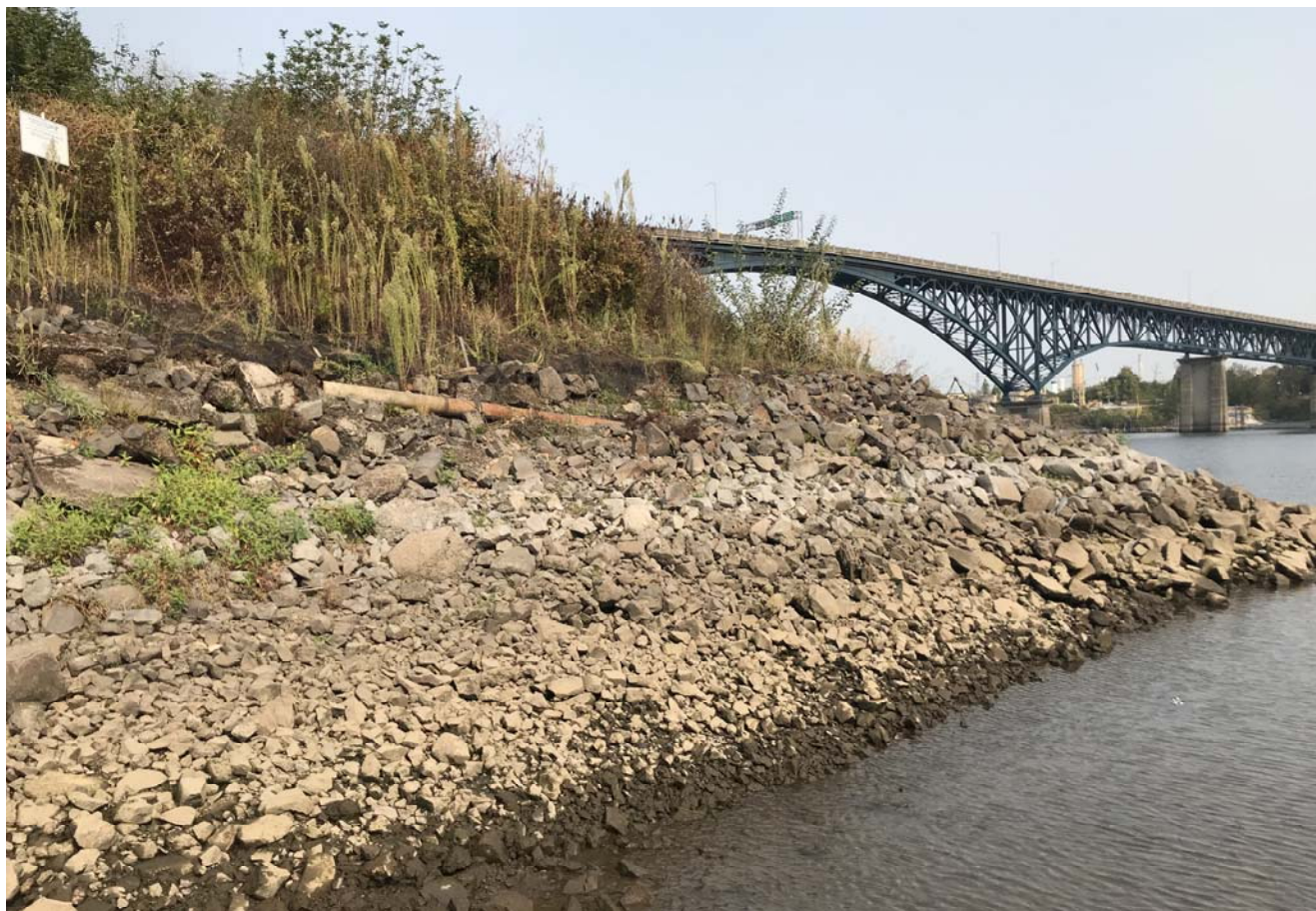
Rock armor on north bank of slipway, looking northeast
