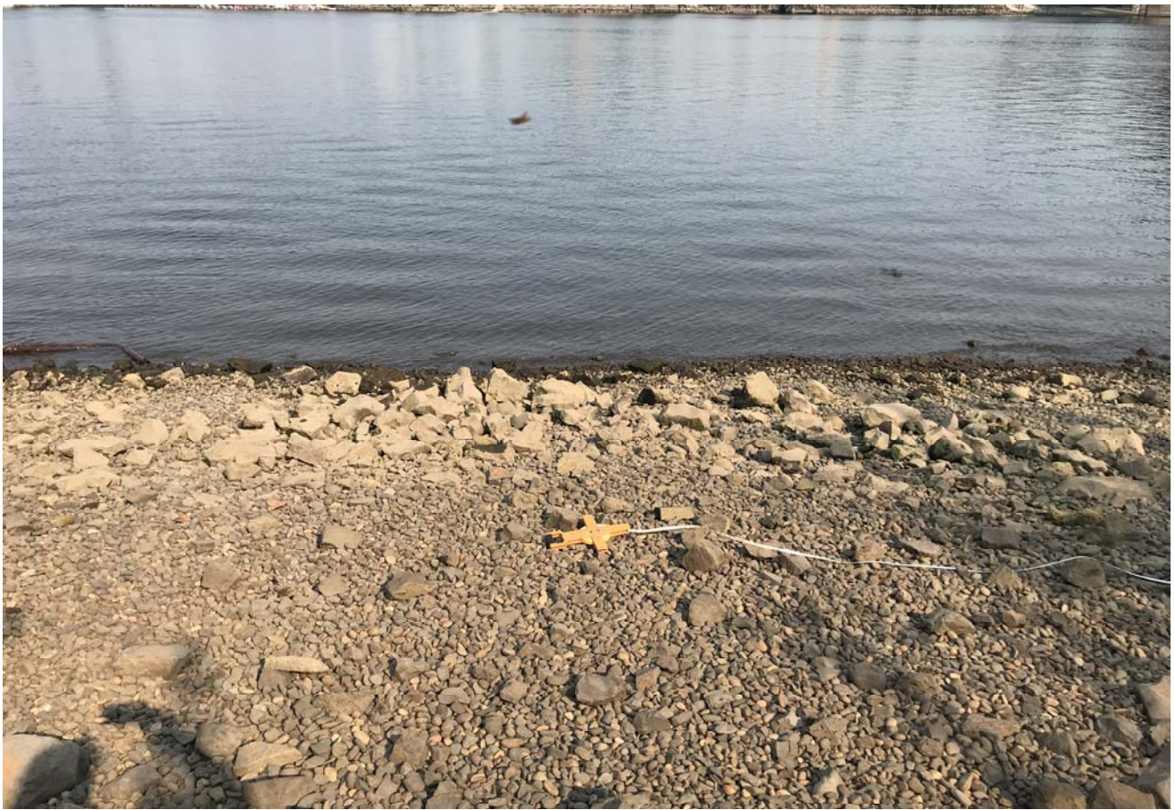
STA: 9+00 - Toe of slope looking east
