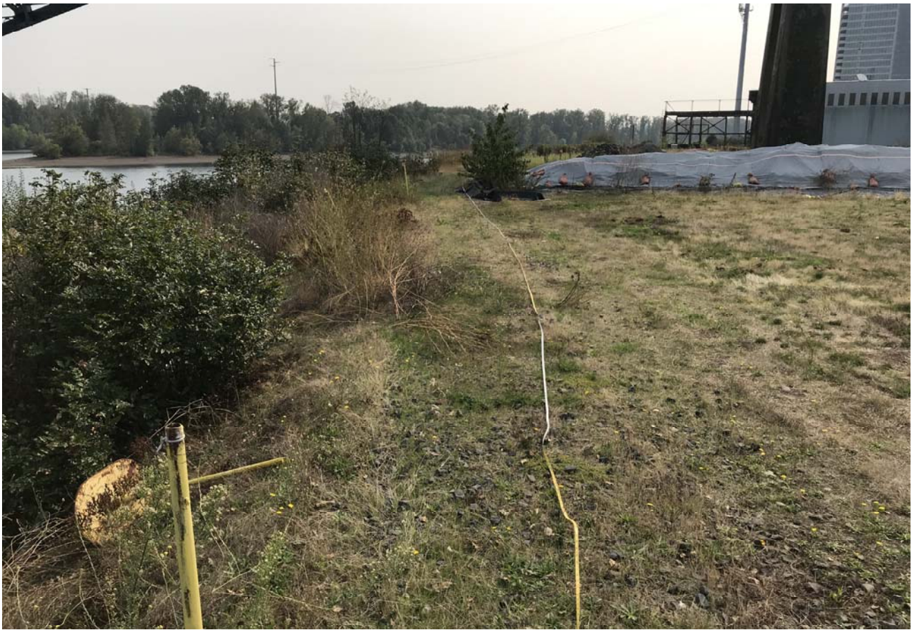
STA: 9+00 - Top of bank looking upstream
