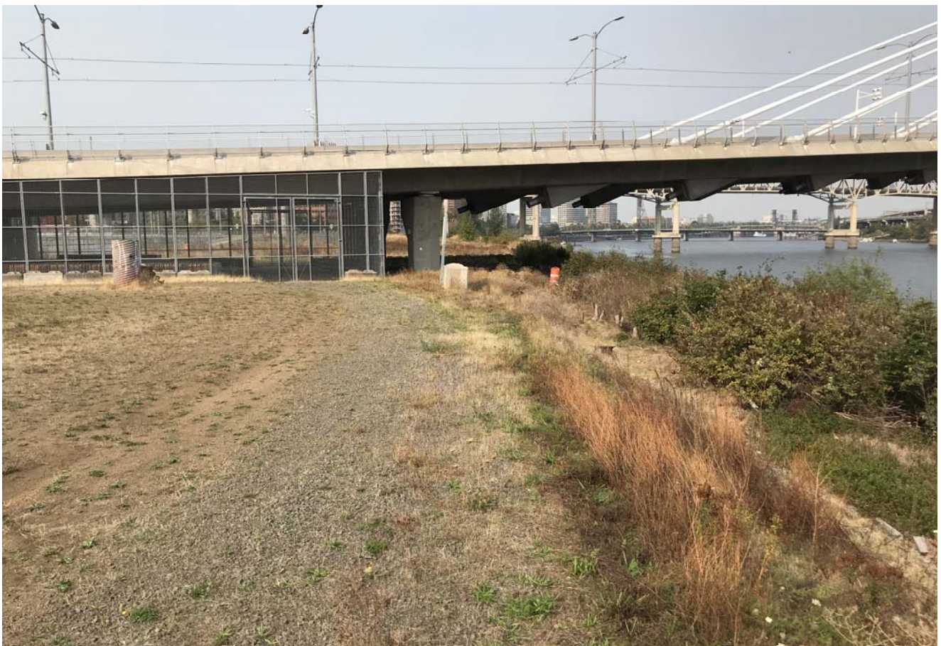
STA: 15+00 - Top of bank looking downstream
