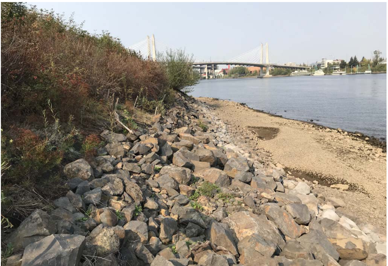
STA: 5+00 - Top of rock armor looking downstream
