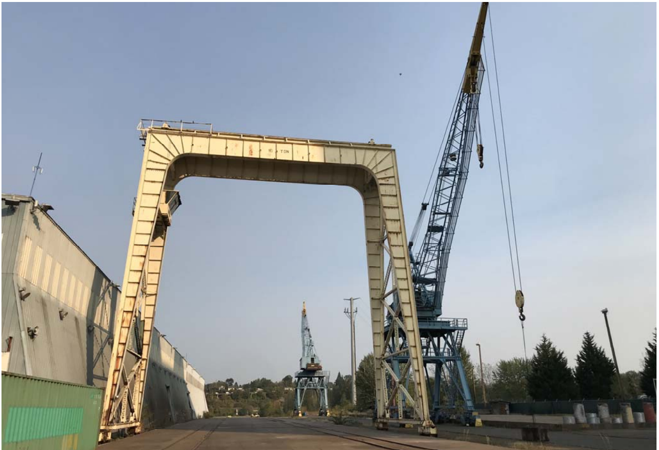
Operational area - Upper fabrication area looking east
