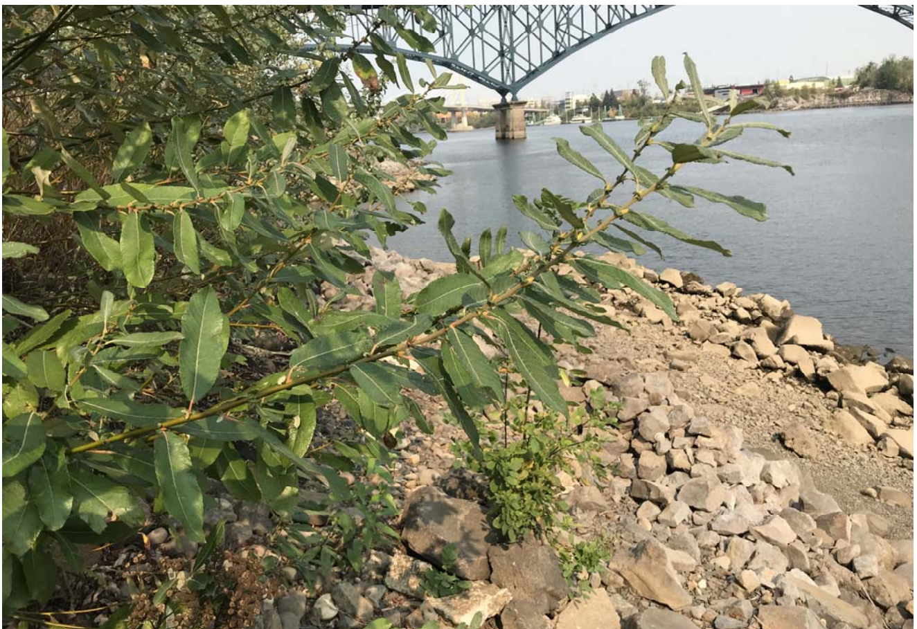
STA: 0+00 Top of rock armor looking downstream
