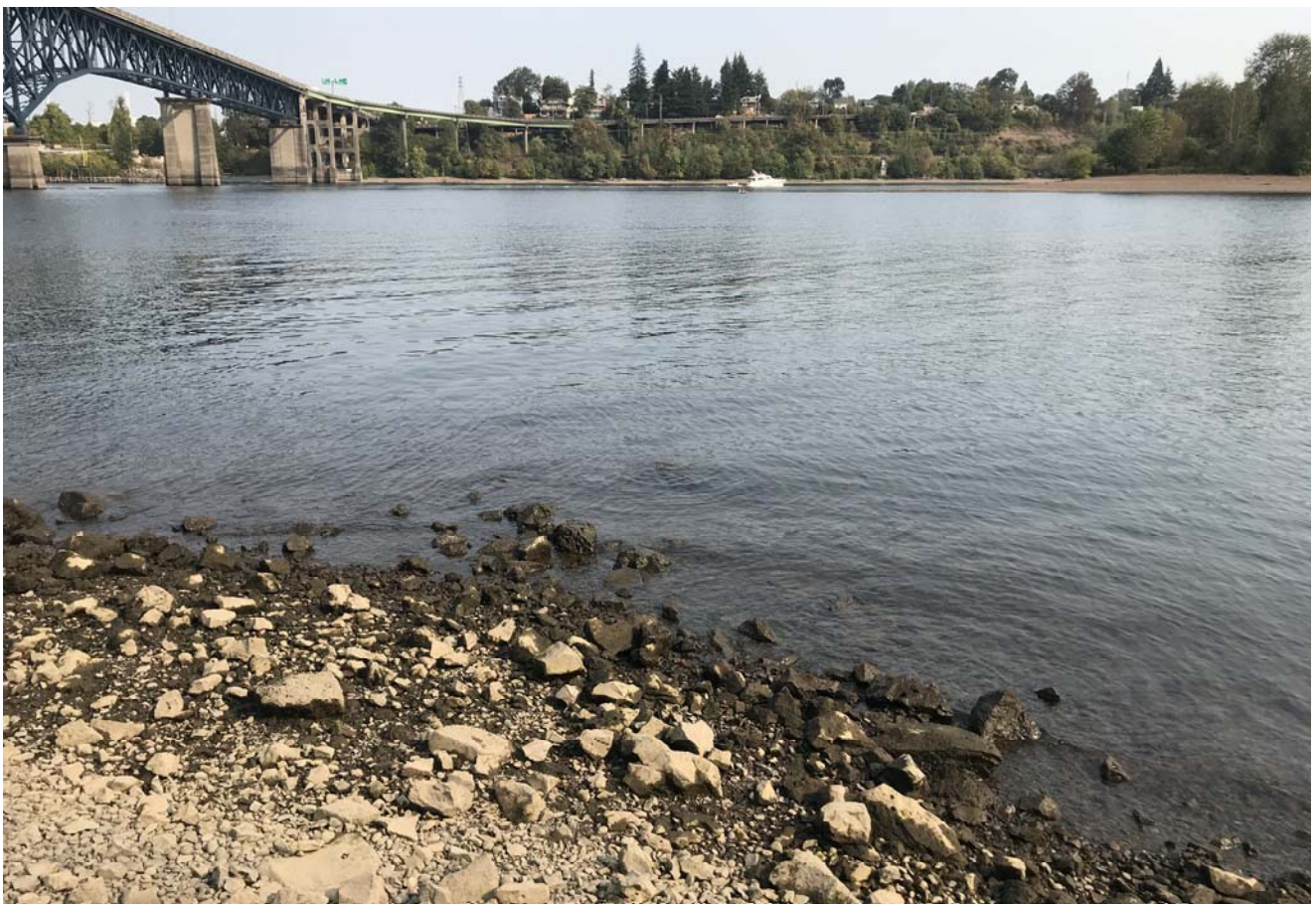
STA: 3+00 - Toe of slope looking east
