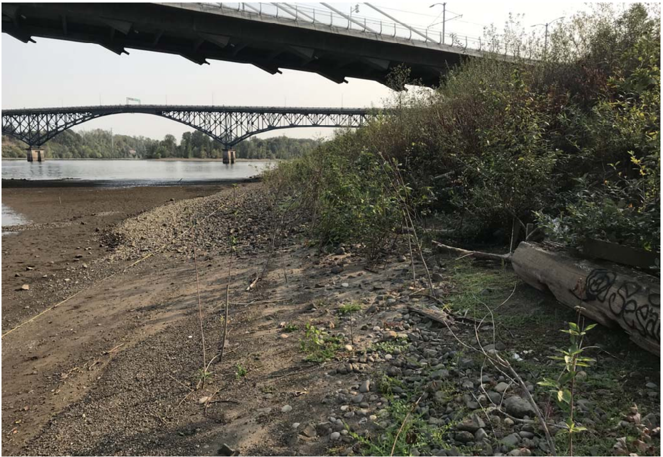
STA: 19+50 - Toe of slope looking upstream
