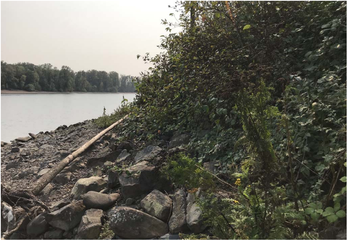
STA: 0+00 - Top of rock armor looking upstream
