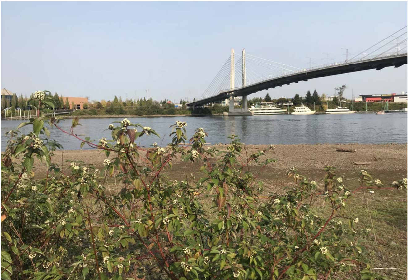
STA: 21+50 - Toe of slope looking east
