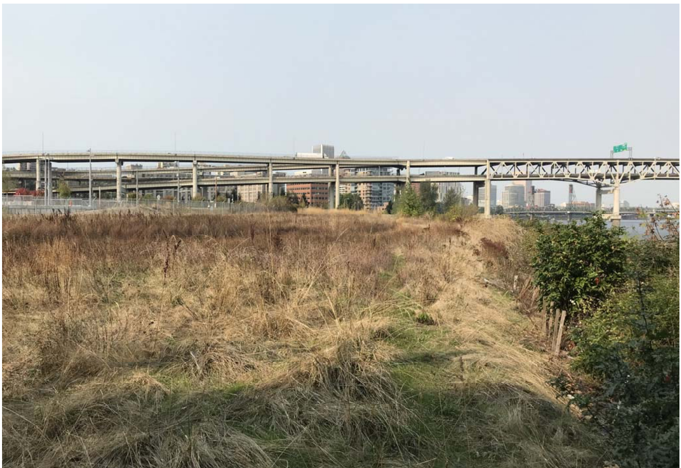
STA: 17+00 - Top of bank looking downstream
