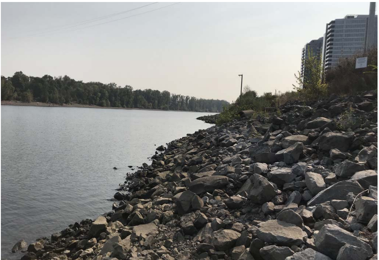
STA: 3+00 - Toe of slope looking upstream
