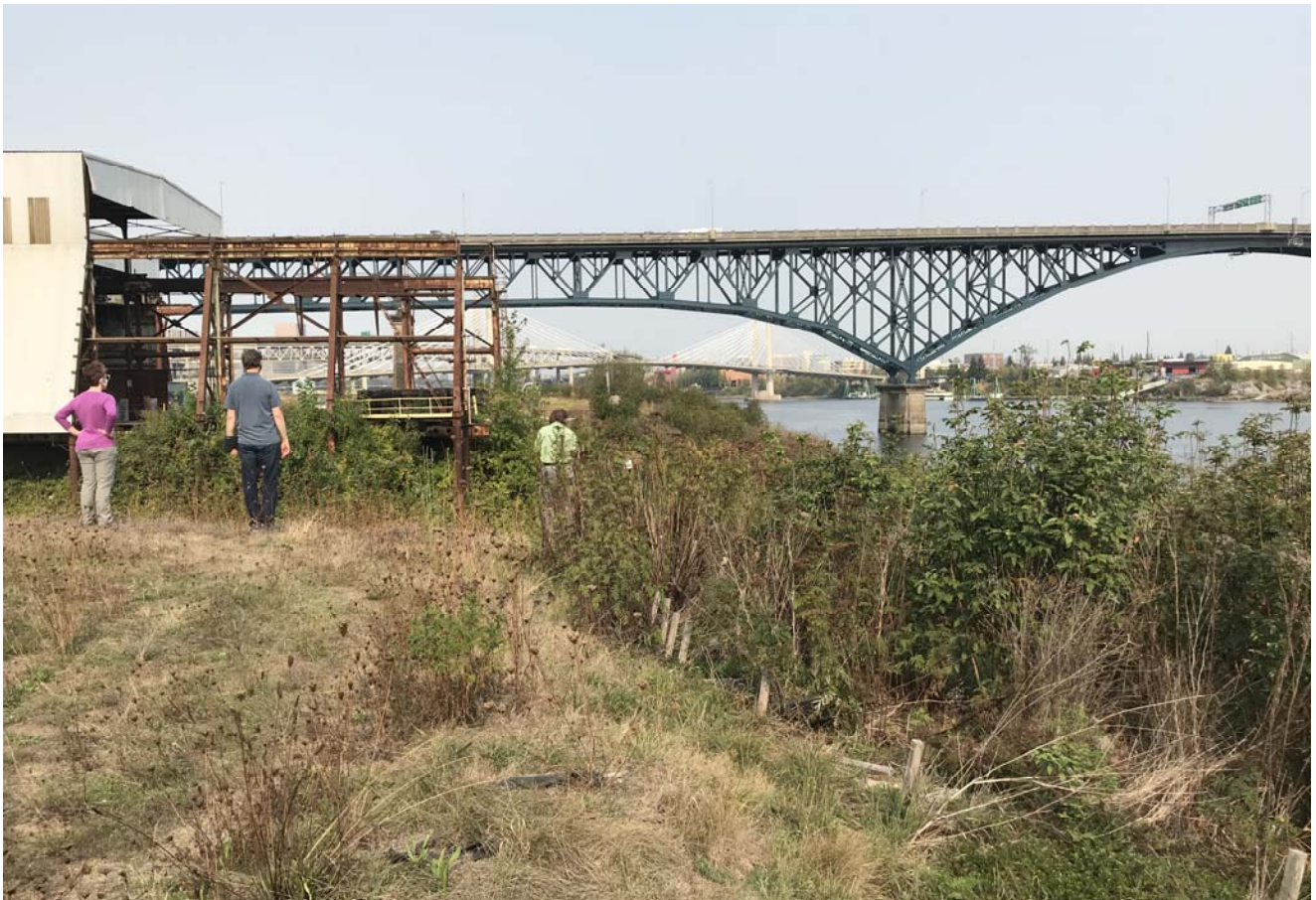
STA: 0+00 - Top of bank looking downstream
