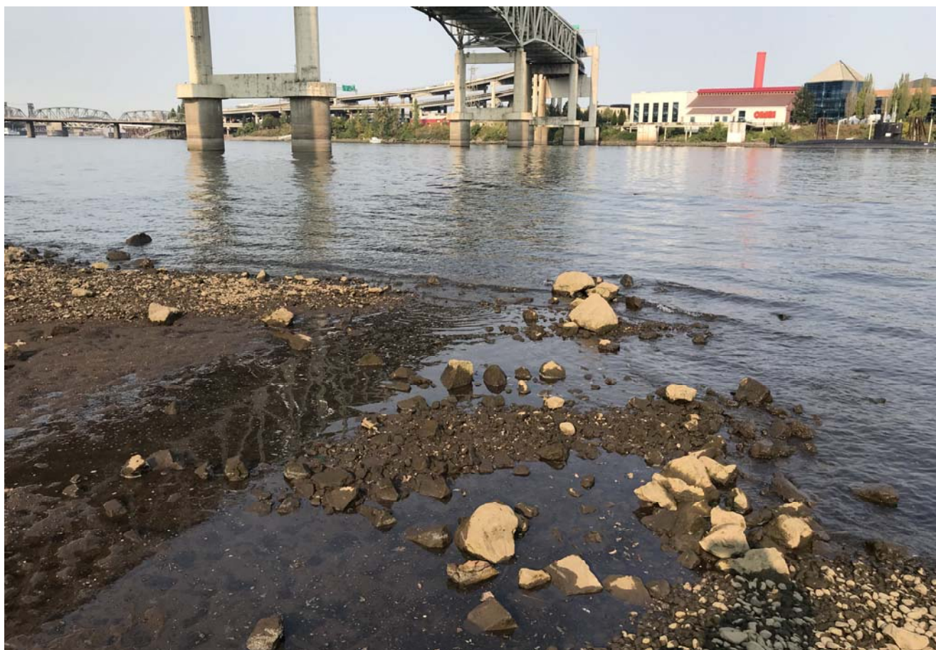
City of Portland outfall 07b flow path, looking northeast
