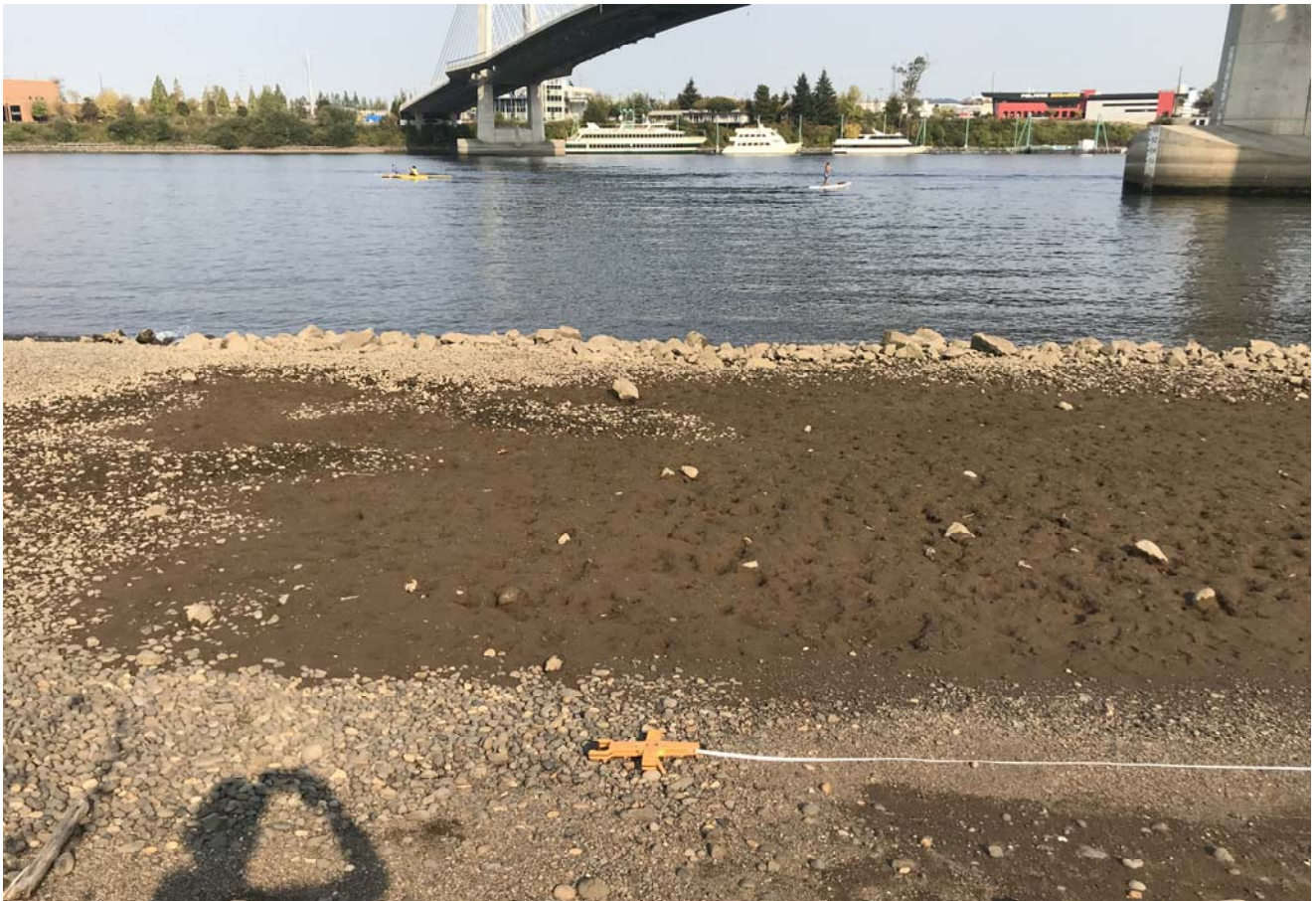
STA: 19+50 - Toe of slope looking east
