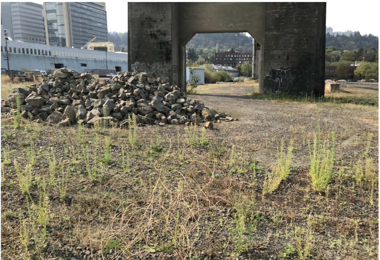
STA: 7+00 - Top of bank looking west
