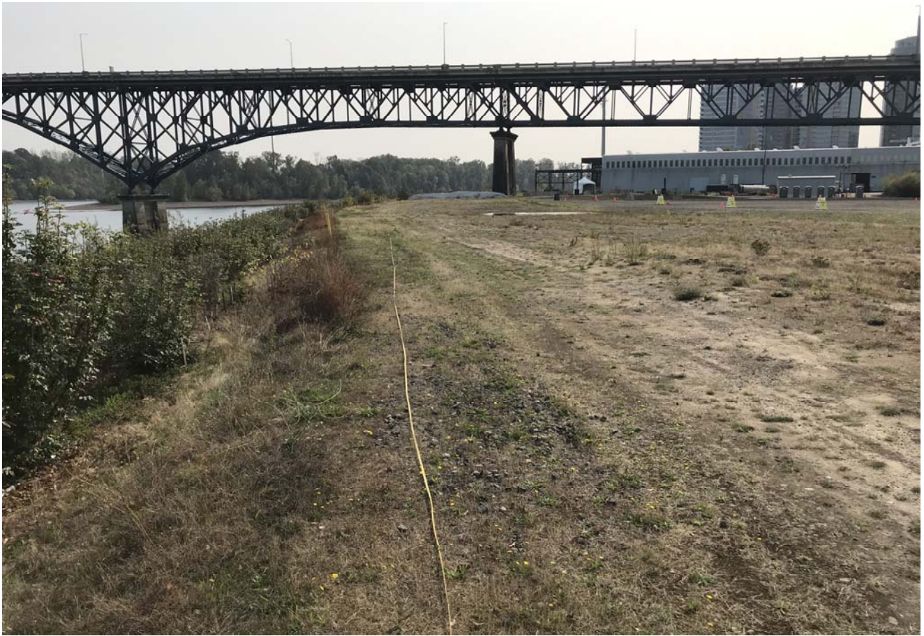
STA: 13+00 - Top of bank looking upstream
