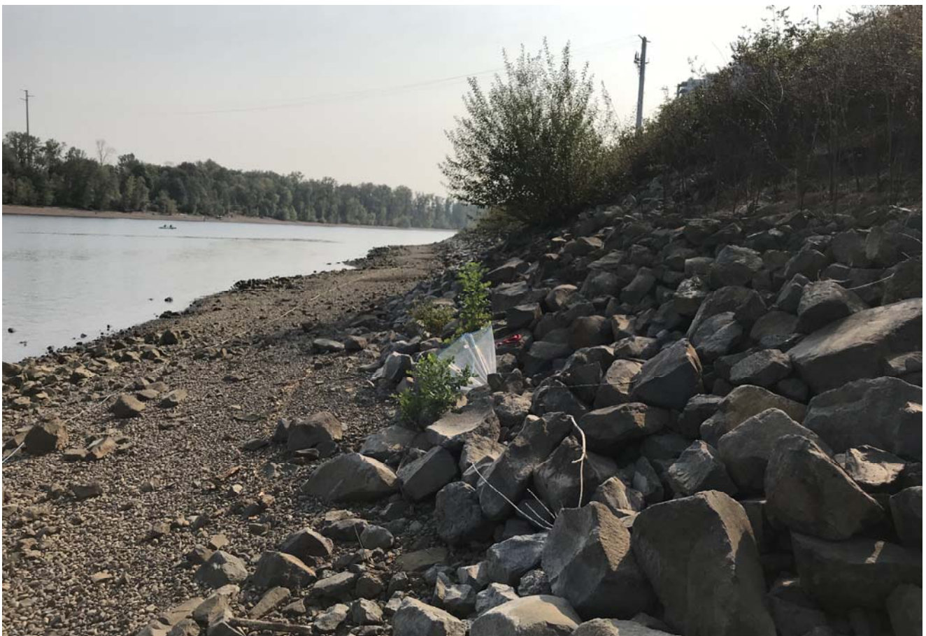
STA: 7+00 - Toe of slope looking upstream
