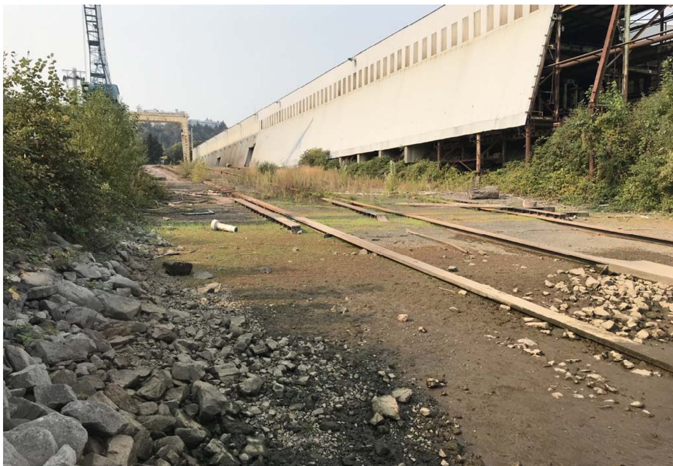
Slipway - Looking west
