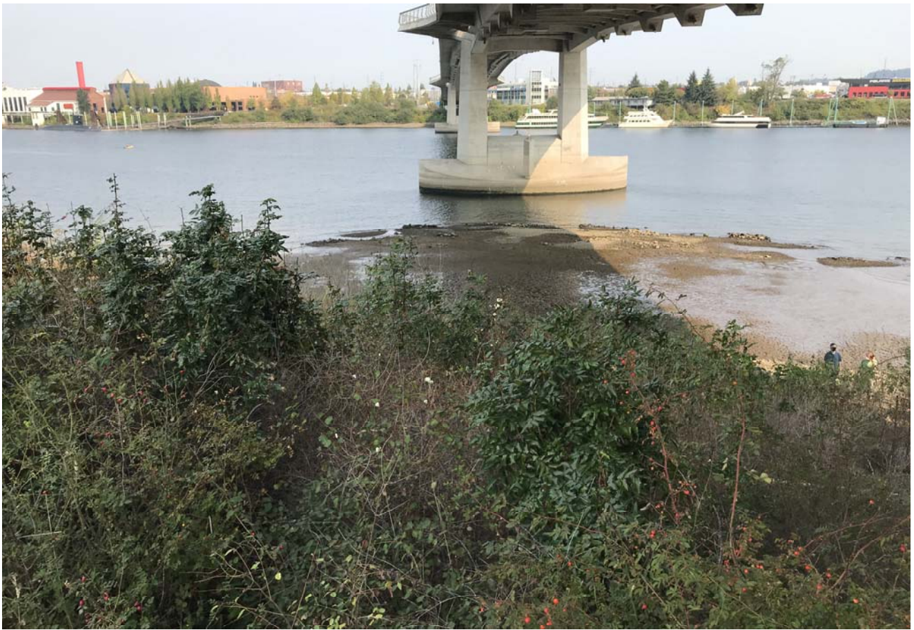
STA: 17+00 - Top of bank looking east
