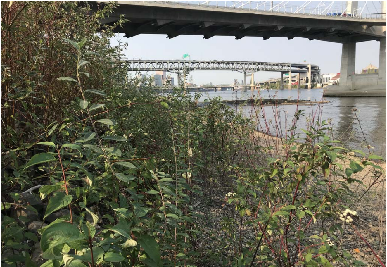
STA: 15+00 - Toe of slope looking downstream
