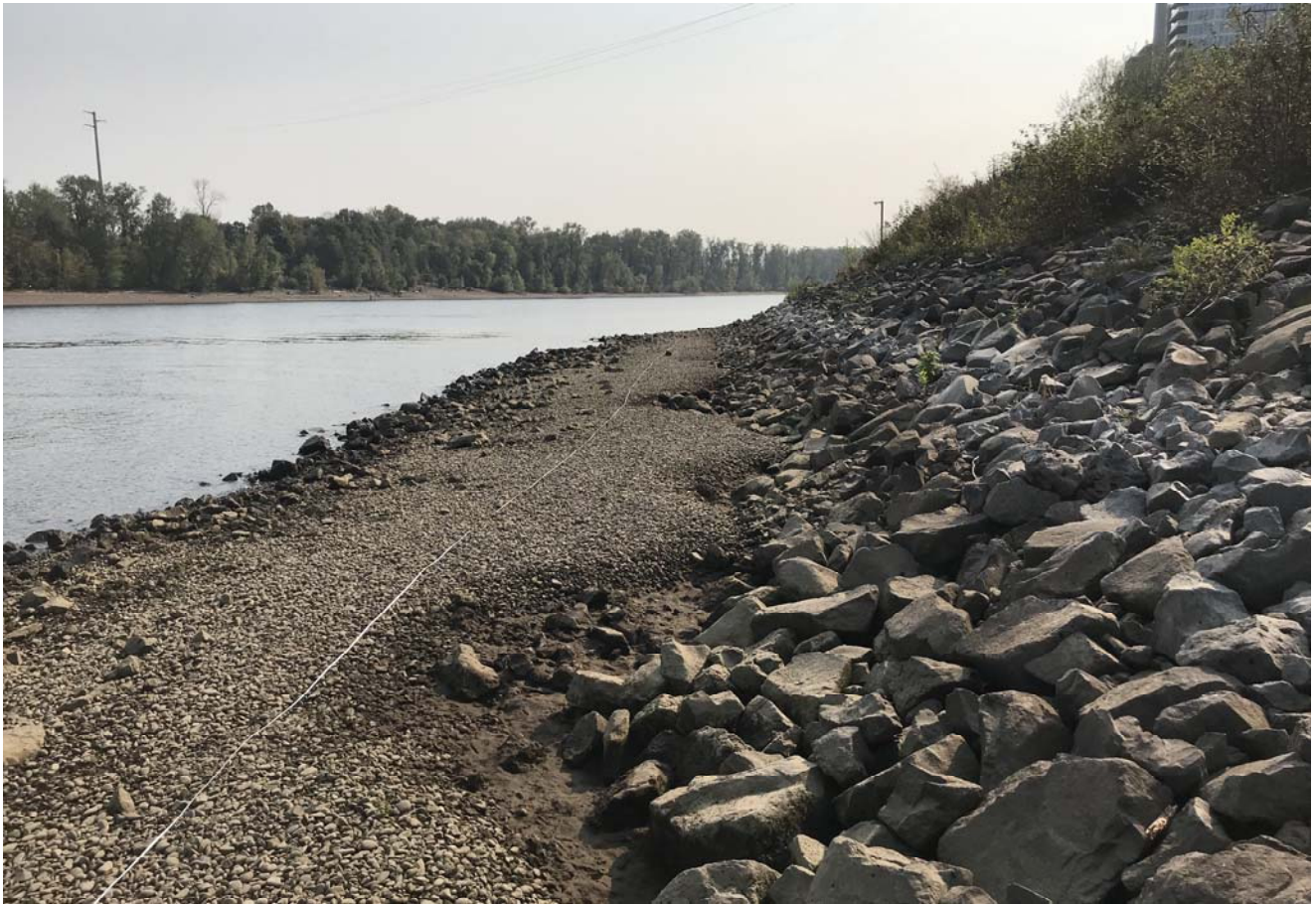
STA: 5+00 - Toe of slope looking upstream
