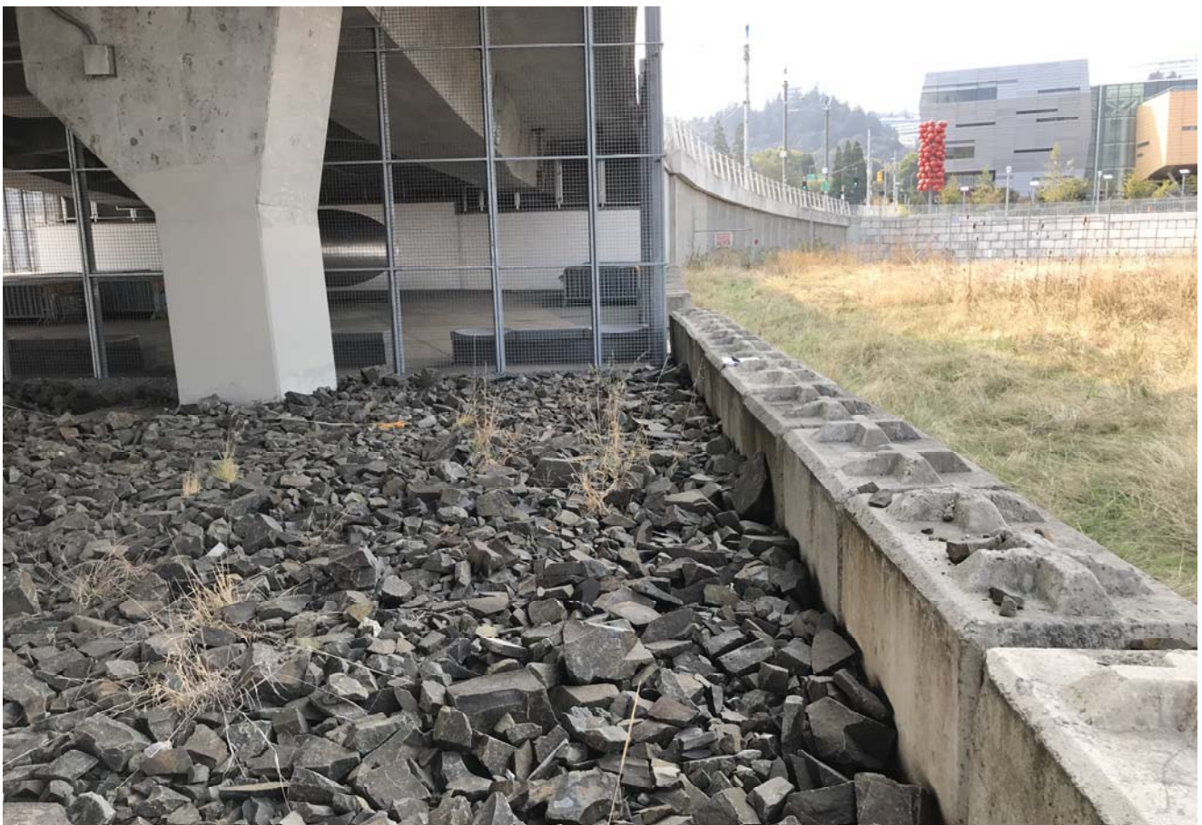
STA: 17+00 - Top of bank looking west
