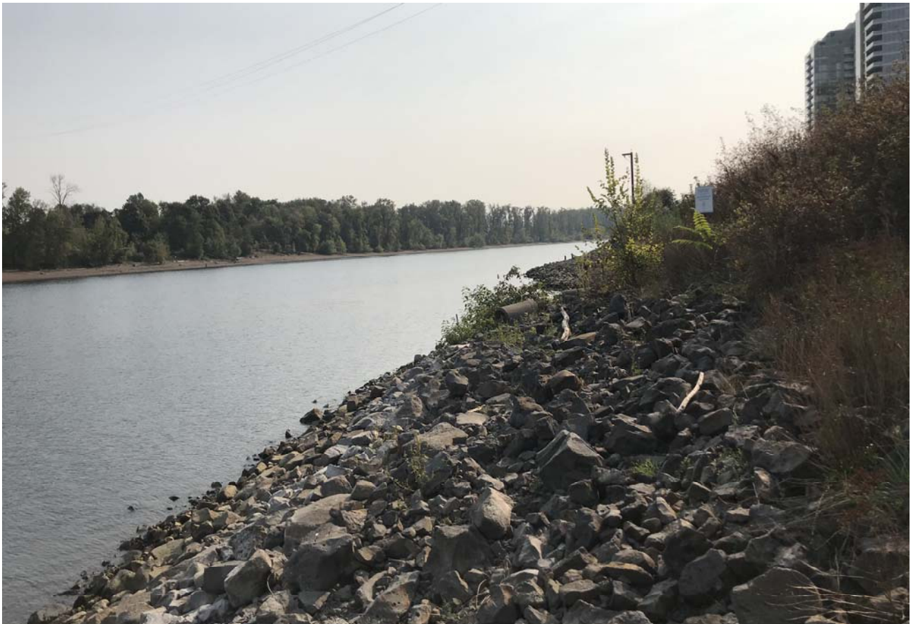
STA: 3+00 - Top of rock armor looking upstream
