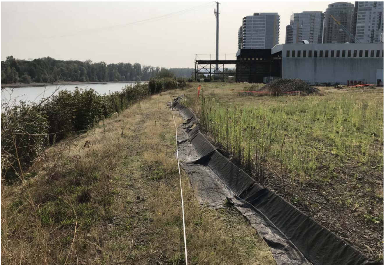
STA: 7+00 - Top of bank looking upstream
