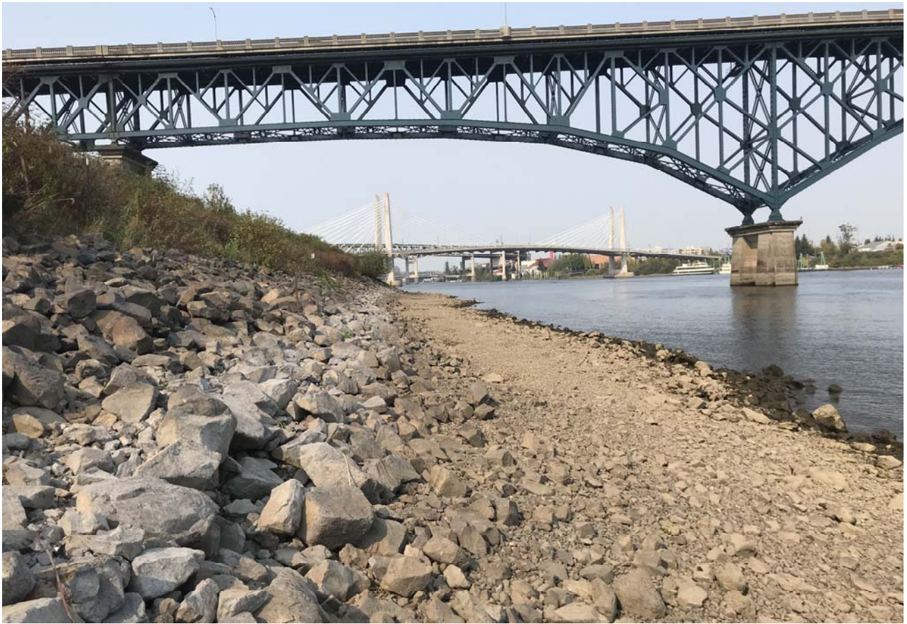
STA: 3+00 - Toe of slope looking downstream
