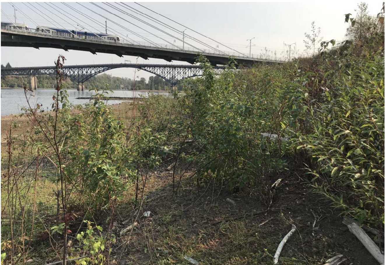
STA: 21+50 - Toe of slope looking upstream
