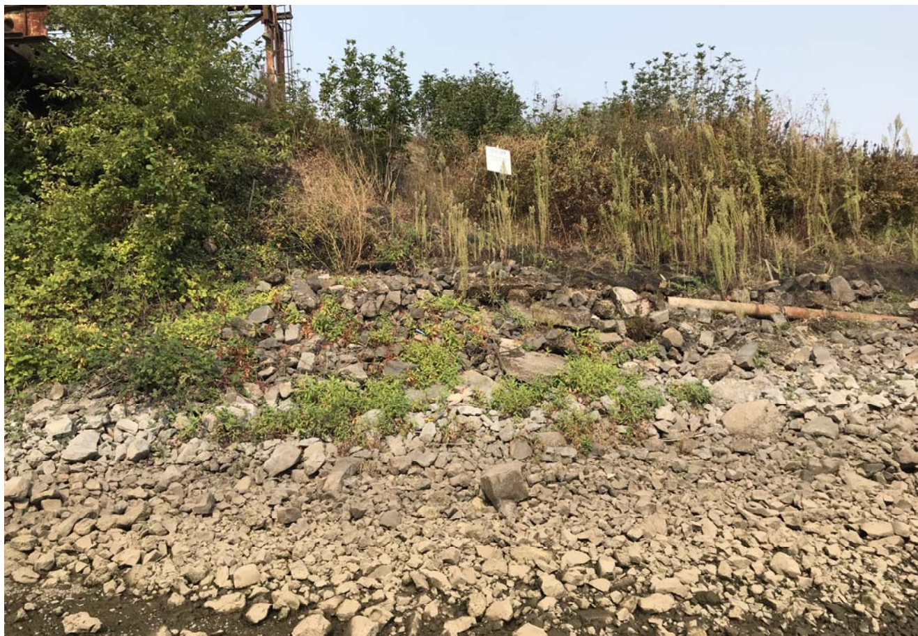
Rock armor on northeast slope of slipway
