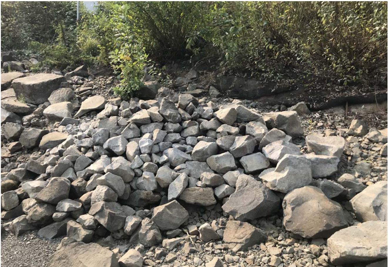
STA: 0+00 - Mounded rock armor over cap
