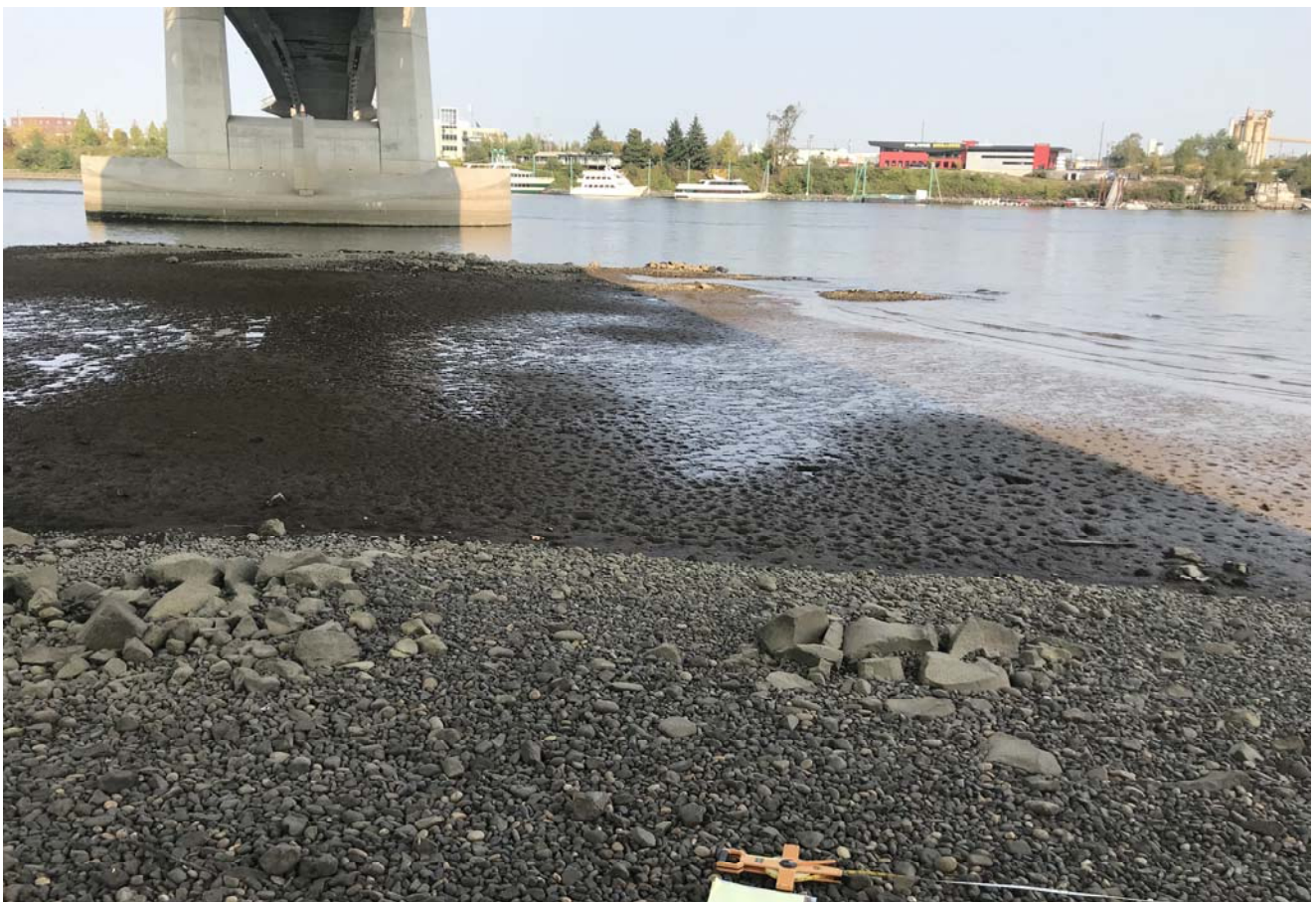
STA: 17+00 - Toe of slope looking east
