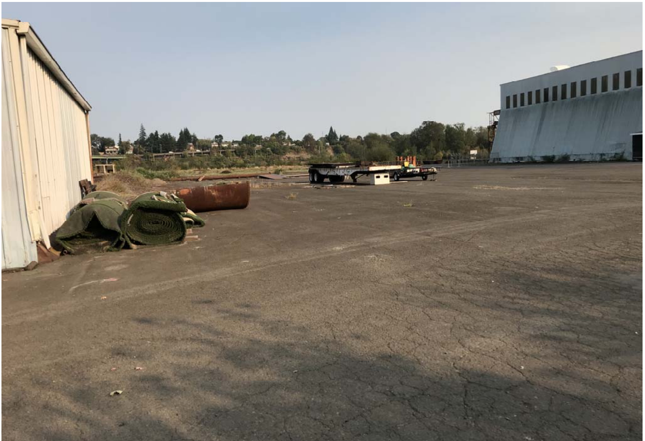
Operational area - East of stormwater pond looking east
