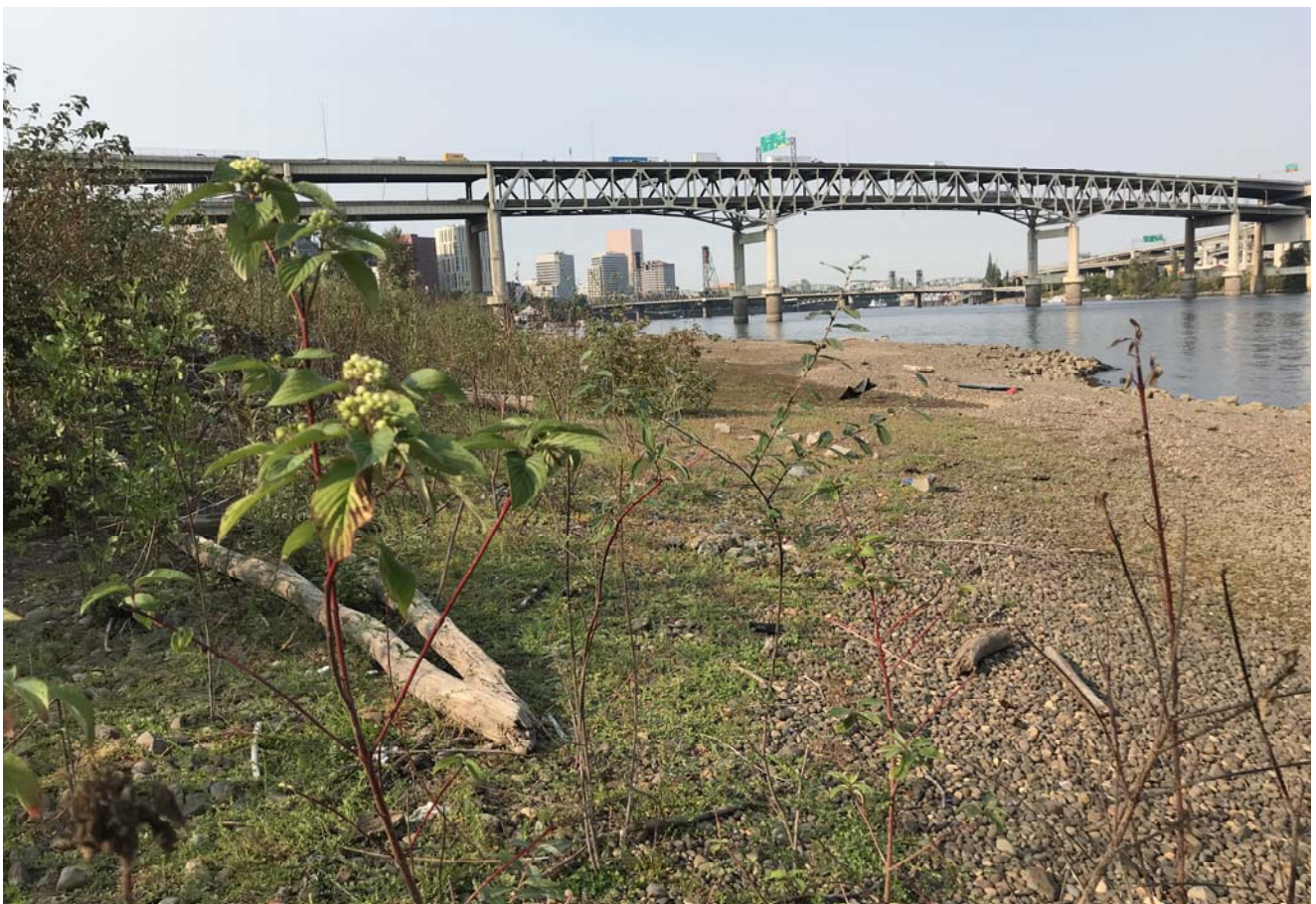
STA: 19+50 - Toe of slope looking downstream
