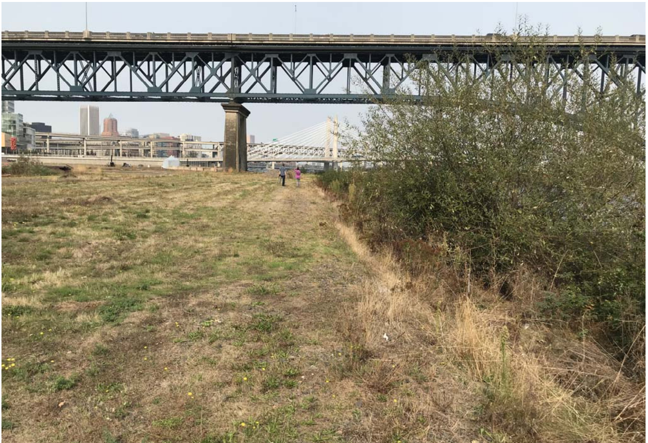
STA: 3+00 - Top of bank looking downstream
