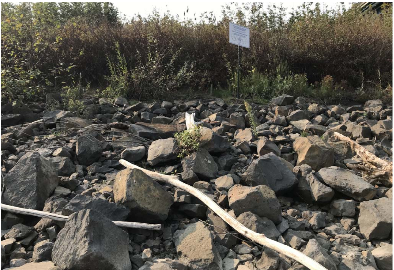
STA: 5+00 - Toe of slope looking west
