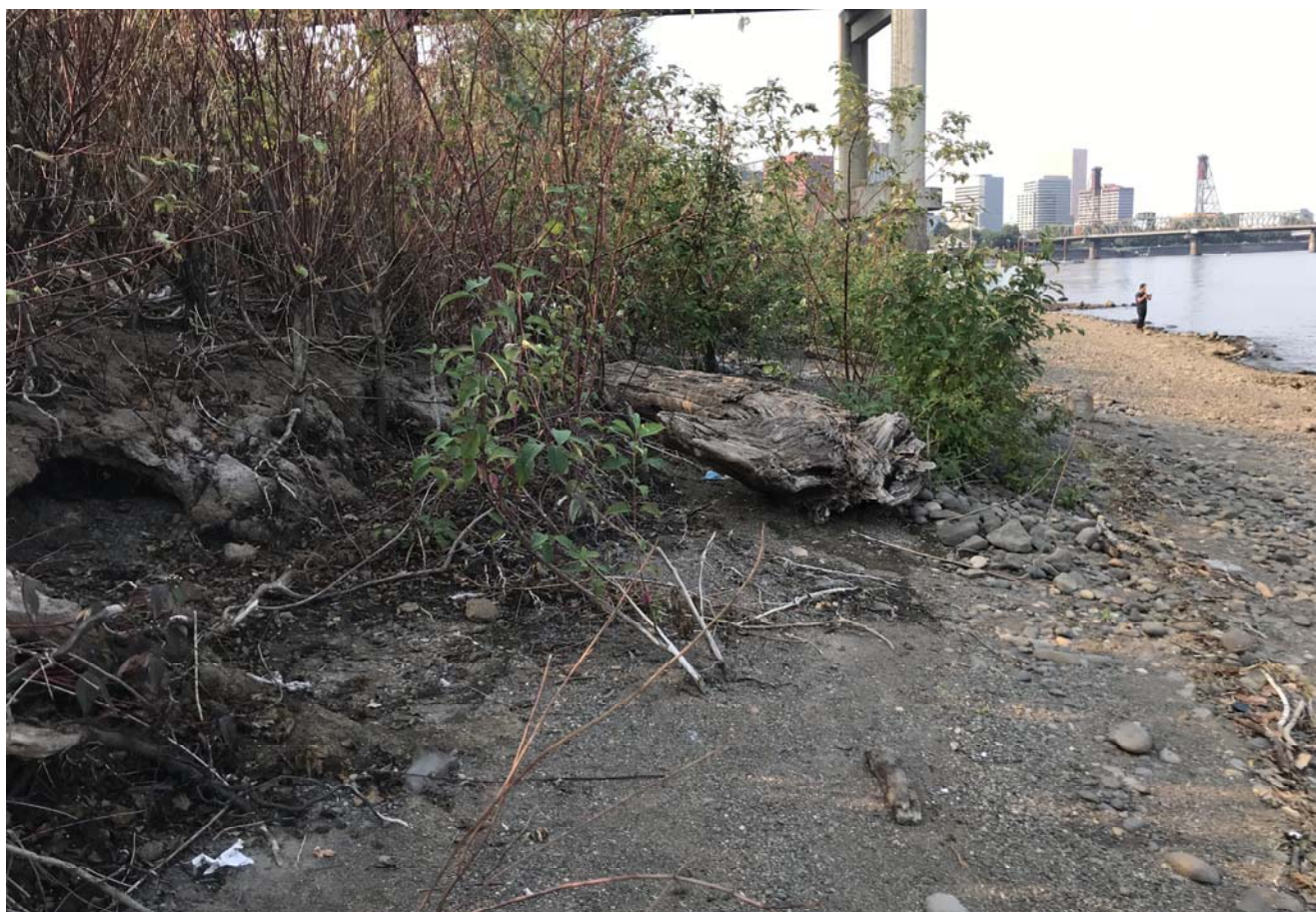
STA: 25+50 - Toe of slope looking downstream
