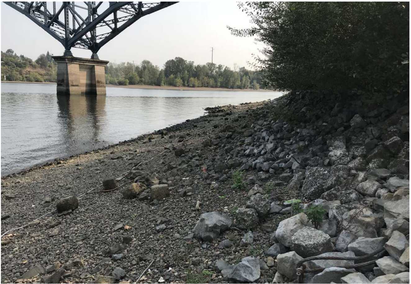
STA: 9+00 - Toe of slope looking upstream
