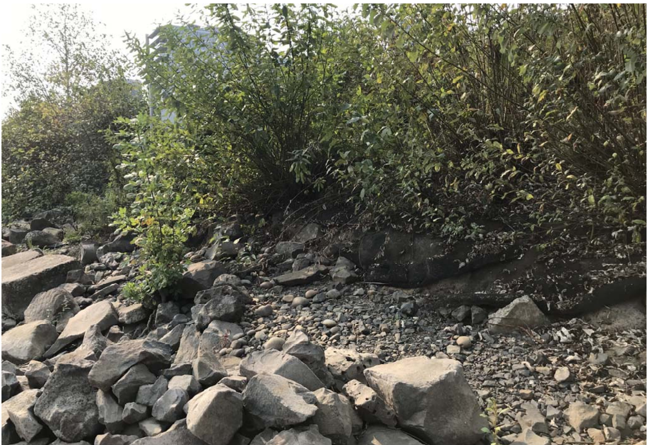
STA: 0+20 - Toe of slope with exposed TRM
