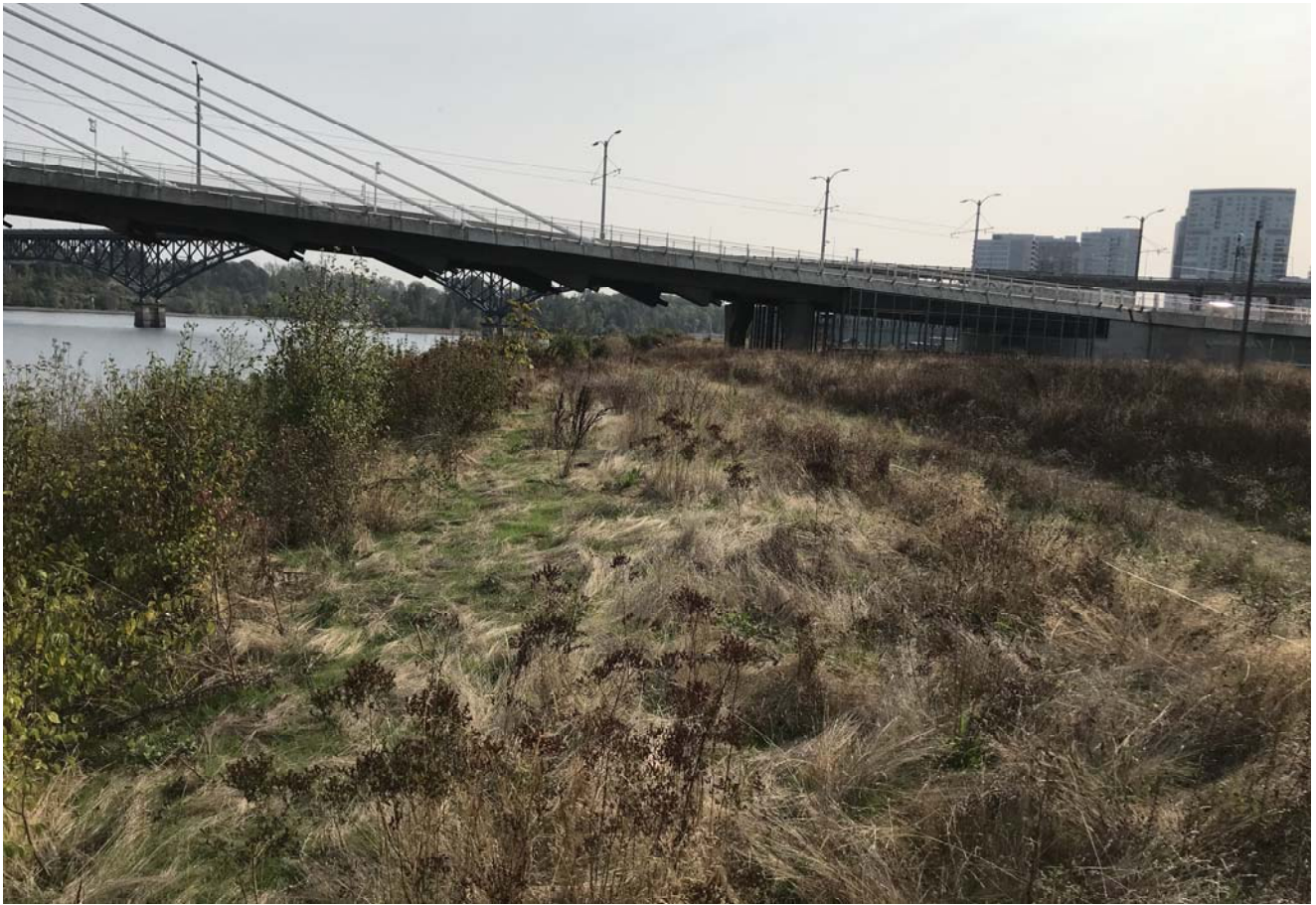
STA: 19+50 - Top of bank looking upstream
