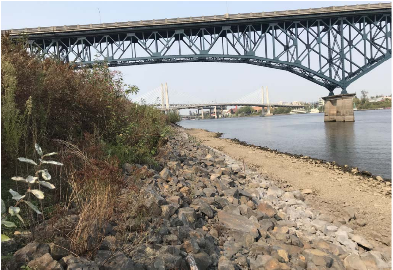
STA: 3+00 - Top of rock armor looking downstream
