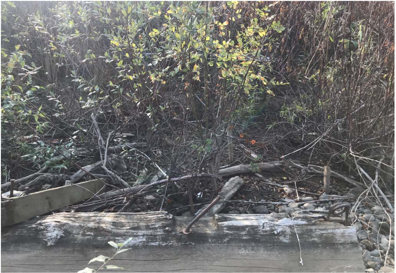
STA: 19+50 - Toe of slope looking west
