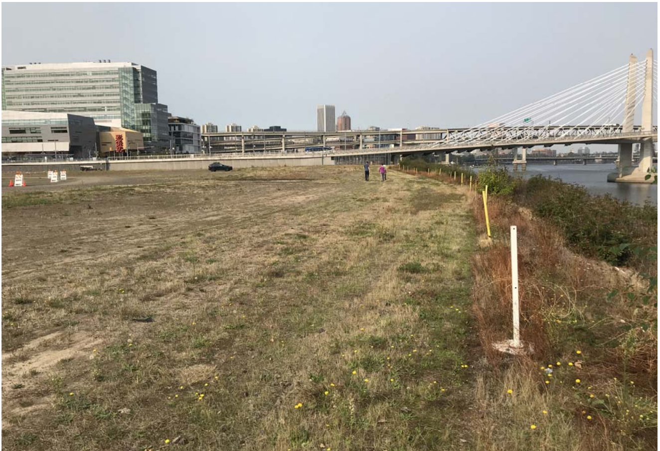
STA: 9+00 - Top of bank looking downstream
