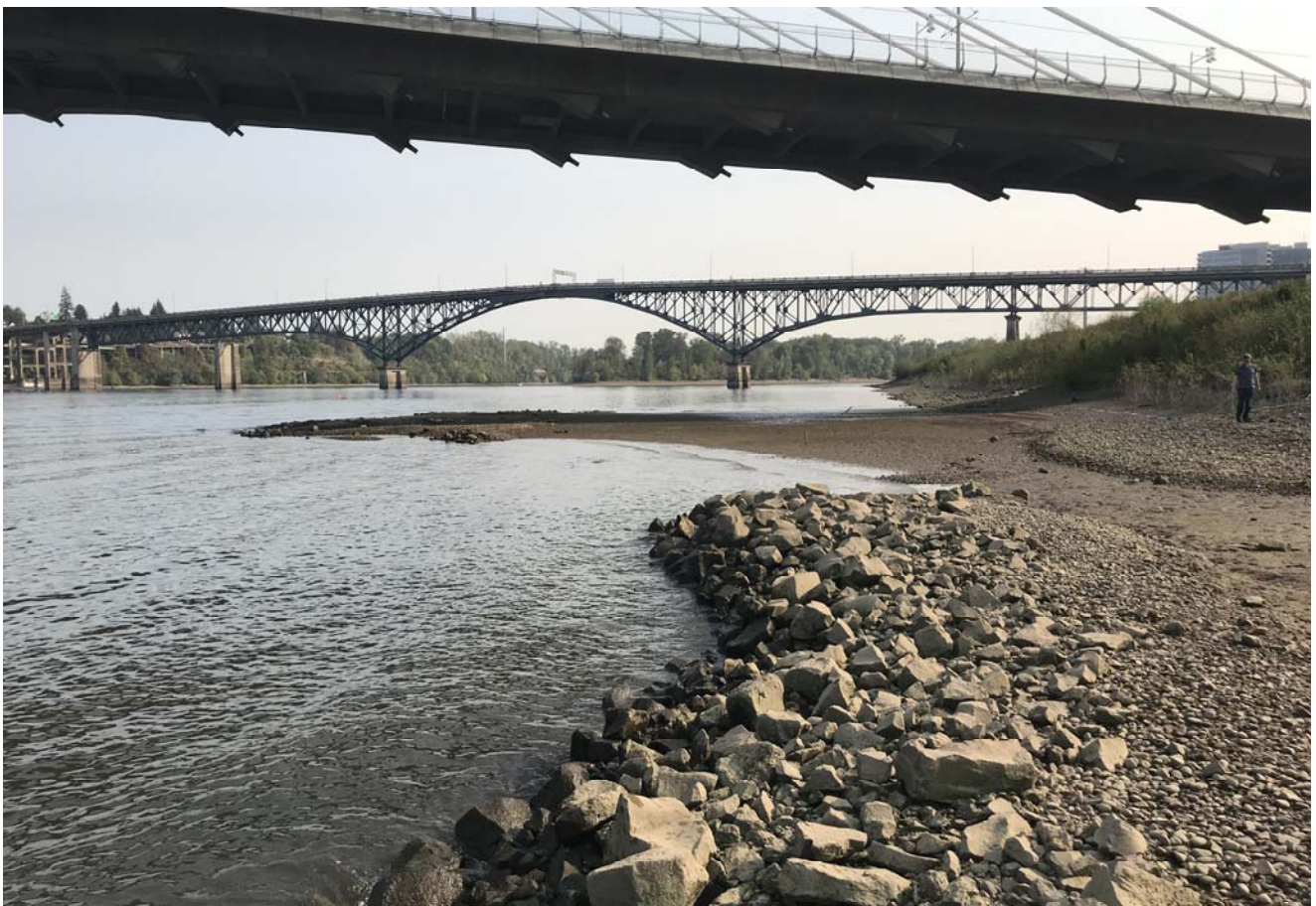
STA: 19+50 - Edge of water looking upstream
