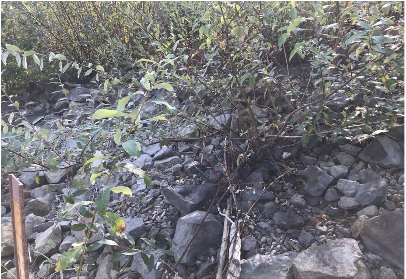
STA: 13+75 - 2018 Bank repair area
