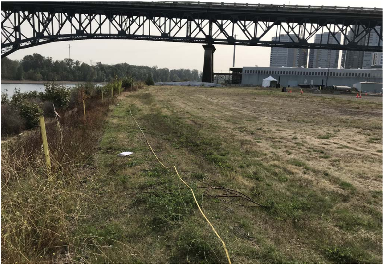
STA: 11+00 - Top of bank looking upstream
