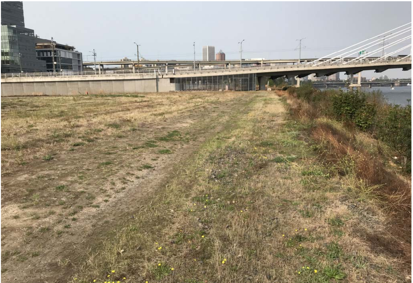
STA: 13+00 - Top of bank looking downstream
