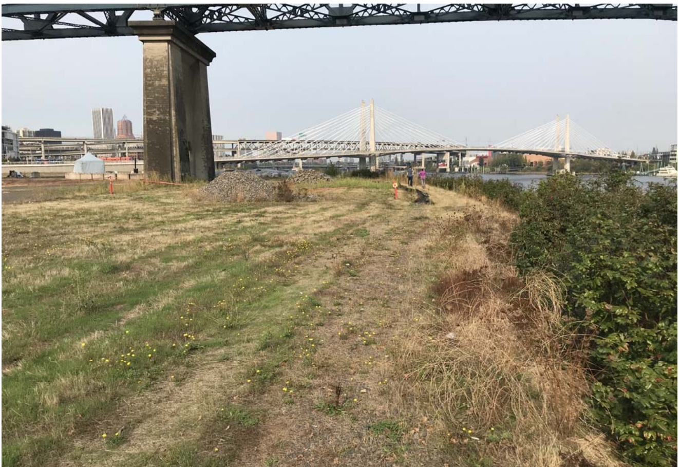
STA: 5+00 - Top of bank looking downstream
