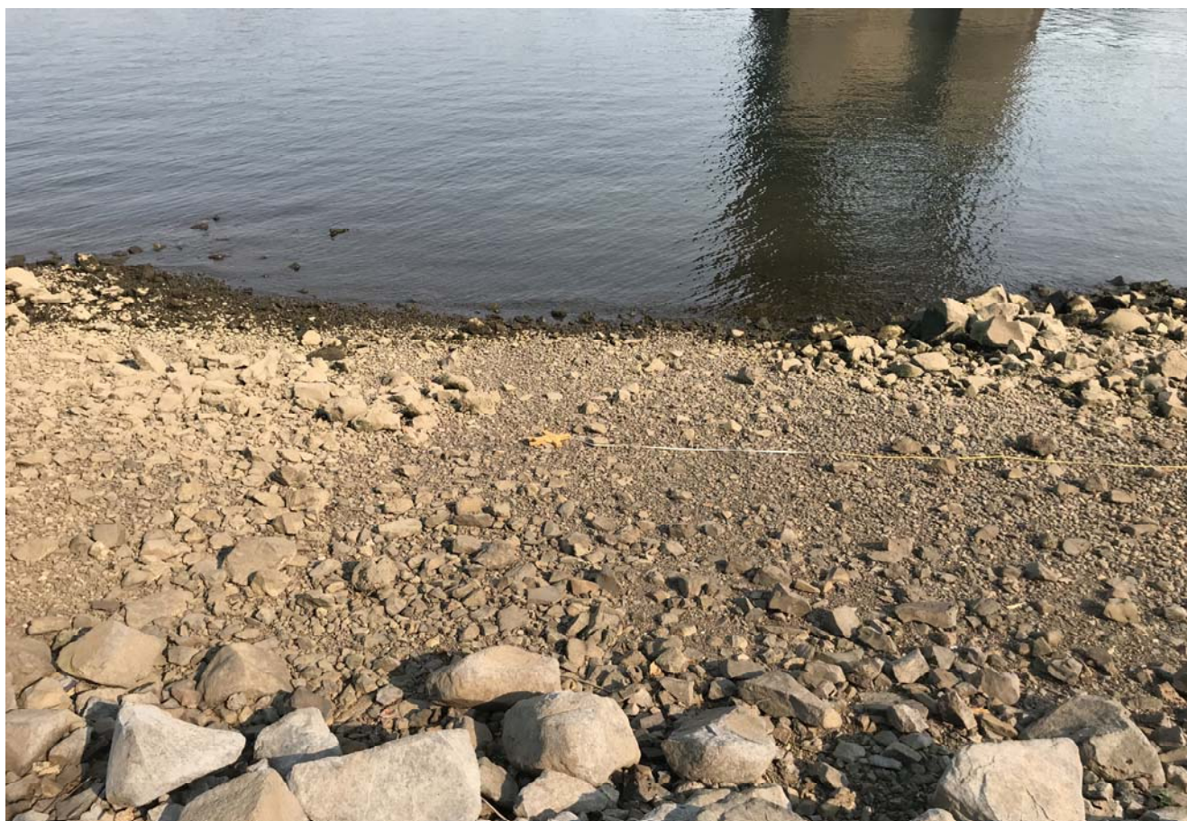
STA: 7+00 - Top of rock armor looking east
