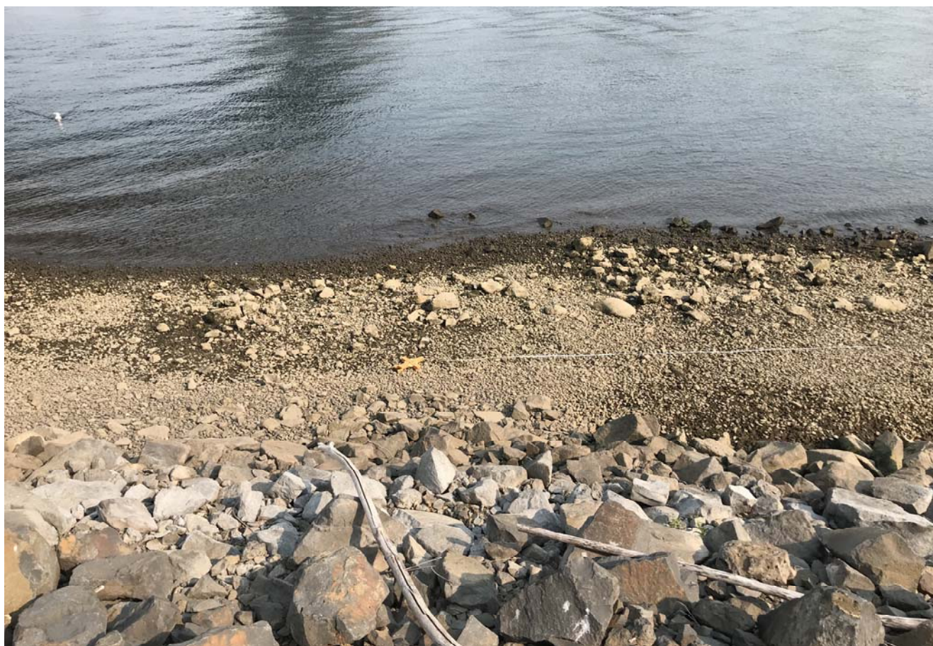
STA: 5+00 - Top of rock armor looking east
