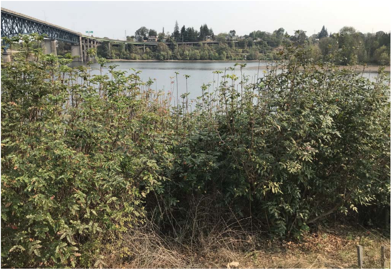
STA: 3+00 - Top of bank looking east
