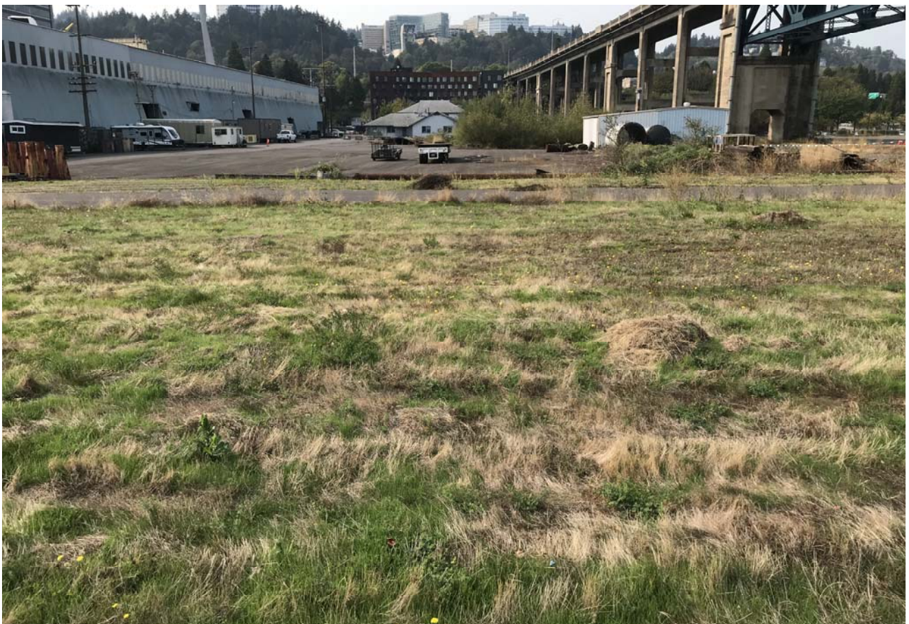
STA: 5+00 - Top of bank looking west
