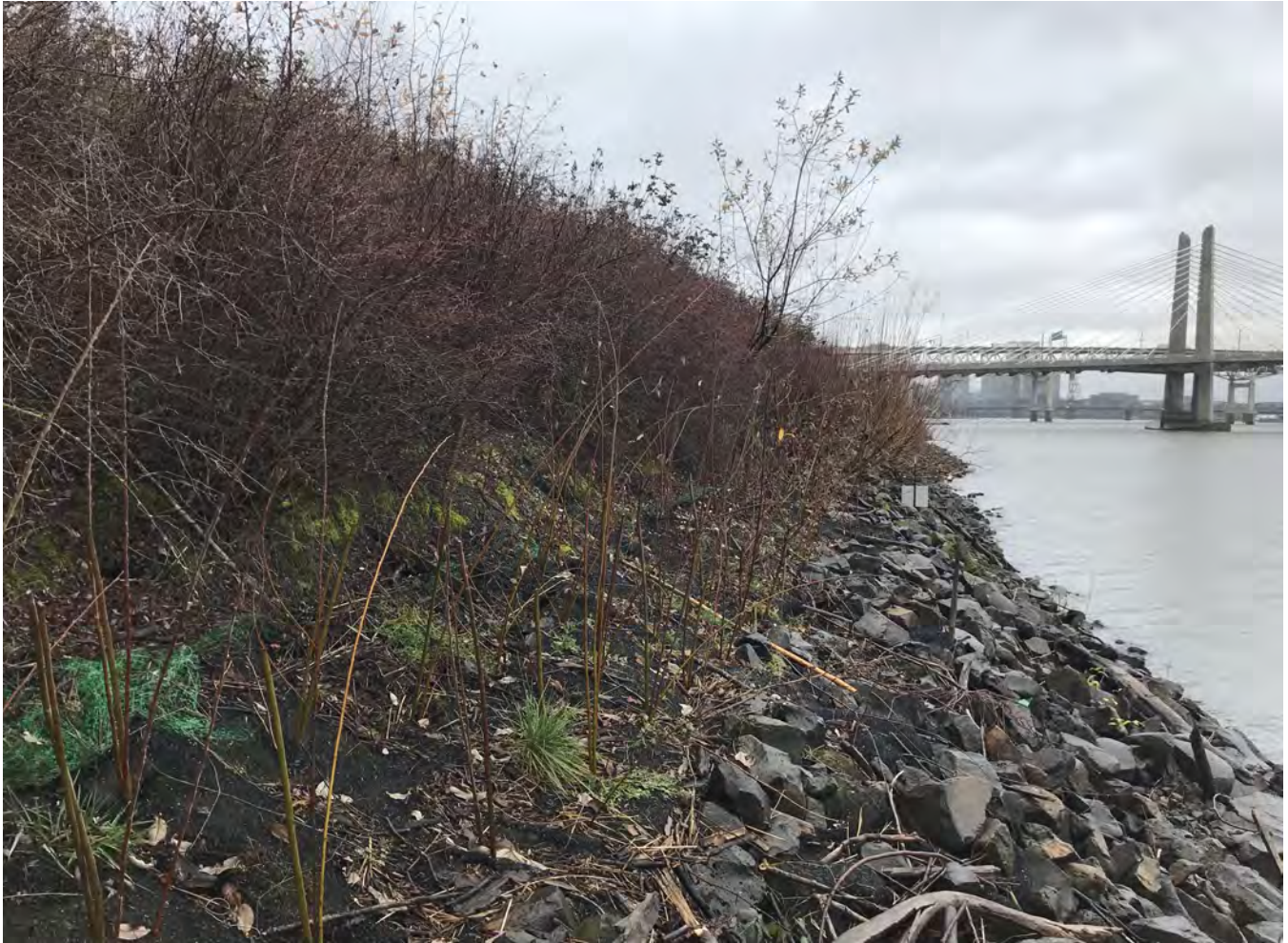
PHOTO 1 - New planting along the North side of the Ross Island Bridge at 16 feet elevation.
