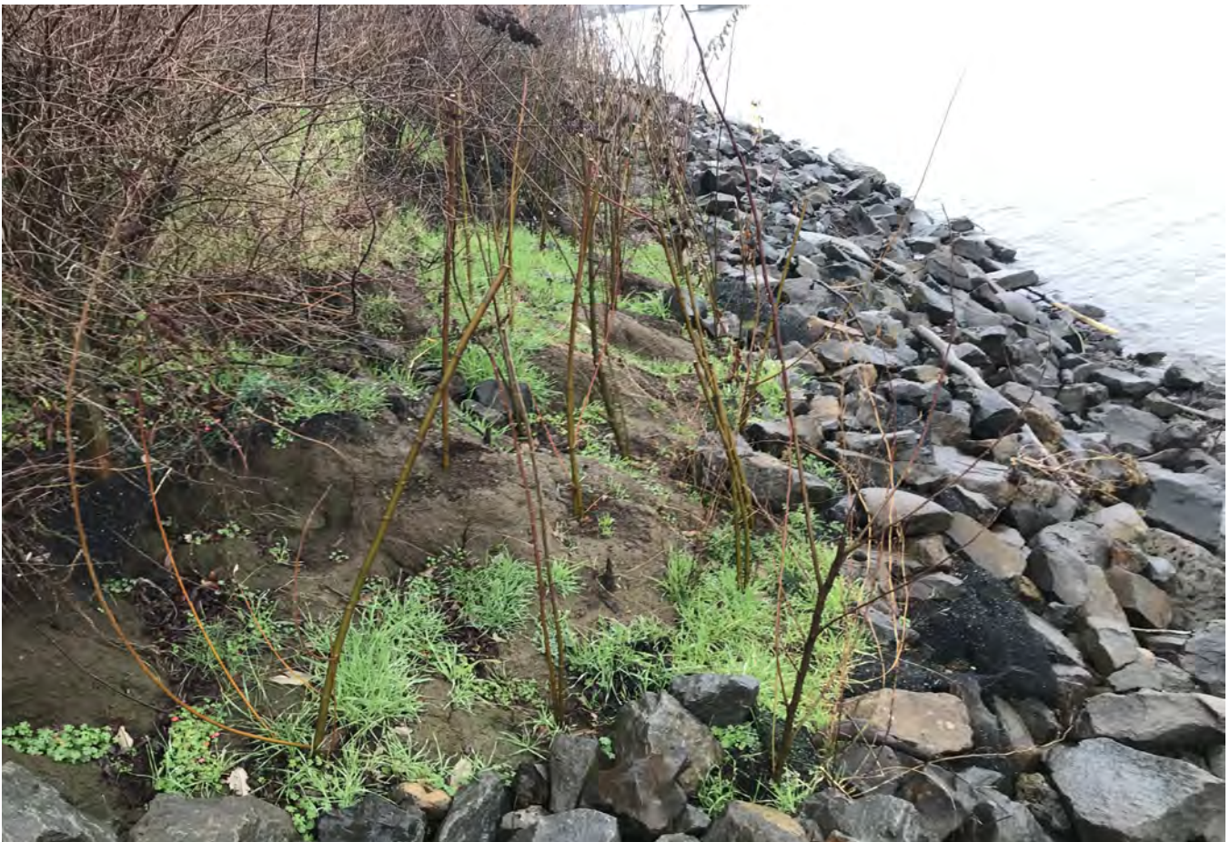
PHOTO 2: New plantings at the top of armor below the North edge of the Ross Island Bridge.
