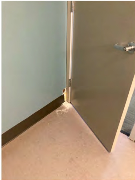
Photo 1 - View of sample location KP5 in the medical office restroom. The joint compound on the gypsum wallboard has 2% chrysotile asbestos and Point Count analysis of all layers had < 1% asbestos. (11/10/2023)
