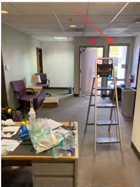
Photo 3 - View of sample locations KP3p, a green paint on gypsum wallboard in the medical office reception, and KP6p, a tan/gray paint on wood window trim (red arrow). (11/10/2023)
