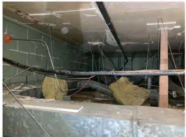
Photo 8 - View of sample location KP9p, a green paint on wood and CMU walls in the landscape shop area. (11/10/2023)
