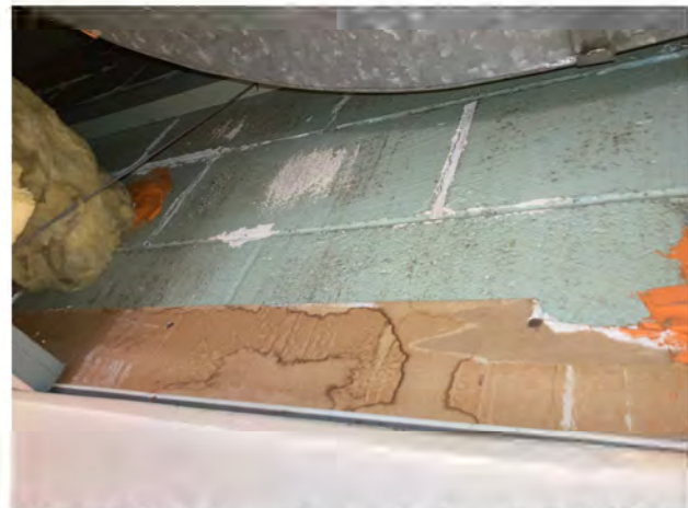
Photo 12 - View of sample location KP15p, a green paint on wood and CMU walls in the landscape area shop. (10/29/2024)
