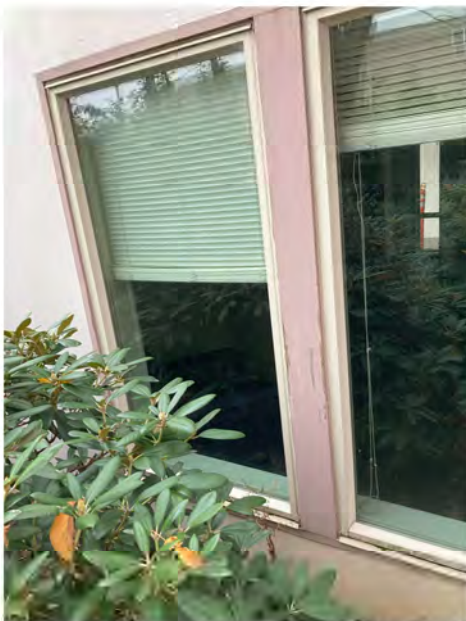
Photo 11 - View of sample locations KP13p, an off-white/rose paint on exterior wood and cement board siding, and KP14p, a brown/pink paint on exterior wood trim. (11/10/2023)
