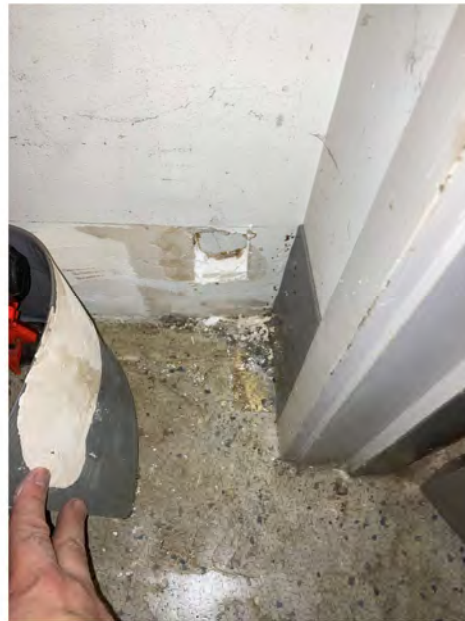
Photo 2 - View of sample location KP30 in the landscape office. The joint compound on the gypsum wallboard has 2% chrysotile asbestos and Point Count analysis of all layers had 0.3% asbestos. (11/10/2023)
