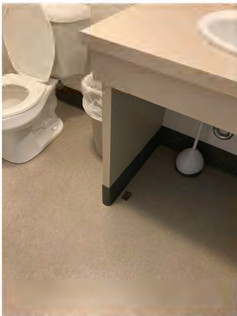
Photo 3 - View of sample location KP9 in the medical office restroom. The black mastic associated with the gray patterned SVT flooring has 5% chrysotile asbestos. (11/10/2023)
