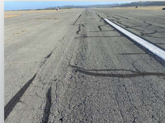
Runway 18-36 Cracking
