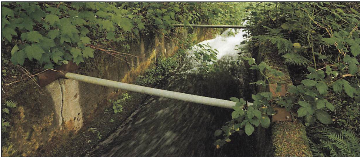
Figure 2-2. View looking downstream at spillway showing cracks in concrete and support struts used to resist landslide creep-induced damage. Photo taken May 9, 2022.
