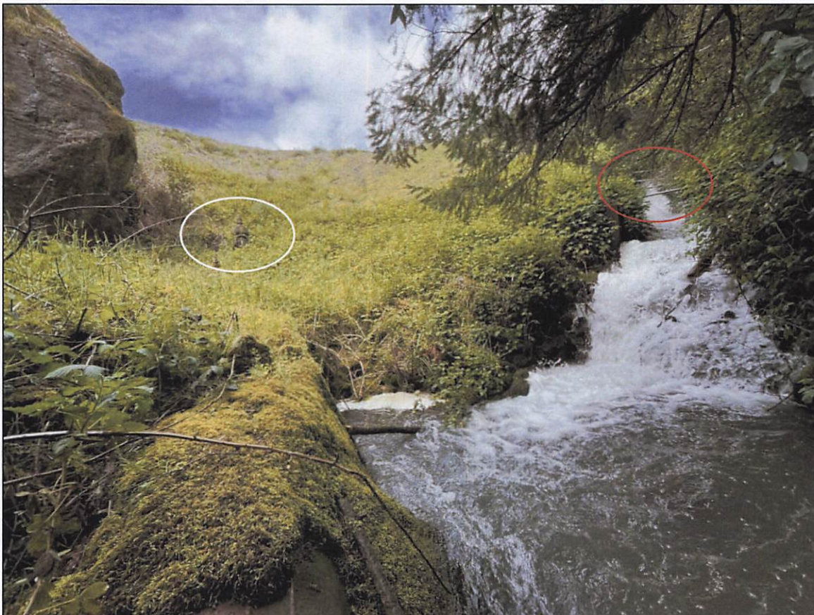
Figure 2-3. View looking upstream at the downstream face and toe of Ferry Creek Dam and the downstream end of the spillway. The metal struts in the spillway are marked with a red circle. The large moss-covered, outlet pipe is visible in the foreground, and additional pipe infrastructure is circled in white. The bimrock is visible on top left. Photo taken May 9, 2022.
