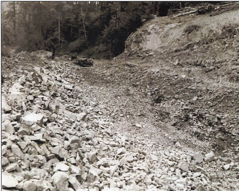
Figure 2-6. Historical photo looking upstream at construction of the berm and ditch on the river-left side of reservoir. Photo taken some time between 1945 and 1960.
