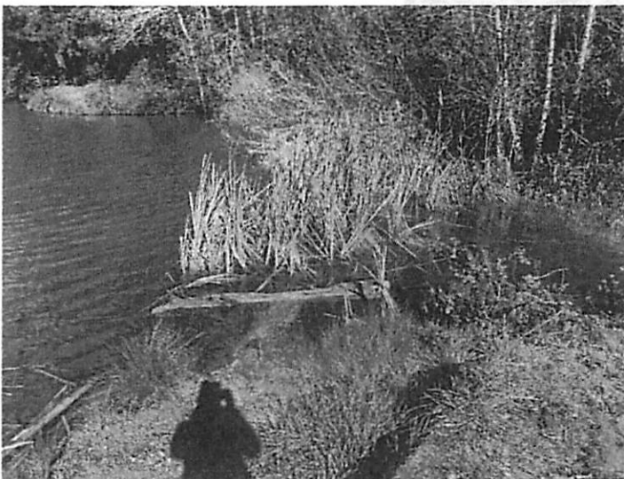
Spillway approach channel overgrown with Cattails
