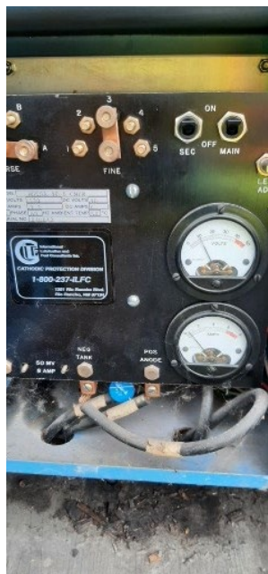
7: Impressed current rectifier
