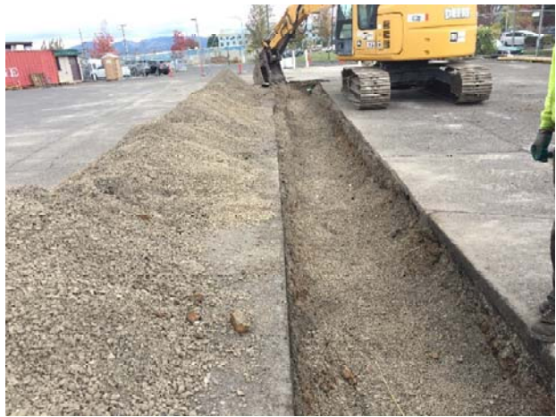
5. Fuel line trench, facing northwest from former fuel pump satellite location.
