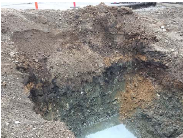
21. Fuel pump satellite pit, east sidewall, and S19 sample location.
