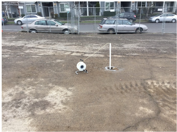
5. B3 temporary well.
