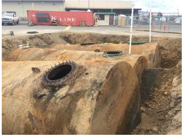
10. Underground storage tanks, facing west.
