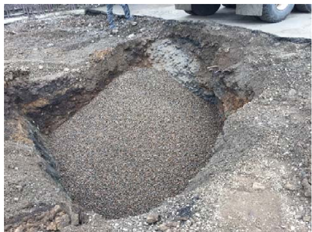
24. Backfilling fuel pump satellite pit.
