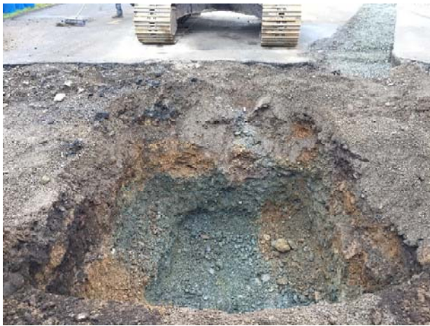
20. Fuel pump satellite pit, west sidewall, and S17 sample location.
