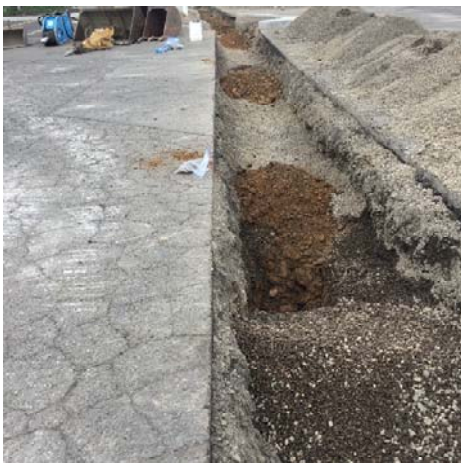
9. S4 through S9 sample locations, along fuel line trench, facing southeast.
