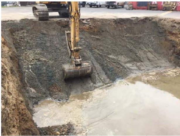
14. Tank pit after tank removal, facing south.
