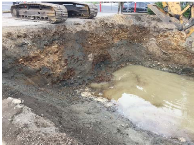
17. Tank pit, facing the west sidewall, and S12 sample location.
