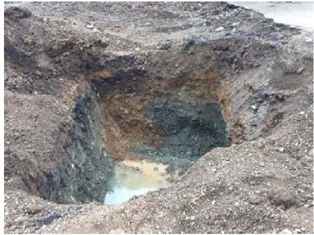
22. Fuel pump satellite pit, south sidewall, and S18 sample location.
