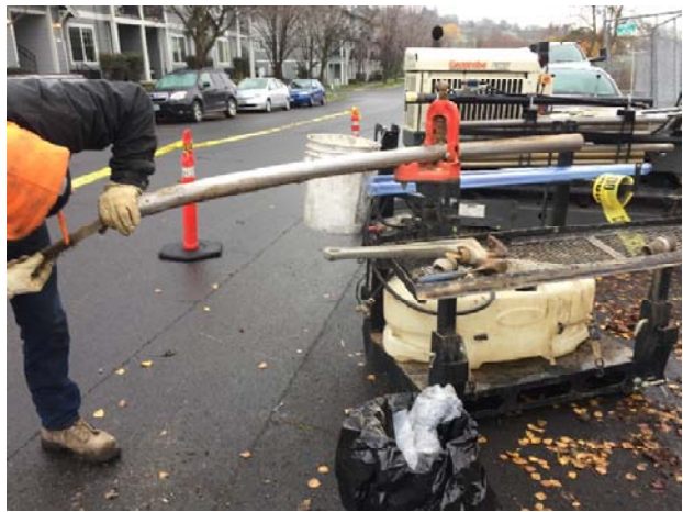
17. Bent drilling road at B4.
