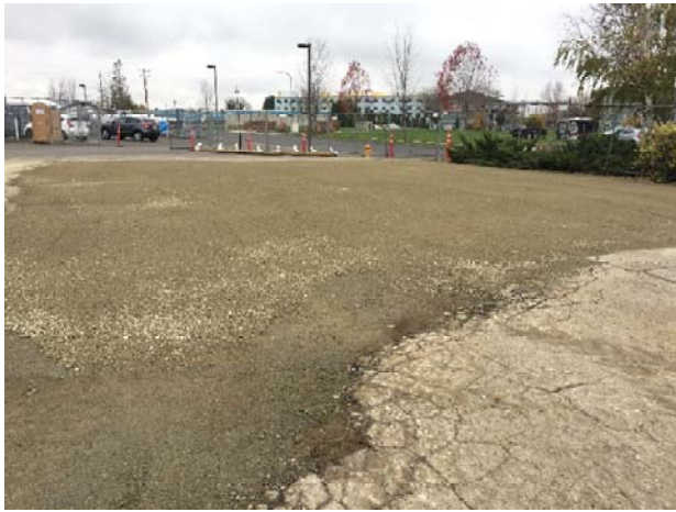
19. Tank pit backfilled.
