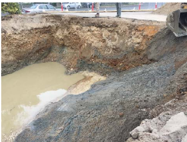
15. Tank pit, facing the east sidewall, and S11 sample location.
