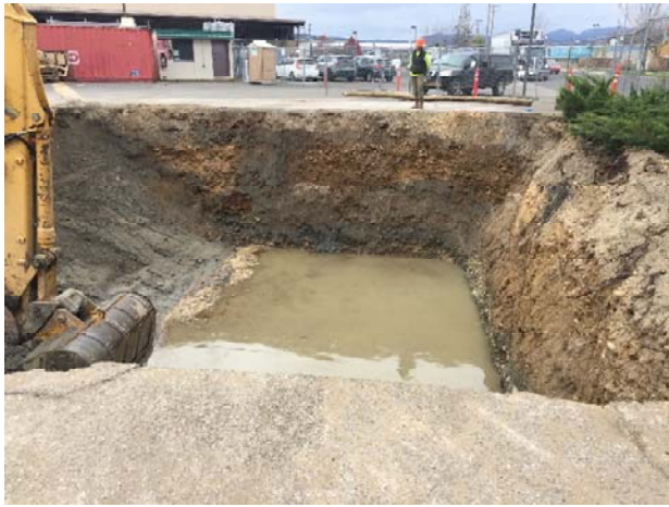
13. Tank pit after tank removal, facing west.
