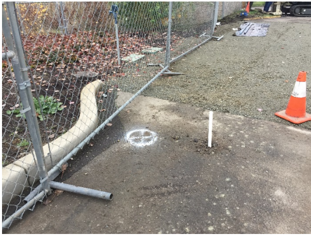
13. B7 temporary well.
