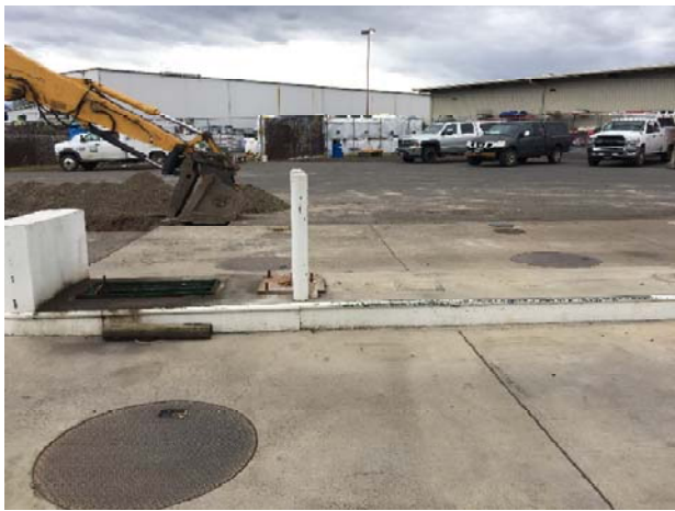
2. Fuel tank pad, facing south, prior to tank removal.
