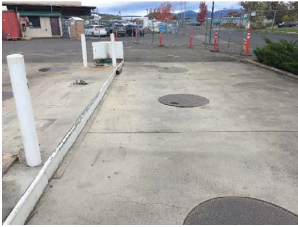
1. Fuel tank pad, facing west, prior to tank removal.
