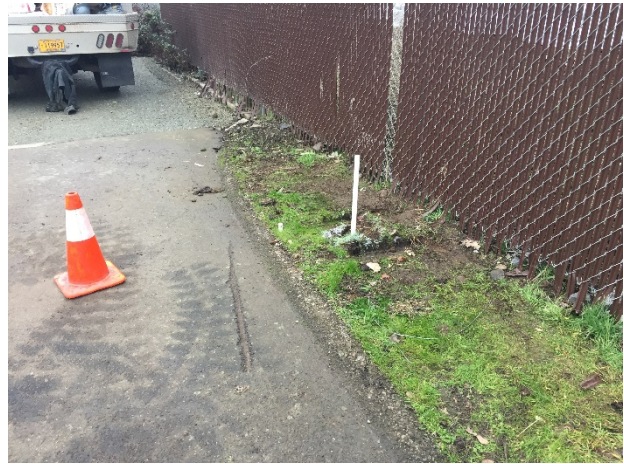
11. B6 temporary well.
