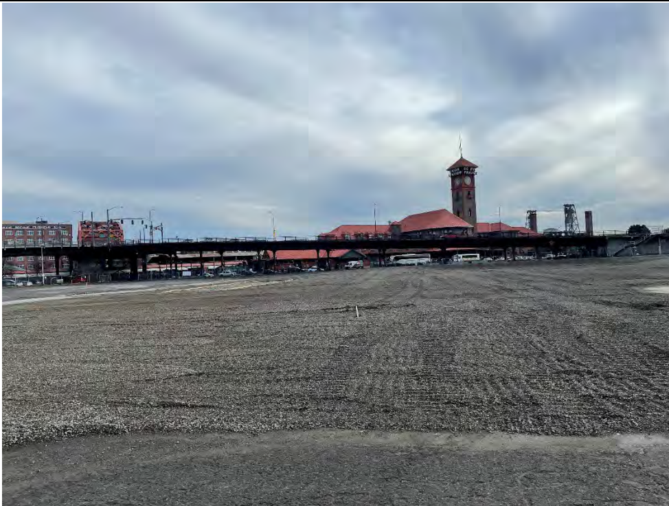
Photo 2: Boring locations at north end of the former building, Looking East.
