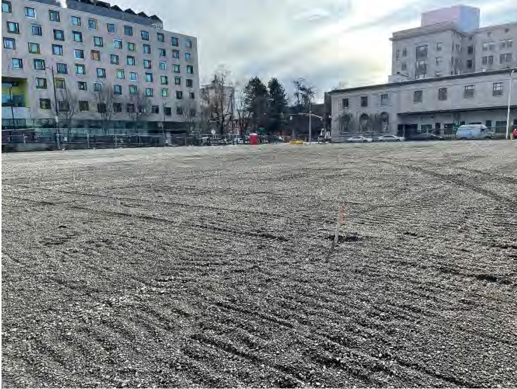
Photo 5: Boring locations at the southeast corner of the former building, Looking Southeast.
