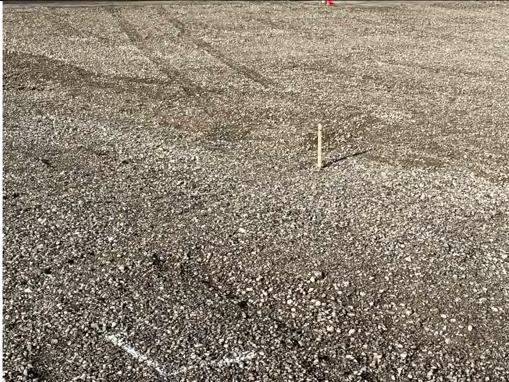
Photo 4: Relocated Boring SB-9 due to mapped deep gravel fill, Looking Northwest.
