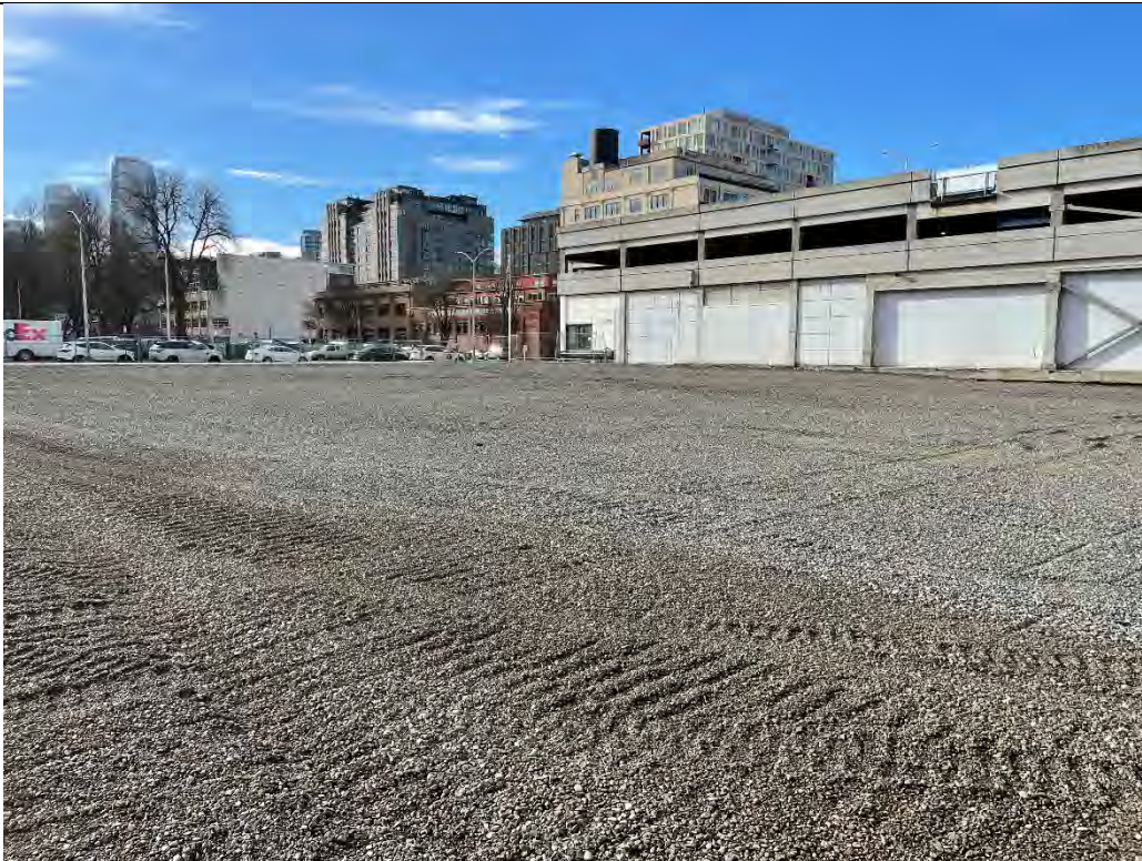
Photo 6: Boring locations at the southwest corner of the former building, Looking Southwest.
