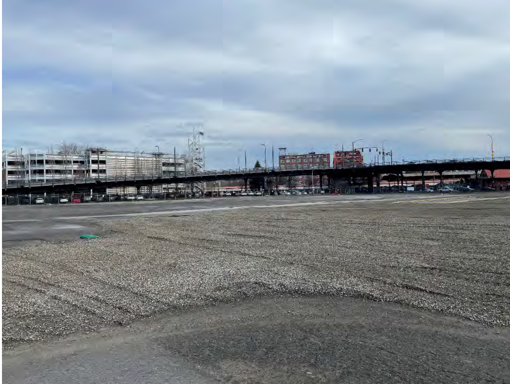
Photo 1: Boring Locations at north end of former building, Looking Northeast.
