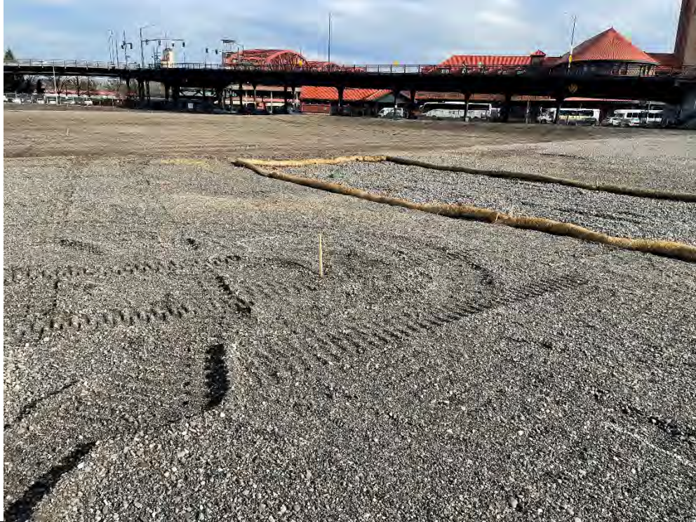
Photo 3: Relocated Boring SB-13 due to unacceptable soil recovery, Looking Northeast.
