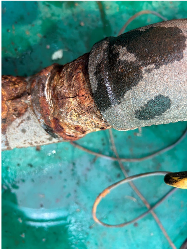
13: Premium sump elbow joint has cracked sealant.
