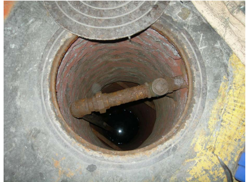
View into possible dry well/cistern.
