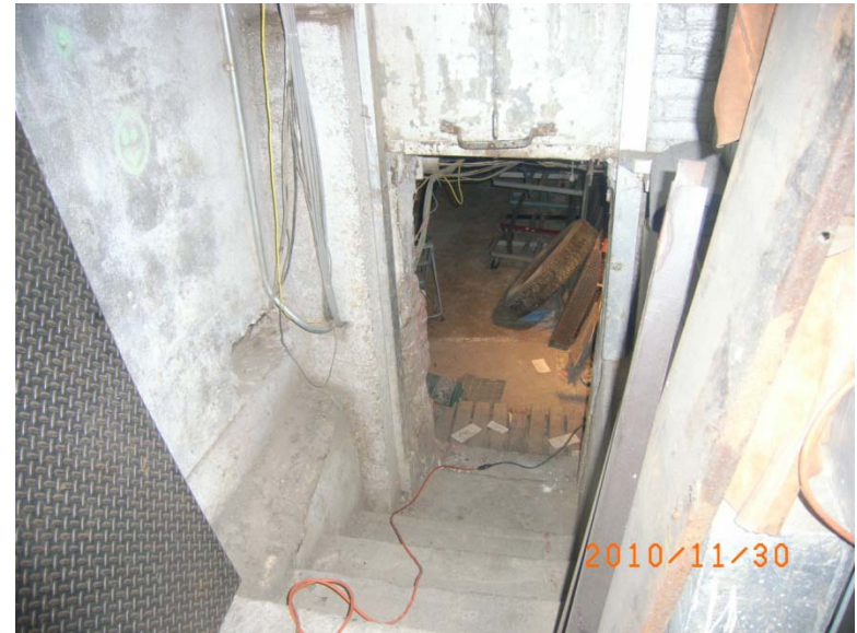
Steps to crawlspace level of facility (southeast portion).
