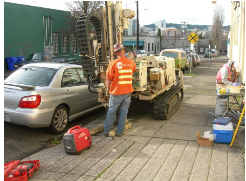
Drilling adjacent to the UST located on the southern portion of the site.
