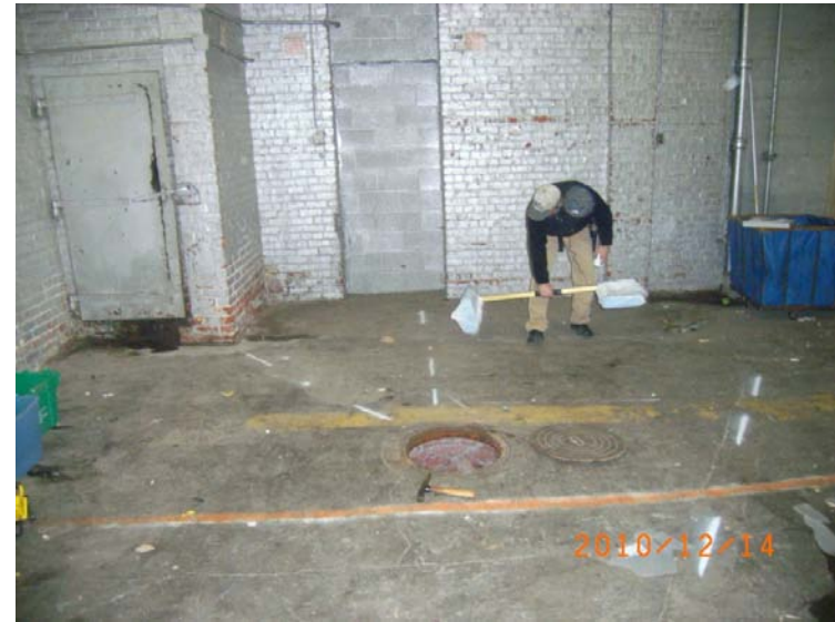
Geophysical clearance around dry well/cistern.
