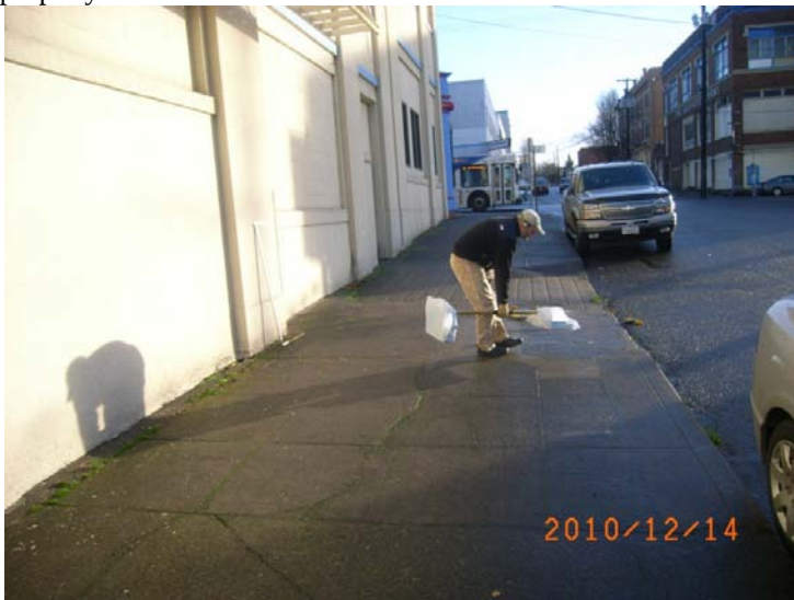
Geophysical clearance for drilling adjacent to the UST.
