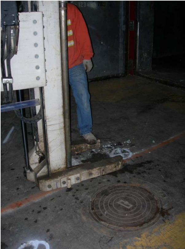
Drilling adjacent to the dry well/cistern.
