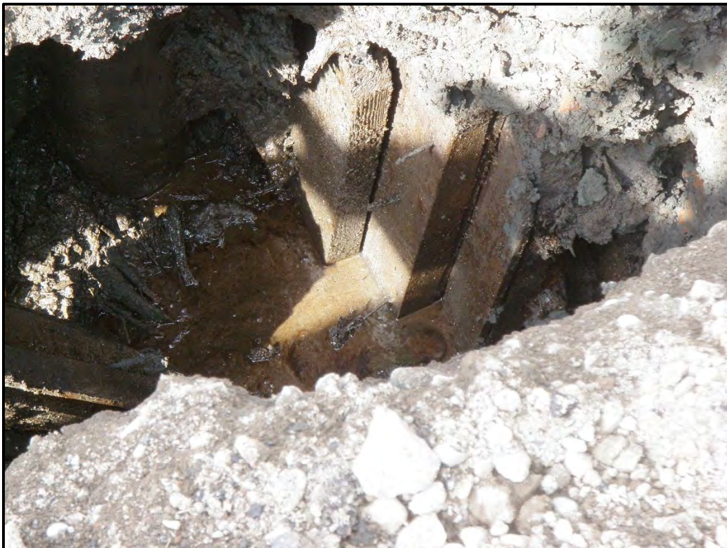
Photograph B-4: In situ condition of cribbing
