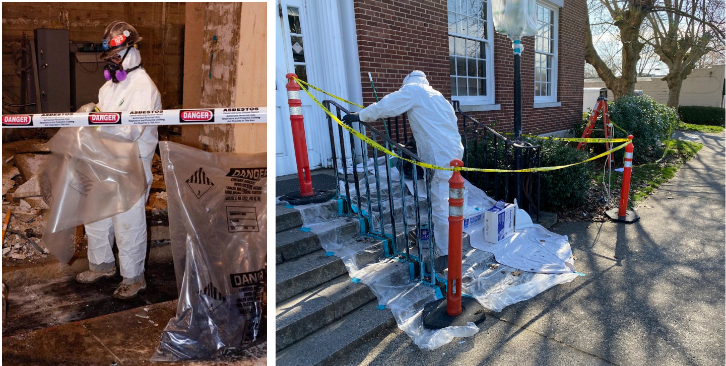
Workers in typical safety equipment for asbestos and lead paint projects. Left photo by Oregon Department of Transportation, 2011.
