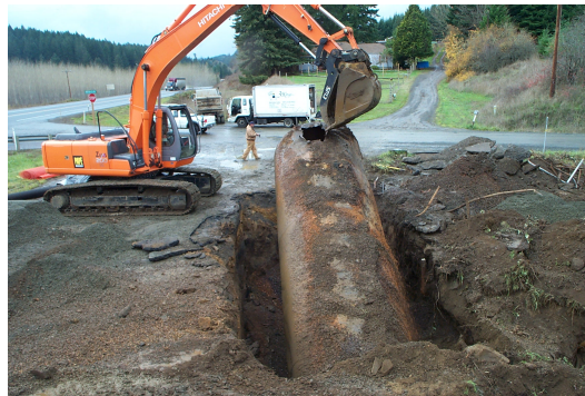
Removal of an underground storage tank prior to subsurface sampling.
