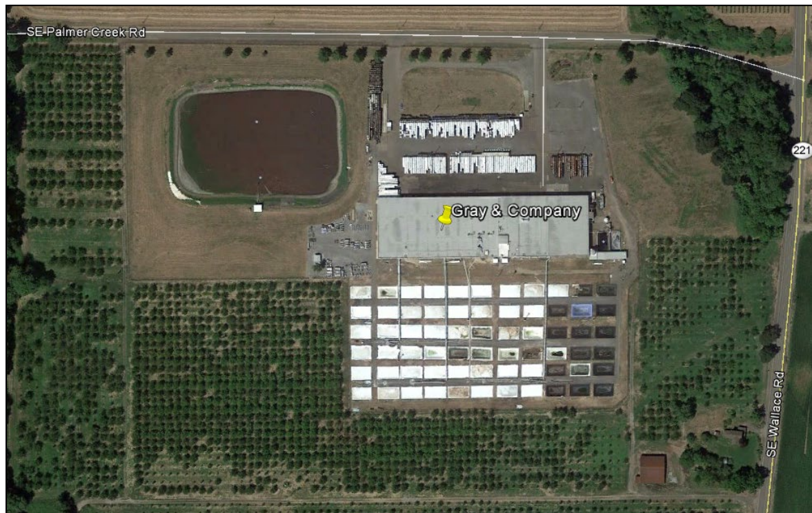
Figure 3-1: Gray and Company – Aerial View
