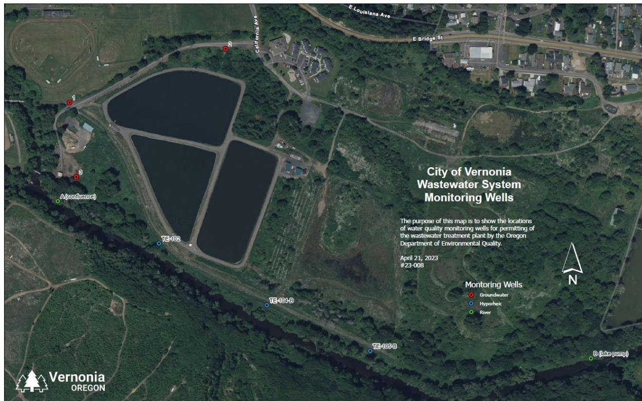
Figure 3-1: Vernonia Monitoring Wells
