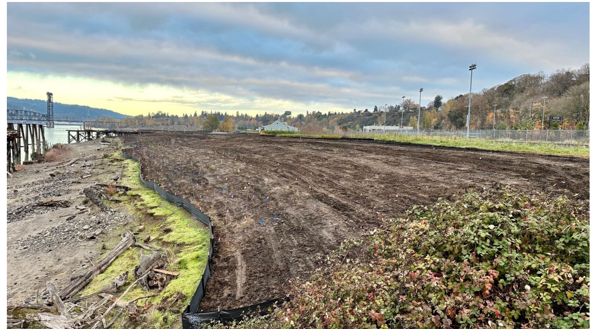
Riparian Restoration, University of Portland Campus
