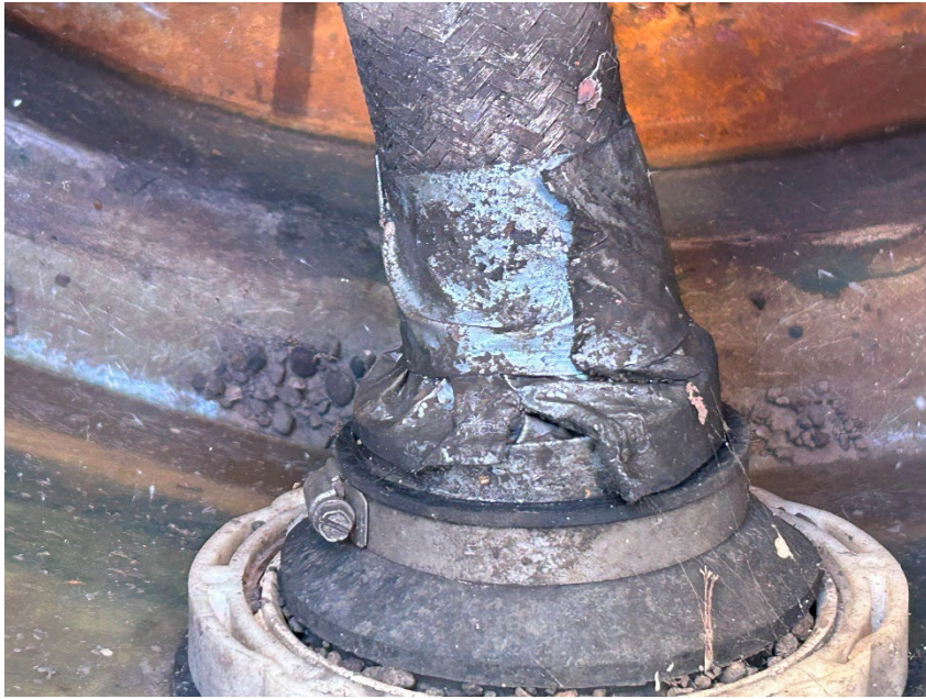
15: Sump #2 – close up of taping
