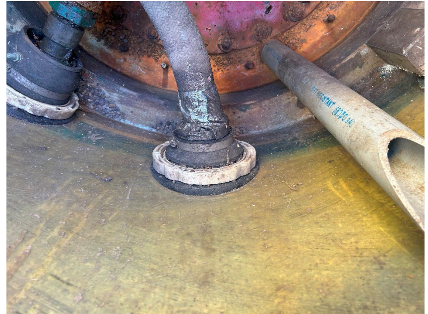
14: Sump #2 – close up of taping
