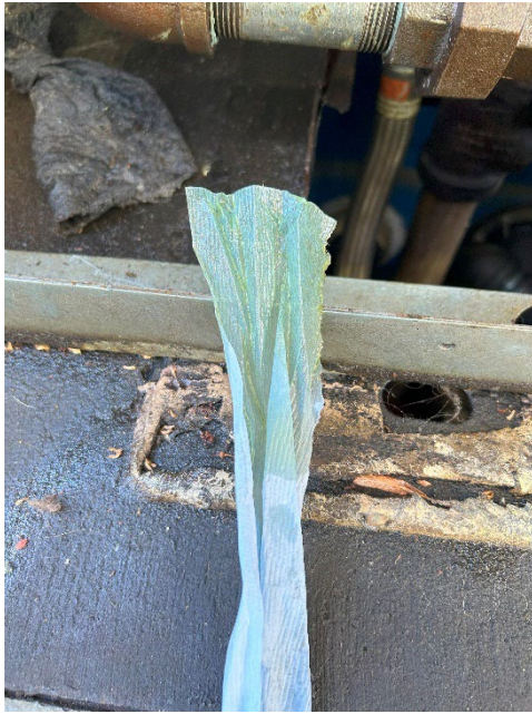
21: Liquid on towel from the bottom of UDC – Dispensers 5 & 6
