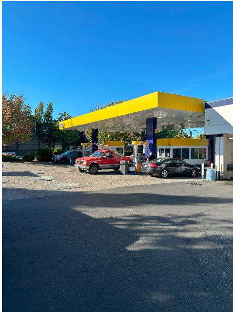
1: East Side of facility
