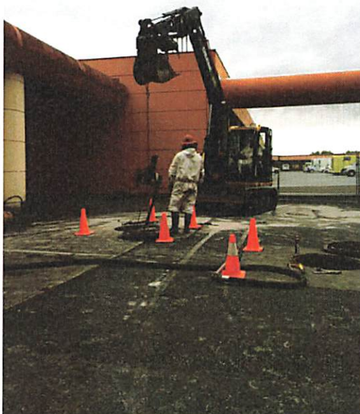
Photo 3. Opening of the manway cover to the diesel UST.
