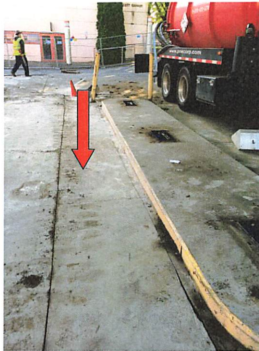
Photo 1. View of the pump island and former dispenser locations. Area of product lines is indicated by arrow.
