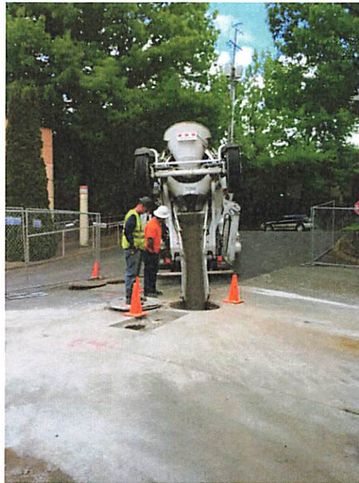
Photo 5. Diesel tank being filled with controlled density fill (CDF).
