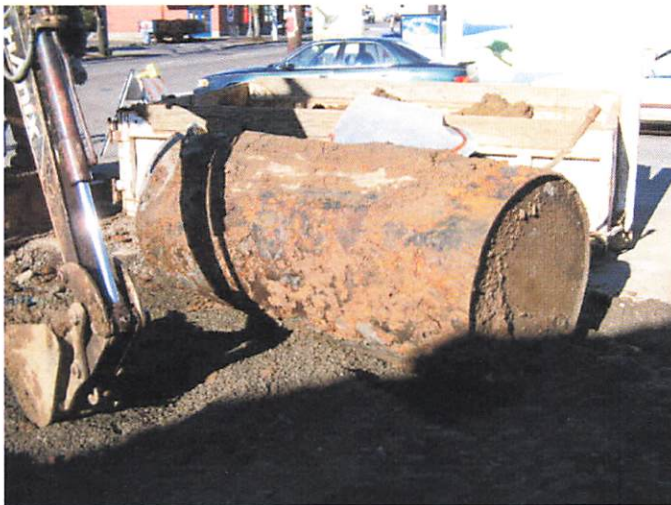
Ladd Inn tank 3 removed
