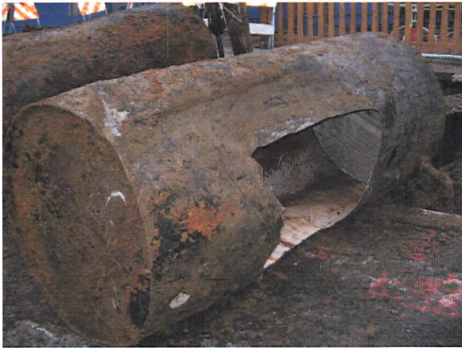
Ladd Inn tanks West and East removed
