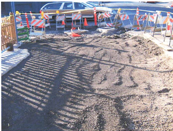
Ladd Inn backfilled excavation
