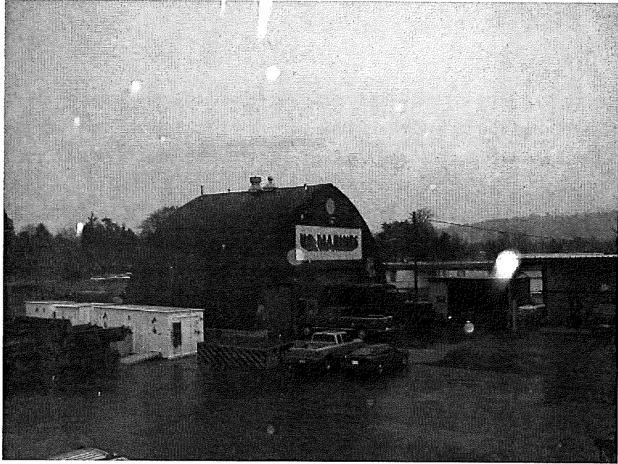
Figure 1: Bldg 6, Maintenance Barn (Former Gun Shed), NW Side
