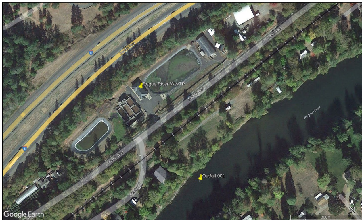
Figure 2-1: Rogue River WWTP Location and Outfall
