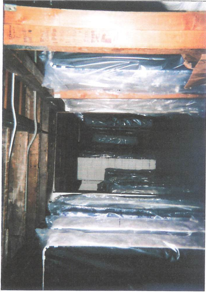
Storage area parallel to showroom area
