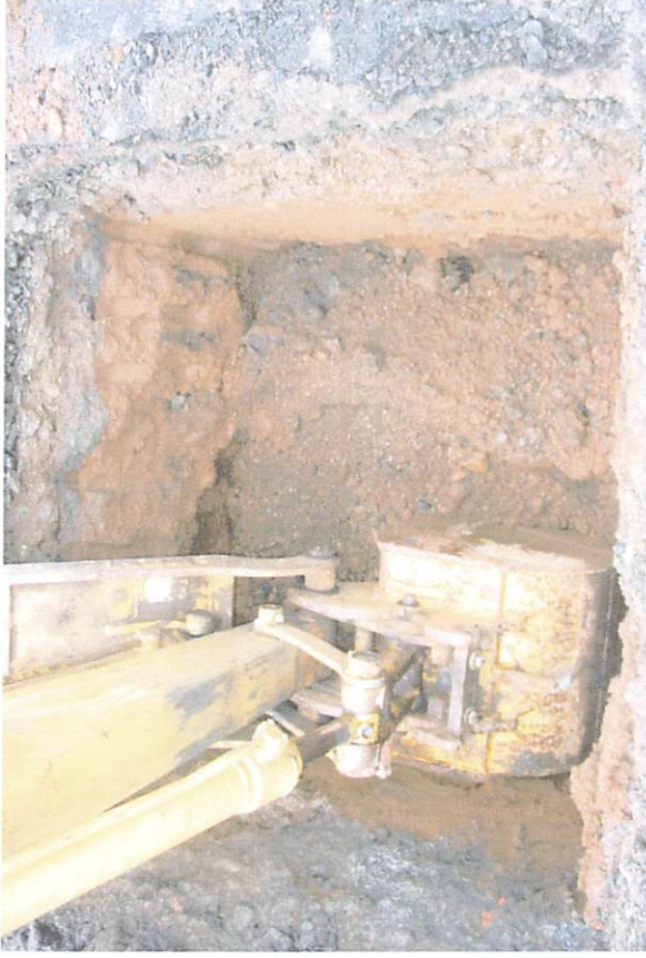
A confirmatory soil sample is collected at a depth of 11.5'
