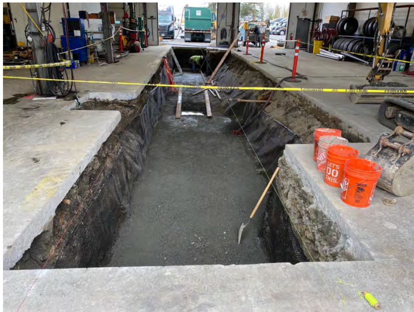
Photo 35. View west of the gravel bedding and geonet placed in the excavation..
