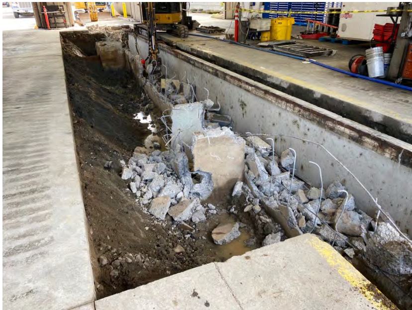
Photo 11. View east of the demolition of the mechanic pit and the west alcove. Note sloped excavation as required by geotechnical assessment.
