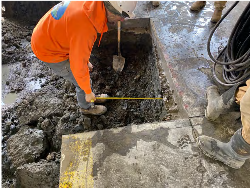
Photo 20. View of probing for the roof column footing to approximate dimensions for structural assessment. Footing was not large enough to support further soil removal to the south of the pit.
