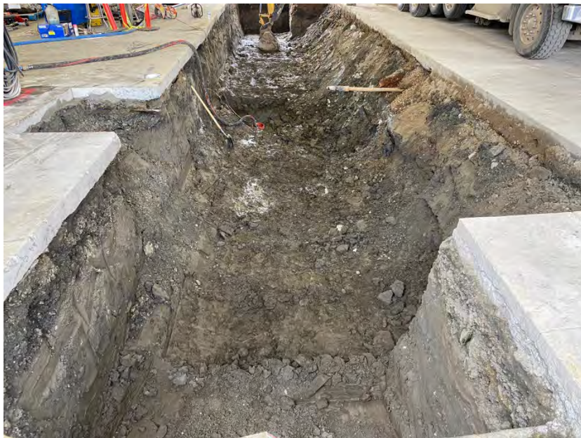
Photo 25. View west of the excavation where the mechanic pit and soil were removed. Note the waste oil pipe, on the right side of the excavation, which will be connected to the new pit alcove.
