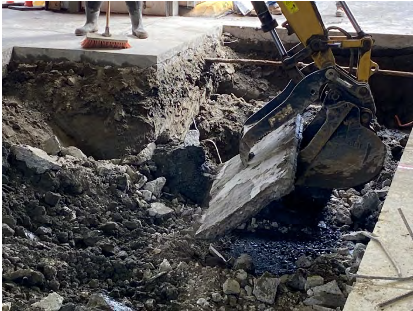
Photo 16. View east of removal of floor at the east end of the mechanic pit. Dark staining is due to release of gear oil in the gravel beneath the pit floor.
