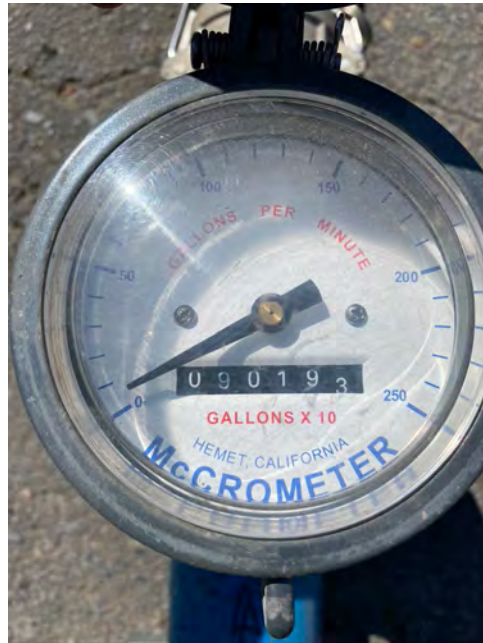
Figure 1. Initial flow meter reading: 090193.
