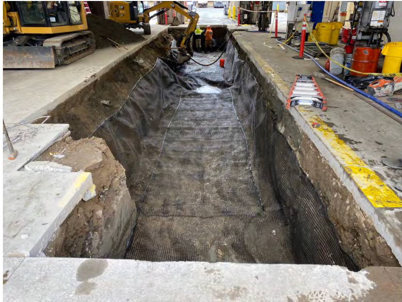
Photo 34. View east of the geonet placed in the excavation prior to rebuilding the mechanic pit.
