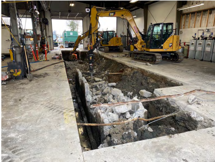
Photo 14. View west of the mechanic pit demolition. In foreground, note the wiring bundle, which was for a former tank monitoring system; the wiring was removed.
