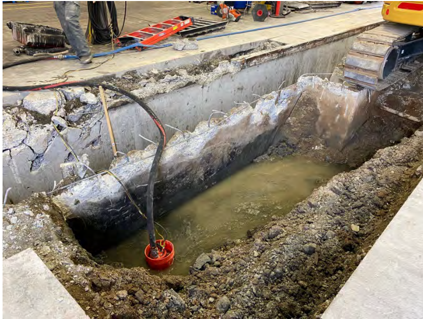
Photo 10. View southwest of the east end of the mechanic pit and east alcove (under the trackhoe). Groundwater seepage was pumped to portable storage tanks. See Photo 28.
