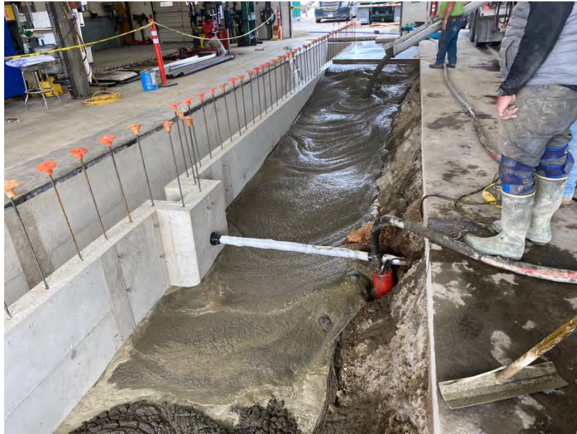
Photo 40. View west of the controlled density fill (CDF) approved for backfill along the north side of the excavation. Note the waste oil pipe connected to the new pit alcove.
