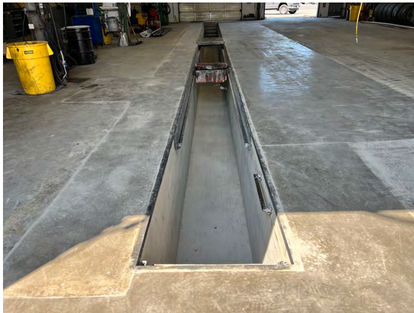
Photo 43. View west of the new mechanic pit.
