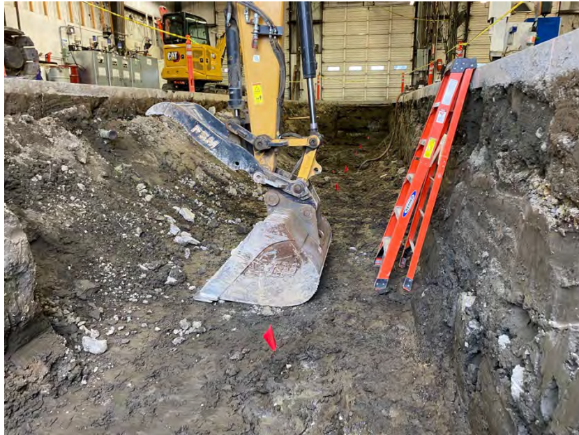
Photo 26. View east of red-flagged locations for the soil grab samples collected from the final excavation bottom. The flag in the foreground identifies the location of Sample G-1.
