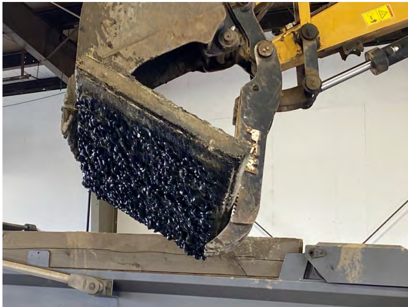
Photo 17. View of a section of concrete floor from the mechanic pit as it is being placed in a dump truck. Note gear-oil stained gravel on the base of the slab.
