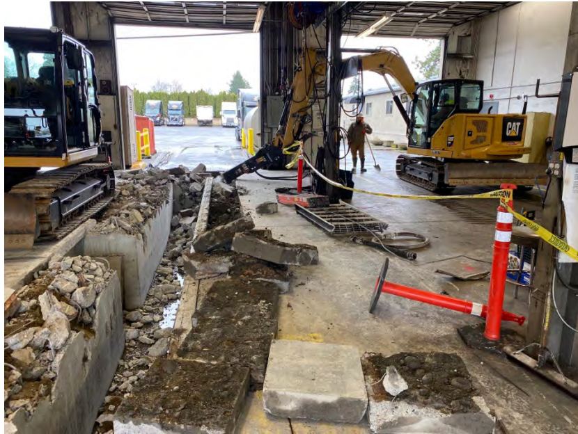
Photo 8. View east of concrete floor removal and initial demolition of the mechanic pit.
