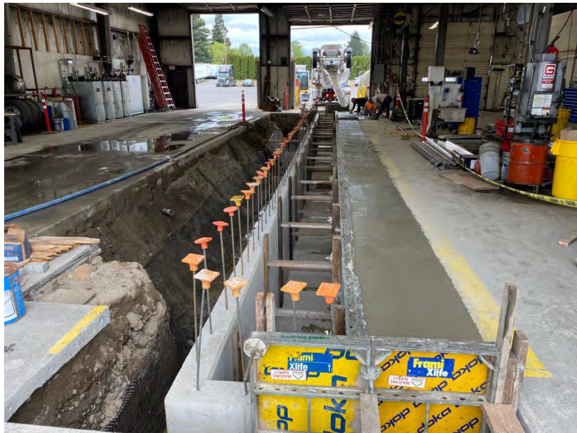
Photo 39. View east of the finished pour of the floor adjacent to the south pit wall.
