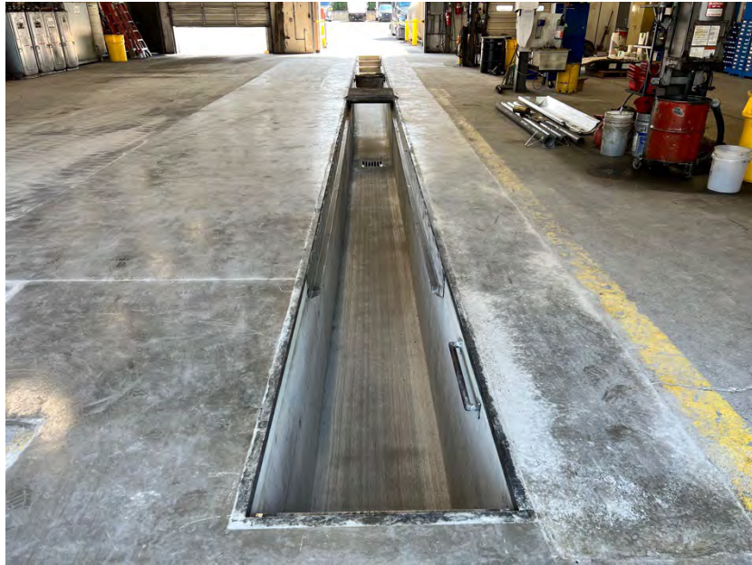
Photo 42. View east of the new mechanic pit.
