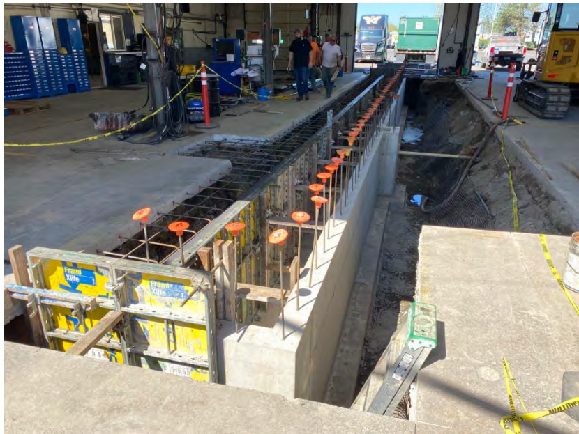
Photo 37. View west of the construction of the new mechanical pit. The north pit wall is in place. The south wall form is in place and ready for a pour.
