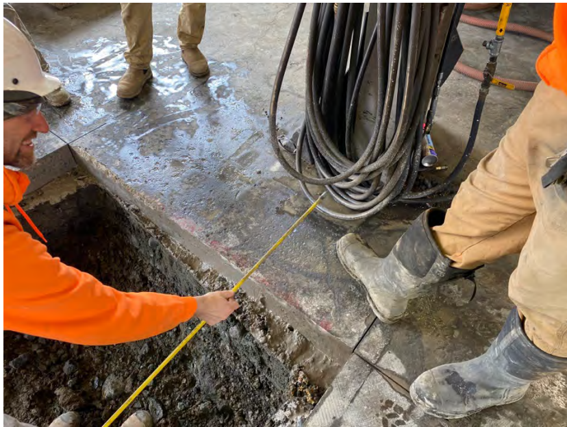
Photo 21. View showing probe length to the roof column footing.
