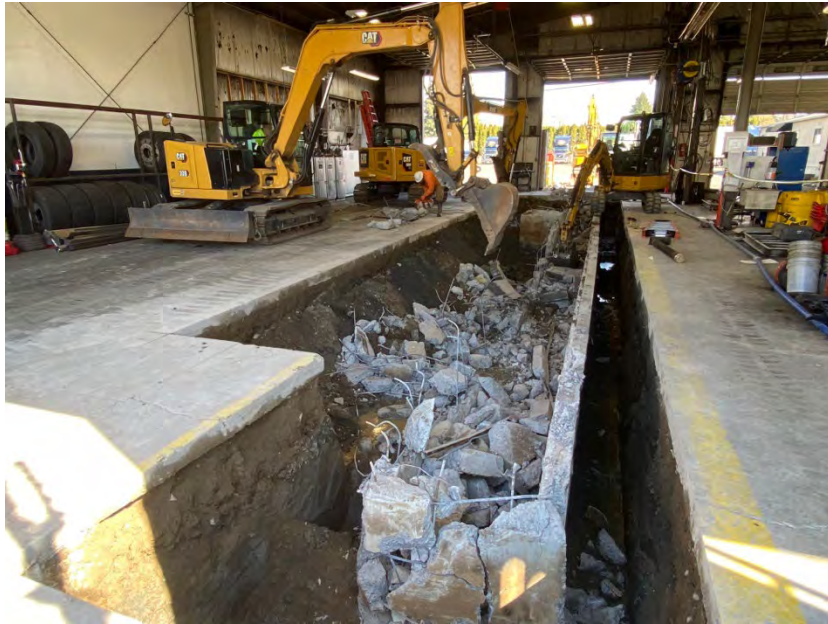
Photo 12. View east of the demolition of the north wall of the mechanic pit.
