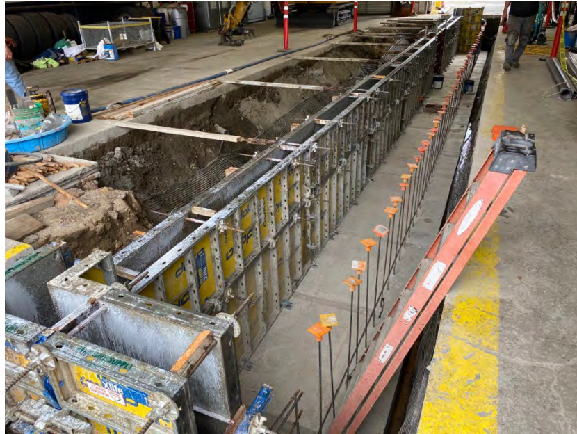
Photo 36. View east of the construction of the new mechanical pit. Forms for the north pit wall are in place.
