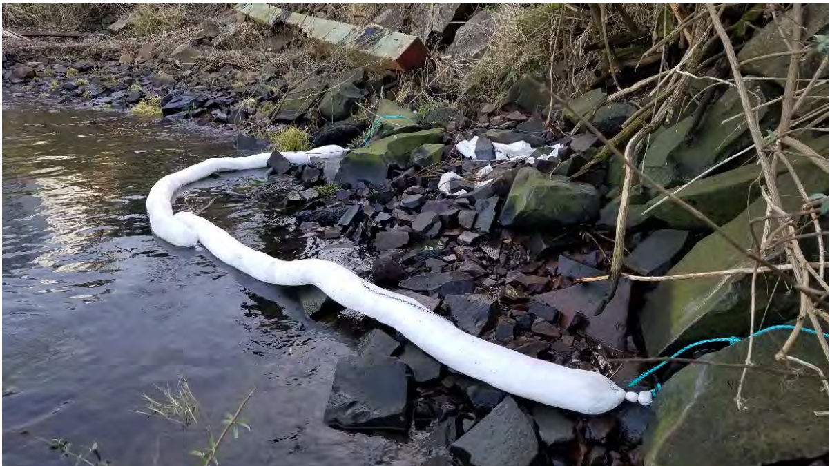
BOOM INSTALLED AT STORMWATER OUTFALL PIPE. PHOTOGRAPH TAKEN MARCH 2, 2021, FACING SOUTH.
