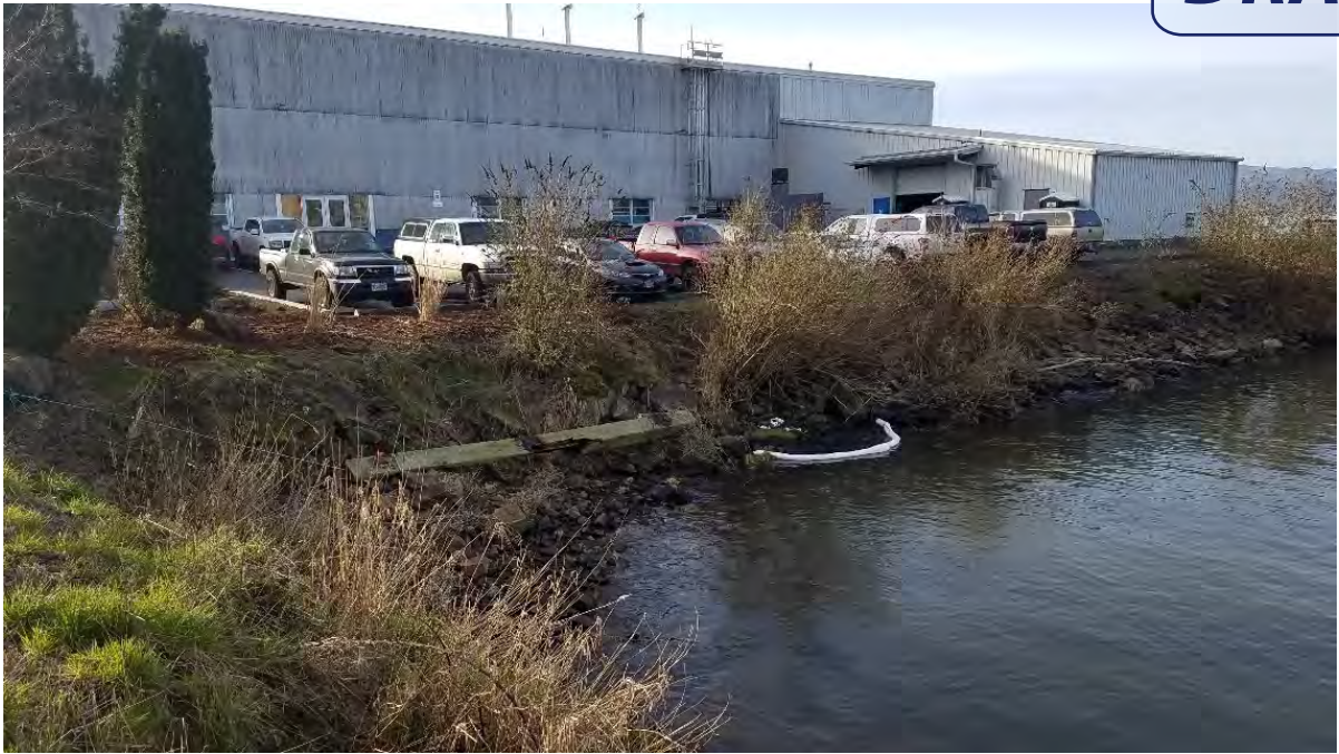
BOOM INSTALLED AT STORMWATER OUTFALL PIPE. PHOTOGRAPH TAKEN MARCH 2, 2021, FACING NORTHWEST.
