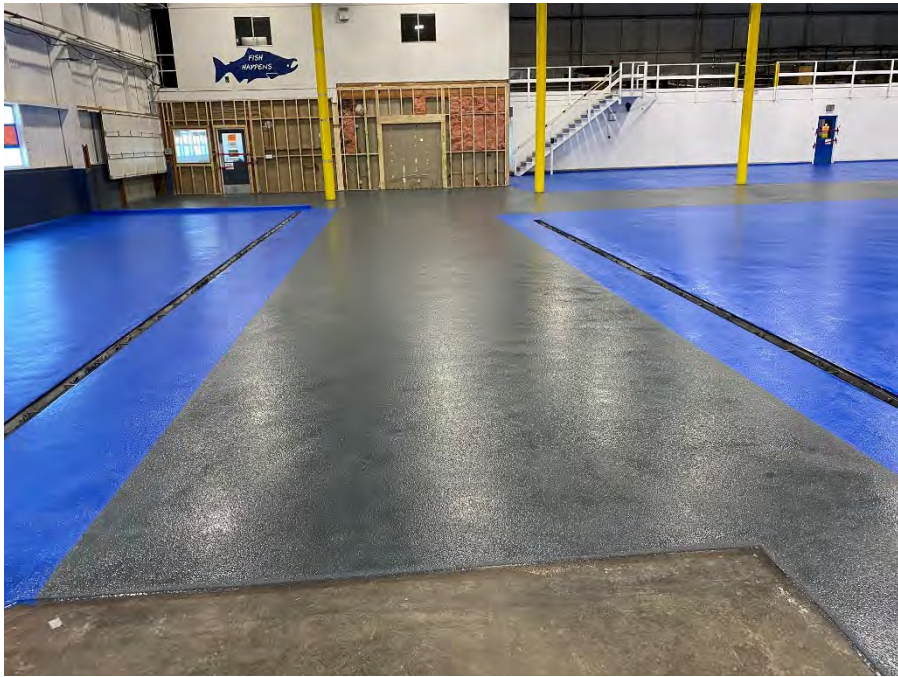
INSTALLING EPOXY IN THE EAST PORTION OF THE FORMER CAN MANUFACTURING WAREHOUSE.
