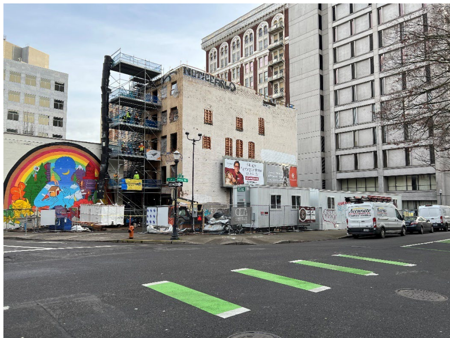
Photo 2. The same view of the Site from January 2022. The Site is being used as a staging area and construction site for a renovation project in the adjacent 333 SW Park Avenue building.
