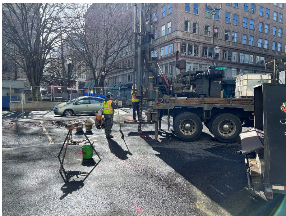
Photo 8. Boring B-8 being completed to the east of B-1.
