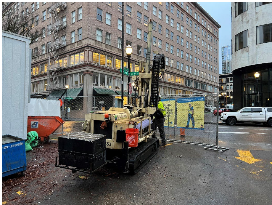
Photo 4. Cascade Drilling completed boring B-1 within the former tank excavation.
