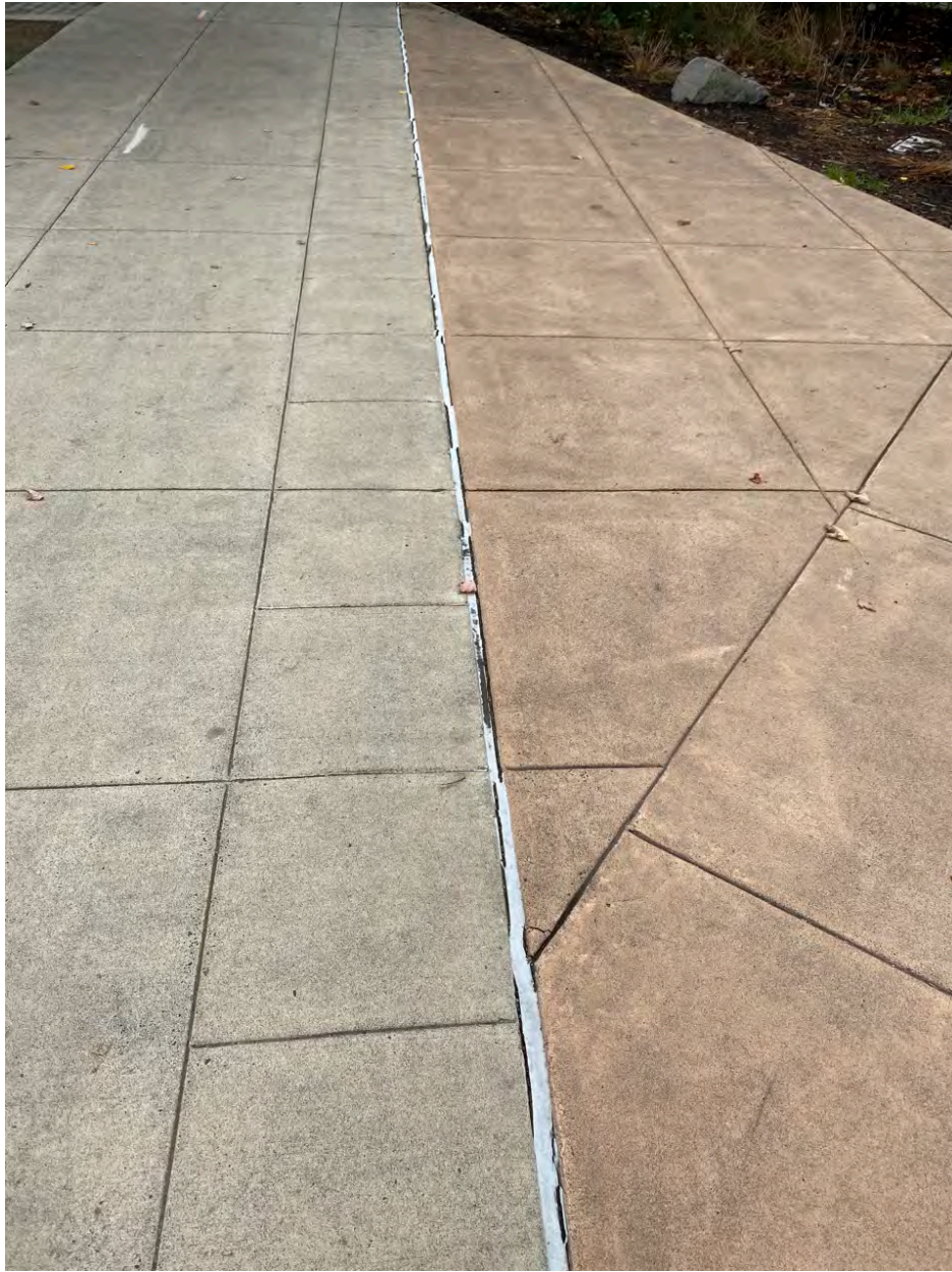
Photo Point 6 – Caulking along seam showing slight separation but in fair condition. No danger to the cap
