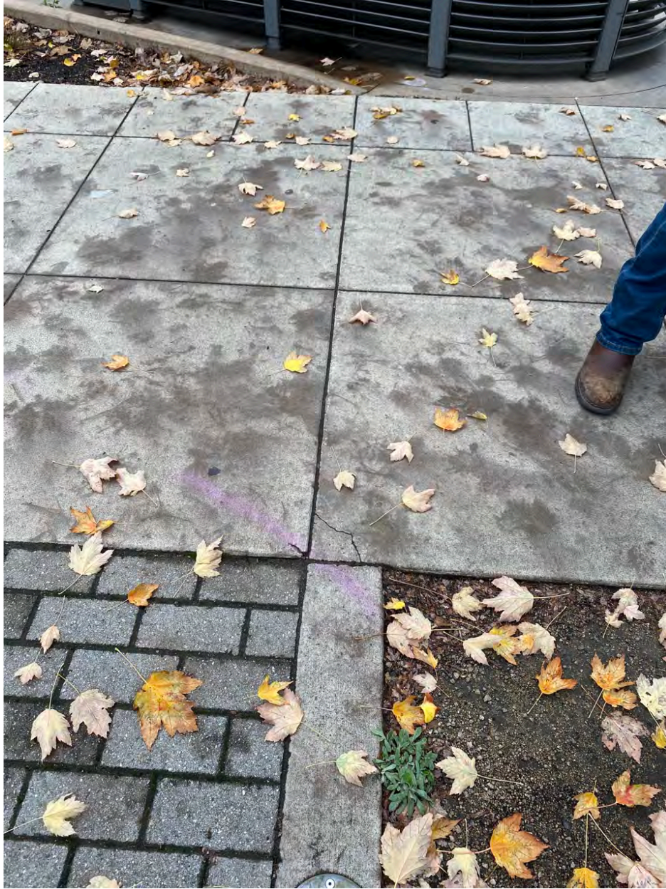
Photo Point 3 – Minor crack in concrete panel near tree well and Portland Loo
