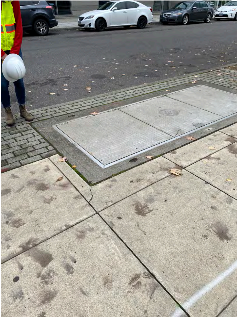
Photo Point 26 – Crack in concrete near vault
