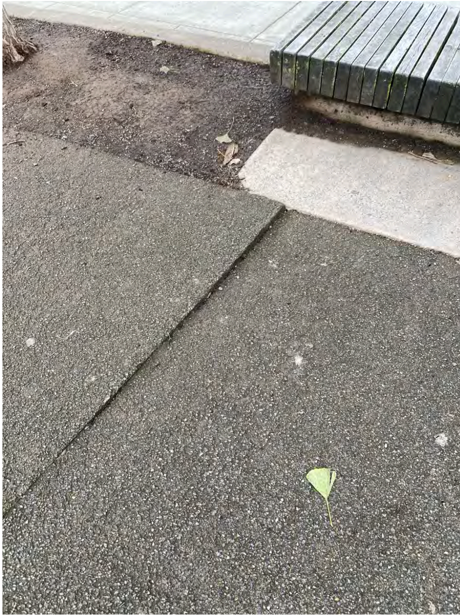
Photo Point 19 – Slight panel uplift along asphalt path
