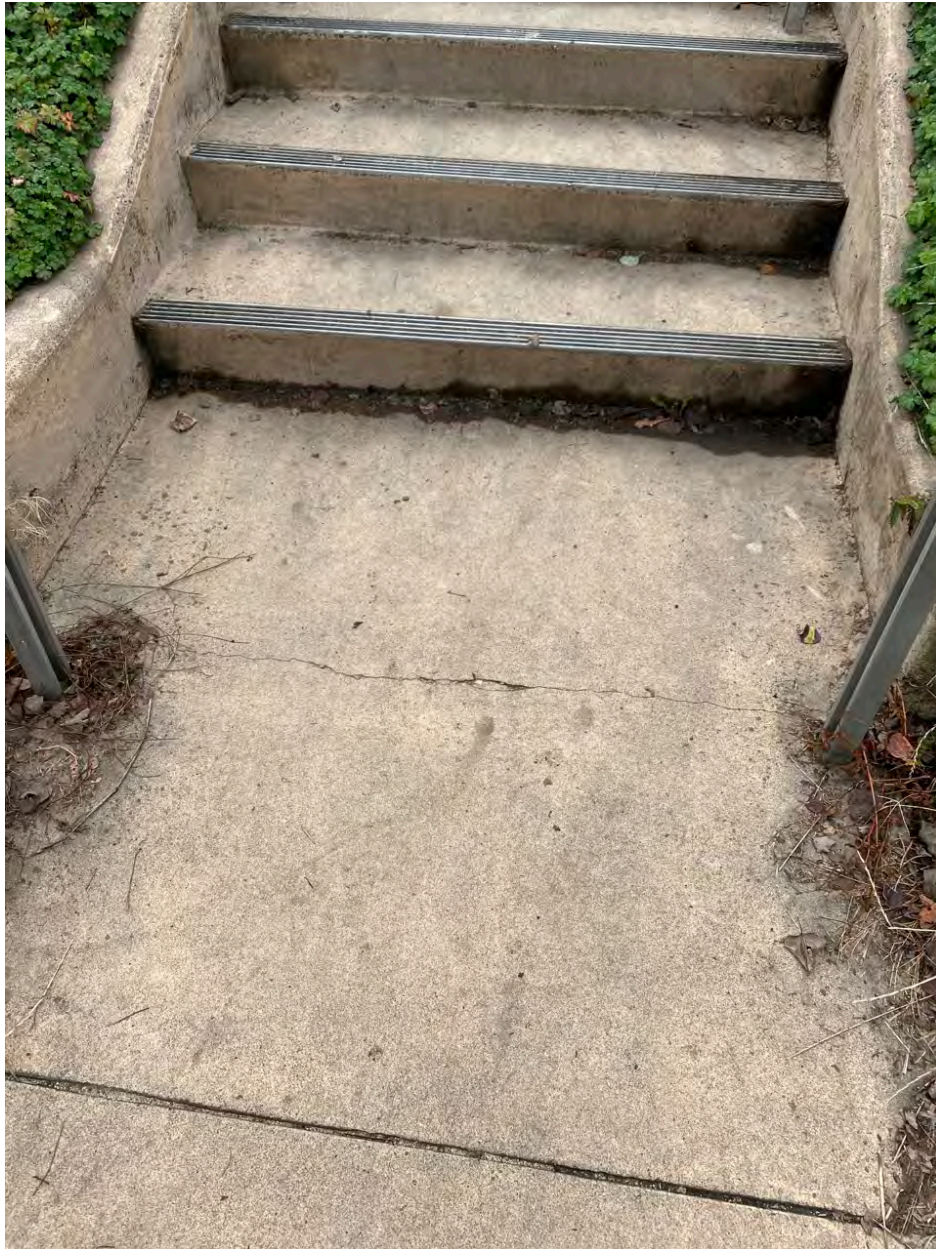
Photo Point 34 – crack in concrete at bottom of stairs looks the same as last year inspection
