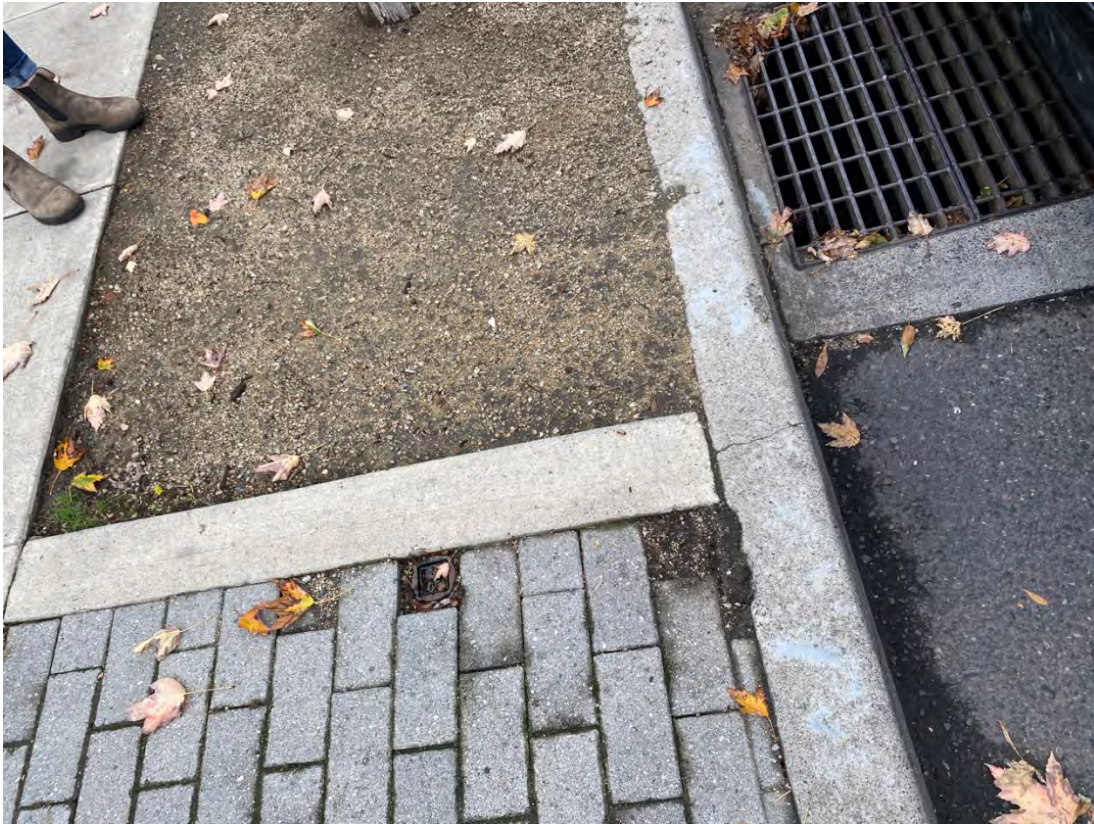
Photo Point 28 – cracks in curb near tree well. No risk to cap.
