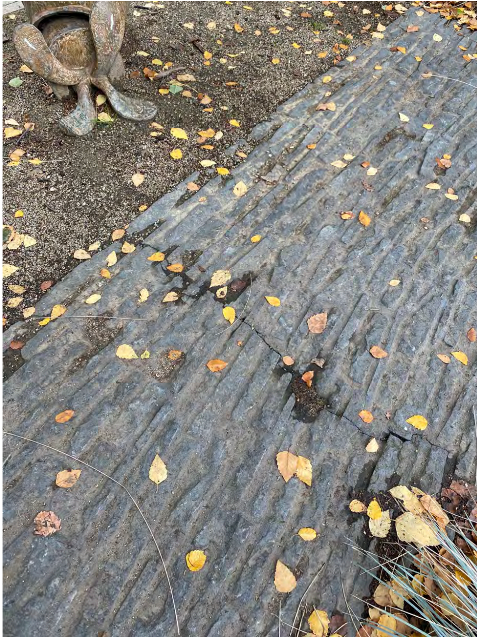
Photo Point 39 – Crack in hardscape side path
