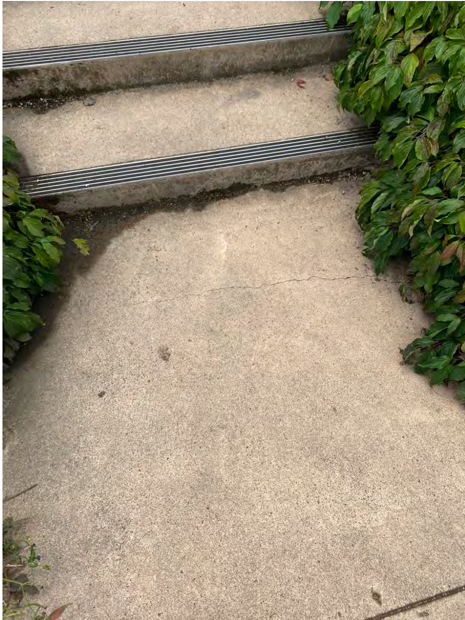
Photo Point 14 – Crack in concrete at bottom of stairs looks the same as last year's inspection
