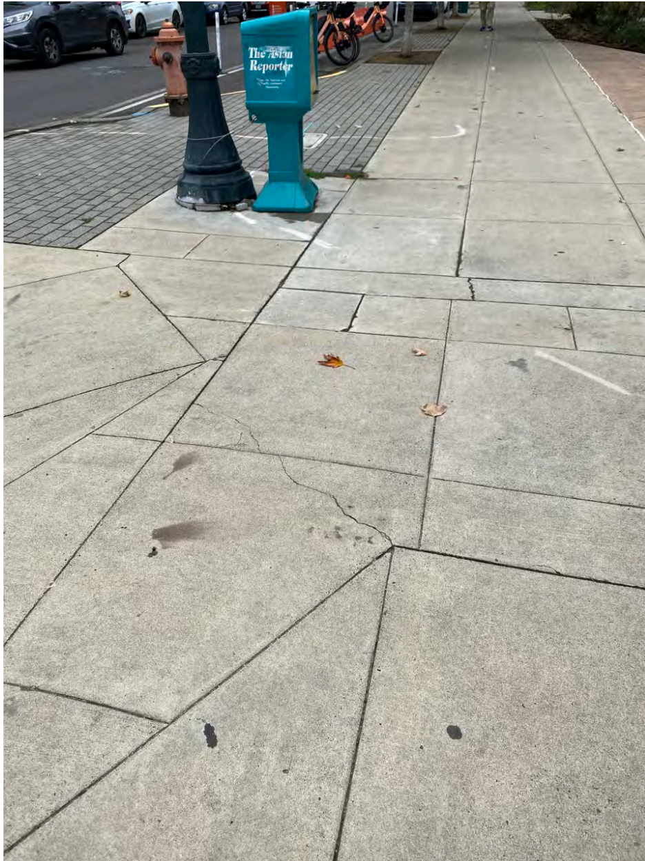
Photo Point 4 – Crack in concrete panel appears the same as last year
