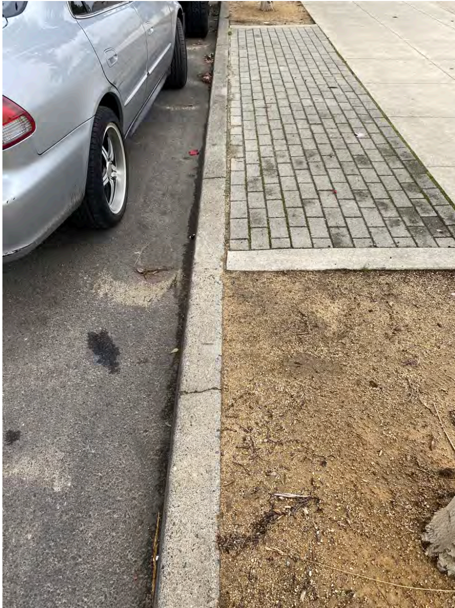
Photo Point 10 – crack in curb, no risk to cap
