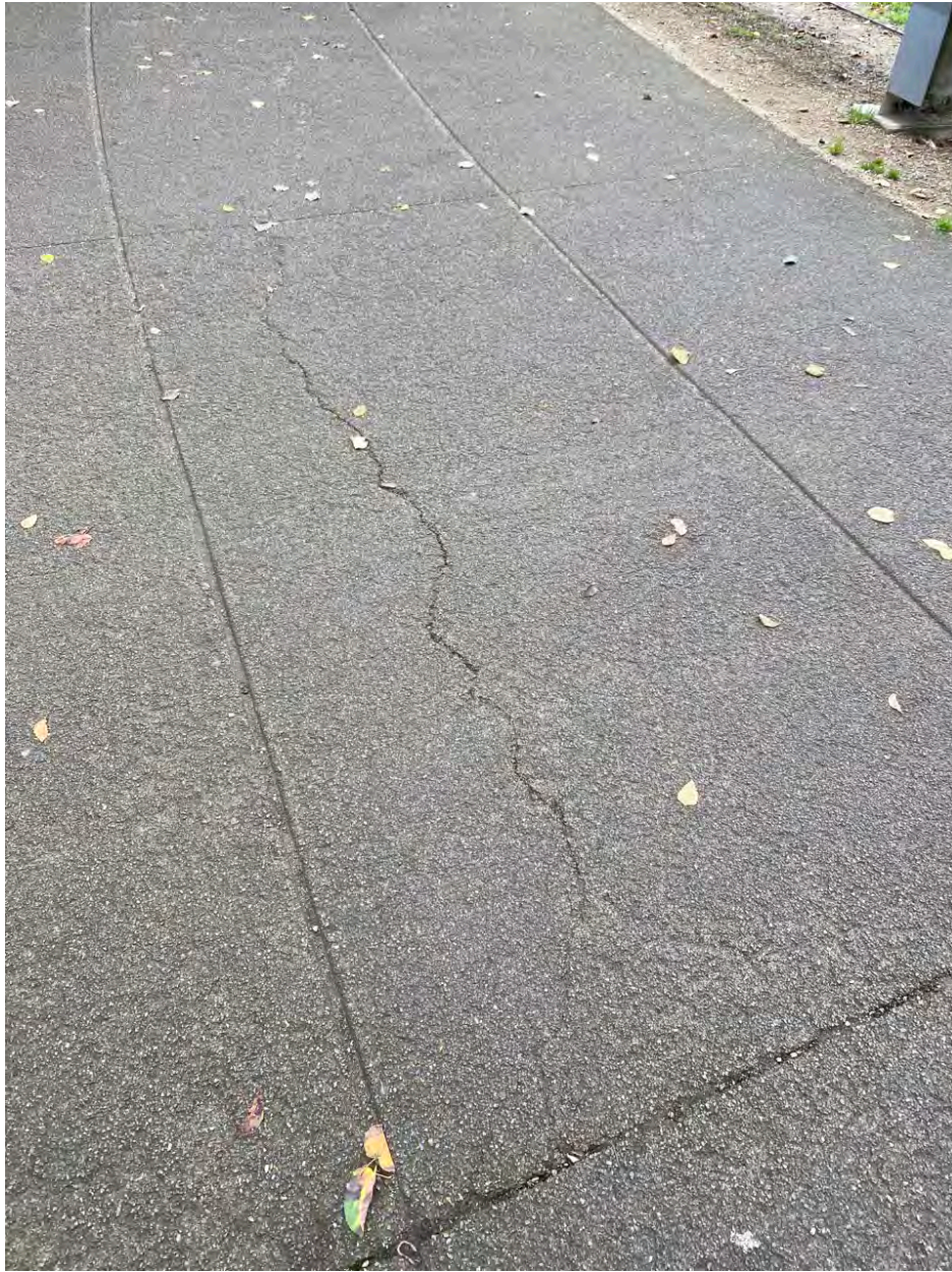
Photo Point 38 – crack in asphalt walkway. Does not penetrate cap.
