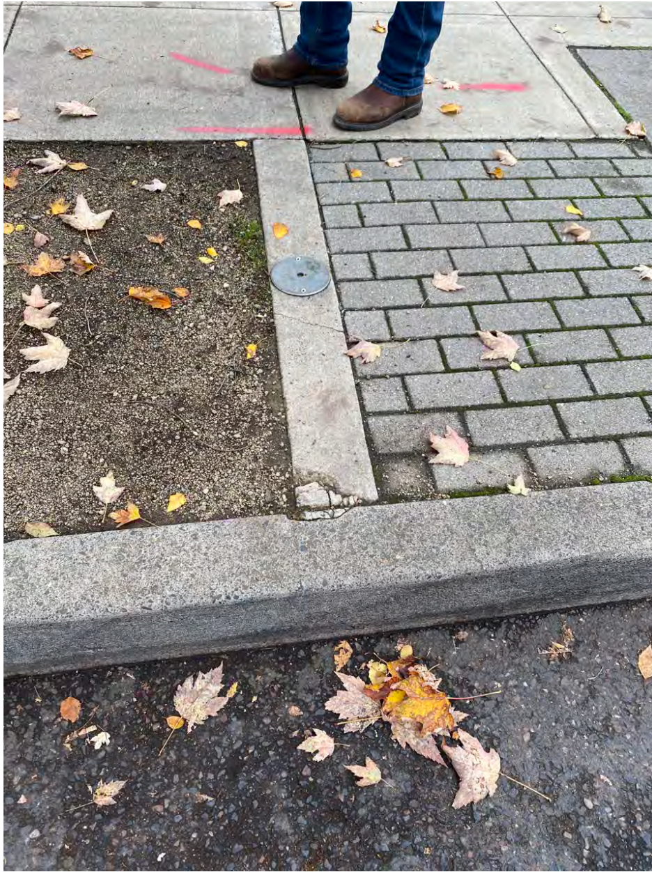
Photo Point 27 – Crack in concrete near curb. No risk to cap.
