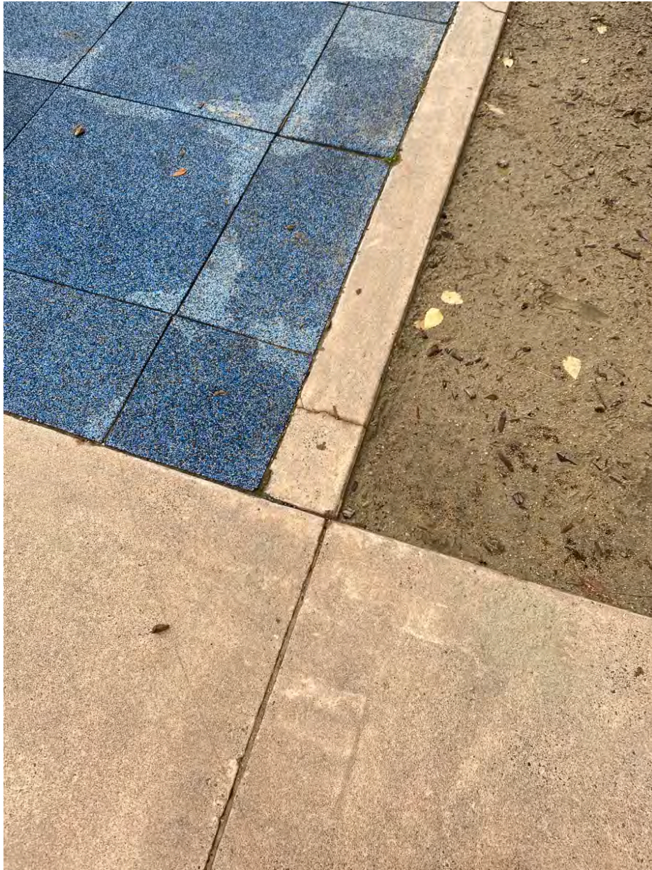
Photo Point 16 – Cracks in cement border in play area. No risk to cap.
