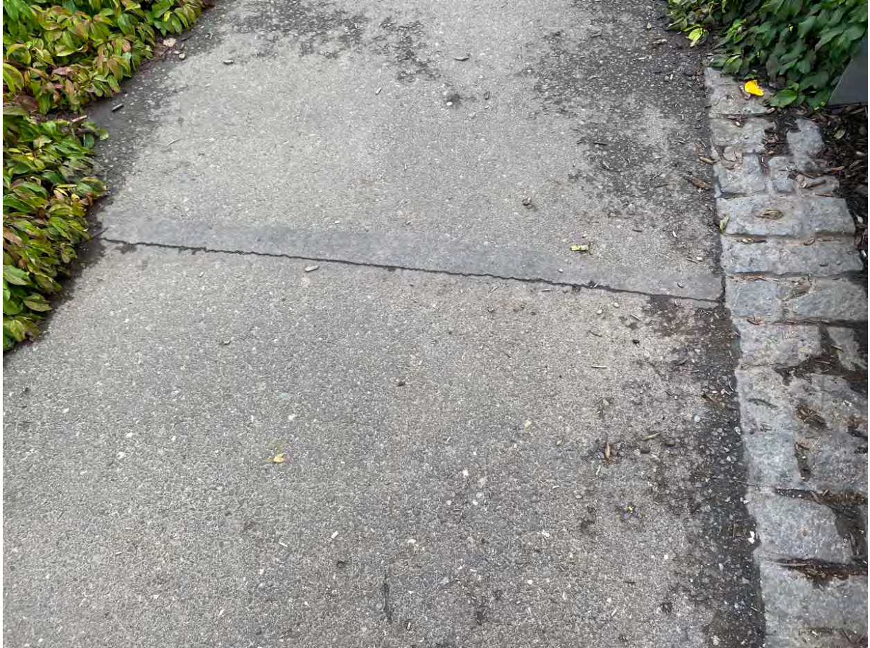
Photo Point 35 – seam appears the same as last year inspection
