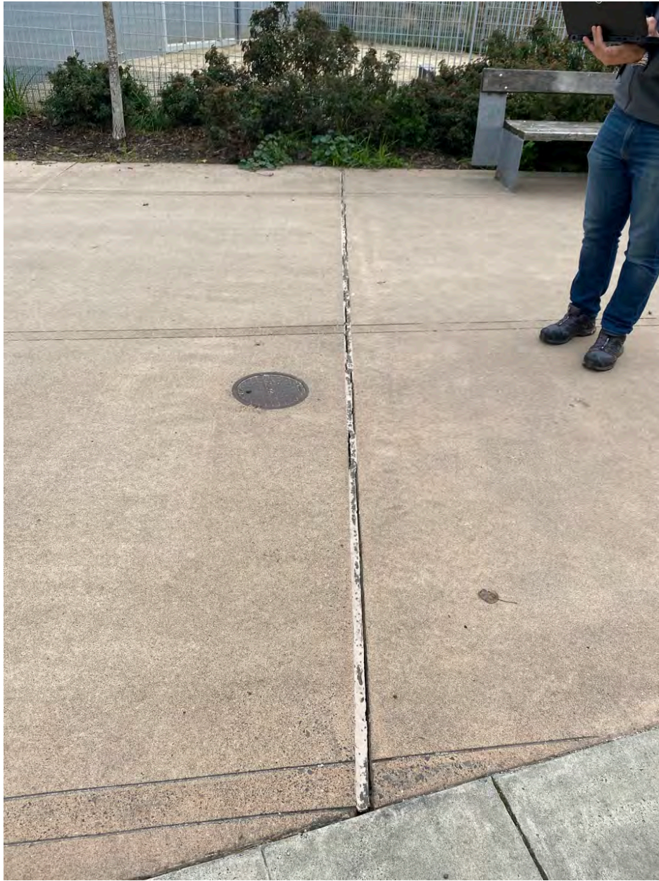
Photo Point 32 – caulking in seam in fair condition, looks the same as last year inspection
