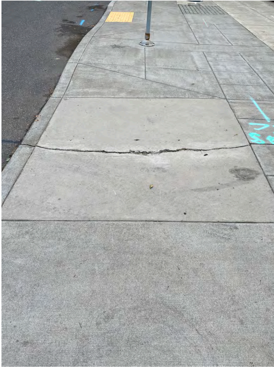
Photo Point 9 – Crack in driveway panel appears the same as last year's inspection
