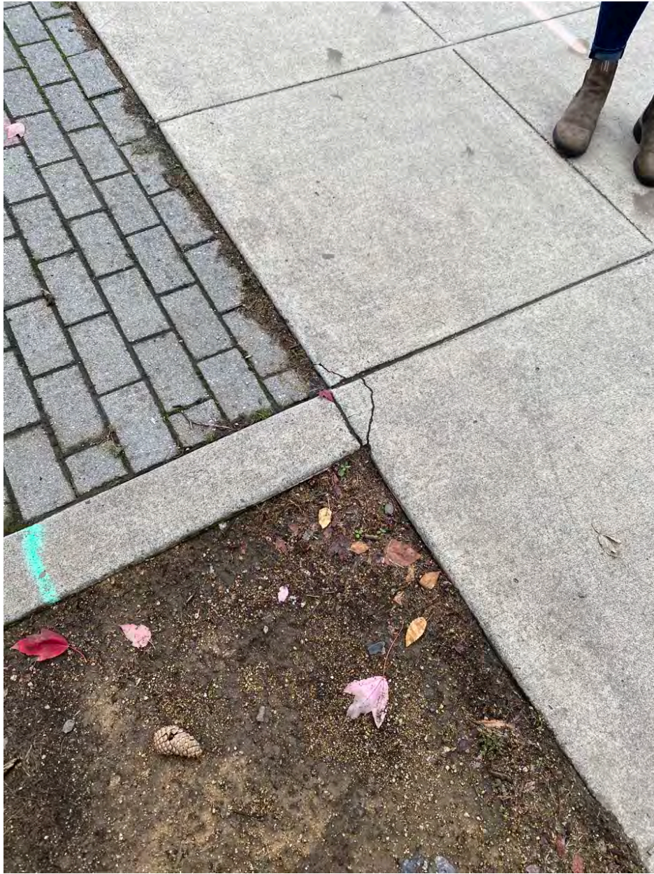
Photo Point 8 – Minor cracks in corners of concrete panels
