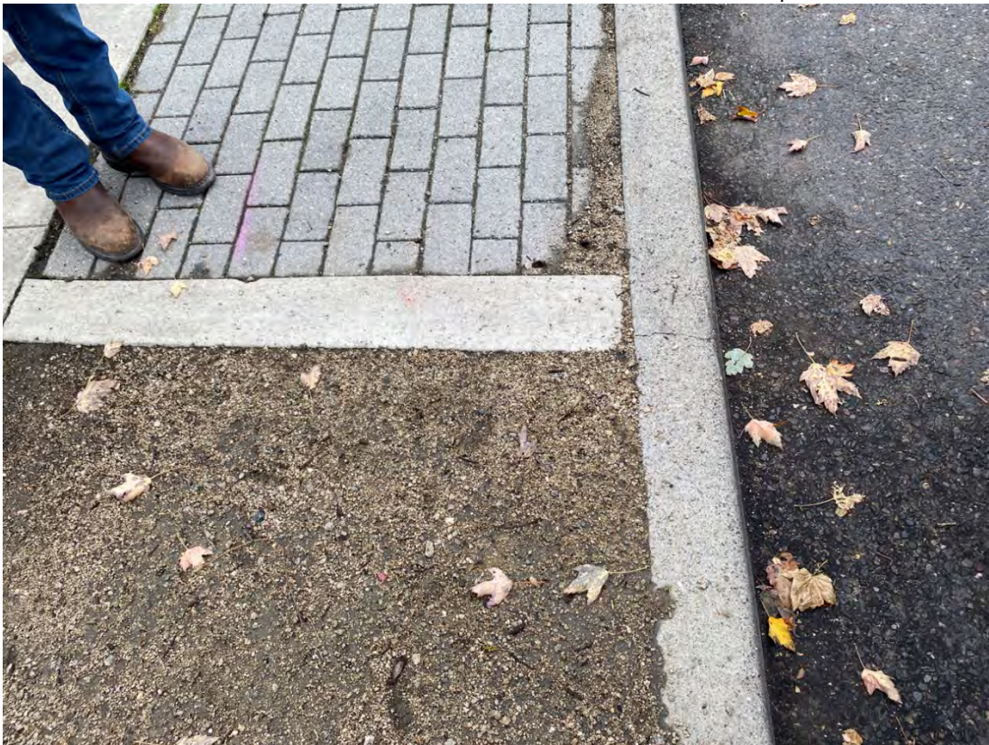
Photo Point 28 – cracks in curb near tree well. No risk to cap.
