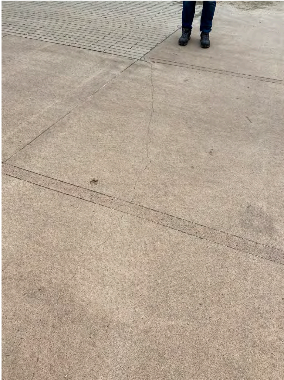
Photo Point 12 – Minor crack in concrete panels, no risk to cap.
