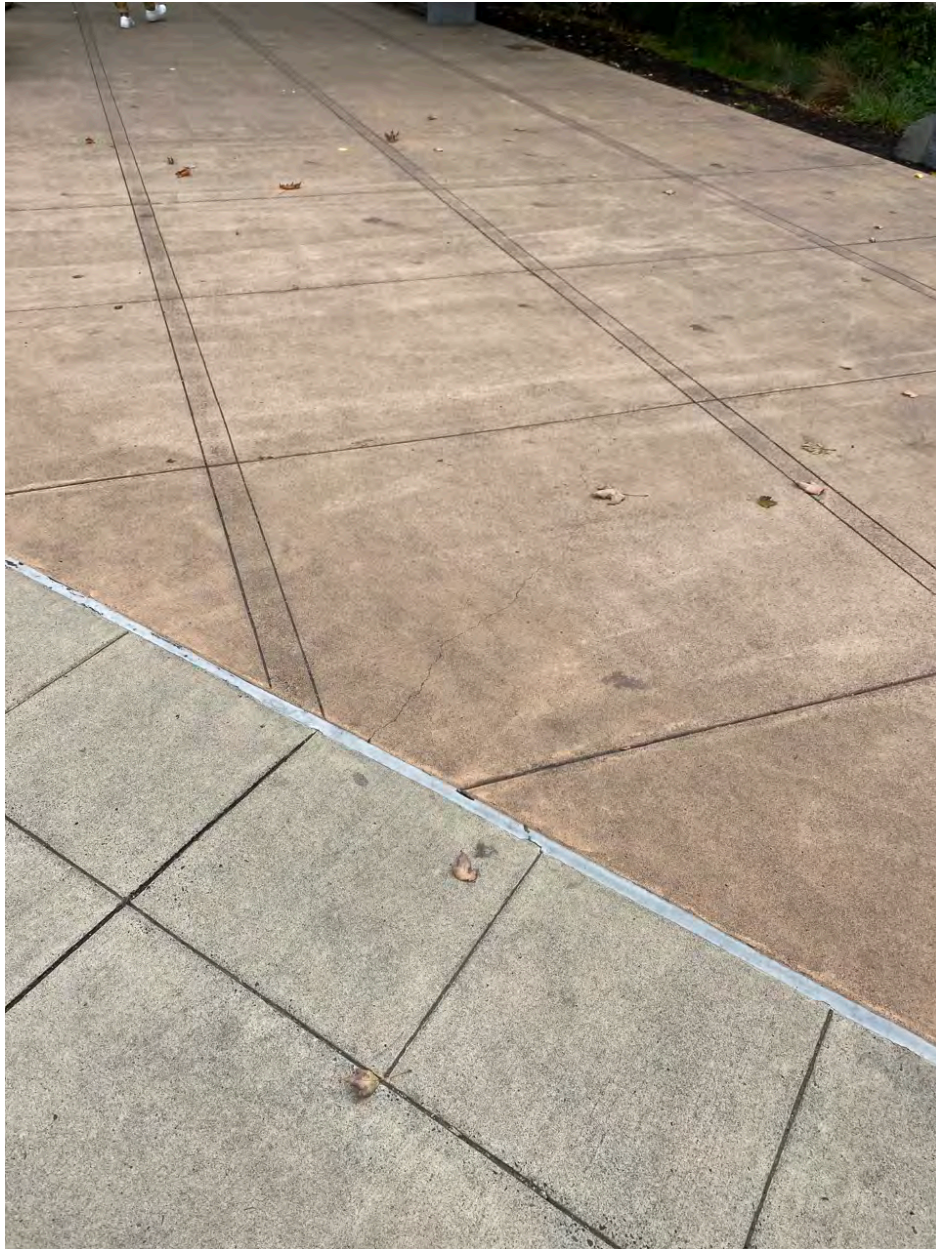
Photo Point 5 – Hairline crack in concrete panel
