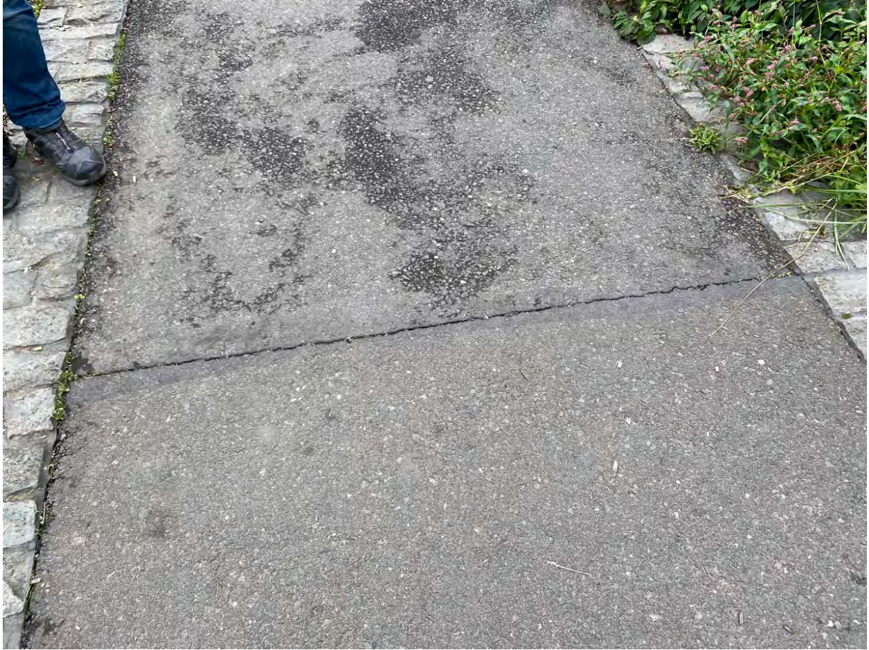
Photo Point 15 – Seams in walkway have not changed since last year's inspection
