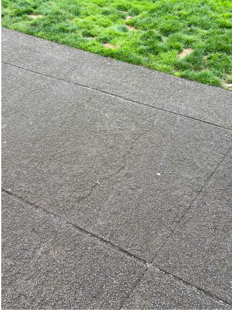
Photo Point 20 - Typical wear/weathering of asphalt path. No risk to cap.
