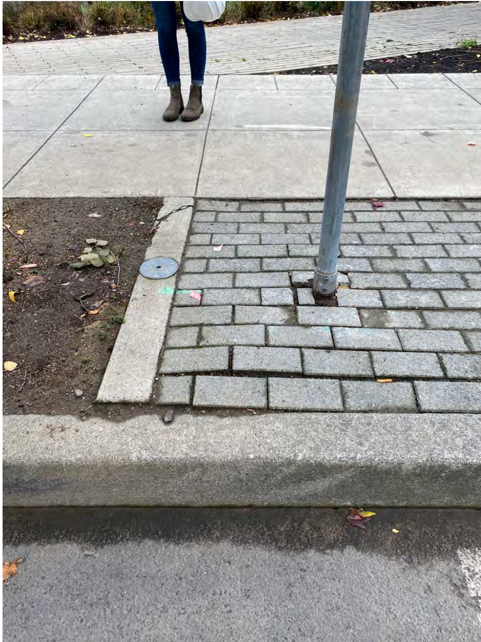
Photo Point 29 – uplift of bricks near tree well.
