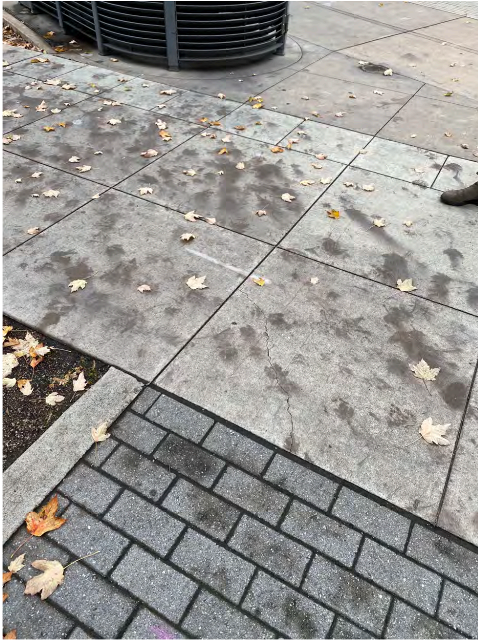
Photo Point 3 – Cracks in concrete panel near the Portland Loo
