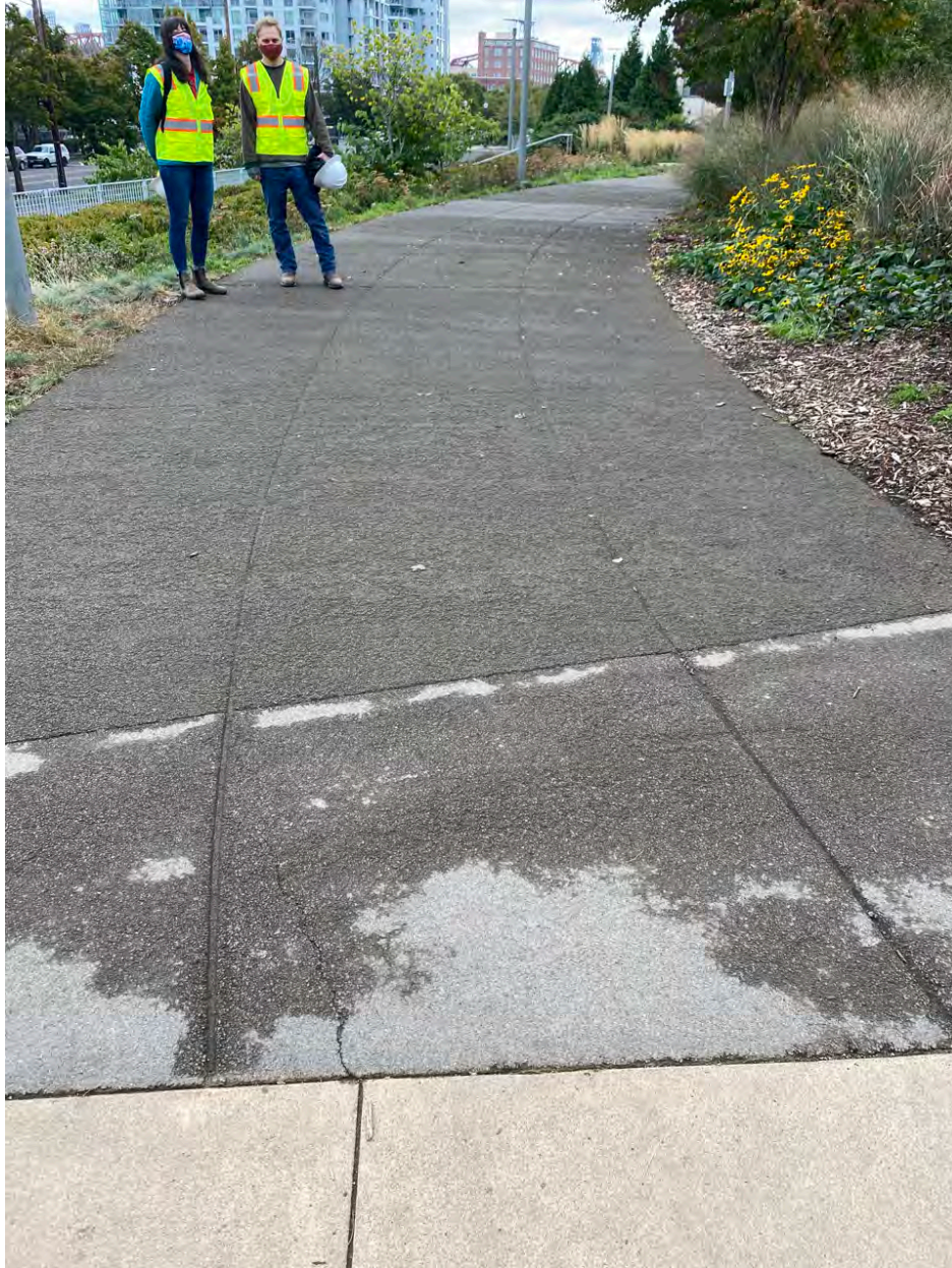
Photo Point 41 – minor cracks and weathering along path
