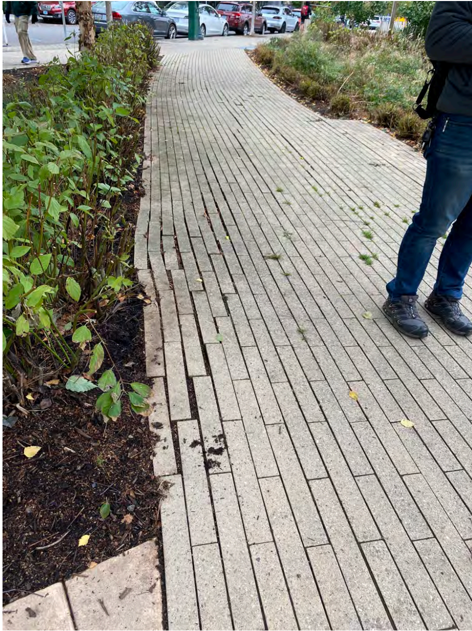
Photo Point 7 – Separation in bricks appears the same as last year's inspection.
