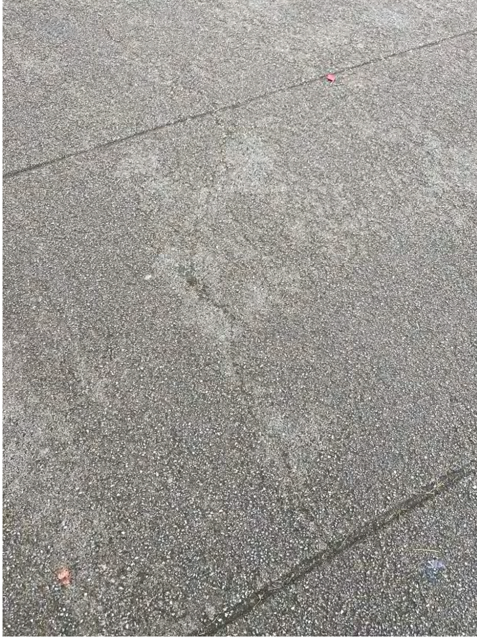
Photo Point 18 – Typical wear/weathering of asphalt path. No risk to cap.
