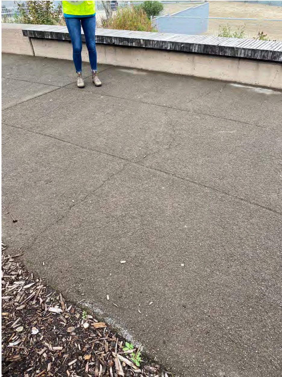
Photo Point 23 - crack in asphalt path. No risk to cap.
