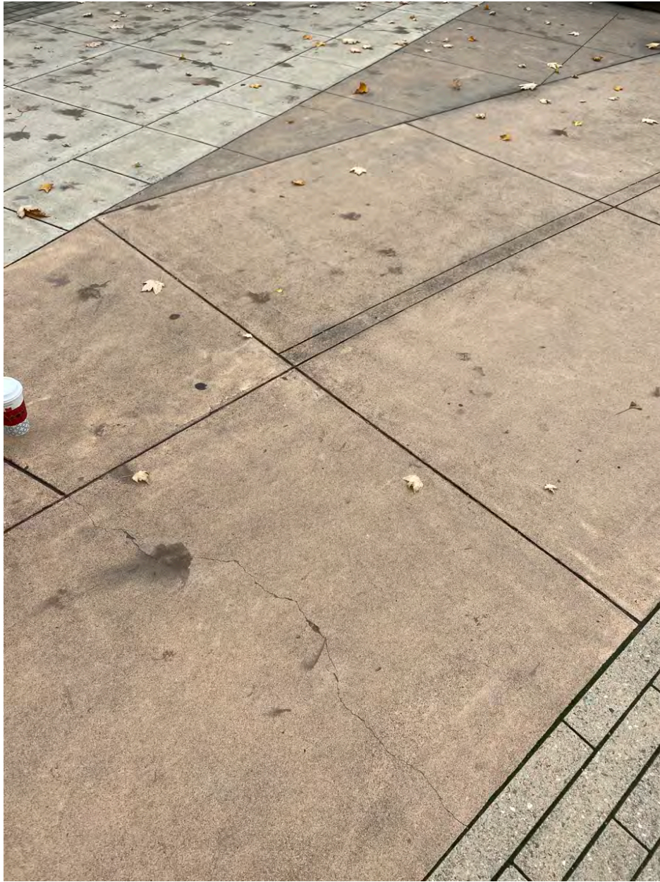
Photo Point 2 – hairline crack in concrete has not changed since last year
