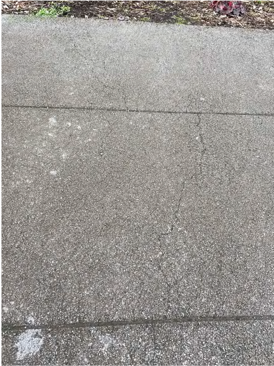
Photo Point 21 – minor cracks in pathway. Does not pose risk to cap.
