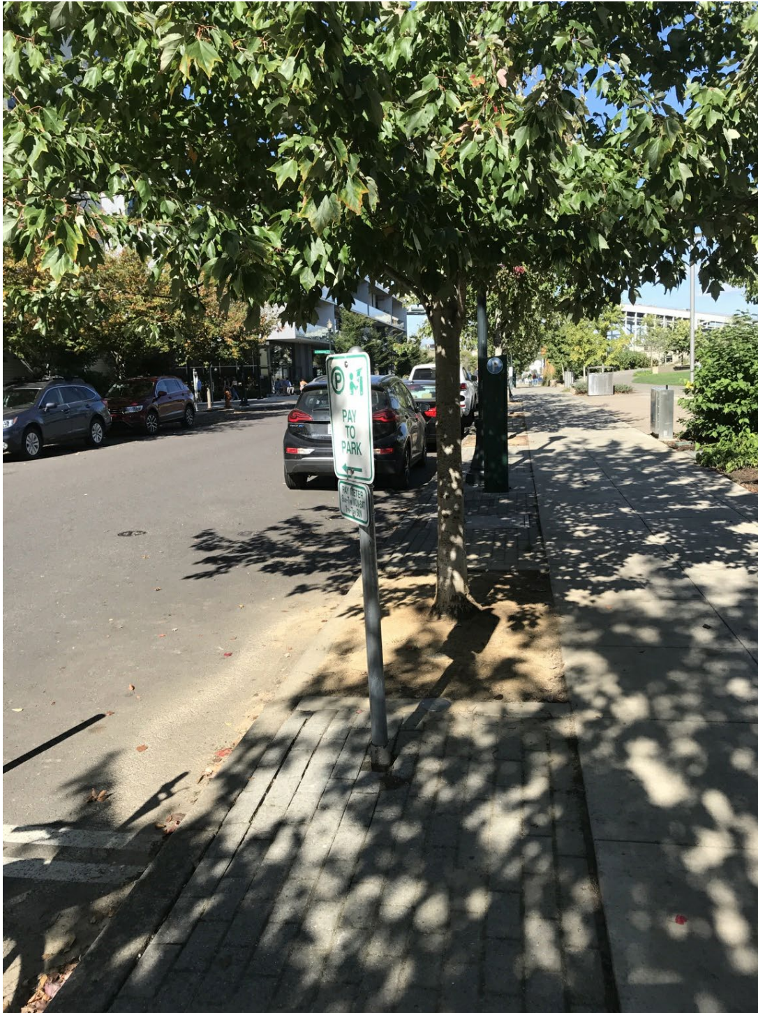
Photo Point 4 – Roots from street tree causing minor lifting of landscape bricks in planting strip. No evidence of subsurface soil or demarcation fabric making it to the surface.
