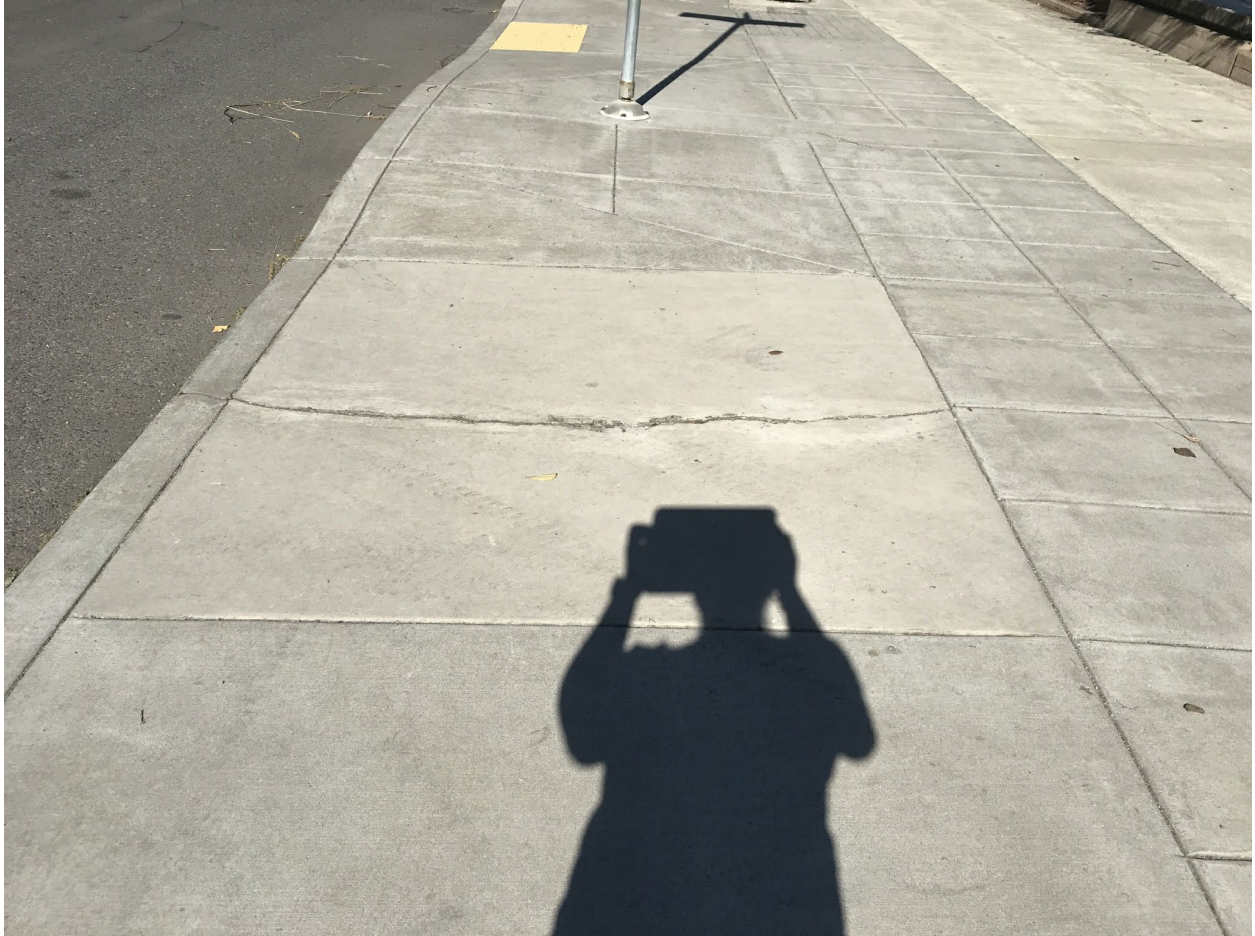
Photo Point 5 – Cracked Concrete Panel on NW 11 th Ave. It appears a patch was attempted but was unsuccessful. The crack itself has not grown since last inspection.
