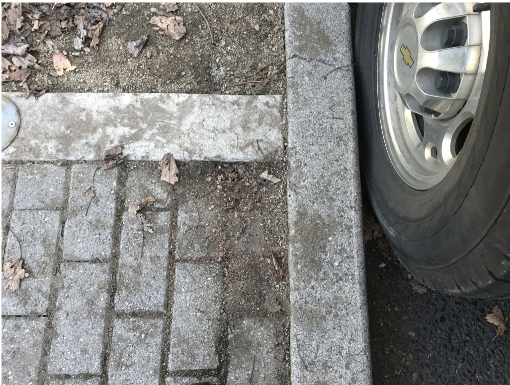
Photo Point 2 – evidence of concrete repair since 2019 inspection
