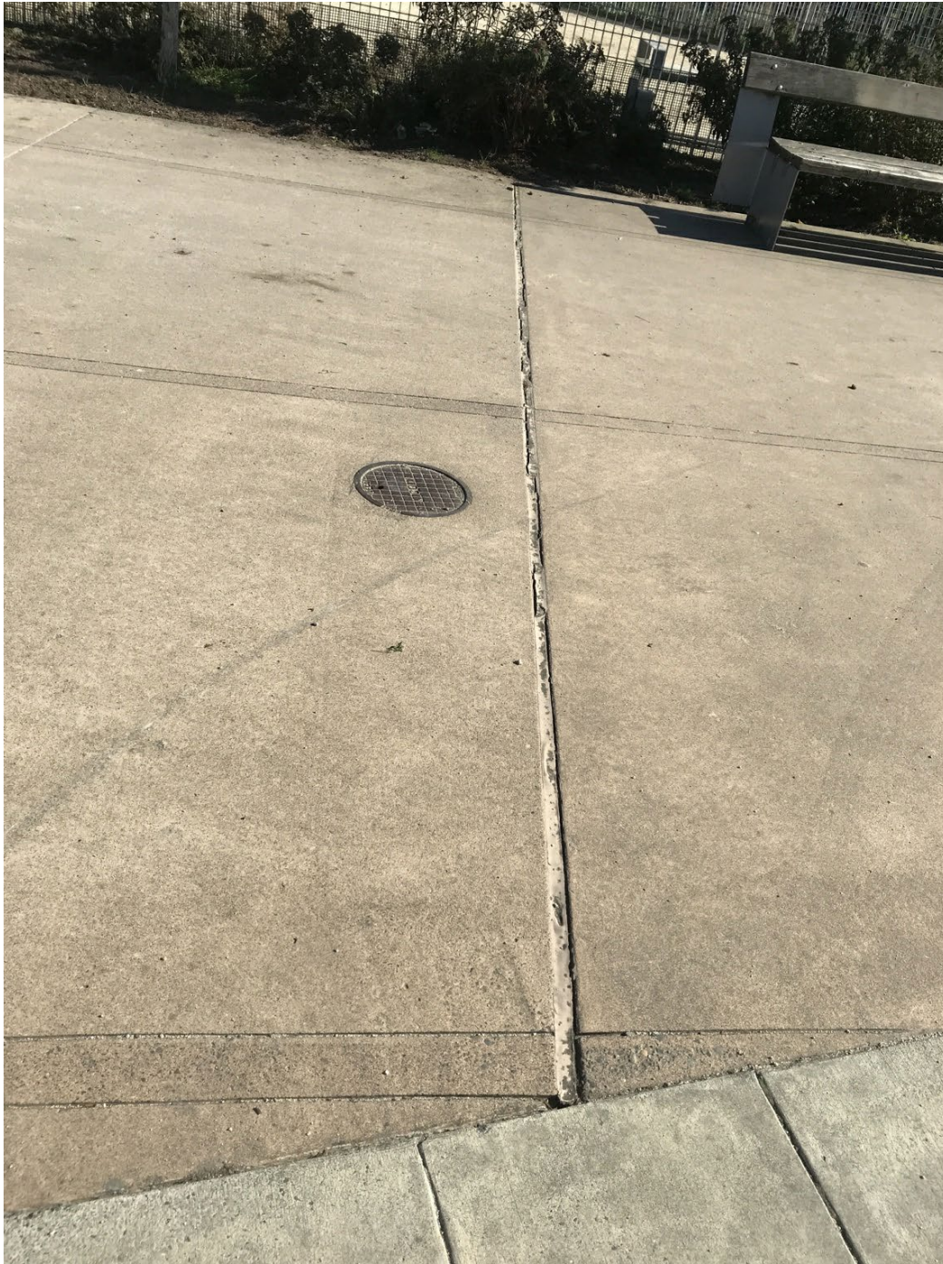
Photo Point 6 – Minor separation at caulked concrete paneling joint, no change from recent years.
