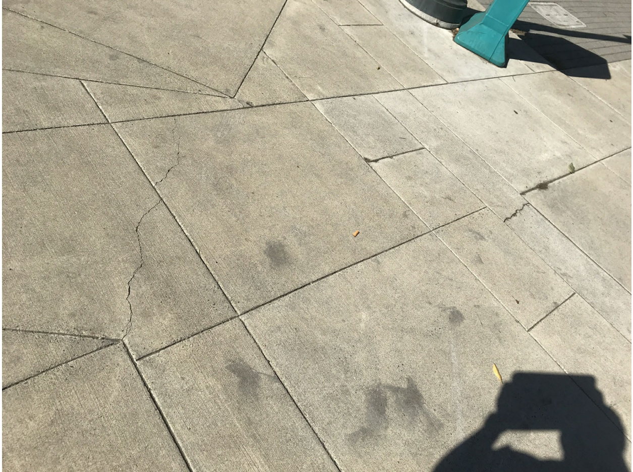
Photo Point 3 – cracks in concrete pavement has not changed since last year's inspection, indicating no new settling.
