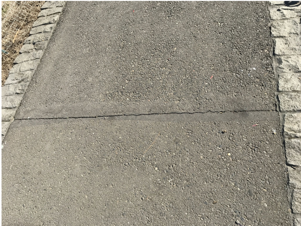
Photo Point 13 – Other crack in asphalt walkway has not changed over recent years.
