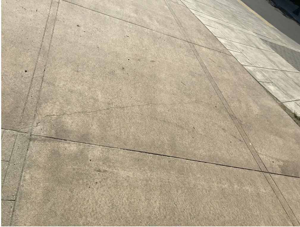
Photo Point 7 – Minor crack in concrete pavement has not changed since last year's inspection
