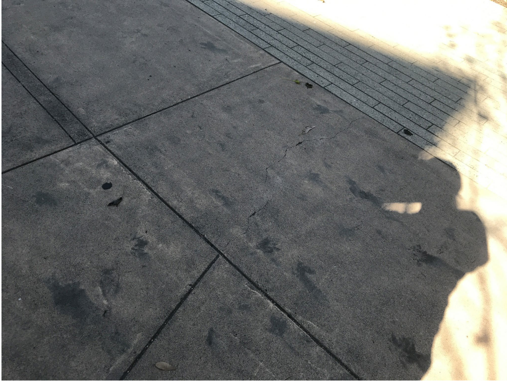
Photo Point 1 – minor cracks in concrete pavement. No change in size as compared to photos from previous inspections of recent years.
