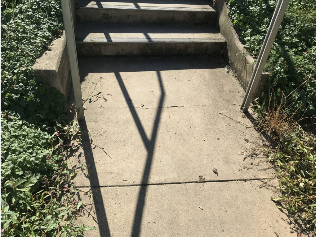
Photo Point 9 – crack at bottom of stairs has not changed in the past few years
