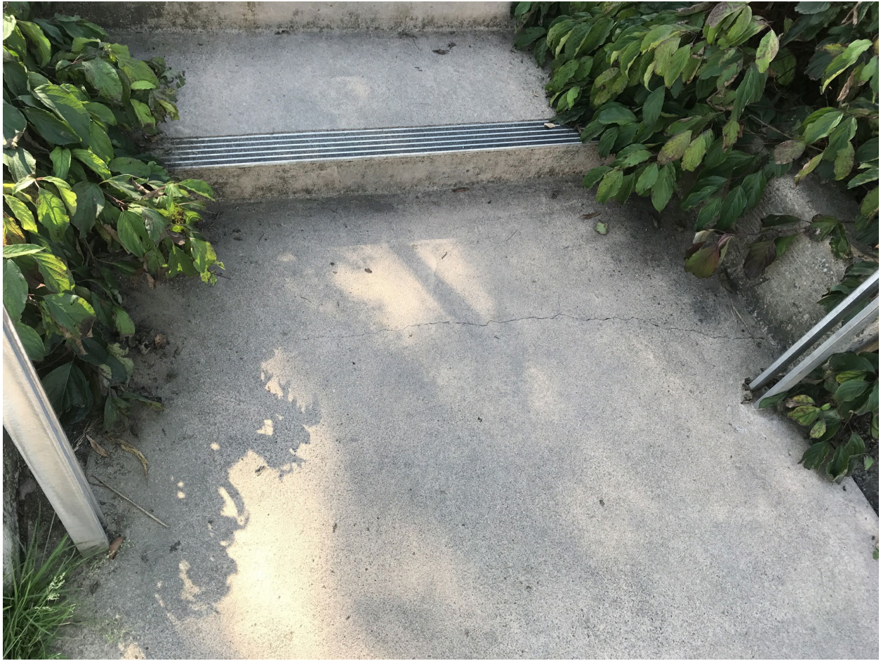
Photo Point 11 – Crack at bottom of stairs has not changed in past few years.
