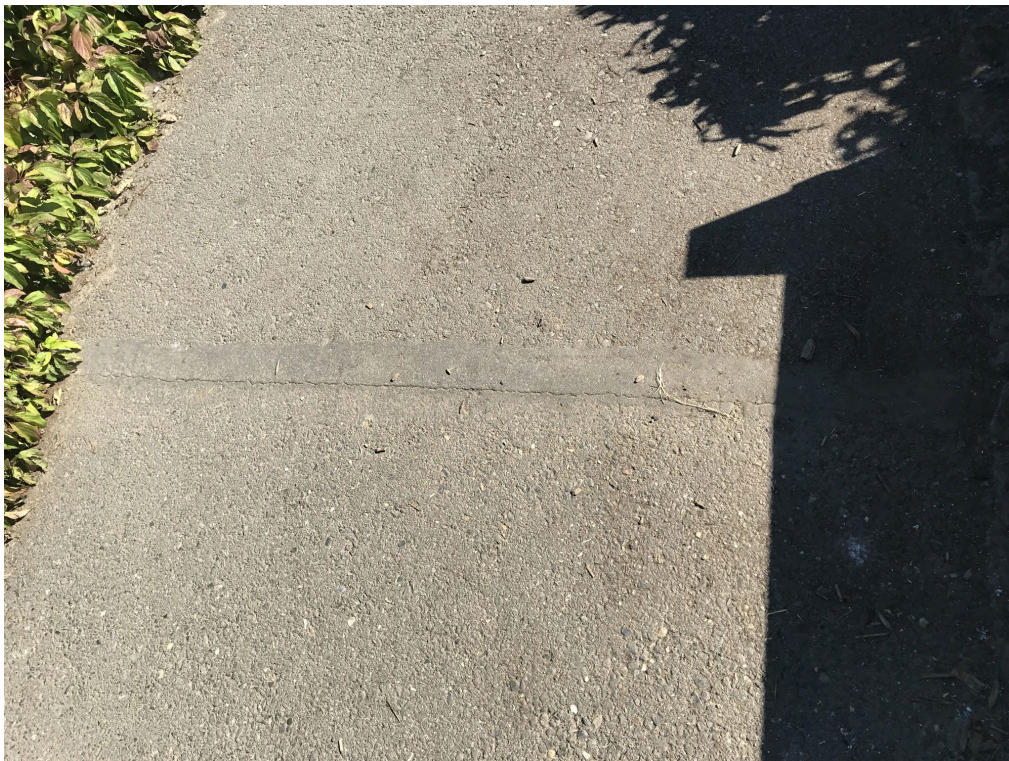
Photo Point 10 – Crack in asphalt walkway has not changed over recent years.
