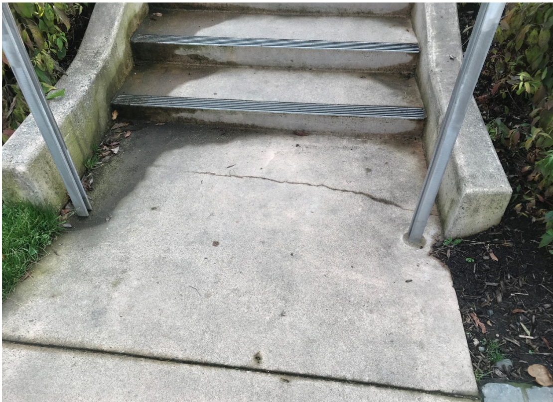
Photo 2: Minor crack in concrete at northern stairs
