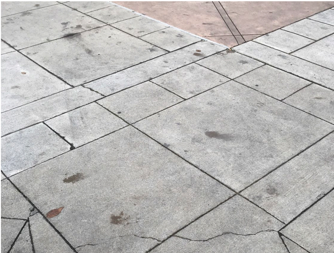
Photo 1: Minor cracks in concrete panels at NW Overton St and NW 11th Ave
