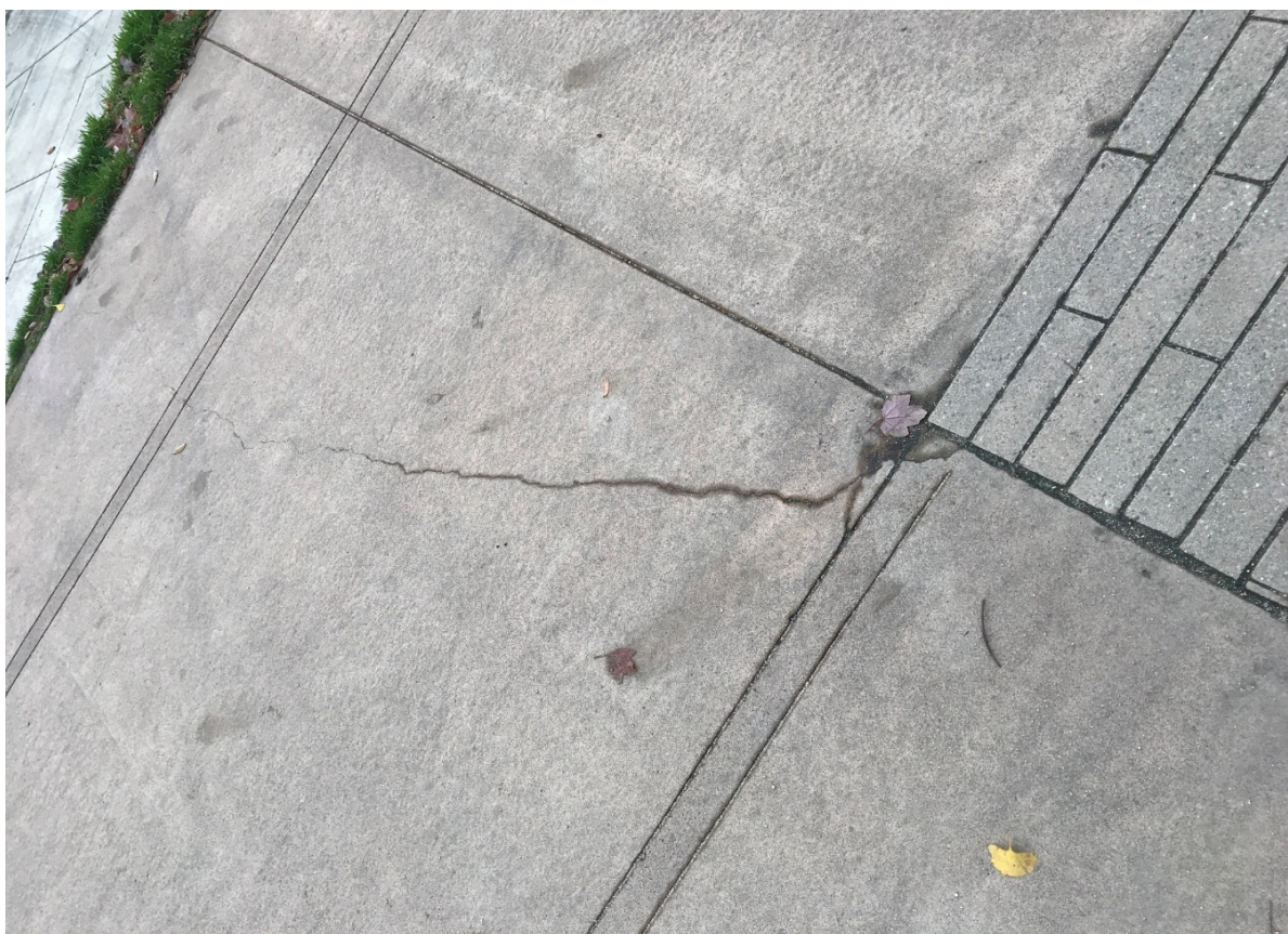
Photo 4: Minor crack in concrete panel
