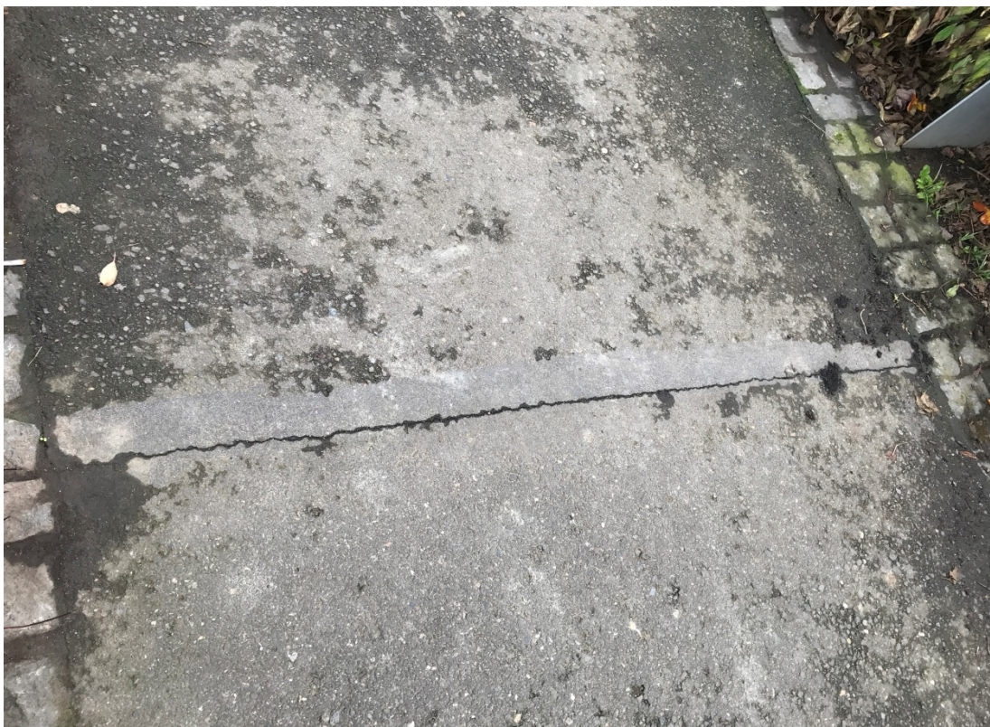
Photo 3: Crack in concrete path adjacent to rail line
