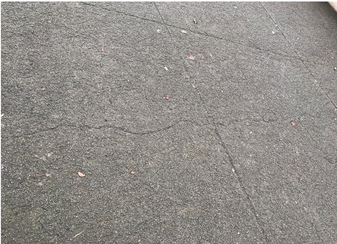
Photo 6: Surficial crack in concrete
