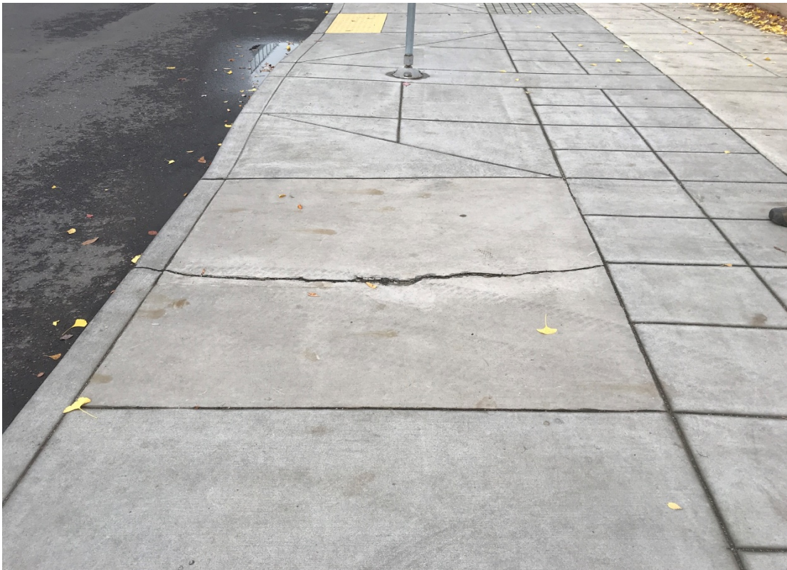
Photo 5: Cracked concrete panel on NW 11th Ave
