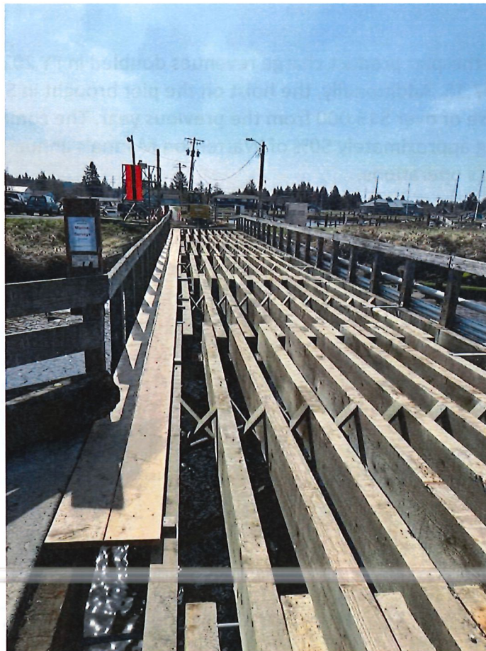
Commercial Work Pier West Trestle under construction
