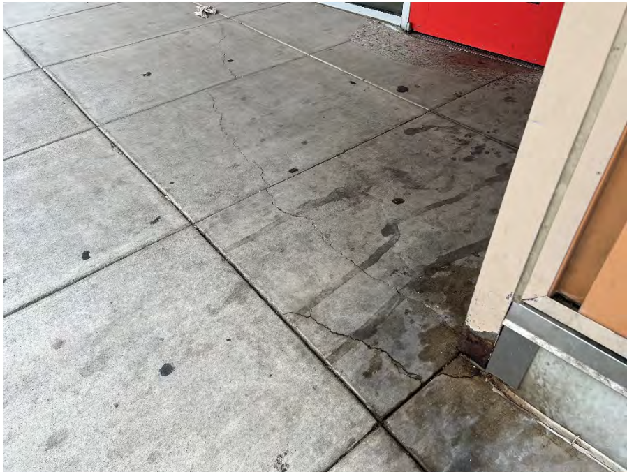
MINOR CRACKS ON THE EXTERIOR SIDEWALK ALONG THE WEST EXTERIOR OF THE SUBJECT PROPERTY STRUCTURE. PHOTOGRAPH TAKEN FACING NORTHEAST.
