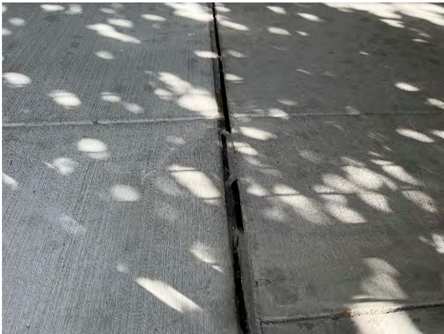
MINOR SEPARATION IN AN EXTERIOR SIDEWALK ON THE SOUTHWEST PORTION OF THE SUBJECT PROPERTY STRUCTURE. PHOTOGRAPH TAKEN FACING NORTH.
