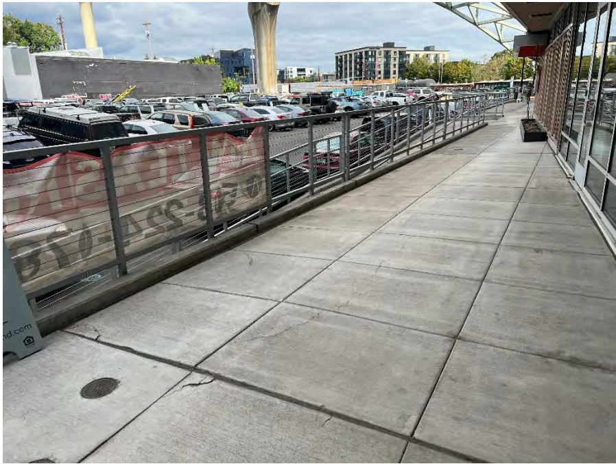
EXTERIOR SIDEWALK ON THE SOUTHWEST PORTION OF THE SUBJECT PROPERTY STRUCTURE, WITH SOME MINOR CRACKS. PHOTOGRAPH TAKEN FACING NORTHWEST.
