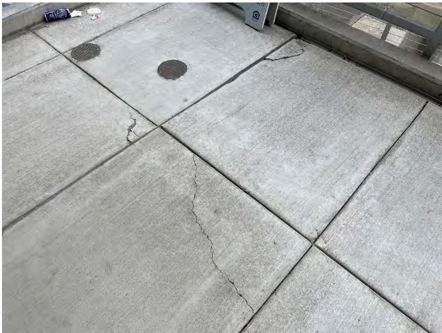
MINOR CRACKS ON THE EXTERIOR SIDEWALK ON THE SOUTHWEST PORTION OF THE SUBJECT PROPERTY STRUCTURE. PHOTOGRAPH TAKEN FACING SOUTHWEST.
