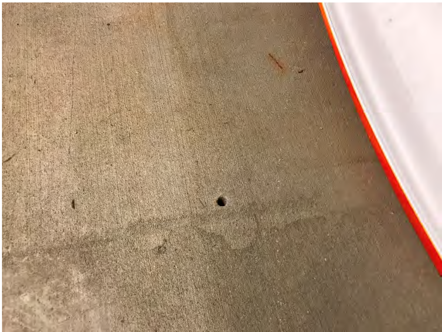
SMALL, APPROXIMATELY 2- TO 3-INCH-DEEP HOLE IN CONCRETE FLOOR SLAB. HOLE DID NOT PENETRATE THE FLOOR SLAB.
