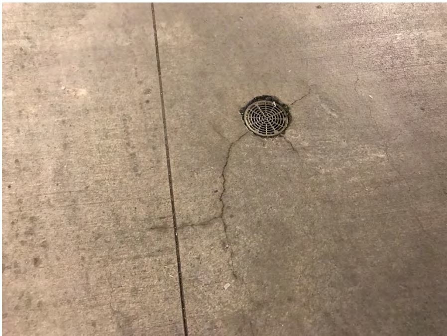
MINOR CRACK AROUND FLOOR DRAIN IN SUBSURFACE PARKING LEVEL
