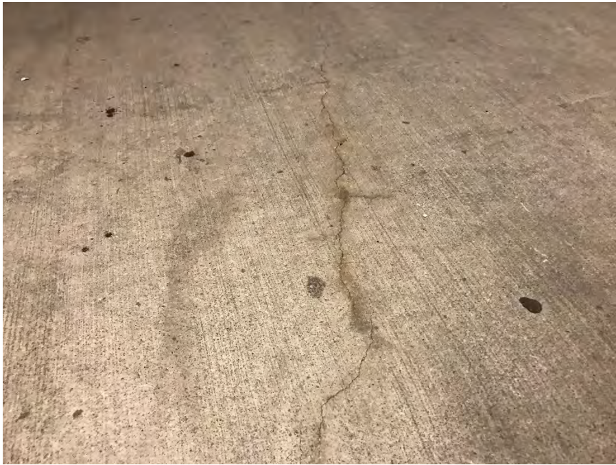
MINOR CRACK IN CONCRETE FLOOR SLAB
