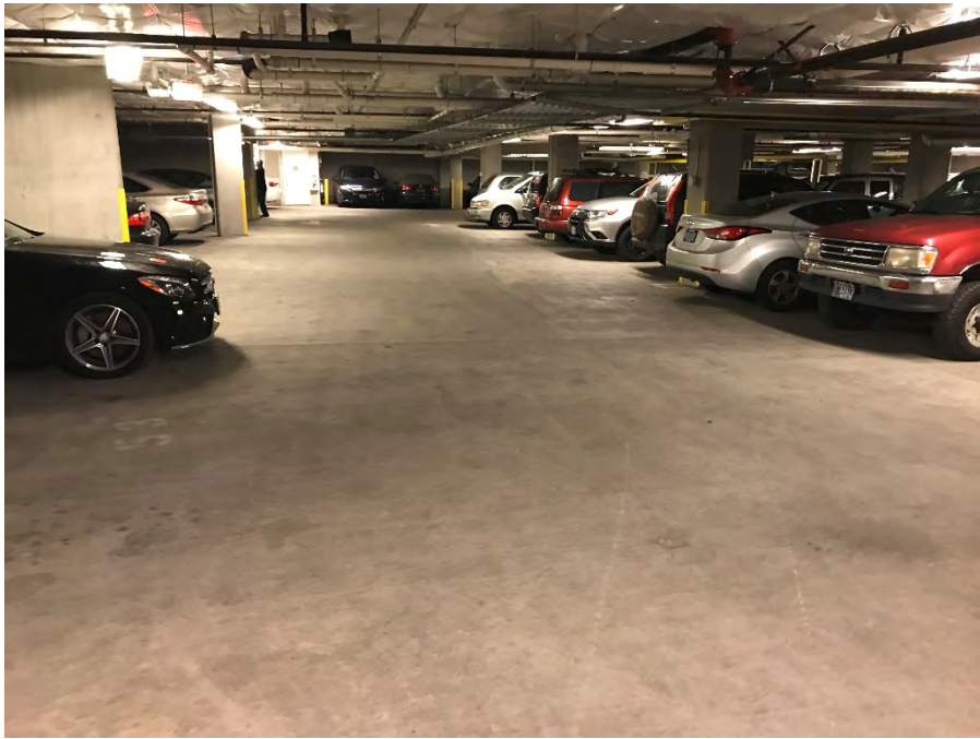
CAP CONSISTING OF CONCRETE FLOOR SLAB IN SUBSURFACE PARKING LEVEL
