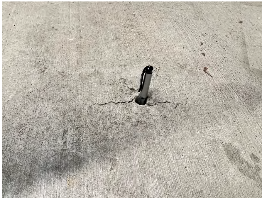
CLOSE-UP OF HOLE OBSERVED IN CONCRETE IN EAST PORTION OF GARAGE ROOM P04A.
