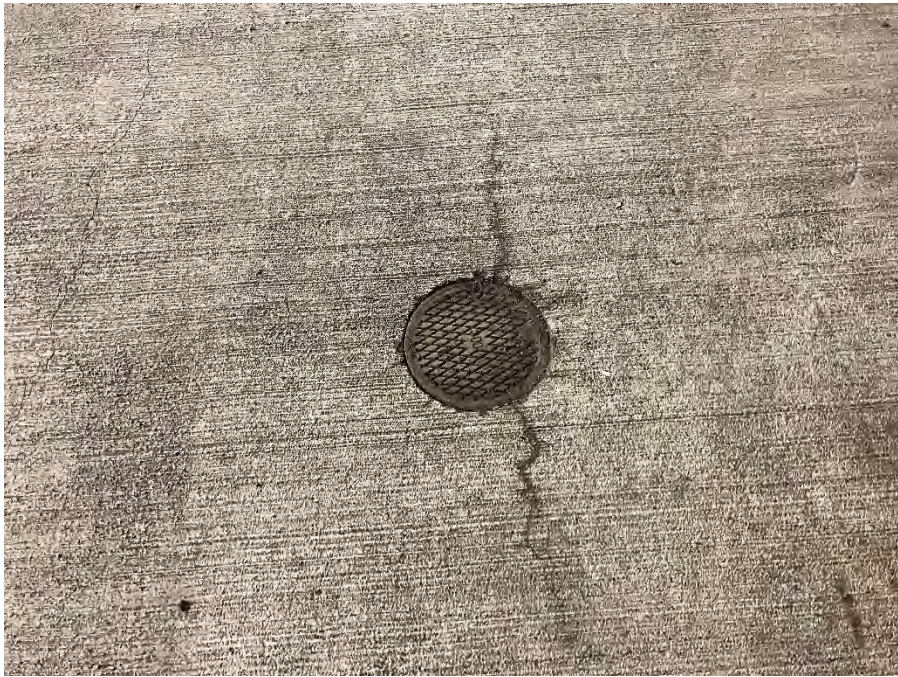
MINOR CRACK AROUND UTILITY COVER IN SUBSURFACE PARKING LEVEL.
