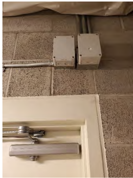
CH4 sensor and relay box
