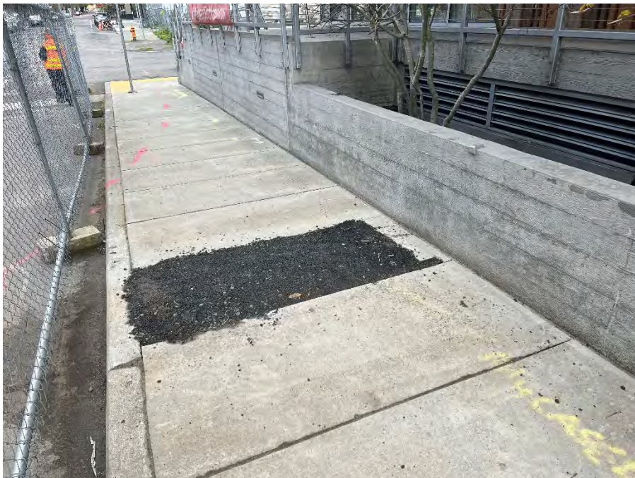
ASPHALT PATCH IN SIDEWALK ALONG BUILDING EXTERIOR.
