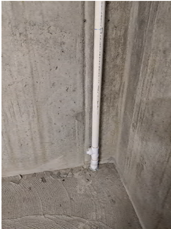
SLAB PENETRATION IN THE PARKING GARAGE SEALED TO THE CONCRETE SLAB WITH CAULKING. PHOTOGRAPH TAKEN FACING NORTH.
