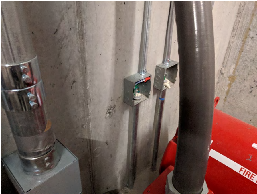
CONDUITS SEALED USING CLOSED CELL POLYURETHANE SPRAY FOAM. PHOTOGRAPH TAKEN FACING NORTHWEST.
