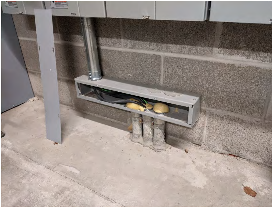
CONDUITS SEALED USING CLOSED CELL POLYURETHANE SPRAY FOAM. PHOTOGRAPH TAKEN FACING NORTHWEST.
