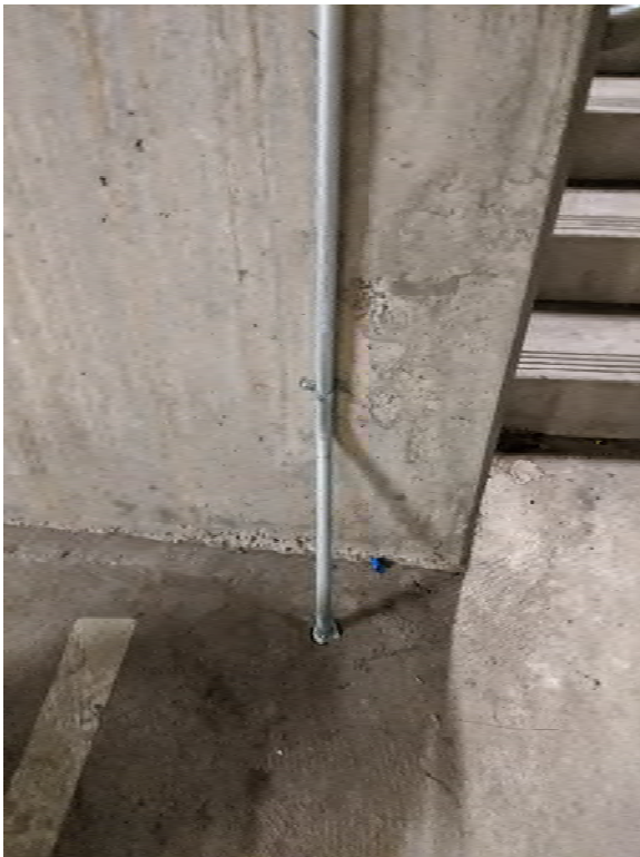
SLAB PENETRATION IN THE PARKING GARAGE SEALED TO THE CONCRETE SLAB WITH CAULKING. PHOTOGRAPH TAKEN FACING WEST.
