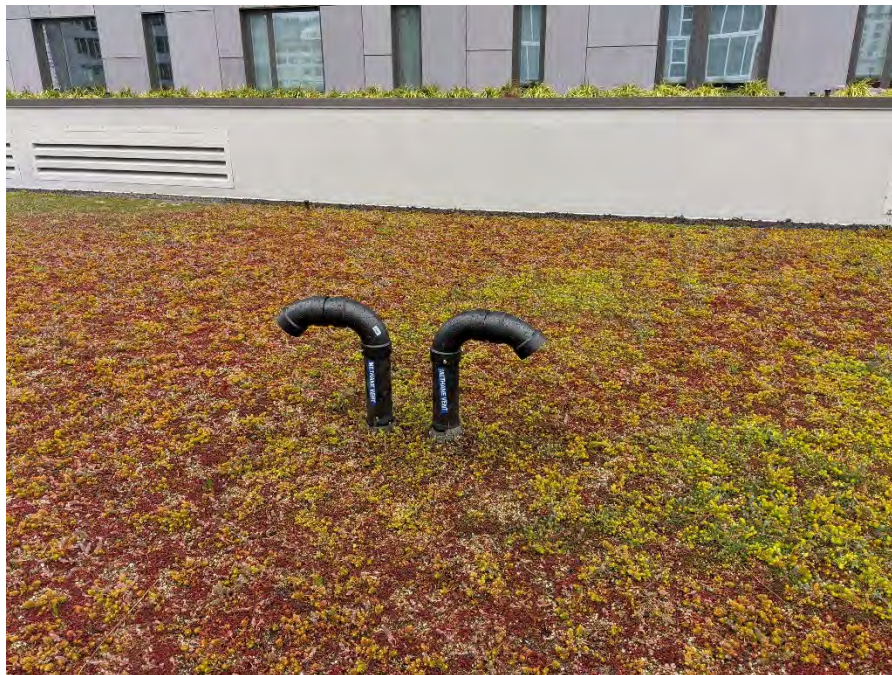
SUB-SLAB VENTILATION SYSTEM ROOF VENTS WITH RAIN GUARDS AND PLACARDS. PHOTOGRAPH TAKEN FACING NORTH.
