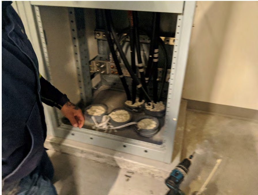
PGE CONDUITS SEALED USING CLOSED CELL POLYURETHANE SPRAY FOAM. PHOTOGRAPH TAKEN FACING WEST.
