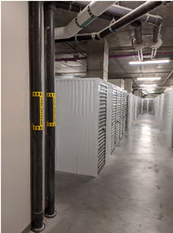
METHANE VENT RISERS WITH PLACARDS AT THE 5 TH FLOOR STORAGE UNIT SPACE. PHOTOGRAPH TAKEN FACING EAST.
