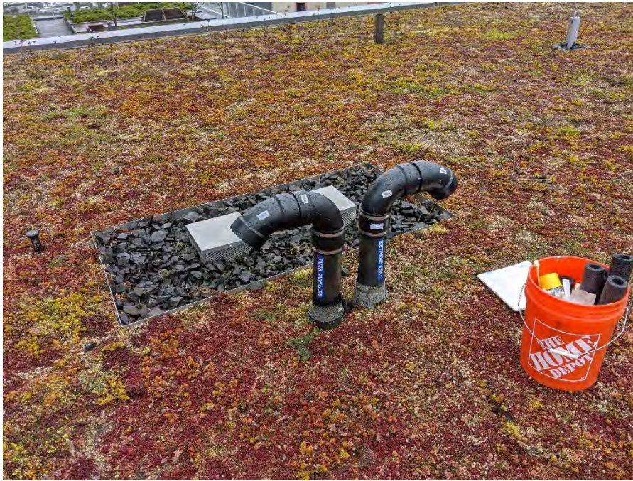
SUB-SLAB VENTILATION SYSTEM ROOF VENTS WITH RAIN GUARDS AND PLACARDS. PHOTOGRAPH TAKEN FACING NORTH.
