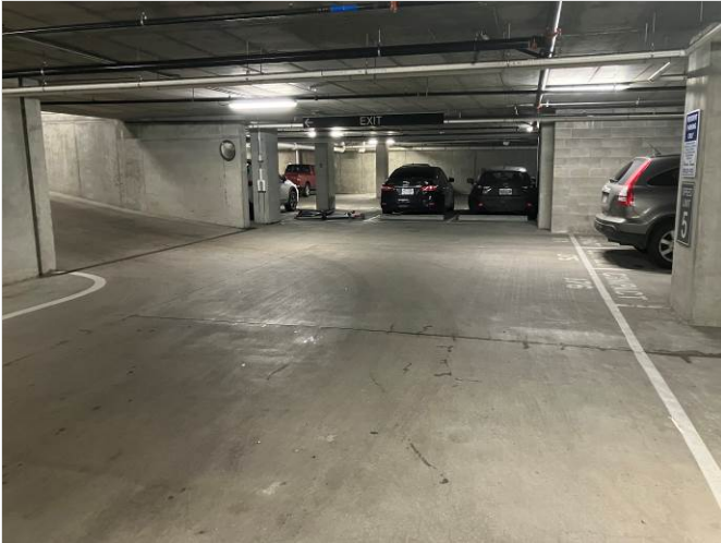
13. Parking garage/foundation view.
