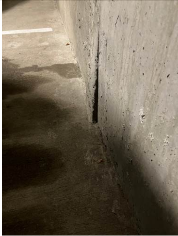
7. Parking garage wall – parking space 110.
