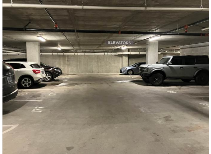
14. Parking garage/foundation view.
