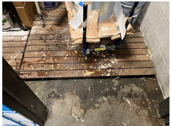
12. Paint storage room.
