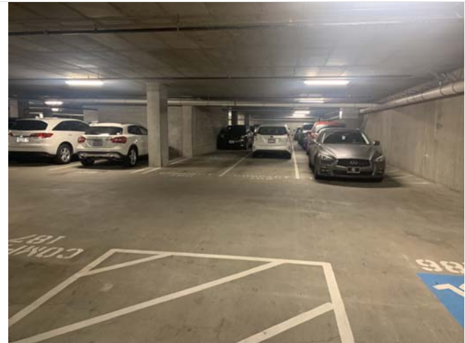
4. Parking garage/building foundation view B
