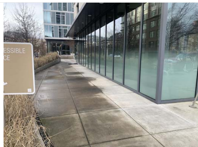
17. Hardscape along NW Overton St.
