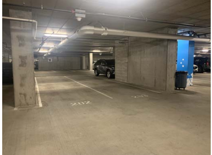
8. Parking garage/building foundation view D
